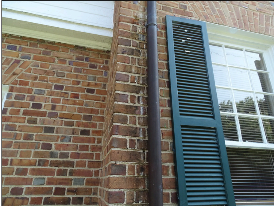
31 - Stained wall on south side of building
