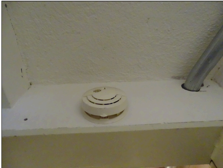
54 - Typical smoke detector
