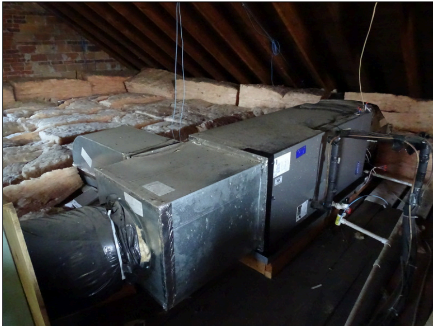
44 - Carrier air Handler unit located in attic
