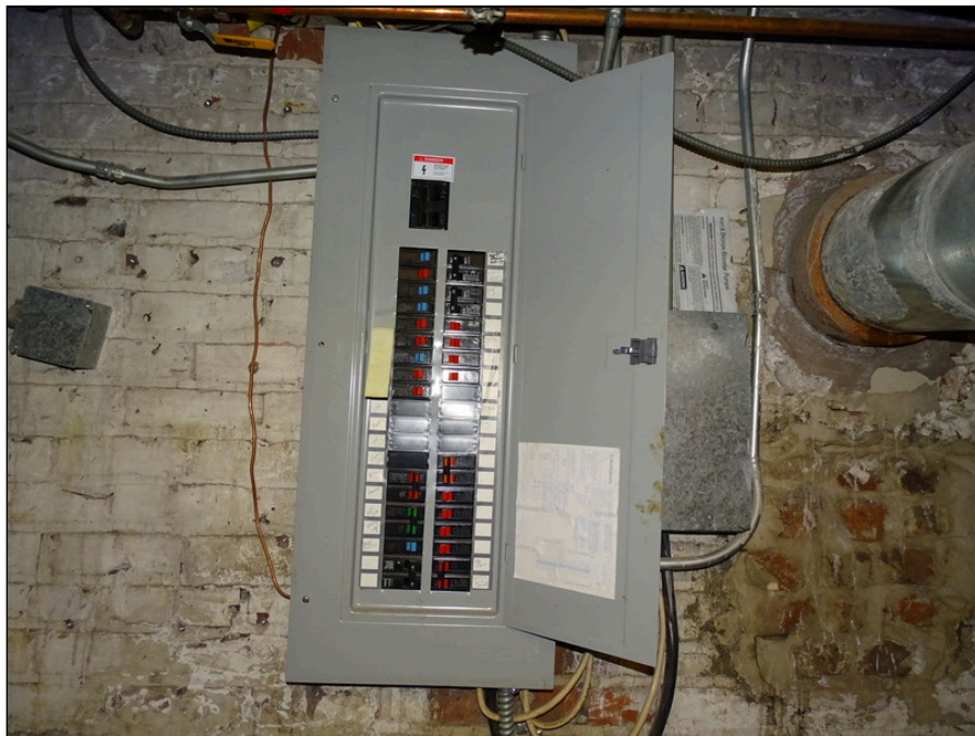
52 - Typical circuit breaker panel
