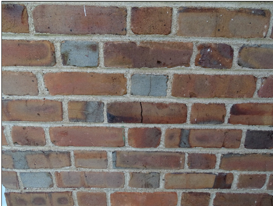
30 - Step cracked on brick wall north
