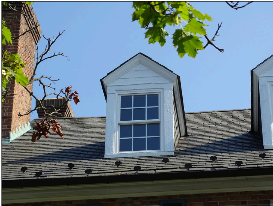
40 - Slate shingle roofing system - note deterioration
