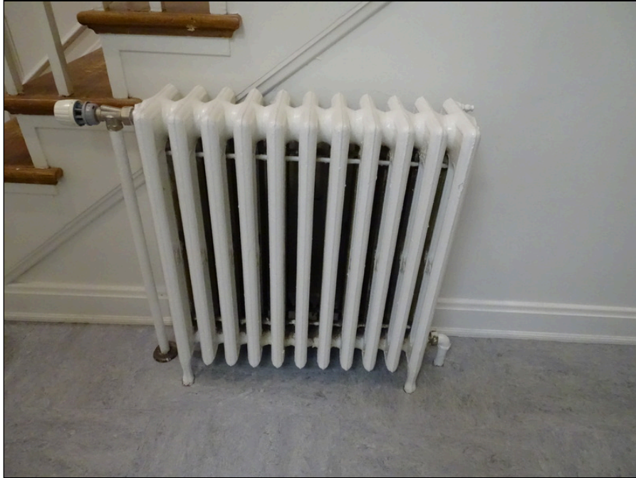
45 - Typical radiator unit with manual control
