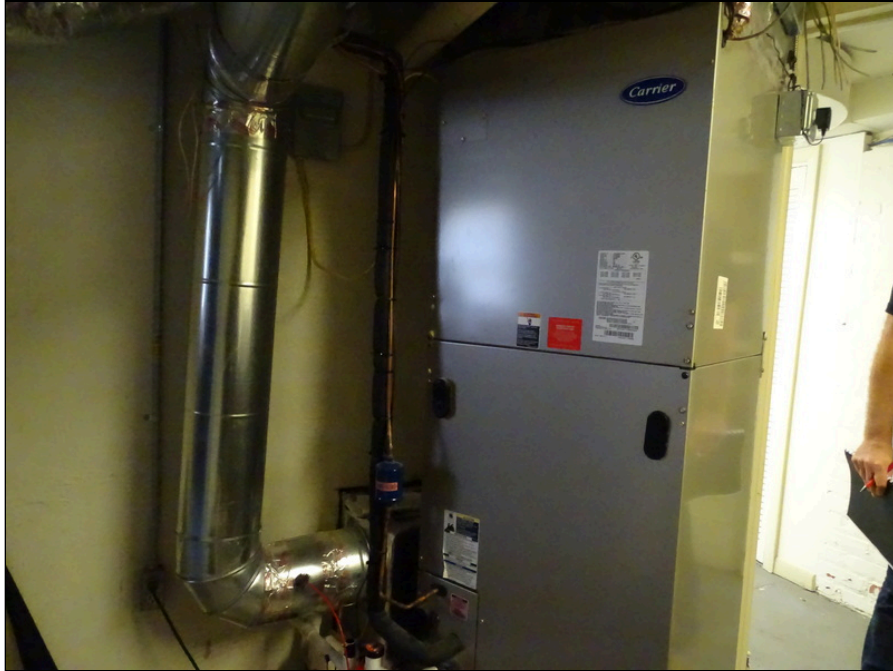
43 - Air Handler unit located in basement
