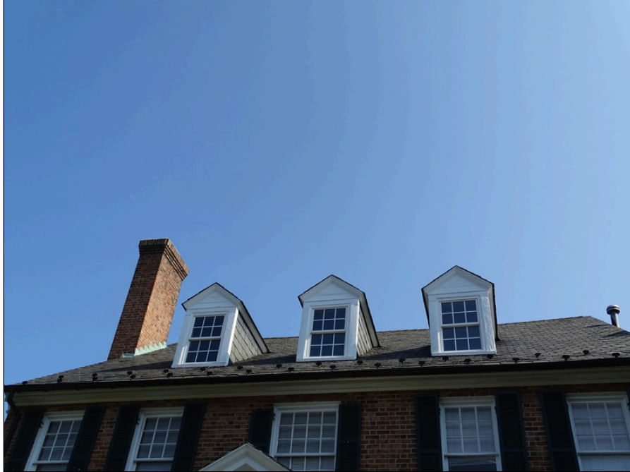
39 - Slate shingle roofing system
