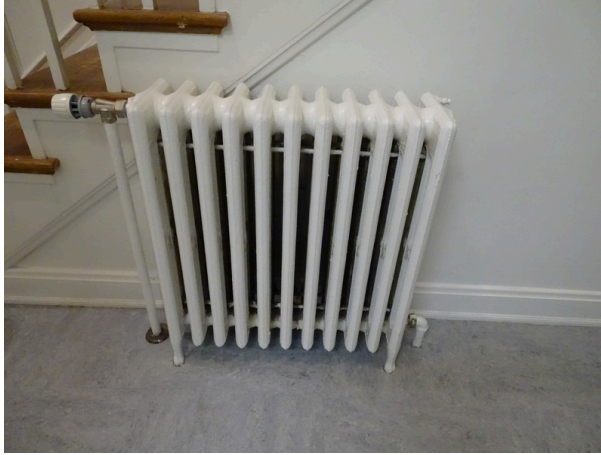
Typical radiator unit with manual control
