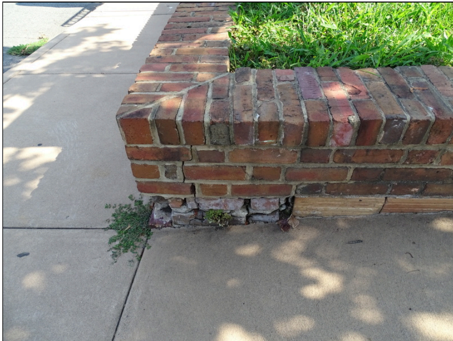
10 - Retaining wall condition on south west corner of the building
