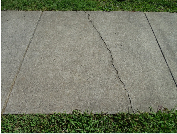
Concrete sidewalk overview - note cracking
