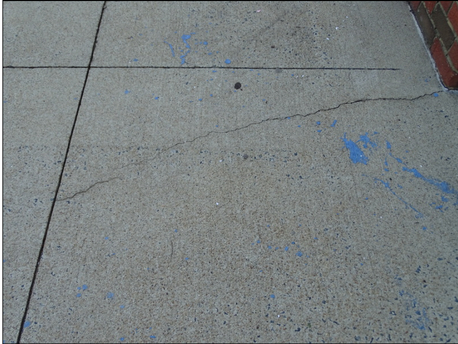
9 - Concrete sidewalk overview - note cracking
