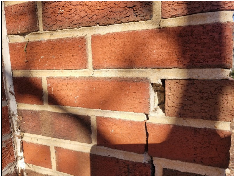
110 - Bath house brick crack
