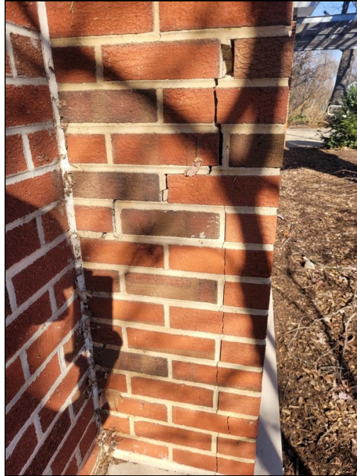
111 - Bath house brick crack
