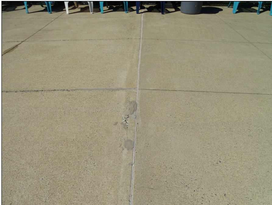
16 - Concrete pavement overview - note sealant condition
