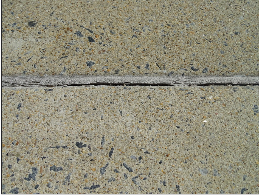
17 - Concrete pavement overview - note sealant condition
