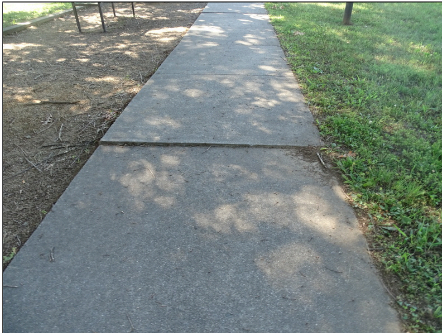
6 - Concrete sidewalk - note tripping hazard
