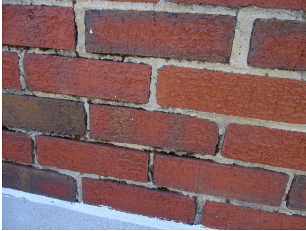
Bath house exterior - note mortar deterioration
