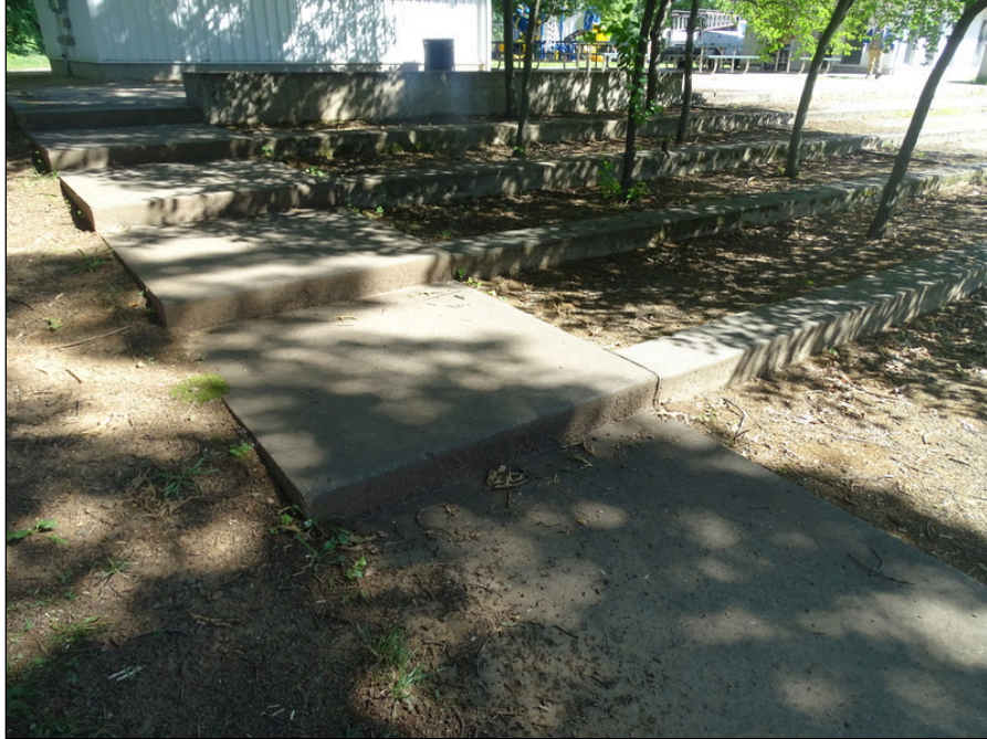
13 - Typical steps - note handrail missing
