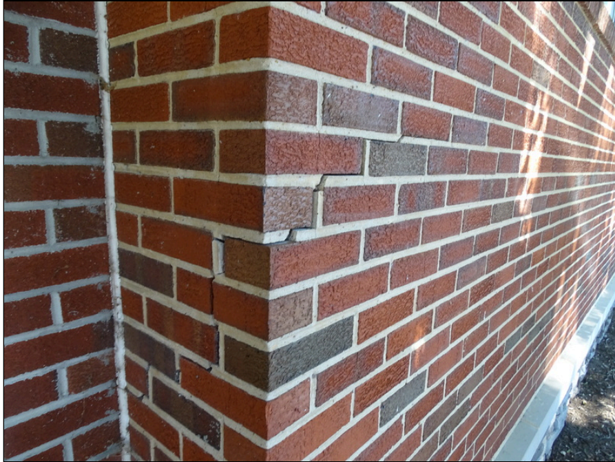
43 - Bath house exterior - note step cracking
