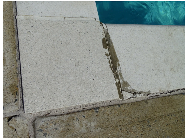
Concrete pavement overview - note sealant condition
