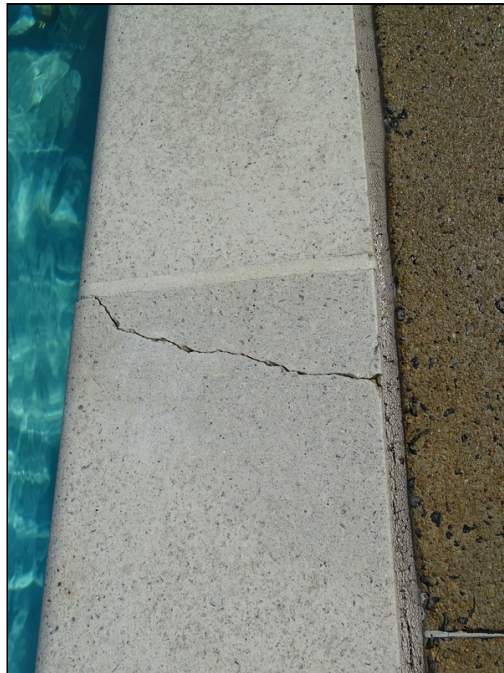
18 - Cracked concrete coping of pool
