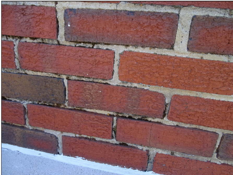
46 - Bath house exterior - note mortar deterioration
