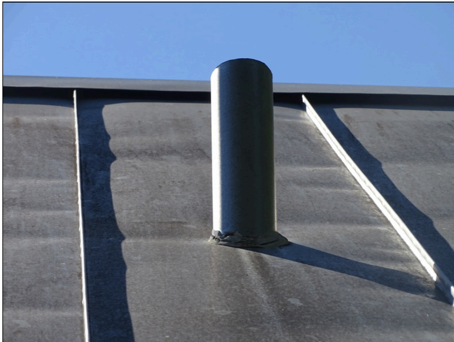
58 - Plumbing Penetration at Bath house roof
