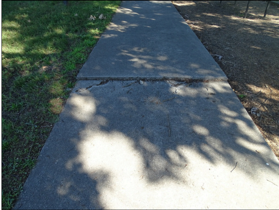
5 - Concrete sidewalk - note tripping hazard
