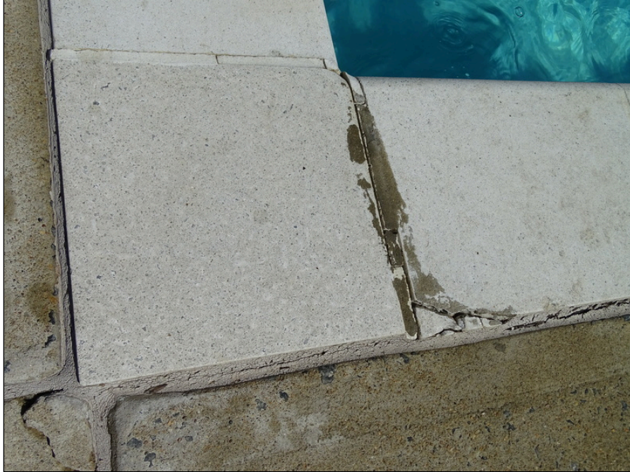
19 - Concrete pavement overview - note sealant condition
