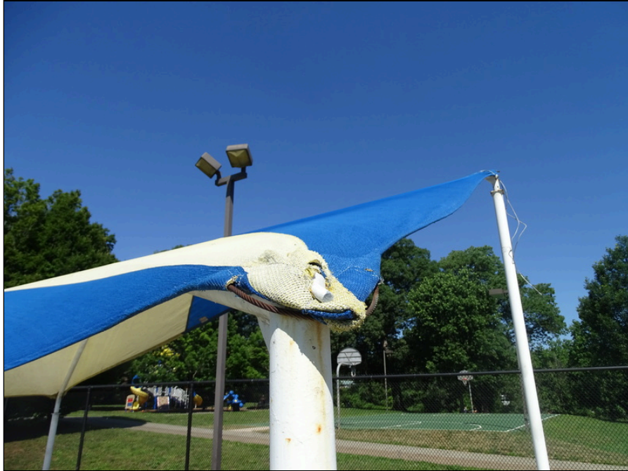
23 - Pool rest area tent overview - note deterioration
