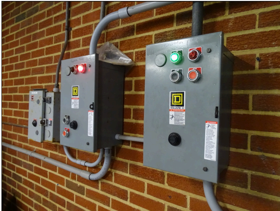
74 - Electrical emergency switch
