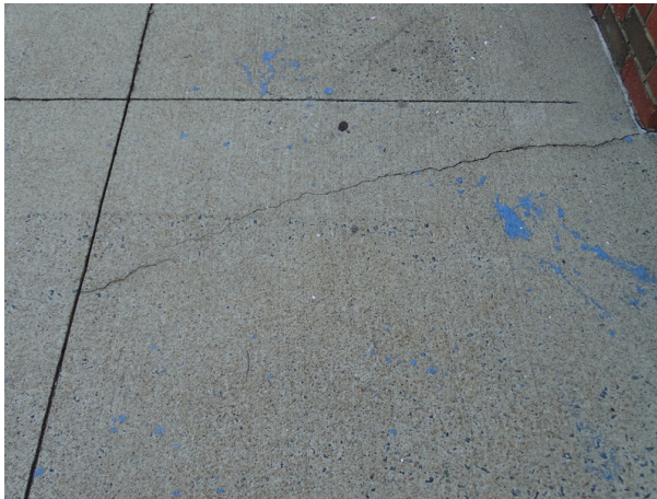
Concrete sidewalk overview - note cracking
