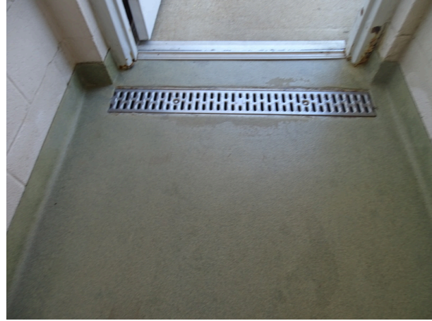
Bath house family restroom drainage - note wear
