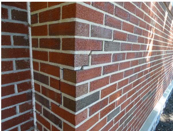
Bath house exterior - note step cracking
