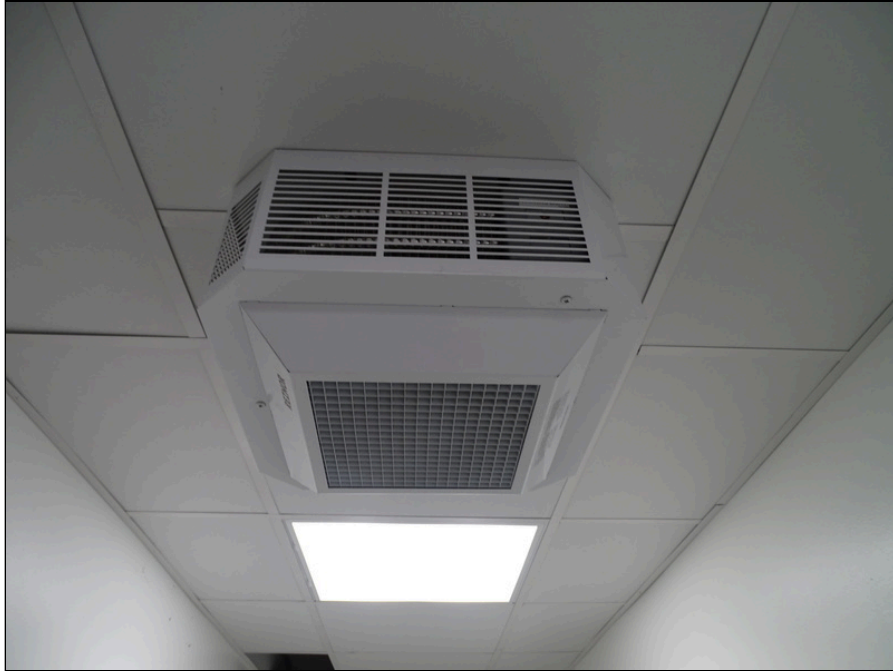
67 - HVAC unit in the Shelter
