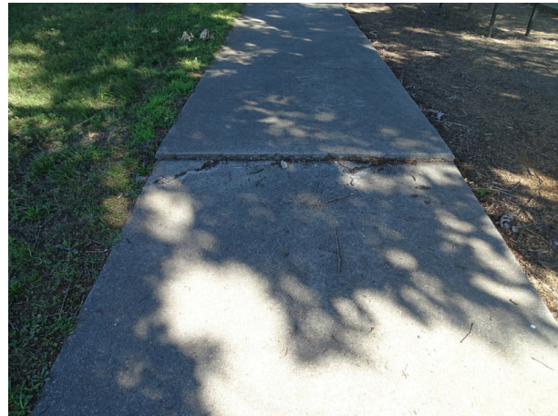
Concrete sidewalk - note tripping hazard
