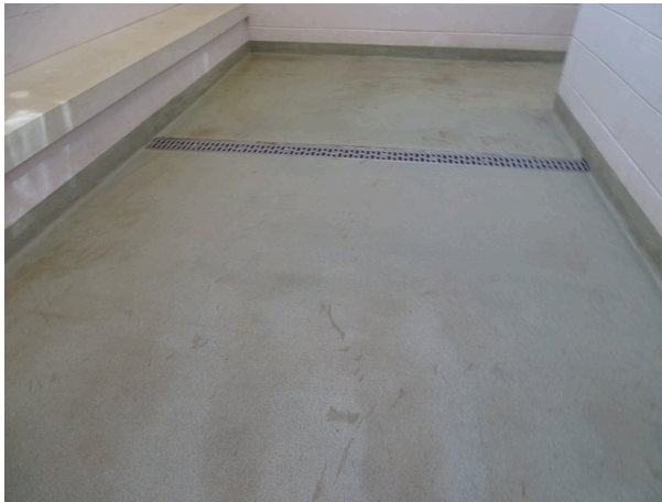
Bath house family restroom floor - note deterioration
