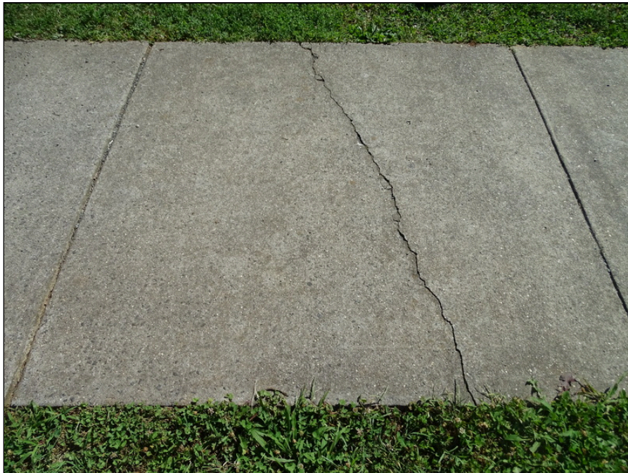
10 - Concrete sidewalk overview - note cracking
