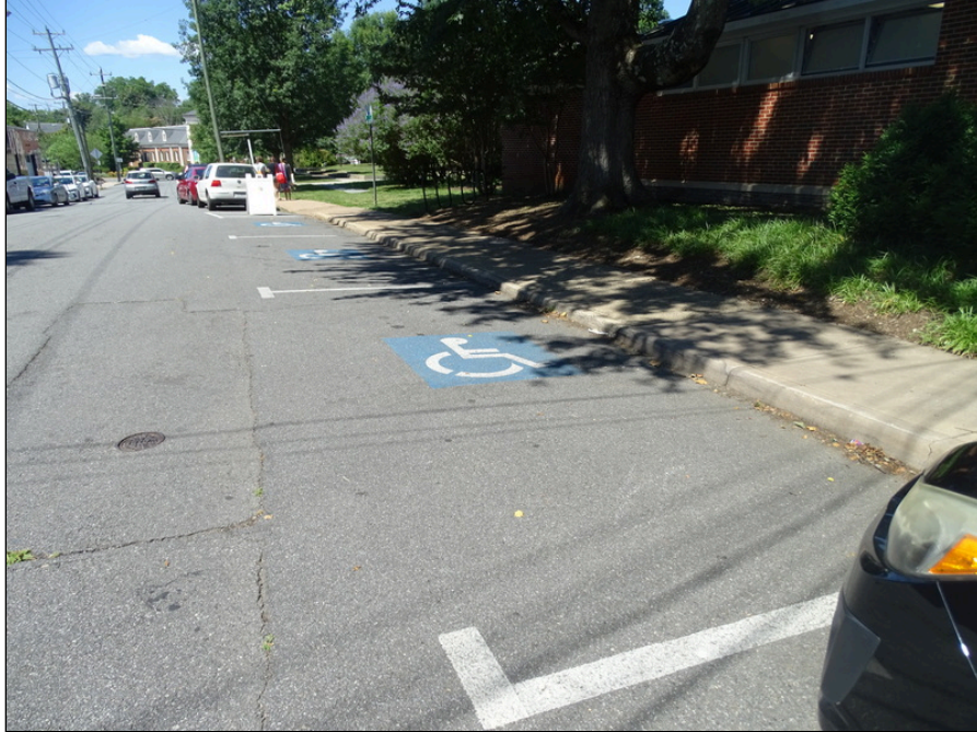
101 - Non-compliant accessible parking
