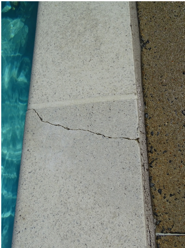
Cracked concrete coping of pool
