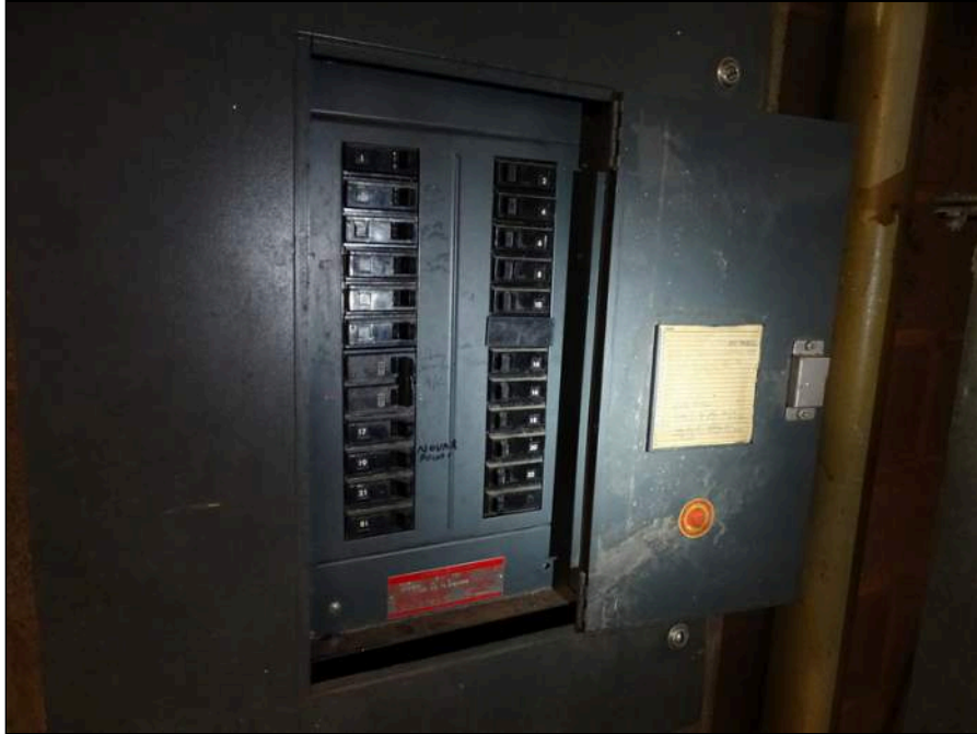
77 - Typical older circuit breaker panel
