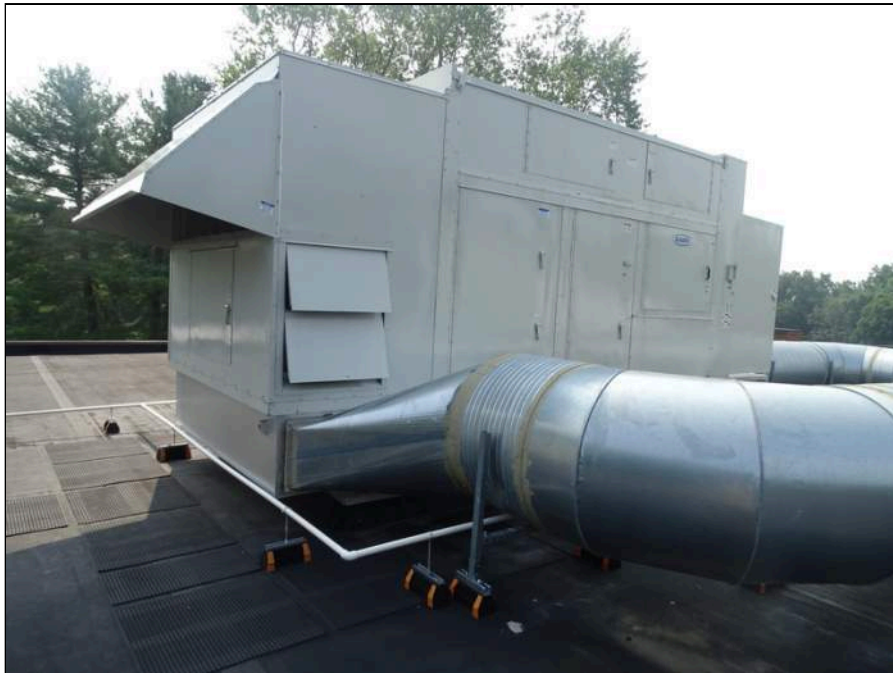
62 - Typical Make Up Air Unit located on roof
