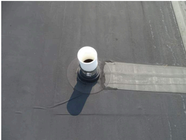
Typical plumbing penetration
