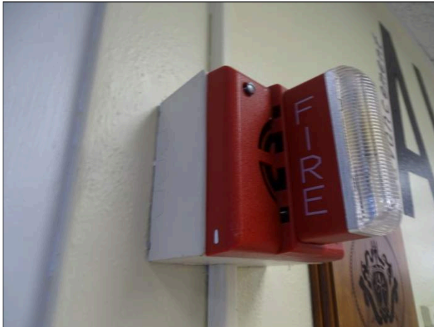
86 - Typical fire alarm bell and strobe
