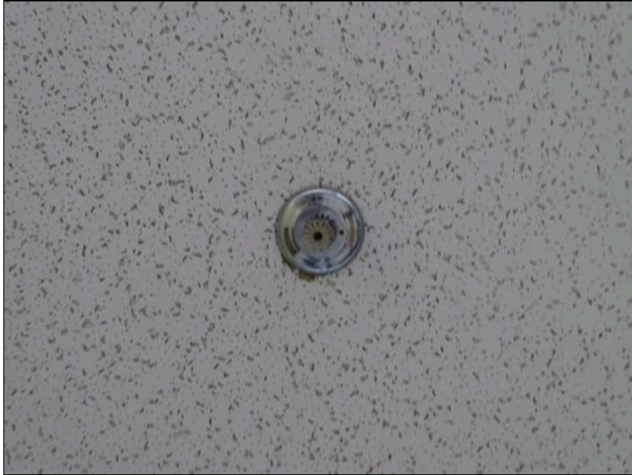
81 - Typical fire sprinkler head
