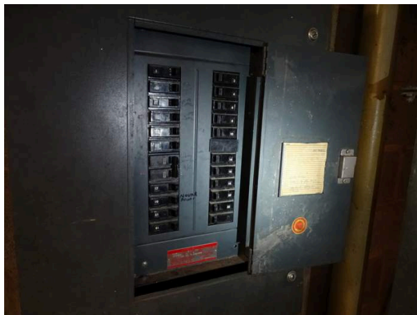
Typical older circuit breaker panel
