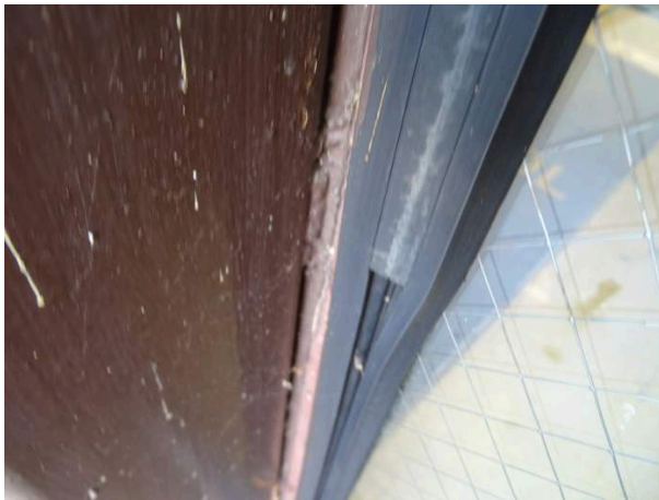
Typical exterior windows - note deterioration
