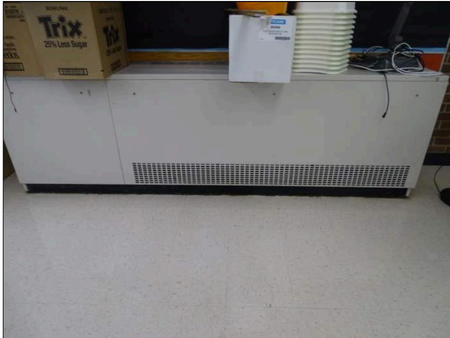
63 - Typical water source heat pump
