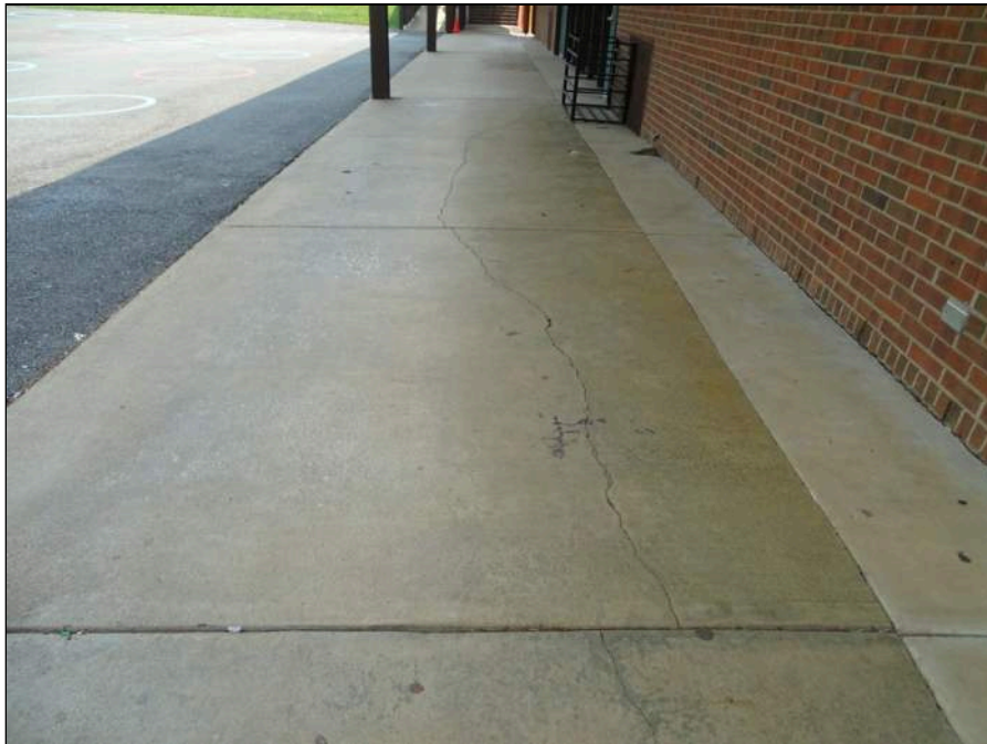
10 - Concrete sidewalk - note deterioration
