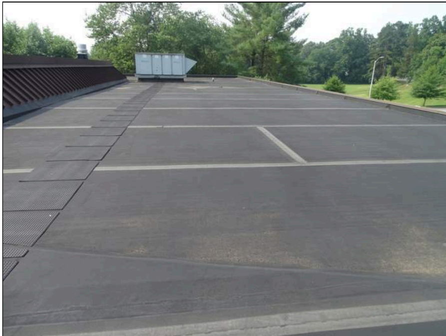
50 - Single-ply membrane roofing system main building looking north
