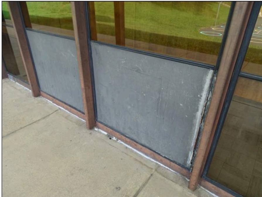
46 - Typical exterior windows - note deterioration
