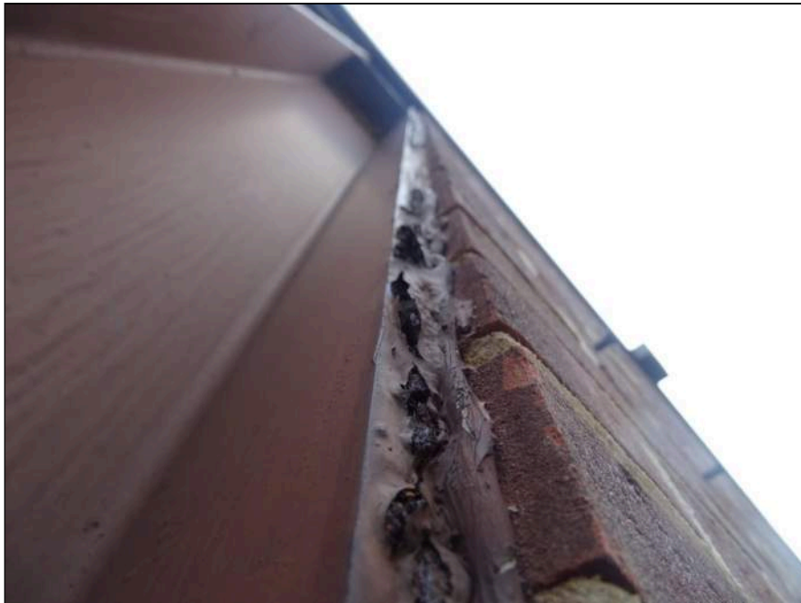
32 - Building exterior - note sealant deterioration
