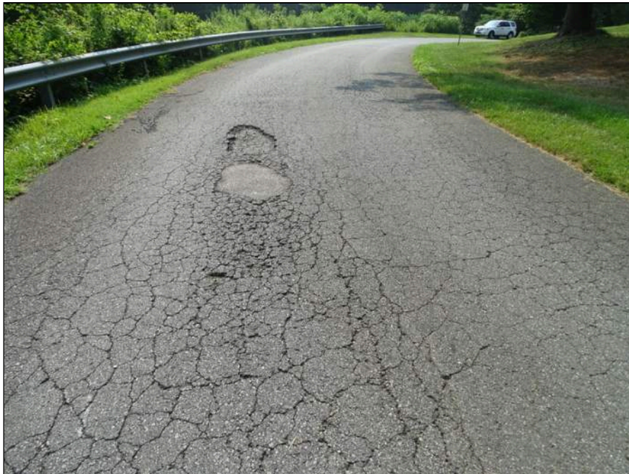
4 - Asphalt drive lane east side of the site - note cracking
