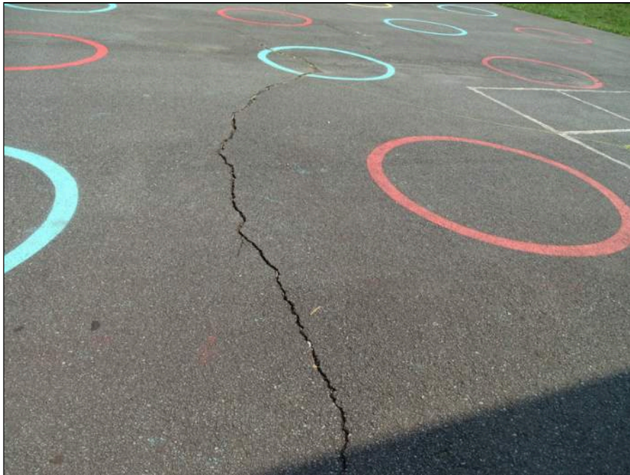
24 - Basketball court located between main building and gym - note cracking
