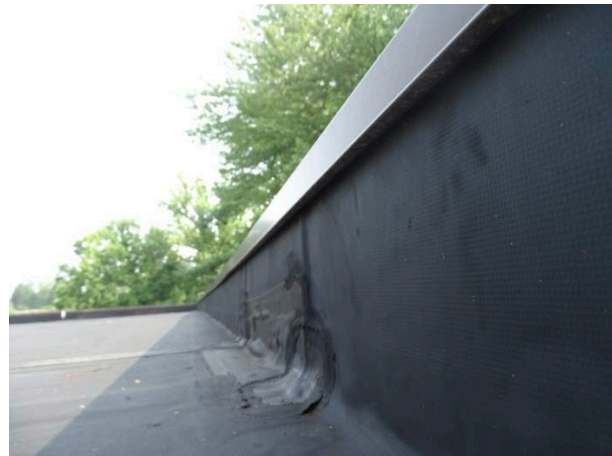
Single-ply membrane roofing system - note patching
