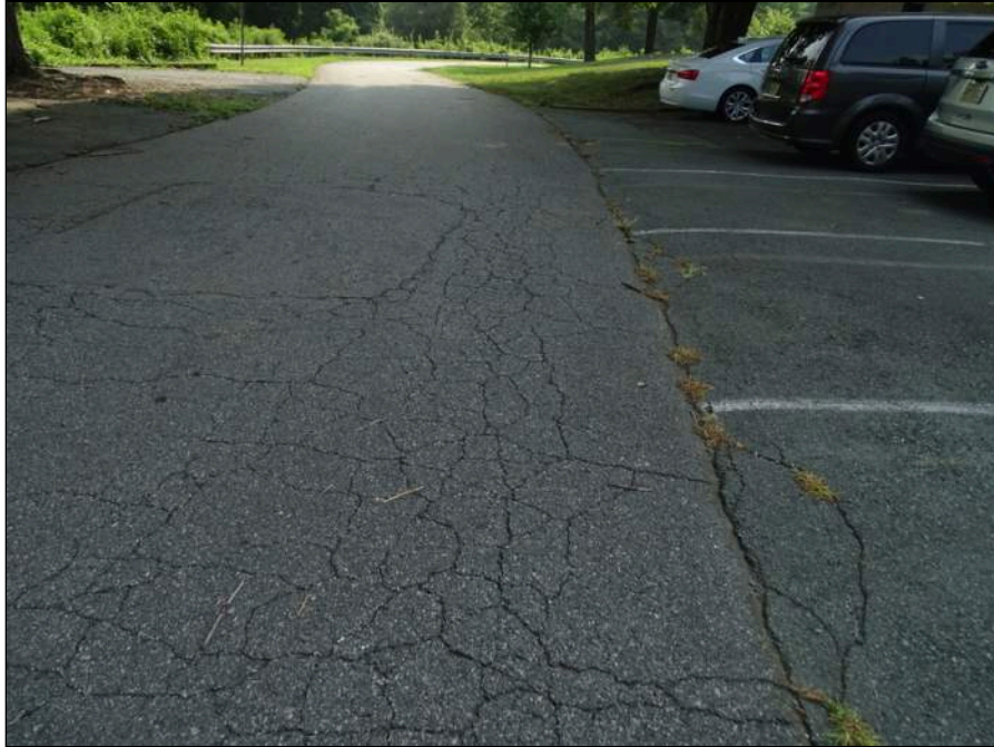
3 - Asphalt pavement parking - note alligator cracks
