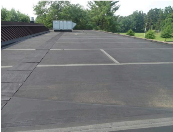
Single-ply membrane roofing system main building looking north
