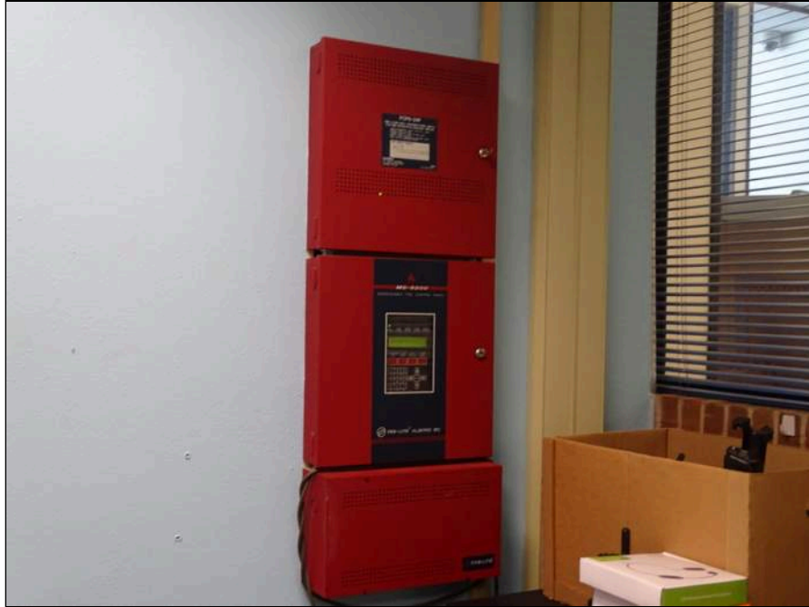
89 - Fire alarm control panel
