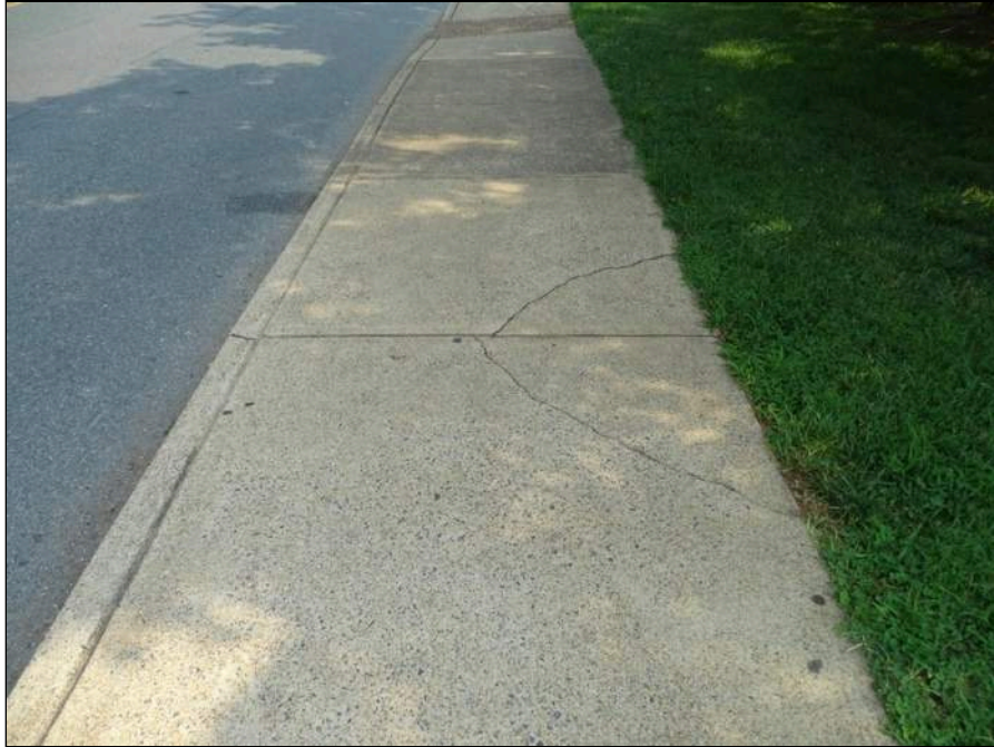
11 - Concrete sidewalk - note deterioration
