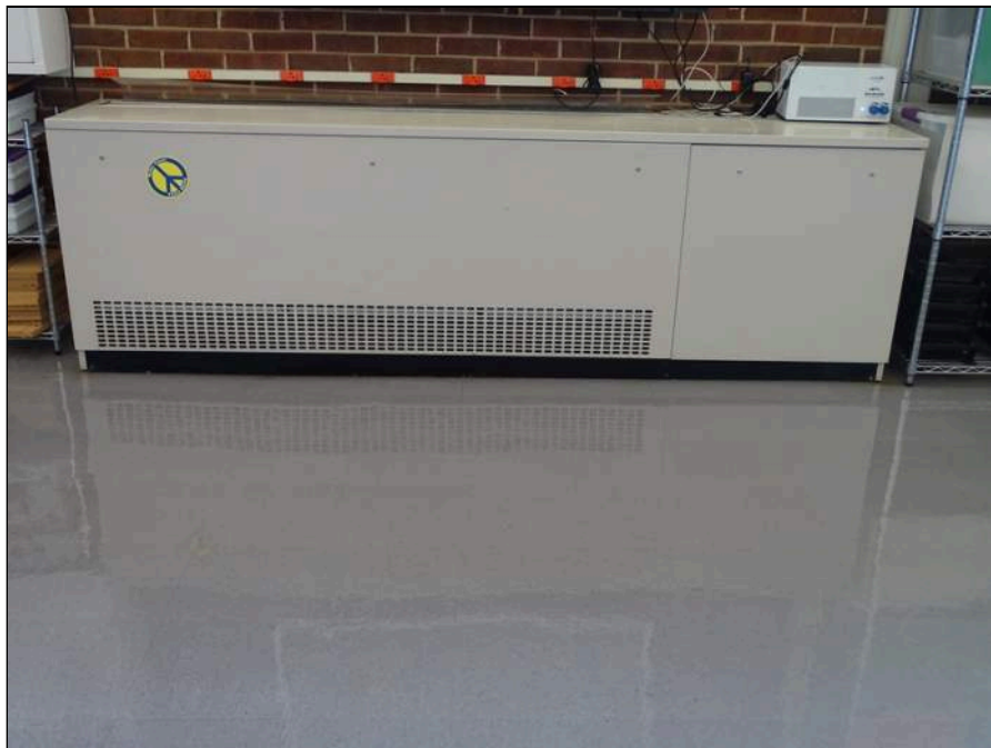
64 - Typical water source heat pump
