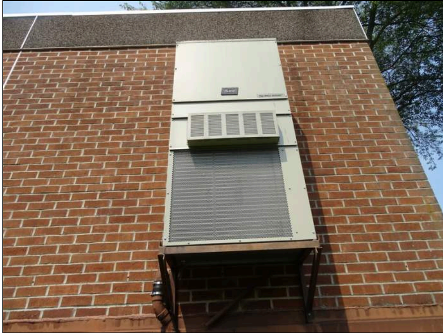
69 - Wall mounted air conditioner unit
