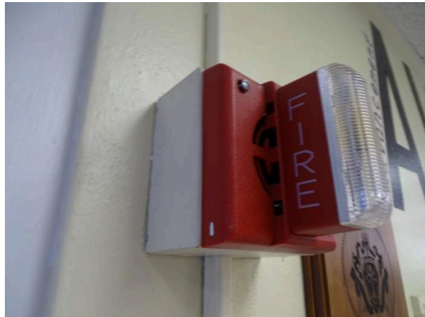
Typical fire alarm bell and strobe
