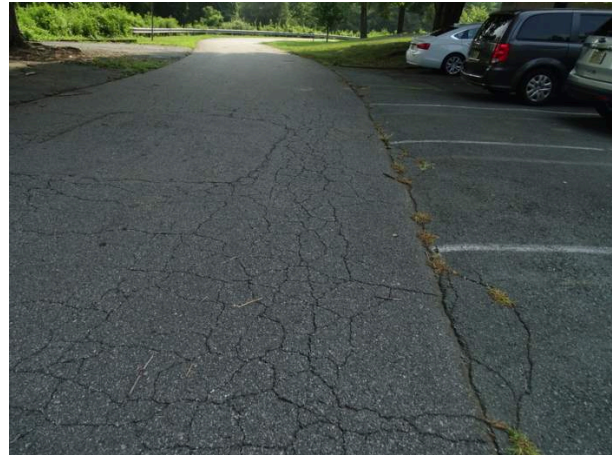
Asphalt pavement parking - note alligator cracks
