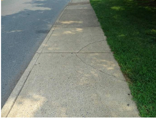
Concrete sidewalk - note deterioration
