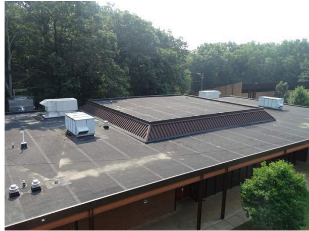
Single-ply membrane roofing system secondary building looking south
