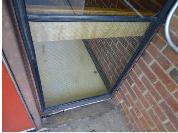
Typical exterior windows - note deterioration
