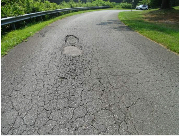
Asphalt drive lane east side of the site - note cracking
