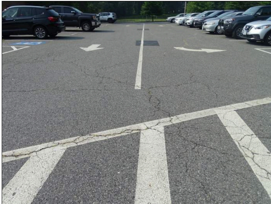
2 - Asphalt parking at west side of the site - note cracking
