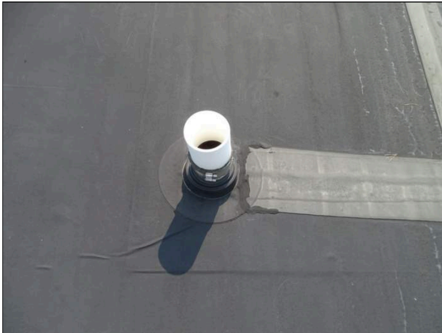
56 - Typical plumbing penetration
