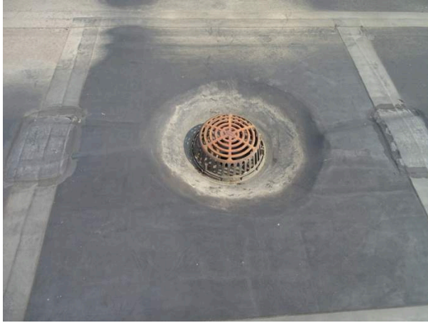
Typical internal drain
