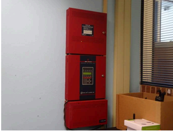
Fire alarm control panel
