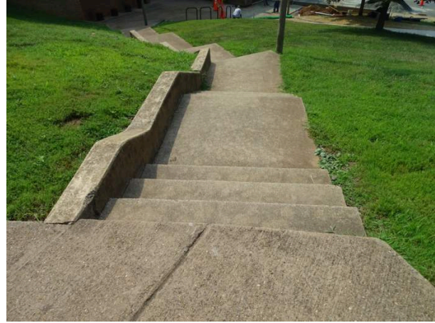
Typical concrete steps - note missing handrail
