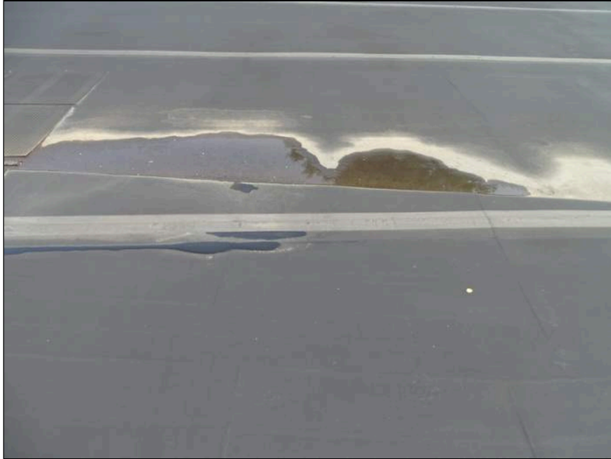
55 - Single-ply membrane roofing system - note ponding
