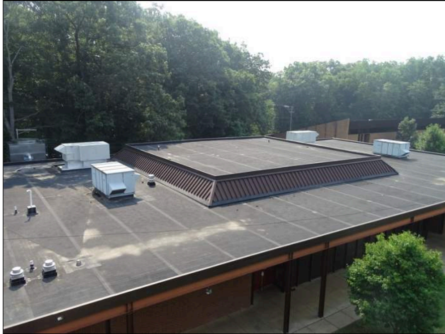
51 - Single-ply membrane roofing system secondary building looking south
