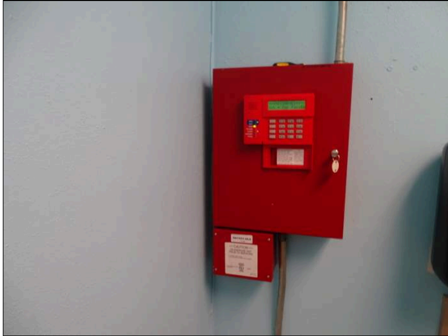
85 - Fire alarm annunciator panel
