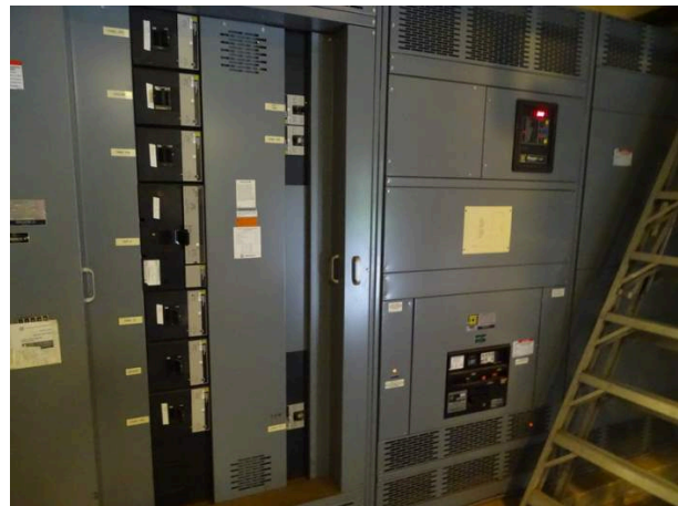
Main electrical switchgear
