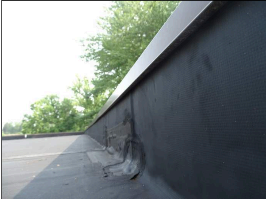
53 - Single-ply membrane roofing system - note patching
