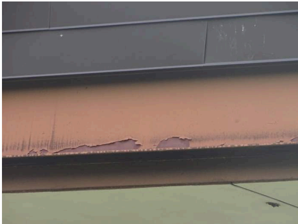
Building exterior - note peeling paint
