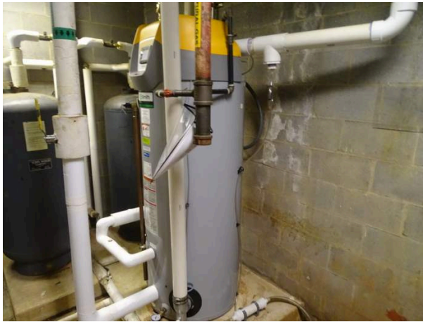
Gas domestic water heater located in main building
