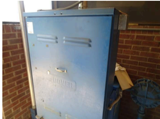
Elevator controls
