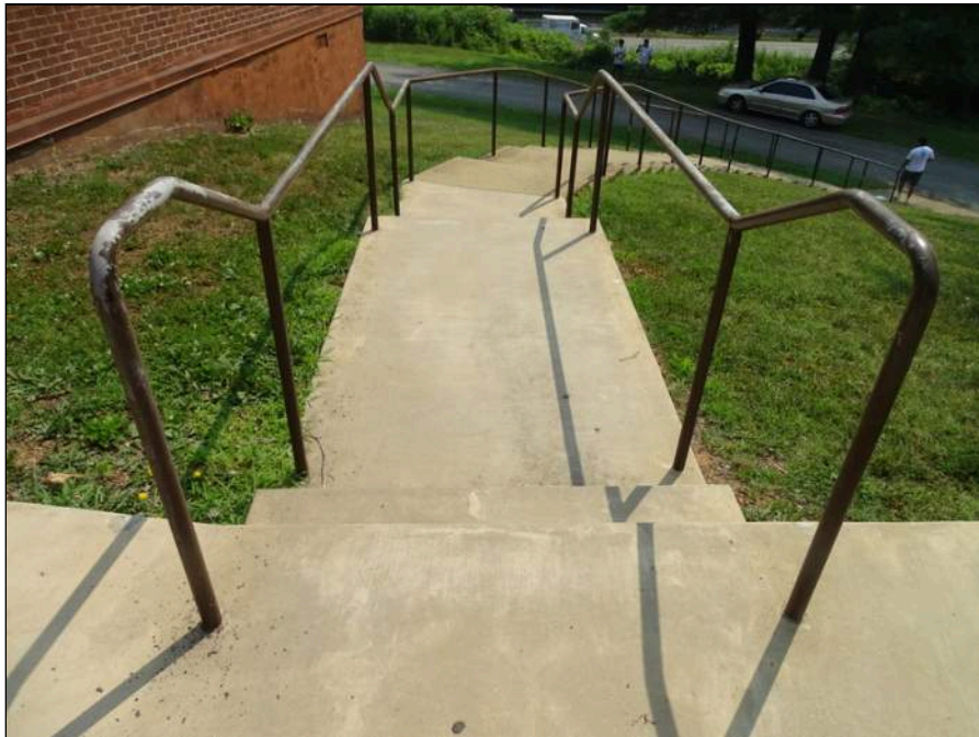
14 - Typical concrete steps handrail - note handrail deterioration
