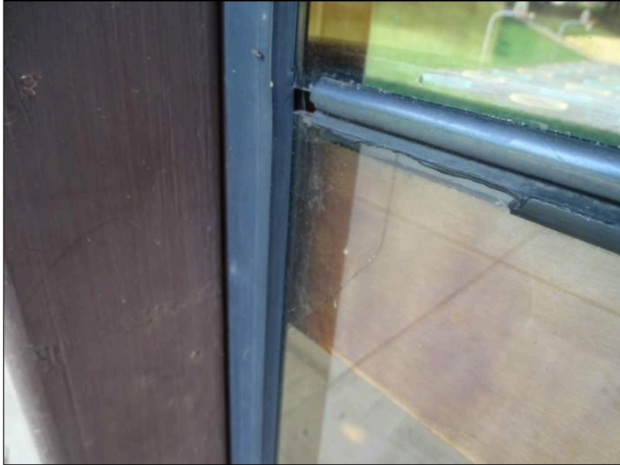
49 - Typical exterior windows - note deterioration
