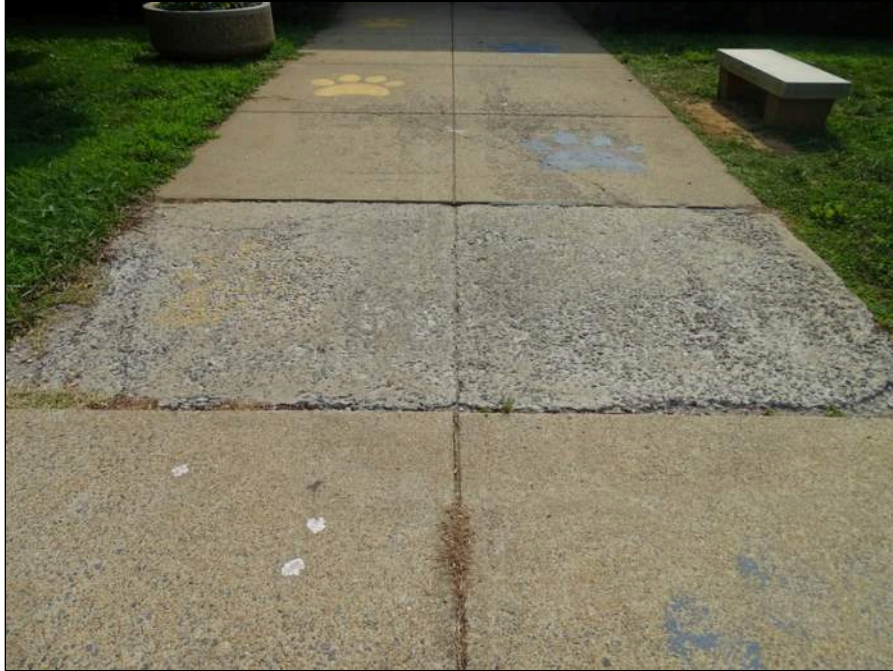
9 - Concrete sidewalk - note deterioration
