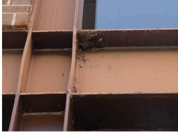
Main building entrance exterior doors upper level - note peeling paint
