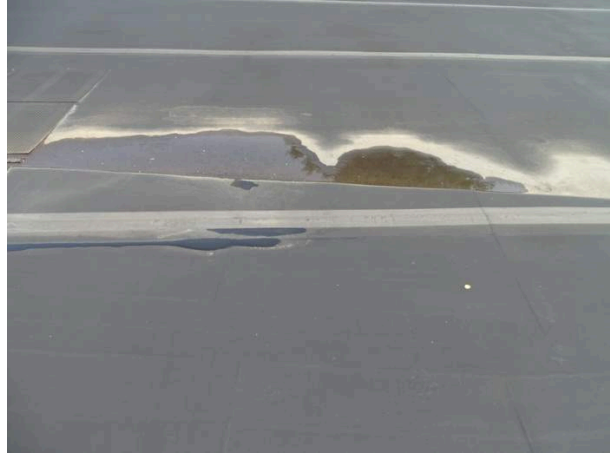
Single-ply membrane roofing system - note ponding
