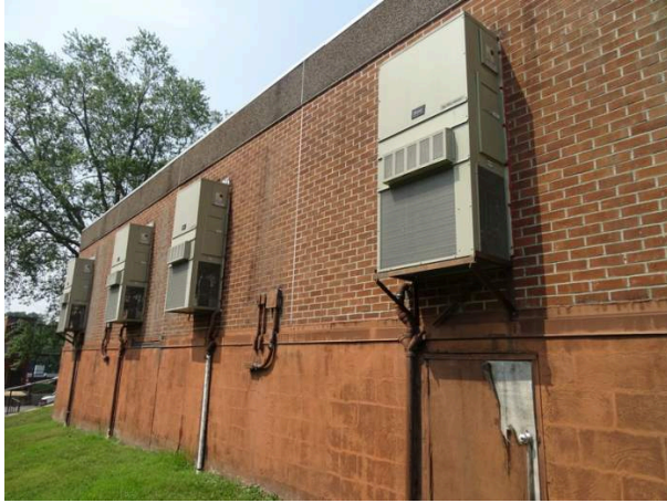
Wall mounted air conditioner unit
