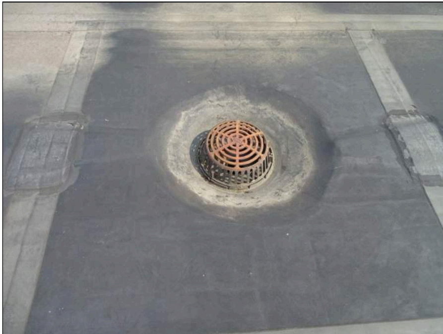
54 - Typical internal drain
