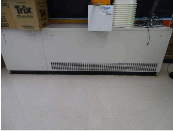
Typical water source heat pump
