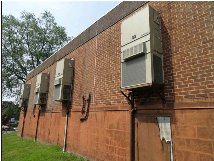
68 - Wall mounted air conditioner unit
