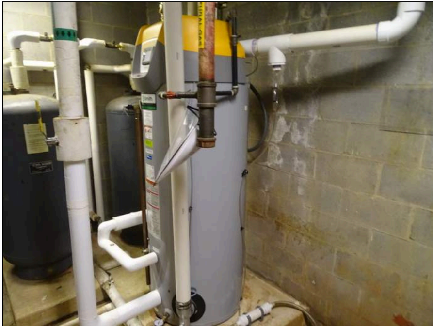
58 - Gas domestic water heater located in main building
