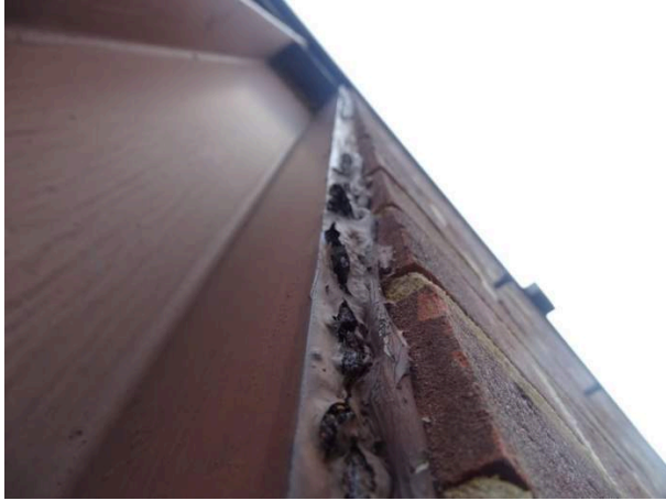
Building exterior - note sealant deterioration
