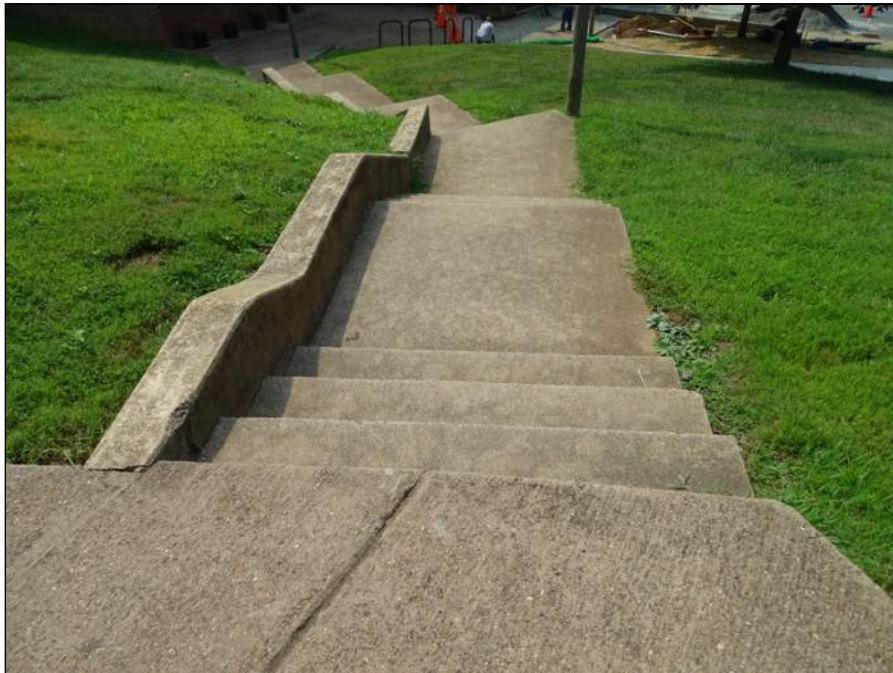
16 - Typical concrete steps - note missing handrail
