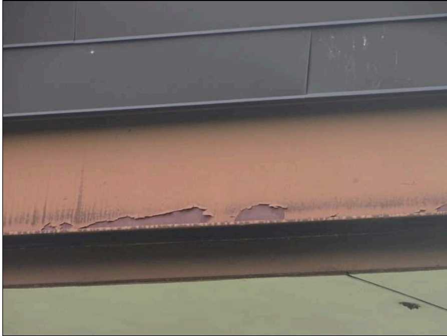
35 - Building exterior - note peeling paint
