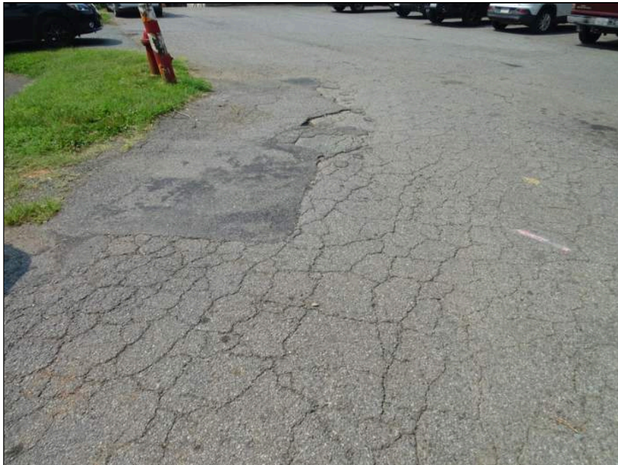
6 - Asphalt drive lane east side of the site - note cracking
