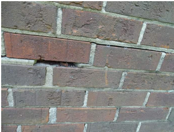
Building exterior - note deterioration
