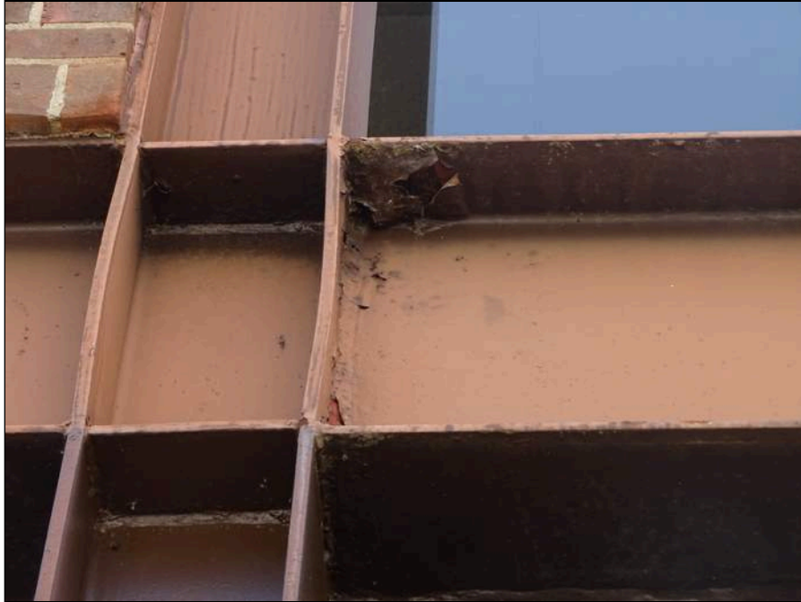
33 - Main building entrance exterior doors upper level - note peeling paint
