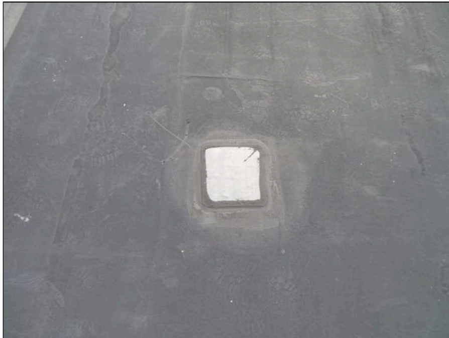
52 - Single-ply membrane roofing system - note patching
