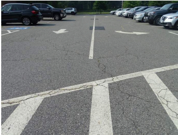
Asphalt parking at west side of the site - note cracking
