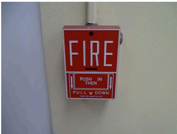
Typical fire alarm pull station
