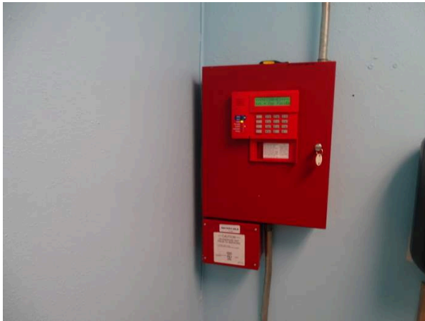
Fire alarm annunciator panel
