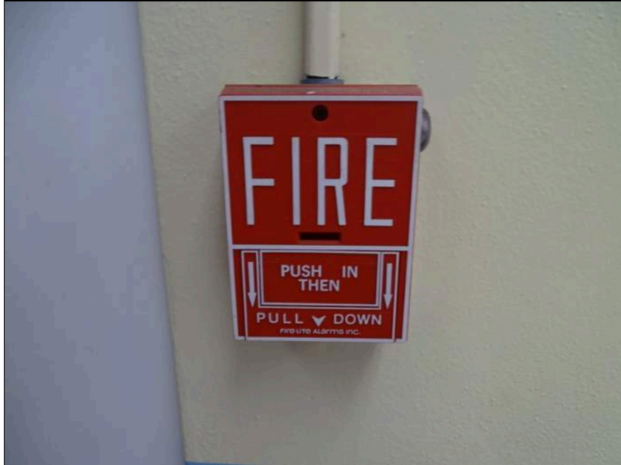
87 - Typical fire alarm pull station
