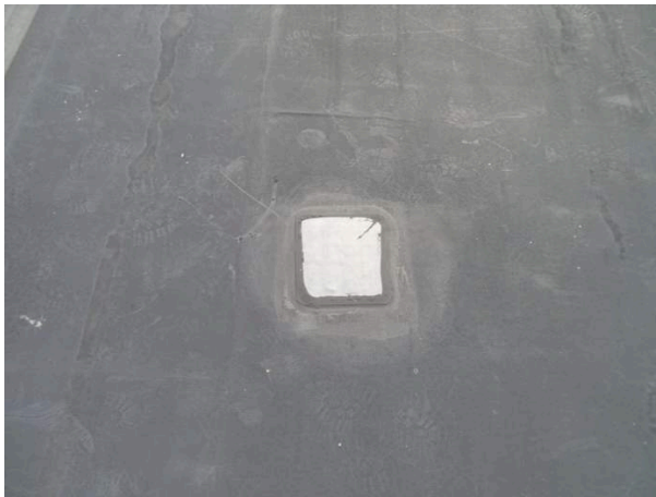
Single-ply membrane roofing system - note patching
