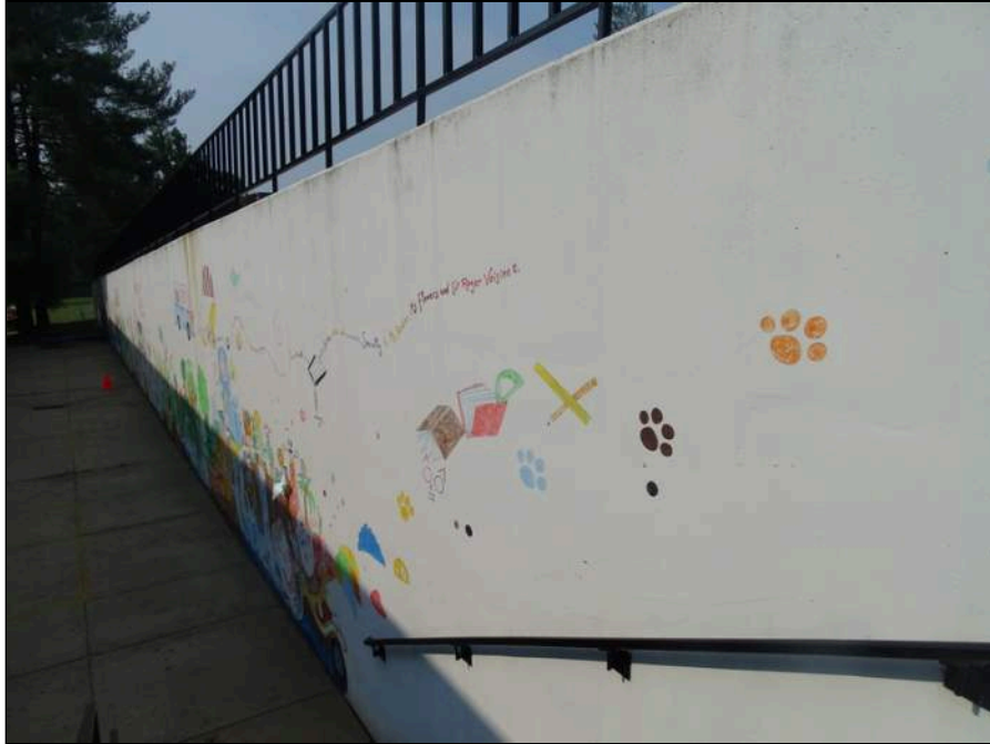
21 - Cast in place concrete retaining wall between main building and west parking area
