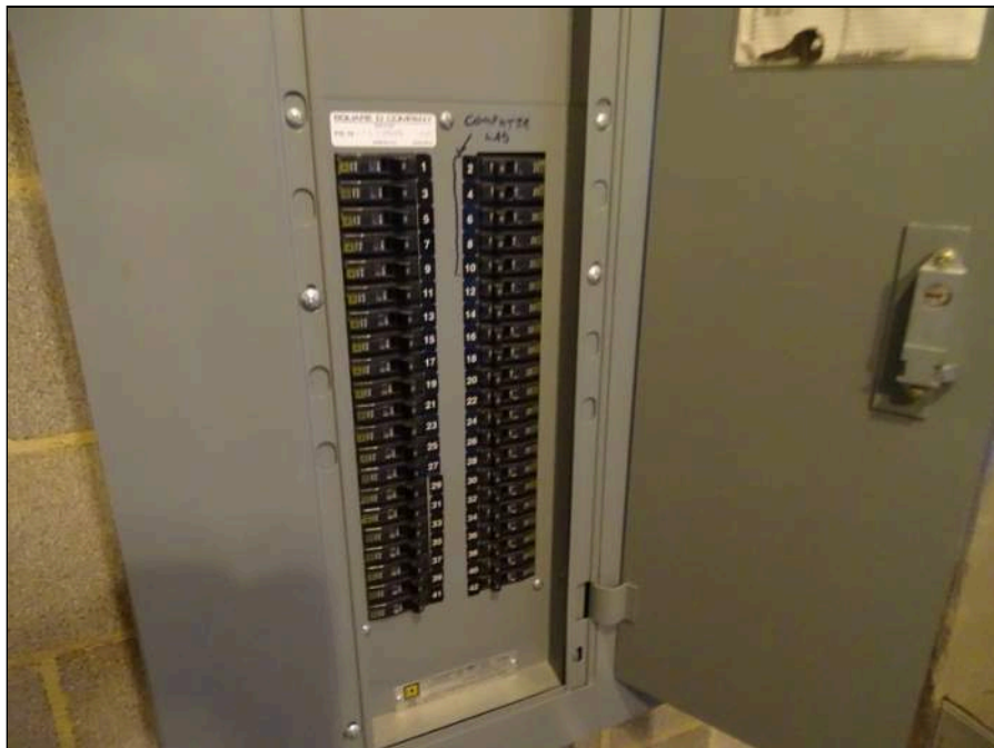
76 - Typical newer electrical circuit breaker panel
