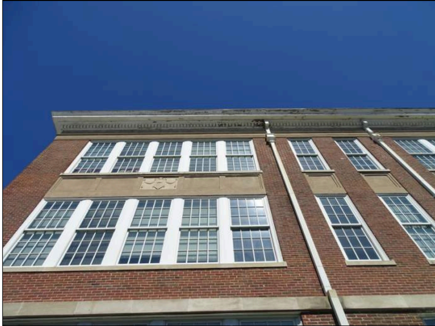
29 - Building exterior - note rotten through cornice work
