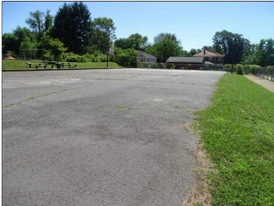
4 - Asphalt pavement - note cracking
