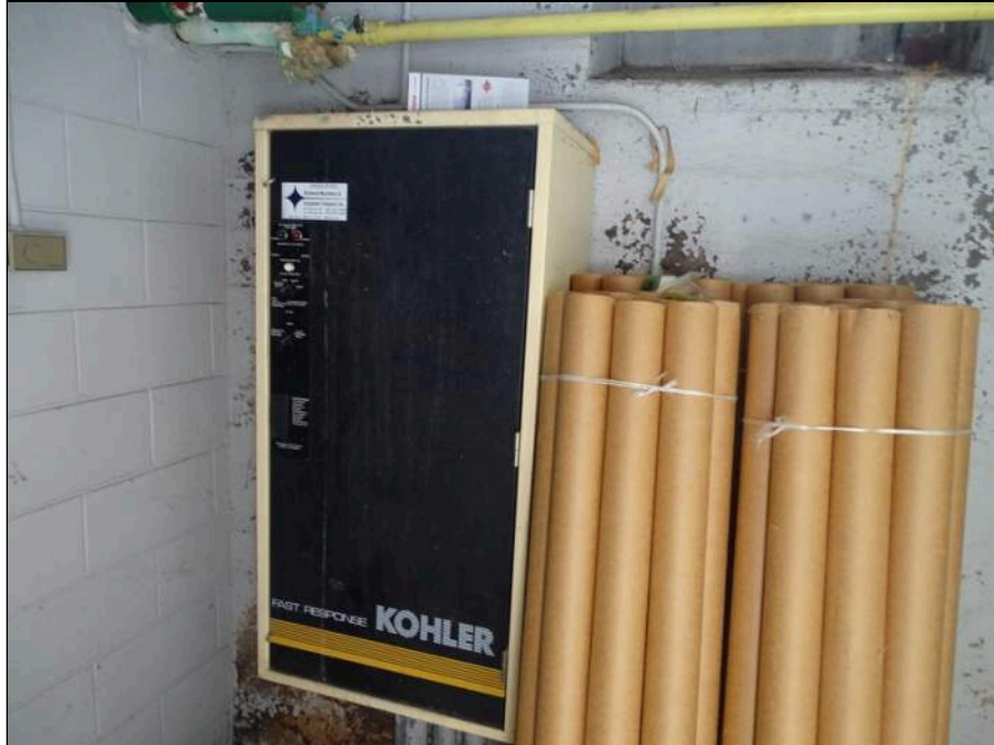
65 - Emergency power transfer switch
