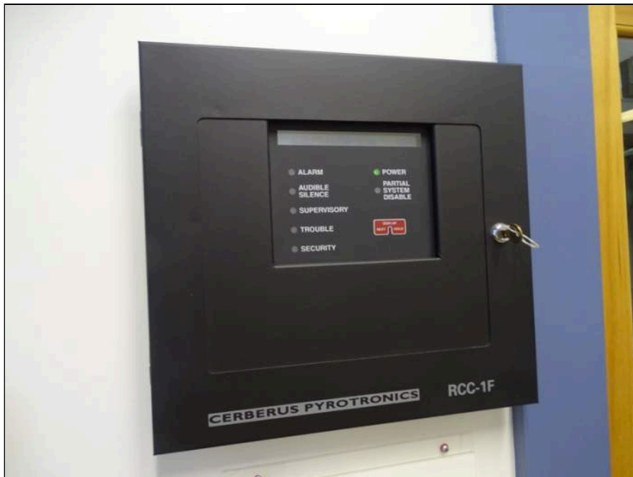
78 - Fire alarm control panel
