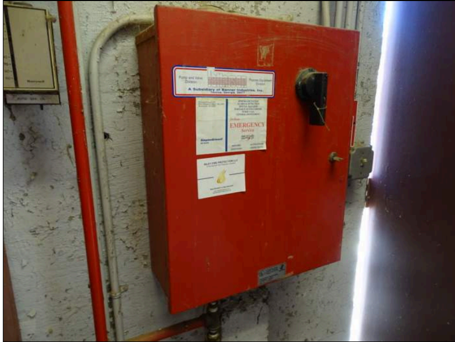
71 - Fire sprinkler pump controller
