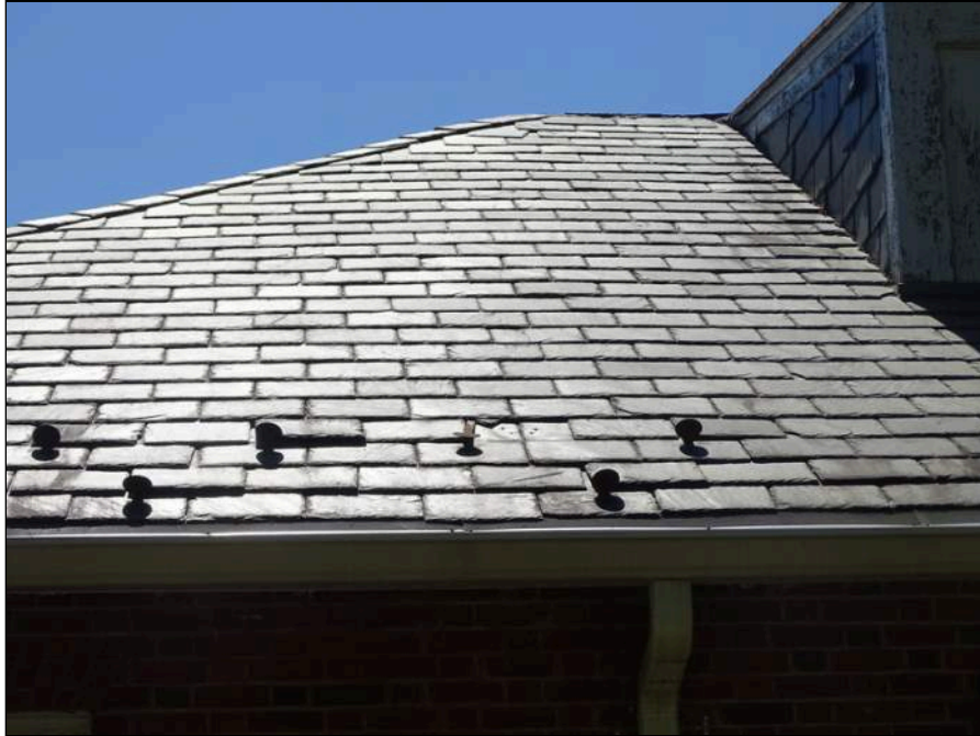
47 - Slate shingle roofing system
