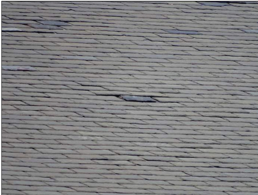
48 - Slate shingle roofing system - note damaged and misaligned shingles
