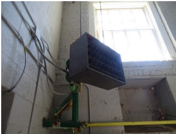
Space heater located in main utility room
