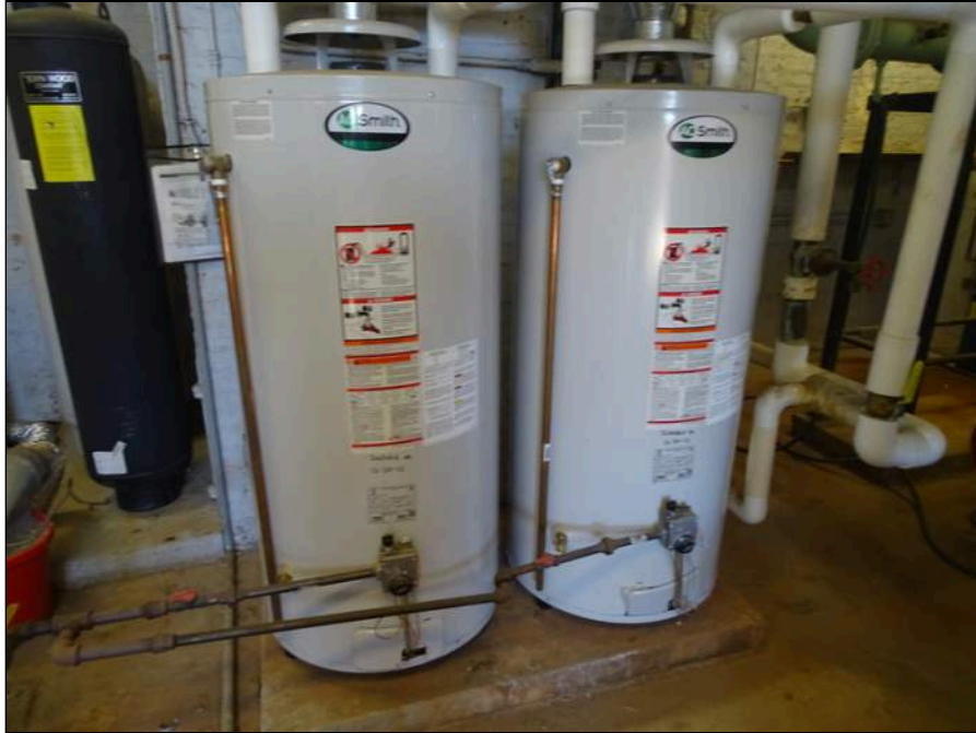
51 - Gas domestic water heaters
