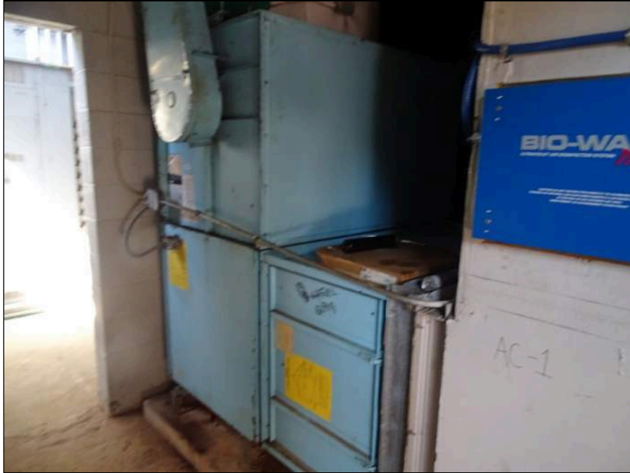
55 - Air Handler Unit located in main utility room
