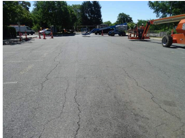
Asphalt pavement - note cracking
