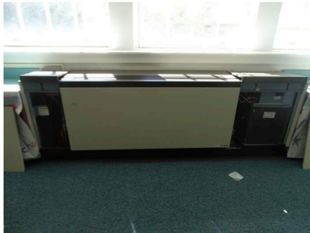
Typical newer Water Source Heat Pump
