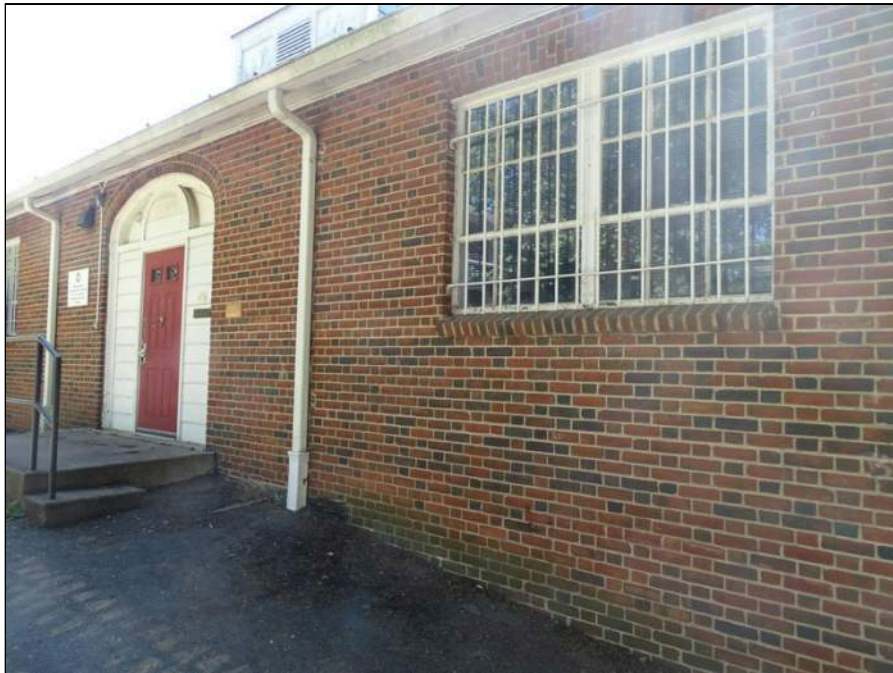
44 - Typical exterior window security fence - note peeling paint
