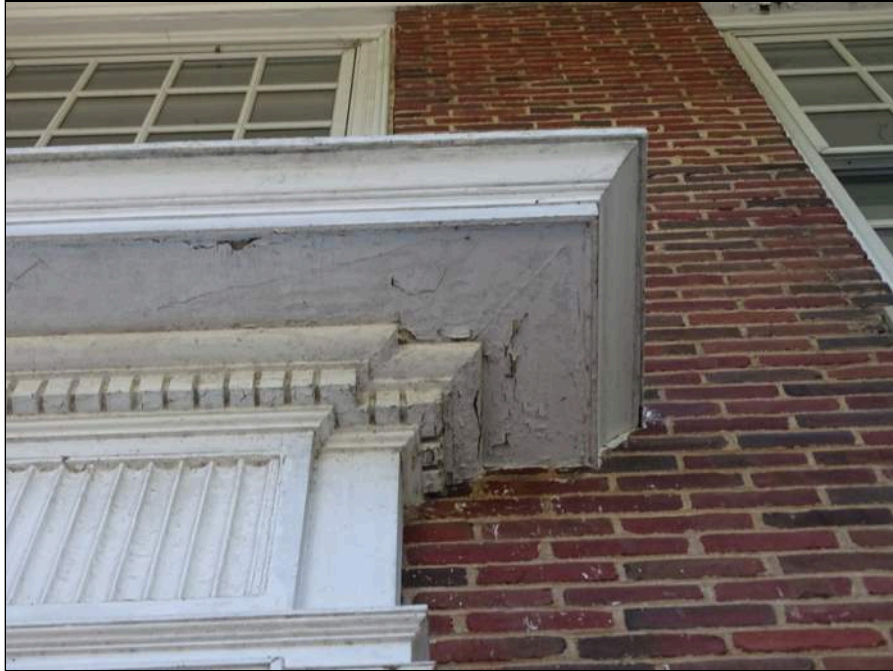
25 - Building exterior - note rotten through cornice work
