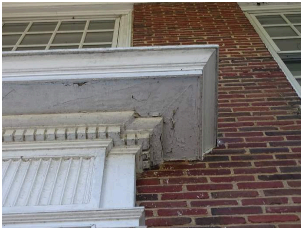
Building exterior - note rotten through cornice work
