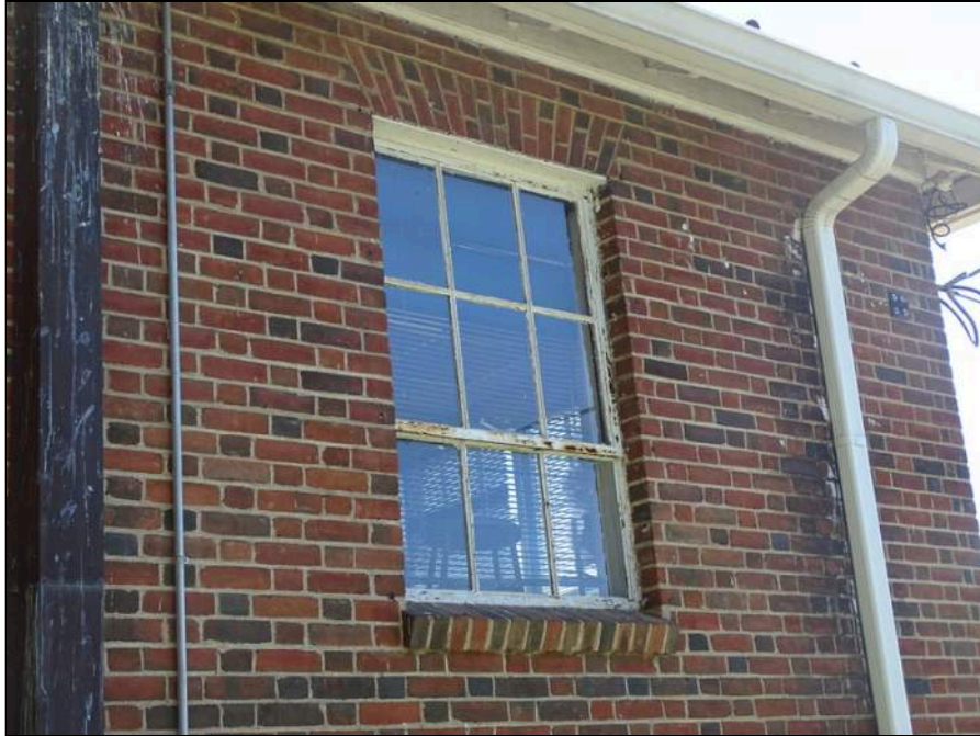
43 - Typical exterior window - note peeling paint
