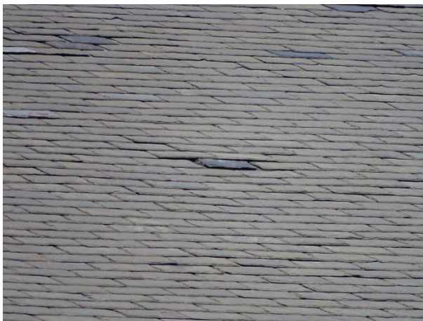
Slate shingle roofing system - note damaged and misaligned shingles
