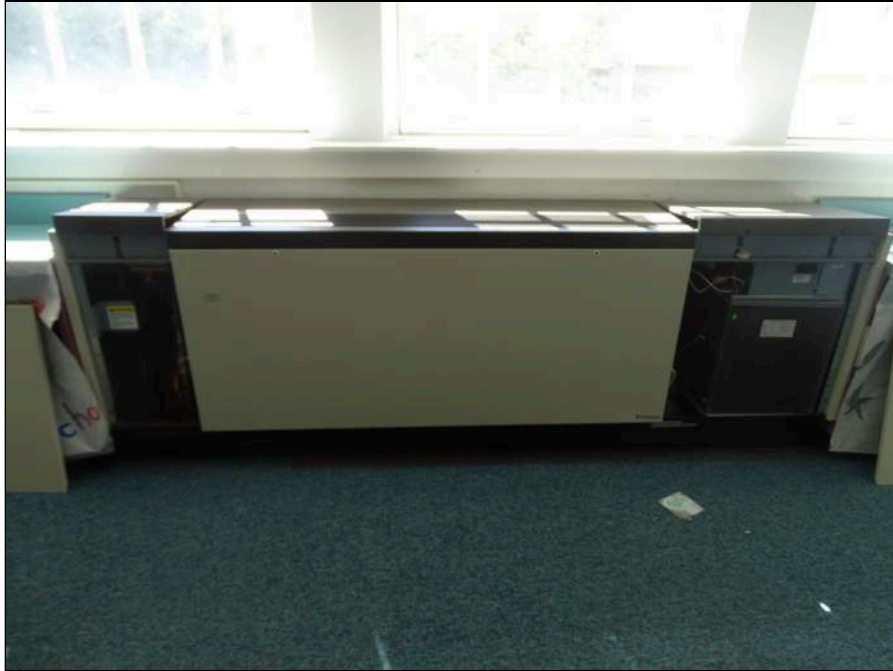
57 - Typical newer Water Source Heat Pump
