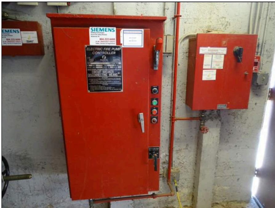
70 - Fire sprinkler pump controller
