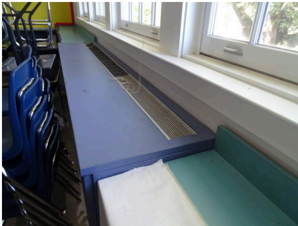
Typical older Water Source Heat Pump
