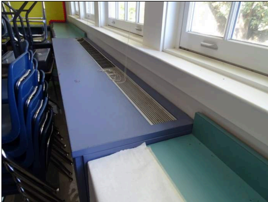
56 - Typical older Water Source Heat Pump
