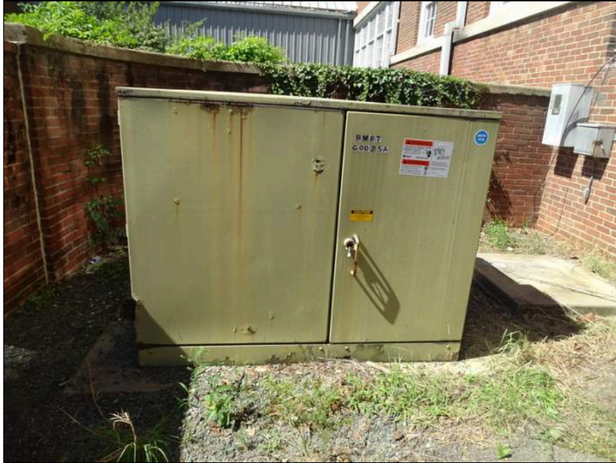
61 - Electric utility transformer
