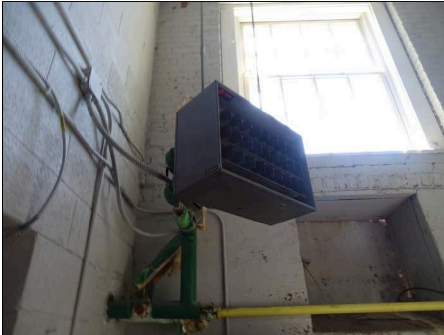
60 - Space heater located in main utility room
