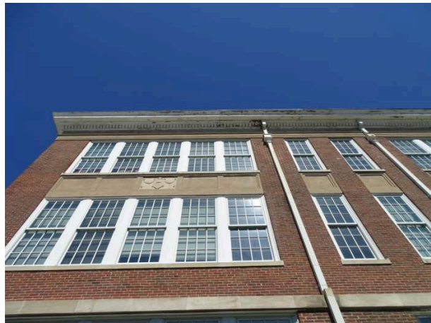
Building exterior - note rotten through cornice work
