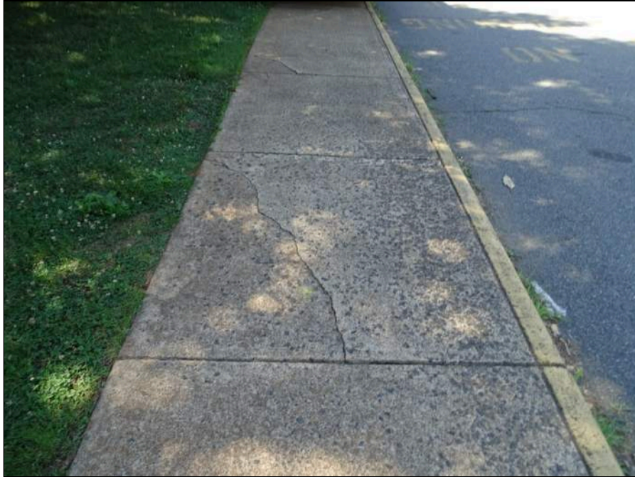
11 - Typical concrete sidewalk - note cracking
