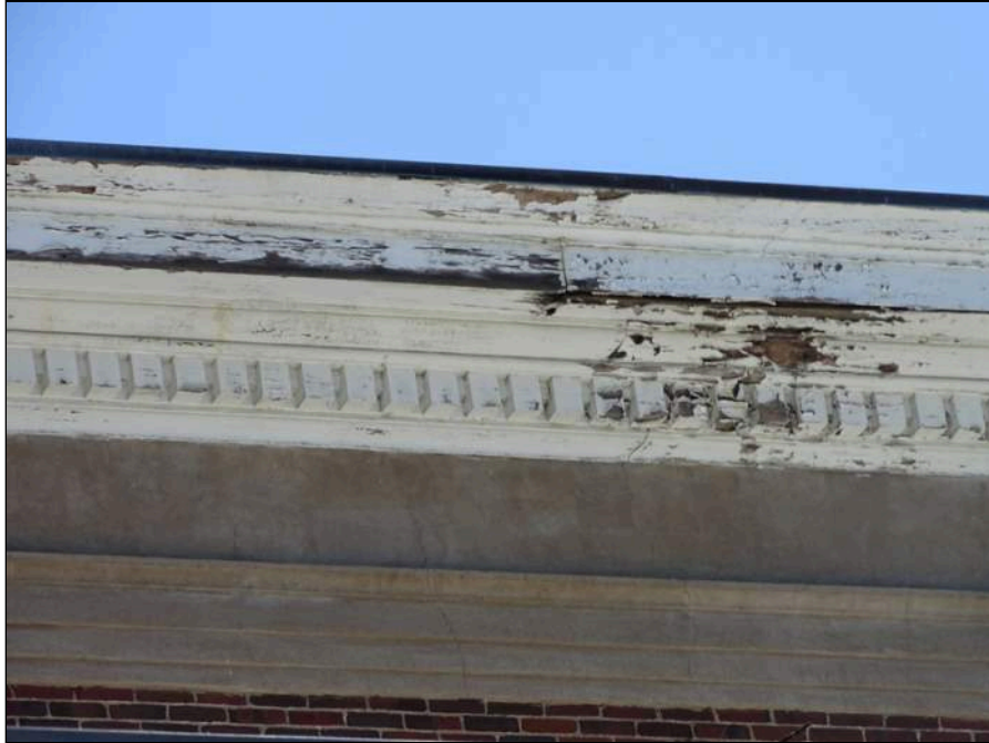
33 - Building exterior - note rotten through cornice work
