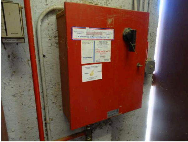
Fire sprinkler pump controller
