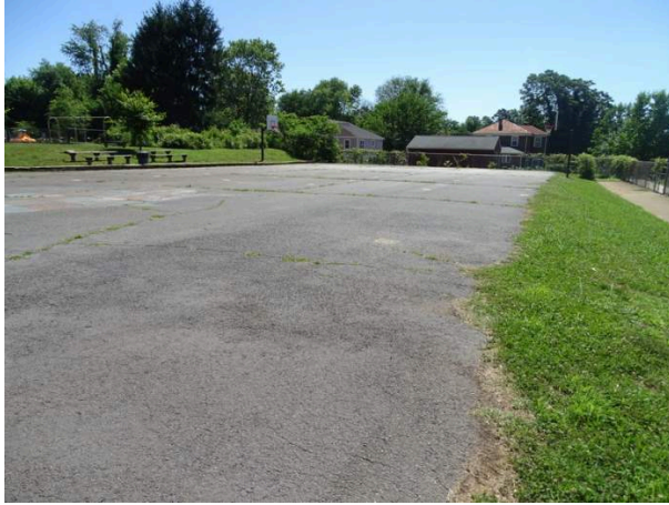
Asphalt pavement - note cracking
