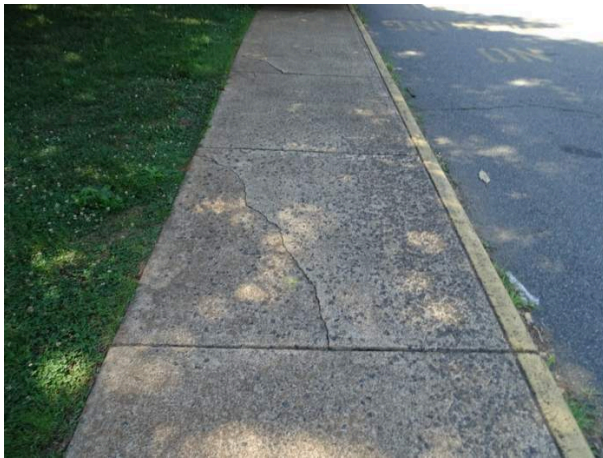
Typical concrete sidewalk - note cracking
