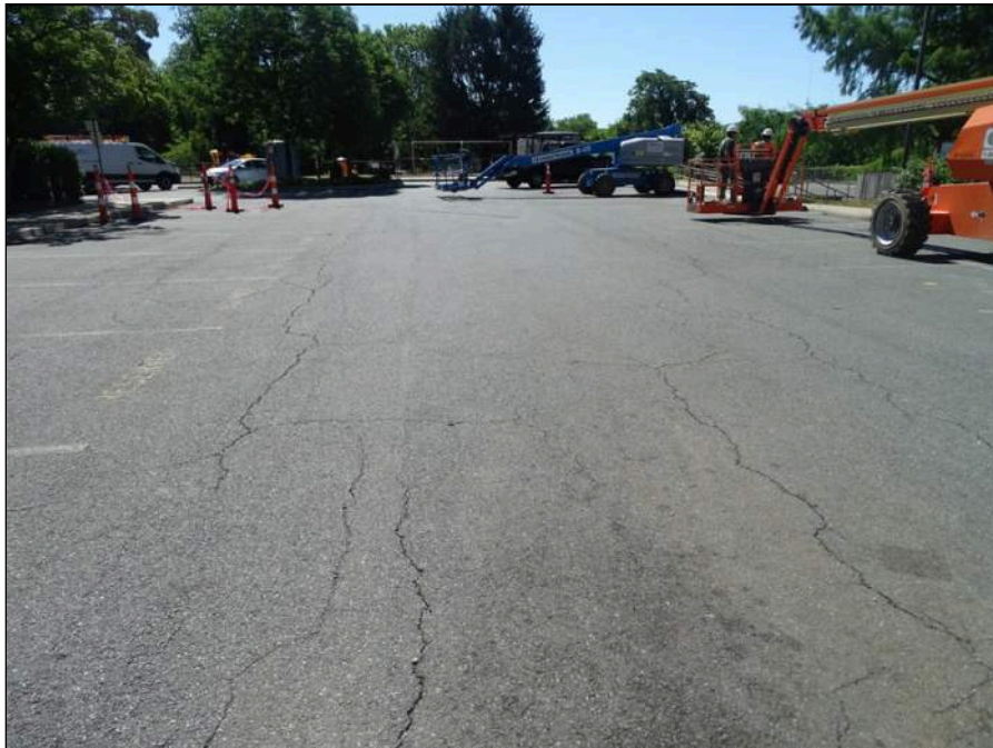
6 - Asphalt pavement - note cracking
