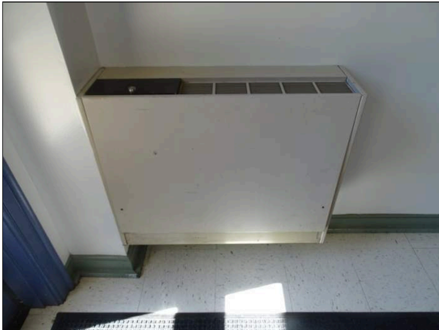
58 - Typical newer Water Source Heat Pump
