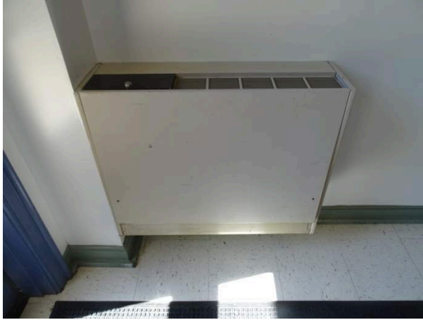
Typical newer Water Source Heat Pump
