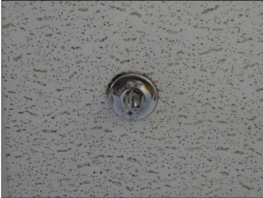
73 - Typical fire sprinkler head
