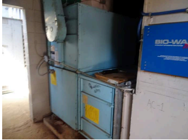
Air Handler Unit located in main utility room
