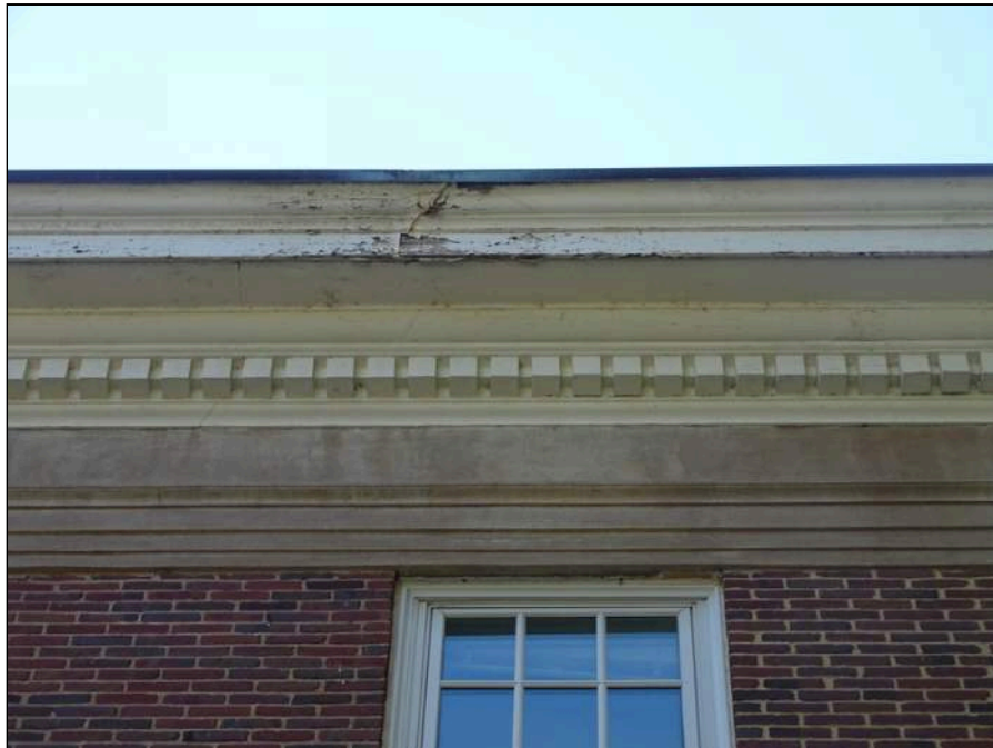
24 - Building exterior - note rotten through cornice work
