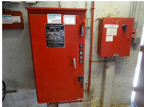
Fire sprinkler pump controller
