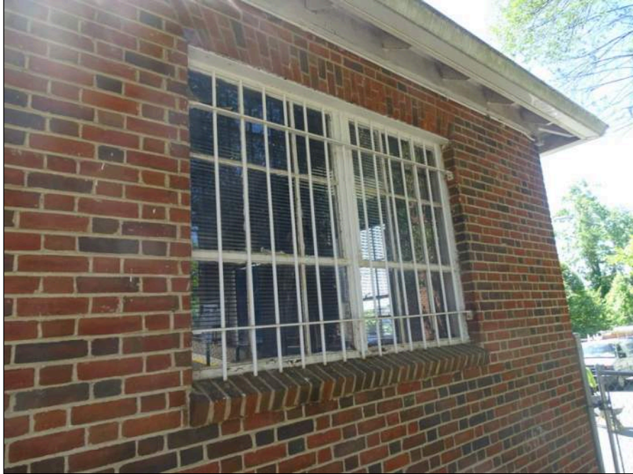
45 - Typical exterior window security fence - note peeling paint
