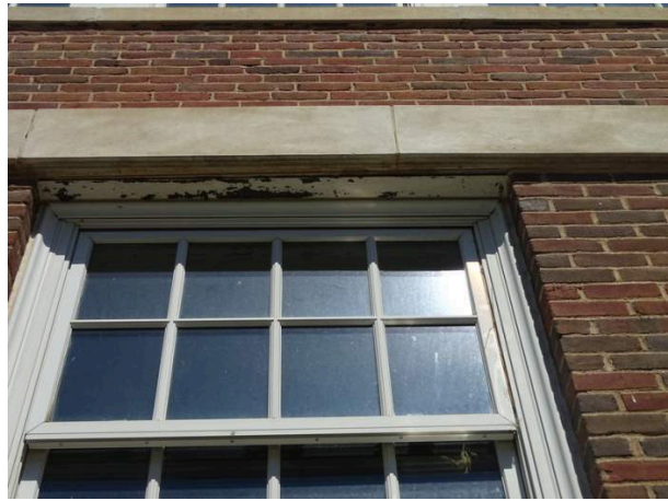
Typical exterior window - note peeling paint
