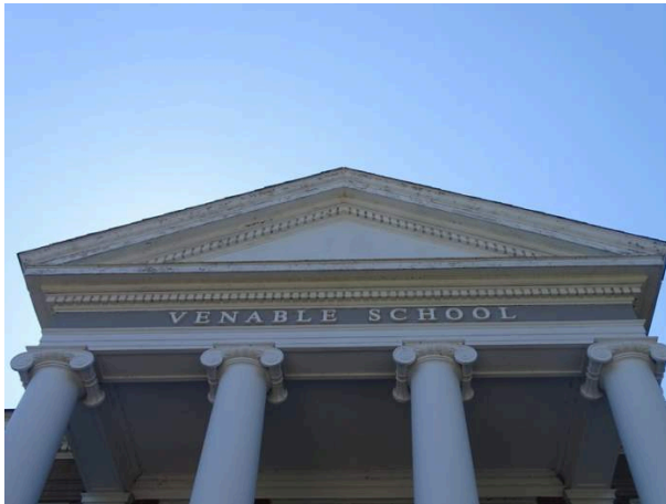
Building exterior - note peeling paint
