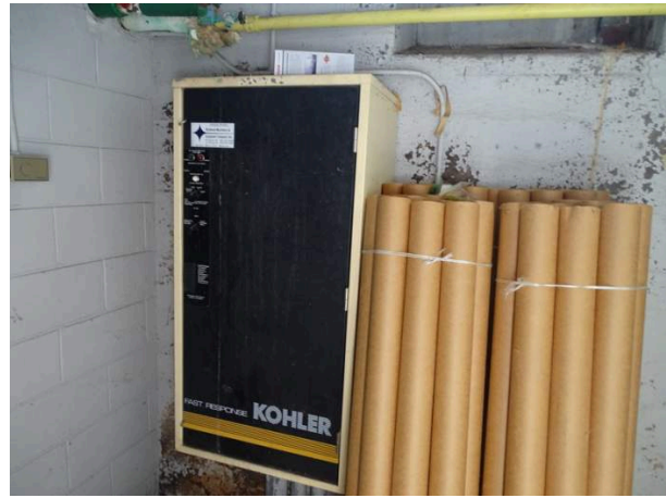
Emergency power transfer switch
