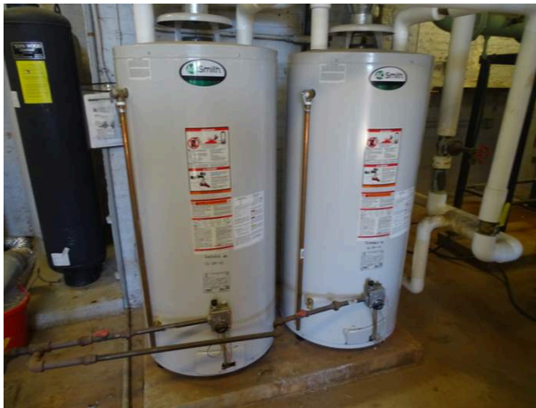
Gas domestic water heaters
