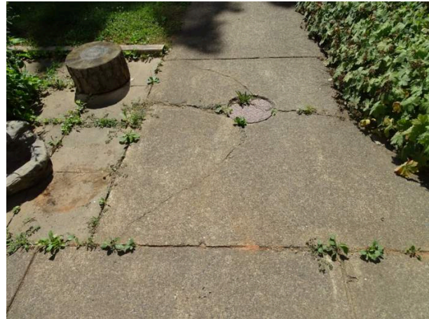
Typical concrete sidewalk - note cracking
