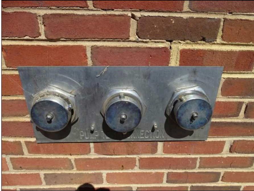
77 - Fire Pump Test Connection
