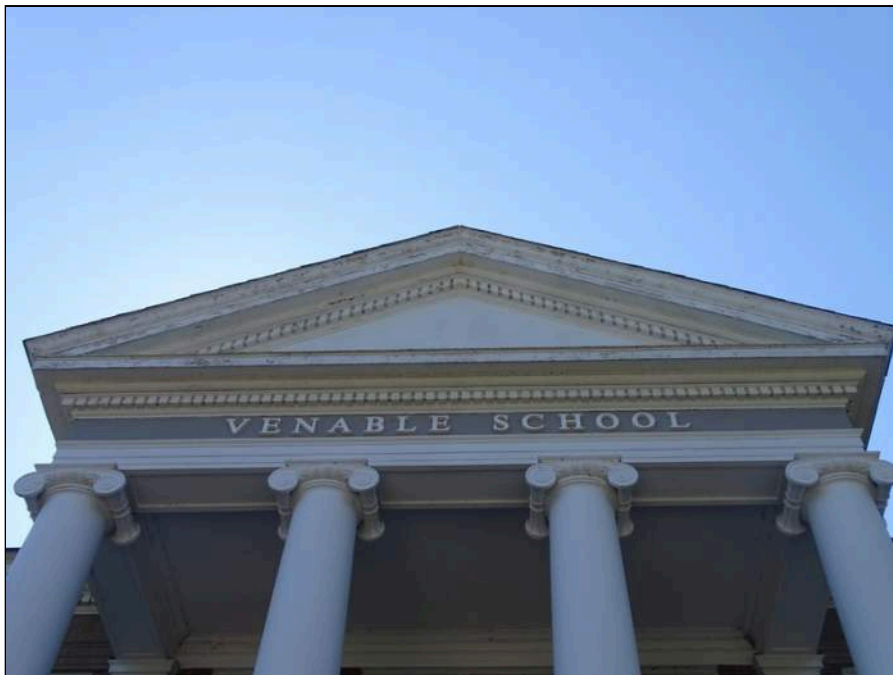
34 - Building exterior - note peeling paint
