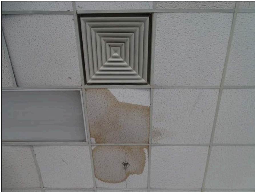
50 - water leakage
