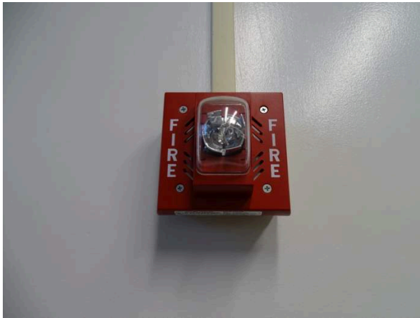
Typical fire alarm bell and strobe
