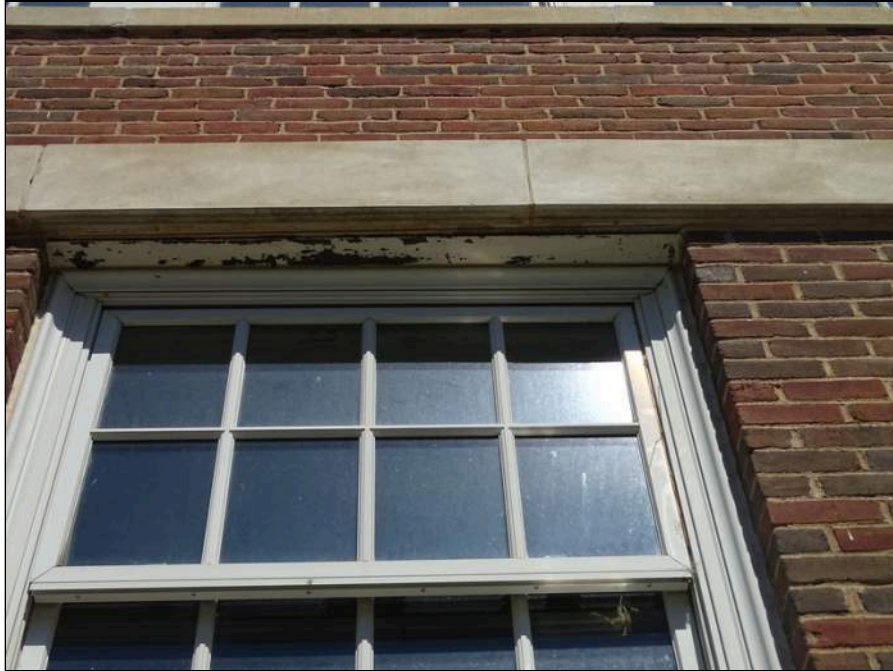
41 - Typical exterior window - note peeling paint
