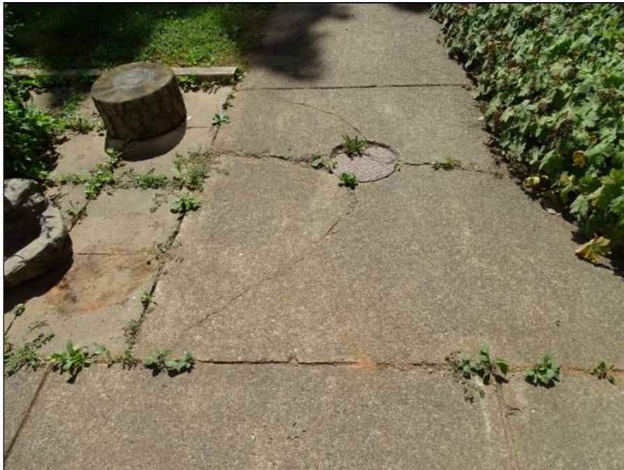
8 - Typical concrete sidewalk - note cracking
