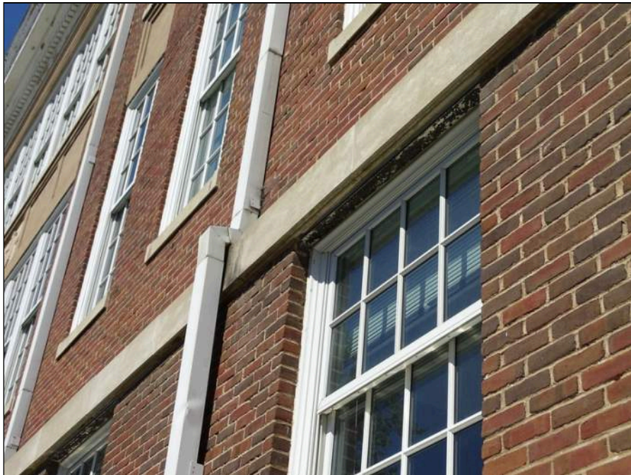
42 - Typical exterior window - note peeling paint
