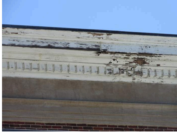
Building exterior - note rotten through cornice work
