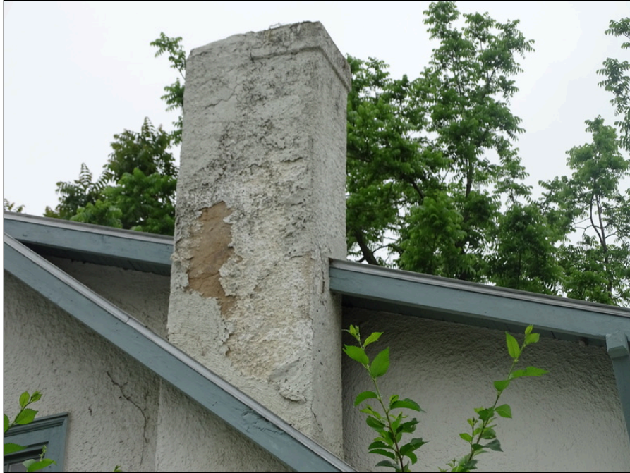
19 - Deterioration of exteriors at chimney
