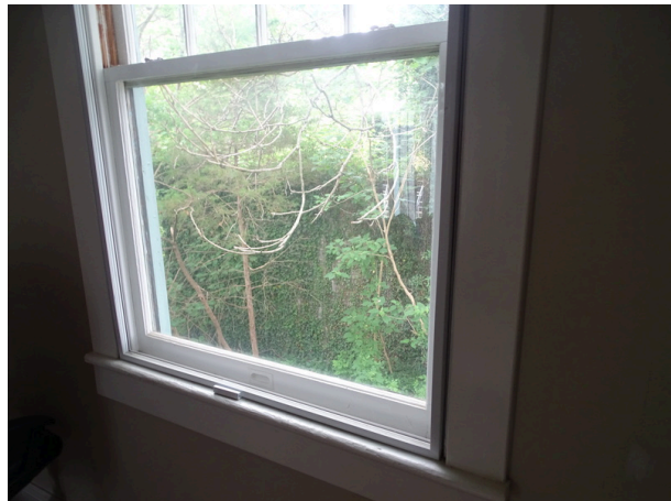
Additional window units installed for energy conservation
