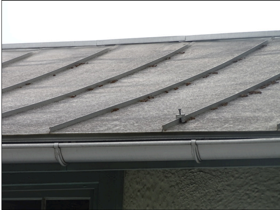
23 - Metal roofing system south side of the building
