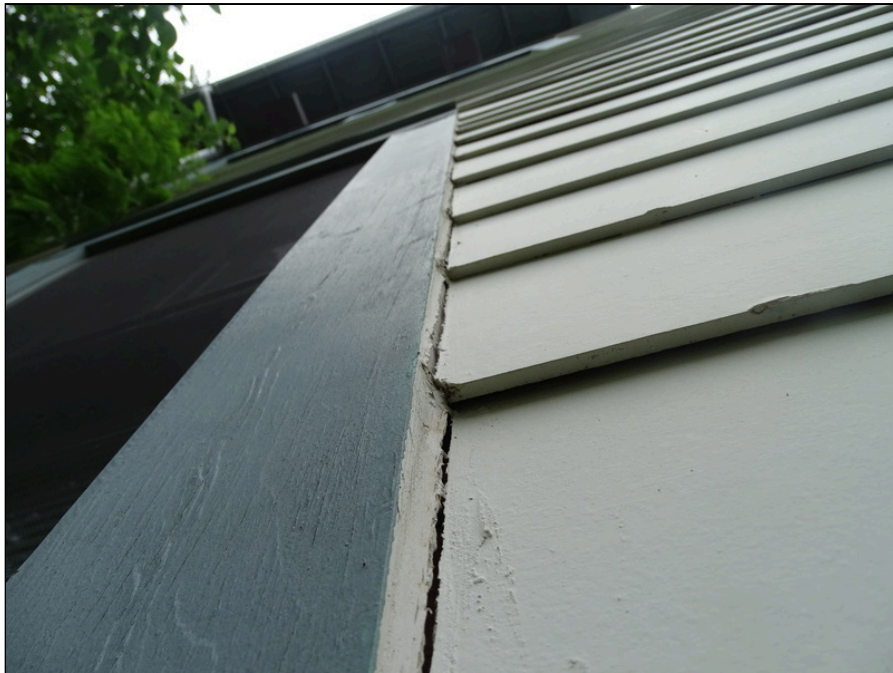
18 - Building exterior sealants - note deterioration
