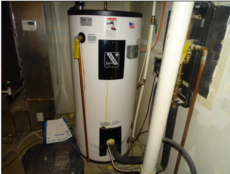
32 - Solar thermal water heater
