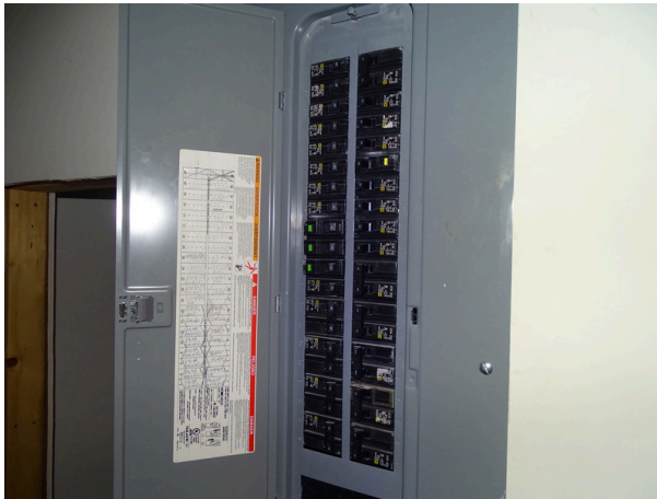
Typical circuit breaker panel
