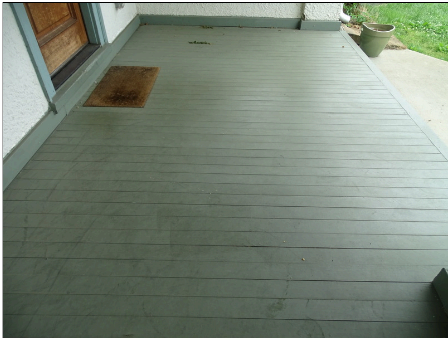
56 - Accessible ramp not provided from sidewalk to porch to threshold of main entrance
