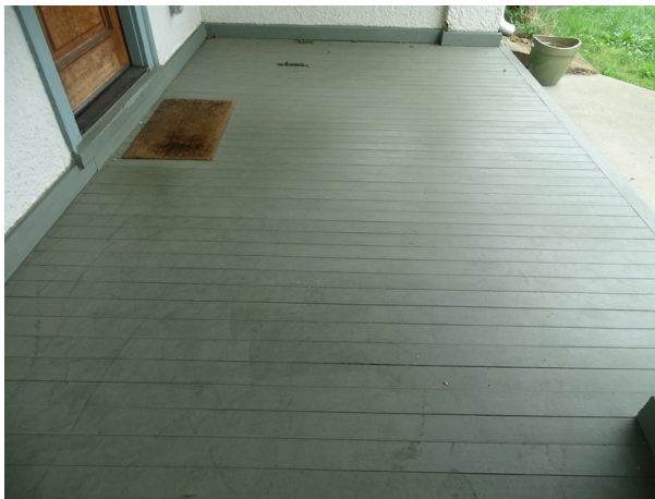
Accessible ramp not provided from sidewalk to porch to threshold of main entrance
