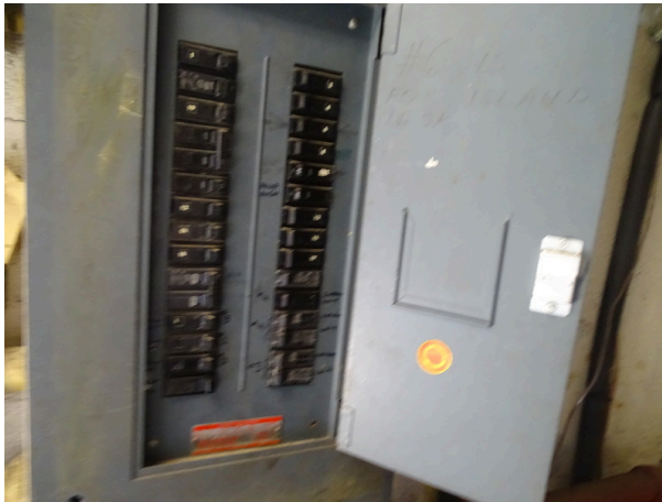
Electrical panel - note missing components
