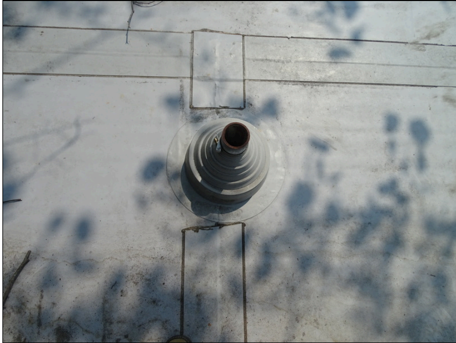
27 - Typical plumbing penetration
