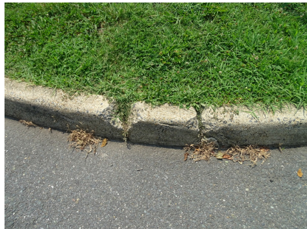
Typical concrete curb - note deterioration
