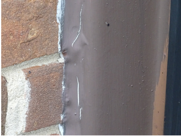
Building exterior overview - note sealant deterioration
