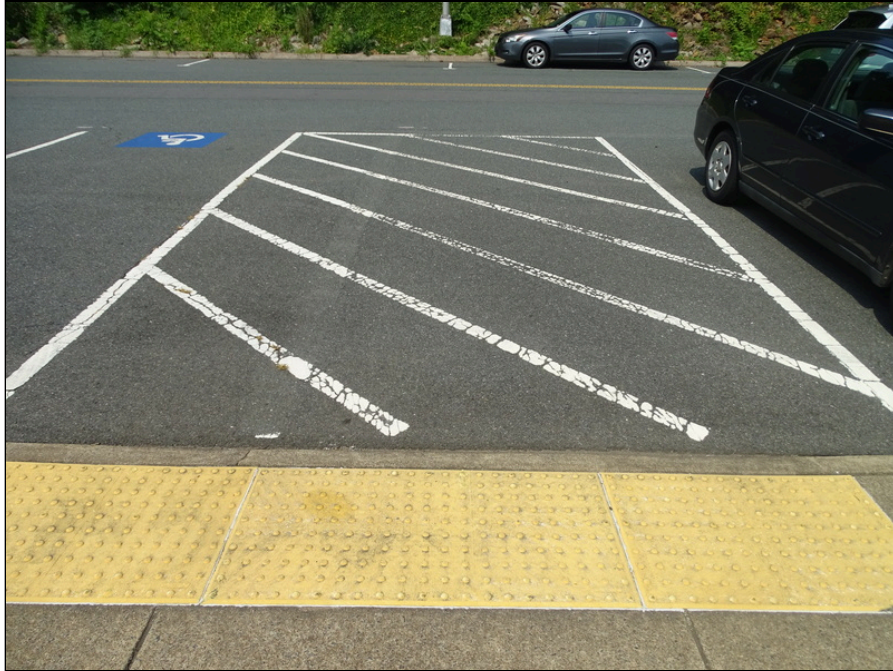
5 - Curb ramp with truncated domes
