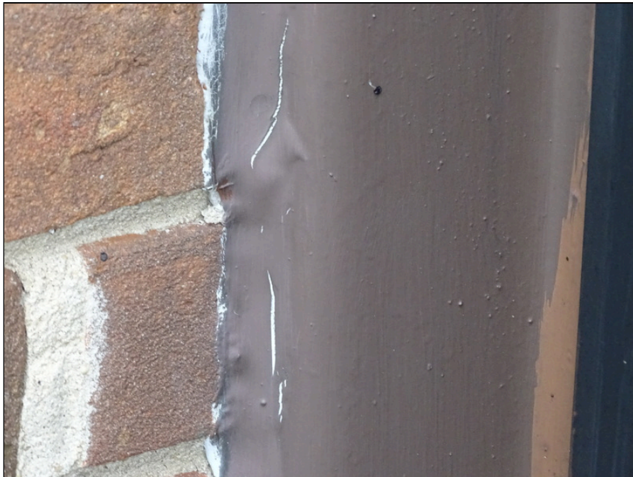
16 - Building exterior overview - note sealant deterioration
