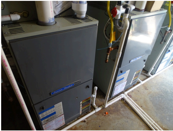
Gas furnace and air handler units
