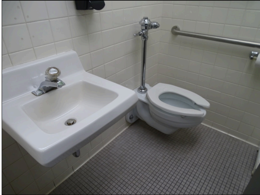
51 - Restroom without required accessible floor area
