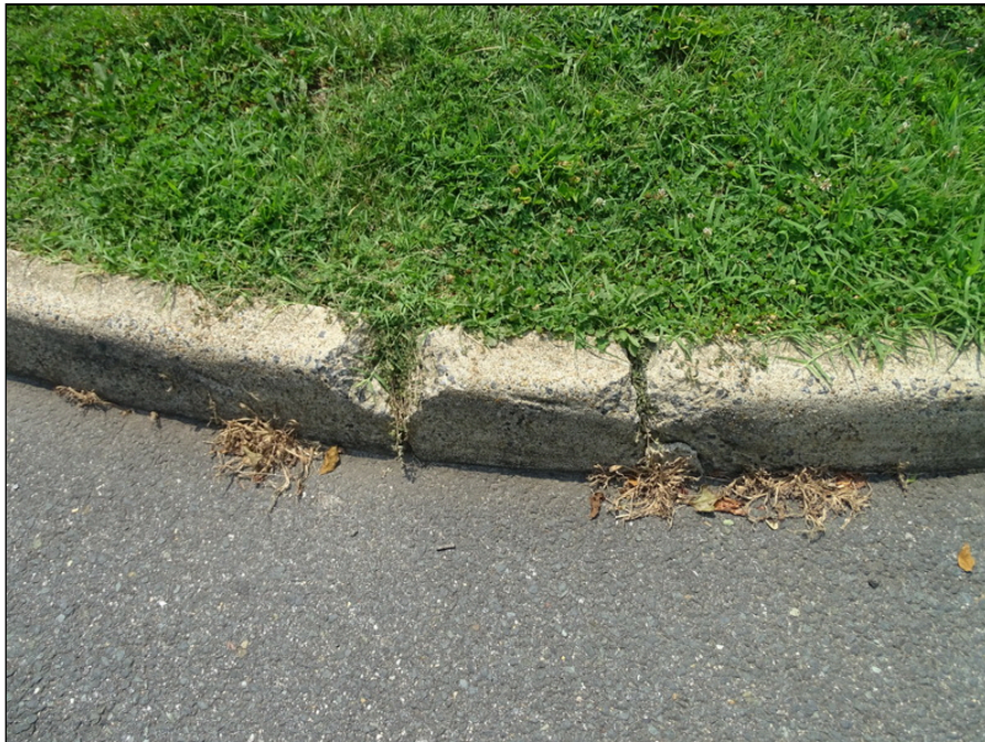
10 - Typical concrete curb - note deterioration
