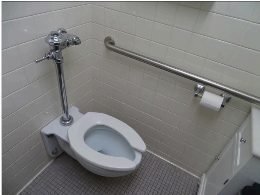
52 - Restroom without required accessible floor area
