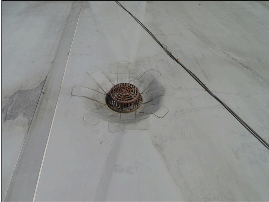
25 - Roof internal drain
