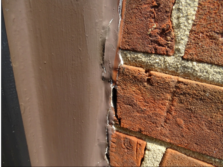
15 - Building exterior overview - note sealant deterioration
