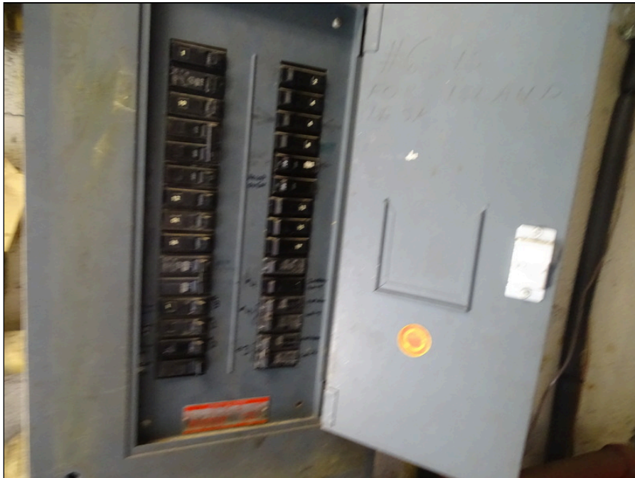
36 - Electrical panel - note missing components
