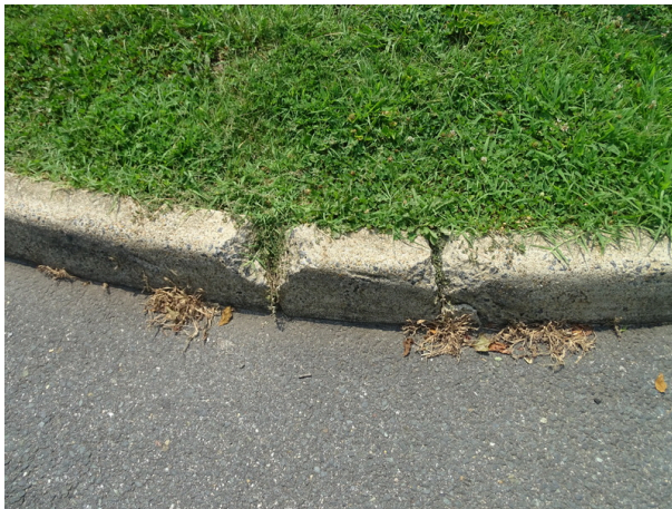
Typical concrete curb - note deterioration
