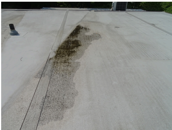
Roof overview - note ponding
