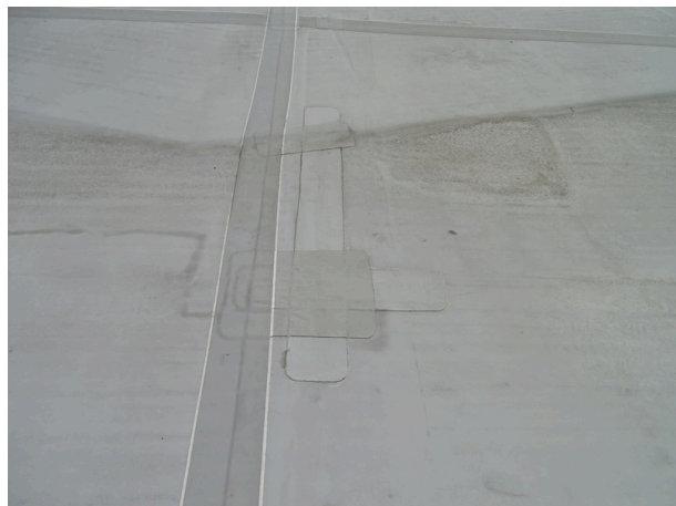
Roof overview - note patching
