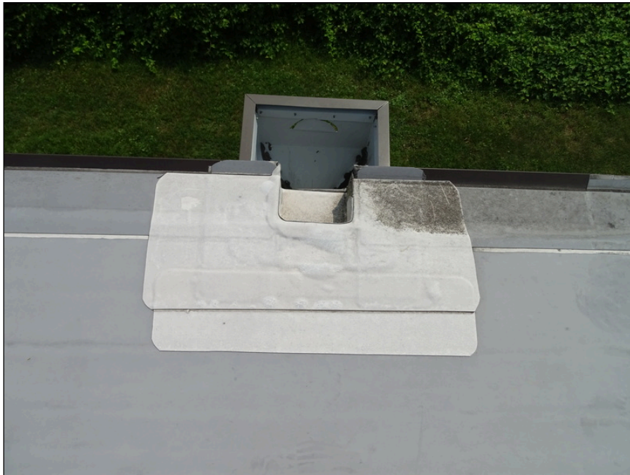
26 - Roof downspout
