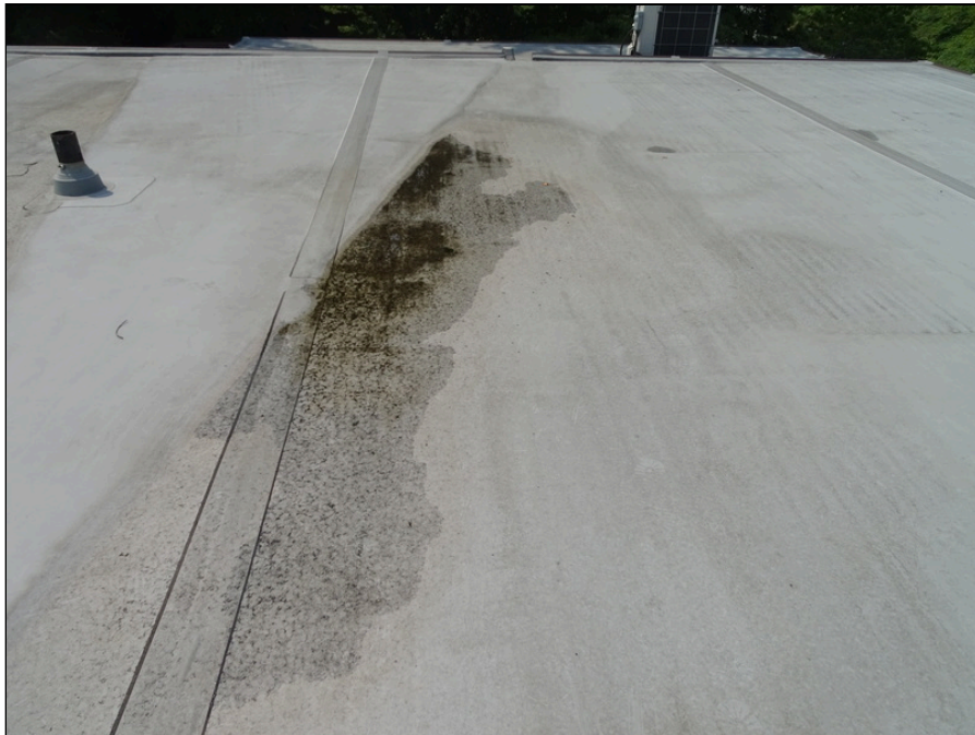
22 - Roof overview - note ponding
