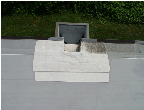
Roof downspout
