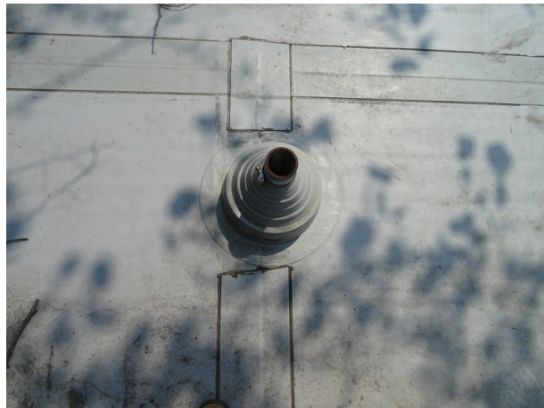
Typical plumbing penetration
