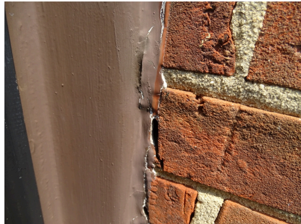
Building exterior overview - note sealant deterioration
