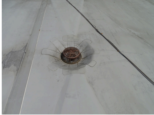
Roof internal drain
