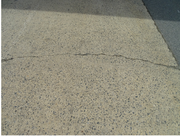
Cracked concrete sidewalk
