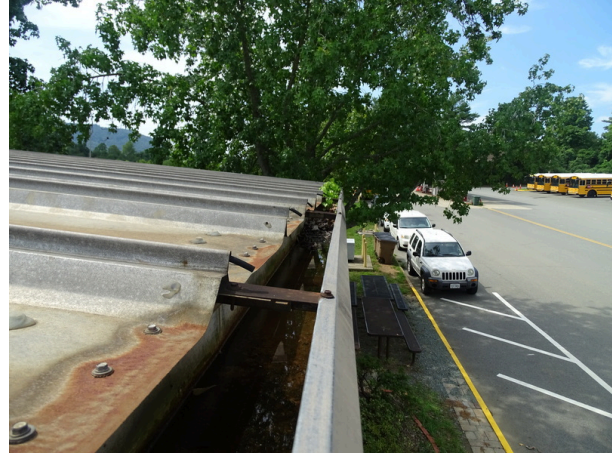
Metal gutter condition
