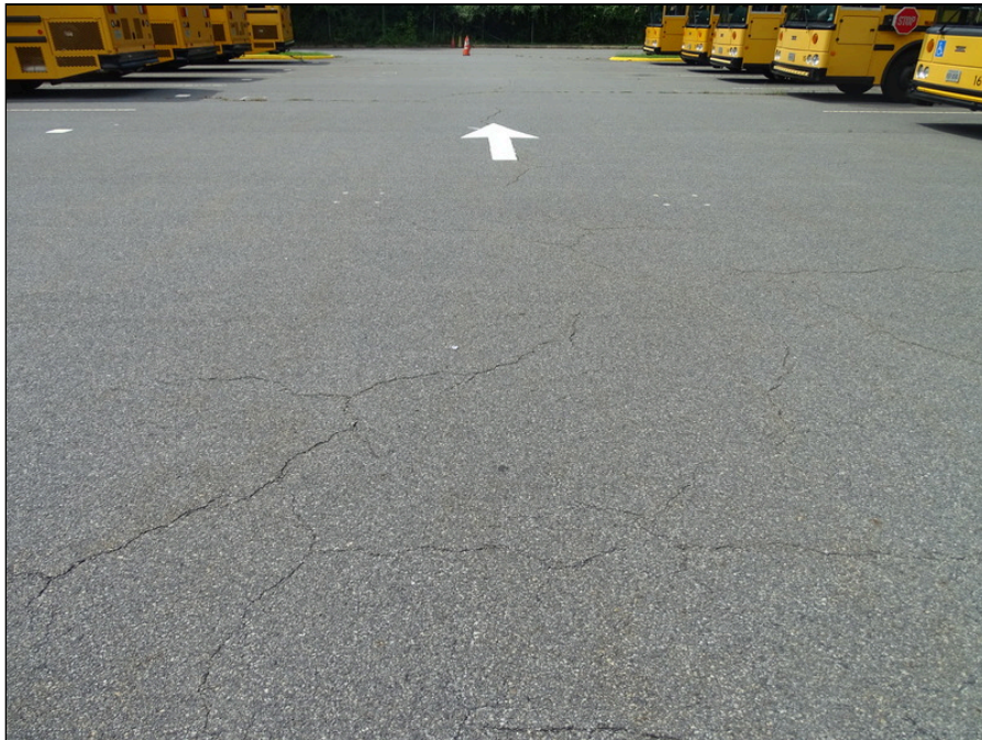
8 - Cracking in bus lot asphalt
