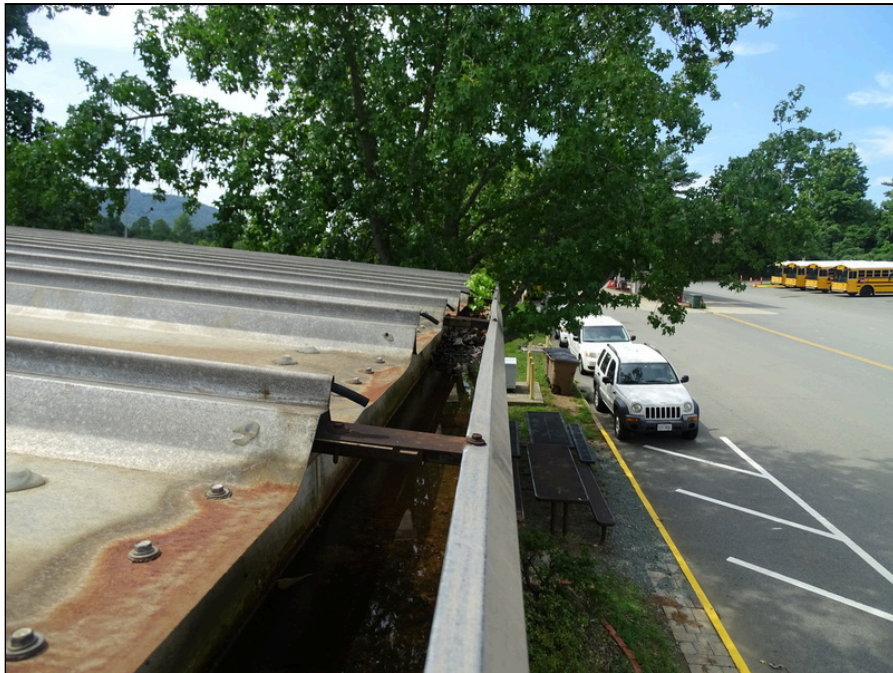
28 - Metal gutter condition
