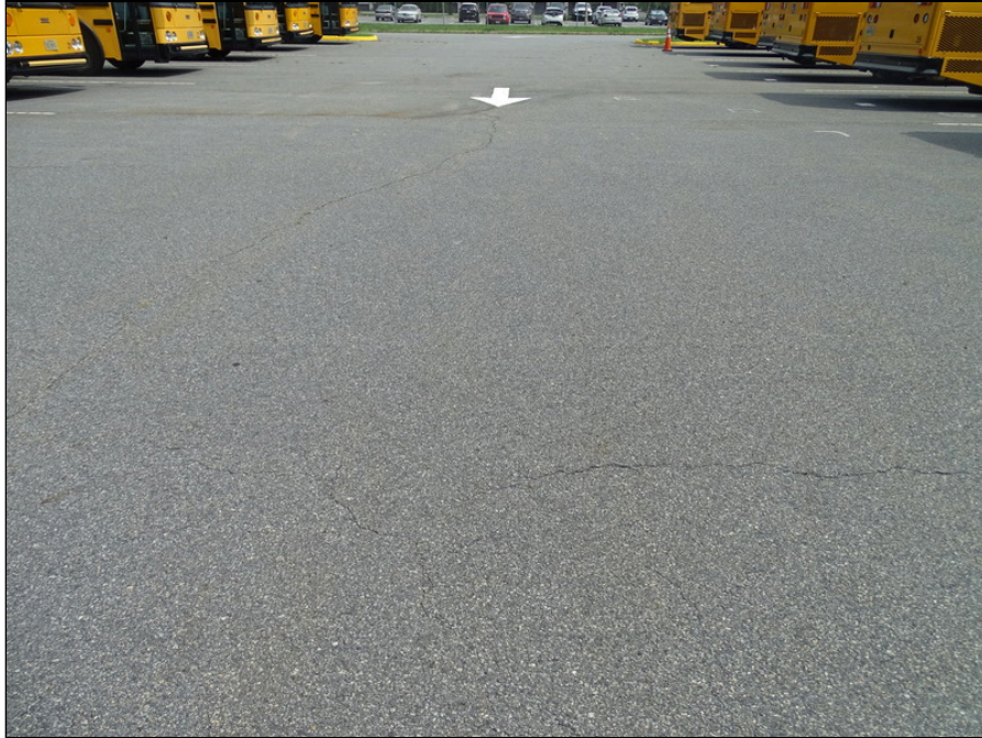
9 - Cracking in bus lot asphalt
