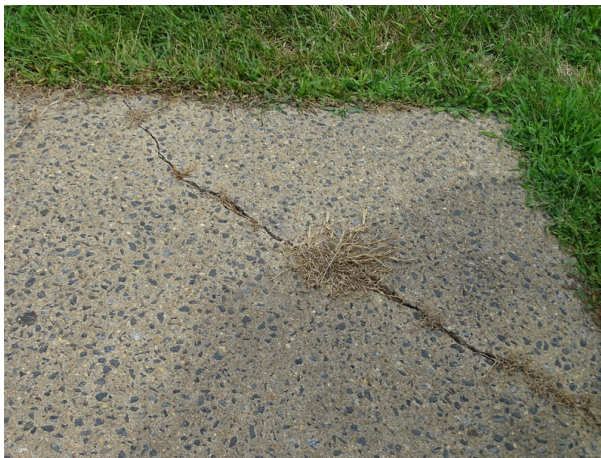
Cracked concrete sidewalk
