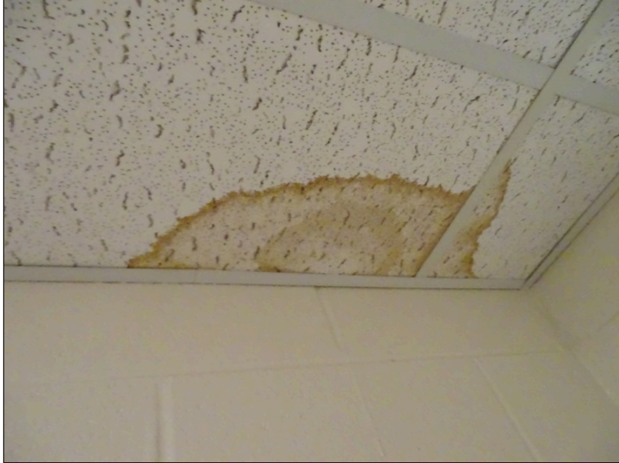
31 - Stained ceiling panel interior
