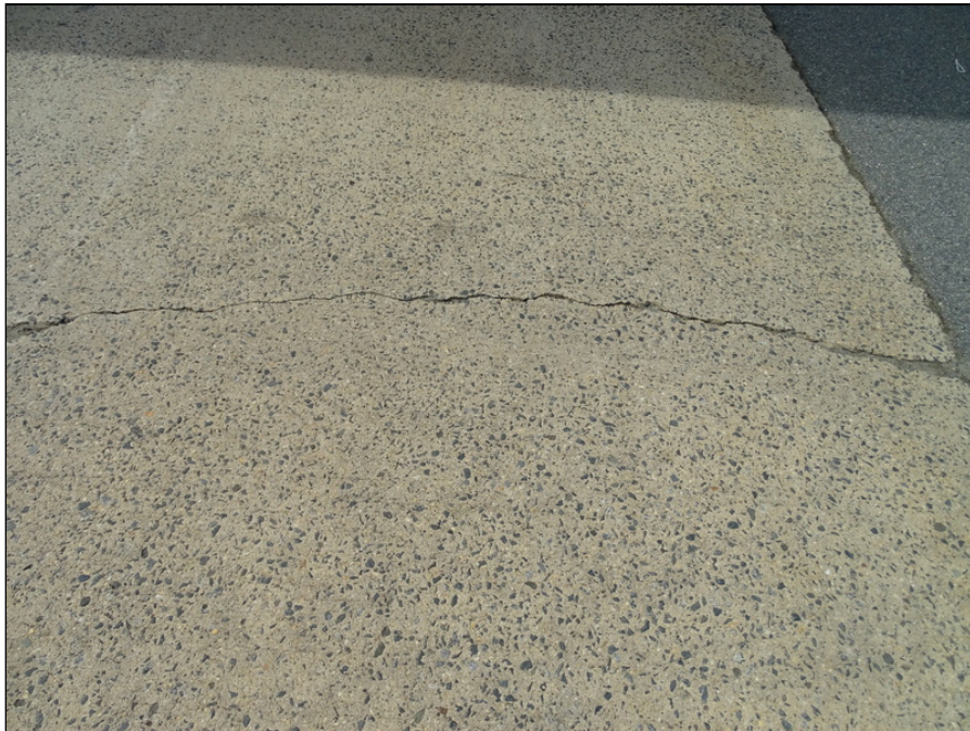
16 - Cracked concrete sidewalk
