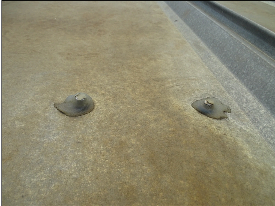
29 - Previous repair on roof top
