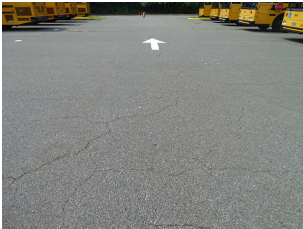
Cracking in bus lot asphalt
