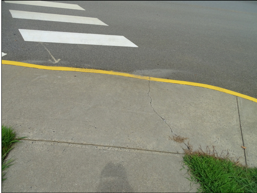
17 - Cracked sidewalk curb ramp
