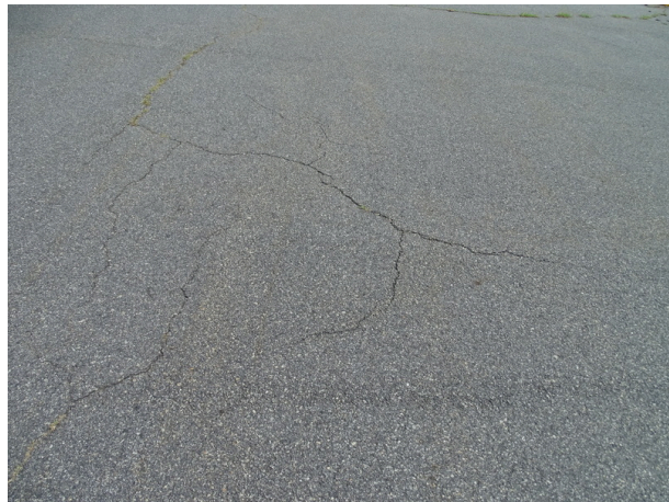
Cracking in bus lot asphalt
