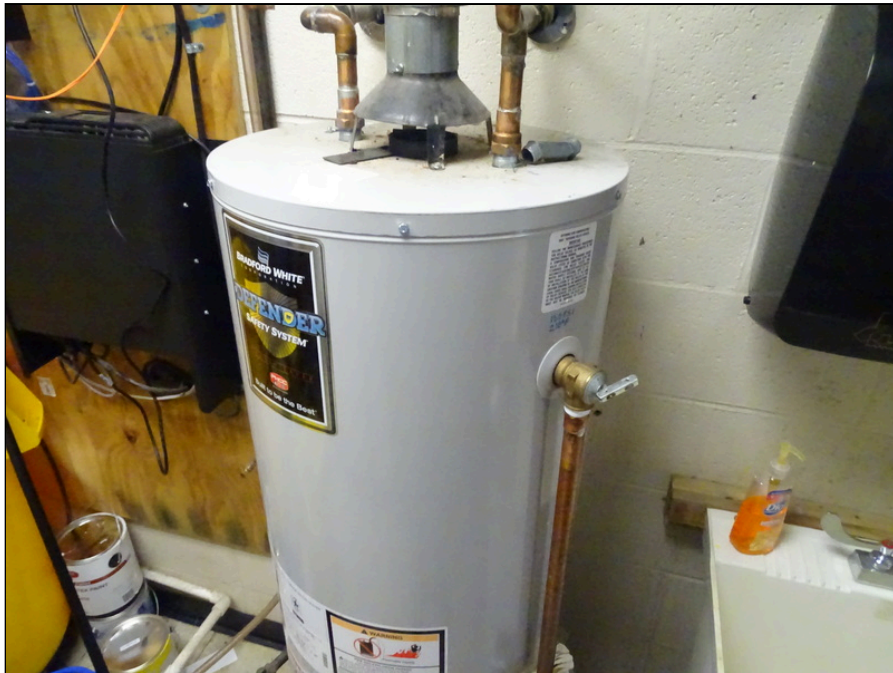
46 - Typical domestic water heater
