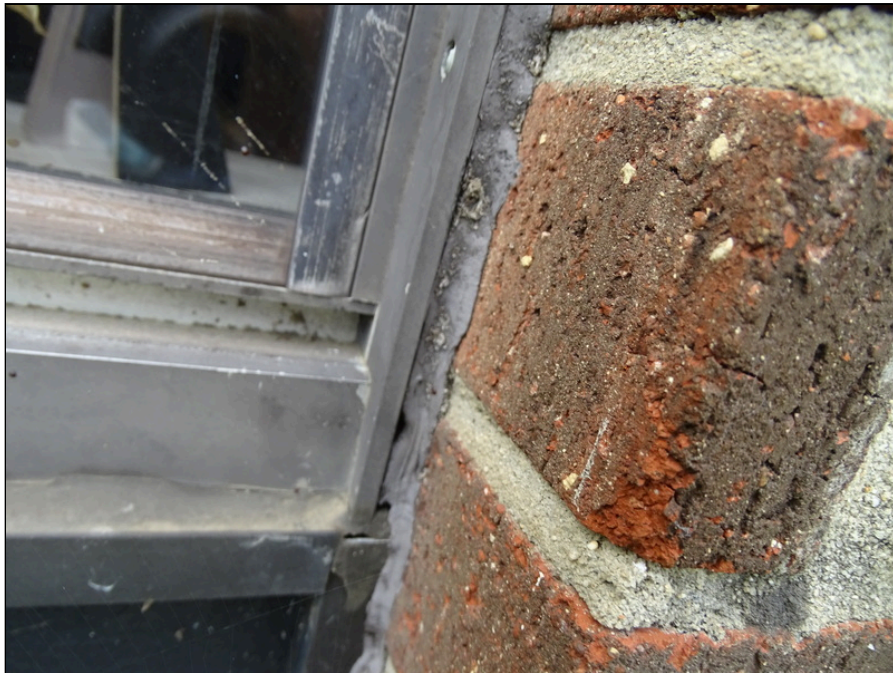
44 - Sealant around window
