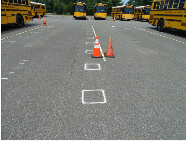
Cracking in bus lot asphalt
