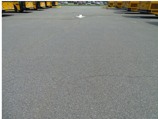
Cracking in bus lot asphalt
