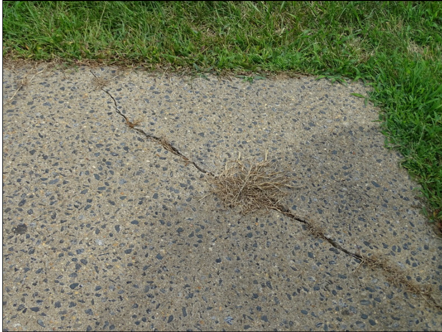
15 - Cracked concrete sidewalk
