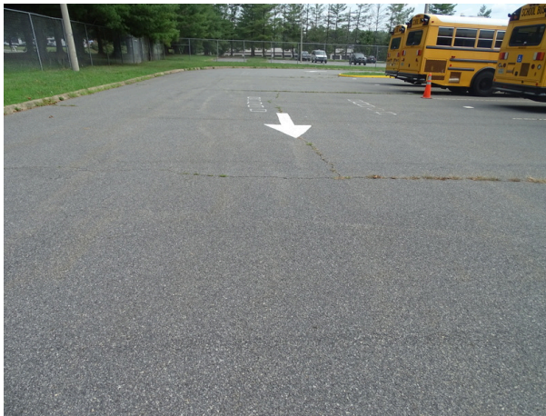
Cracking asphalt and curb
