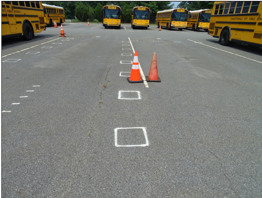
10 - Cracking in bus lot asphalt
