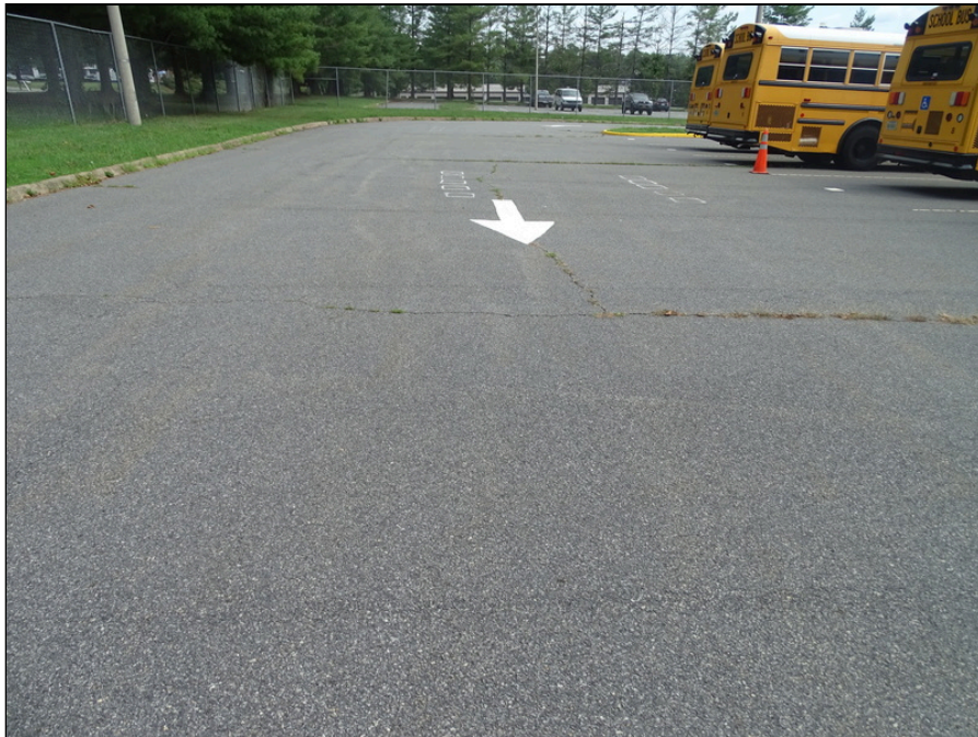
12 - Cracking in bus lot asphalt
