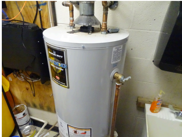
Typical gas domestic water heater
