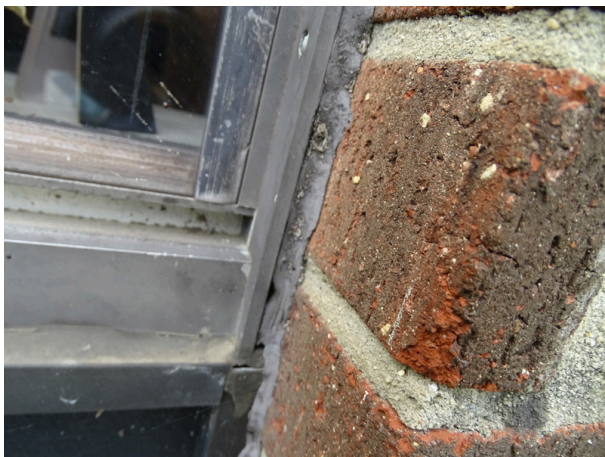
Sealant around window
