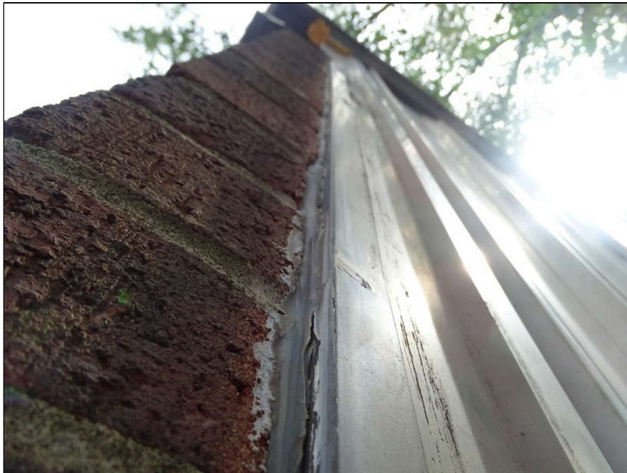
36 - Sealant condition around metal siding wall
