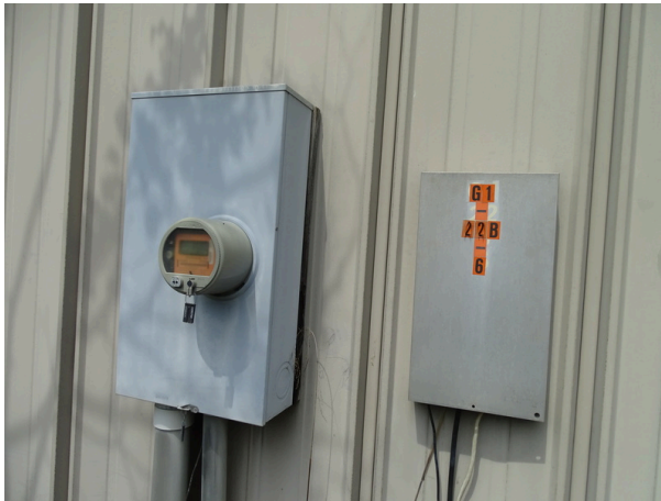
Typical electric meter
