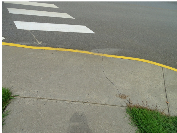
Cracked sidewalk
