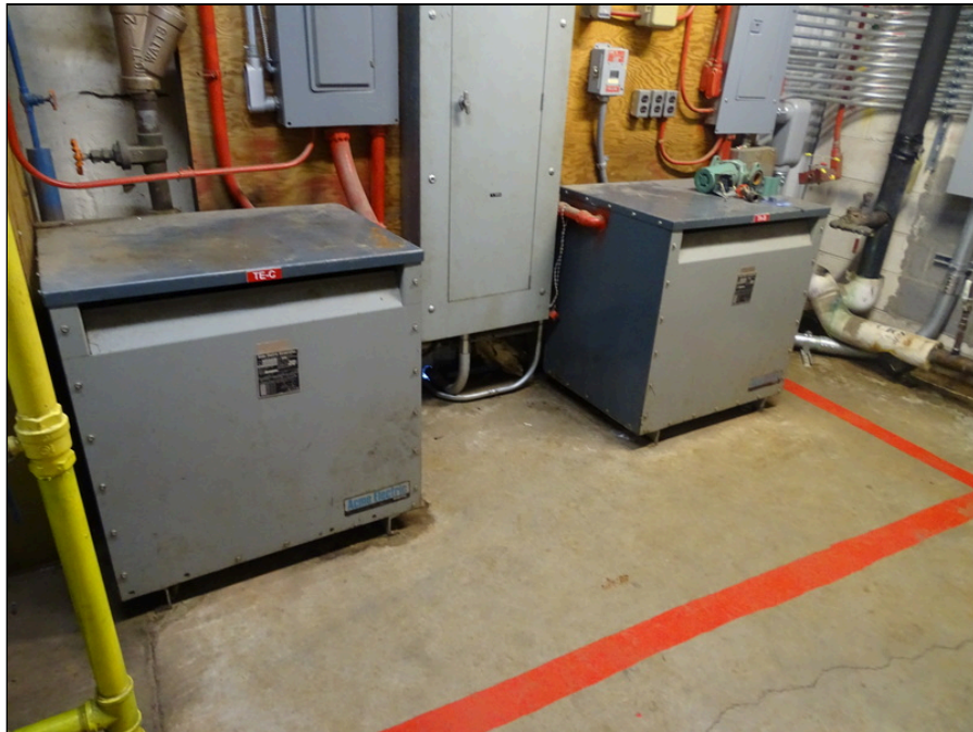
48 - Typical building transformer
