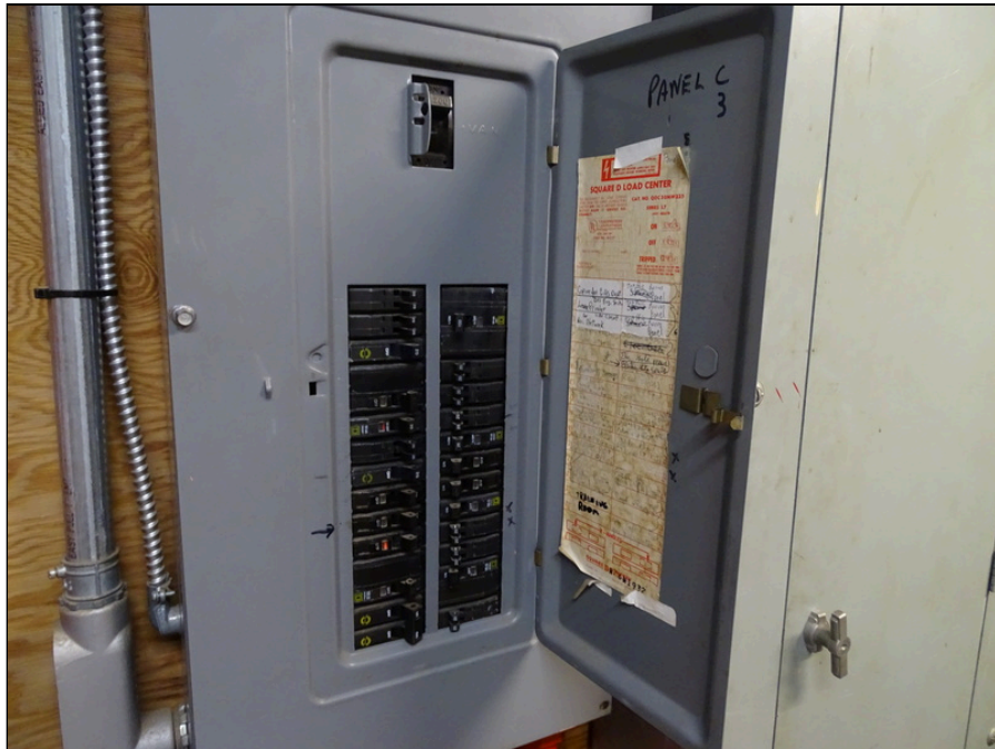
46 - Typical circuit breaker panel
