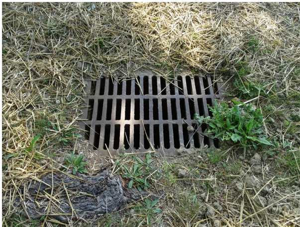
Typical yard inlet drainage
