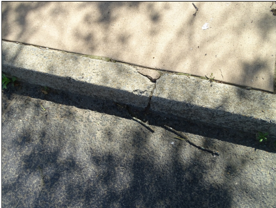
12 - Typical concrete sidewalk - note cracking
