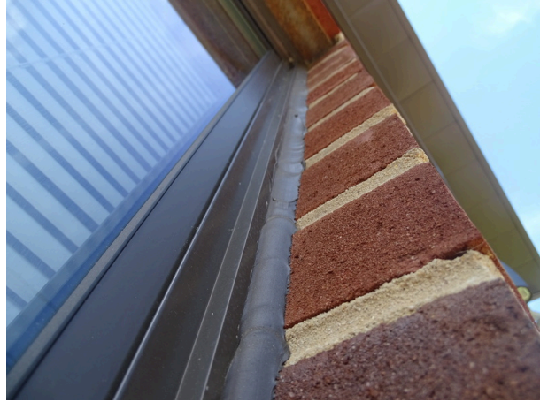
Typical exteriors - note sealant deterioration
