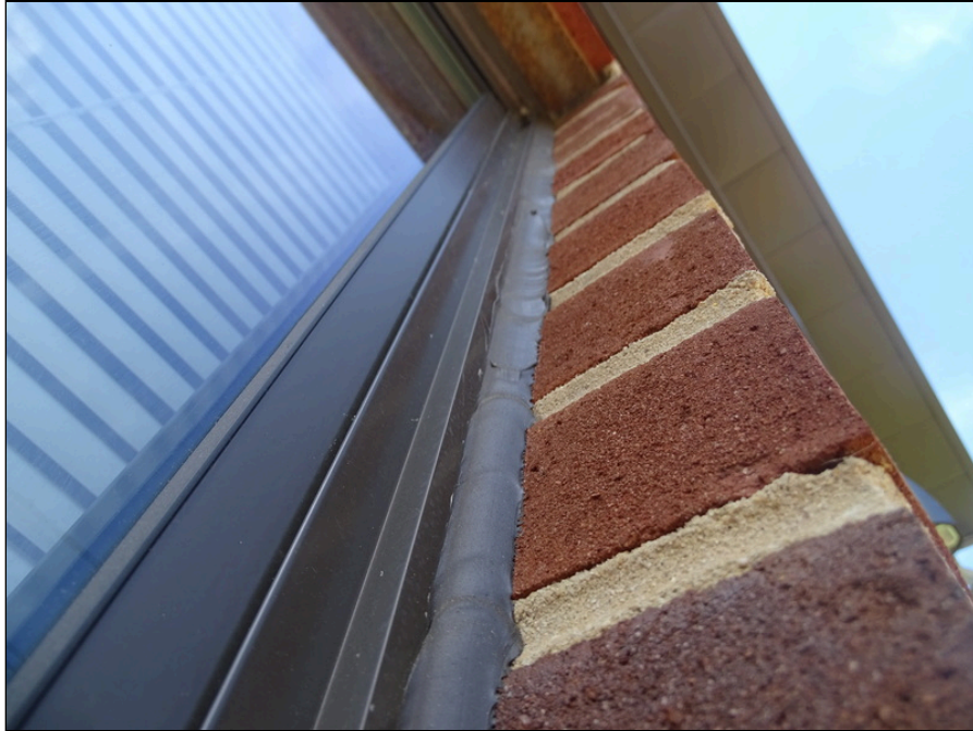
29 - Typical exteriors - note sealant deterioration
