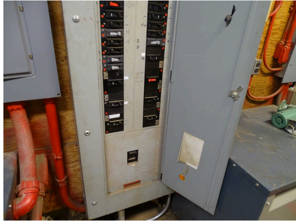
Main electrical switchgear
