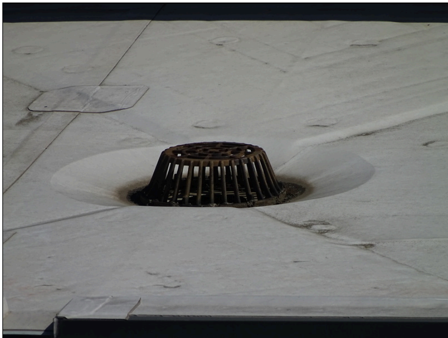
32 - Typical internal drain
