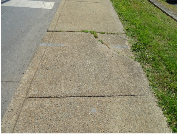
Typical concrete sidewalk - note cracking
