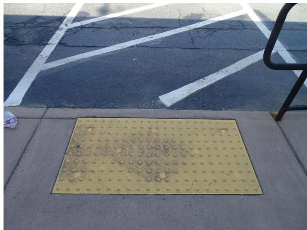
Accessible curb ramp with truncated domes
