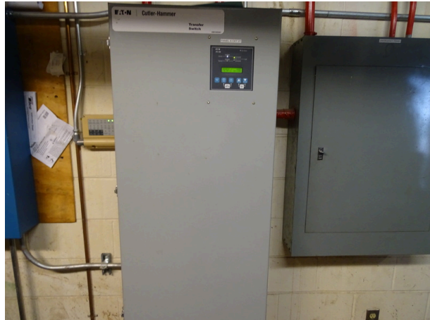
Emergency power transfer switch
