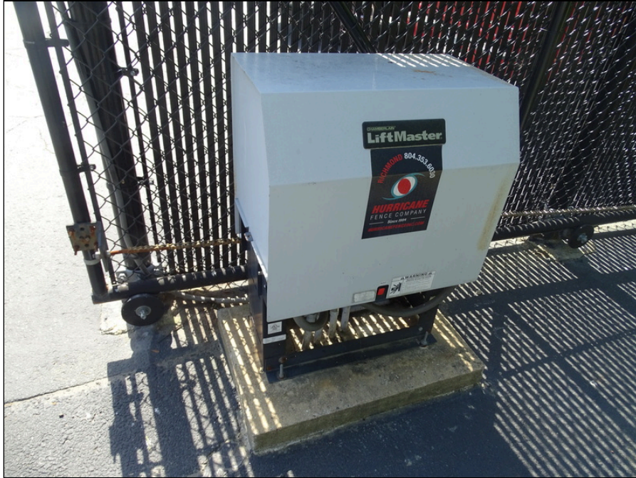
19 - Typical fences controller system
