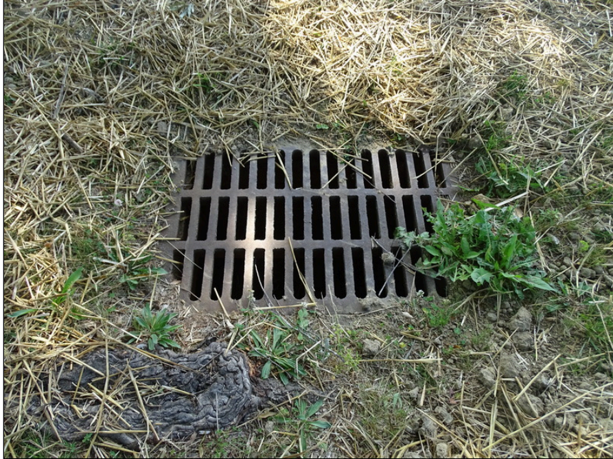
5 - Typical yard inlet drainage
