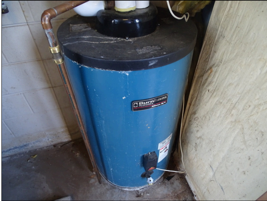
35 - Boiler system domestic hot water supply
