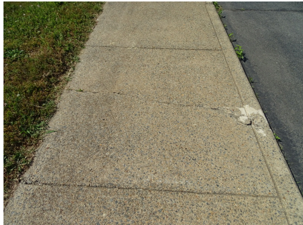
Typical concrete sidewalk - note cracking
