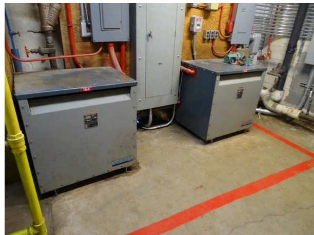
Typical building transformer
