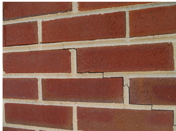
Typical building exterior - note step cracking and deterioration of mortar
