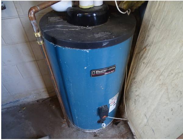
Boiler system domestic hot water supply
