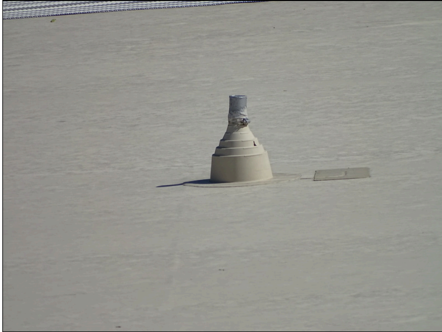
33 - Typical plumbing penetration
