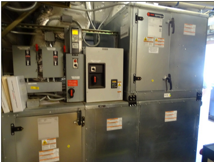
38 - Air Handler Unit located in main utility room
