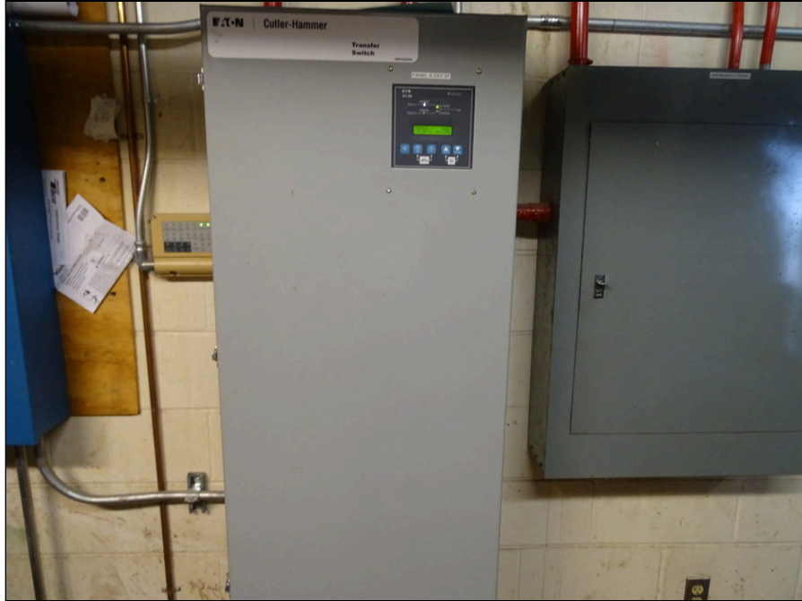
45 - Emergency power transfer switch
