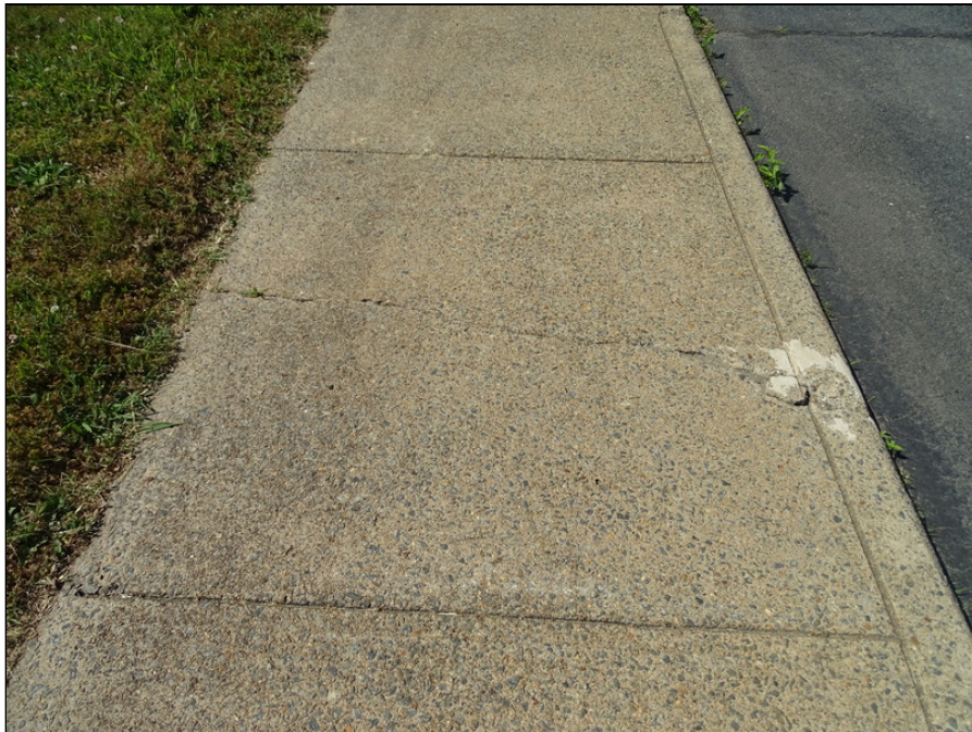
10 - Typical concrete sidewalk - note cracking
