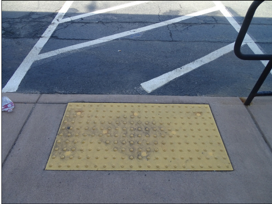
65 - Curb ramp with truncated domes
