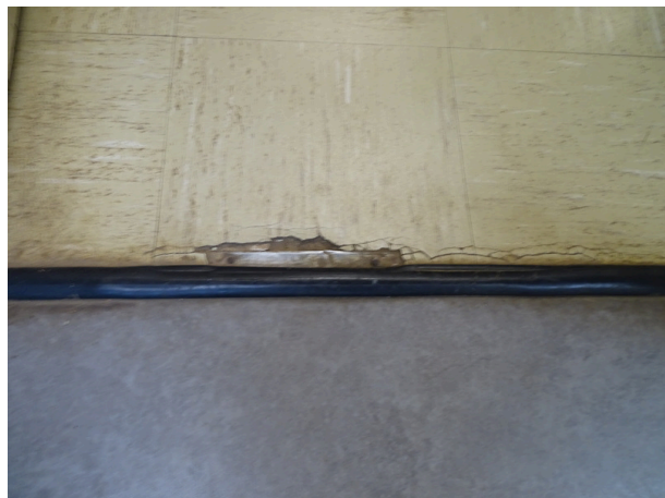
Interior finishes of restroom area - note deterioration
