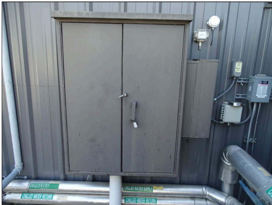
42 - Main electrical service and utility meter
