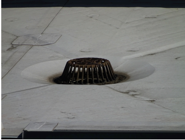
Typical internal drain
