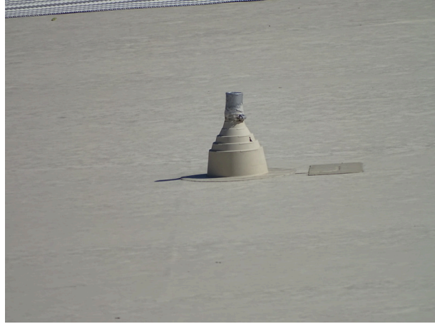
Typical plumbing penetration
