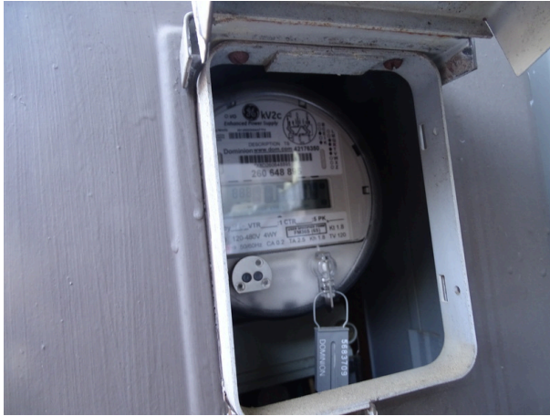
Typical electrical meter
