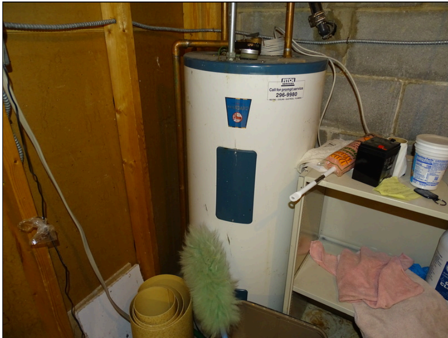
24 - Electric domestic water heater
