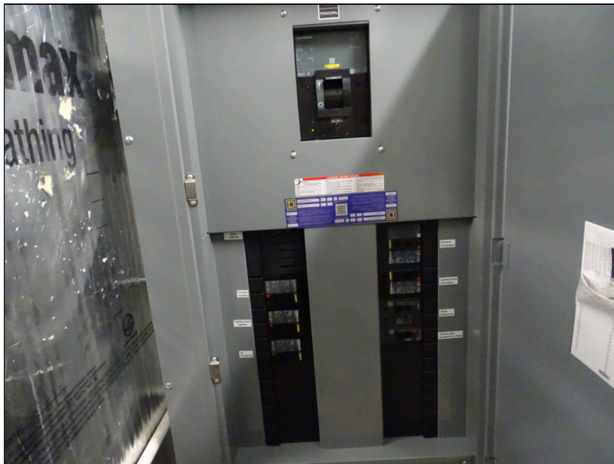
34 - Main electrical disconnect
