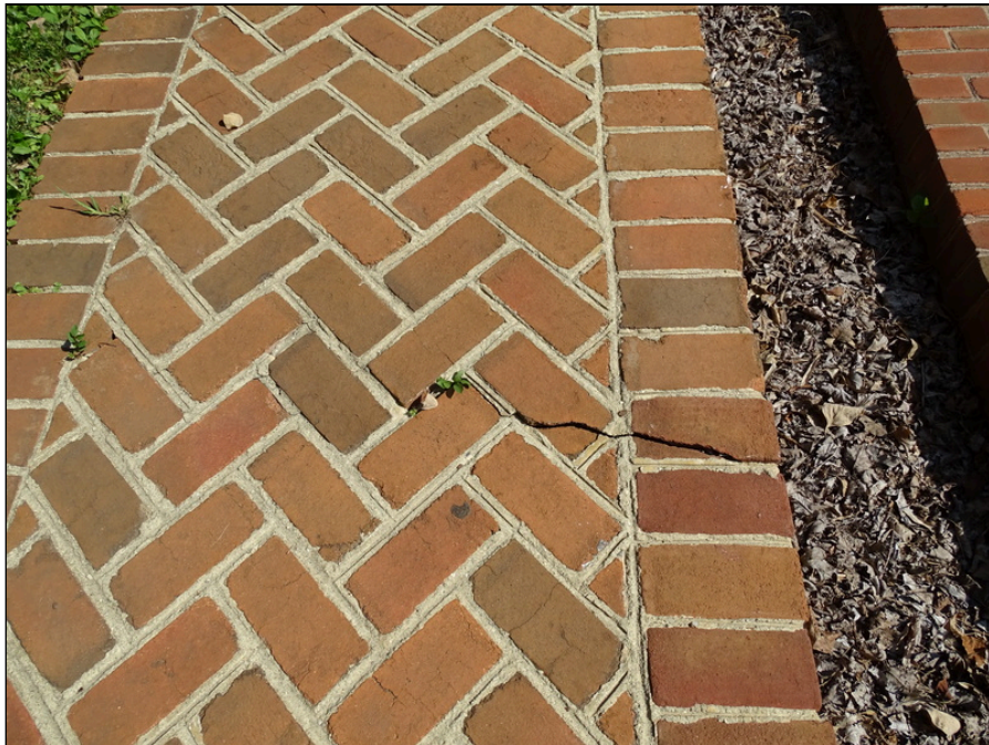
4 - Cracked brick sidewalk at south side of building
