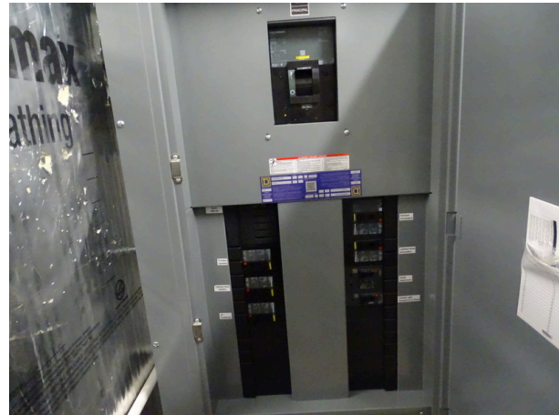
Main electrical disconnect
