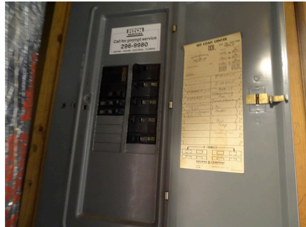
Typical circuit breaker panel manufactured by Square D
