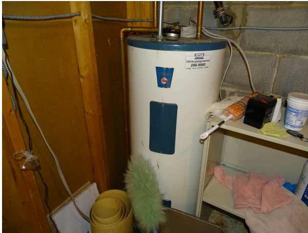
Electric domestic water heater
