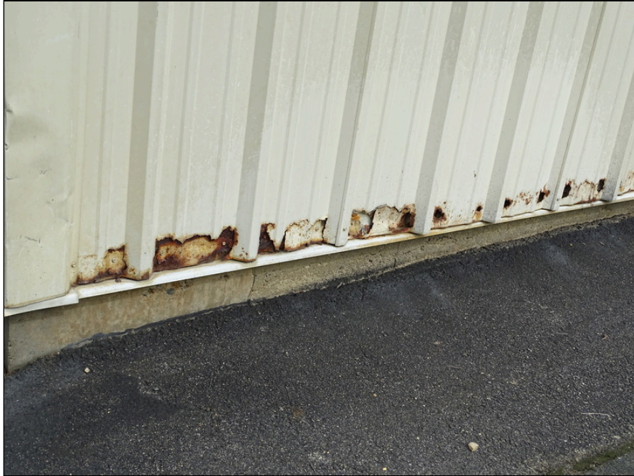
29 - Parks Shop windows and corrosion at base of metal panels
