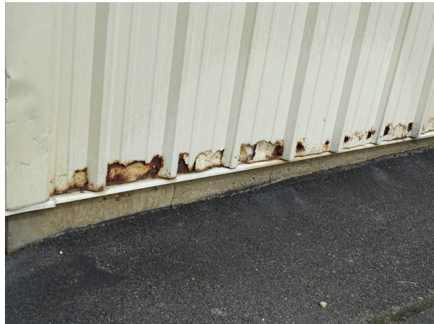
Parks Shop windows and corrosion at base of metal panels
