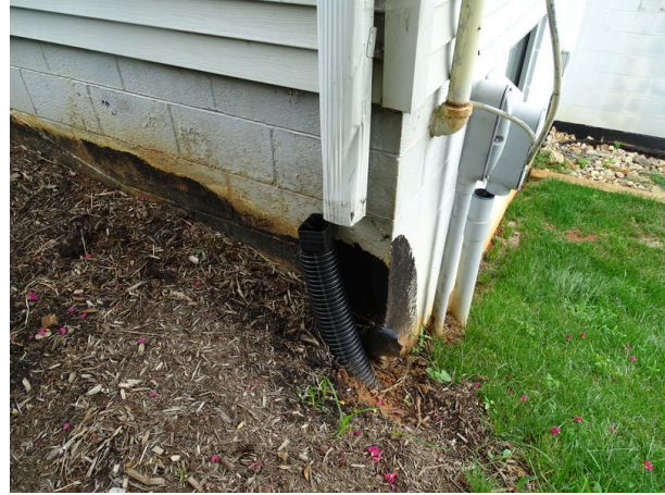
Division office typical downspout deterioration
