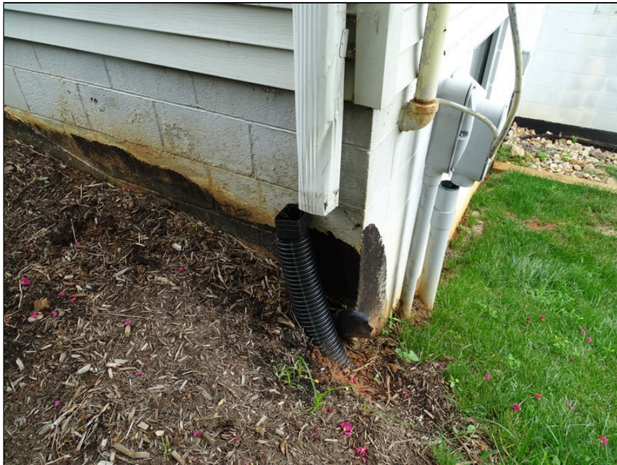
80 - Division office typical downspout deterioration
