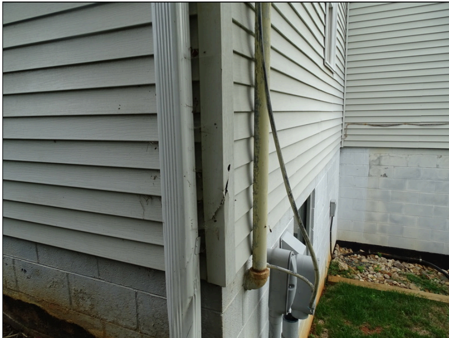
22 - Division Office damaged siding
