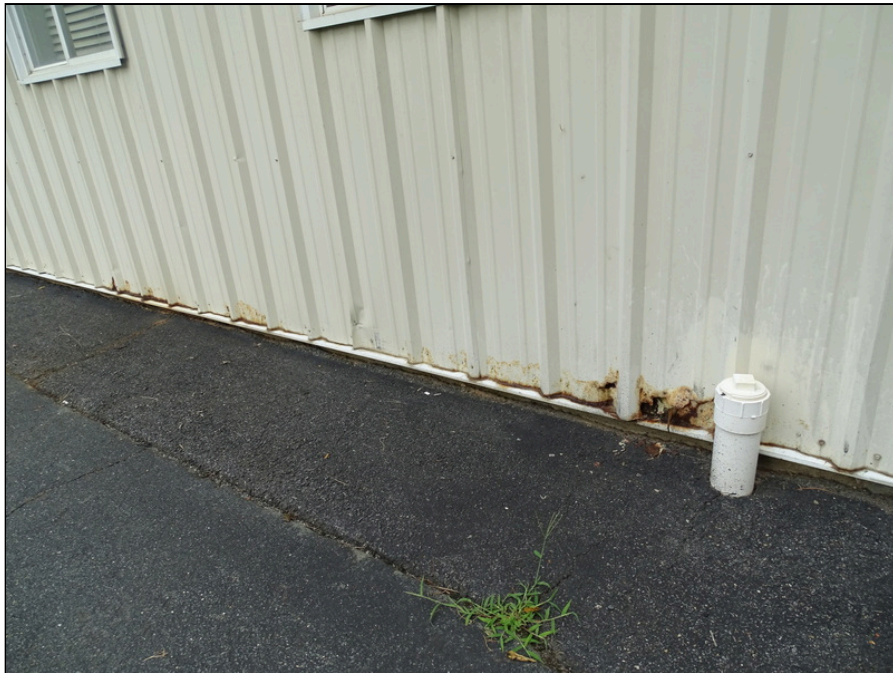
30 - Parks Shop windows and corrosion at base of metal panels
