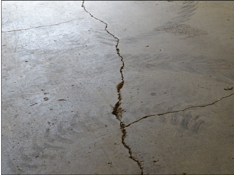
15 - Parks shop slab on-grade crack
