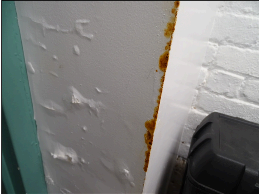
55 - Typical wall - note efflorescence
