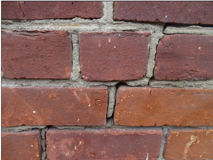
8 - Typical building exterior - note step cracking at brick
