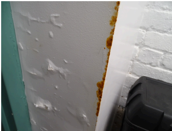
Typical wall - note efflorescence
