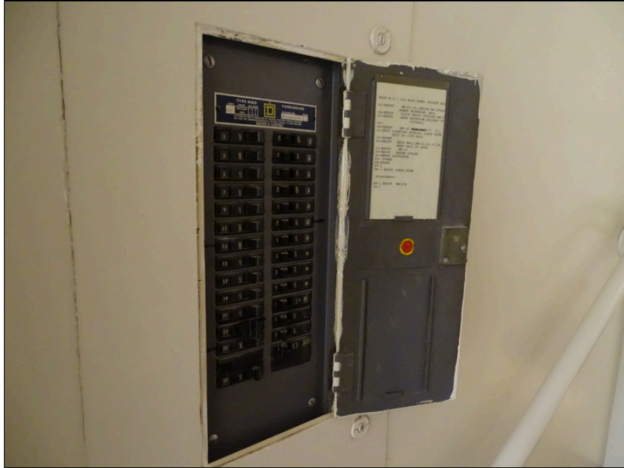
31 - Older circuit breaker panel
