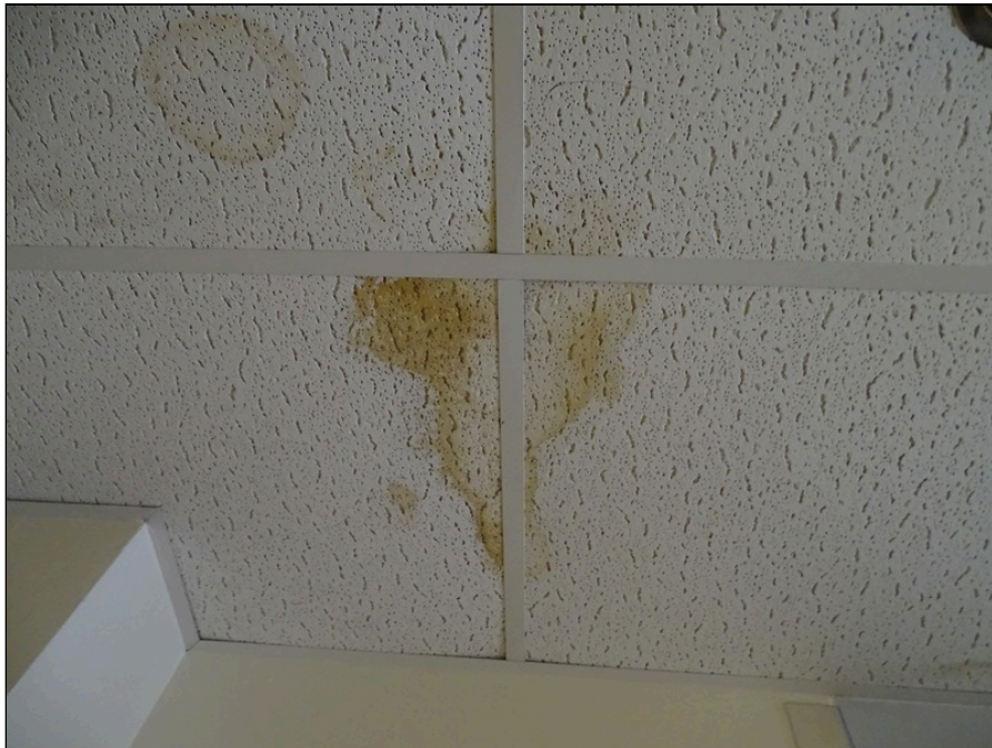
28 - Water leakage at ceiling
