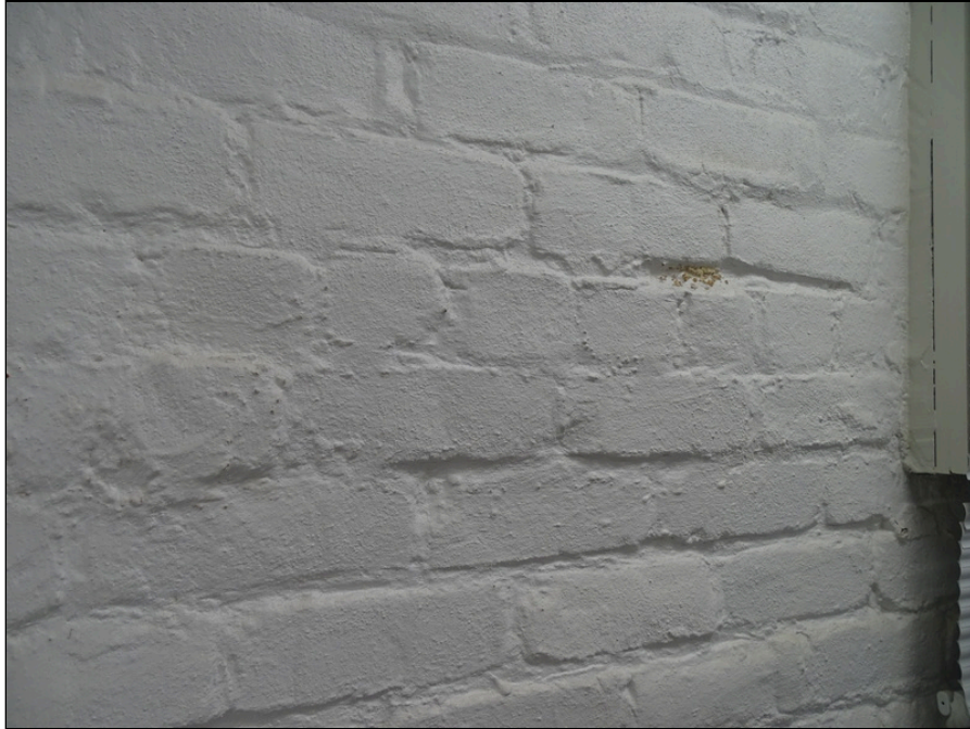
53 - Typical wall - note efflorescence
