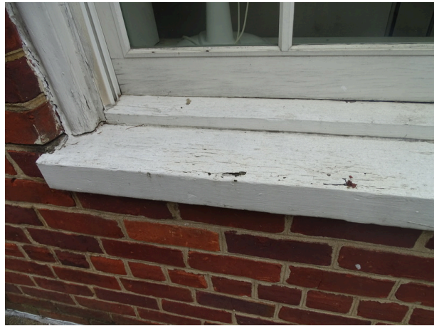
Exterior window - note deterioration
