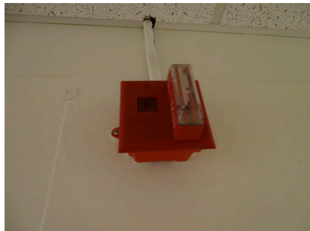
Typical fire alarm bell and strobe
