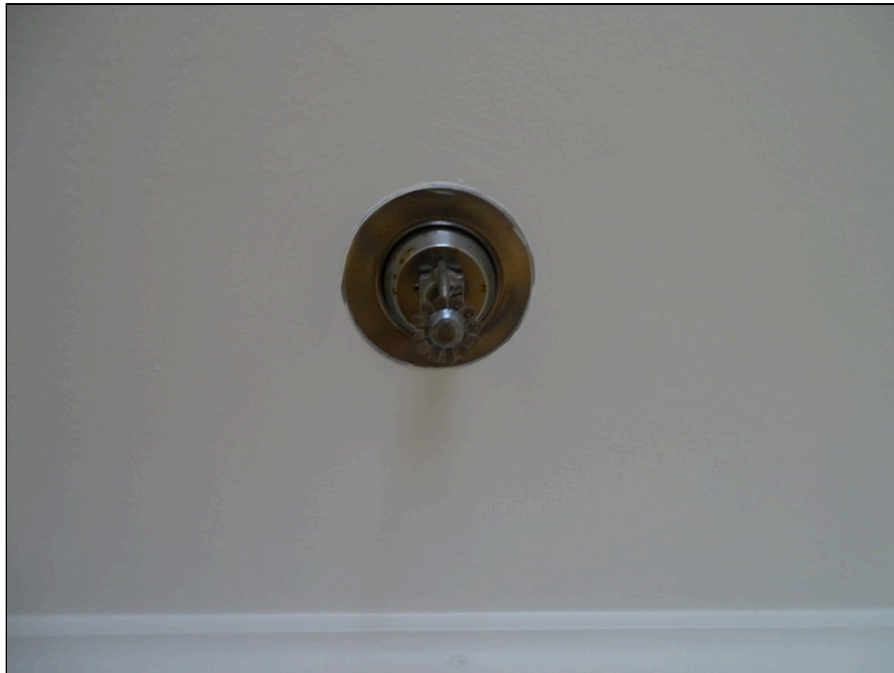
34 - Typical sprinkler head
