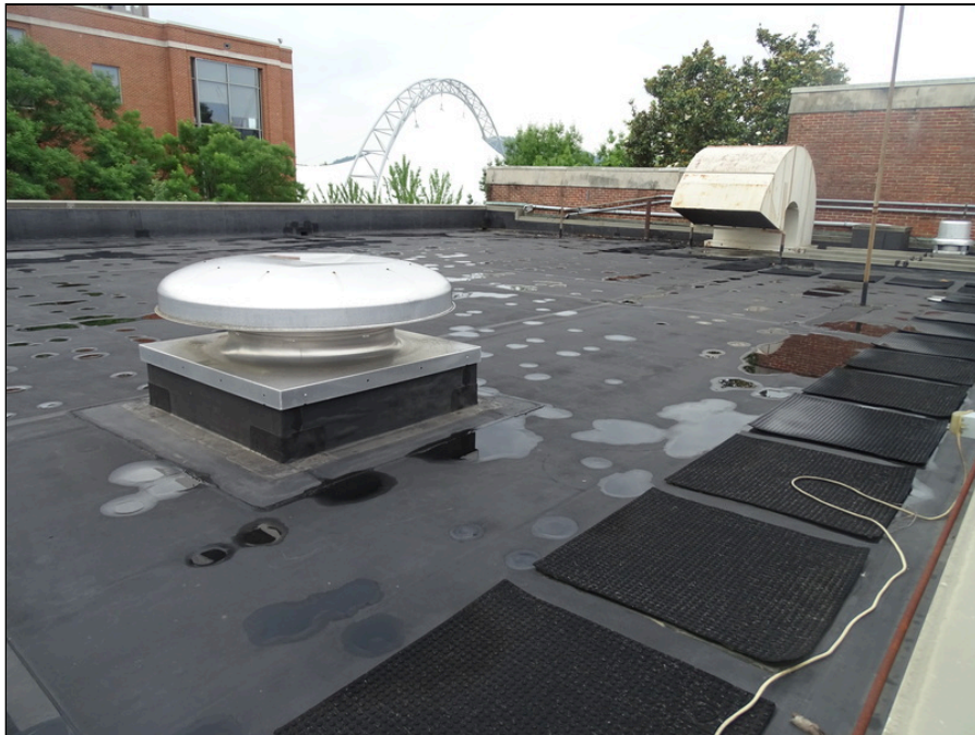
22 - Single-ply membrane roofing system looking north
