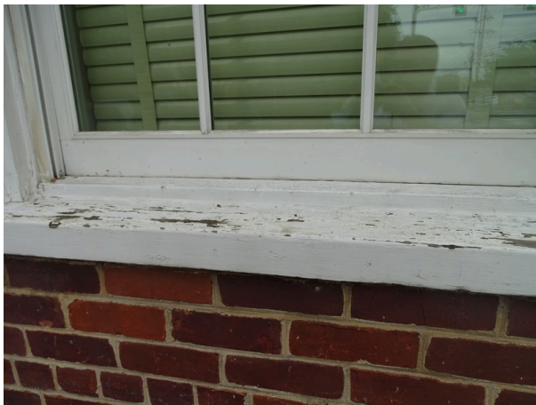
Exterior window - note deterioration
