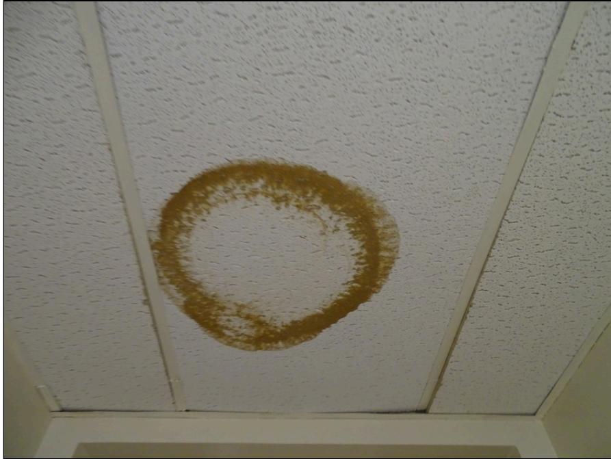
27 - Water leakage at ceiling
