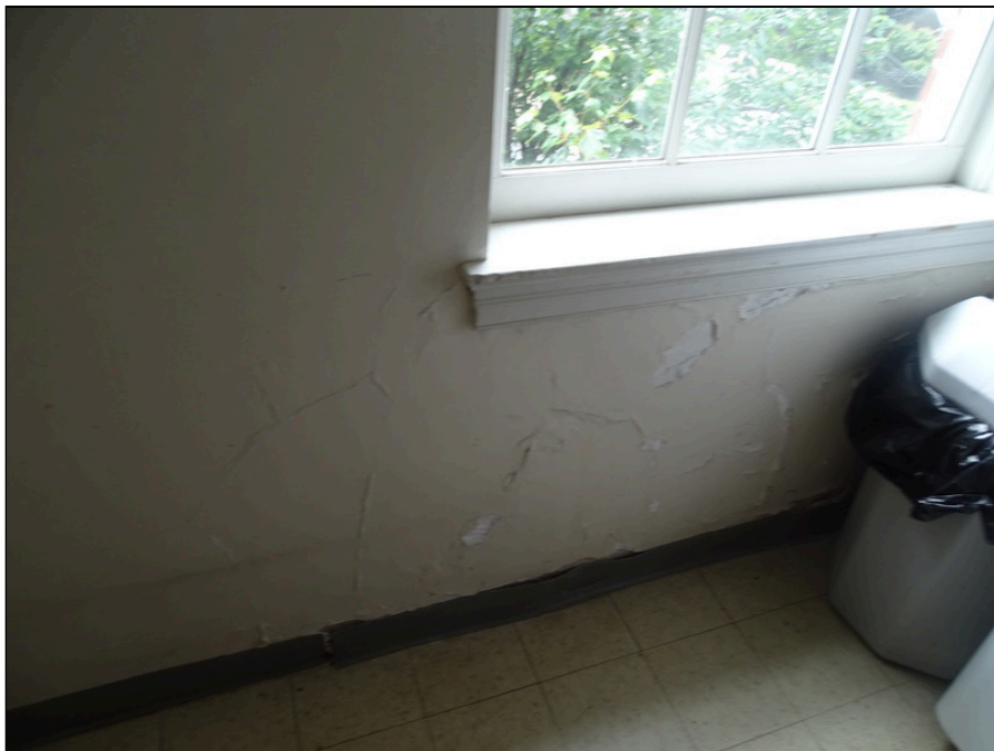
20 - Exterior window - note leakage
