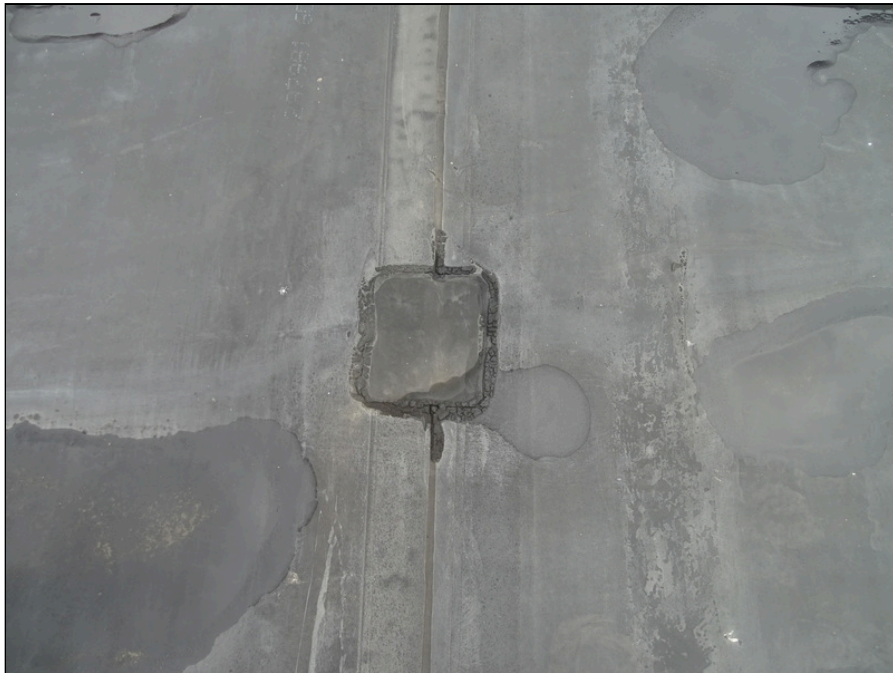
26 - Single-ply membrane roofing system - note patching
