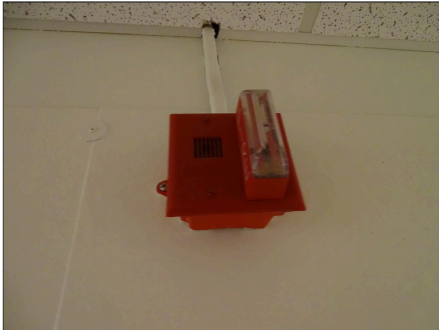
38 - Typical fire alarm bell and strobe
