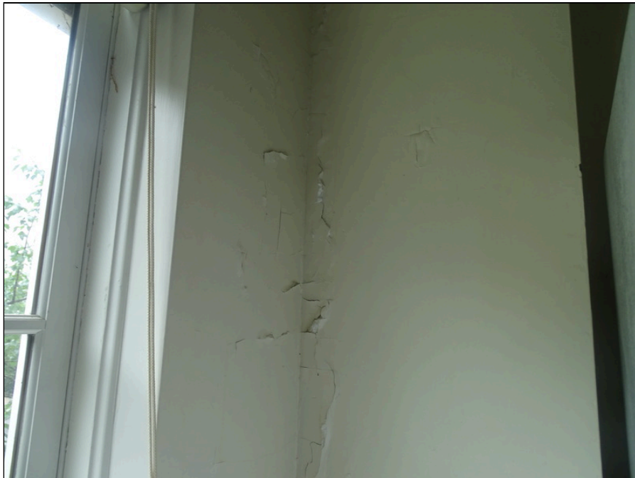
56 - Typical wall - note efflorescence
