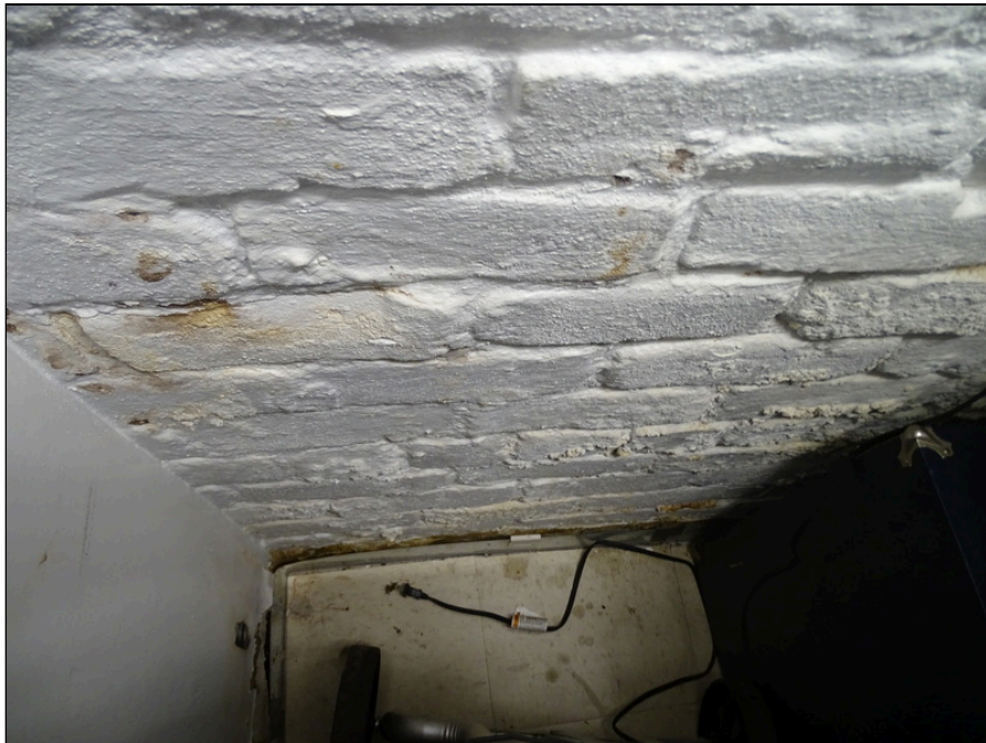
54 - Typical wall - note efflorescence
