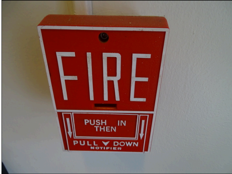
37 - Typical fire alarm pull station
