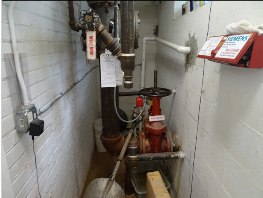
33 - Fire sprinkler system
