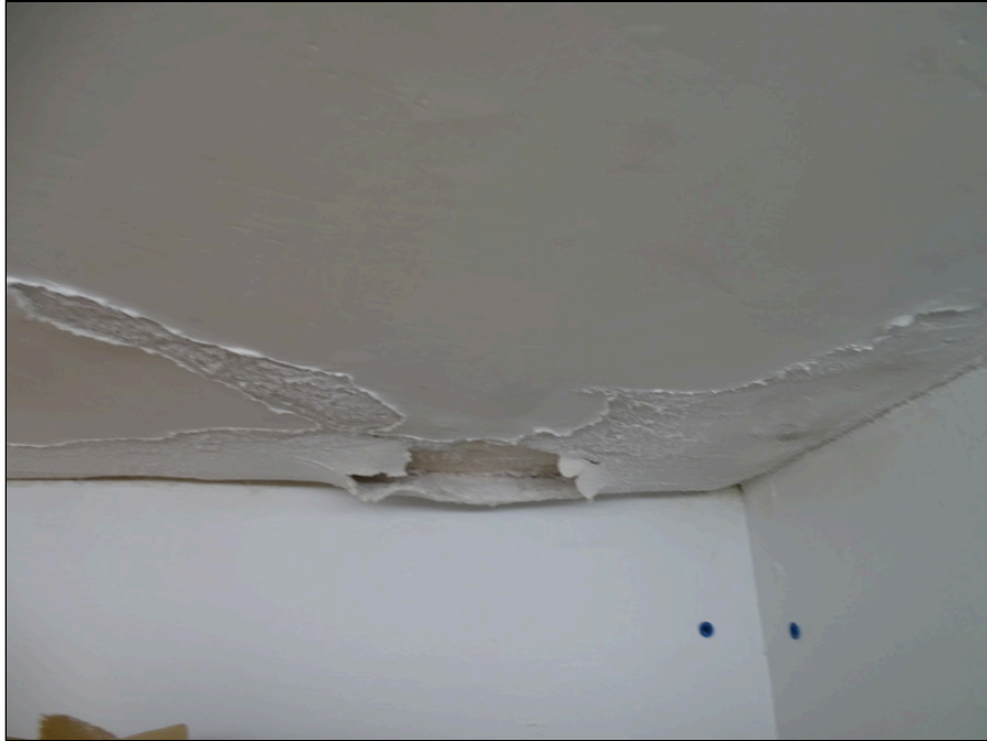
29 - Water leakage at ceiling
