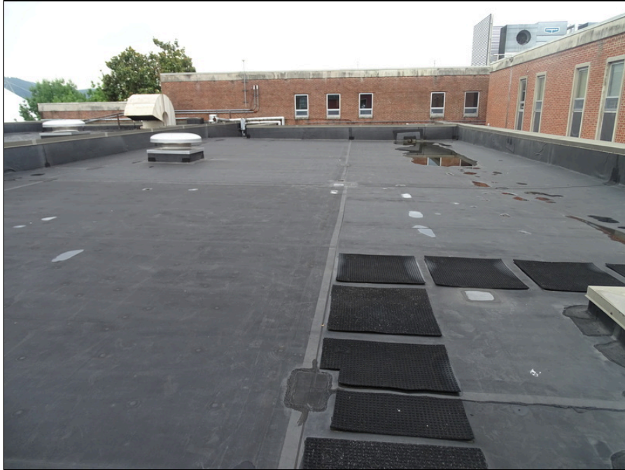
21 - Single-ply membrane roofing system looking north
