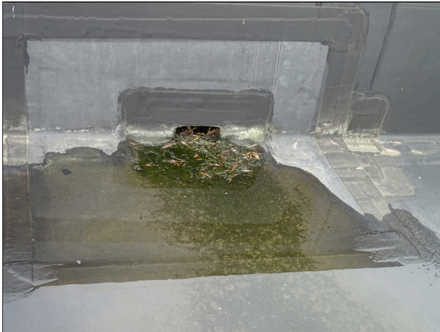
24 - Typical through wall scupper drain - note ponding
