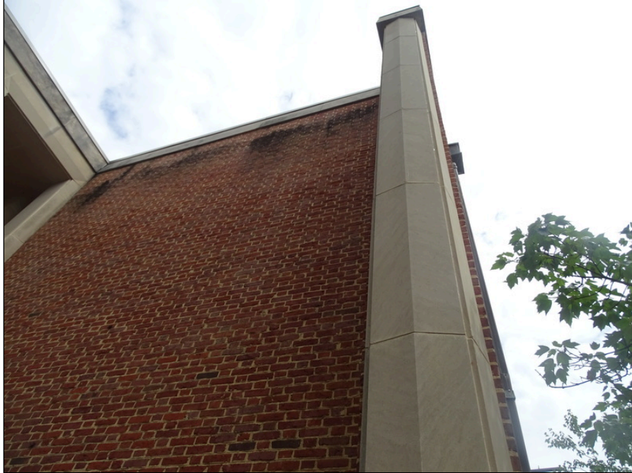
7 - Typical building exterior - note efflorescence
