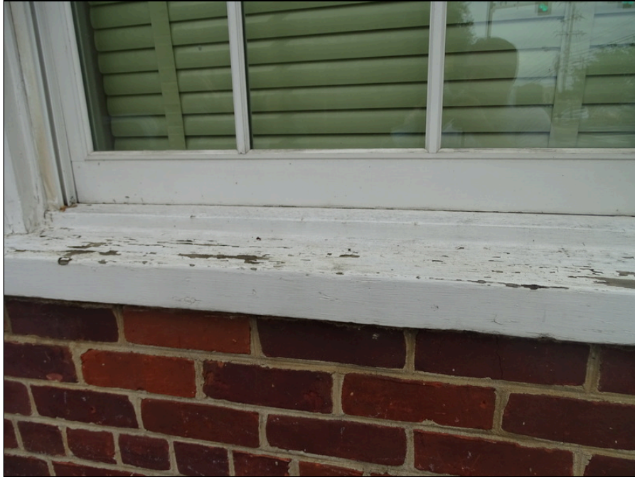
19 - Exterior window - note deterioration
