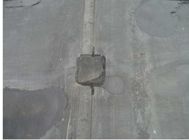
Single-ply membrane roofing system - note patching
