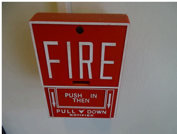
Typical fire alarm pull station
