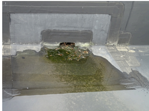
Typical through wall scupper drain - note ponding
