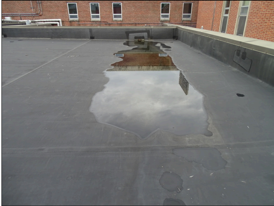
23 - Single-ply membrane roofing system looking south - note ponding
