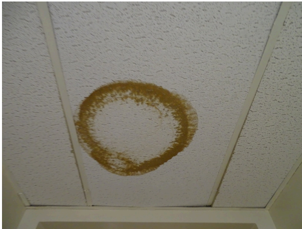
Water leakage at ceiling
