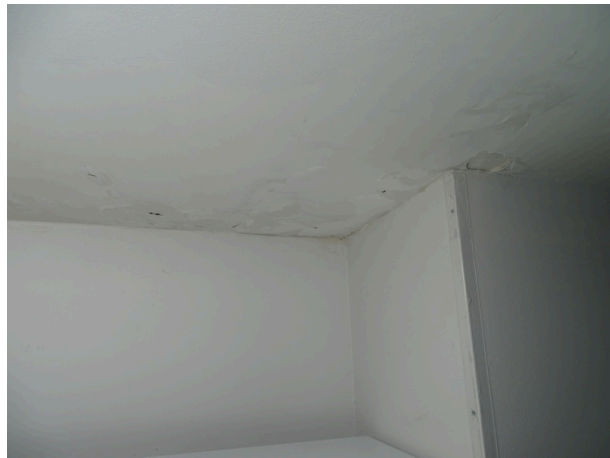
Water leakage at ceiling
