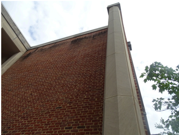
Typical building exterior - note efflorescence
