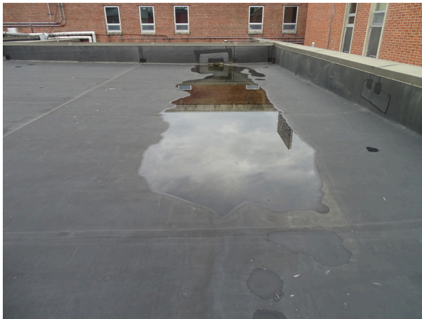
Single-ply membrane roofing system looking south - note ponding
