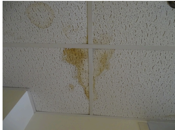
Water leakage at ceiling
