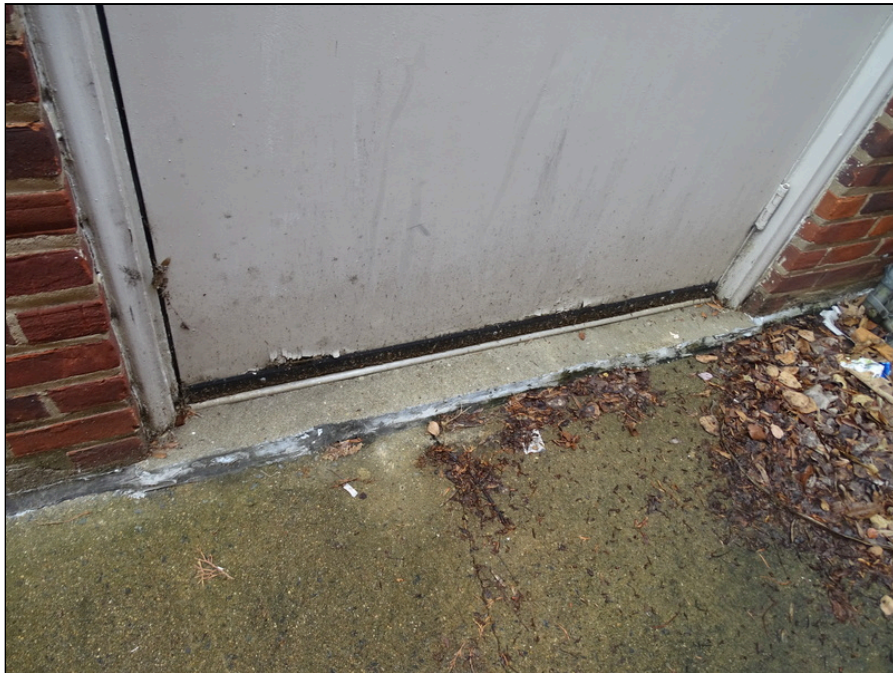
16 - Typical steel personal door - note peeling paint
