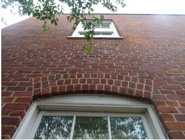
Typical building exterior - note step cracking at brick
