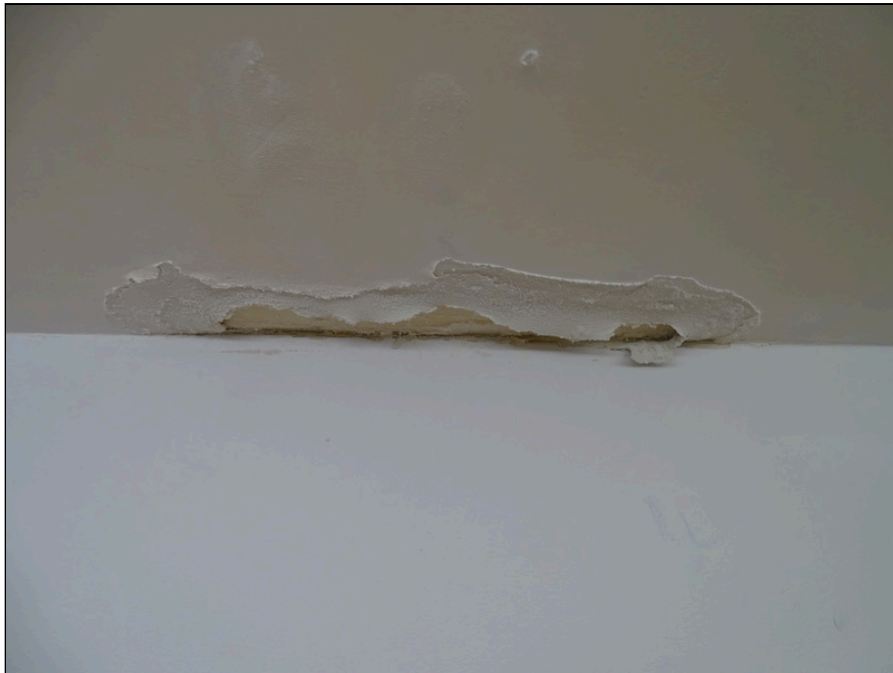
30 - Water leakage at ceiling
