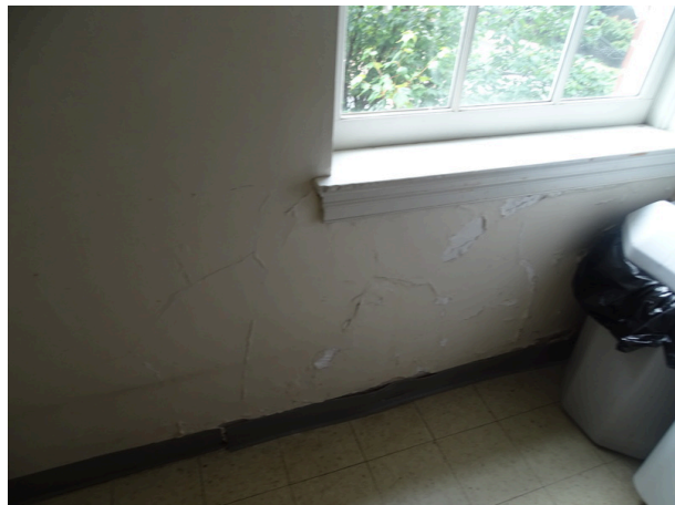
Exterior window - note leakage
