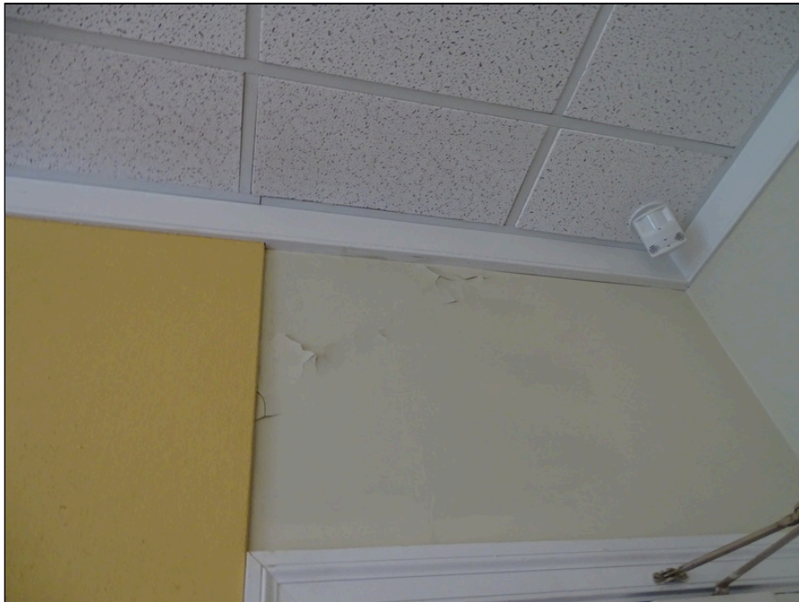
52 - Typical wall - note efflorescence
