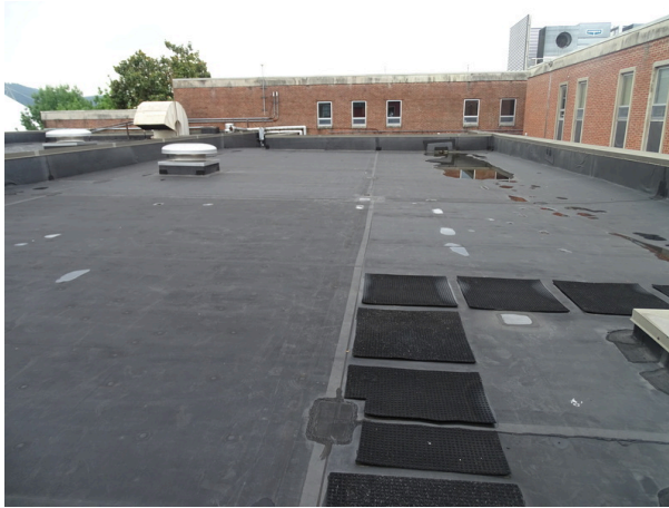
Single-ply membrane roofing system looking north
