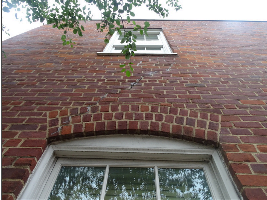
5 - Typical building exterior - note step cracking at brick
