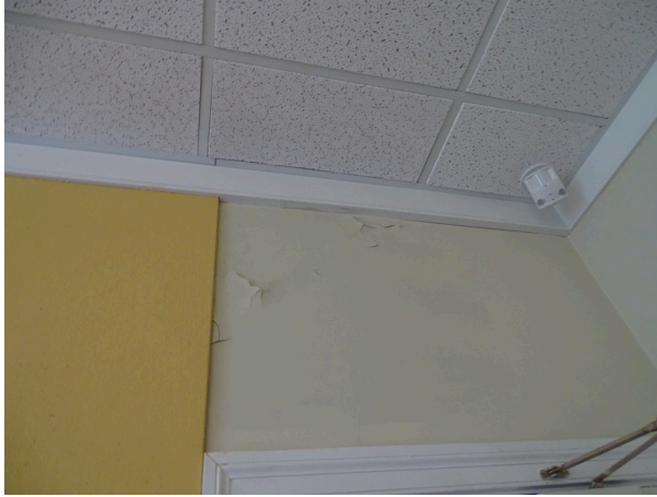
Typical wall - note efflorescence
