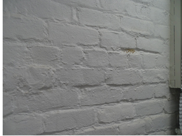
Typical wall - note efflorescence
