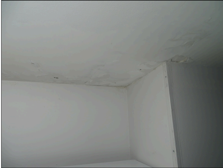
51 - Water leakage at ceiling
