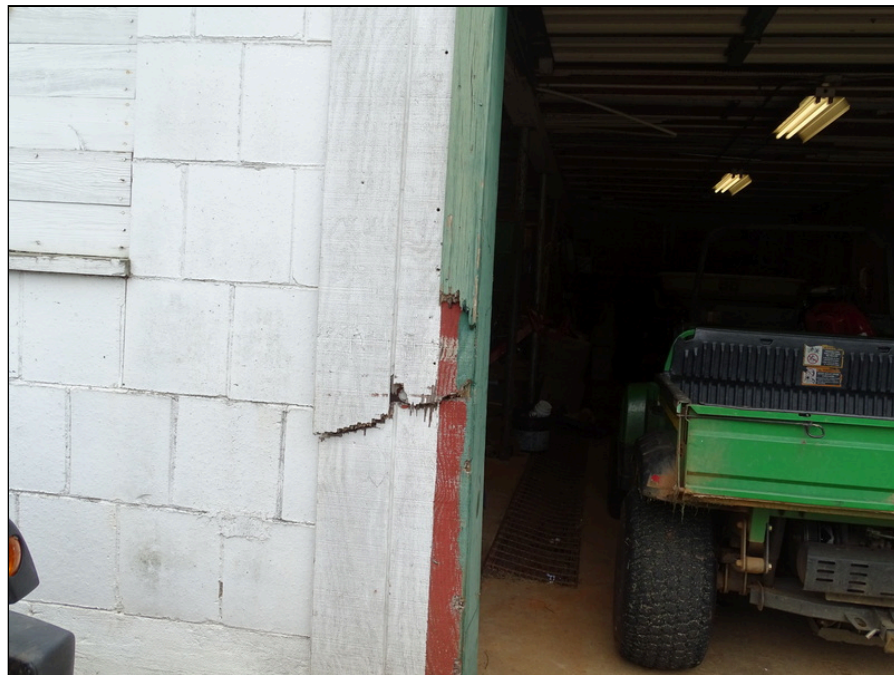
38 - Storage building rotten and broken wood trim
