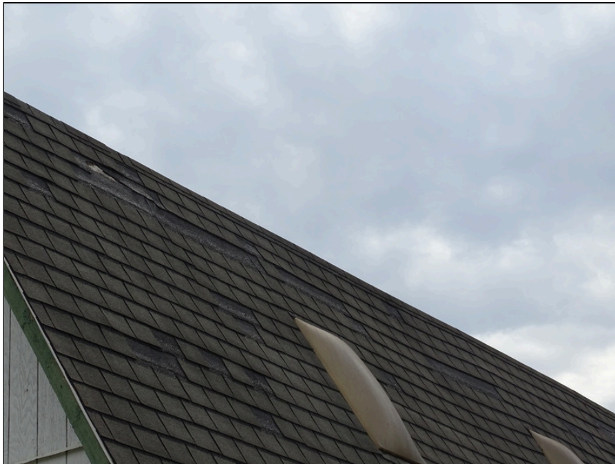
36 - Storage building roof - note deterioration of asphalt shingle
