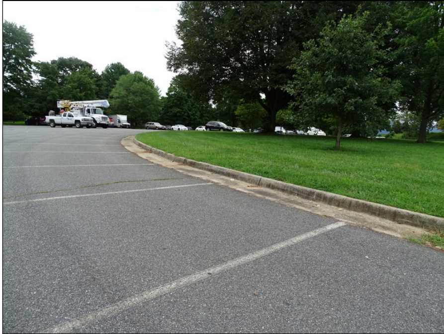
15 - Faded striping and cracks in asphalt pavement
