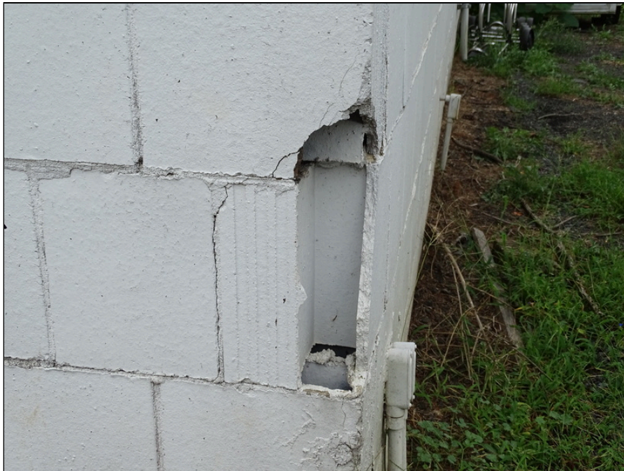
42 - Storage building - note wall deterioration
