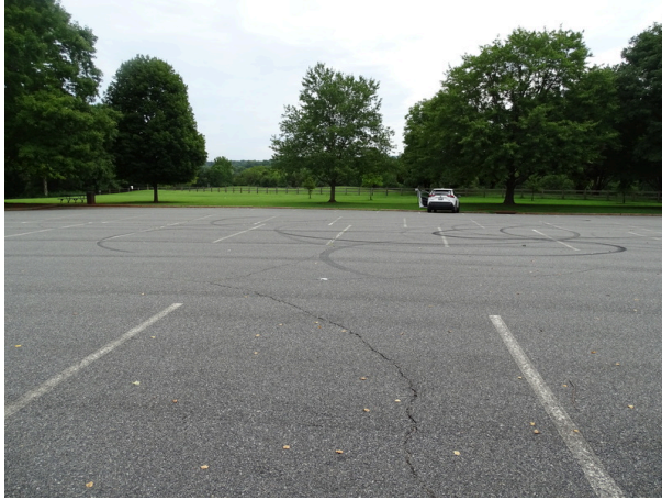
Faded striping and cracks in asphalt pavement
