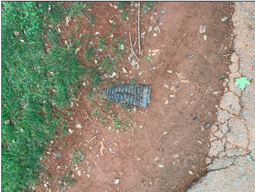
82 - Crushed Downspout Drainage
