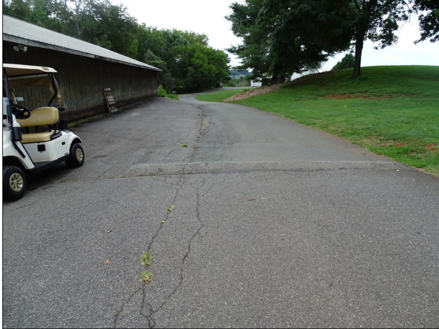
23 - Golf cart shed side pavements - note asphalt deterioration
