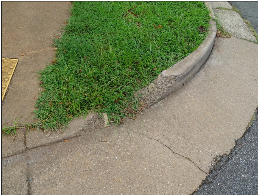
20 - Concrete curb - note deterioration
