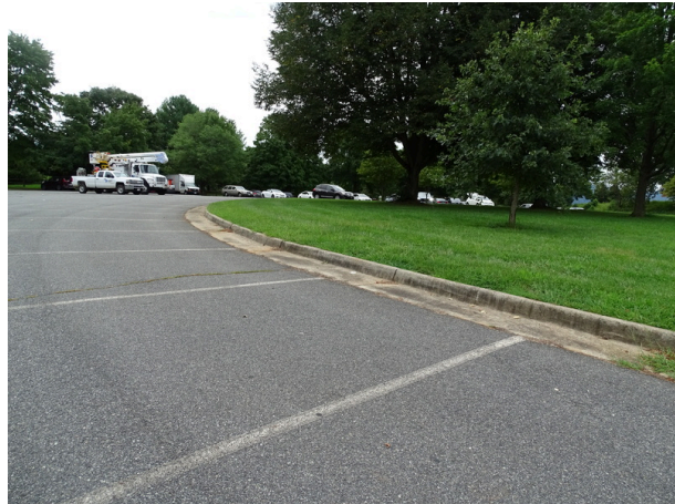
Faded striping and cracks in asphalt pavement
