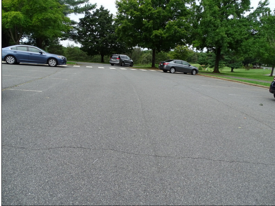
11 - Asphalt parking - note cracks in the asphalt pavement
