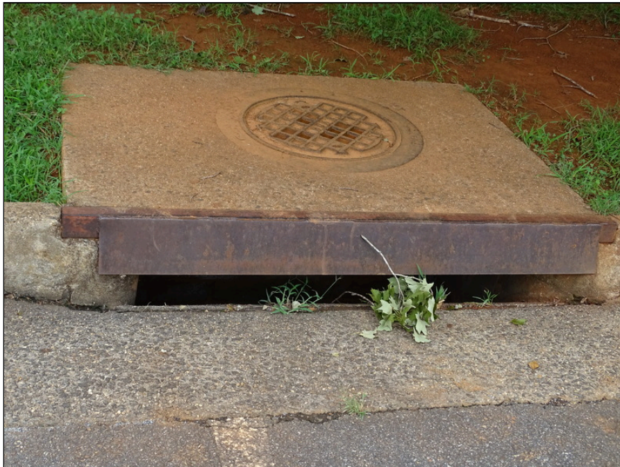
8 - Stormwater drainage at parking lot
