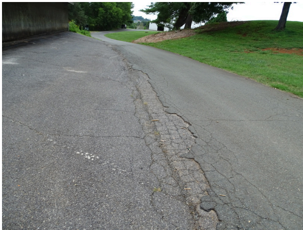
Golf cart shed side pavements - note asphalt deterioration
