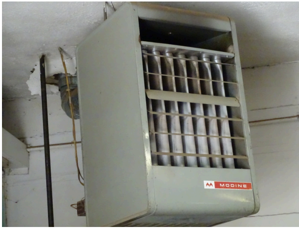
Maintenance Shop unit heater
