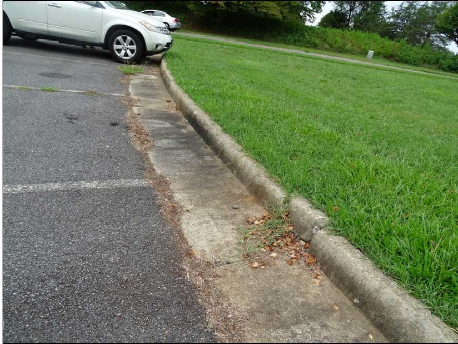
17 - Concrete curb - note deterioration
