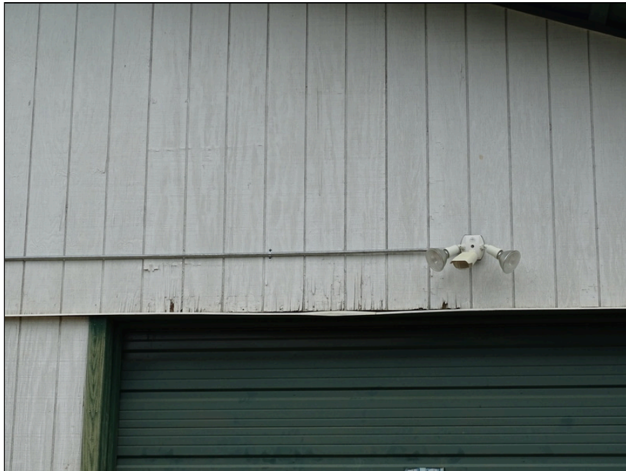
30 - Maintenance Shop exterior - note wood siding deterioration
