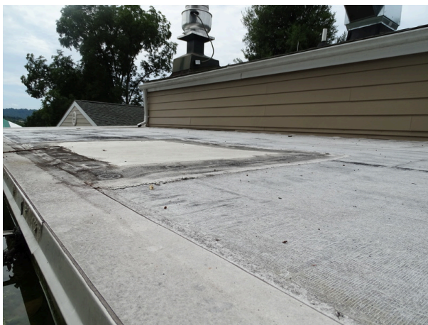
Clubhouse single-ply roof - note deterioration
