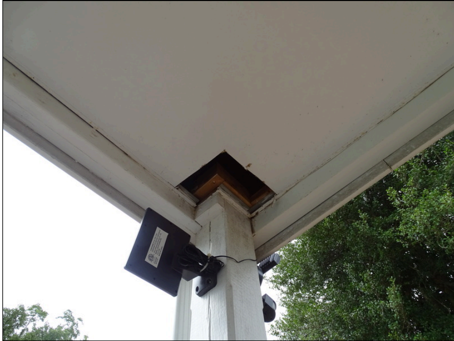
81 - Clubhouse column - note deterioration
