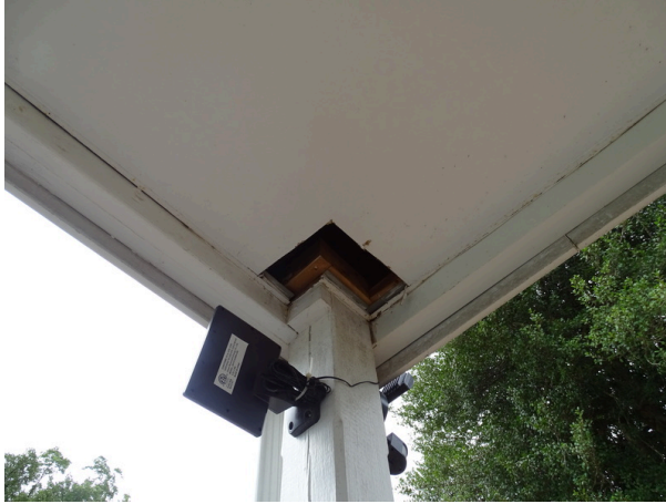
Clubhouse column - note deterioration
