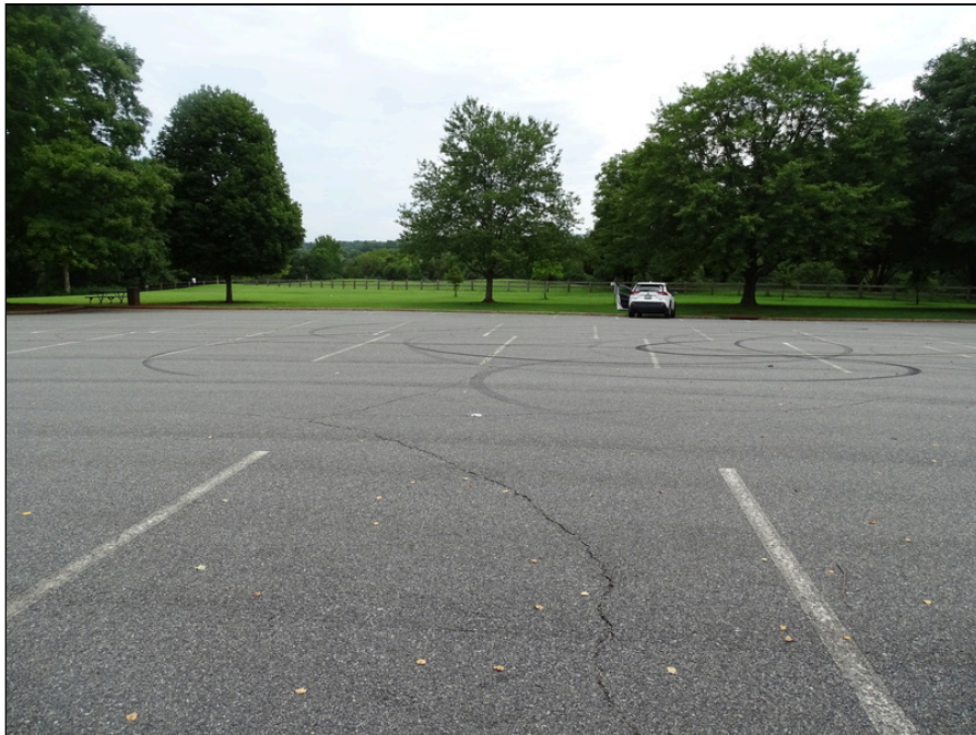
16 - Faded striping and cracks in asphalt pavement
