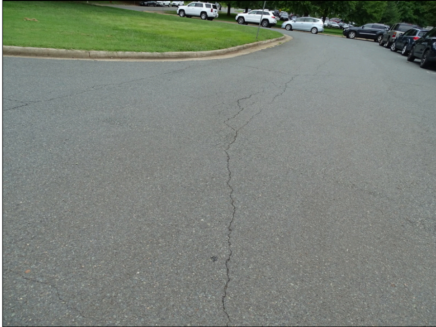
21 - Asphalt pavement - note cracks
