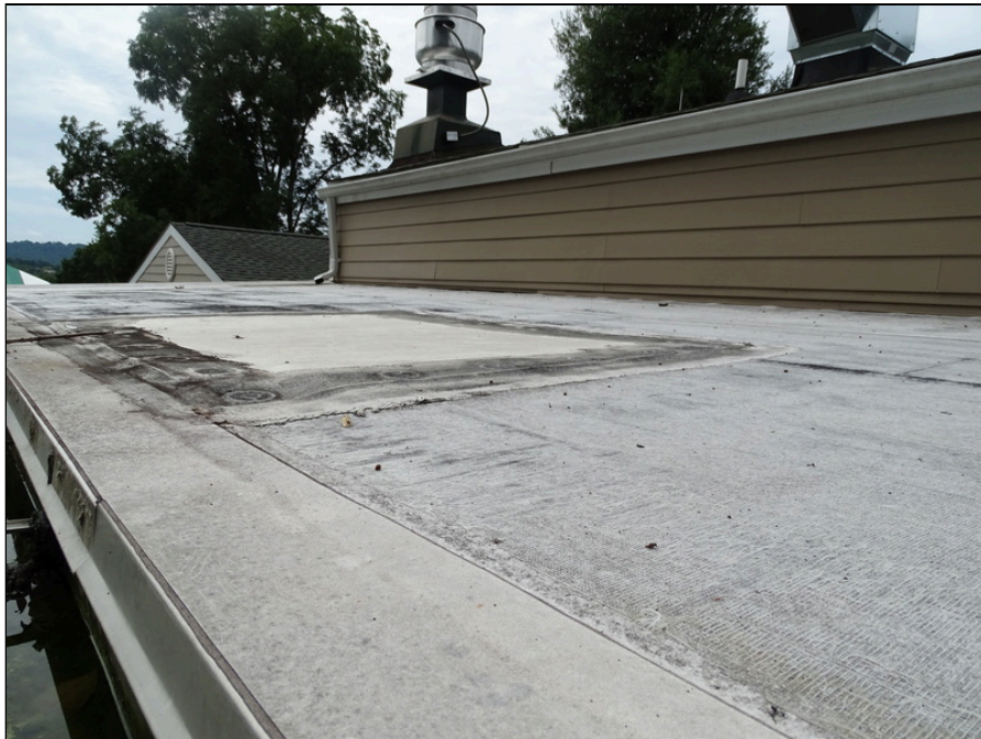
64 - Clubhouse single-ply roof - note deterioration
