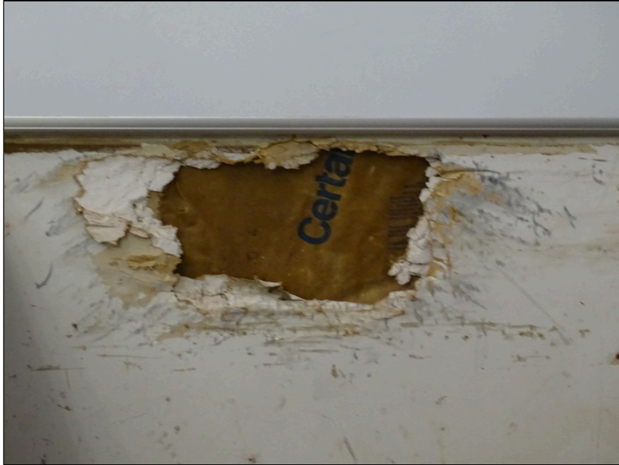
33 - Maintenance Shop - note wall deterioration
