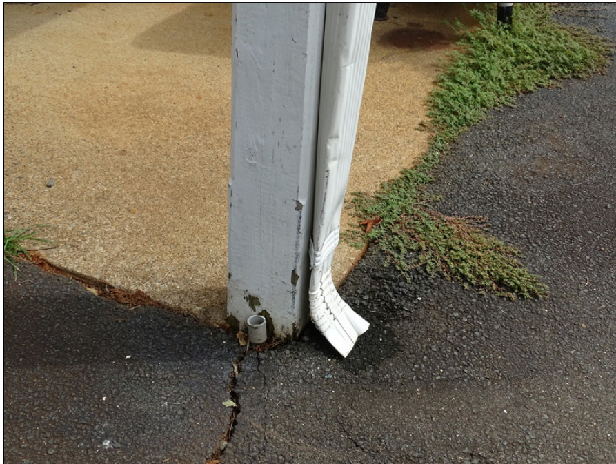
46 - Clubhouse downspout - note damaged
