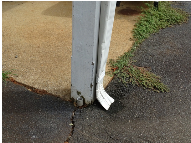
Clubhouse downspout - note damaged
