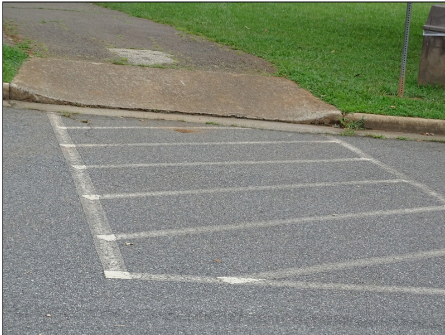
12 - Concrete apron condition - note no truncated domes
