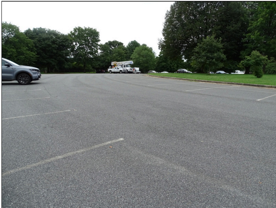
14 - Faded striping and cracks in asphalt pavement
