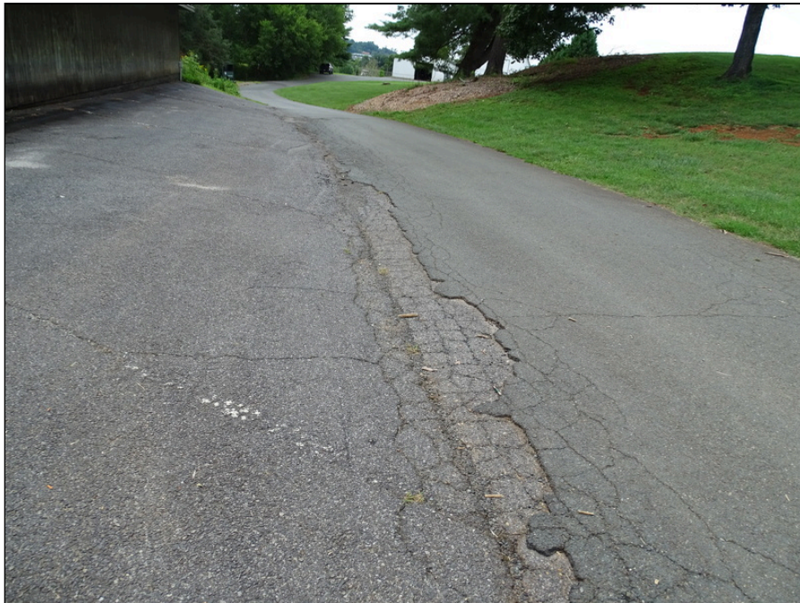
24 - Golf cart shed side pavements - note asphalt deterioration
