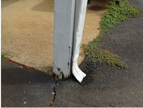
Clubhouse downspout - note damaged
