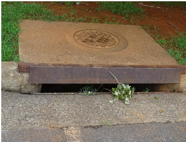
Stormwater drainage at parking lot
