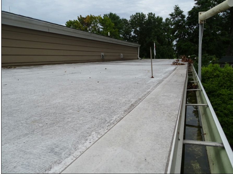
63 - Clubhouse single-ply roof and gutter
