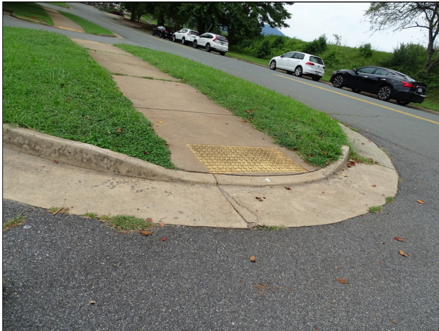
18 - Concrete ramp - note cracks in the apron
