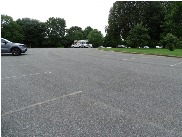
Faded striping and cracks in asphalt pavement
