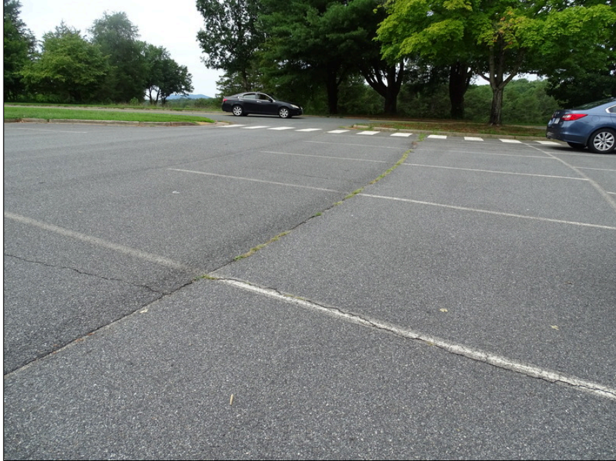
13 - Faded striping and cracks in asphalt pavement
