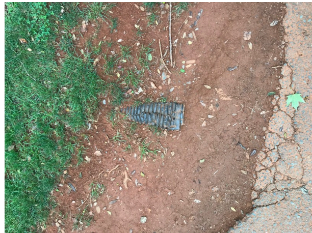
Crushed Downspout Drainage
