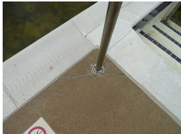
Typical concrete sidewalk - note cracking
