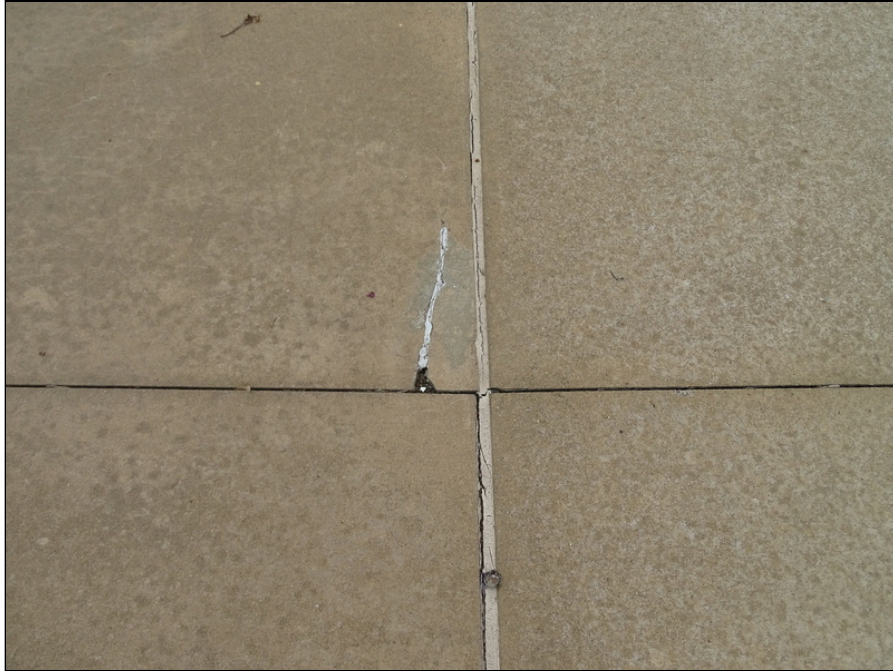
29 - Deteriorated pool deck sealant
