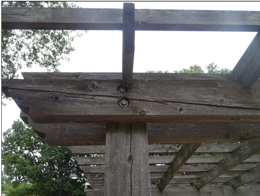
80 - Wood trellis - note weathering
