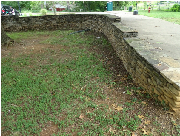
Typical retaining wall - note efflorescence
