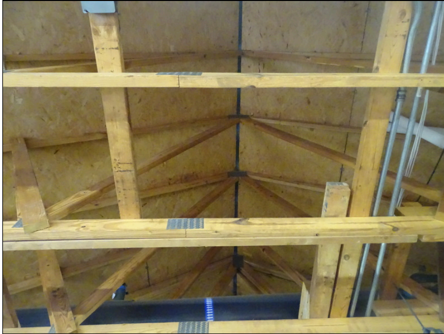
35 - Wood roof framing
