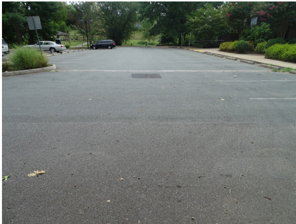
Asphalt pavement and parking - note striping faded
