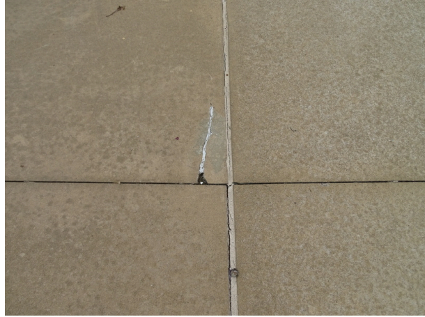
Deteriorated pool deck sealant
