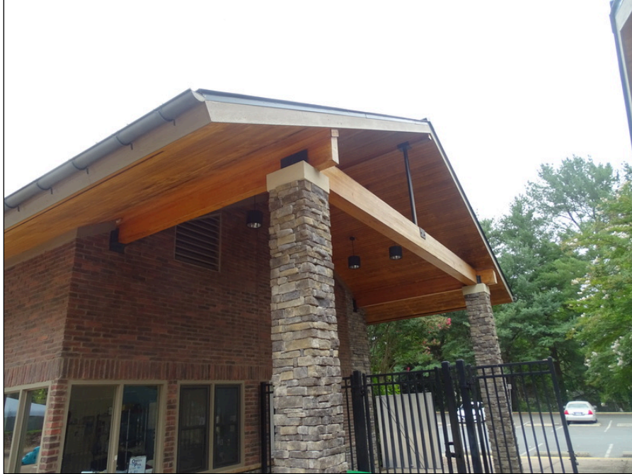
33 - Wood roof framing and steel columns
