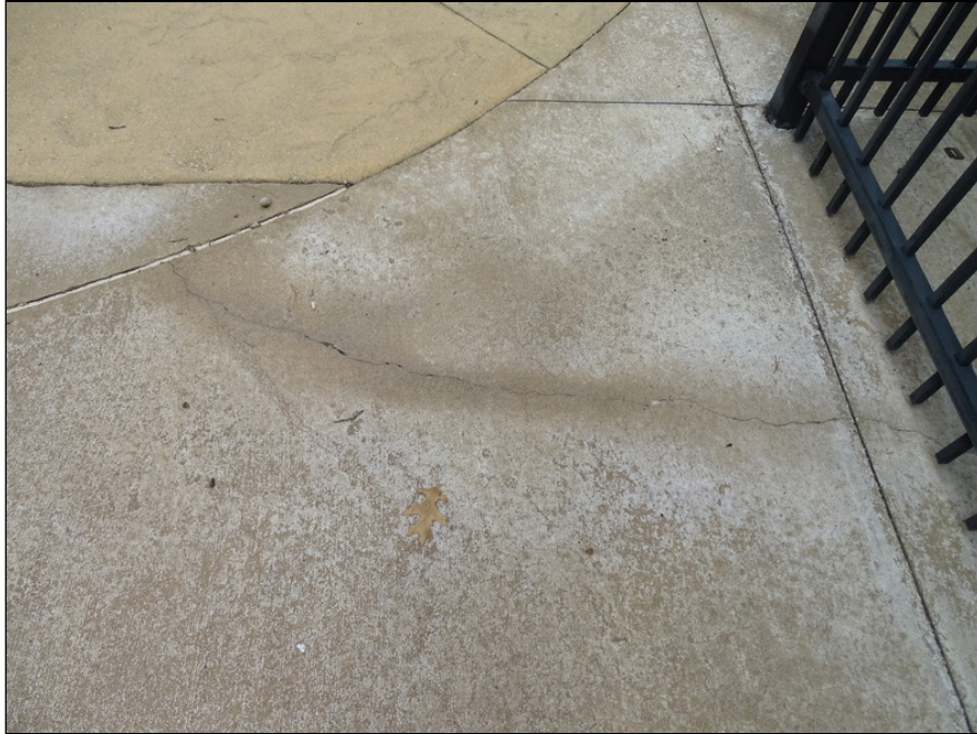
7 - Typical concrete sidewalk - note cracking
