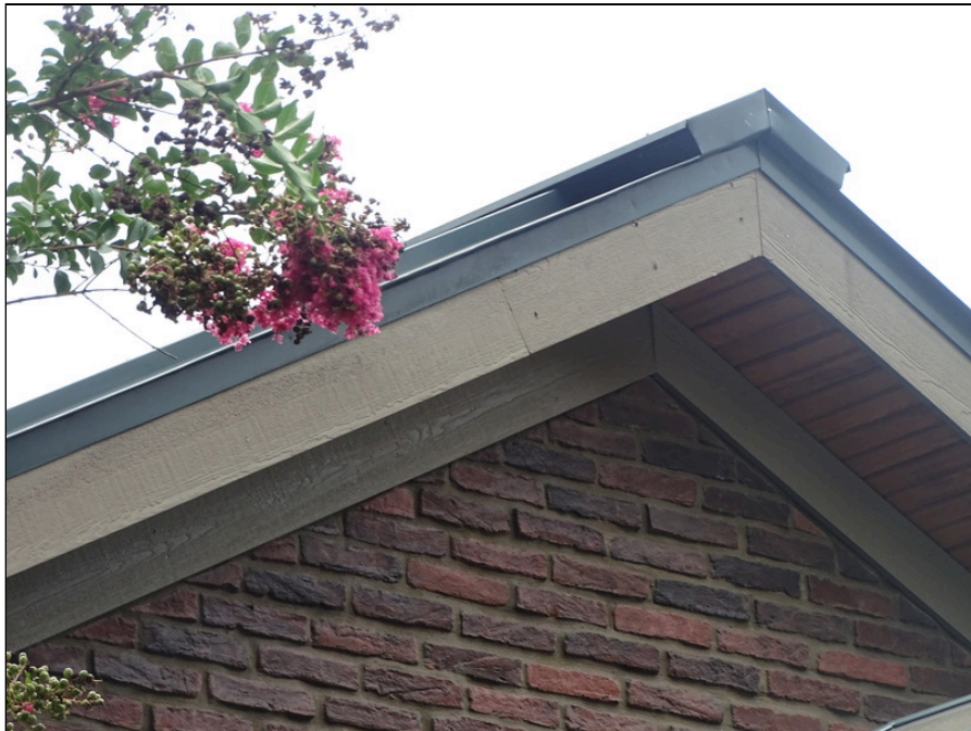
50 - Typical wooden soffit overview
