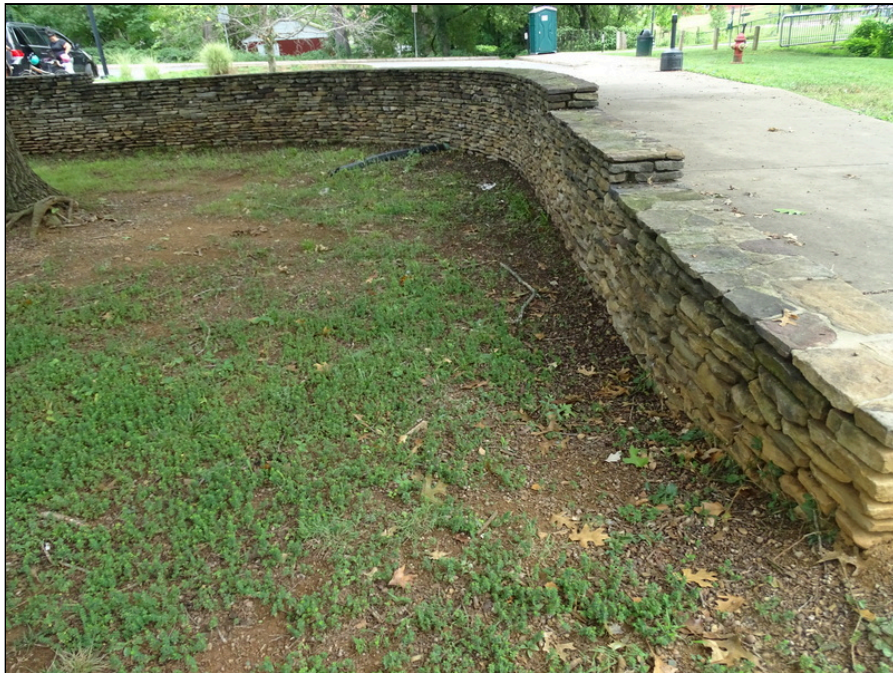
16 - Typical retaining wall - note efflorescence
