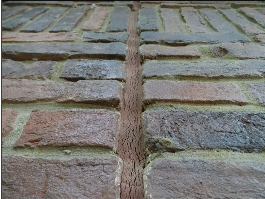
41 - Typical exterior building - note vertical sealant deterioration
