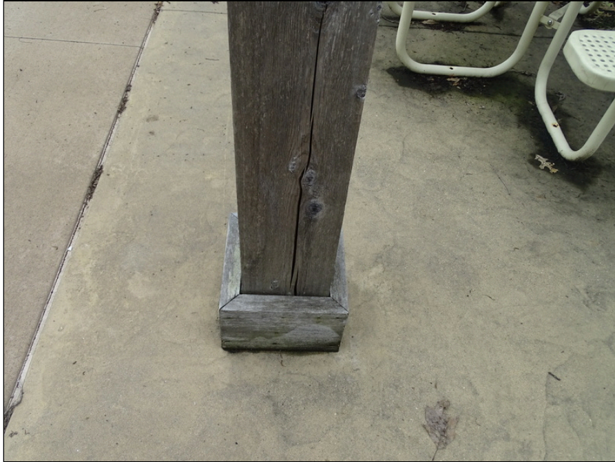
79 - Wood trellis post - note deterioration
