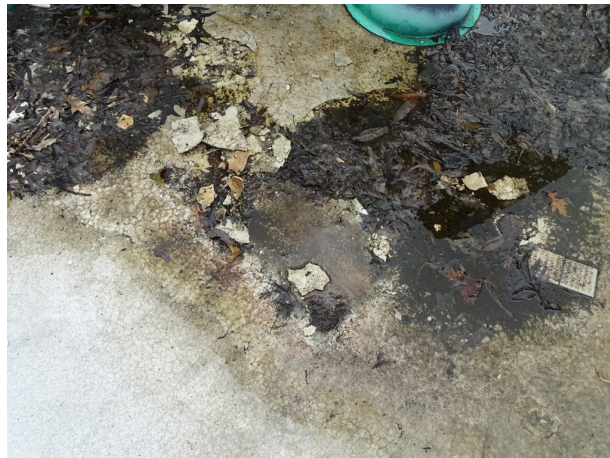
Pool liner deterioration
