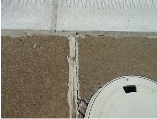
Deteriorated pool deck sealant
