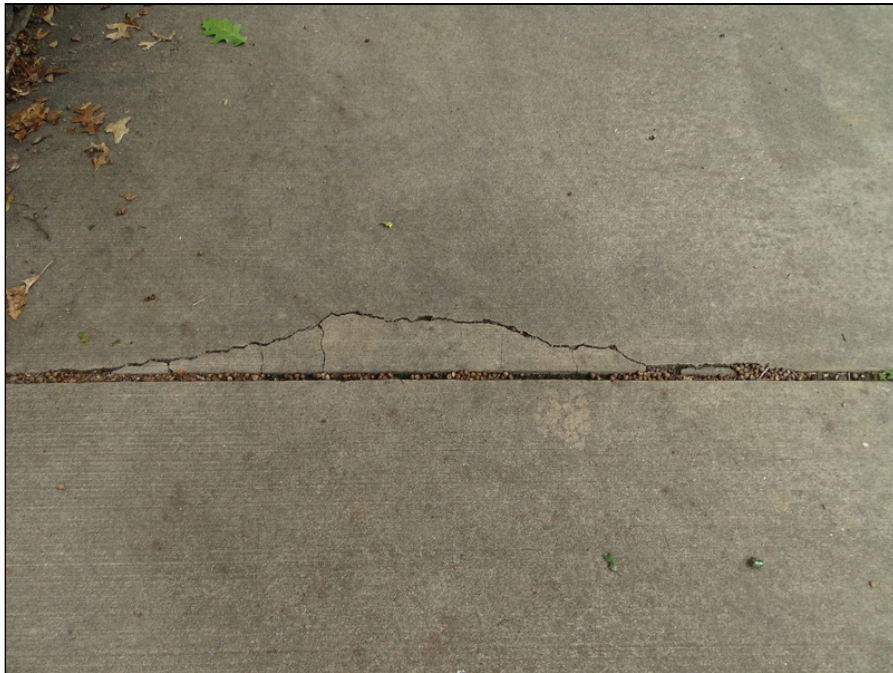
6 - Typical concrete sidewalk - note cracking
