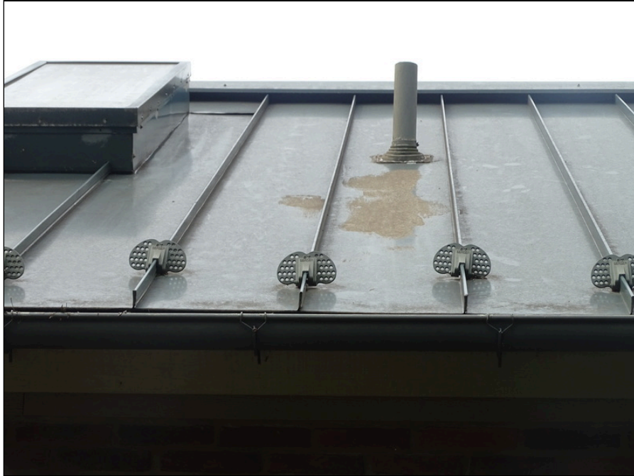
49 - Typical plumbing penetration
