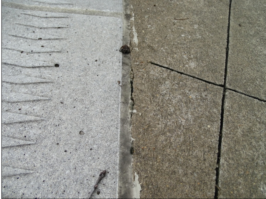
31 - Pool deck - note cracking
