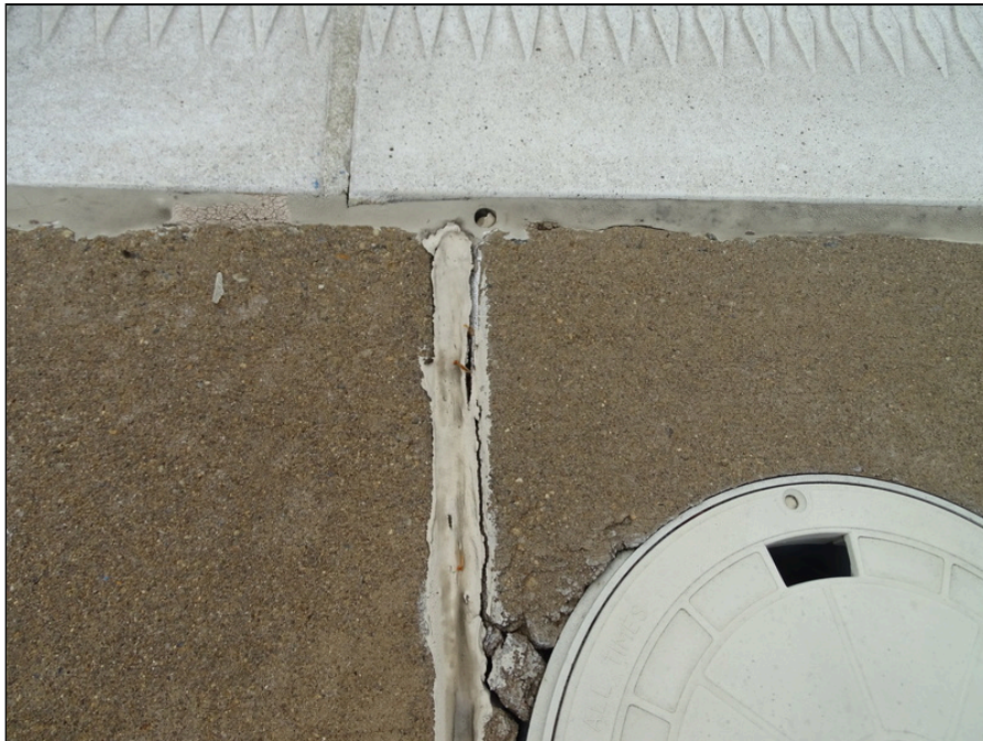
28 - Deteriorated pool deck sealant
