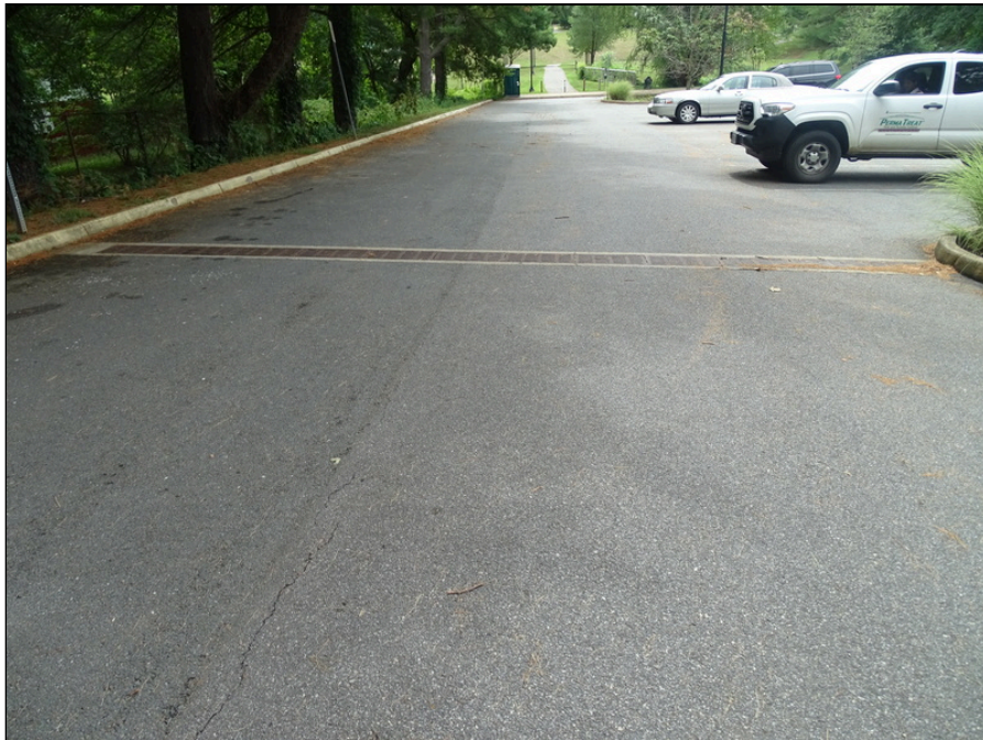
2 - Stormwater drainage and asphalt pavement - note cracking
