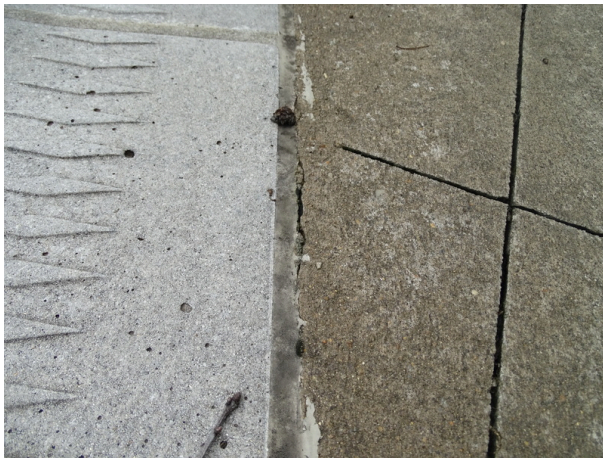
Pool deck - note cracking
