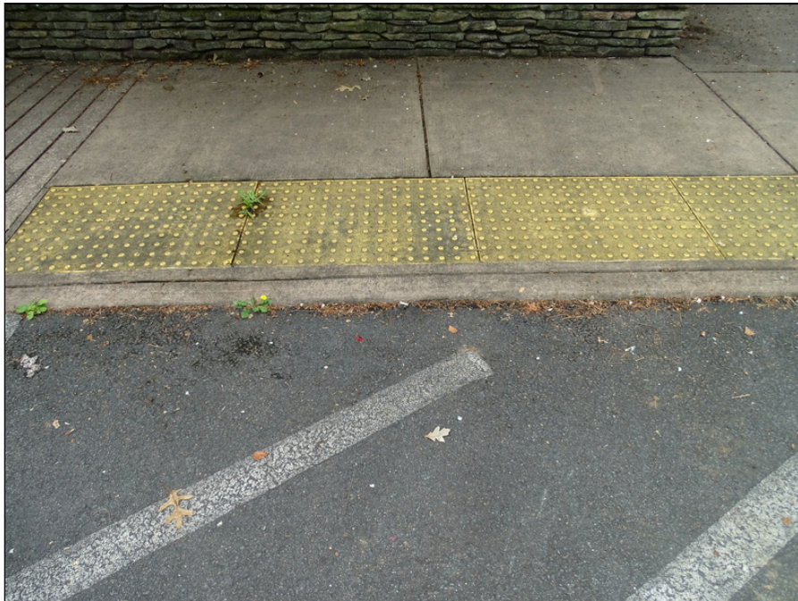
78 - Truncated domes at curb ramp from parking lot
