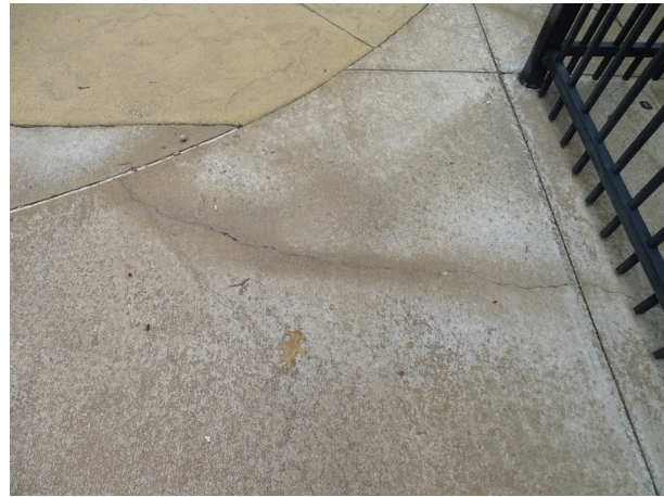
Typical concrete sidewalk - note cracking
