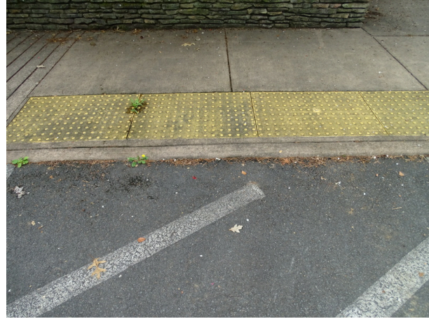
Truncated domes at curb ramp from parking lot
