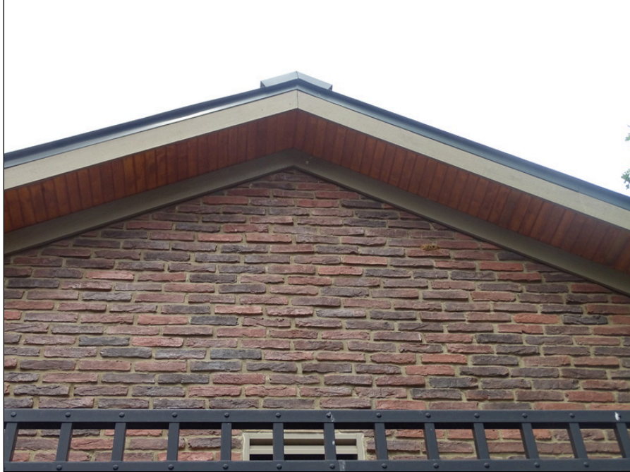
39 - Brick joints and sealant at exterior
