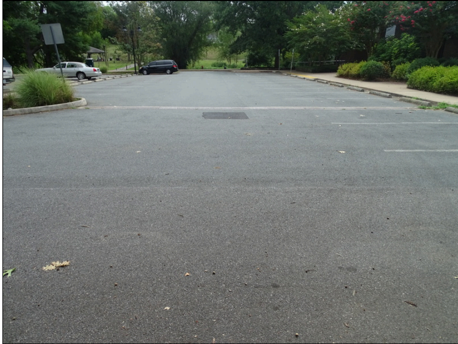
3 - Asphalt pavement and parking - note stripping faded
