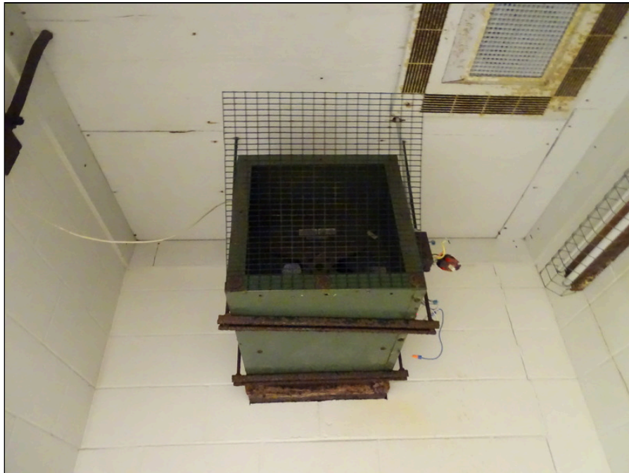
54 - Typical space heater - note deterioration
