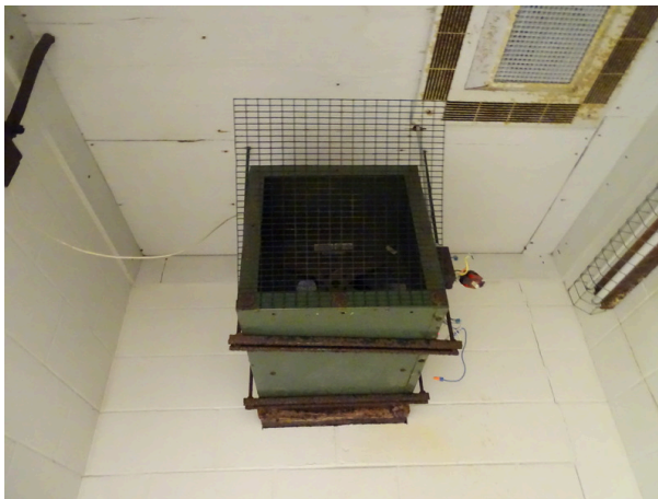
Typical space heater - note deterioration
