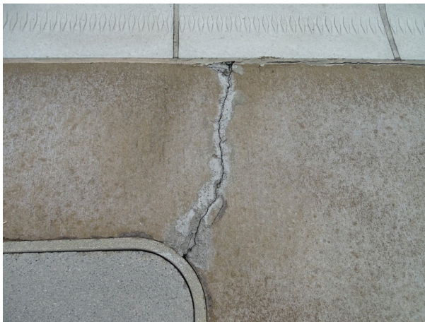
Typical concrete sidewalk - note cracking
