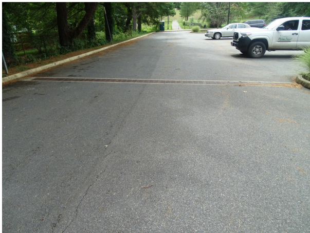
Stormwater drainage and asphalt pavement - note cracking
