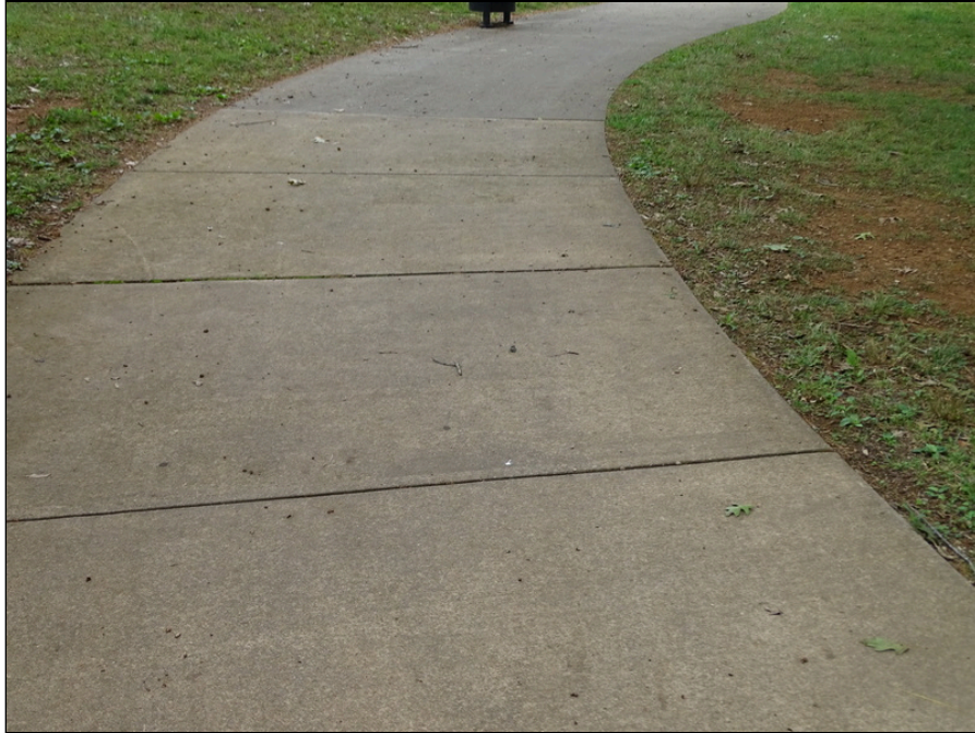
5 - Typical concrete sidewalk
