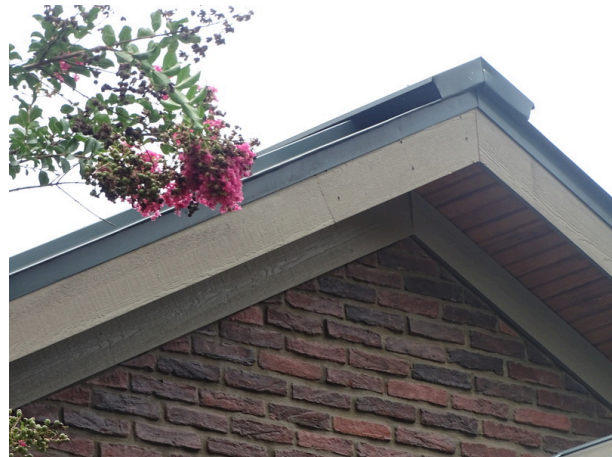
Typical wooden soffit overview
