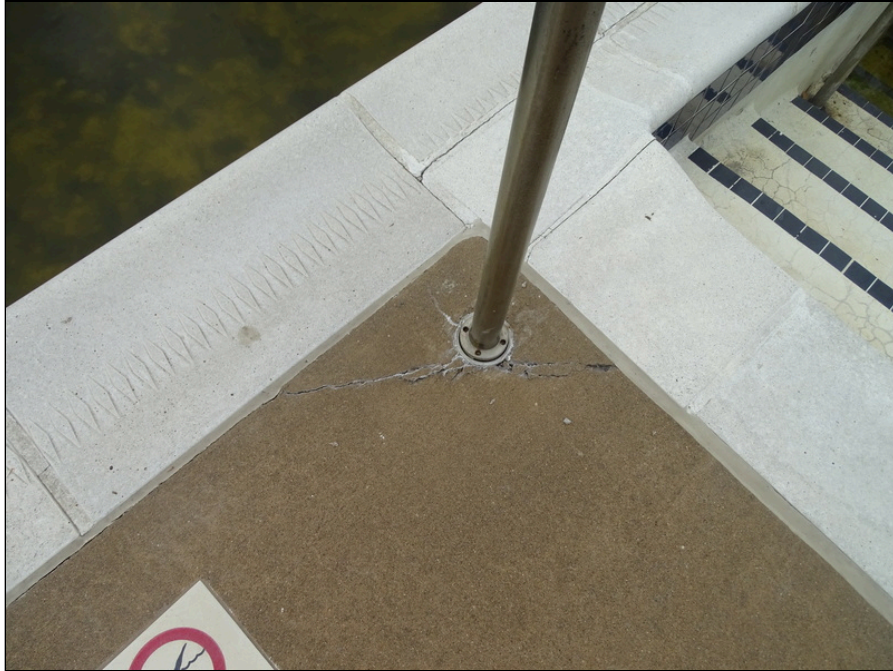
9 - Typical concrete sidewalk - note cracking
