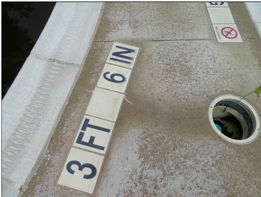
30 - Pool deck - note cracking
