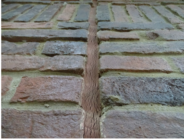
Typical exterior building - note vertical sealant deterioration
