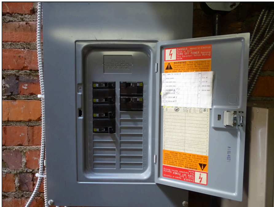
58 - Electrical main disconnect switch
