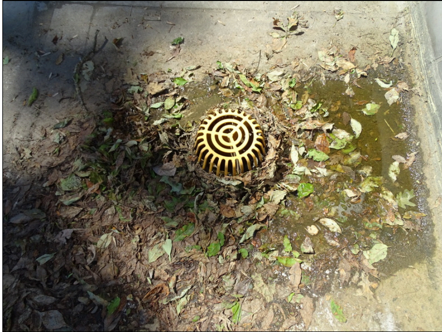
39 - Typical internal roof drain - note maintenance needed
