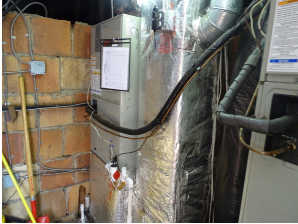
Typical air handler located in second level attic space
