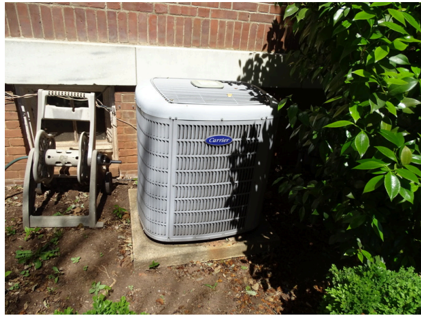
Condenser located at exterior ground level
