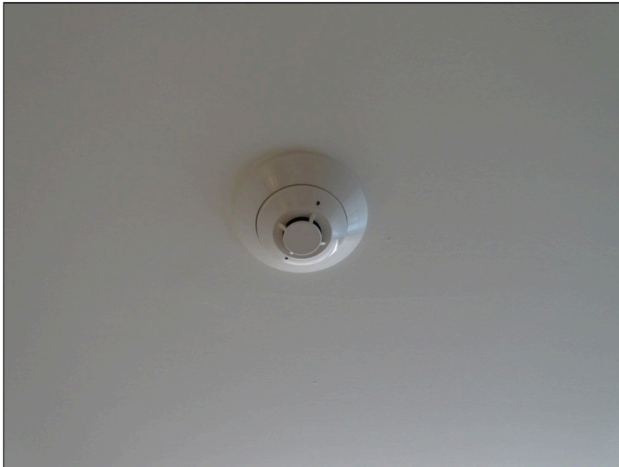
60 - Typical smoke detector
