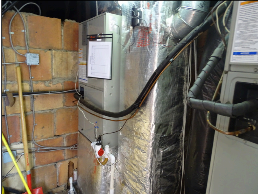
47 - Typical air handler located in second level attic space
