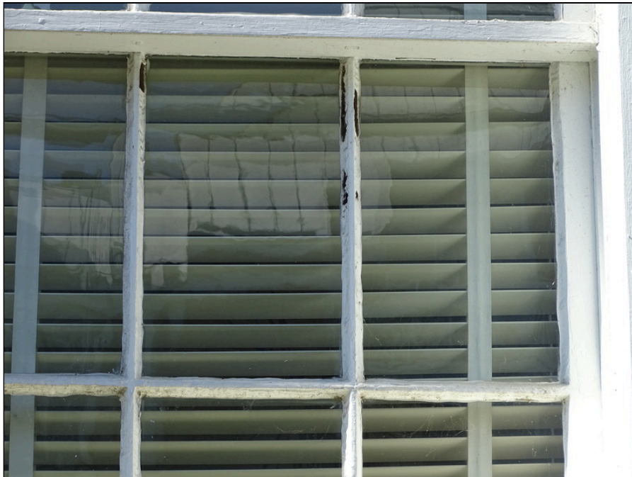
30 - Typical exterior window - note deterioration
