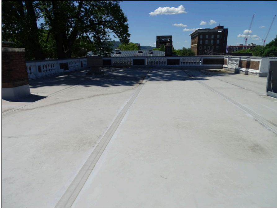
35 - roofing system Roofing system single-ply sheet membrane
