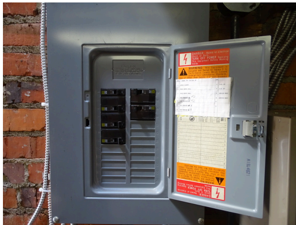
Electrical main disconnect switch
