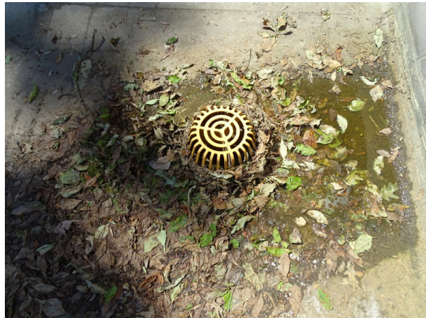
Typical internal roof drain - note maintenance needed
