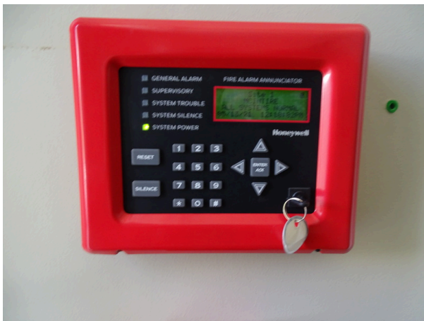
Typical fire alarm annunciator
