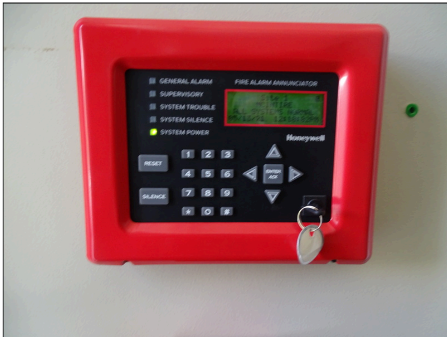
62 - Typical fire alarm annunciator
