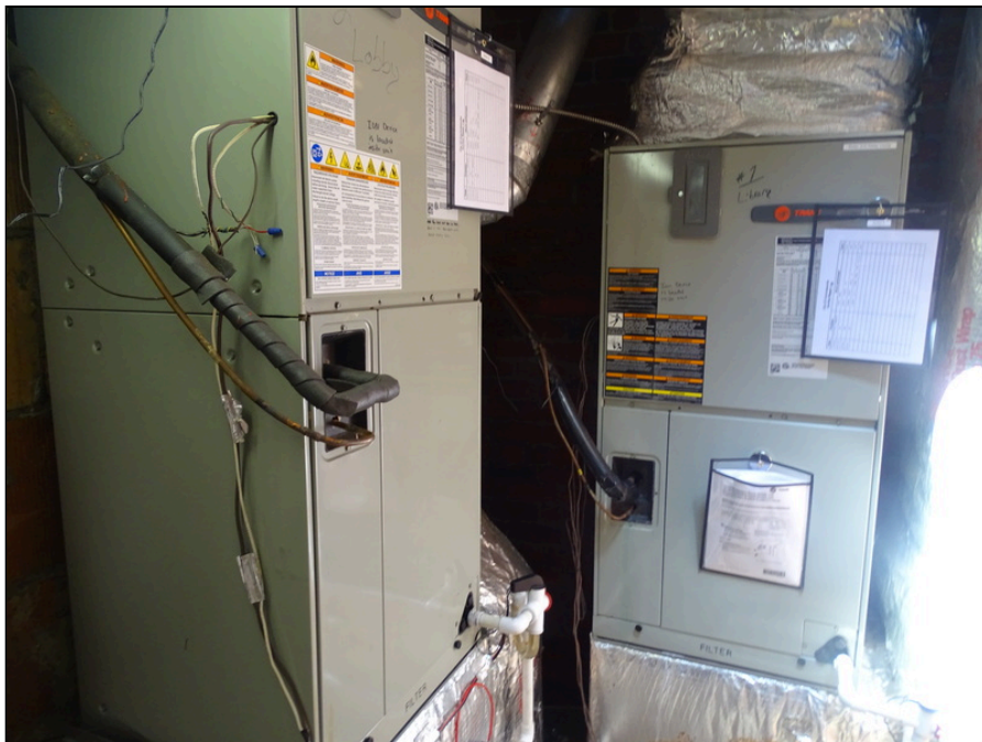
46 - Typical air handler located in second level attic space
