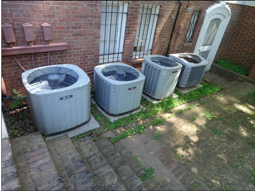
45 - Condensers and heat pump located at exterior ground level
