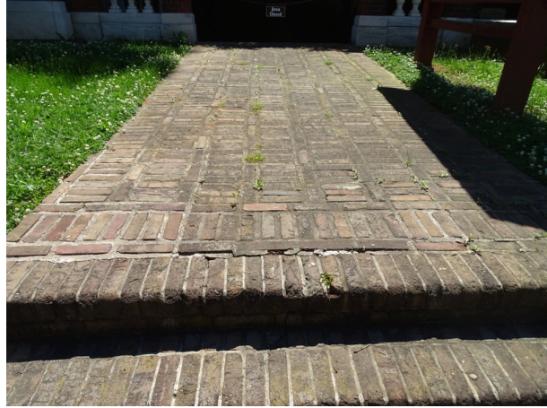
Brick pavers and steps at southwest end of site - note Deterioration
