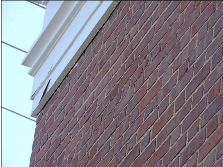
25 - Building exterior - note some deterioration of mortar
