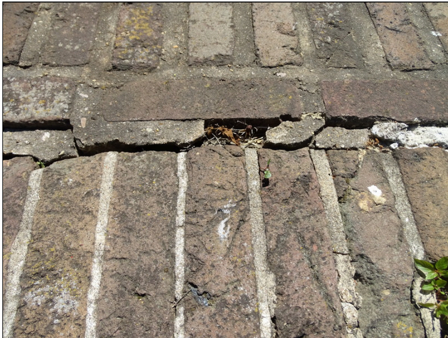
6 - Brick pavers and concrete sidewalk at east side of the site - note deterioration
