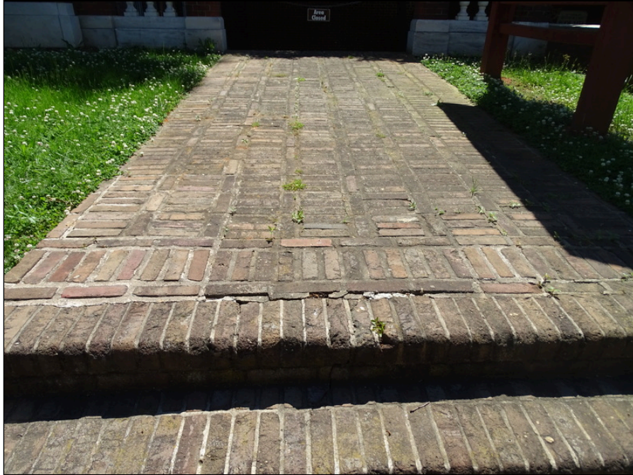
5 - Brick pavers and steps at southwest end of site - note Deterioration
