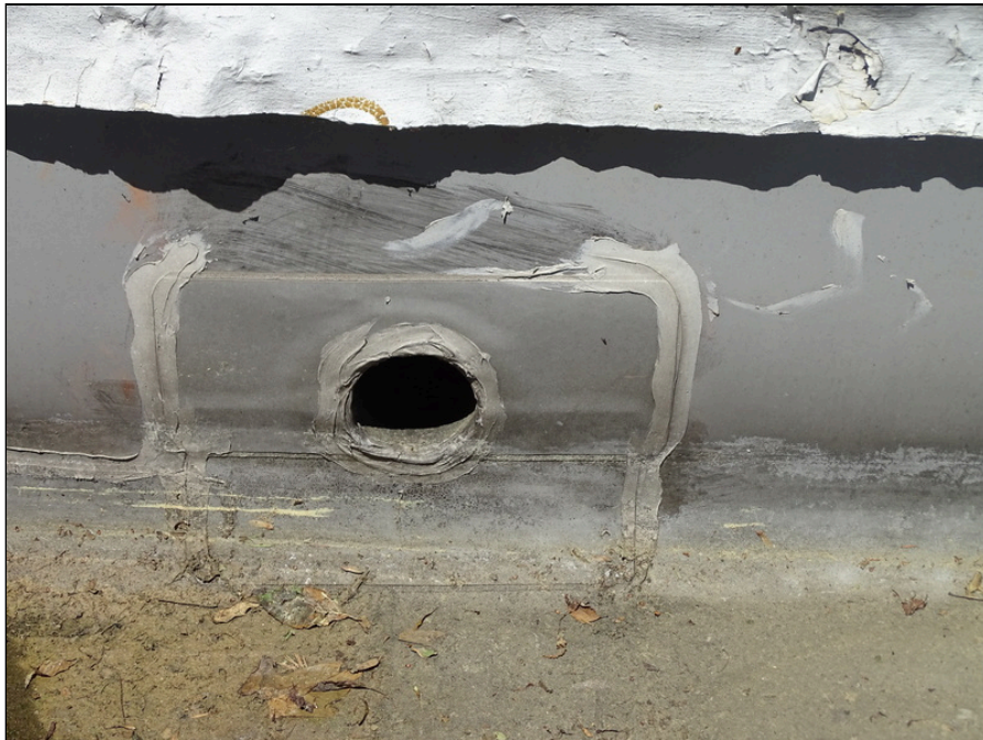
40 - Parapet wall and through wall drain - note patching
