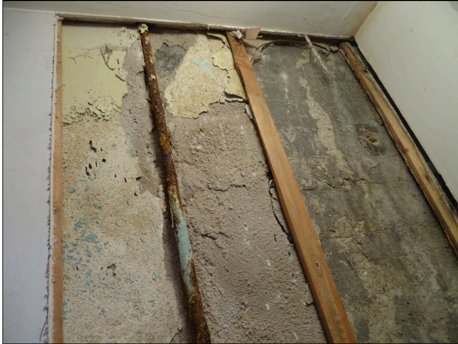
21 - Structure framing - note deterioration
