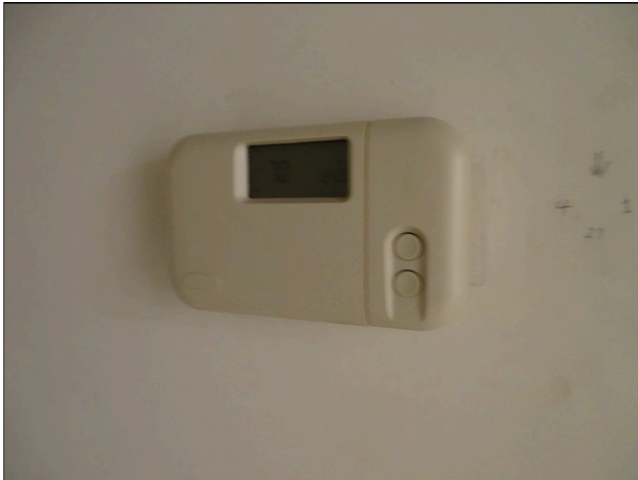
56 - Typical digital thermostat
