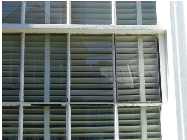
Typical exterior window - note deterioration
