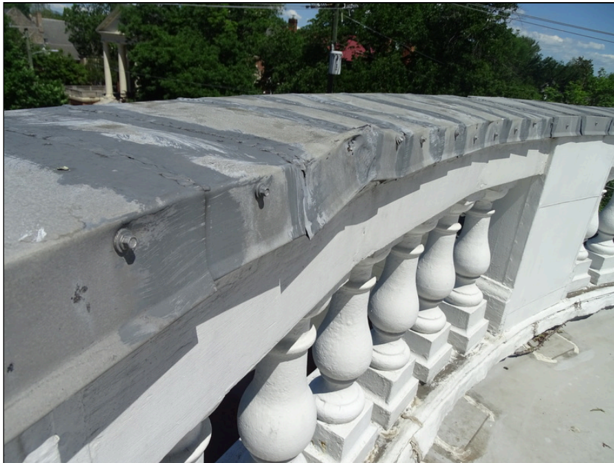
38 - Metal coping and wood parapet framing
