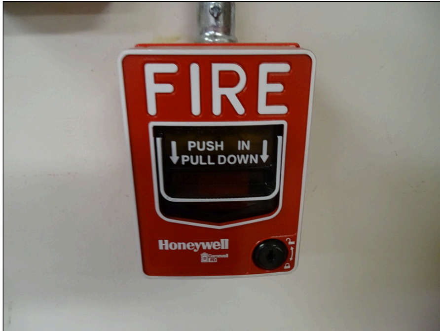
61 - Typical fire alarm pull station
