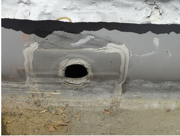
Parapet wall and through wall drain - note patching
