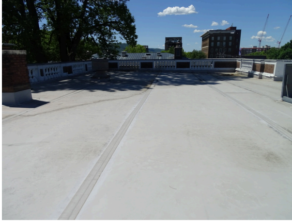
roofing system Roofing system single-ply sheet membrane
