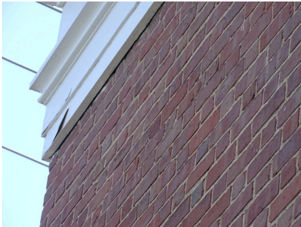
Building exterior - note some deterioration of mortar
