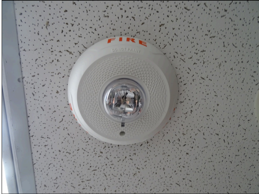
63 - Typical fire alarm bell and strobe
