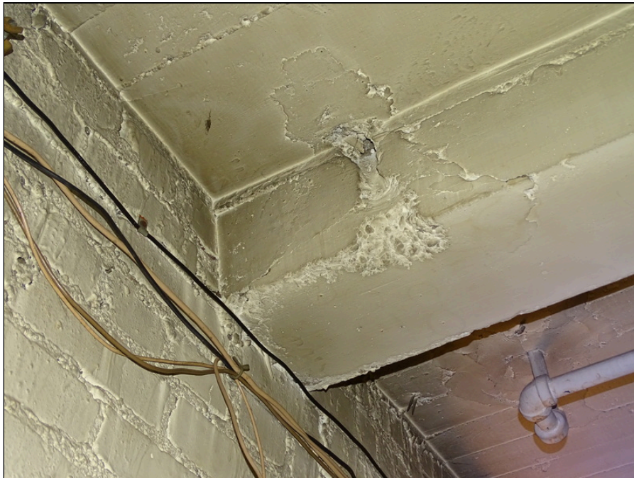
22 - Structure framing - note deterioration
