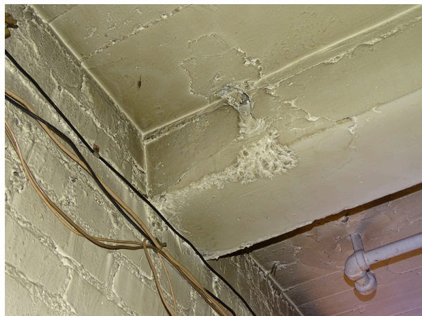
Structure framing - note deterioration
