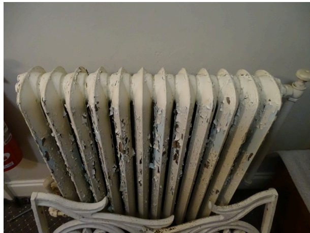
Typical radiator - note deterioration
