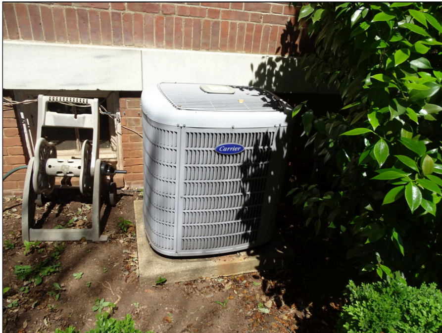
44 - Condenser located at exterior ground level
