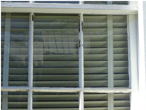
Typical exterior window - note deterioration
