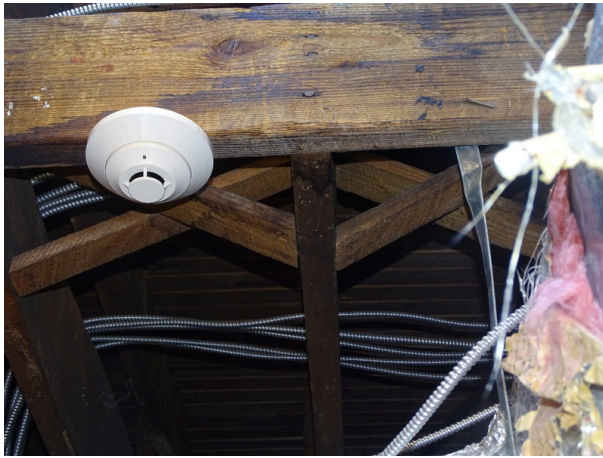
Typical smoke detector
