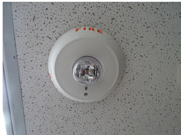
Typical fire alarm bell and strobe
