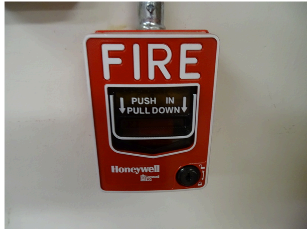
Typical fire alarm pull station
