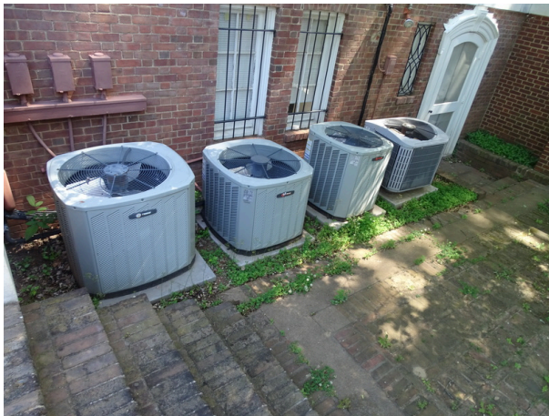
Condensers and heat pump located at exterior ground level
