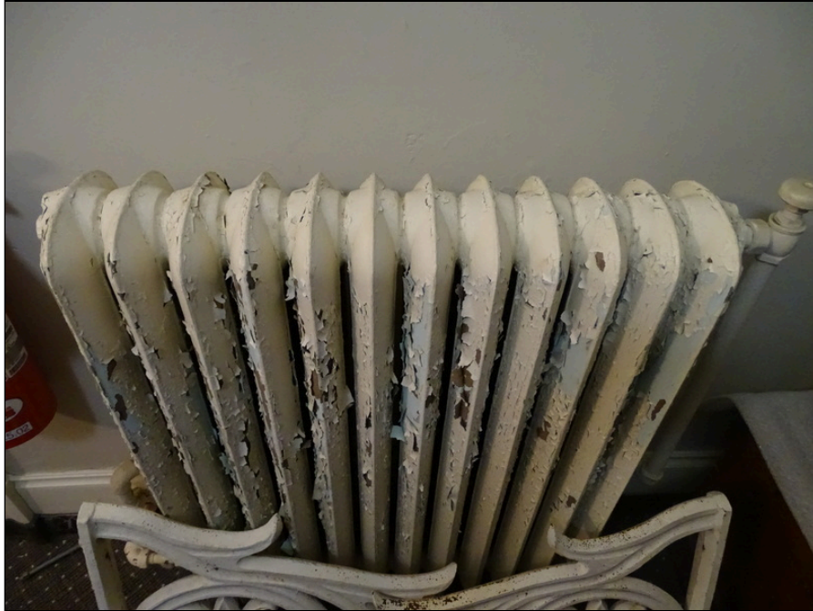
55 - Typical radiator - note deterioration
