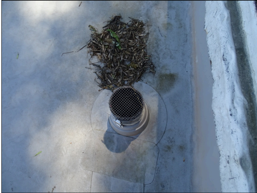
41 - Mechanical vent
