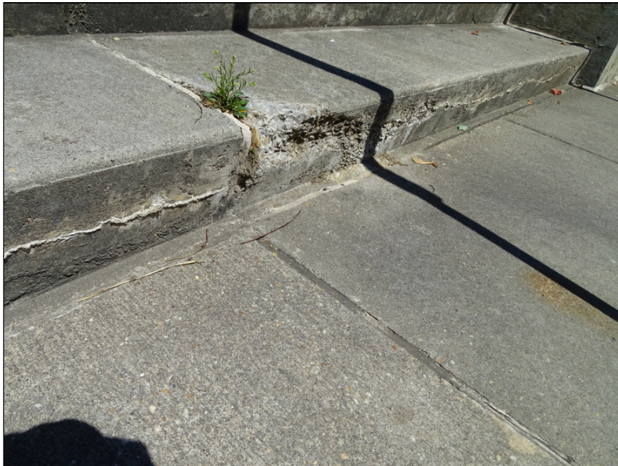
6 - Typical concrete sidewalks - note deterioration
