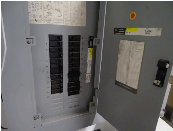
Typical circuit breaker panel
