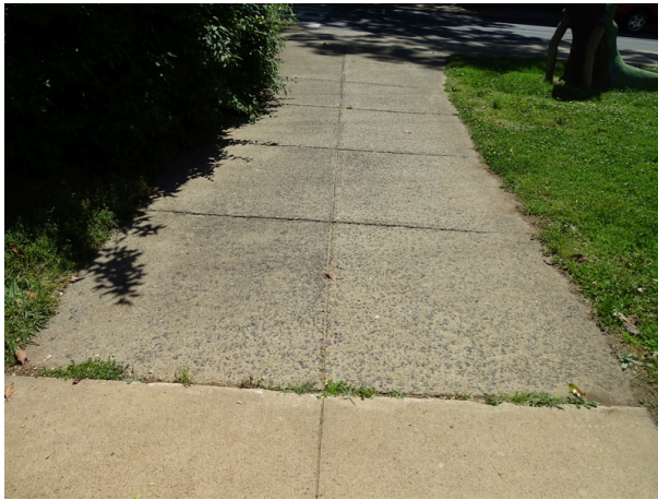
Typical concrete sidewalks - note spalling
