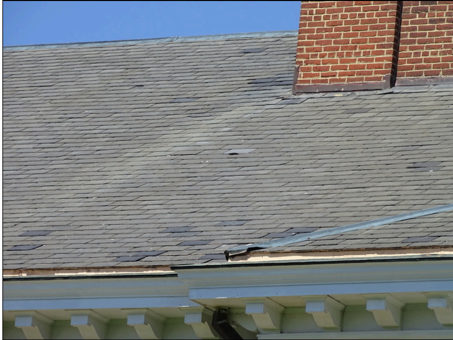
37 - Slate shingle roofing system - note deterioration
