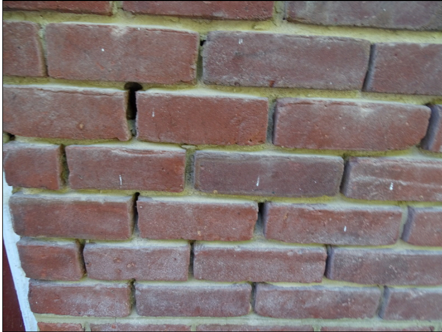
29 - Typical exterior wall - note deterioration of mortar
