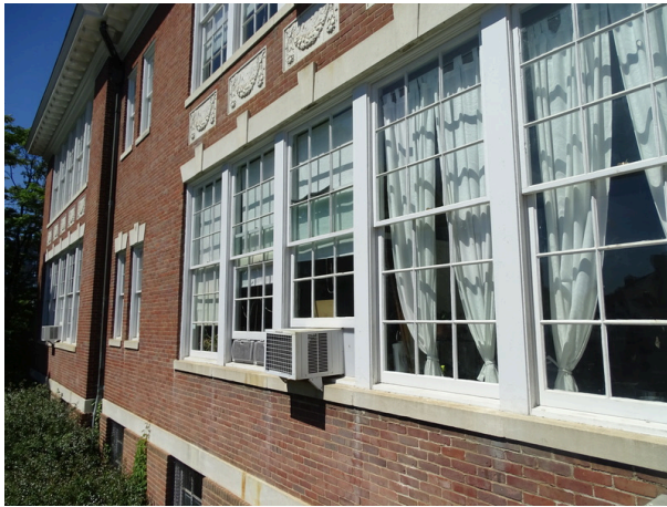
Typical exterior window units - note recent restoration
