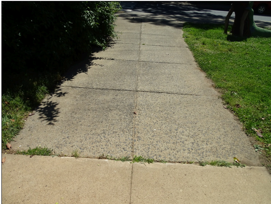
4 - Typical concrete sidewalks - note spalling
