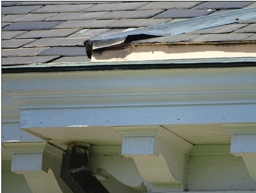
38 - Slate shingle roofing system - note deterioration
