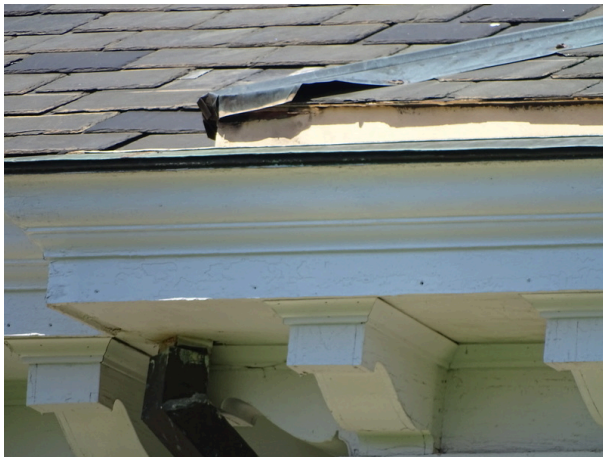
Slate shingle roofing system - note deterioration
