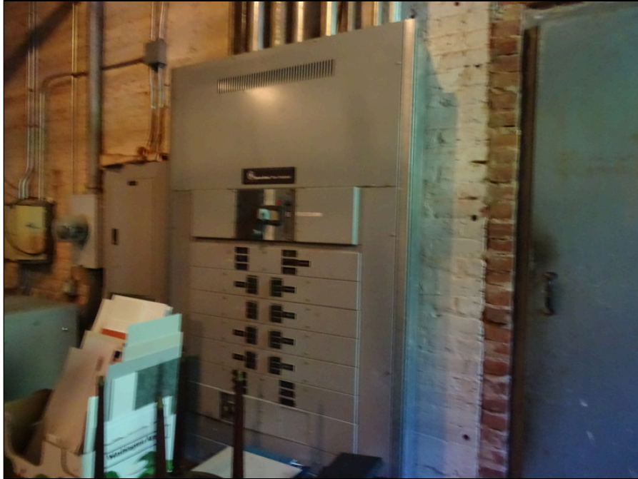
49 - Main electrical switchgear located in the main utility room
