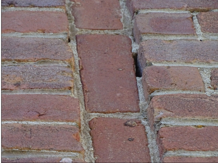
27 - Typical exterior wall - note deterioration of mortar
