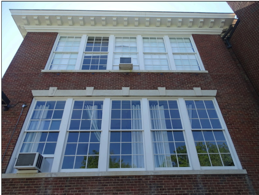
34 - Typical exterior window units - note recent restoration
