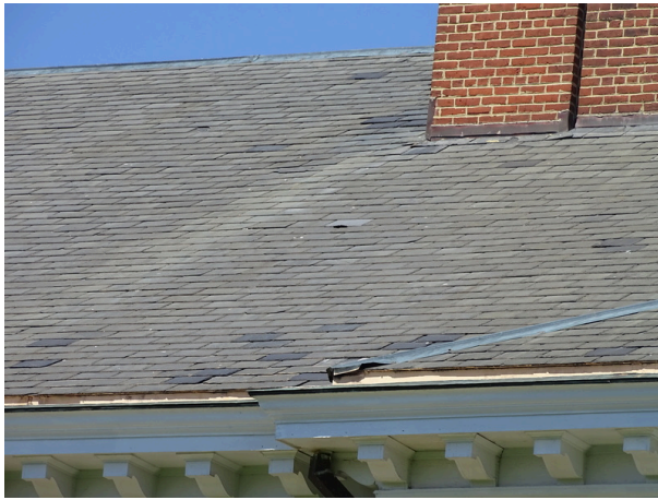
Slate shingle roofing system - note deterioration
