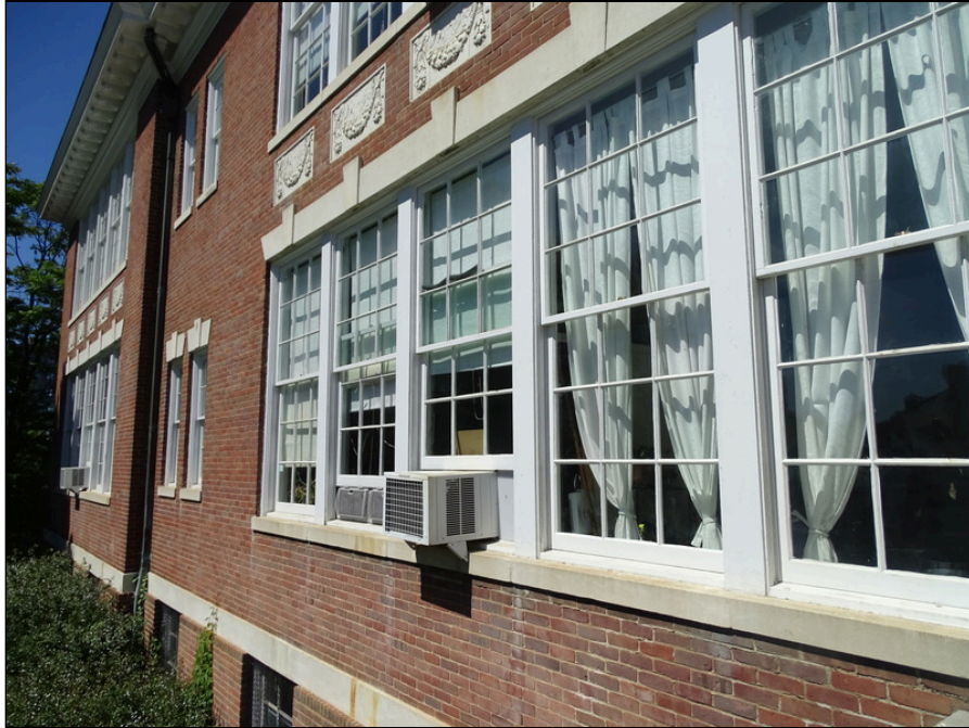
33 - Typical exterior window units - note recent restoration
