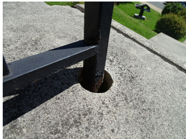
Typical steel hand rail - note deterioration
