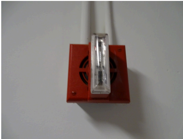
Typical fire alarm strobe and bell
