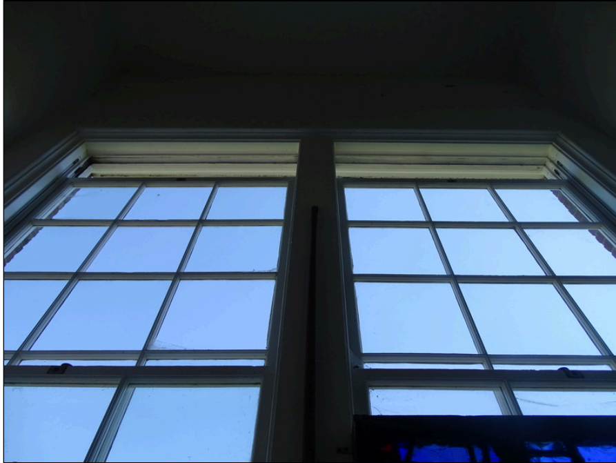
35 - Typical exterior window units - note recent restoration
