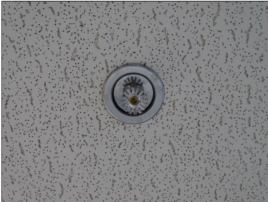
58 - Typical sprinkler head
