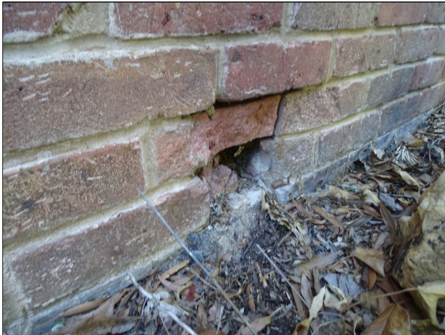
28 - Typical exterior wall - note deterioration of mortar
