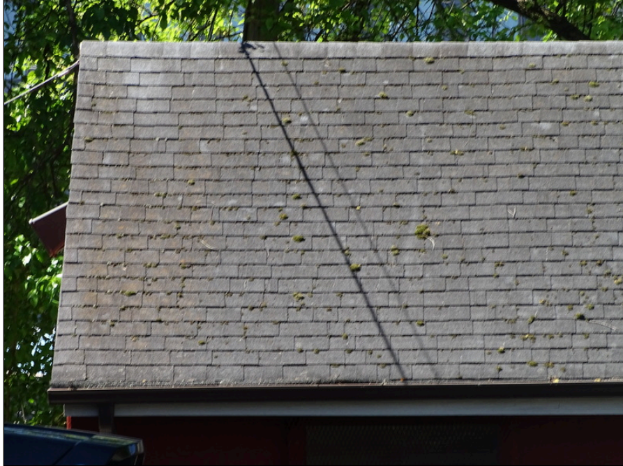
41 - Asphalt shingle roofing system located over studio area
