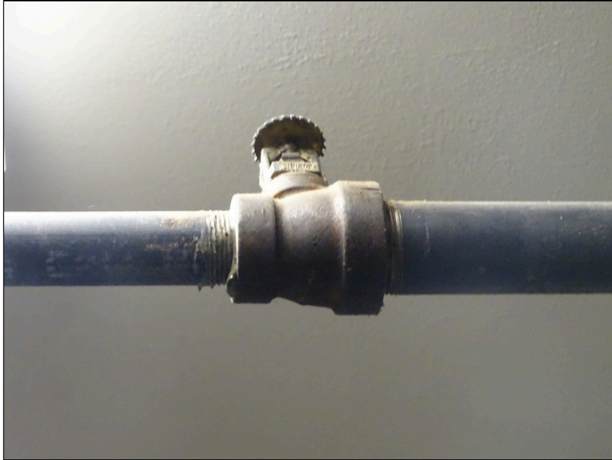
57 - Typical sprinkler pipe and sprinkler head
