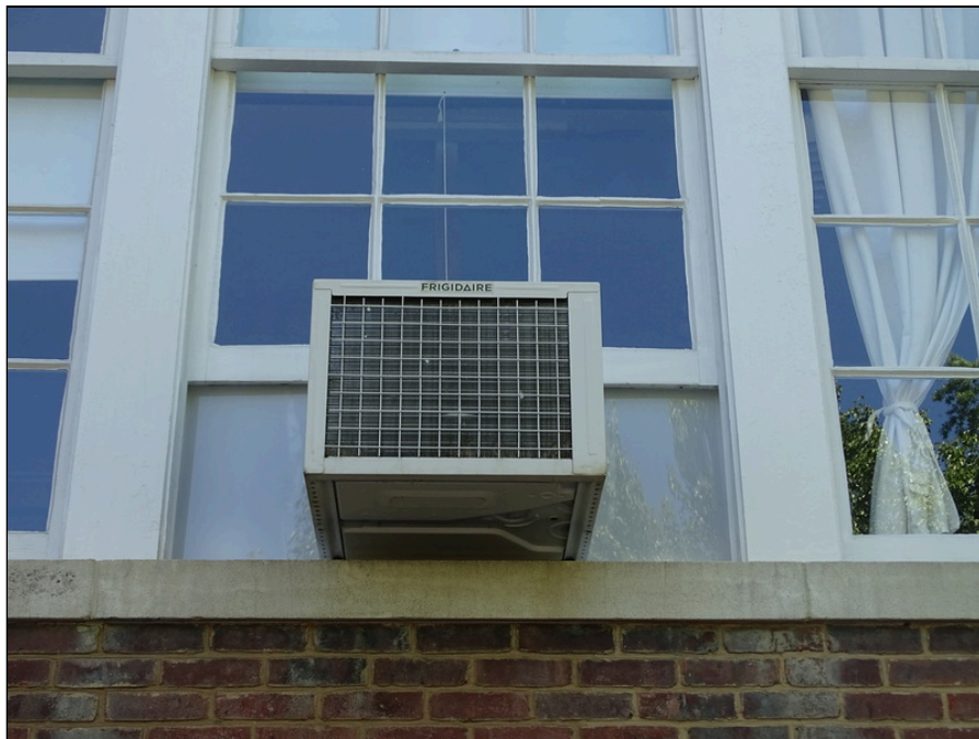
46 - Typical window air conditioning unit
