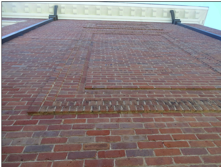
20 - Typical scupper and downspouts
