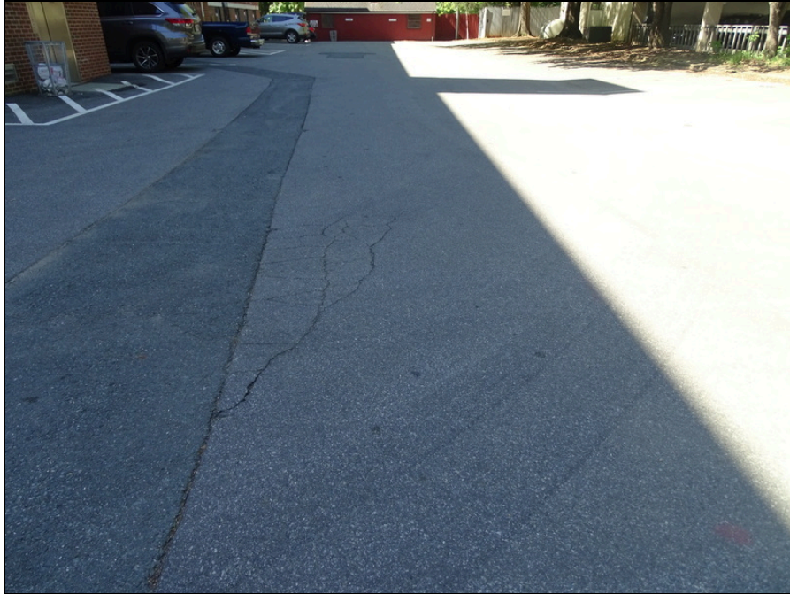
3 - Asphalt paving - note fading of striping and some cracking
