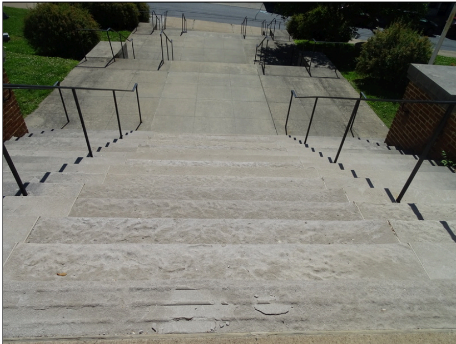
8 - Typical concrete steps- note spalling
