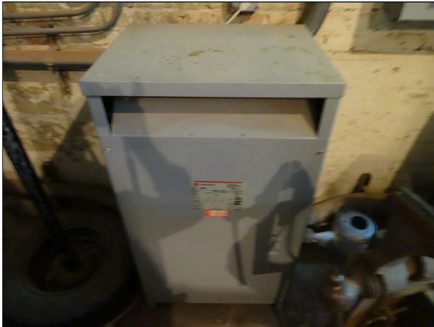
50 - Building transformer located in main utility room
