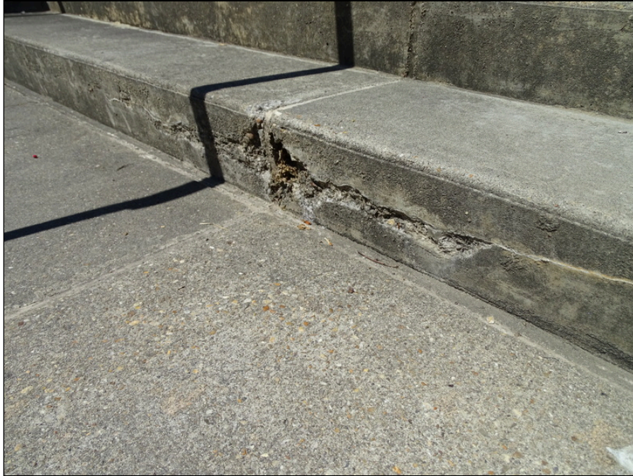
7 - Typical concrete sidewalks - note deterioration
