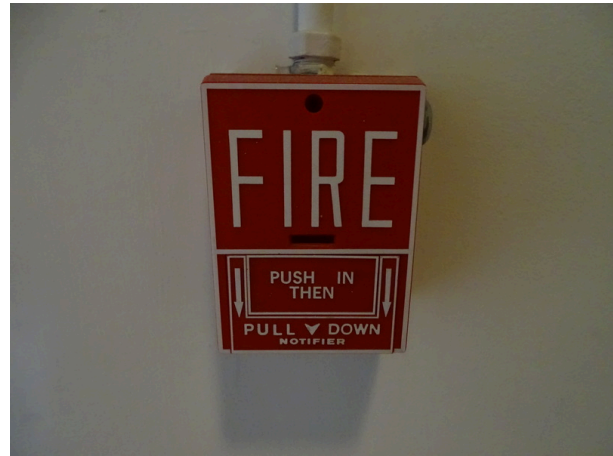
Typical fire alarm pull down station
