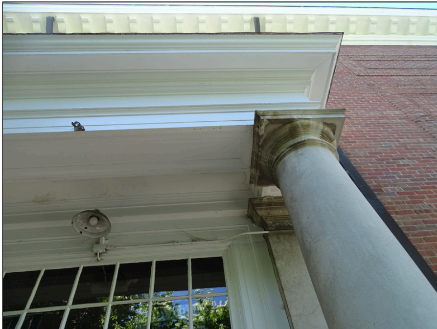
30 - Typical column - note efflorescence
