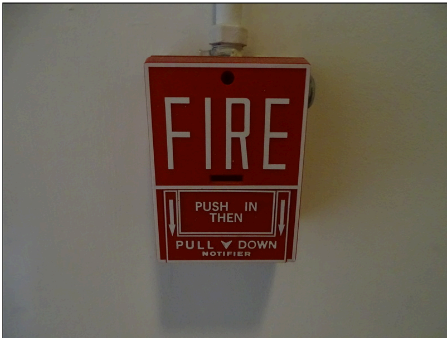
60 - Typical fire alarm pull down station
