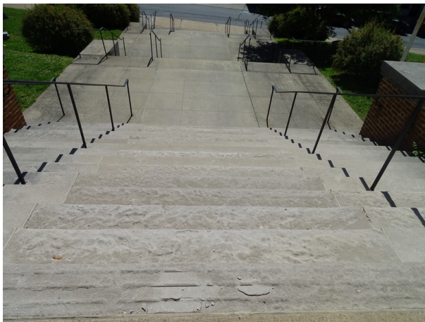
Typical concrete steps- note spalling
