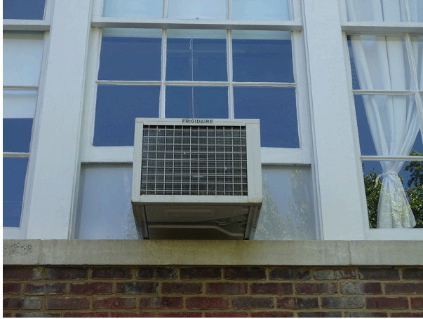
Typical window air conditioning unit
