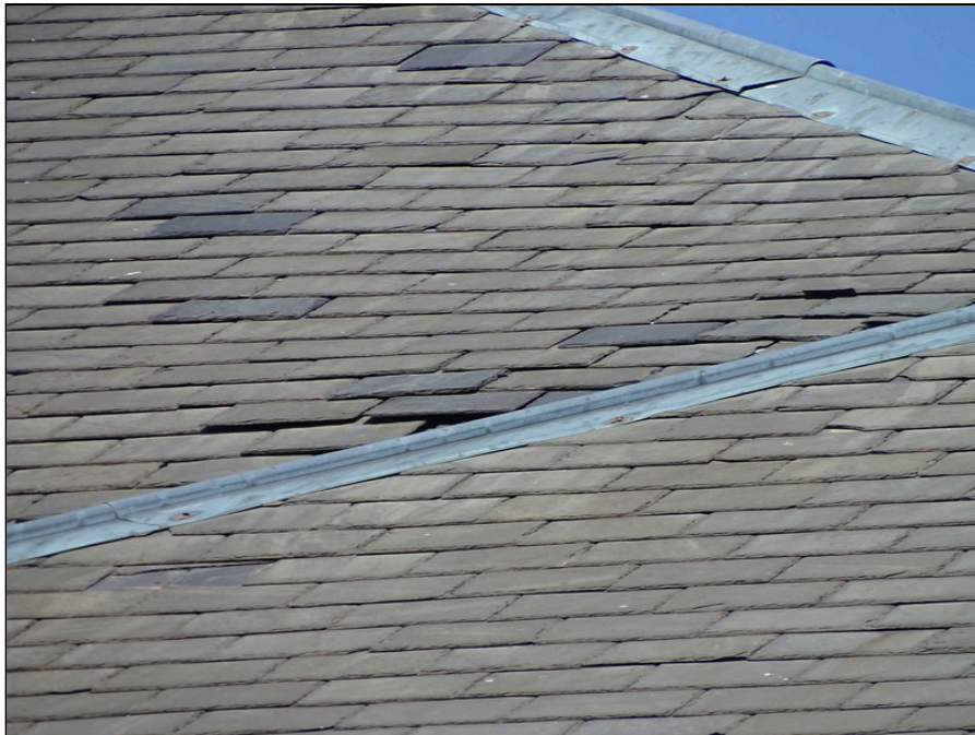
40 - Slate shingle roofing system - note deterioration
