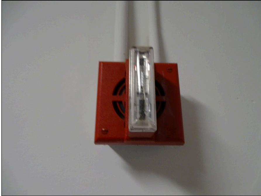
59 - Typical fire alarm strobe and bell
