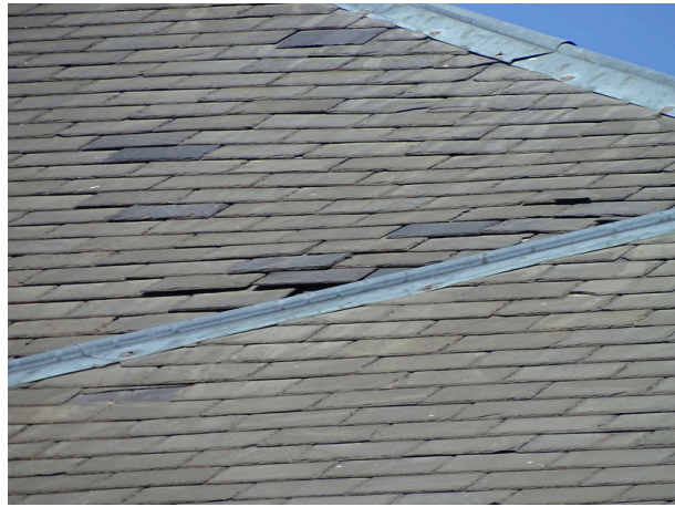
Slate shingle roofing system - note deterioration
