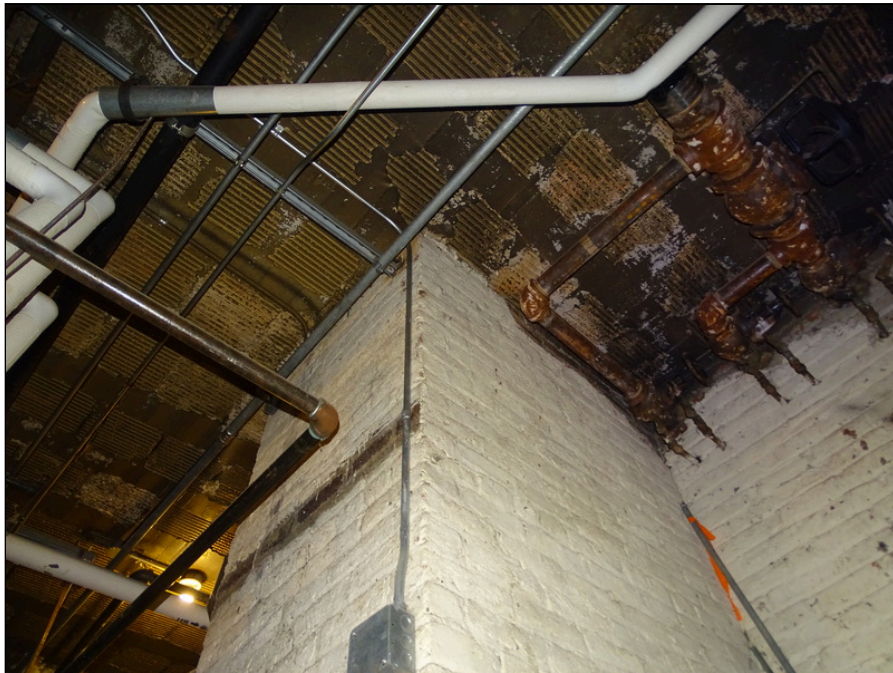
14 - Clay block first floor framing and masonry wall
