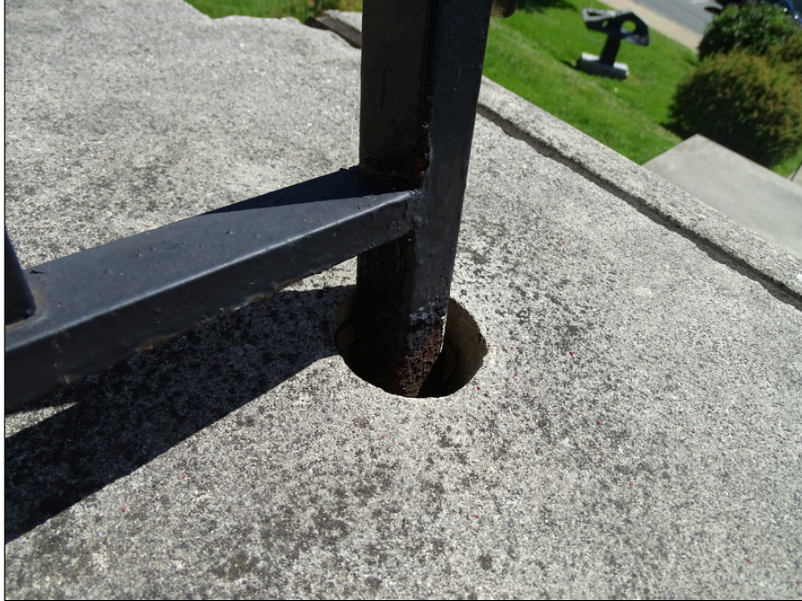
11 - Typical steel hand rail - note deterioration
