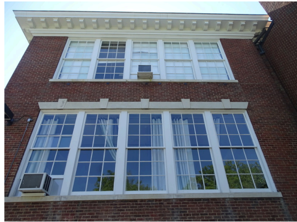
Typical exterior window units - note recent restoration
