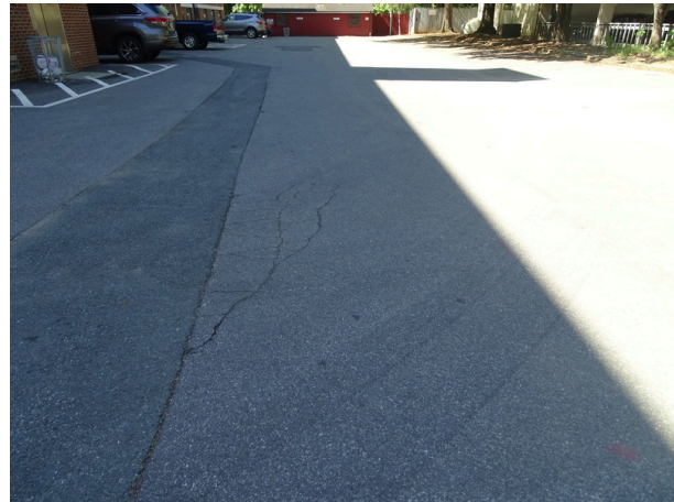
Asphalt paving - note fading of striping and some cracking
