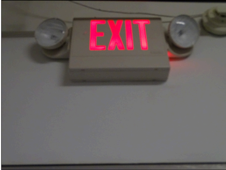
61 - Typical exit sign and emergency lighting
