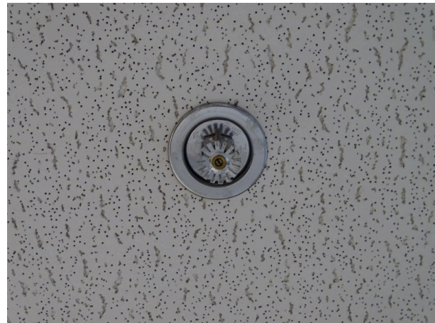
Typical sprinkler head
