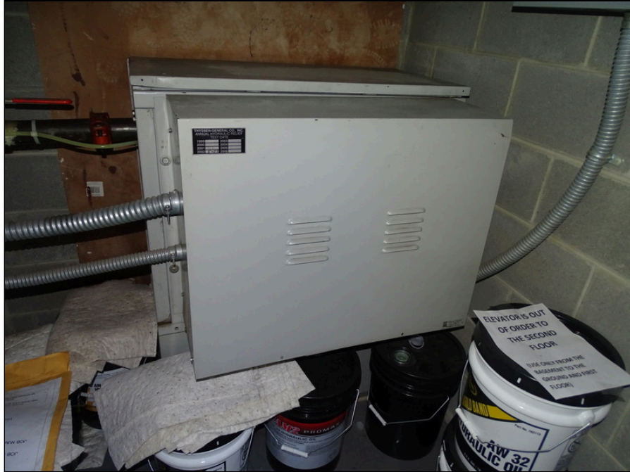
55 - Elevator machinery and controls
