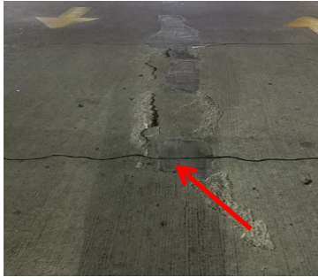
Figure 1: Failing Concrete Patch
