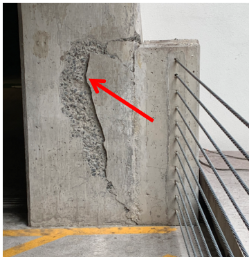
Figure 3: Concrete Spall
