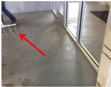
Figure 2: Concrete Delamination
