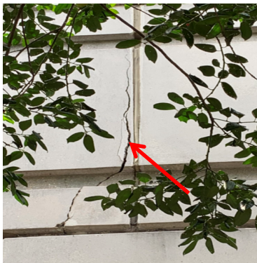
Figure 6: Wide Crack
