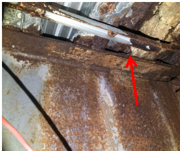
Figure 9: Structural Steel Corrosion and Scaling
