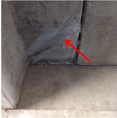
Figure 7: Leaking and Leaching Concrete
