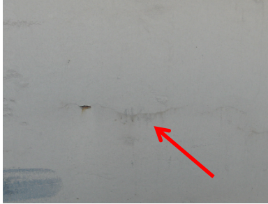
Figure 4: Fine Crack
