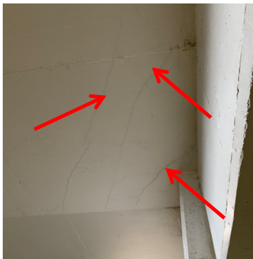
Figure 5: Medium Crack
