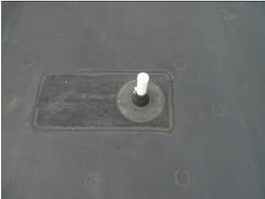
36 - Typical plumbing penetration and patching
