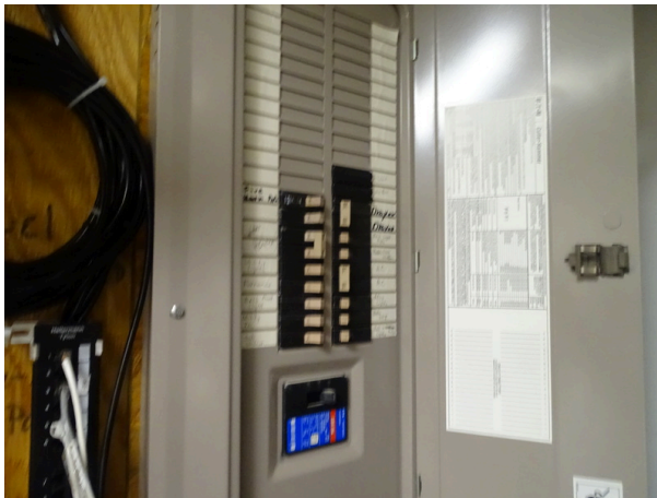
Typical electrical circuit breaker panel
