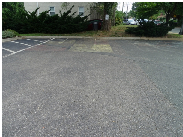
Asphalt parking - note faded striping
