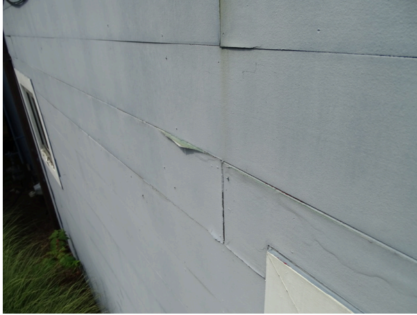
Typical exterior wall - note peeling paint and deterioration
