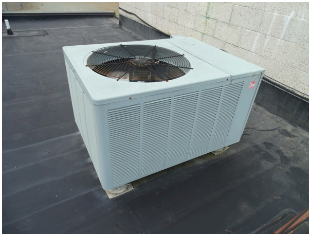
Typical condenser unit
