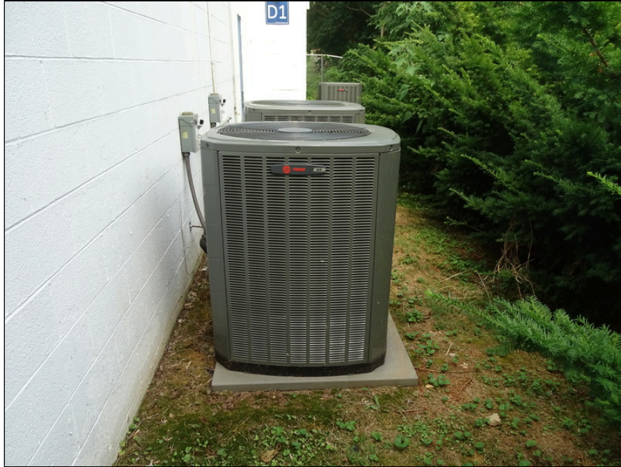
47 - Typical condenser unit at north building
