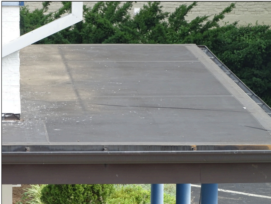
42 - Single-ply roofing system
