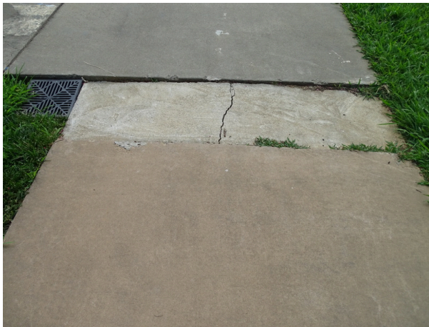
Typical concrete sidewalk - note deterioration
