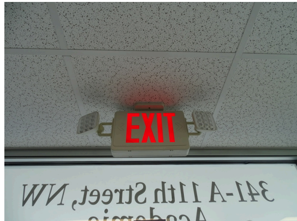
Exit sign and emergency lighting
