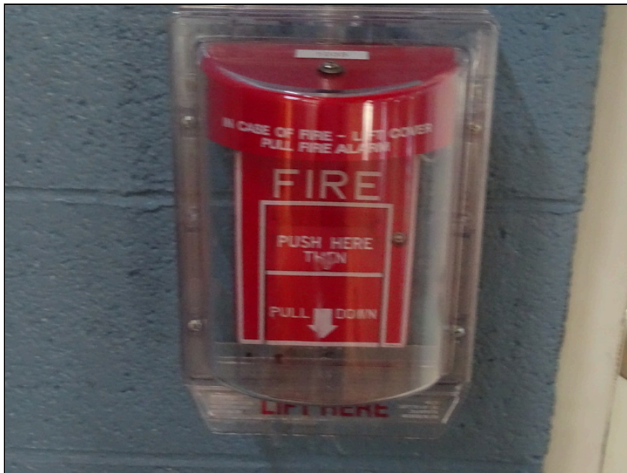
62 - Fire alarm pull down station
