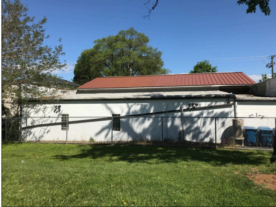
85 - Slanted Downspout - North Building
