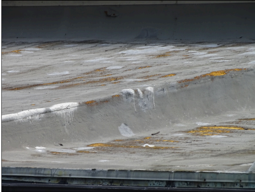
37 - Coated polyurethane roofing system
