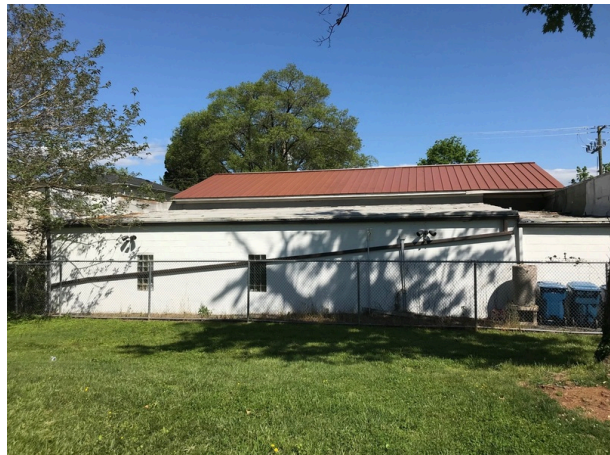
Slanted Downspout - North Building
