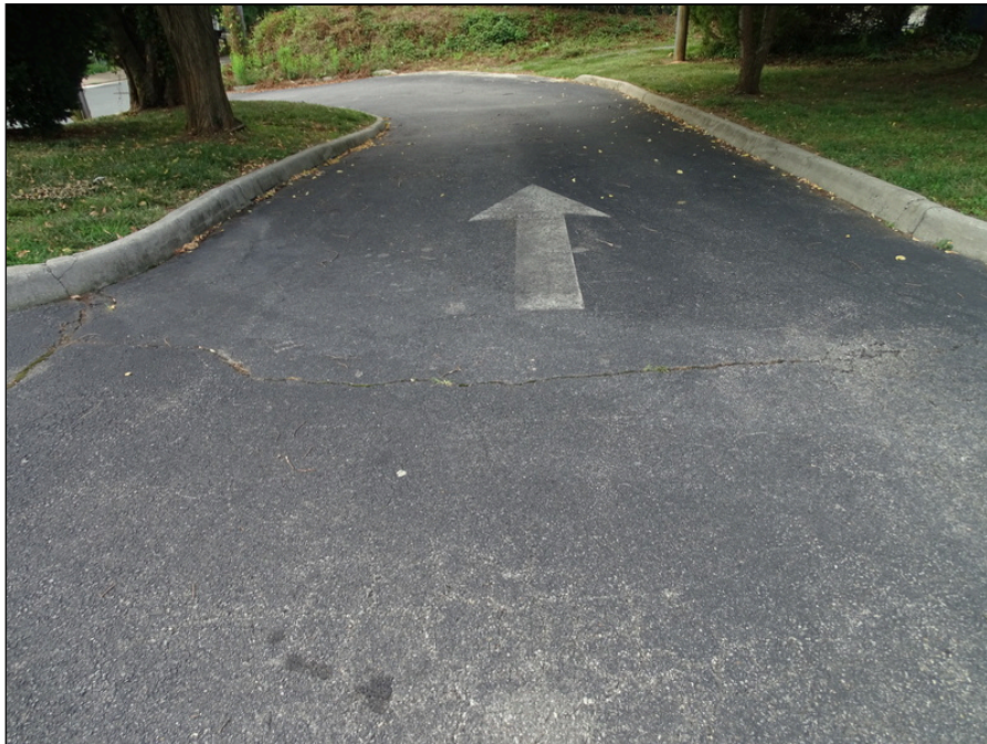
4 - Asphalt drive lane looking north - note cracking
