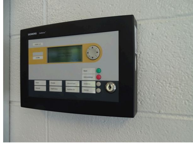
Fire alarm control panel
