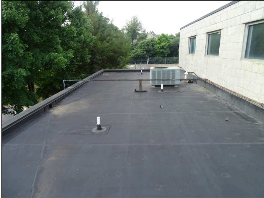
35 - Single-ply roofing system
