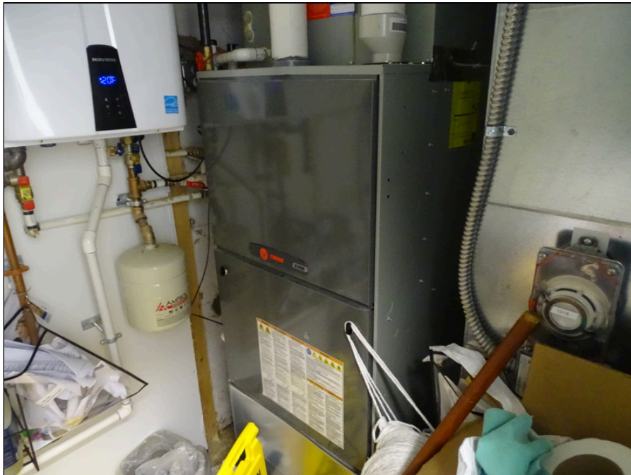
46 - Typical furnace-air handler unit at north building
