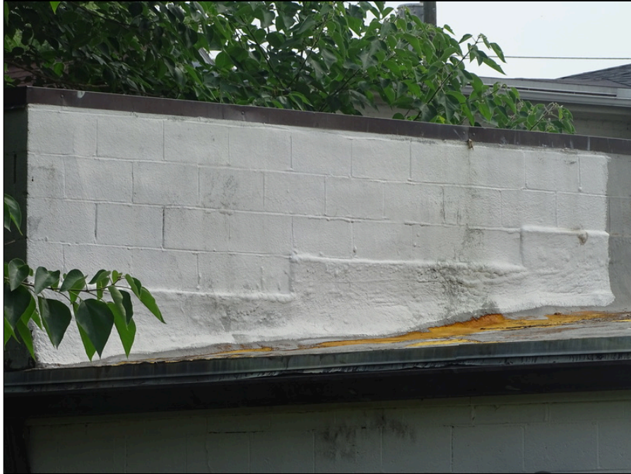
39 - Typical parapet wall - note deterioration
