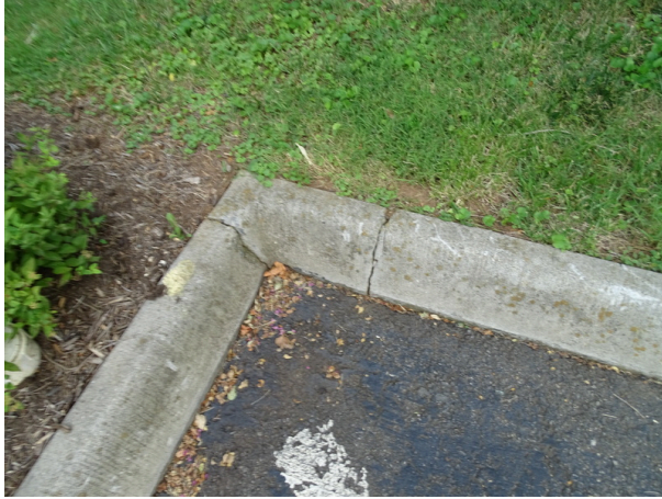
Typical concrete curb - note deterioration
