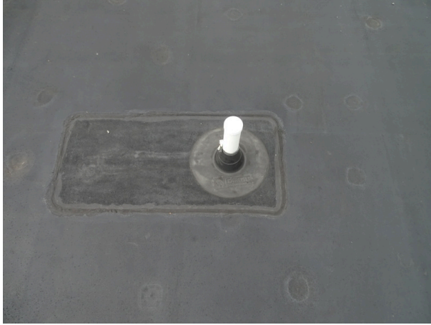
Typical plumbing penetration and patching
