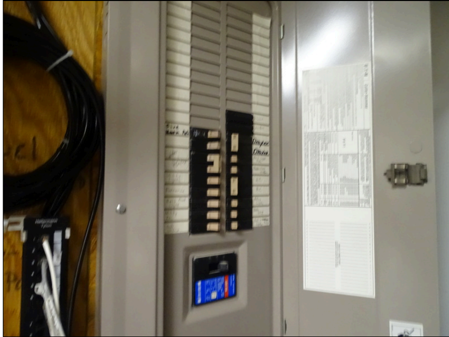
55 - Typical electrical circuit breaker panel
