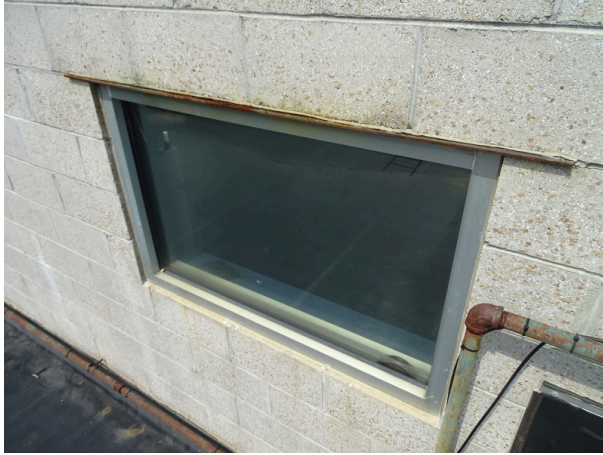
Typical exterior windows - note gasket deterioration
