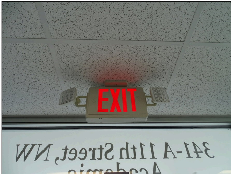
64 - Exit sign and emergency lighting
