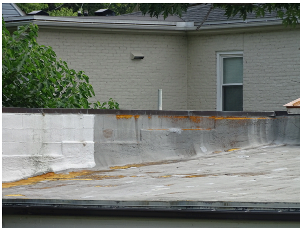
Typical parapet wall - note deterioration
