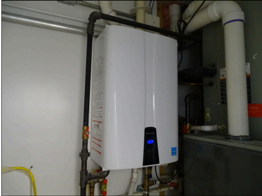
43 - Tankless water heater in north building
