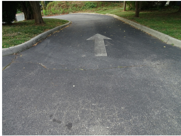
Asphalt drive lane looking north - note cracking
