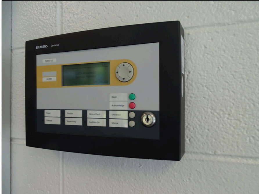
59 - Fire alarm control panel
