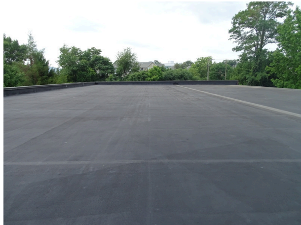
Single-ply roofing system
