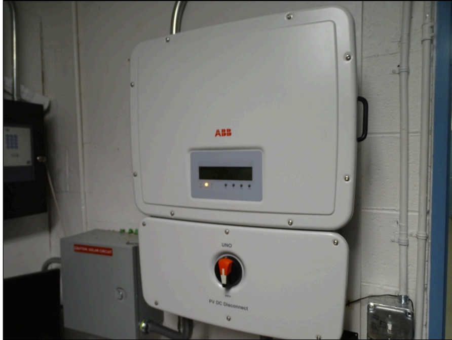
57 - Solar Power System electronic controls located in north building electrical room
