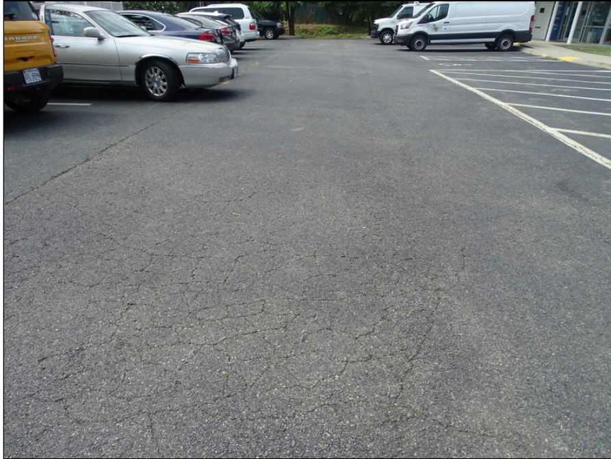
3 - Asphalt drive lane and parking - note cracking
