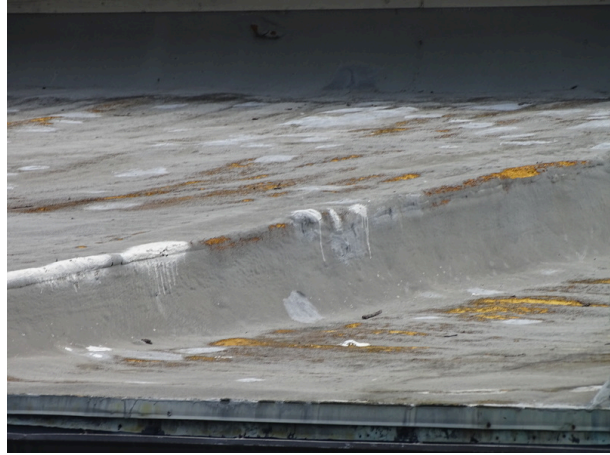
Coated polyurethane roofing system
