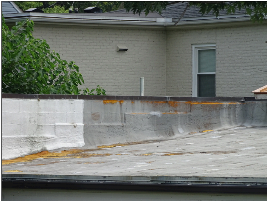
38 - Typical parapet wall - note deterioration
