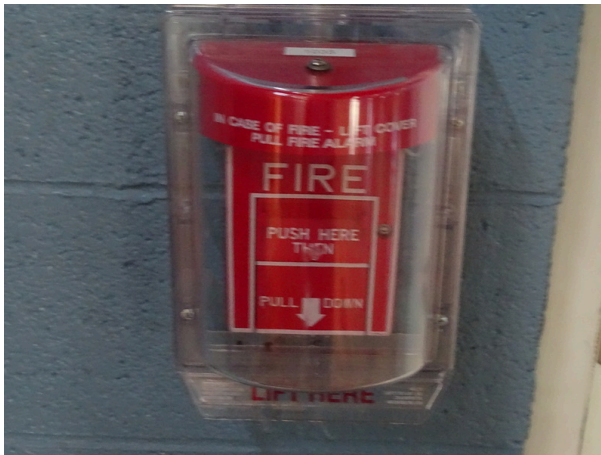
Fire alarm pull down station
