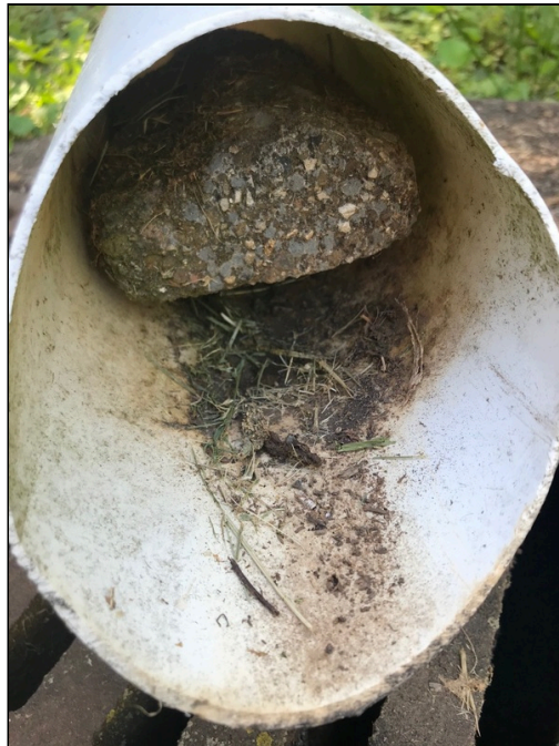
86 - Rock Weighing Down CB Drain
