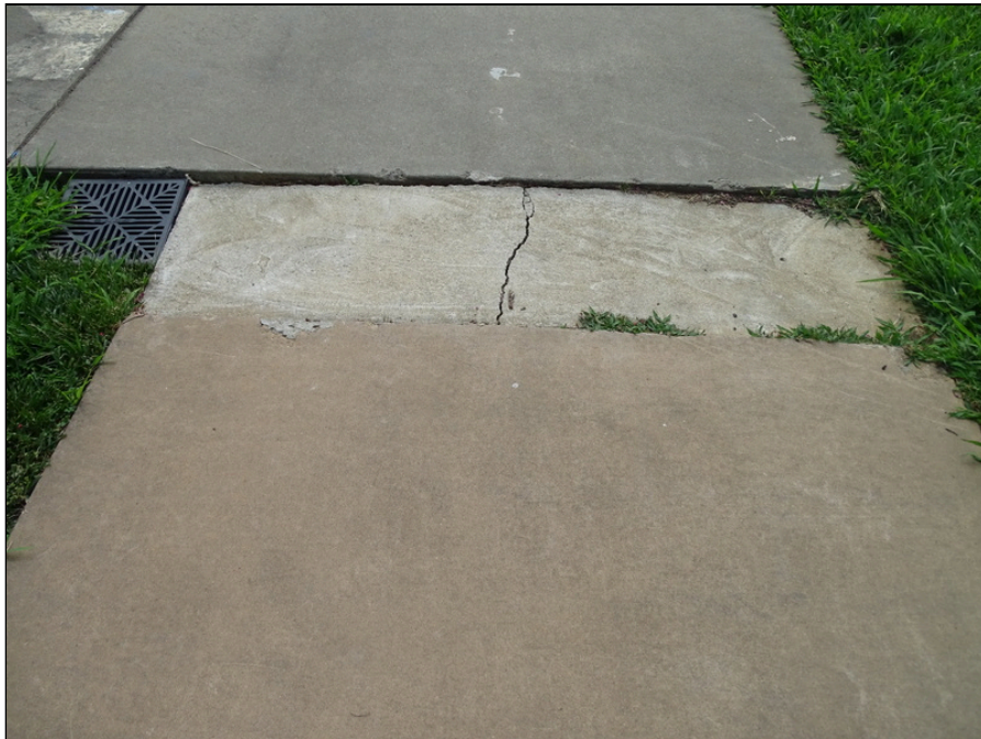
8 - Typical concrete sidewalk - note deterioration
