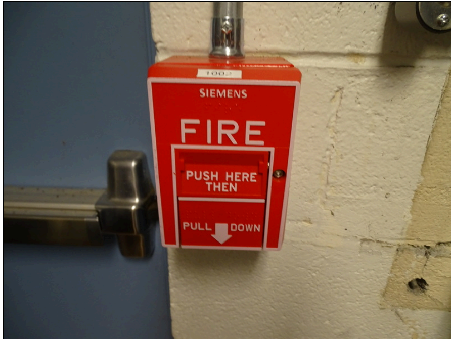
63 - Fire alarm pull down station
