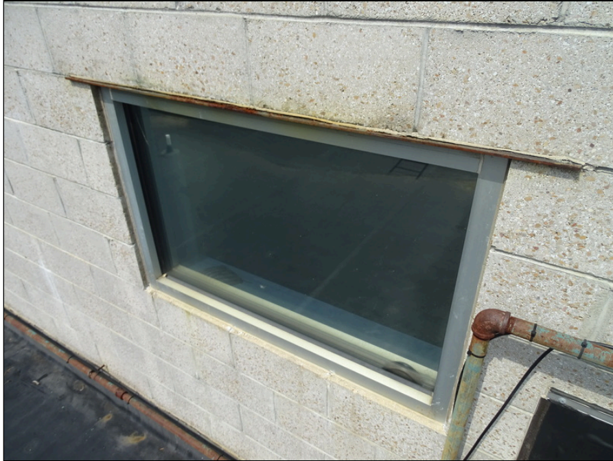
31 - Typical exterior windows - note gasket deterioration
