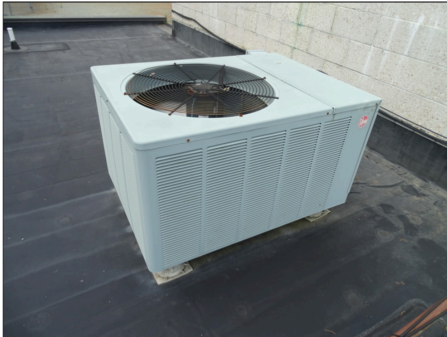
48 - Typical condensing unit
