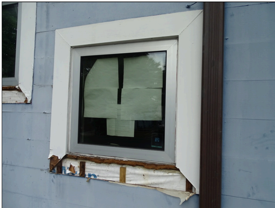
30 - Typical exterior windows - note deterioration
