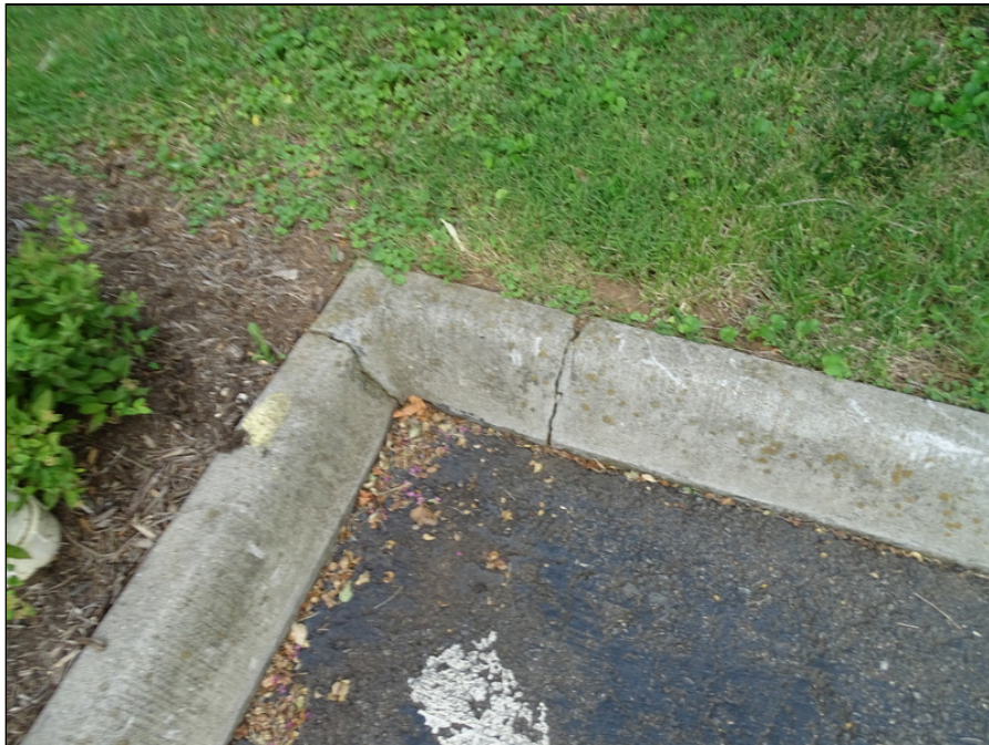
10 - Typical concrete curb - note deterioration
