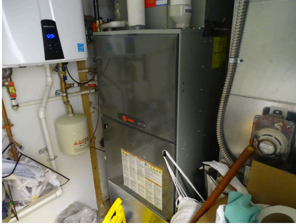
Typical furnace-air handler unit at north building
