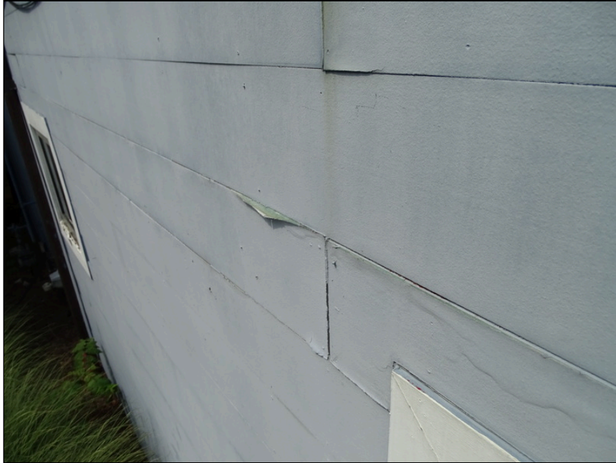
23 - Typical exterior wall - note peeling paint
