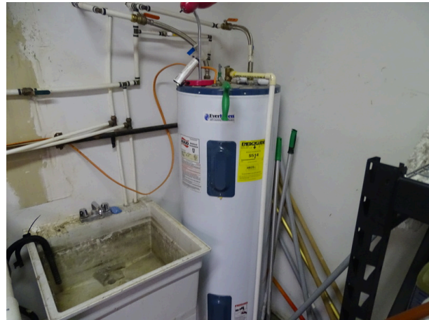
Electric water heater in south building
