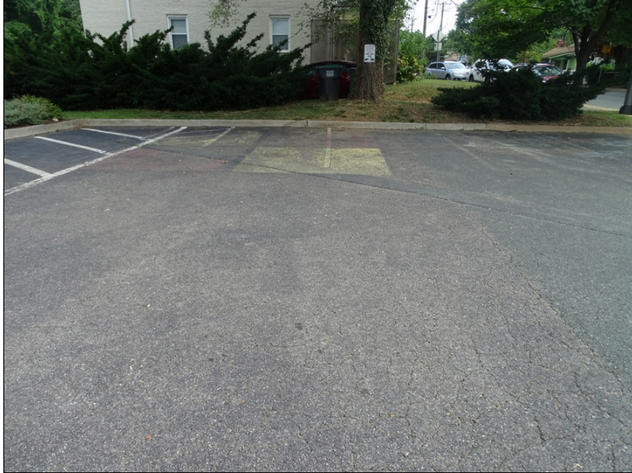
7 - Asphalt parking - note faded stripping
