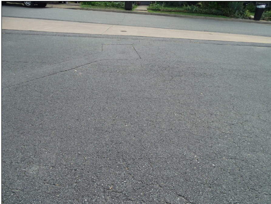
6 - Asphalt drive lane looking east - note cracking
