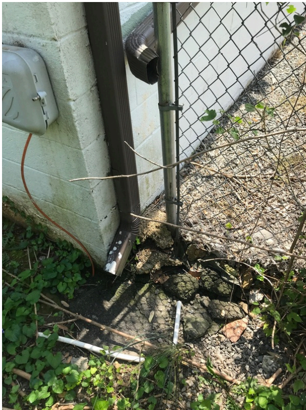
Downspout Discharge - North Building
