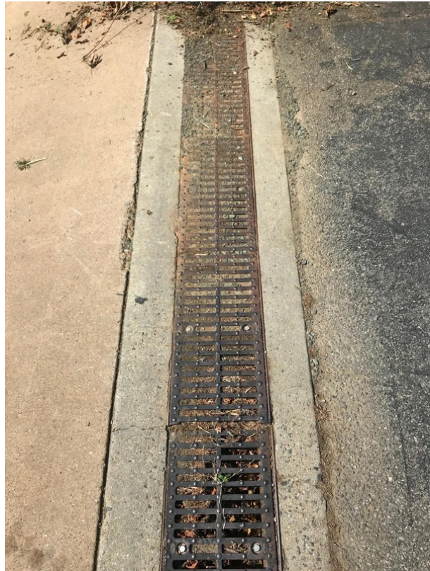
Channel Drain - Clogged
