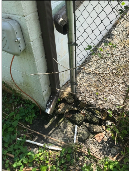
87 - Downspout Discharge - North Building
