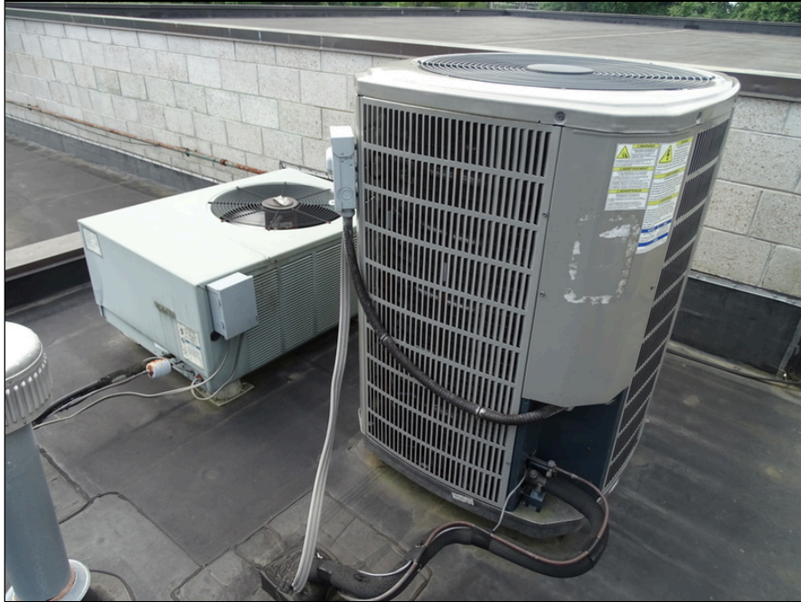
49 - Typical condensing unit
