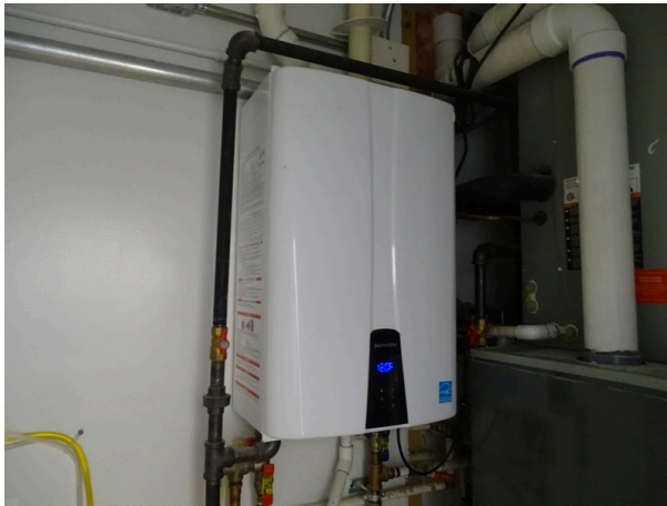
Tankless water heater in north building
