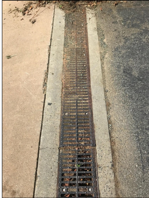
83 - Channel Drain - Clogged
