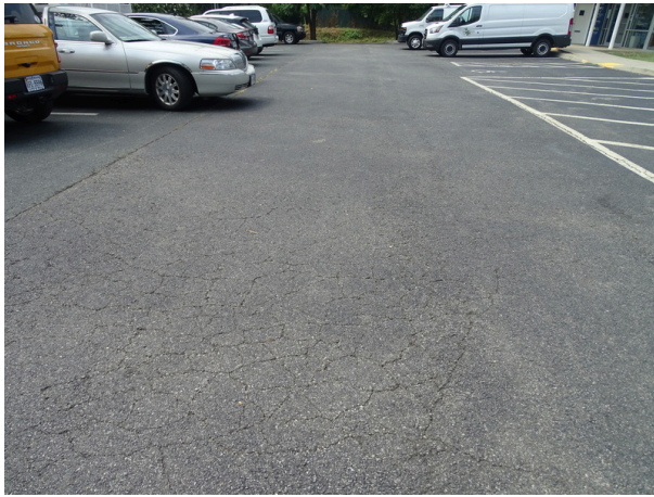
Asphalt drive lane and parking - note cracking
