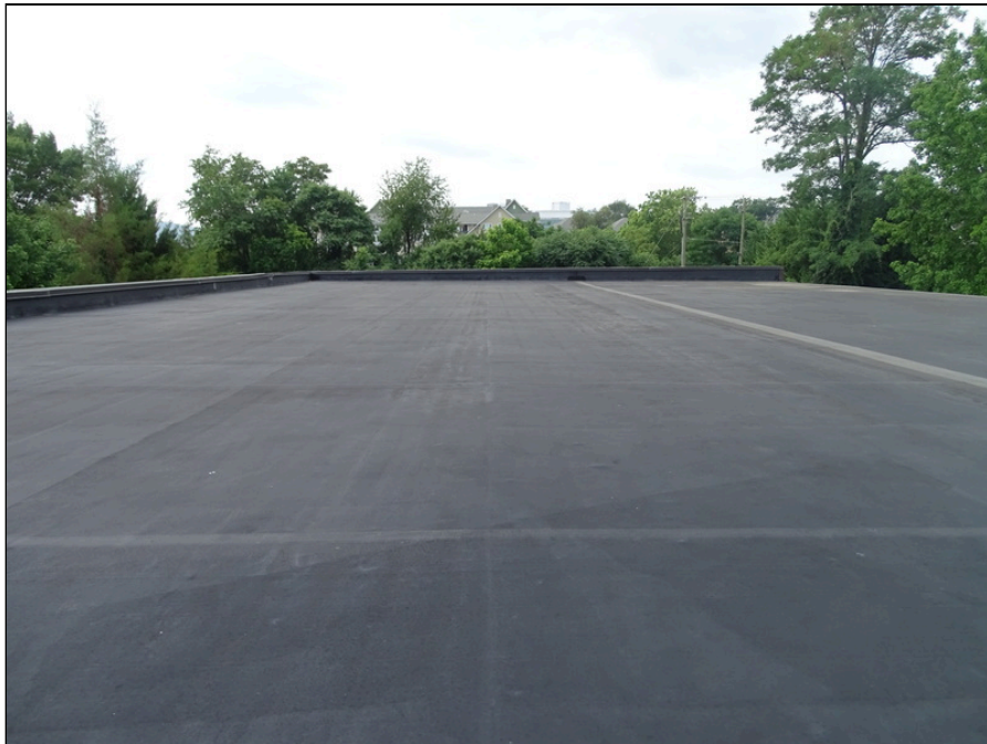
34 - Single-ply roofing system
