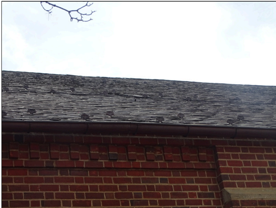
28 - Slate shingle roofing system - note deterioration
