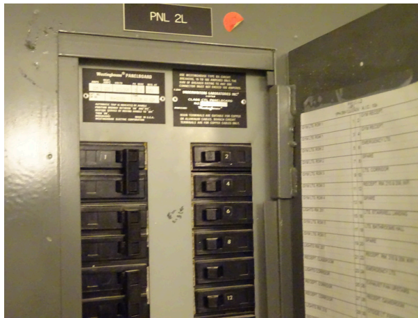
Typical older electrical circuit breaker panel
