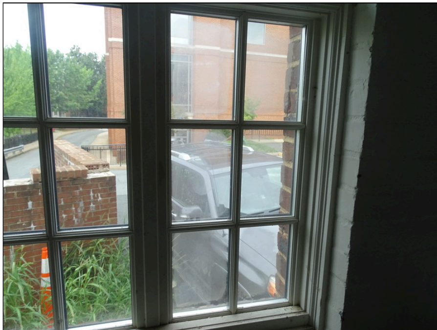
24 - Exterior windows - note fogging and deterioration
