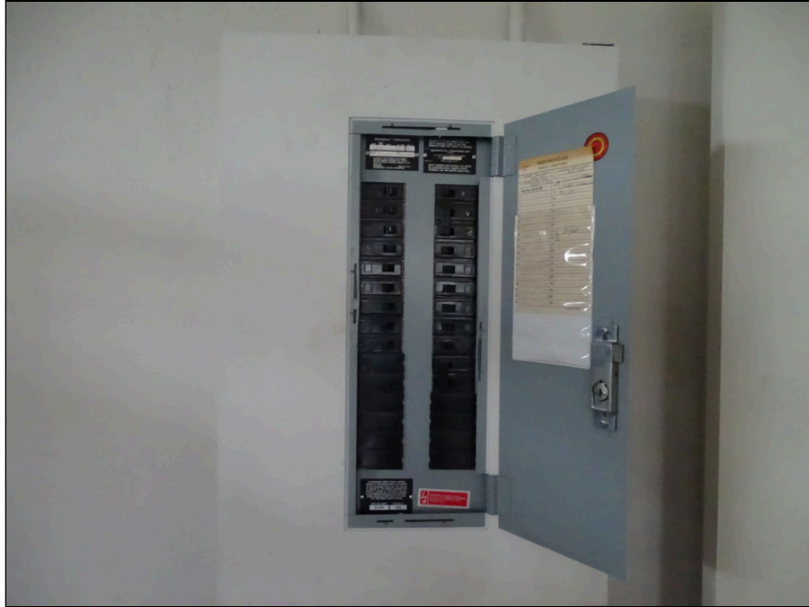
61 - Typical newer electrical circuit breaker panel
