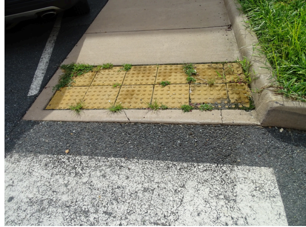
Accessible curb cut ramp with truncated domes
