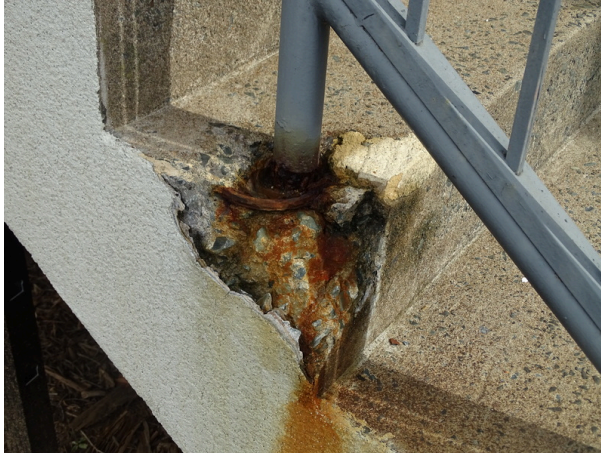
Concrete steps on south side of the building - note deterioration
