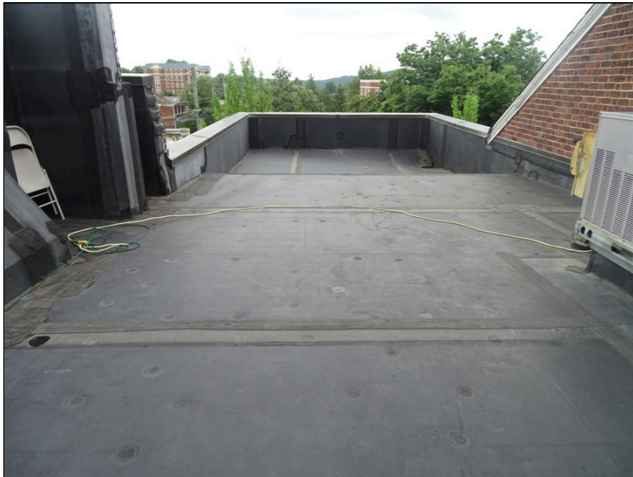
30 - Single-ply membrane roofing system - note deterioration
