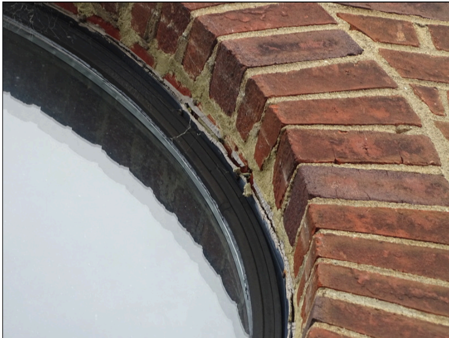
14 - Building exterior sealants - note deterioration
