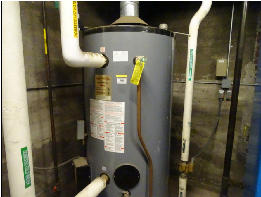
40 - Natural gas domestic water heater
