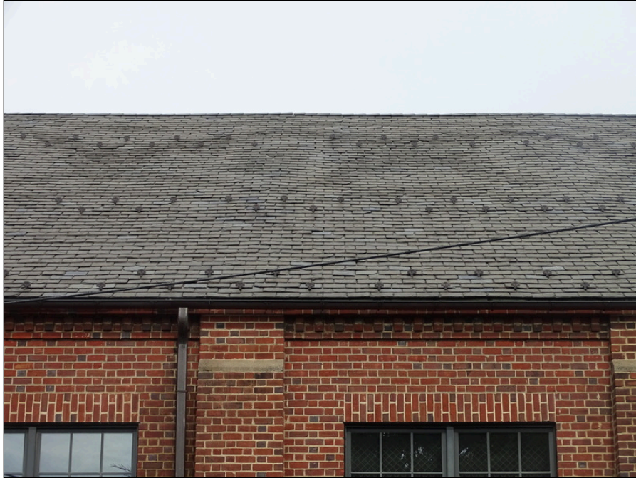
25 - Slate shingle roofing system - note deterioration
