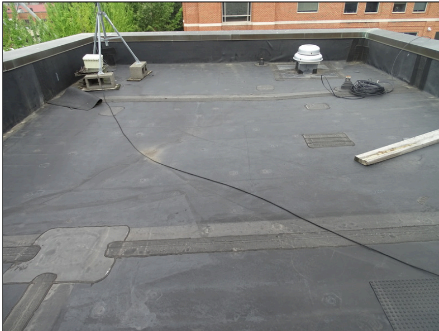
36 - Single-ply membrane roofing system parapet wall - note deterioration
