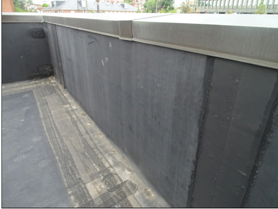
33 - Single-ply membrane roofing system parapet wall - note deterioration
