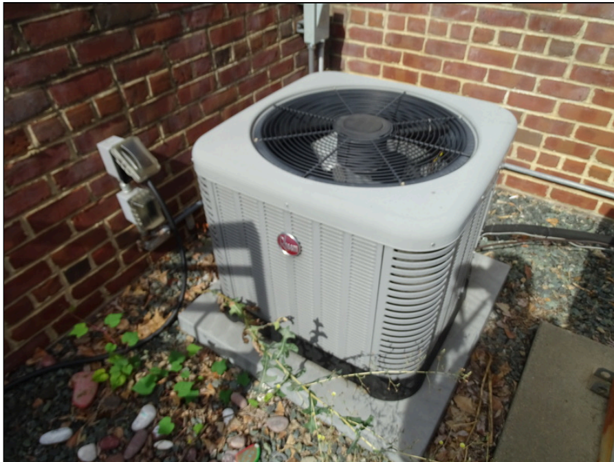
46 - Split system condenser unit located on east side of the building
