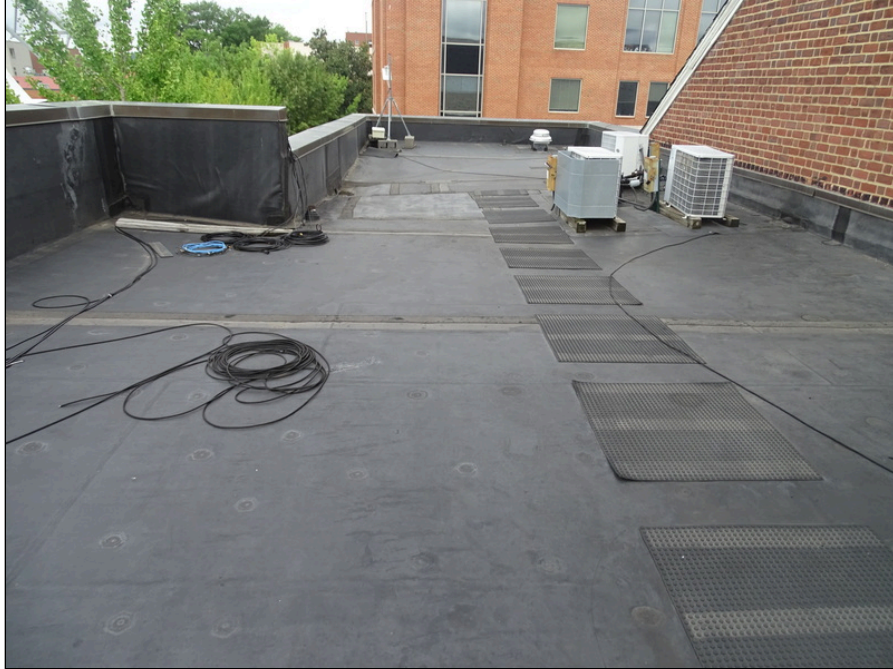
37 - Single-ply membrane roofing system parapet wall - note deterioration
