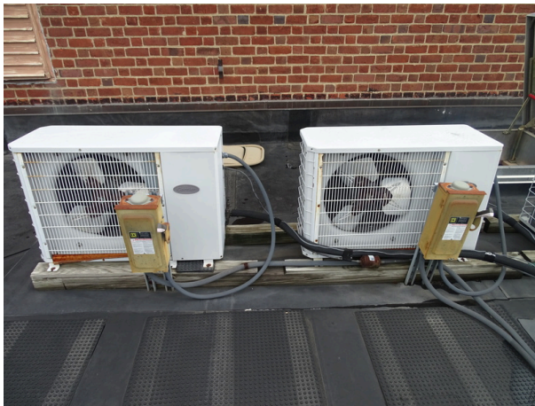
Split system ductless outdoor units
