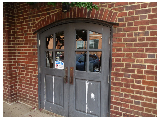
Typical wood doors - note deterioration
