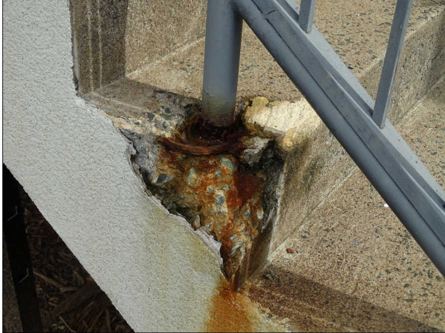
7 - Concrete steps on south side of the building - note deterioration
