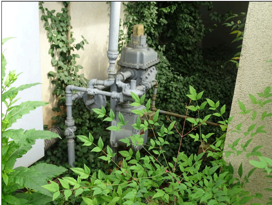
38 - Natural gas utility supply and meter
