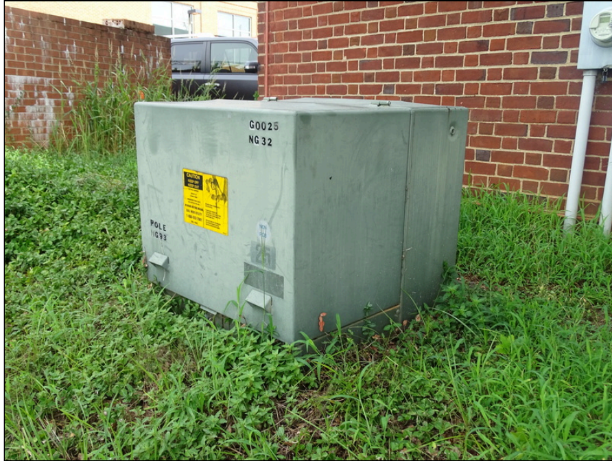
57 - Electrical utility transformer
