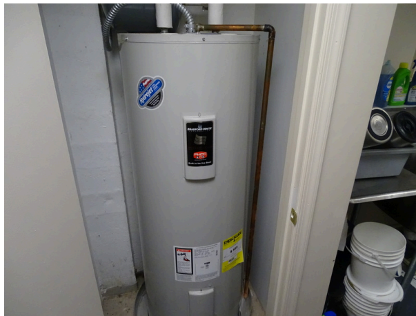
Electric domestic water heater
