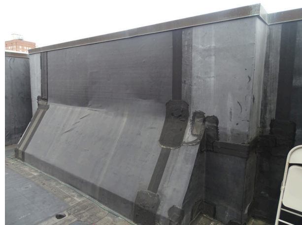
Single-ply membrane roofing system parapet wall - note patching and deterioration
