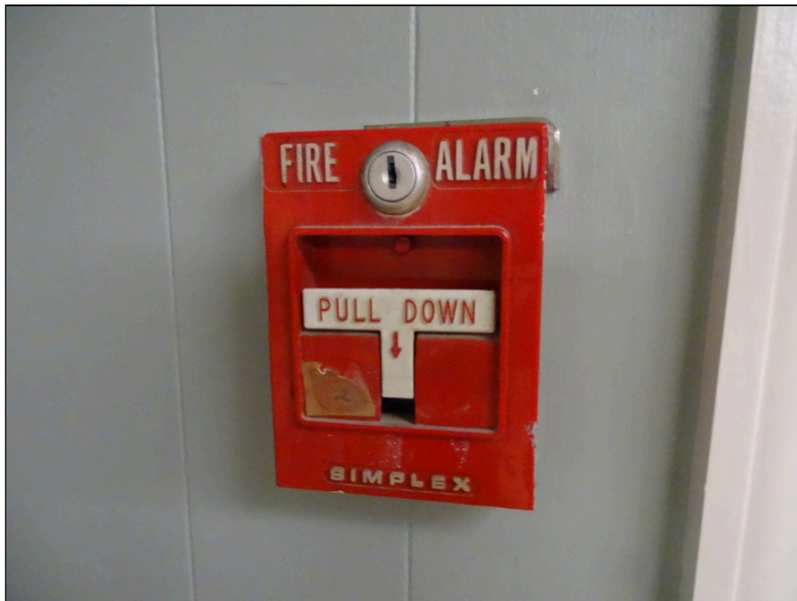
64 - Fire alarm pull station
