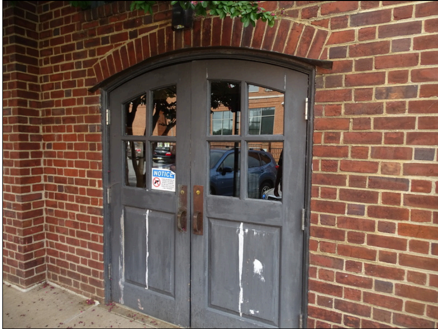
21 - Typical wood doors - note deterioration
