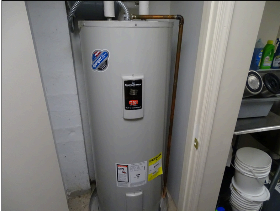
39 - Electric domestic water heater
