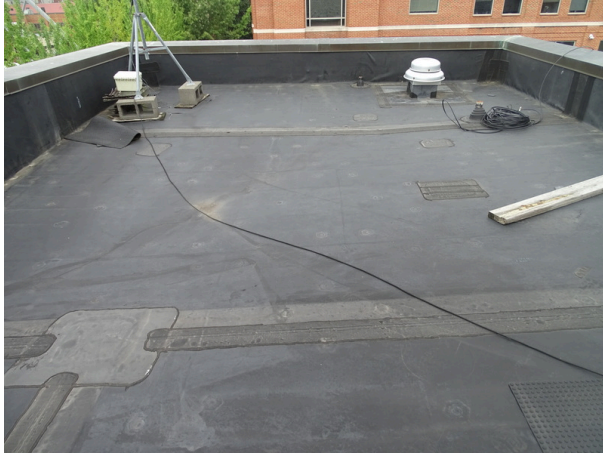
Single-ply membrane roofing system parapet wall - note deterioration
