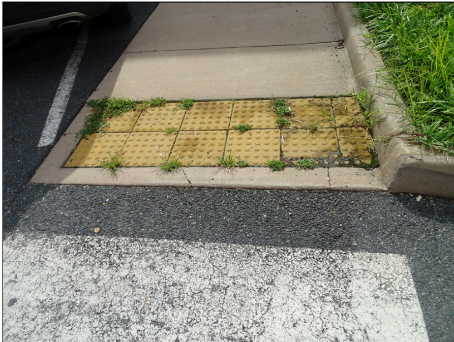
84 - Accessible curb cut ramp with truncated domes
