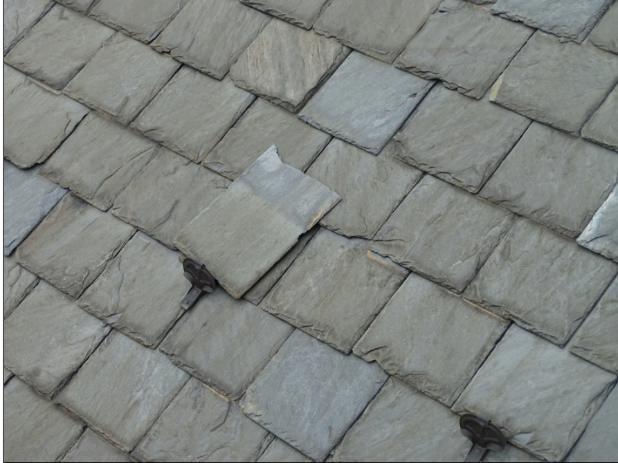
29 - Slate shingle roofing system - note deterioration
