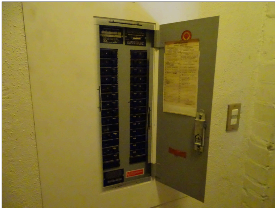
60 - Typical older electrical circuit breaker panel
