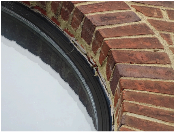
Building exterior sealants - note deterioration
