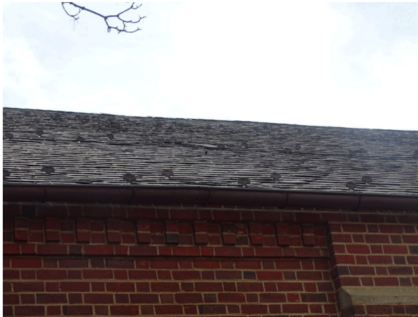
Slate shingle roofing system - note deterioration
