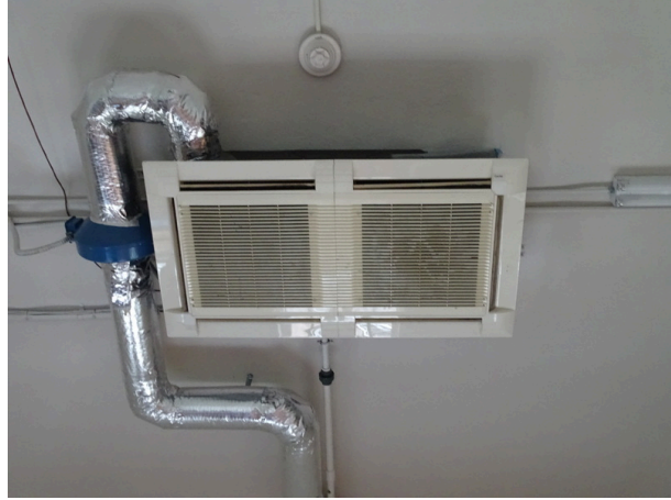
Split system ductless interior unit
