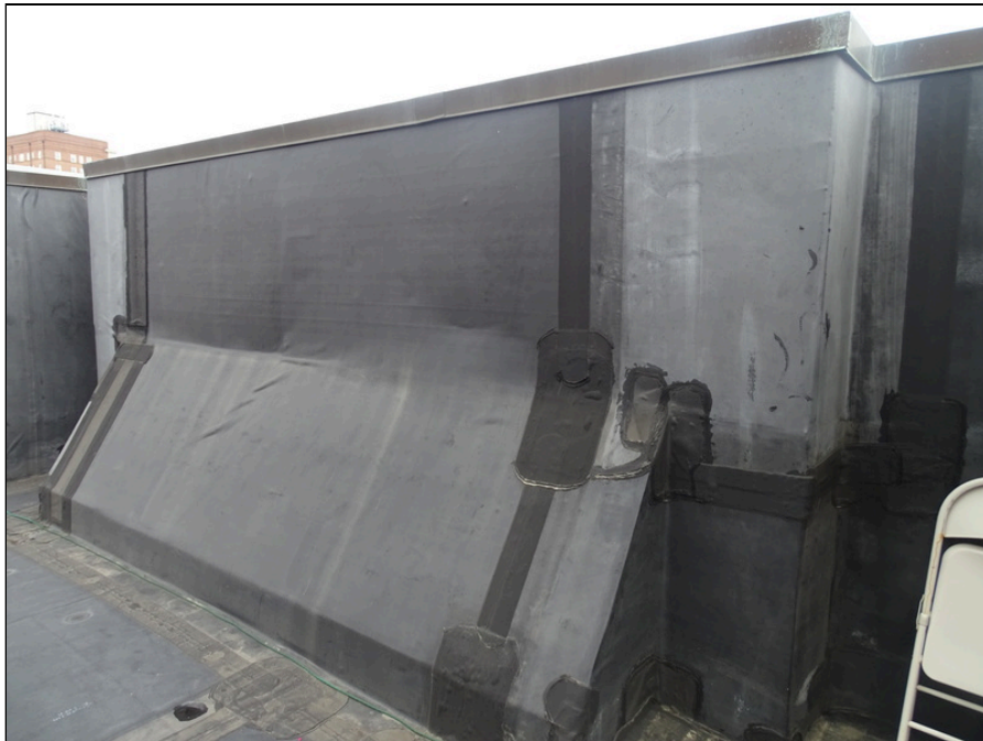
34 - Single-ply membrane roofing system parapet wall - note patching and deterioration
