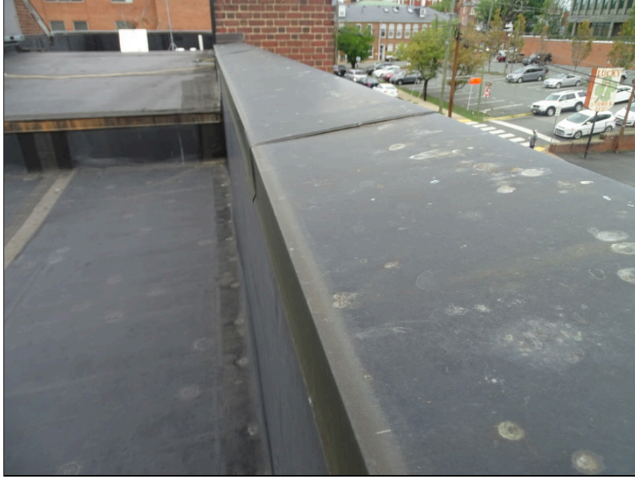
35 - Single-ply membrane roofing system parapet wall - note deterioration
