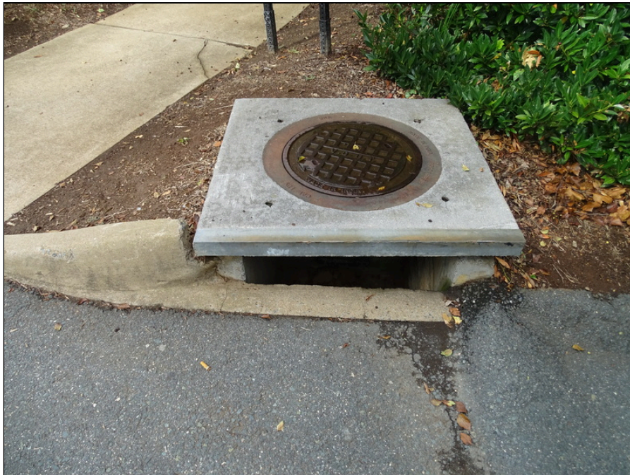
2 - Storm sewer curb inlet
