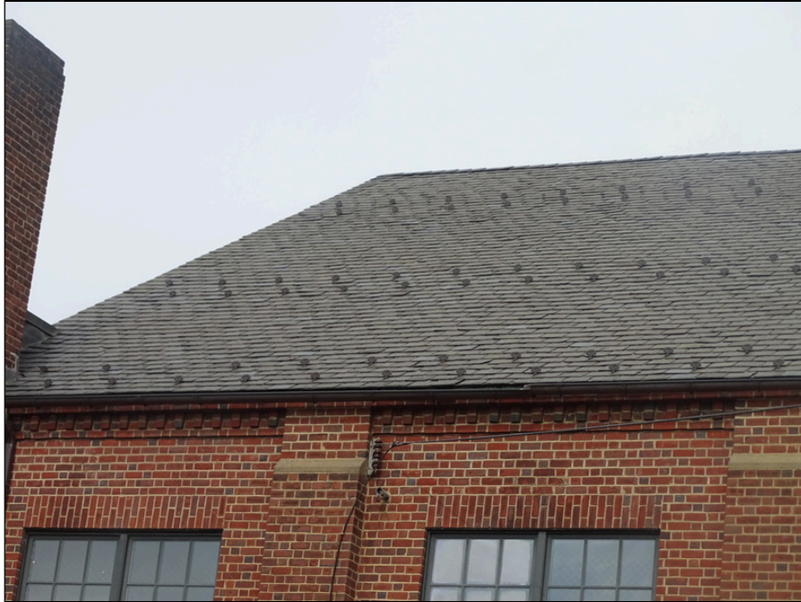
27 - Slate shingle roofing system - note deterioration
