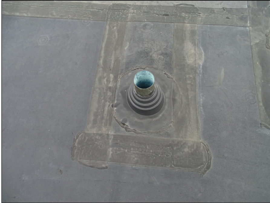
31 - Single-ply membrane roofing system - plumbing penetration
