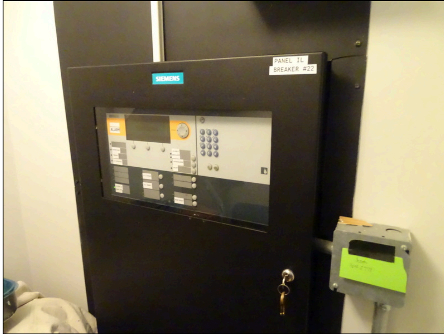
63 - Fire alarm control panel
