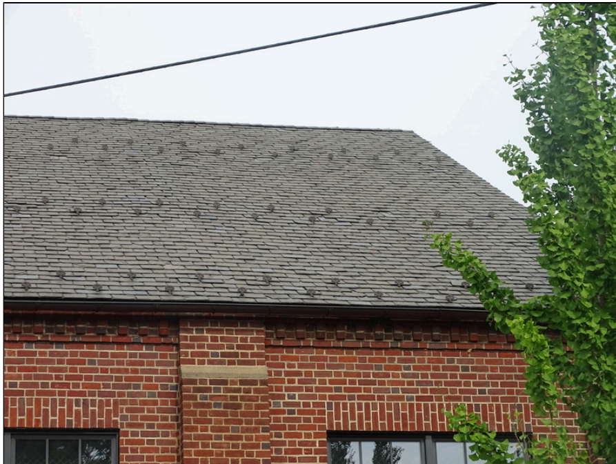
26 - Slate shingle roofing system - note deterioration
