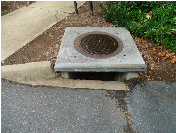
Storm sewer curb inlet
