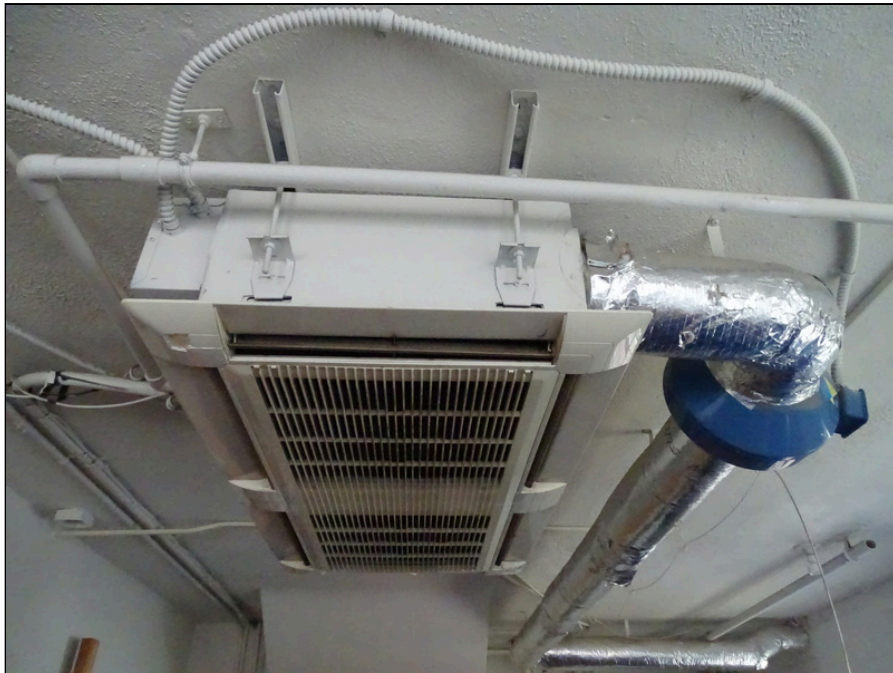
52 - Split system ductless interior unit
