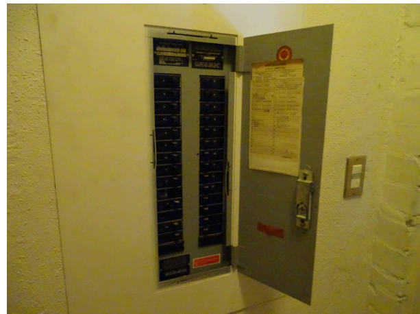
Typical older electrical circuit breaker panel
