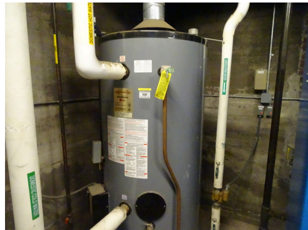
Natural gas domestic water heater
