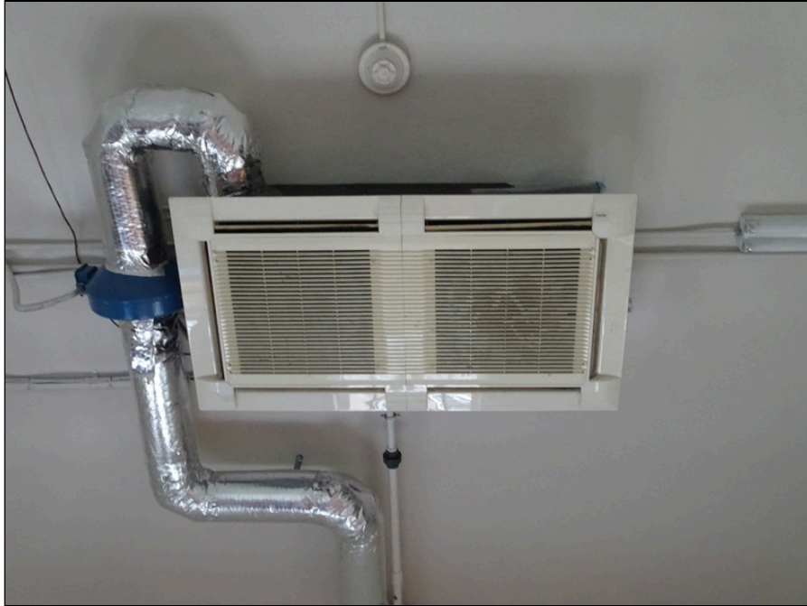
51 - Split system ductless interior unit
