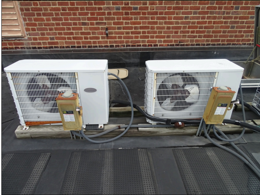
53 - Split system ductless outdoor units
