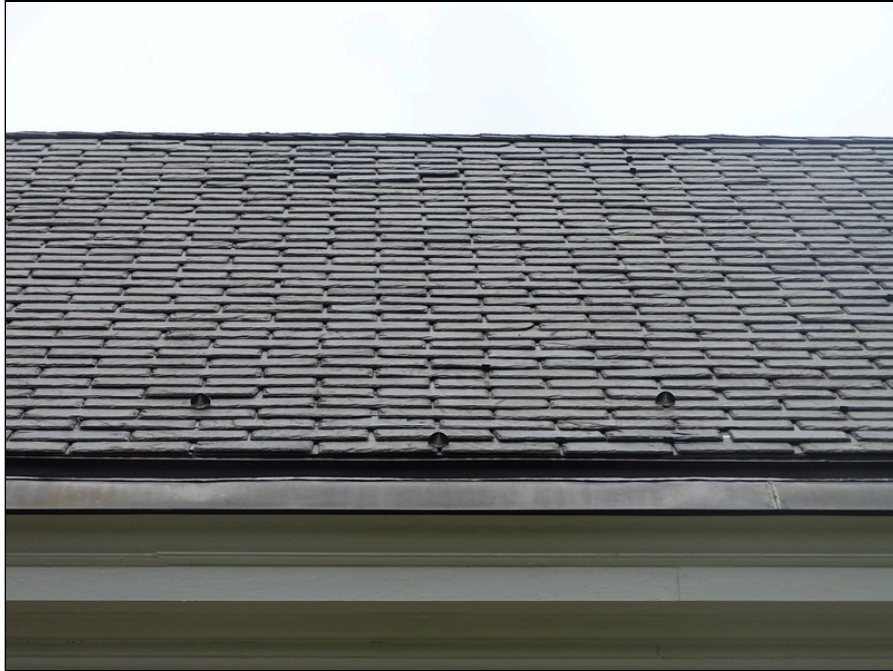
45 - Slate shingle roofing system
