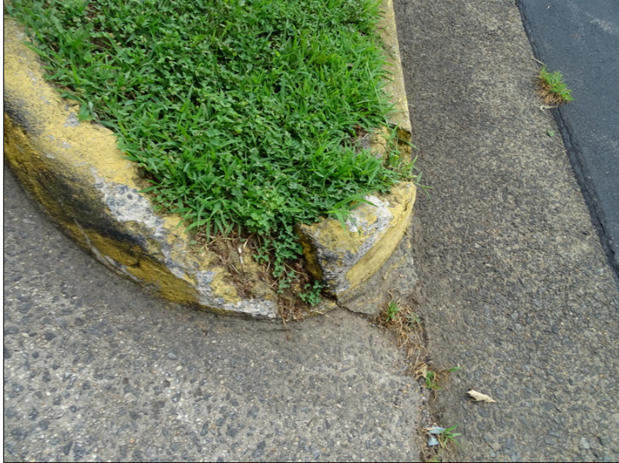
13 - concrete curb - note deterioration
