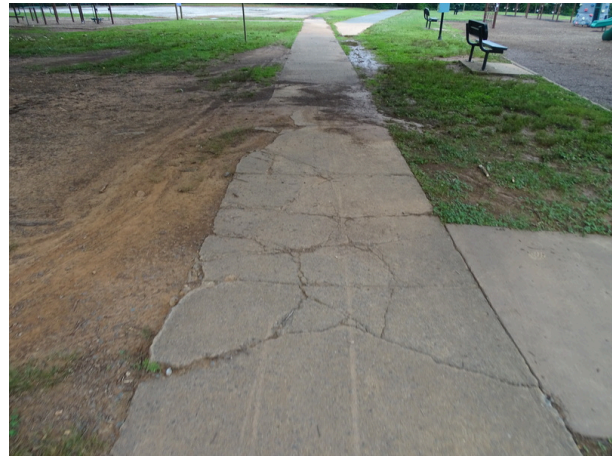
Typical concrete sidewalk - note cracking
