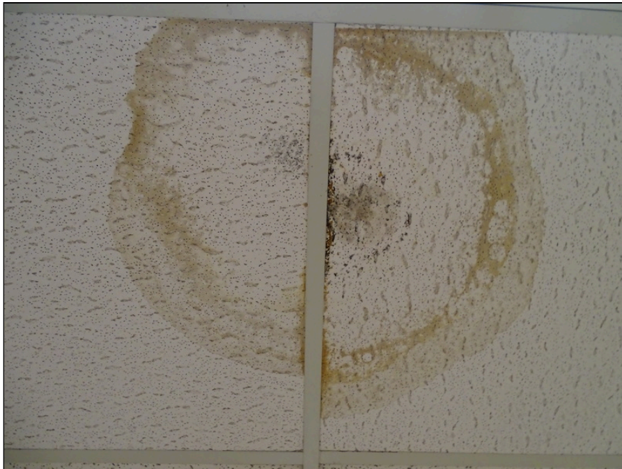
84 - Typical ceiling - note water leakage
