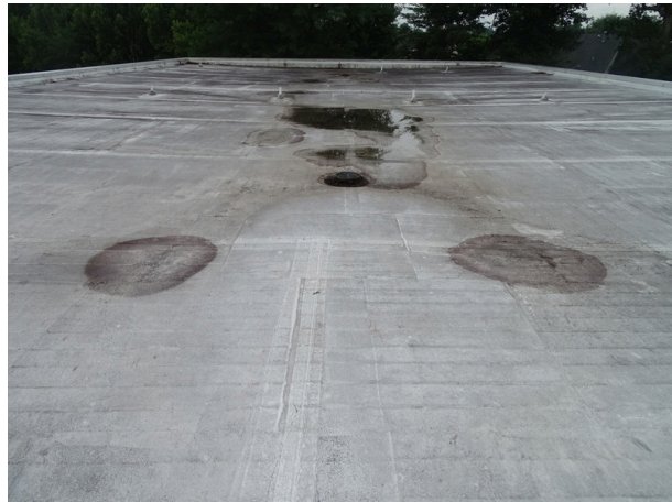
Single-ply membrane roofing system - note ponding
