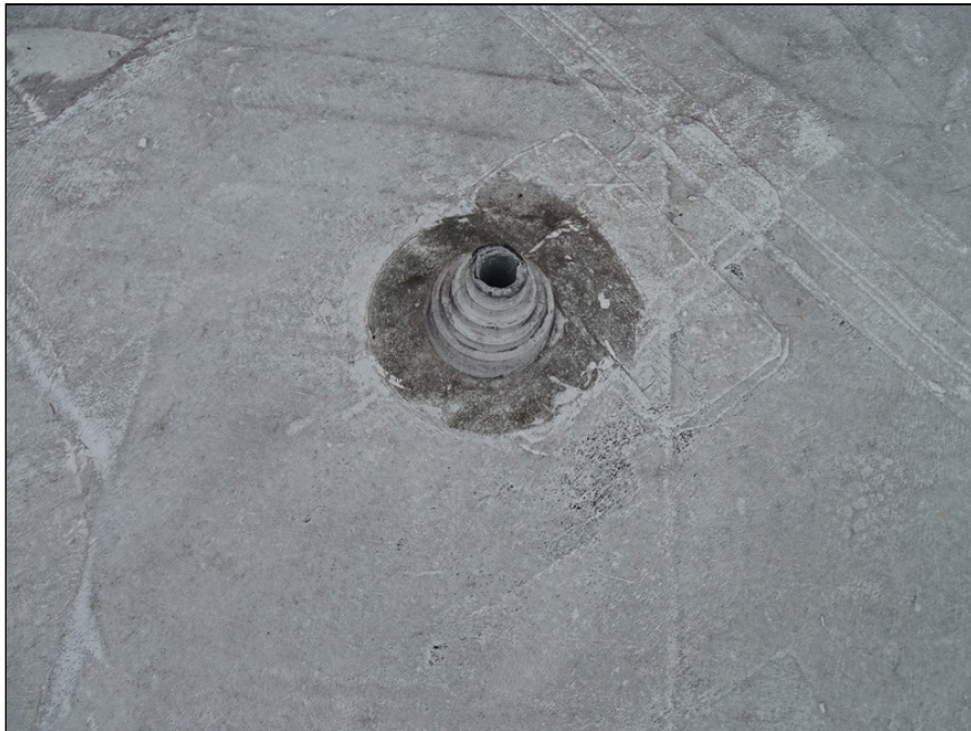
42 - Typical mechanical vent
