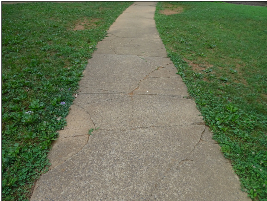
10 - Typical concrete sidewalk - note cracking
