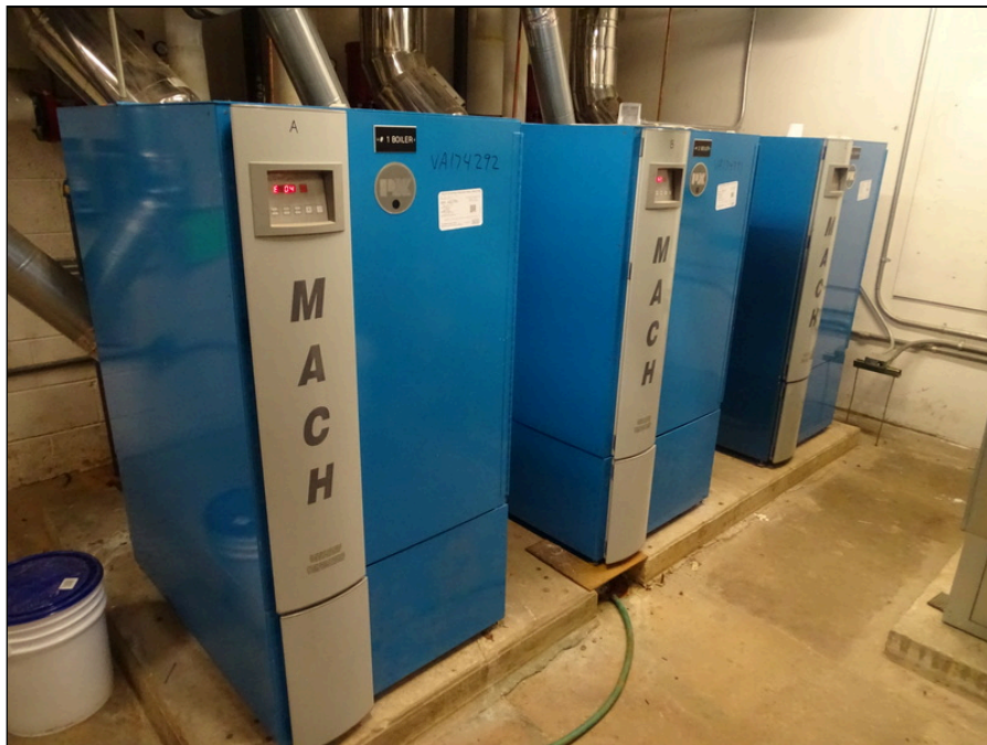
48 - Boilers located in mechanical room
