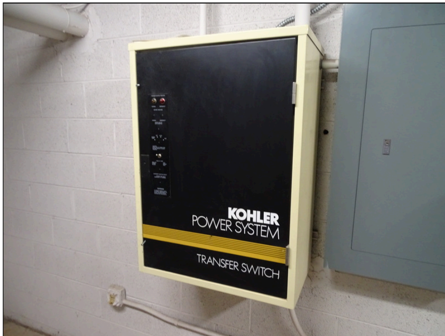
64 - Emergency power transfer switch
