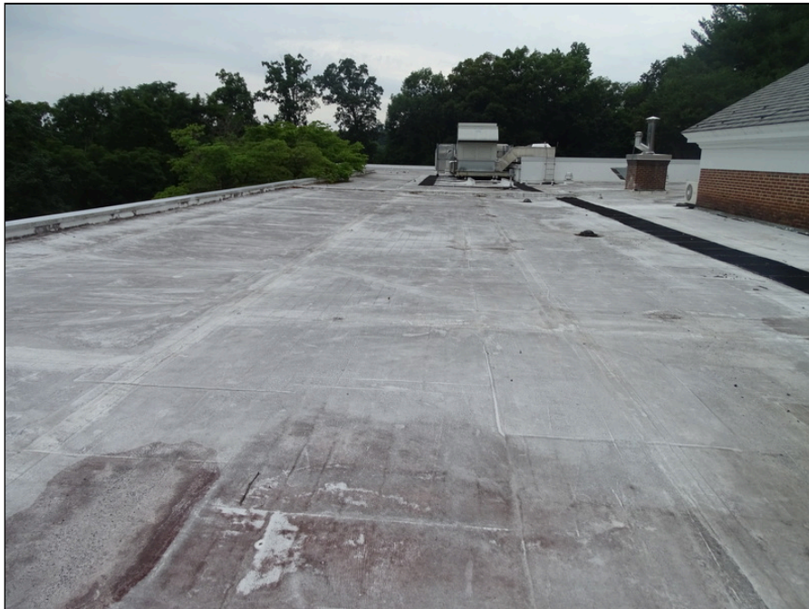
36 - Single-ply membrane roofing system looking west
