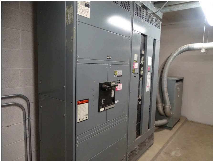
62 - Main electrical switchgear
