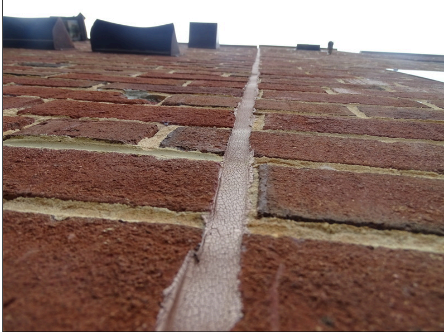
29 - Building exterior - note vertical sealant condition
