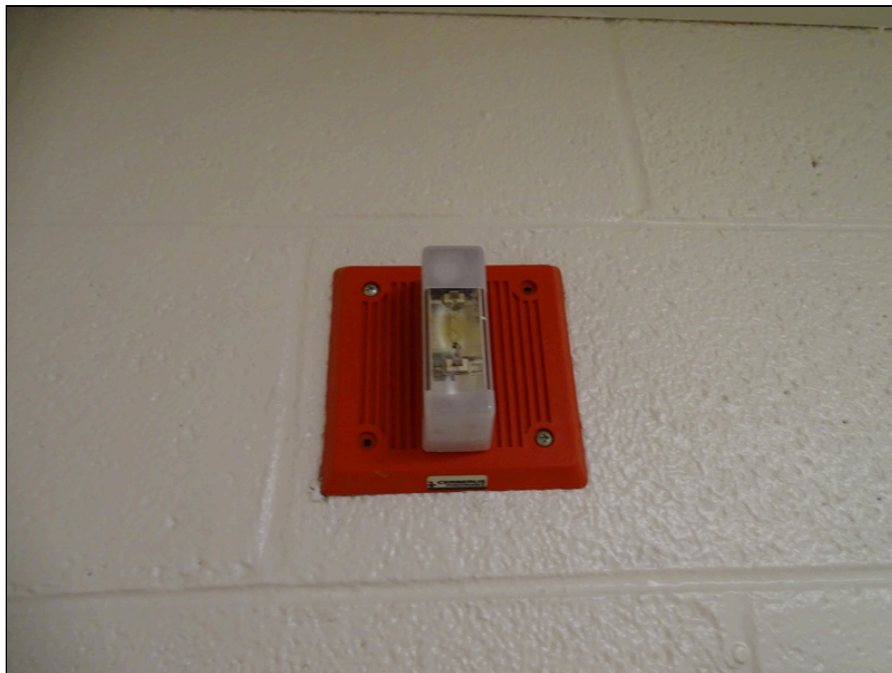
72 - Typical fire alarm bell and strobe
