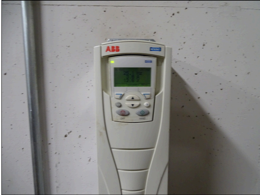
61 - Variable frequency drive for mechanical system
