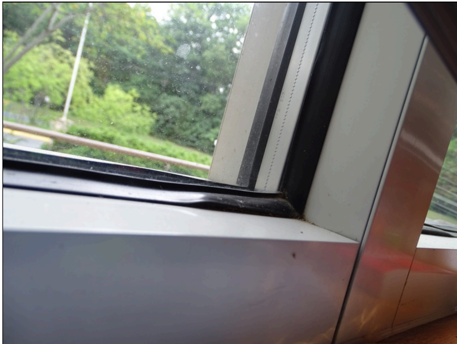
34 - Typical exterior windows - note separation of gasket
