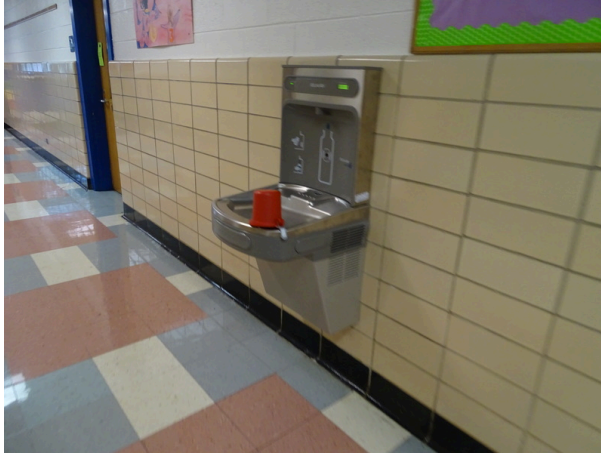
Water fountain - note protruding and not accessible
