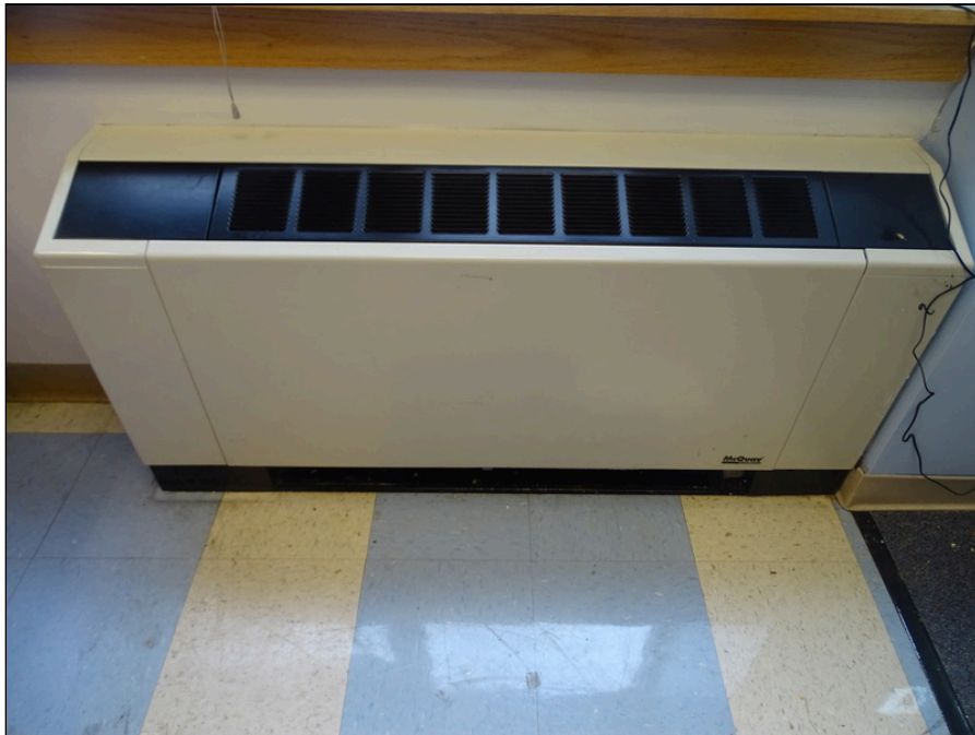
56 - Typical Water Source Heat Pump
