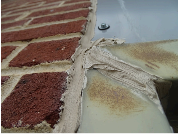
Building exterior - note sealant condition
