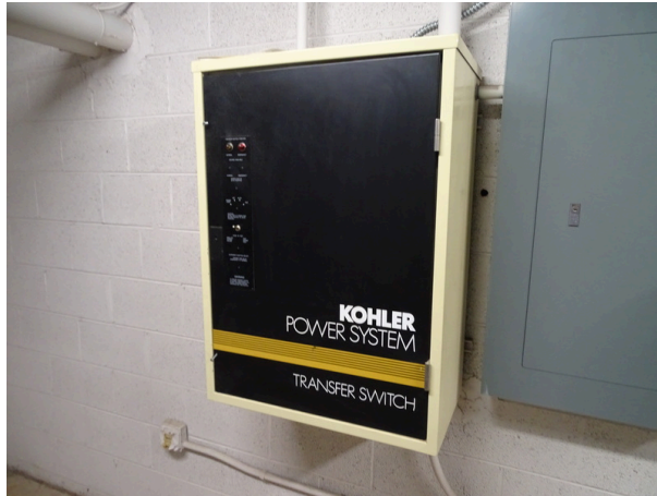
Emergency power transfer switch
