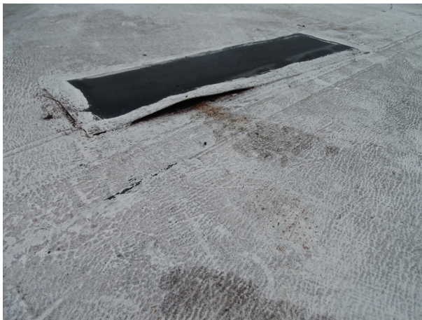
Single-ply membrane roofing system - note patching separation
