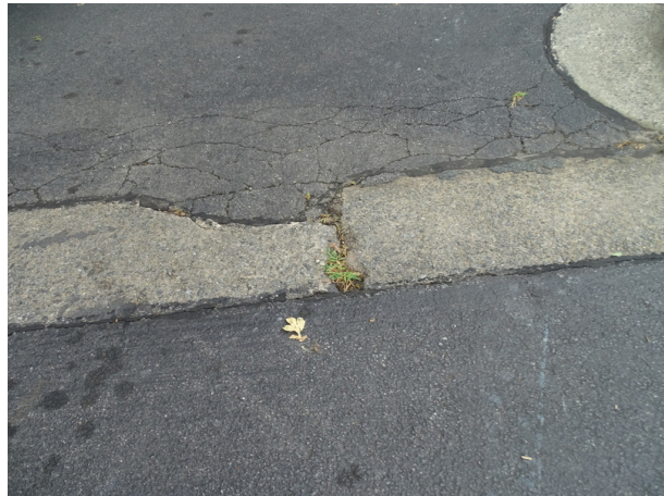
Asphalt apron - alligator cracking
