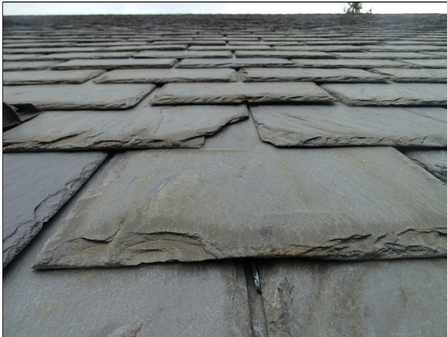
46 - Slate shingle roofing system - note misalignment of slate
