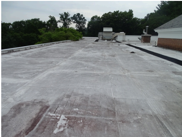
Single-ply membrane roofing system looking west
