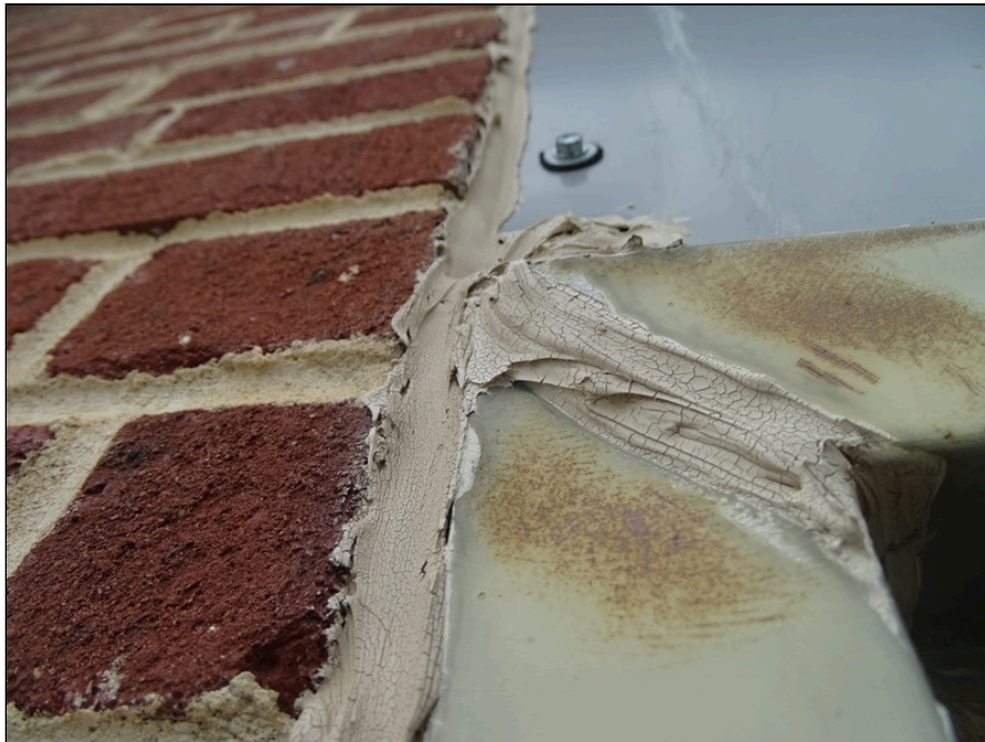
26 - Building exterior - note sealant condition
