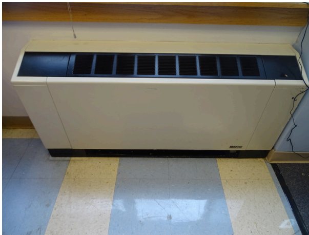
Typical Water Source Heat Pump
