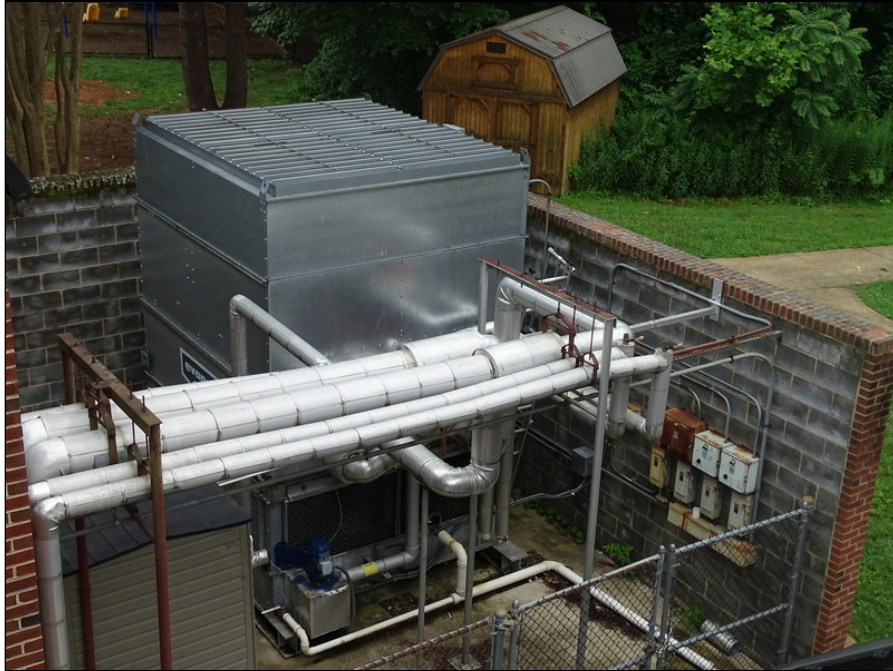
49 - Cooling Tower located at north side of the building
