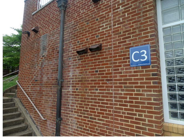
Building exterior - note efflorescence
