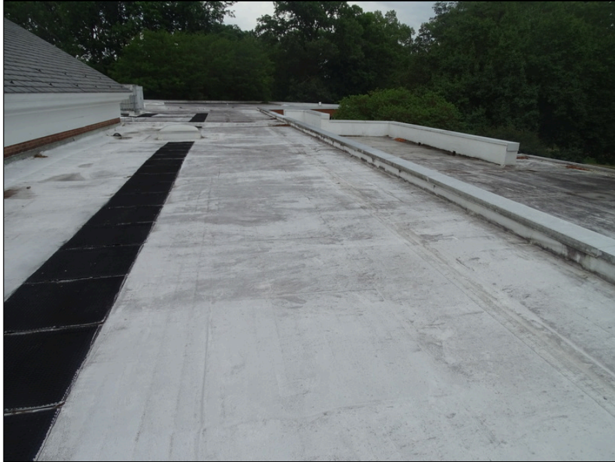
39 - Single-ply membrane roofing system looking east
