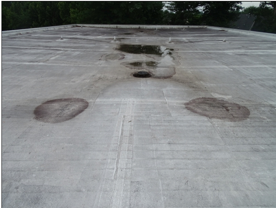
38 - Single-ply membrane roofing system - note ponding
