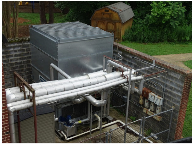
Cooling Tower located at north side of the building
