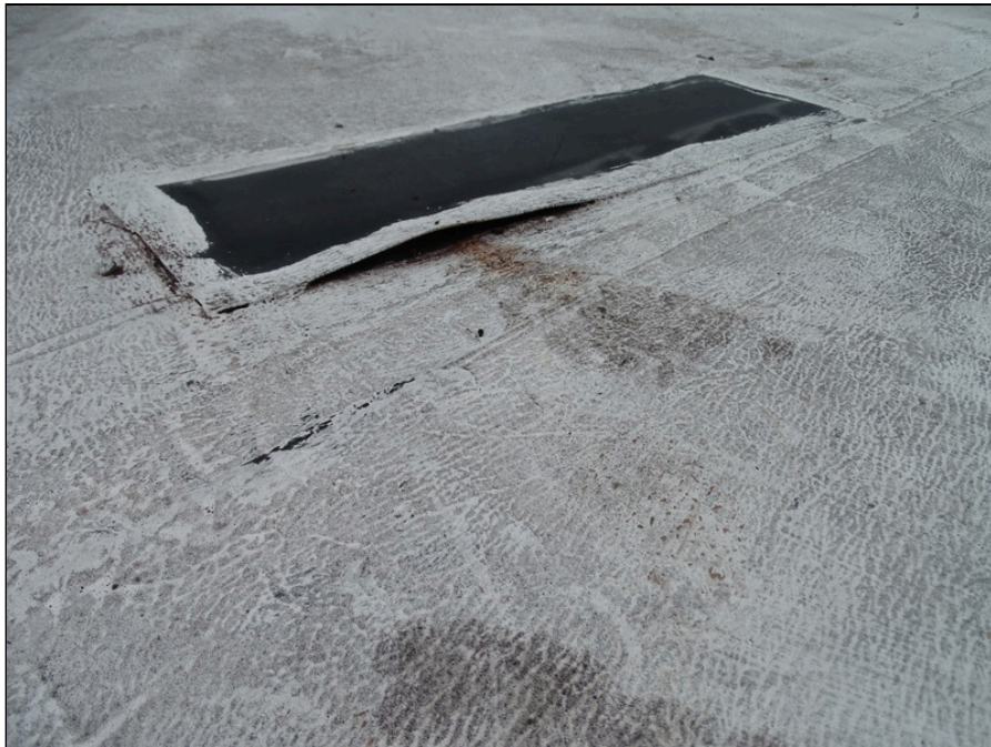
40 - Single-ply membrane roofing system - note patching separation
