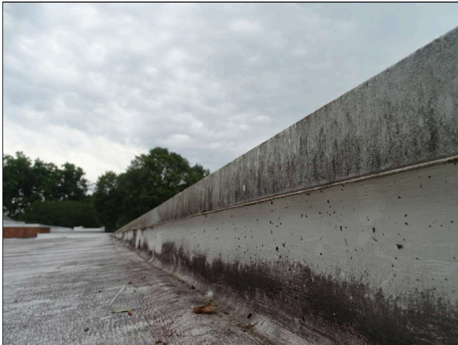
44 - Parapet wall - note deterioration
