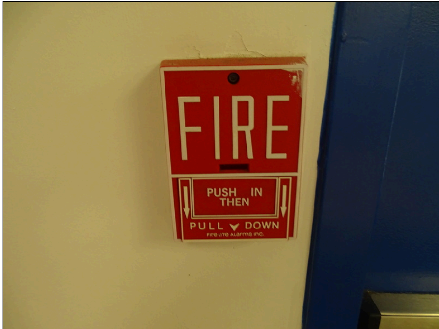
73 - Fire alarm pull station
