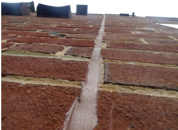
Building exterior - note vertical sealant condition
