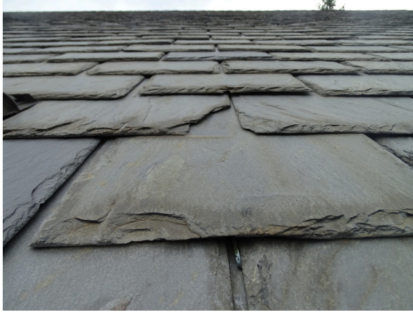
Slate shingle roofing system - note misalignment of slate
