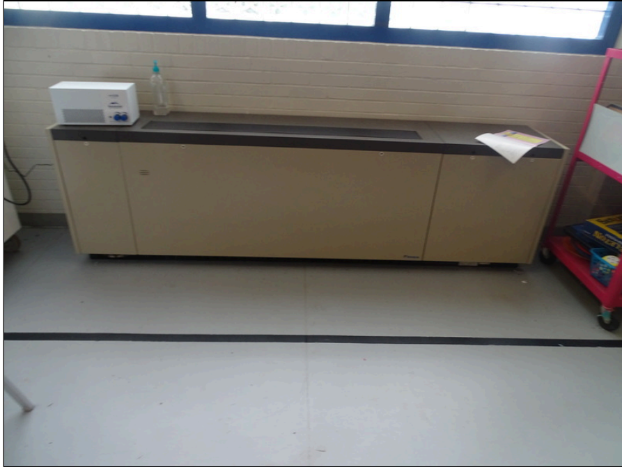
55 - Typical Water Source Heat Pump
