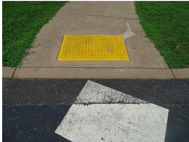
Accessible curb cut ramp with truncated domes
