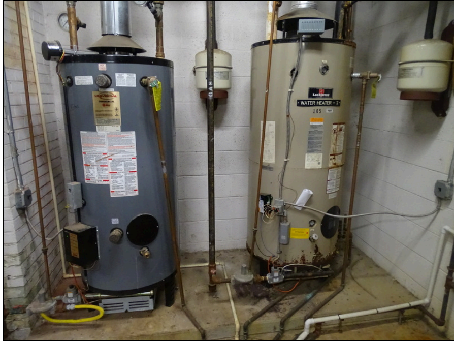
47 - Gas domestic water heaters
