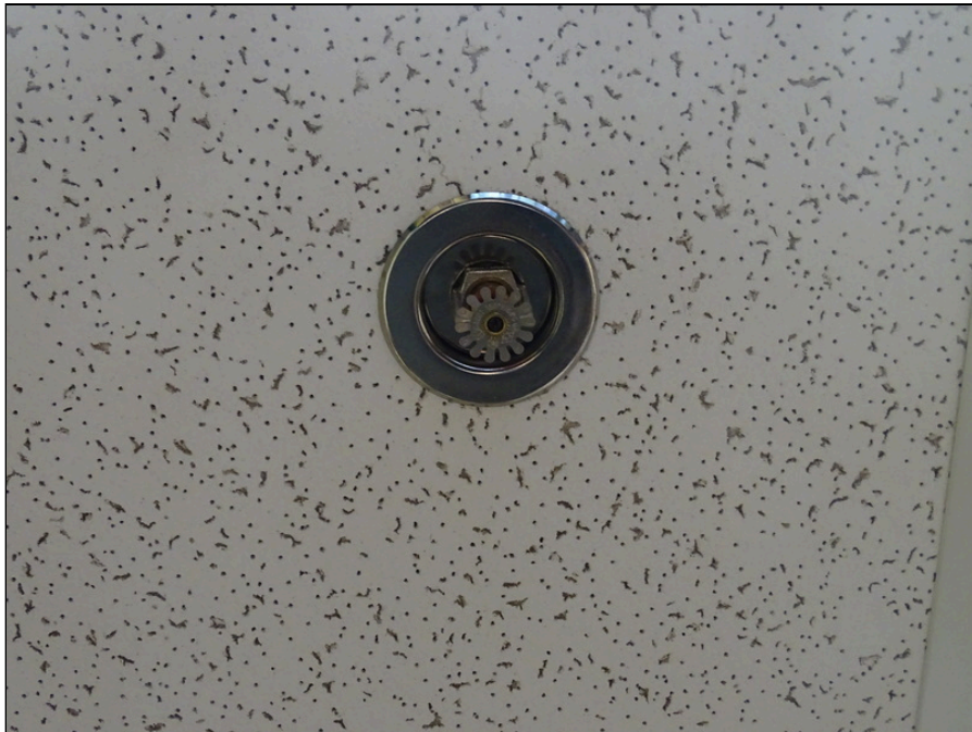
68 - Typical fire sprinkler head
