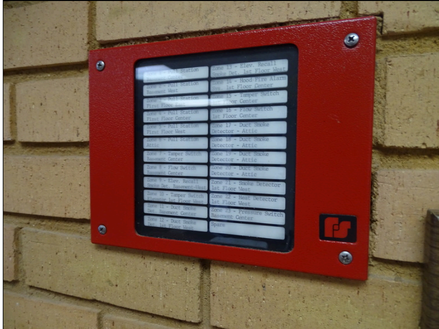
71 - Fire alarm panel - note older panel
