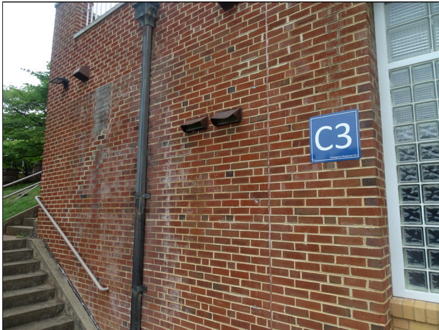
28 - Building exterior - note efflorescence
