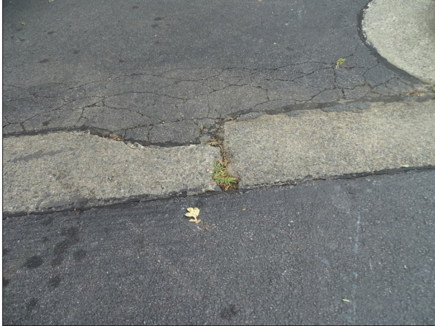
5 - Asphalt apron - alligator cracking
