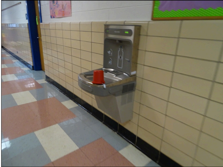
91 - Water fountain - note protruding and not accessible
