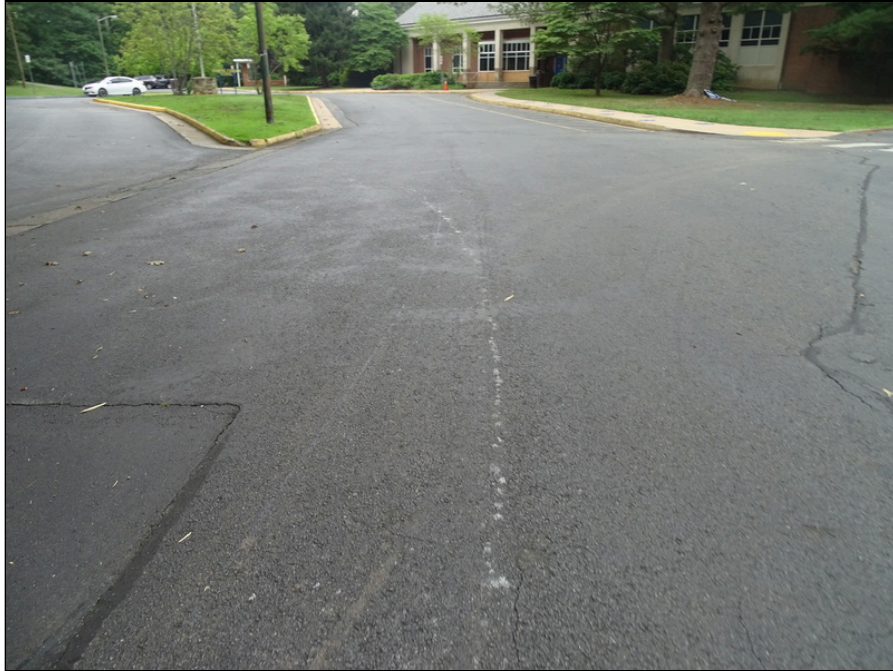
3 - Asphalt drive lane - note cracks and previous repair
