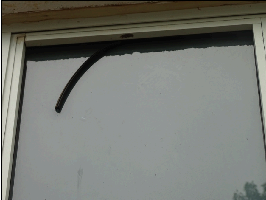
35 - Typical exterior windows - note separation of gasket
