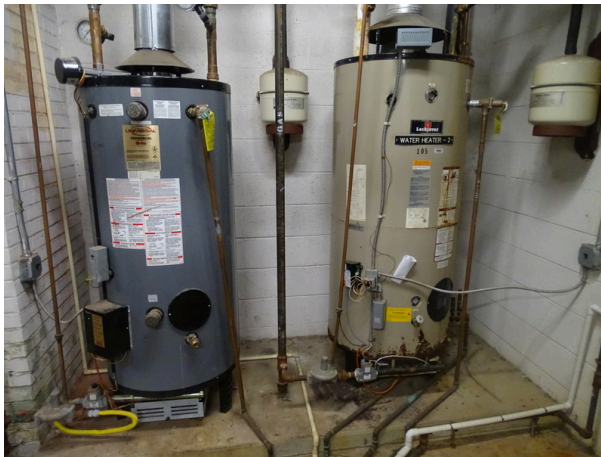
Gas domestic water heaters
