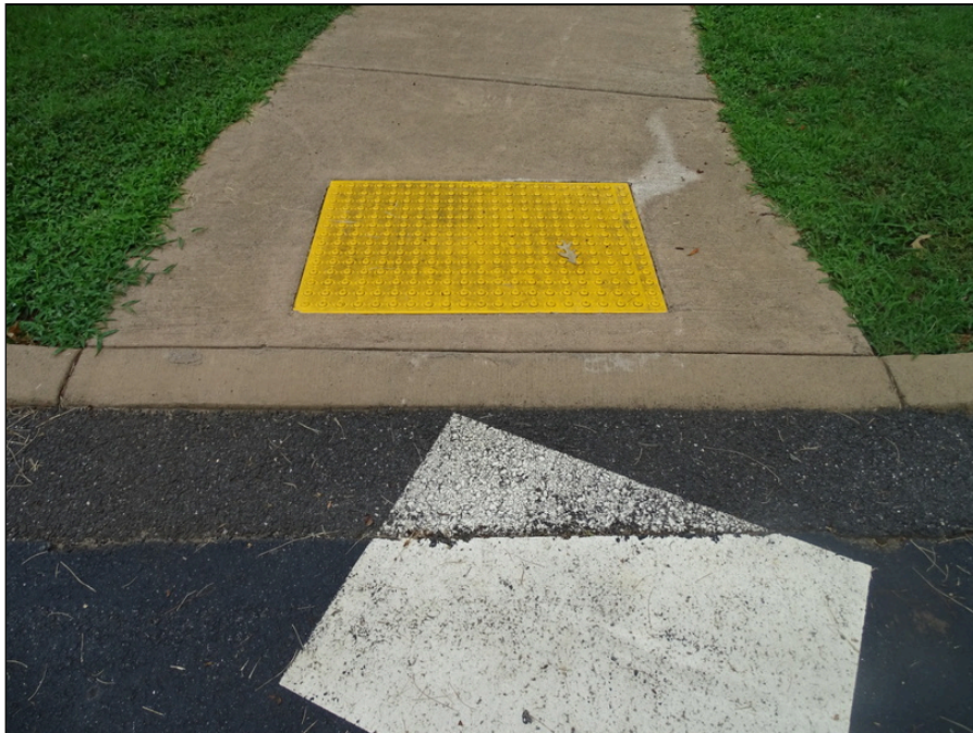
88 - Accessible curb cut ramp with truncated domes
