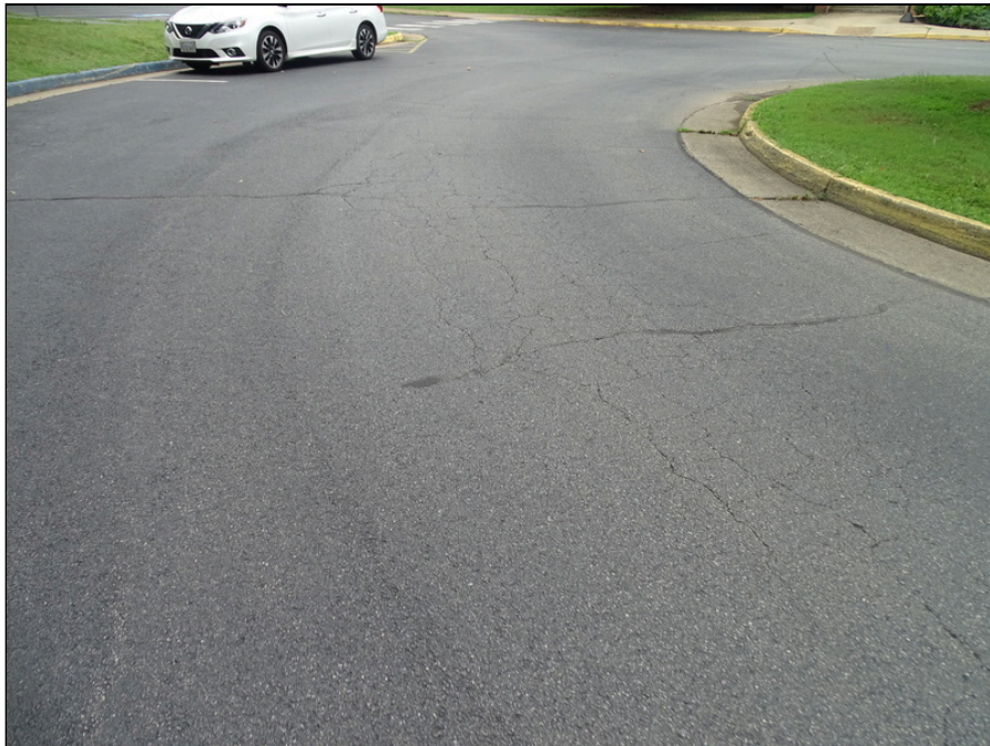
4 - Asphalt drive lane - note cracking
