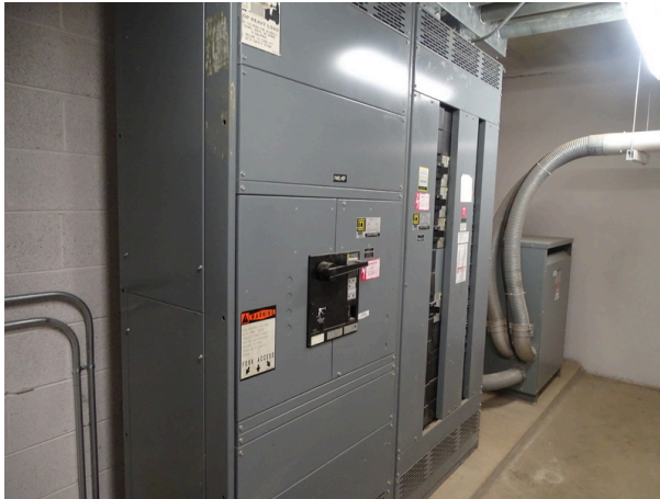
Main electrical switchgear
