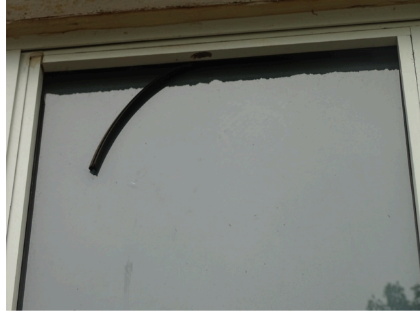
Typical exterior windows - note separation of gasket
