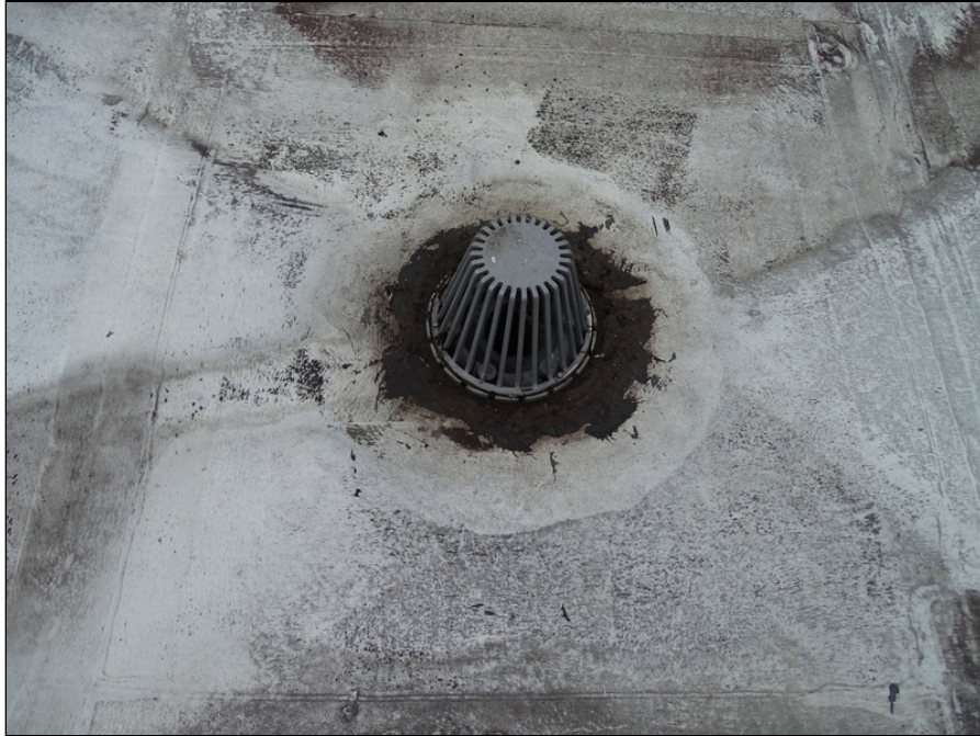
41 - Typical internal drain
