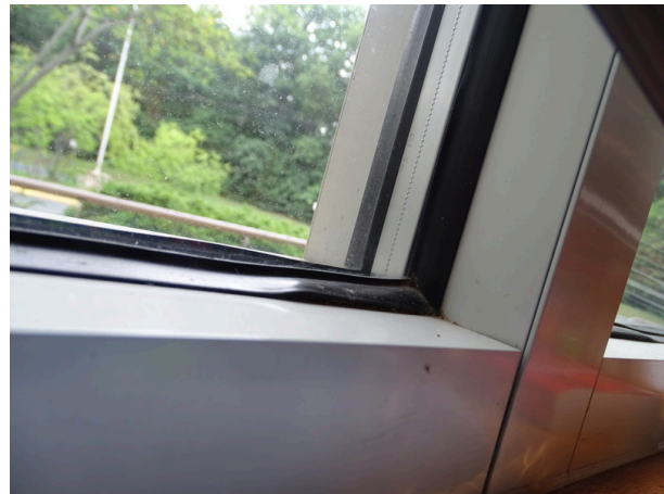
Typical exterior windows - note separation of gasket
