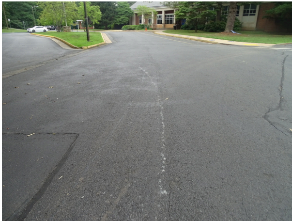
Asphalt drive lane - note cracks and previous repair
