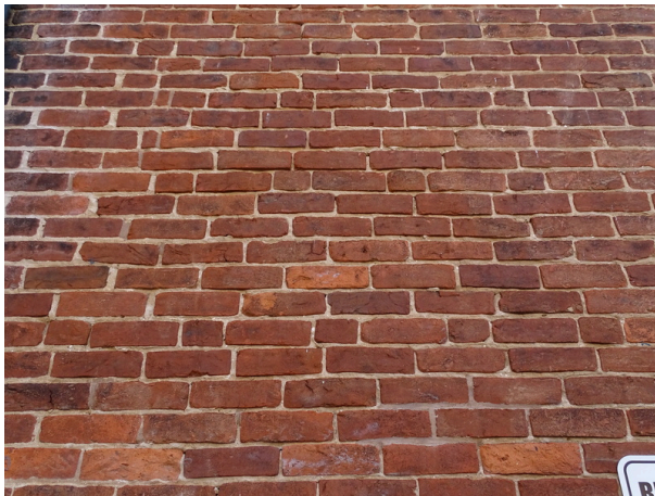
Building exterior wall - note mortar joint deterioration
