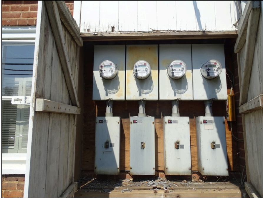
57 - Typical electric service panels and meters
