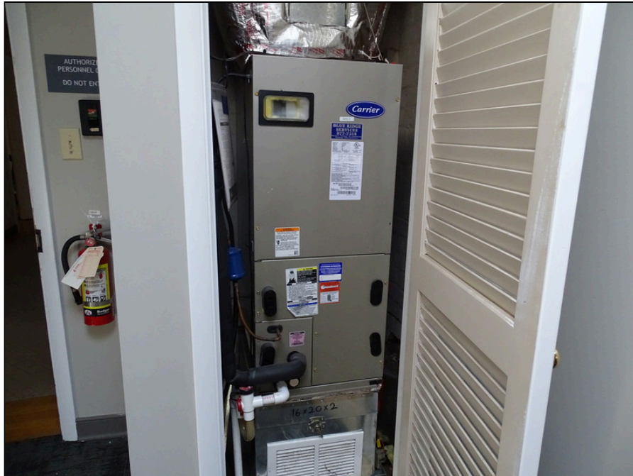
51 - Typical air handler located in second floor closet
