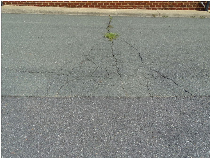
4 - Asphalt pavement- note alligator cracks
