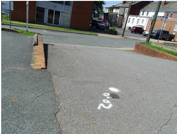
Site access from E Jefferson Street - note asphalt and brick wall deterioration
