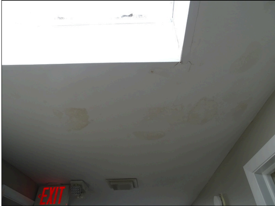
47 - Water leakage at ceiling of first floor corridor
