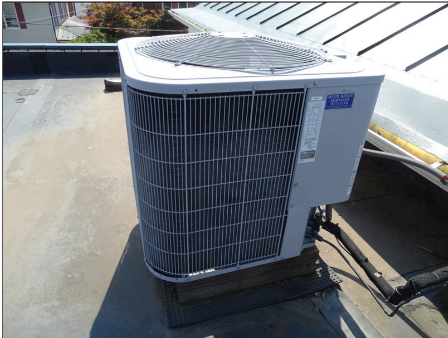
54 - Typical condensing unit
