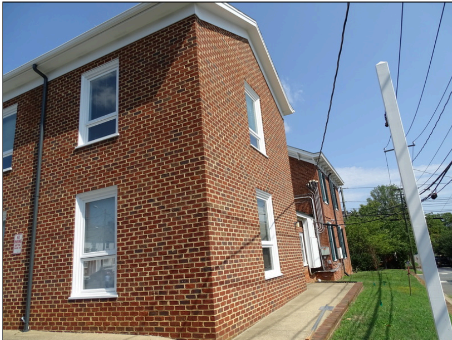
26 - Gutter and downspouts
