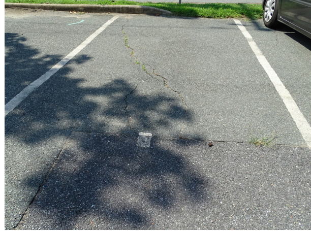
Asphalt parking- note alligator cracks
