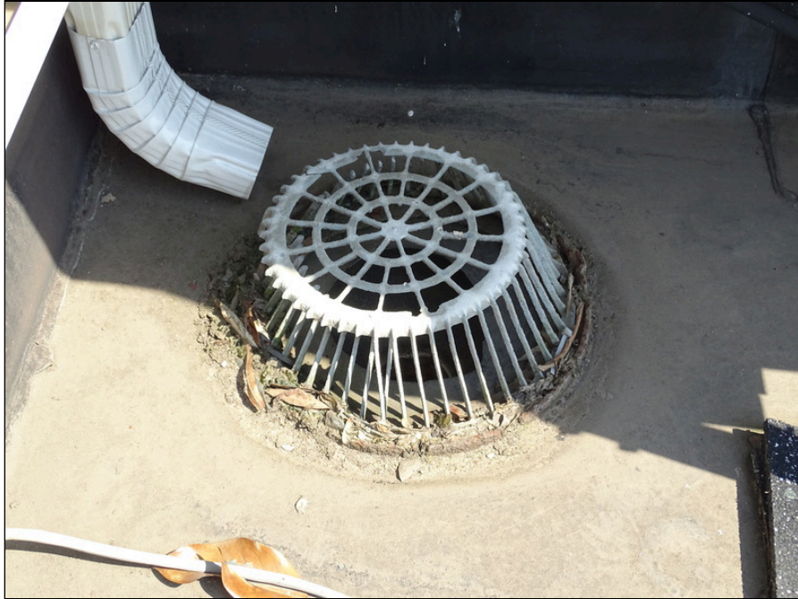
43 - Typical downspouts and internal drain overview - note need maintenance
