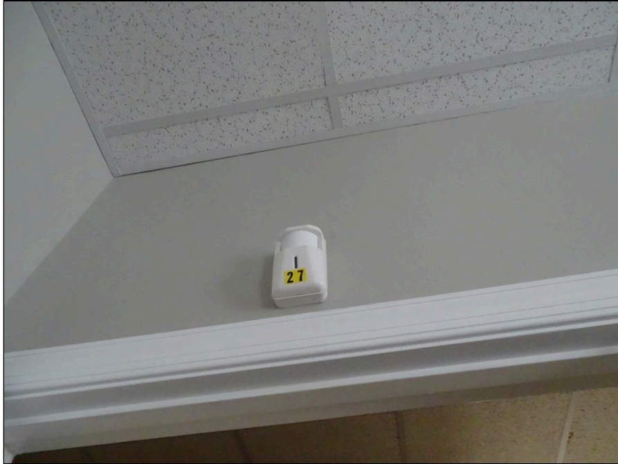
63 - Typical motion sensor
