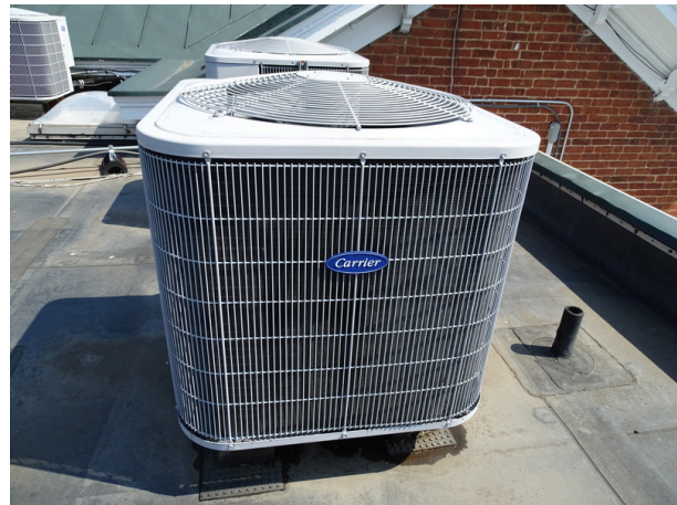
Typical condensing unit
