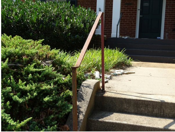
Exterior concrete stair handrail - note not with standard height
