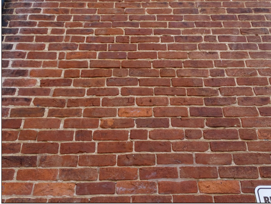
23 - Building exterior wall - note mortar joint deterioration
