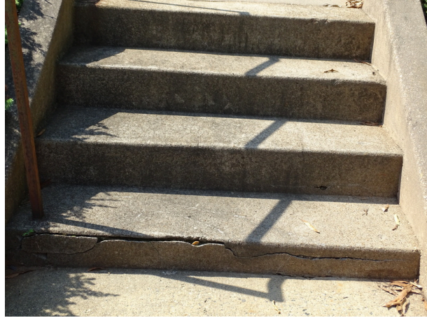
Exterior concrete stair - note deterioration
