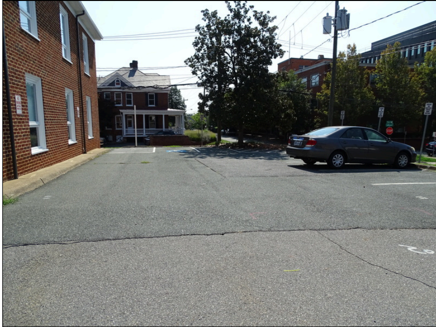
5 - Asphalt pavements - note cracks
