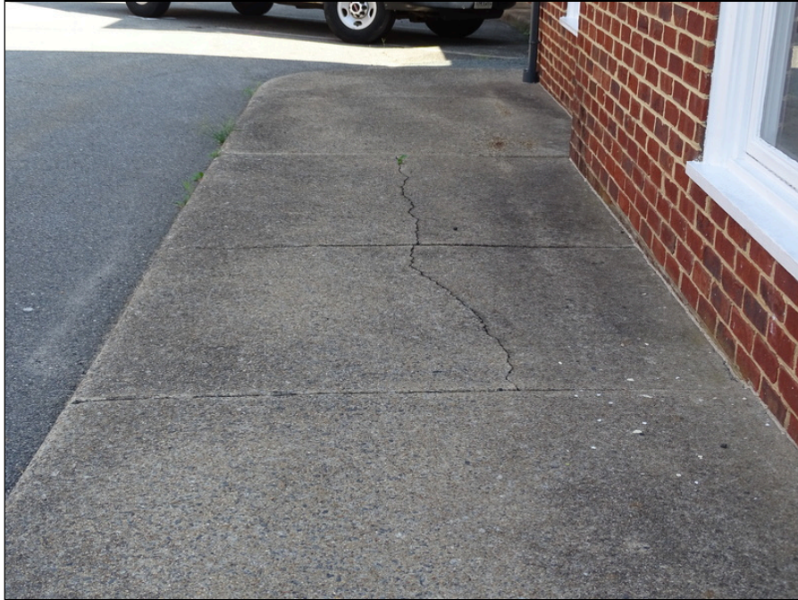
7 - Sidewalks - note cracks in concrete
