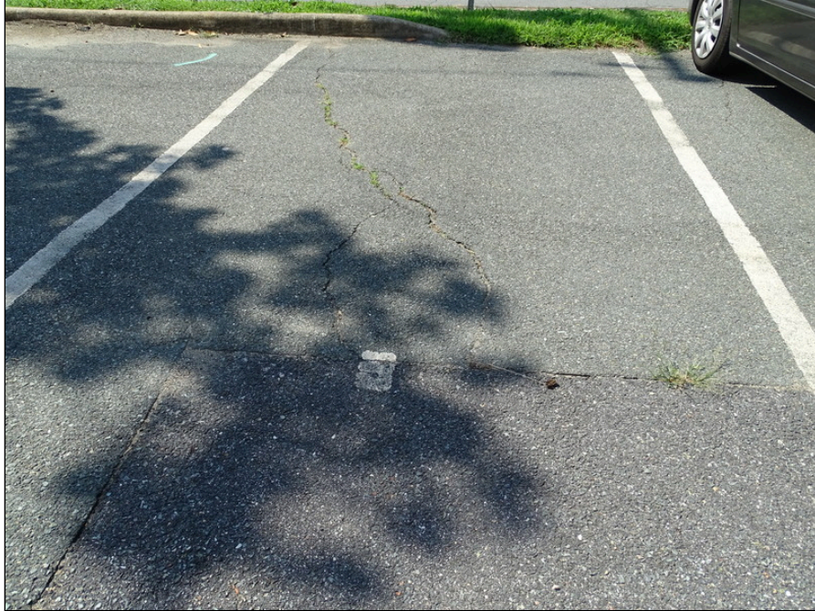
3 - Asphalt parking- note alligator cracks
