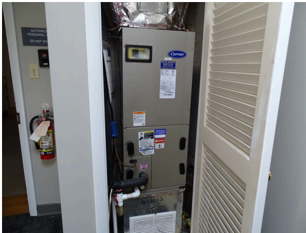
Typical air handler located in second floor closet
