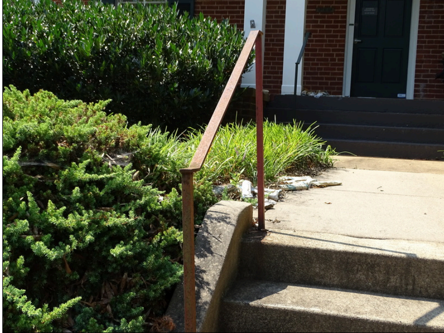
11 - Exterior concrete stair handrail - note not with standard height
