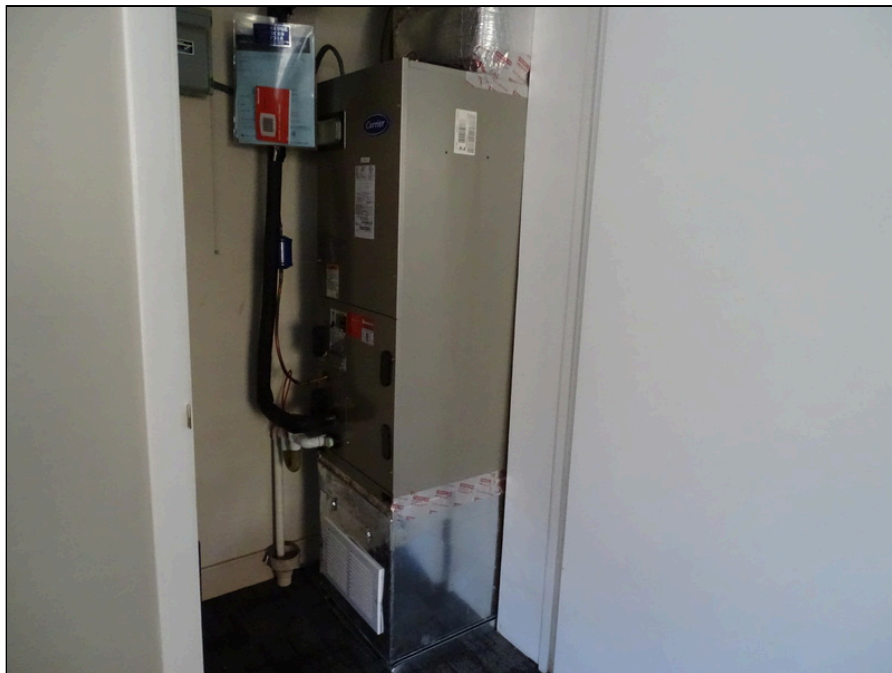
52 - Typical air handler located in second floor closet
