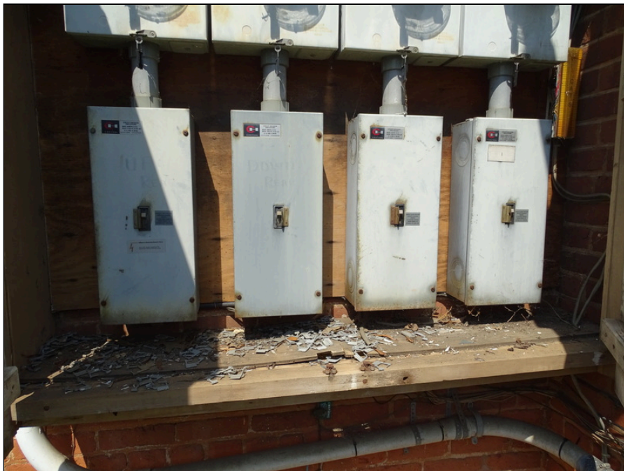
58 - Main electrical disconnects
