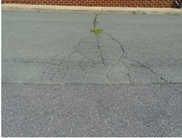
Asphalt pavement- note alligator cracks
