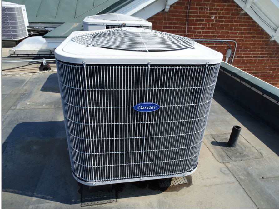
53 - Typical condensing unit
