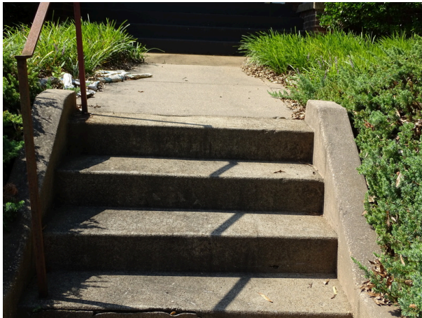
Exterior concrete stair - note installation of handrail in right side of stair
