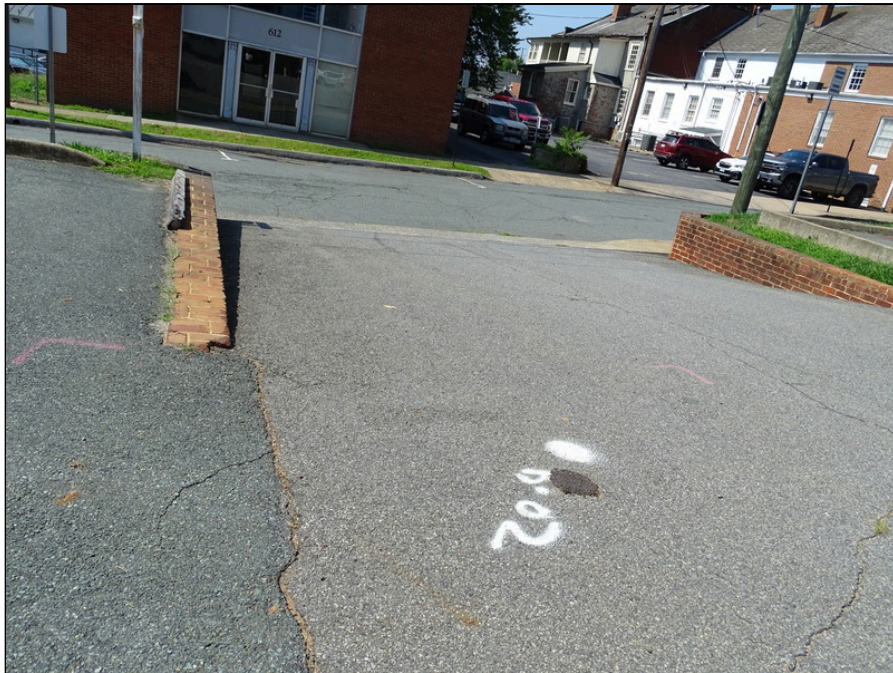
2 - Site access from E Jefferson Street - note asphalt and brick wall deterioration
