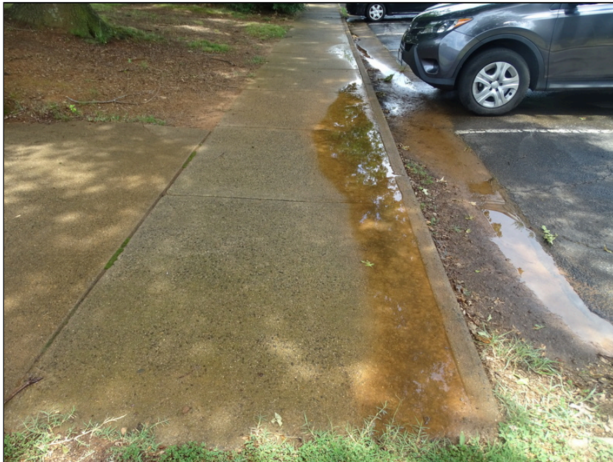
22 - Concrete sidewalk - note ponding
