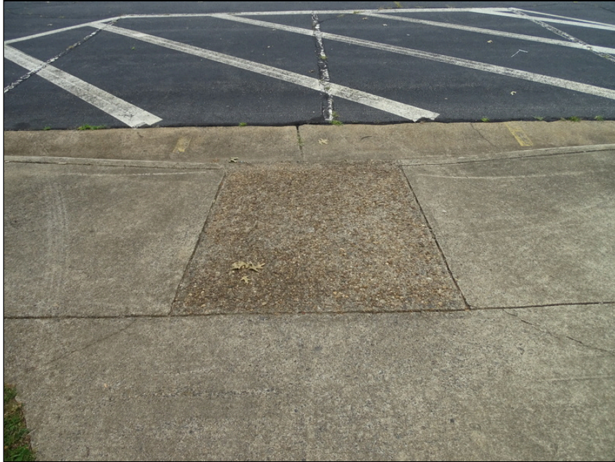
19 - Concrete ramp - note need to install truncated domes
