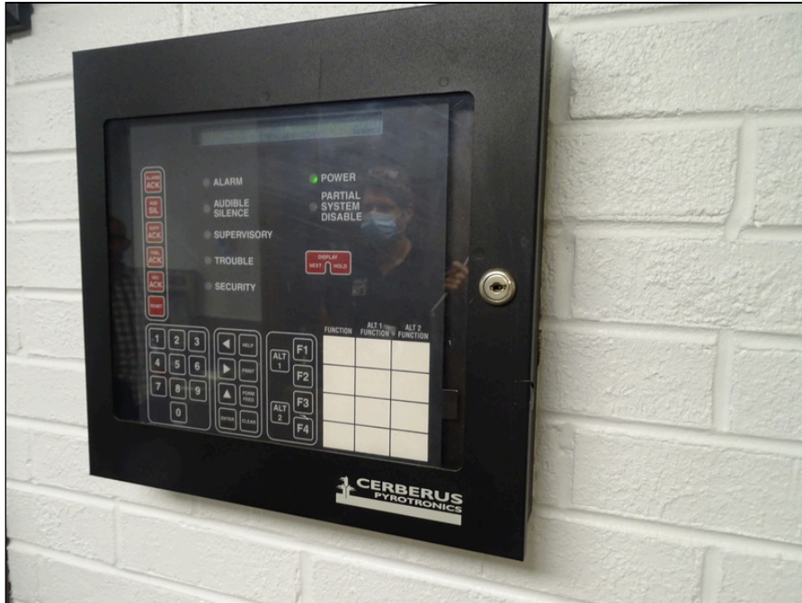
97 - Fire alarm annunciator panel
