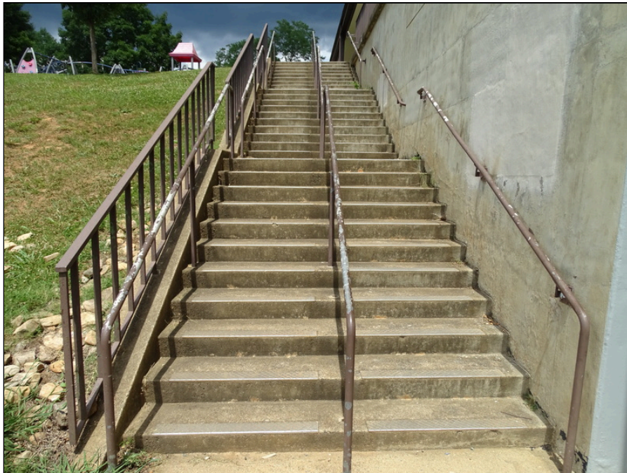
34 - Concrete stair handrail - note deterioration
