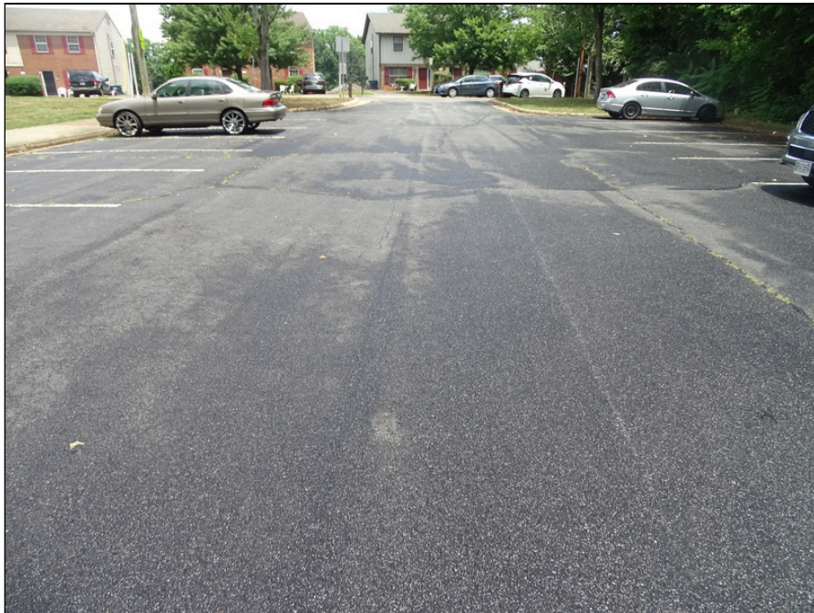
24 - Asphalt parking - note cracking
