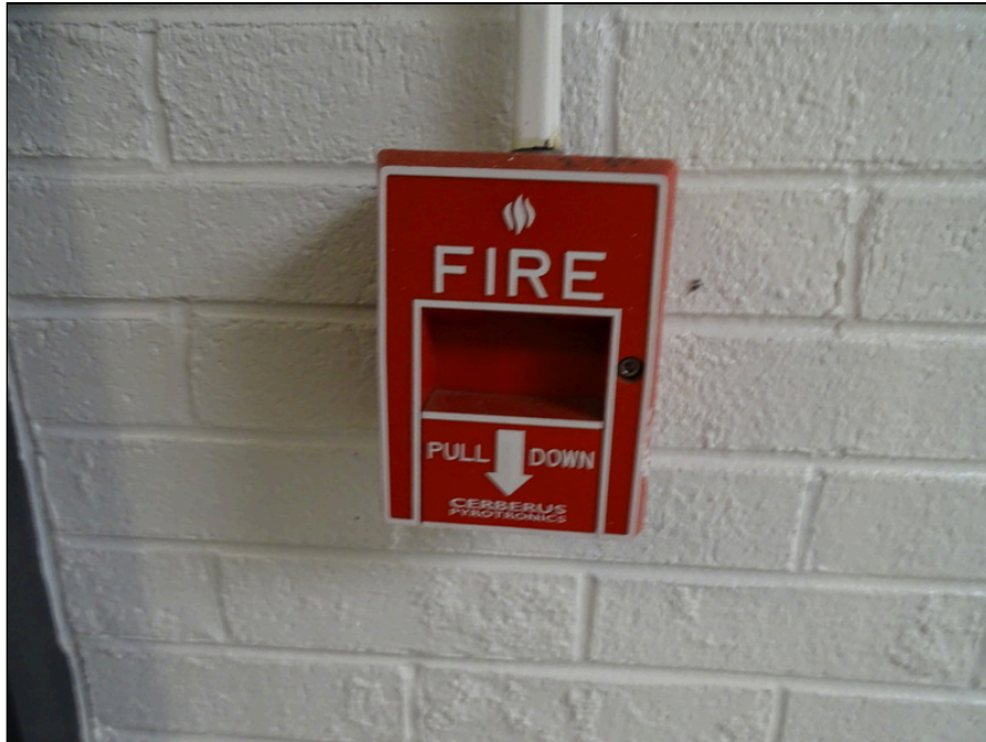
107 - Typical fire alarm pull station
