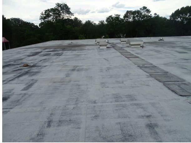
Single-ply membrane roofing system looking west
