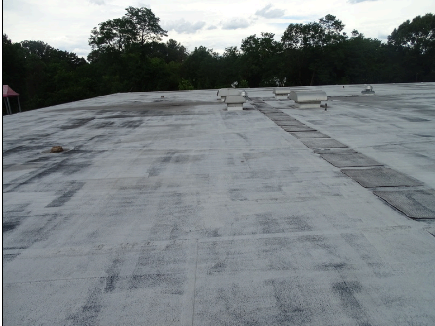
73 - Single-ply membrane roofing system looking west
