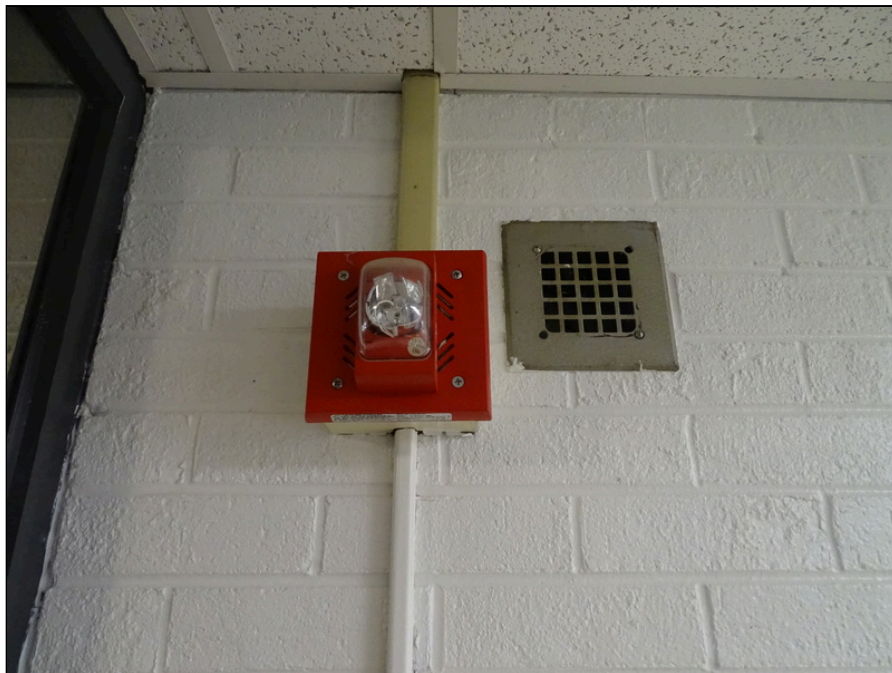
108 - Typical fire alarm bell and strobe
