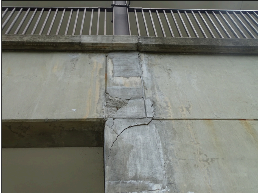
55 - Building exterior - note column cracking
