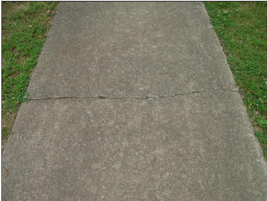
20 - Concrete sidewalk - note cracking
