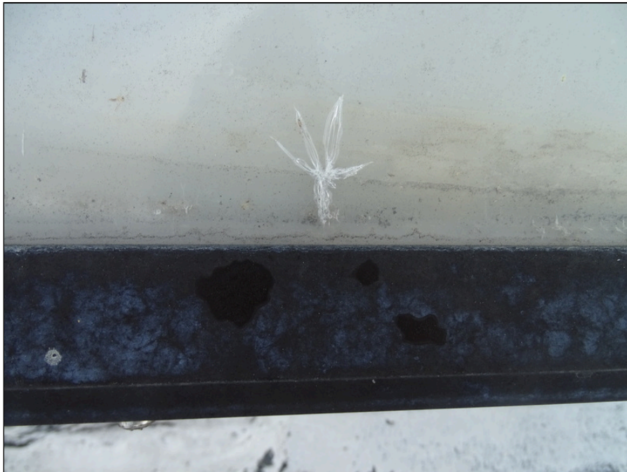
78 - Skylights located on north side of the building - note glass cracked
