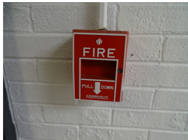
Typical fire alarm pull station
