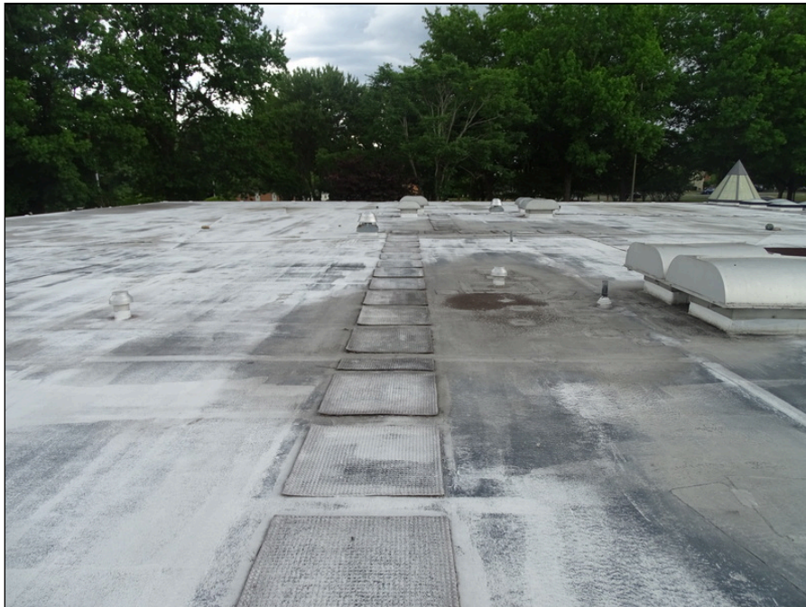
74 - Single-ply membrane roofing system looking west - note ponding
