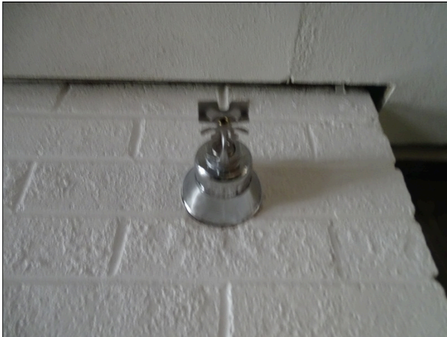
106 - Typical sprinkler head
