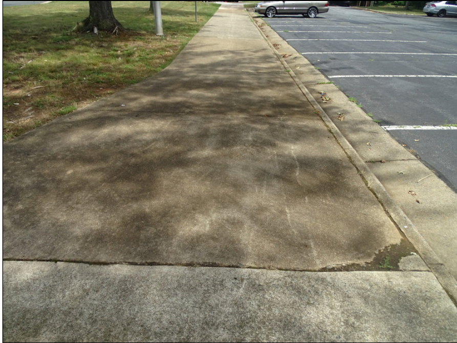
23 - Concrete sidewalk - note cracking
