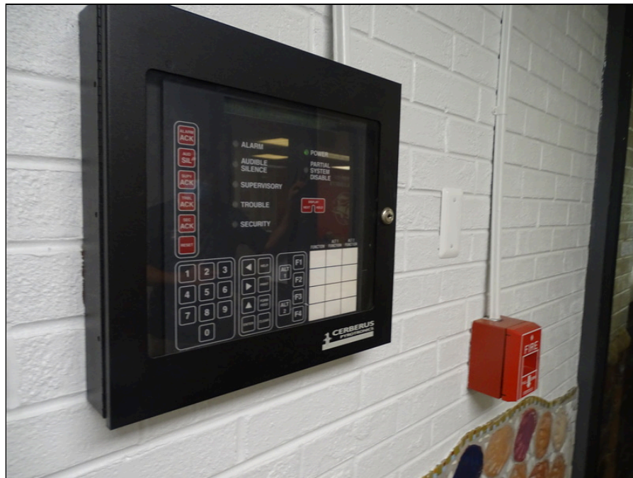
96 - Fire alarm annunciator panel
