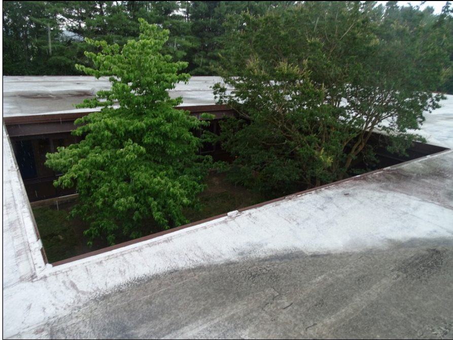
75 - Single-ply membrane roofing system
