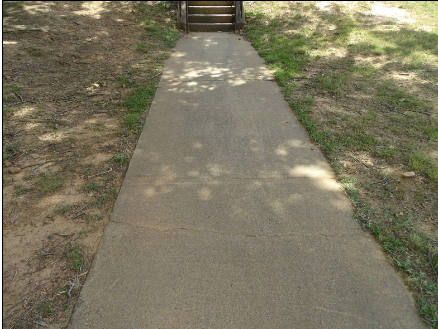
25 - Concrete sidewalk - note cracking
