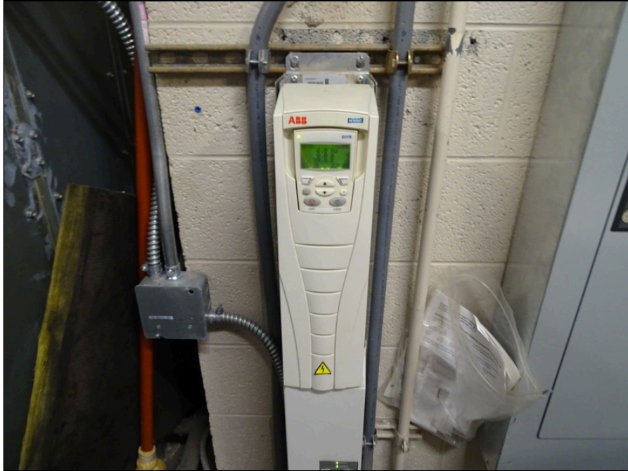
89 - Variable frequency drive mechanical controls
