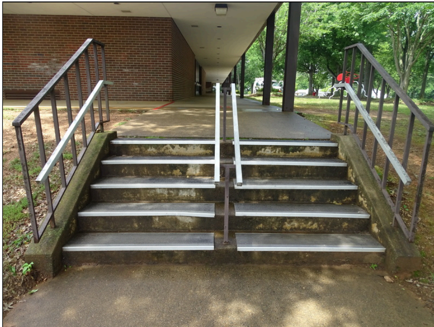
32 - Concrete stair - note stained
