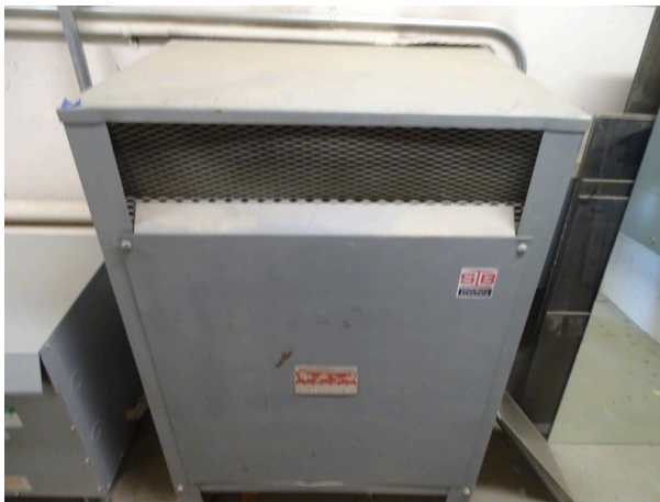
Typical building transformer
