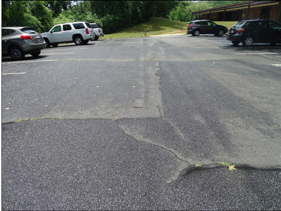
11 - Asphalt parking east side of site - note cracking
