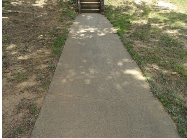
Concrete sidewalk - note cracking
