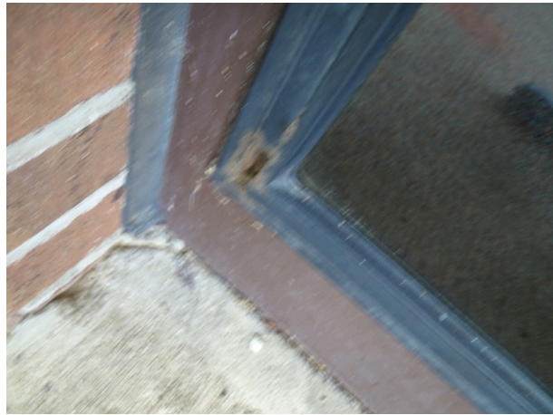
Typical exterior window - note deterioration of gasket
