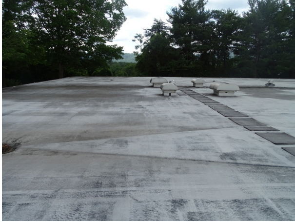
Single-ply membrane roofing system looking west
