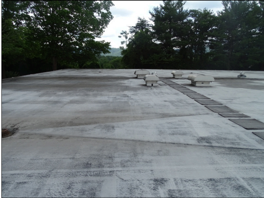
69 - Single-ply membrane roofing system looking west
