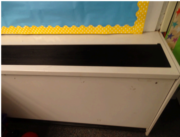
Typical fan coil unit
