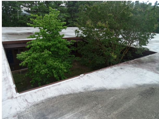
Single-ply membrane roofing system
