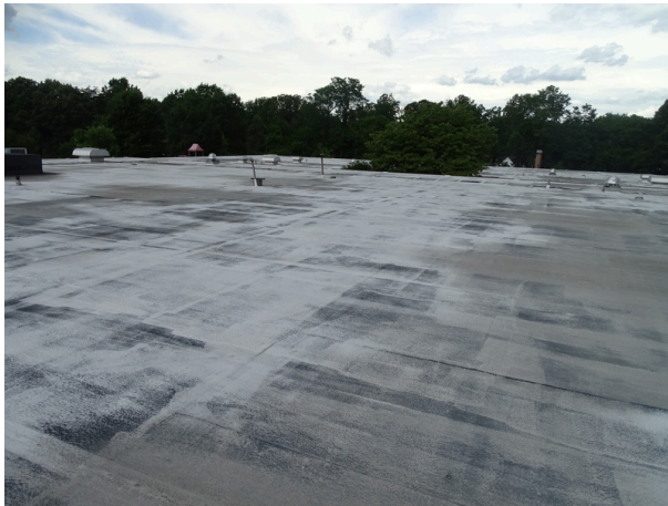
Single-ply membrane roofing system
