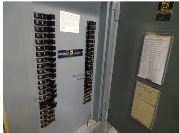
Typical electrical circuit breaker panel
