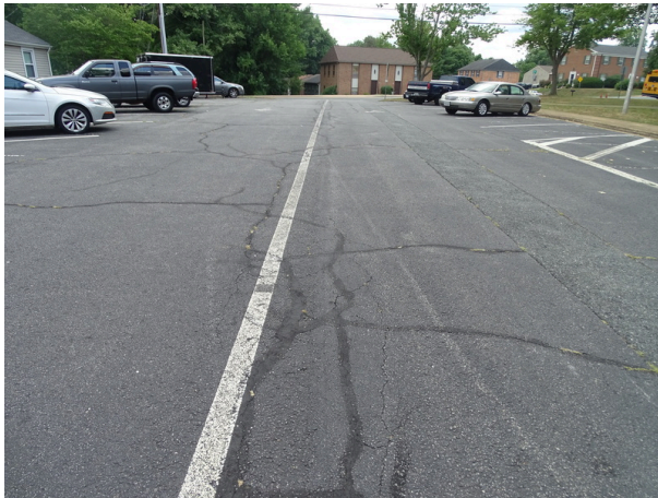
Asphalt drive lane east side of the site - note cracking and previous repair
