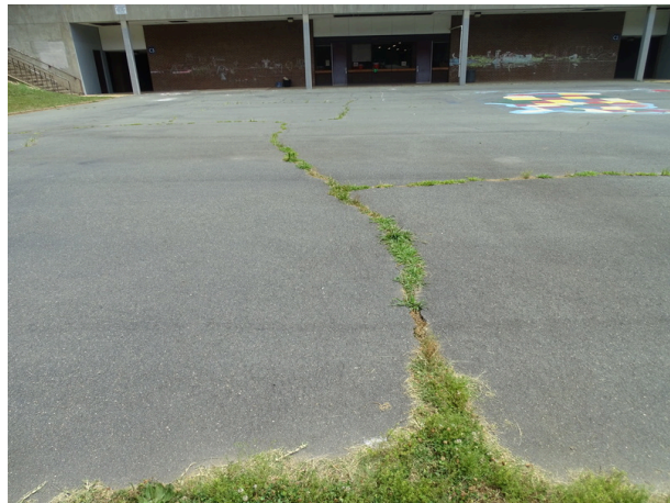
Asphalt playing surface - note cracking and grass growing
