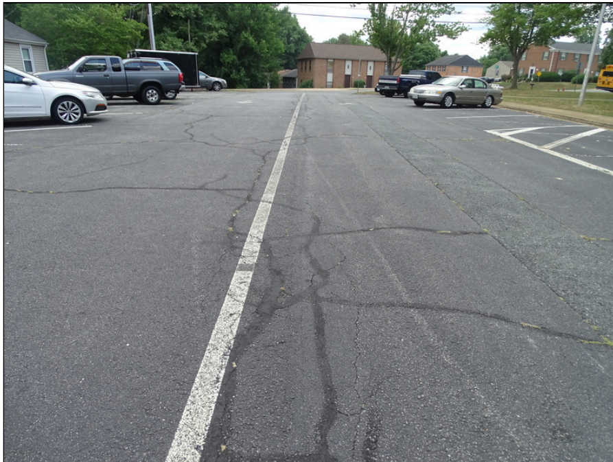
10 - Asphalt drive lane east side of the site - note cracking and previous repair
