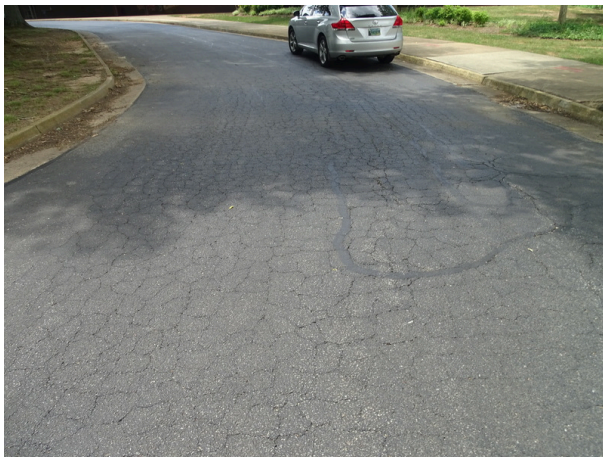
Asphalt drive lane entrance - note cracking
