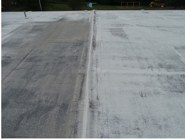
Single-ply membrane roofing system - note patching
