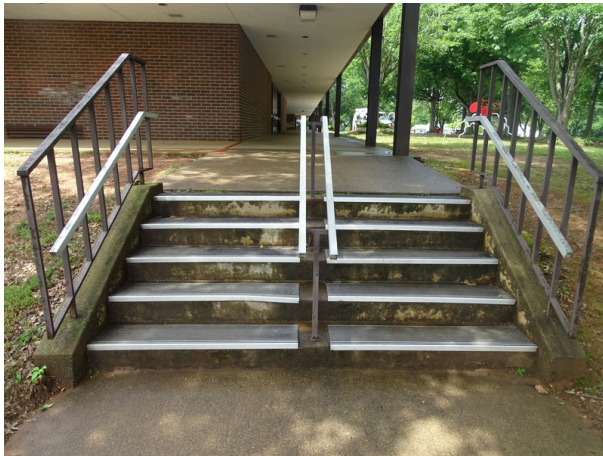
Concrete stair - note stained
