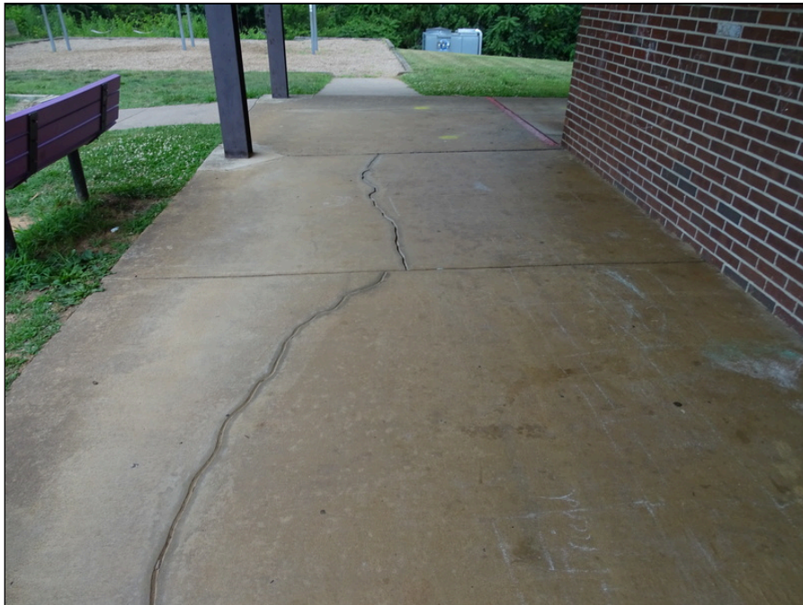
28 - Concrete sidewalk - note cracking
