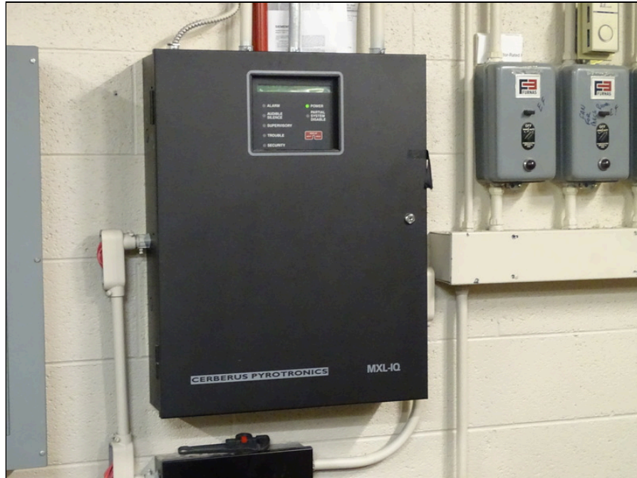
95 - Fire alarm control panel
