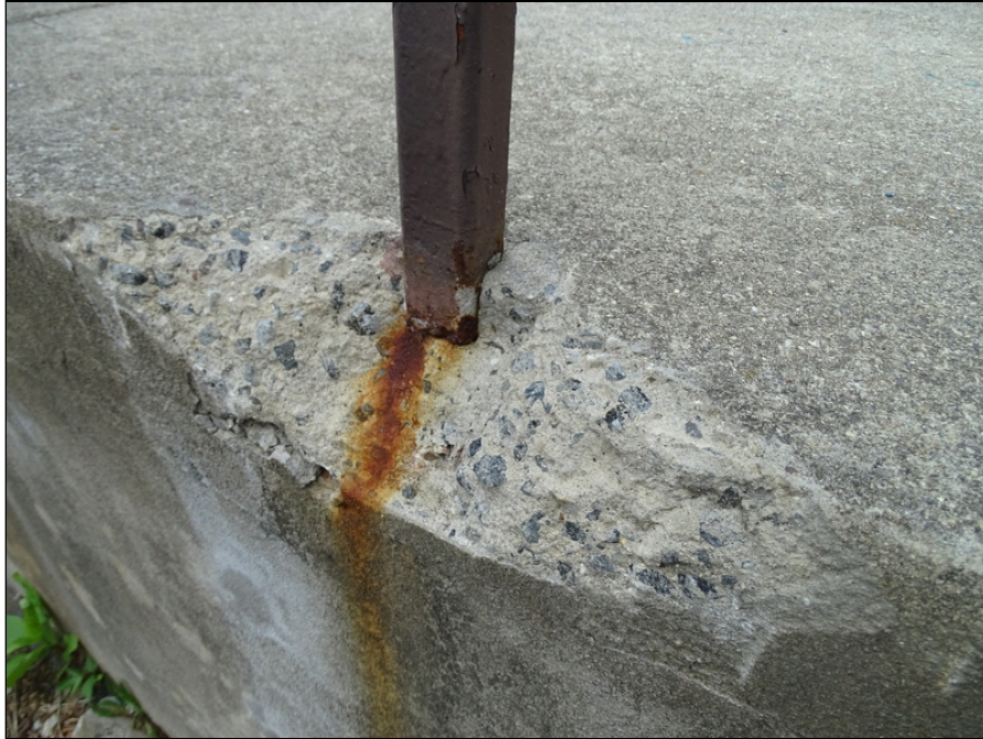
37 - Concrete ramp- note deterioration
