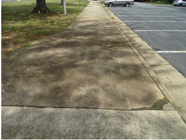
Concrete sidewalk - note cracking
