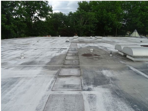
Single-ply membrane roofing system looking west - note ponding
