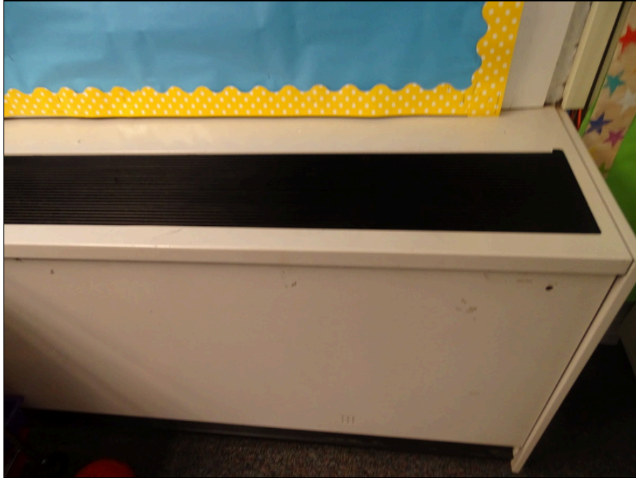
139 - Typical fan coil unit
