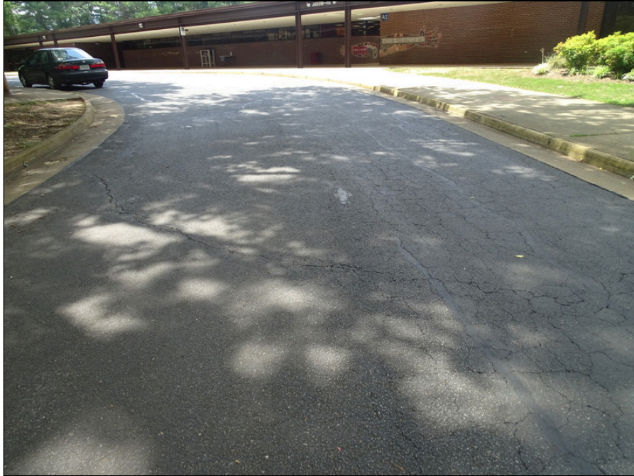
7 - Asphalt drive lane west side of the site - note alligator cracks
