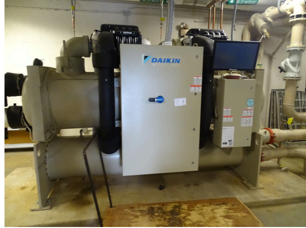
Chiller located in mechanical room
