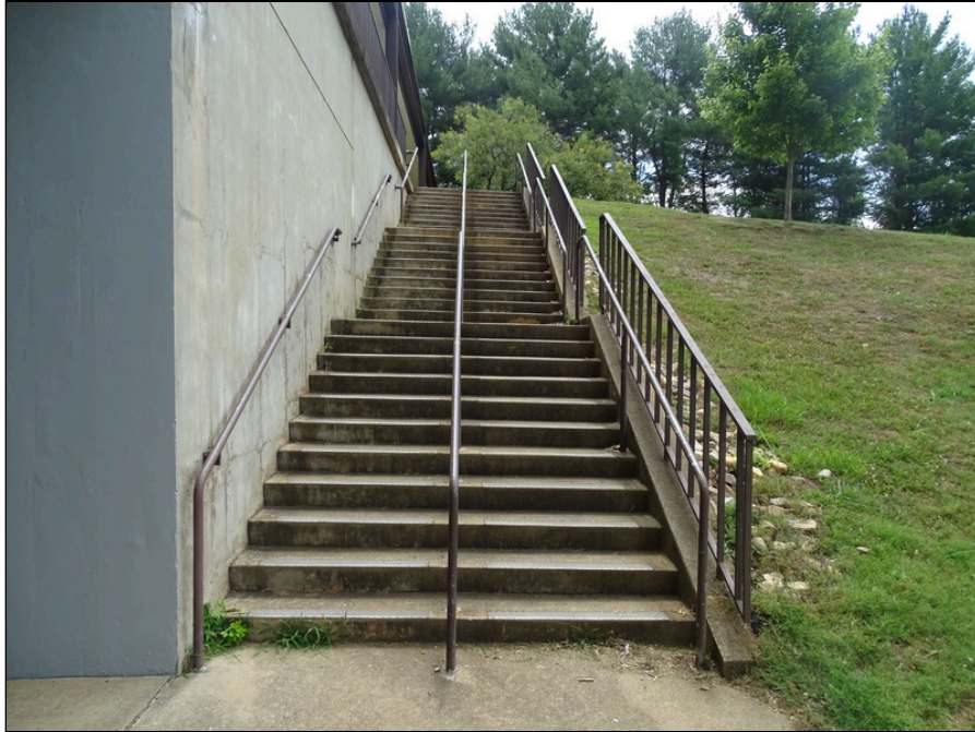
33 - Concrete stair - note stained and wall cracking
