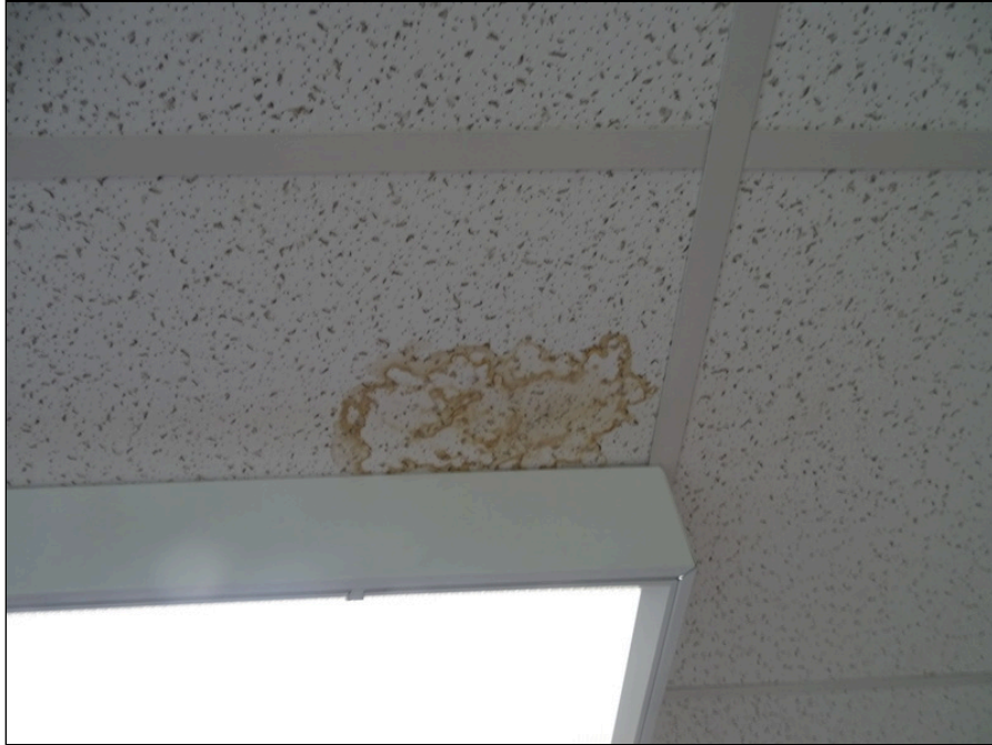
129 - Ceiling interior - water leakage
