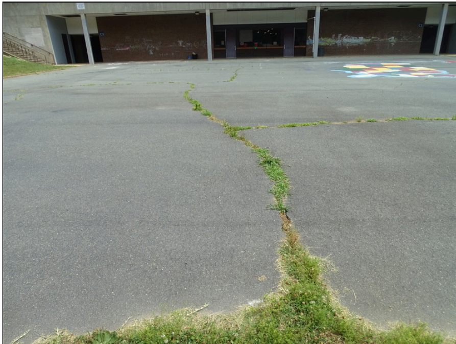
14 - Asphalt playing surface - note cracking and grass growing
