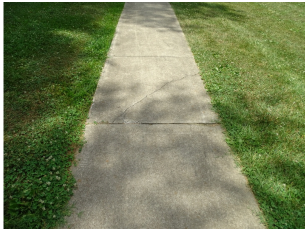
Concrete sidewalk - note cracking
