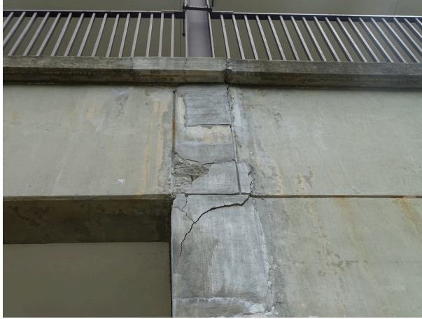
Building exterior - note column cracking
