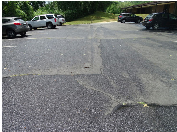
Asphalt parking east side of site - note cracking
