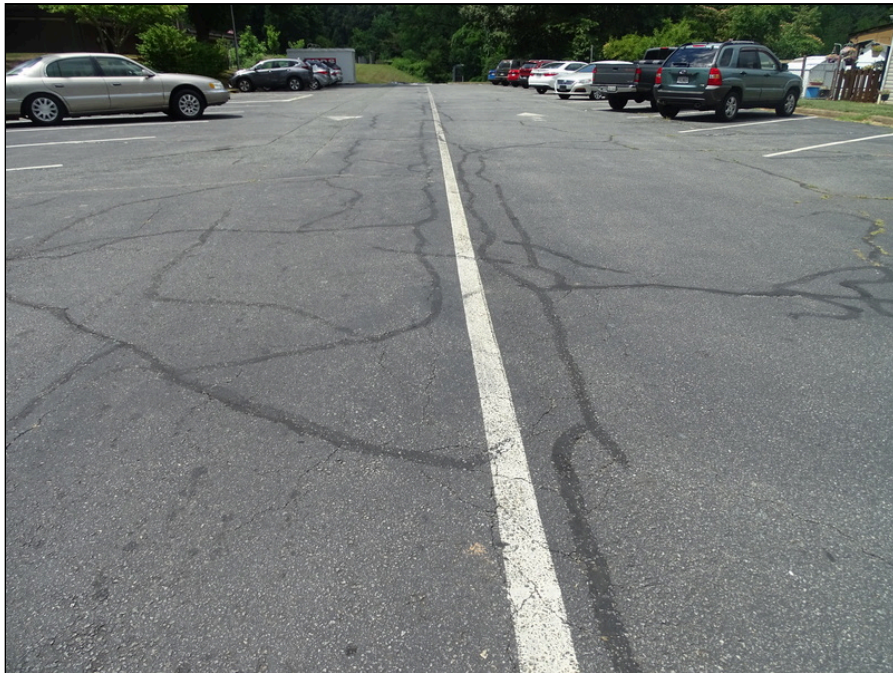
4 - Asphalt drive lane east side of the site - note cracking and previous repair
