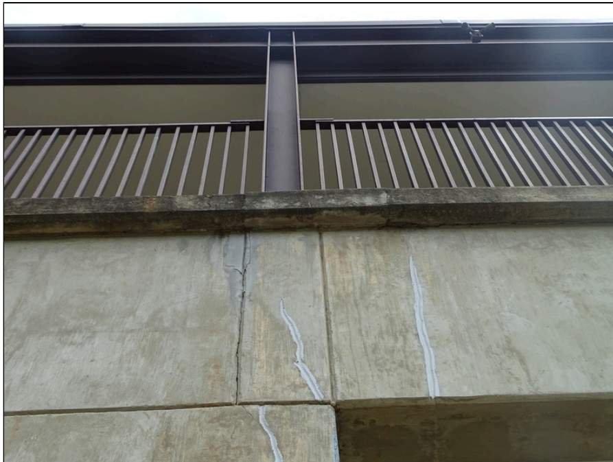
56 - Building exterior - note stained and sealant repair
