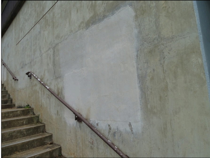
115 - Building exteriors concrete - note recent repairs
