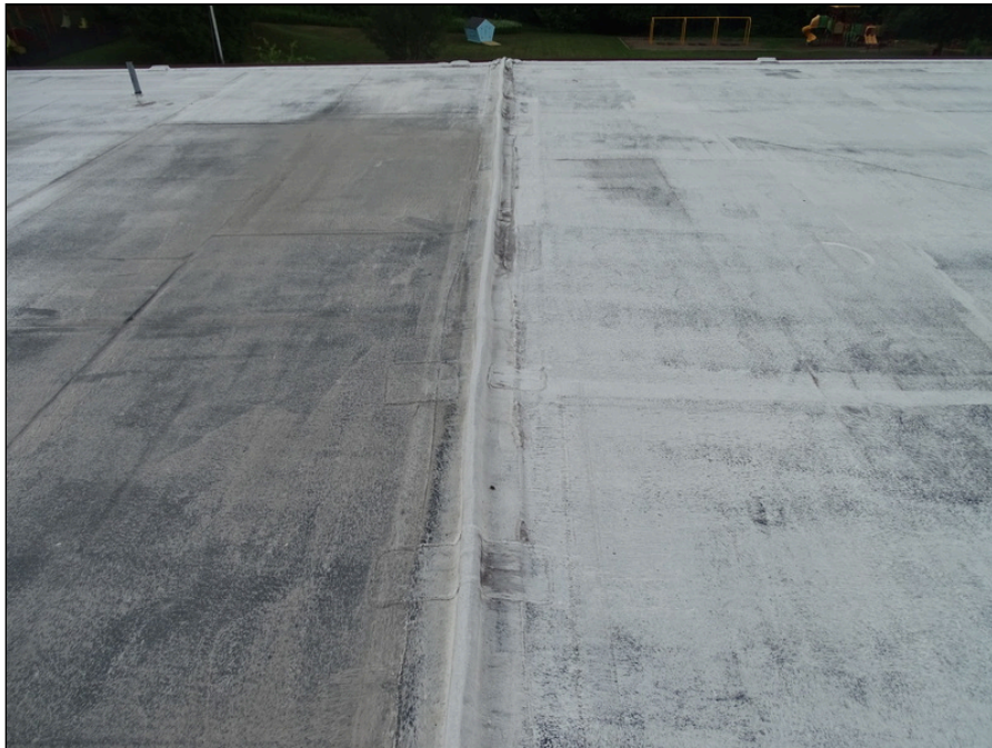
72 - Single-ply membrane roofing system - note patching
