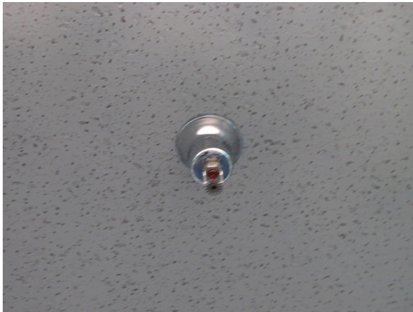
Typical sprinkler head
