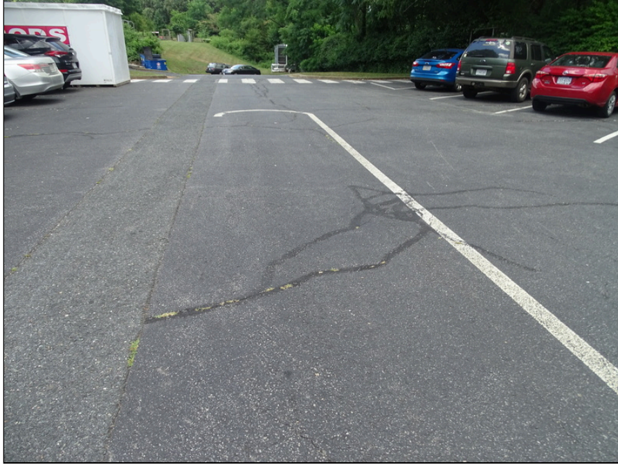
9 - Asphalt drive lane east side of the site - note cracking and previous repair
