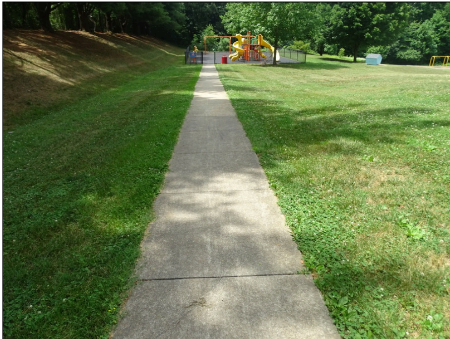
26 - Concrete sidewalk - note cracking
