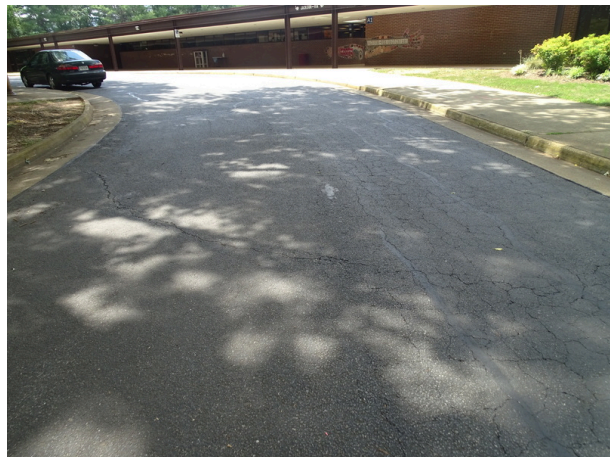
Asphalt drive lane west side of the site - note alligator cracks
