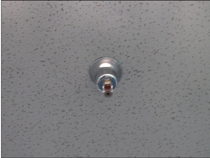
105 - Typical sprinkler head
