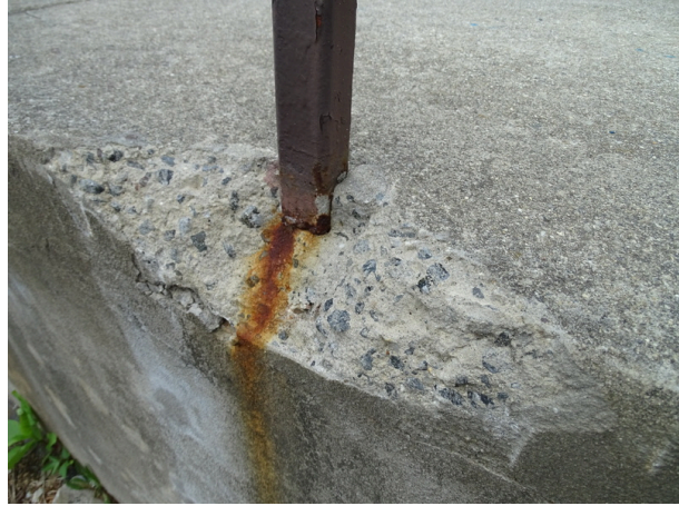
Concrete ramp- note deterioration
