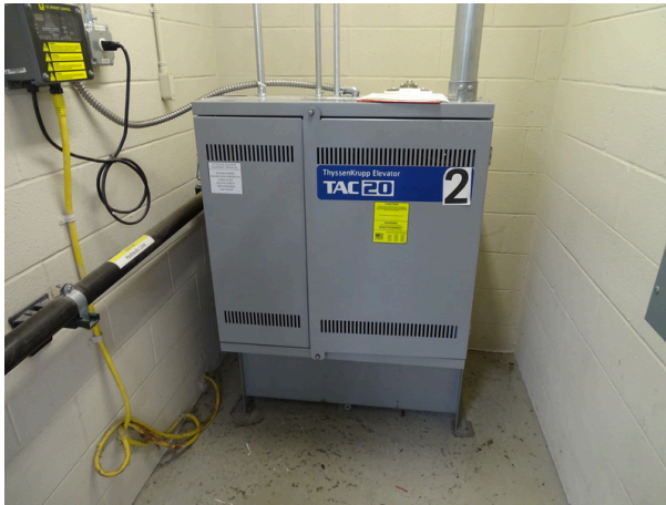
Hydraulic elevator machine and controls
