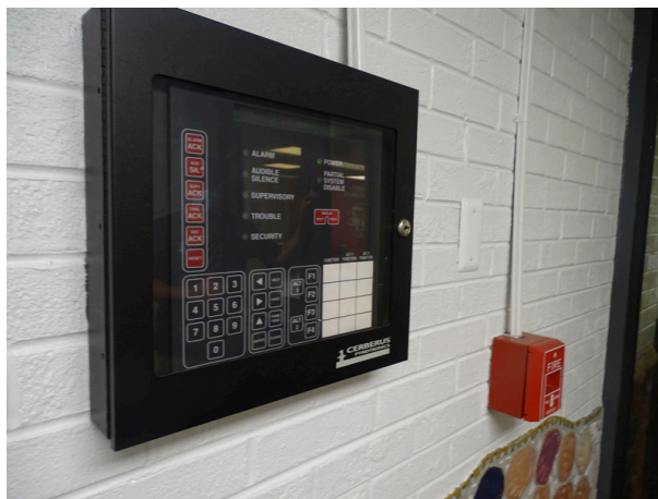
Fire alarm annunciator panel
