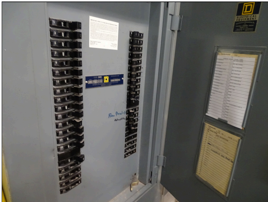
102 - Typical electrical circuit breaker panel
