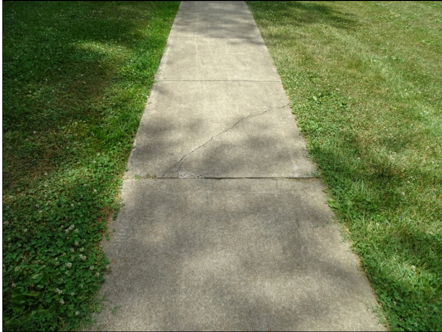
27 - Concrete sidewalk - note cracking
