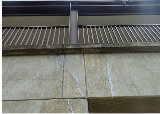
Building exterior - note stained and sealant repair
