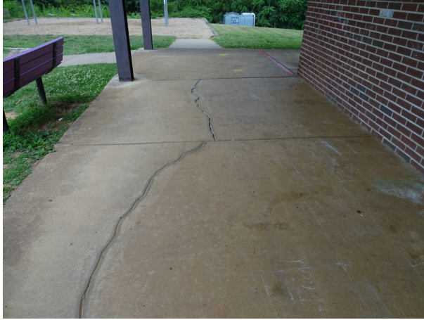
Concrete sidewalk - note cracking
