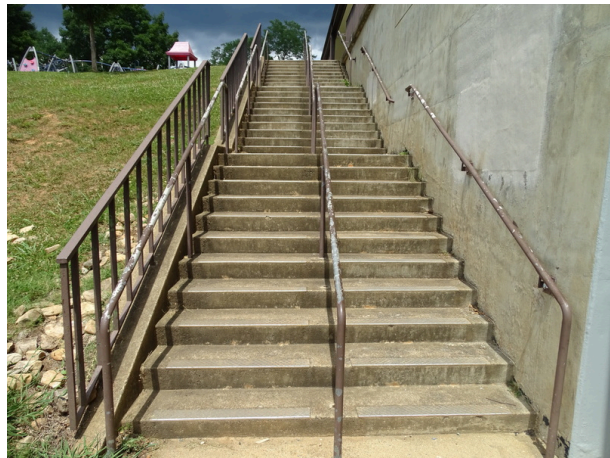
Concrete stair handrail - note deterioration
