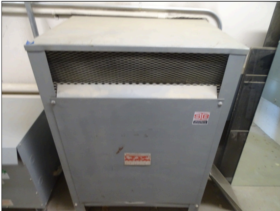
92 - Typical building transformer
