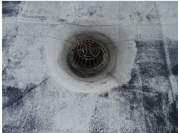
Typical interior drain
