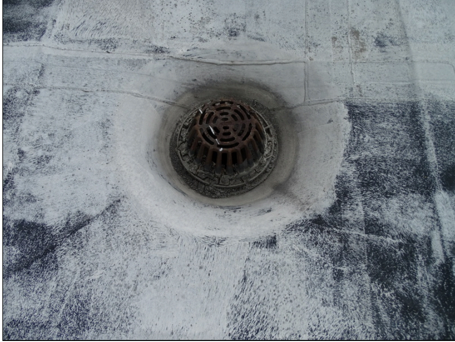
67 - Typical interior drain
