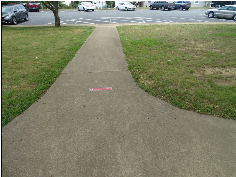
18 - Concrete sidewalk - note cracking
