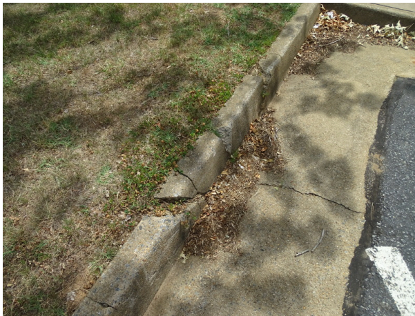
Concrete curb and gutter- note deterioration
