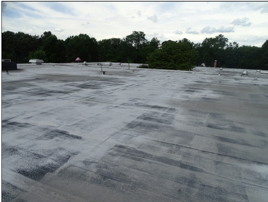
66 - Single-ply membrane roofing system
