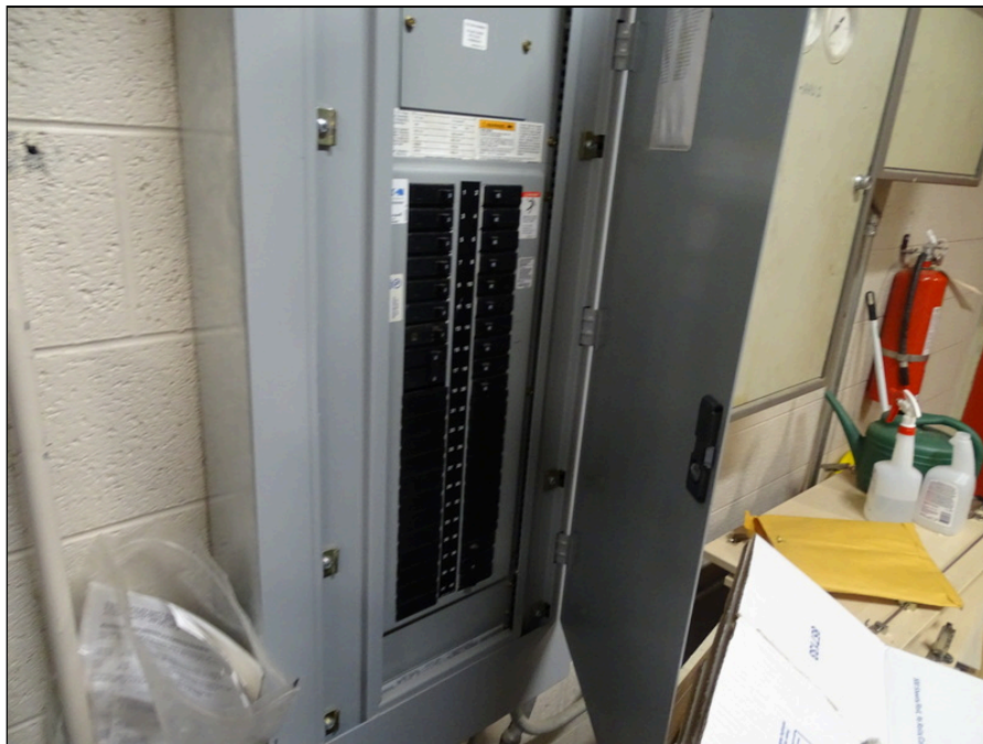
98 - Typical electrical circuit breaker panel
