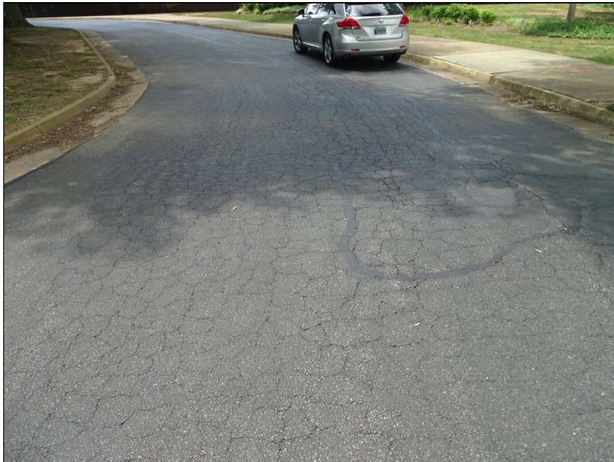
6 - Asphalt drive lane west side of the site - note cracking
