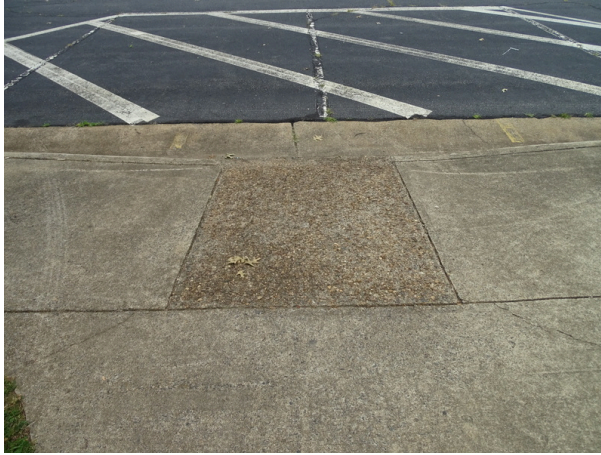
Concrete ramp - note need to install truncated domes
