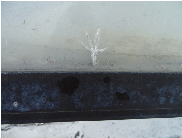
Skylights located on north side of the building - note glass cracked
