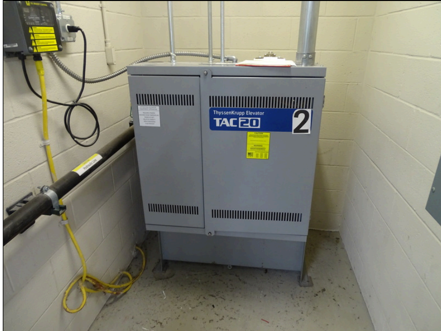
93 - Hydraulic elevator machine and controls
