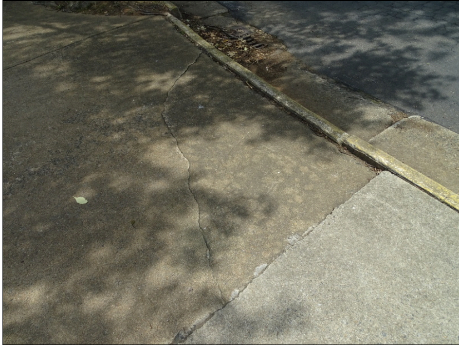
21 - Concrete sidewalk - note cracking
