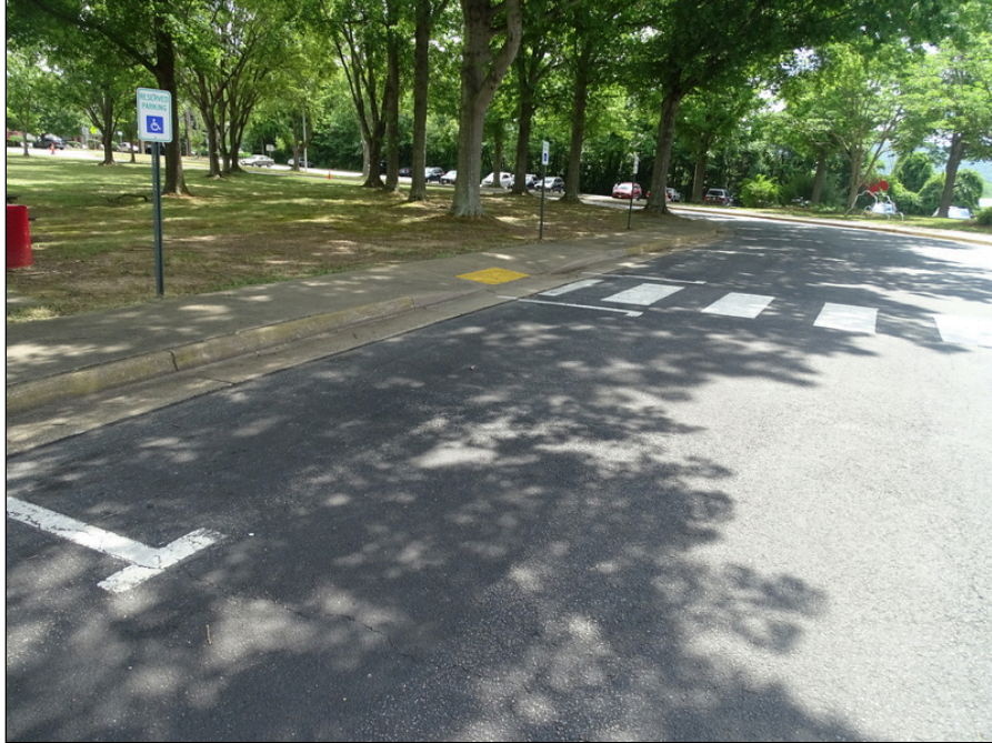
135 - Accessible parking spaces - note only two of five needed spaces provided
