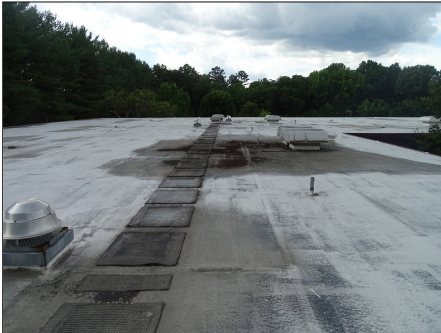
70 - Single-ply membrane roofing system looking west - note ponding
