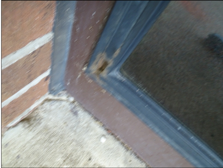
63 - Typical exterior window - note deterioration of gasket
