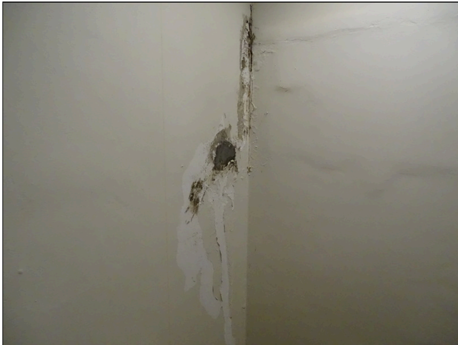
98 - Interior stair - note efflorescence
