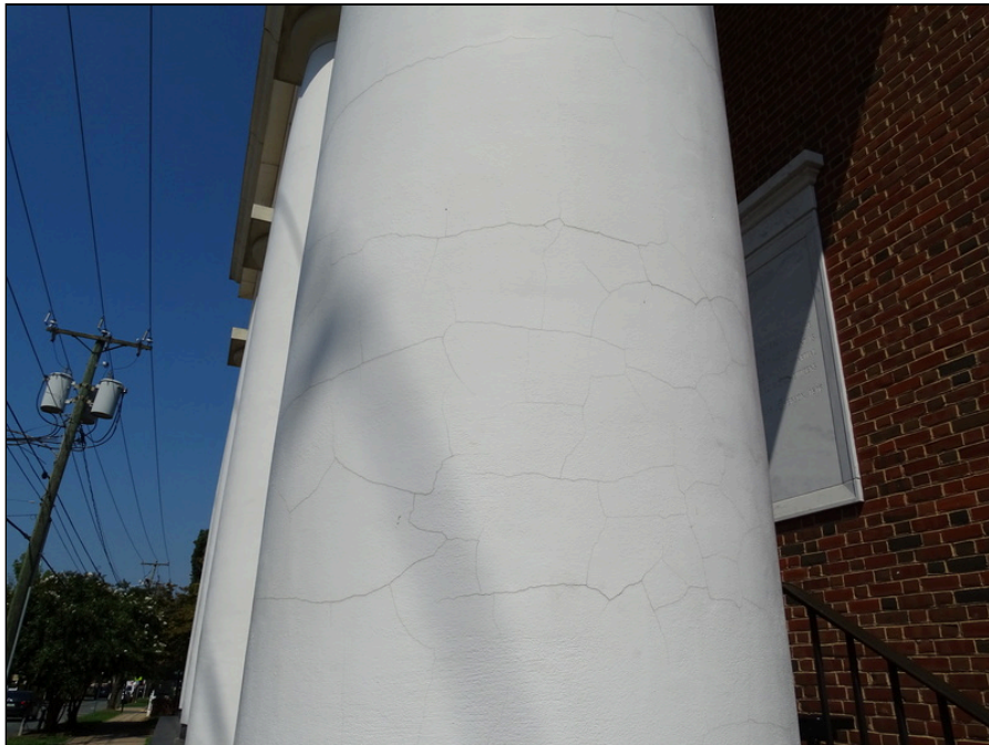
24 - Cracks in column at south side of Juvenile and Domestic Courts - Sheriff's Office - Parking Garage Complex
