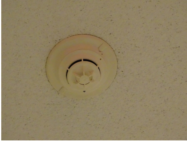
Typical smoke detector
