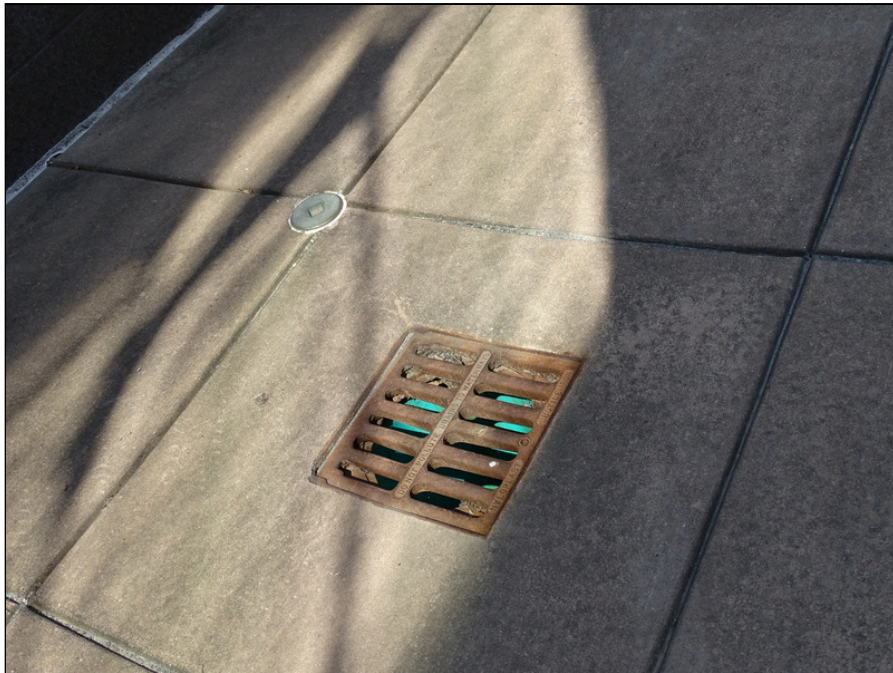
12 - Storm water yard inlet drainage
