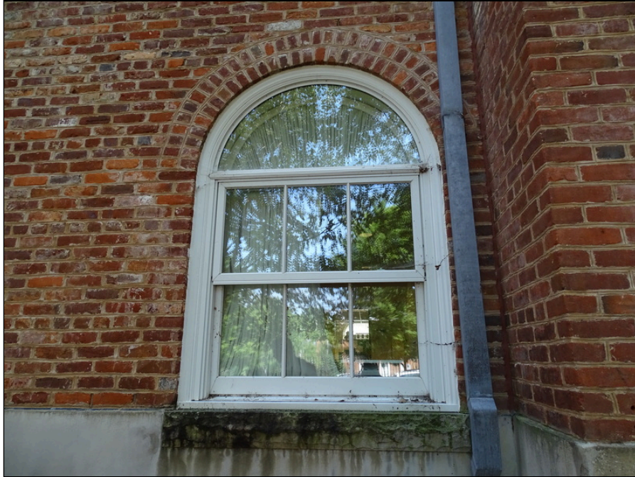
33 - Typical window at courthouse - note efflorescence
