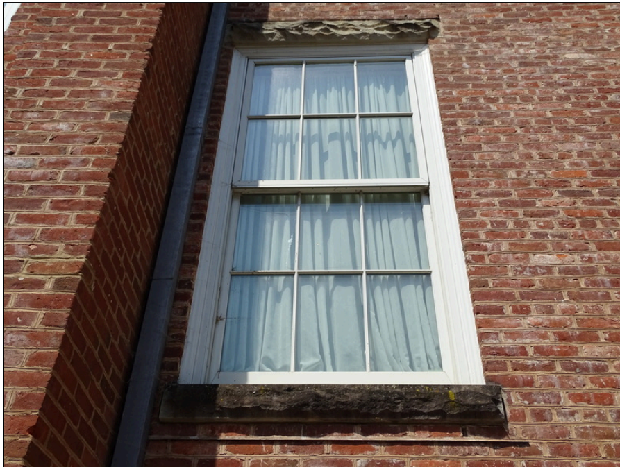
34 - Typical window at courthouse - note efflorescence
