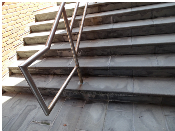
Typical stair at north side of courthouse - note efflorescence
