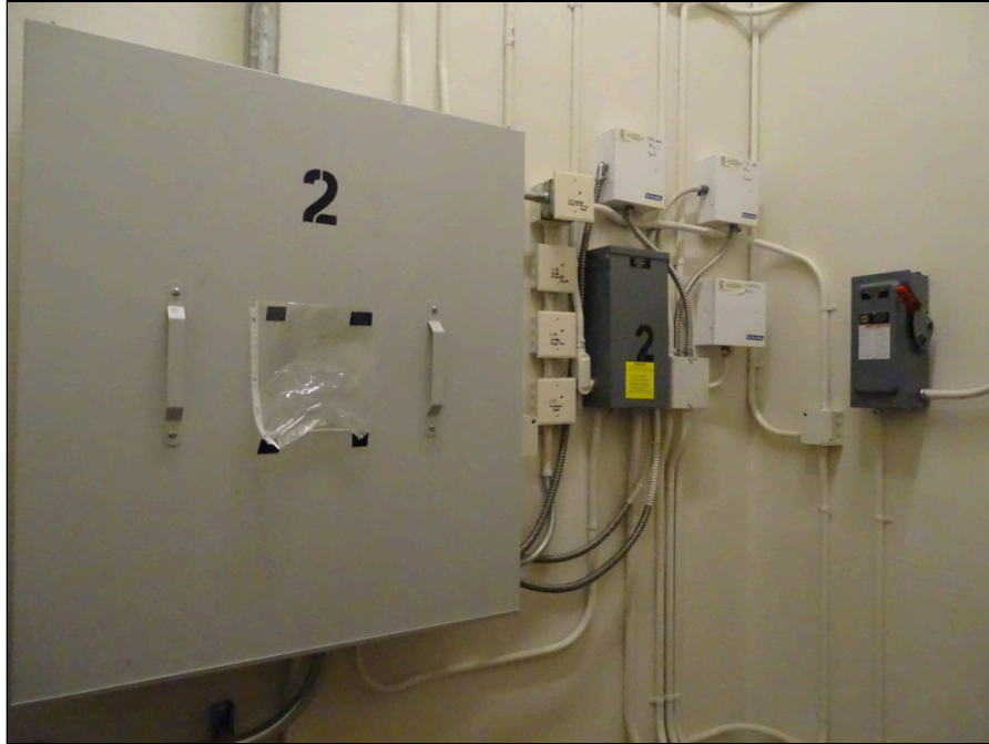
65 - Elevator controls
