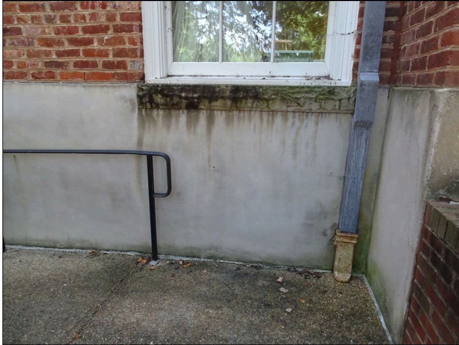
15 - Typical downspout and efflorescence in wall
