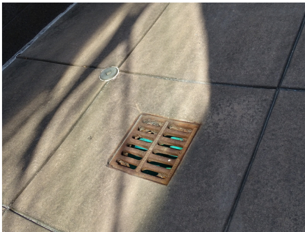
Storm water yard inlet drainage
