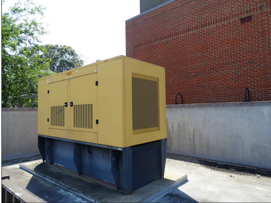
59 - Emergency back up power generator
