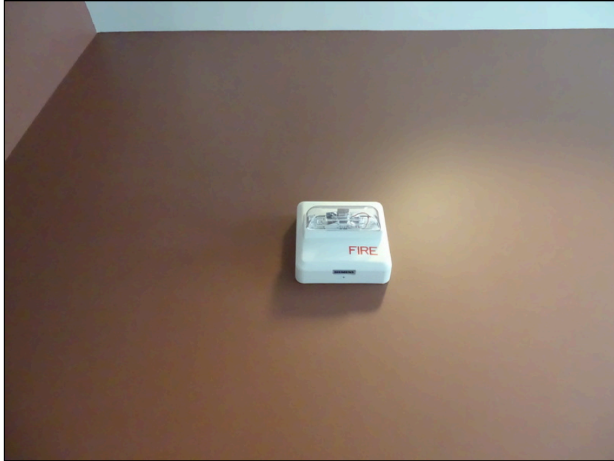
75 - Typical fire alarm bell and strobe
