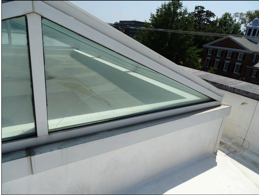
45 - Skylight - note crack in glass on east side
