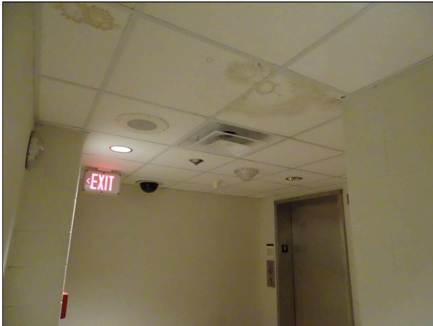
102 - Interior lobby - note water leakage and stains in the ceiling
