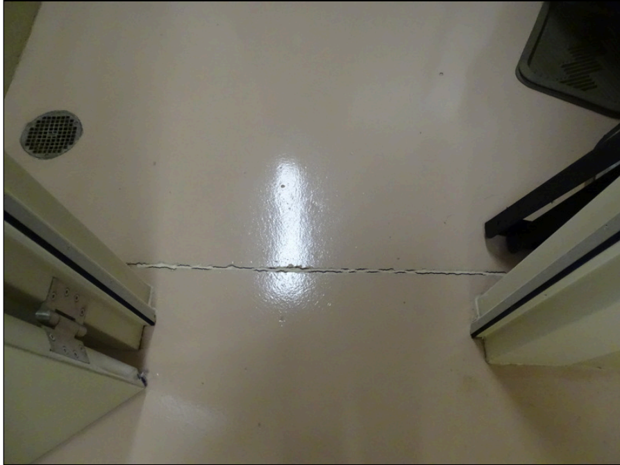
23 - Parking garage - note crack in floor
