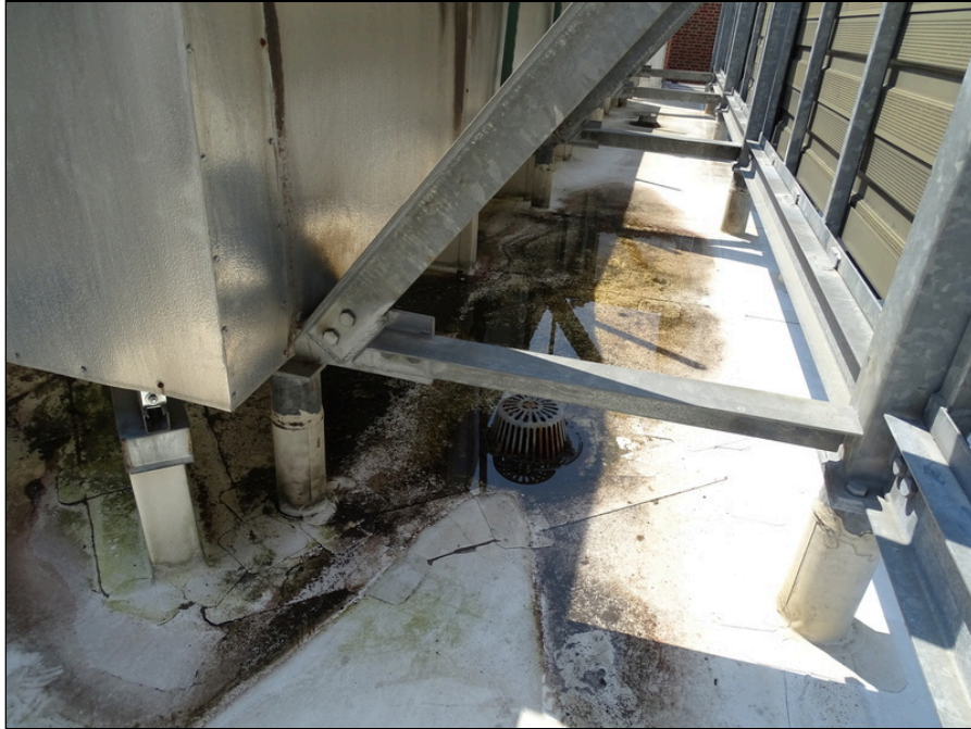
49 - Roofing system at center portion of courthouse - note ponding
