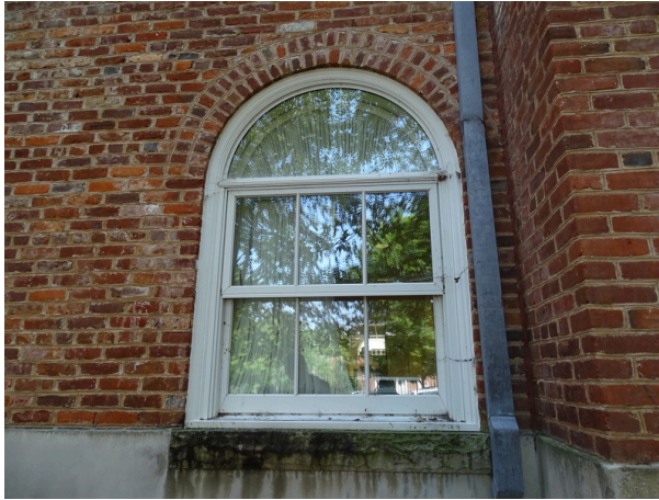
Typical window at courthouse - note efflorescence
