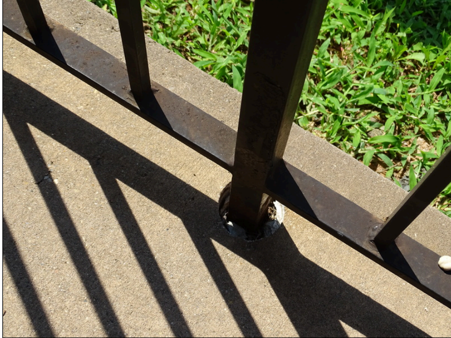
5 - Ramp at southwest side of courthouse building. Note deterioration of handrail base
