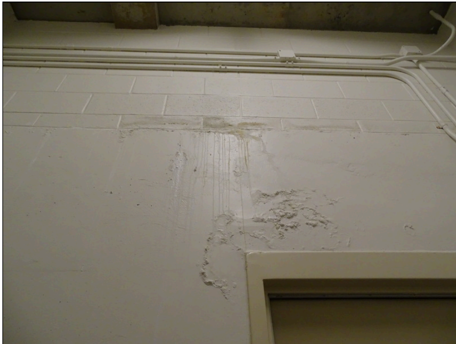
96 - Interior stair - note efflorescence
