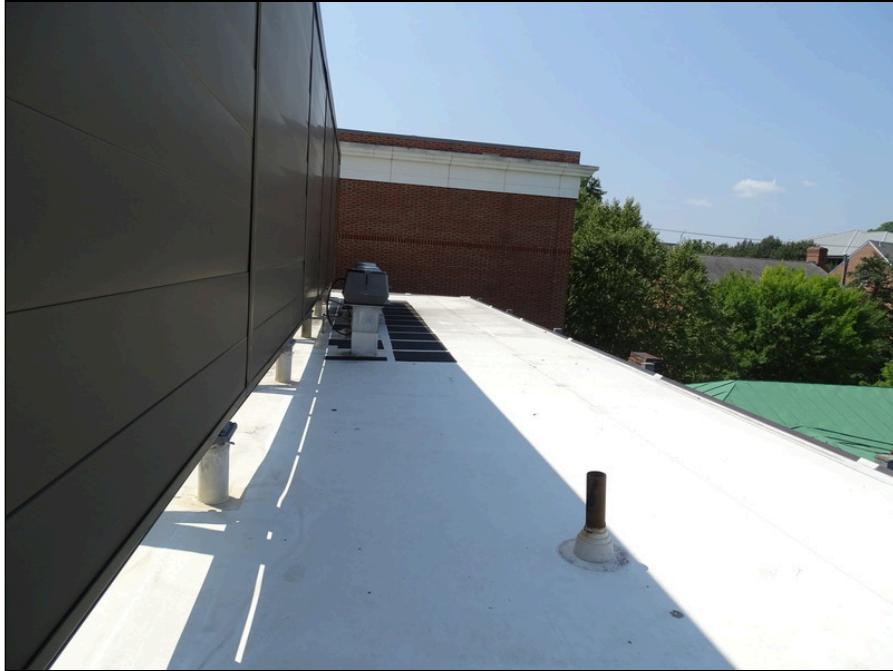
47 - Typical plumbing vent roof penetration
