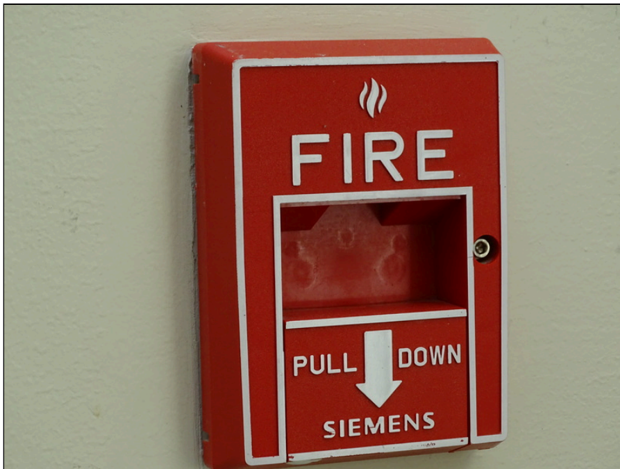
74 - Typical fire alarm pull station
