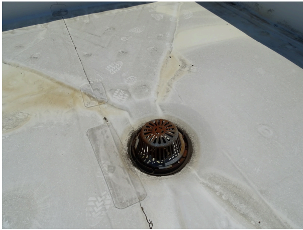
Typical internal drain
