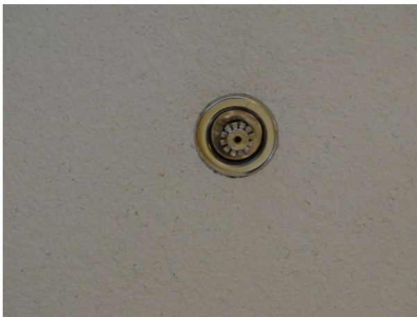
Typical sprinkler head
