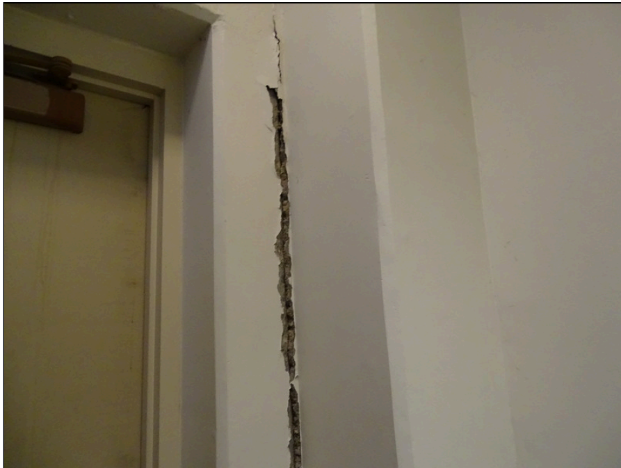
22 - Building frame at sheriffs office north side at lower level entrance - note cracking
