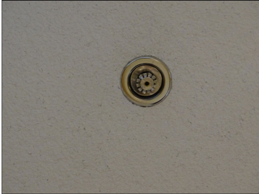
69 - Typical sprinkler head
