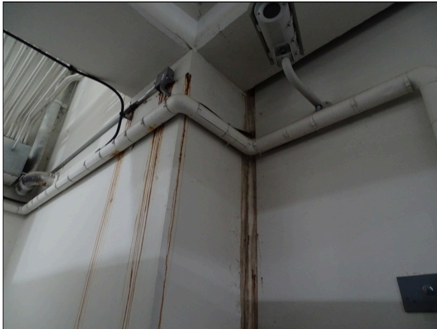
106 - Parking garage - note water leakage
