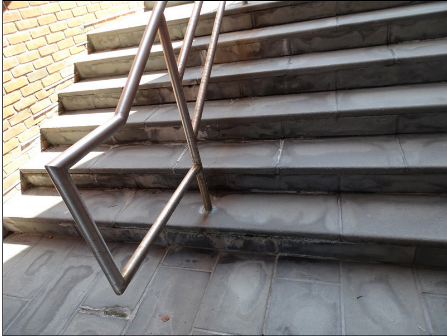
9 - Typical stair at north side of courthouse - note efflorescence
