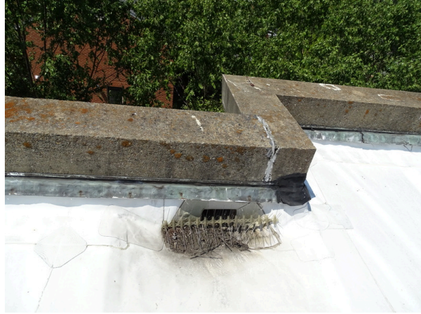
Parapet wall on courts building center portion - note patching
