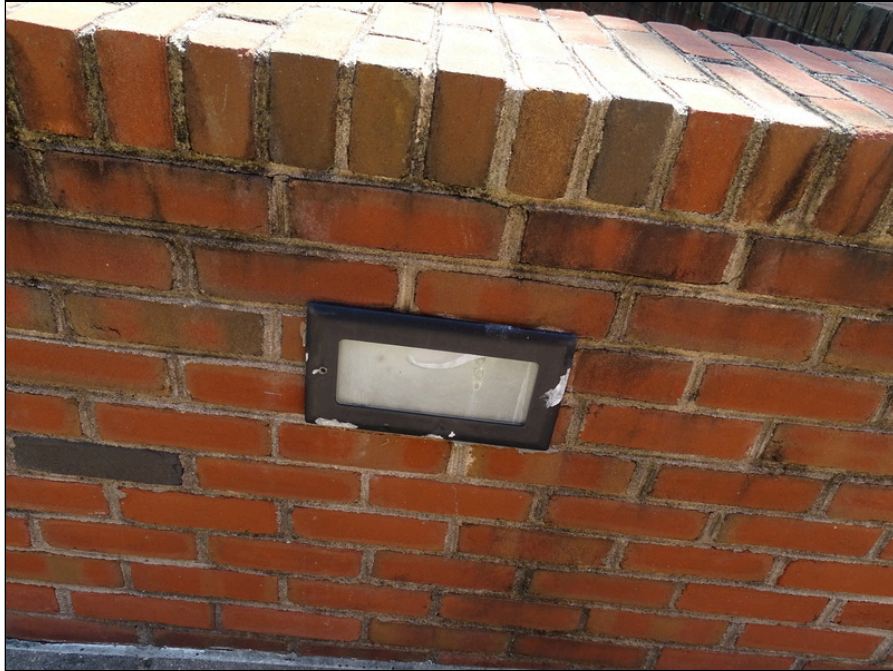
21 - Retaining wall at west side of the property - note efflorescence
