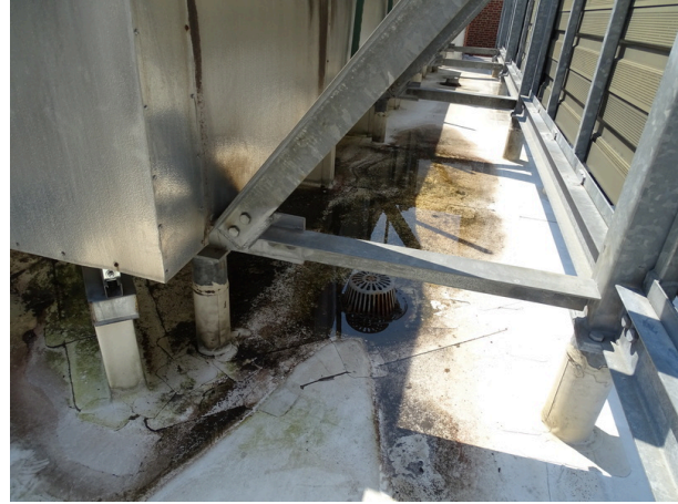
Roofing system at center portion of courthouse - note ponding
