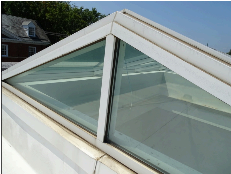
44 - Skylight - note crack in glass on east side
