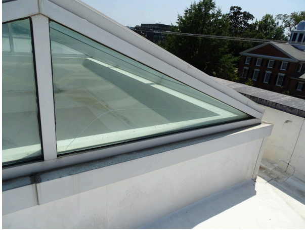
Skylight - note crack in glass on east side
