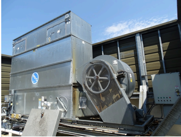
Roof top cooling tower
