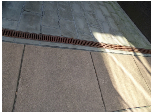
Storm water yard inlet drainage
