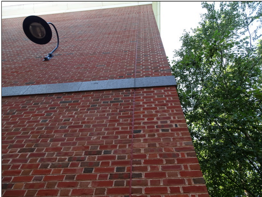
26 - Vertical sealant at east side of the building
