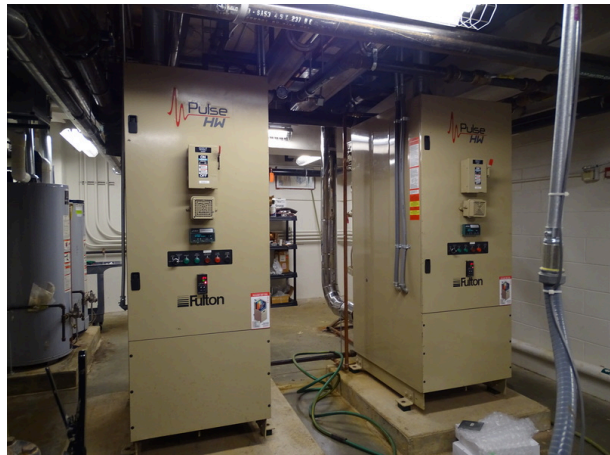
Boilers located in main utility room
