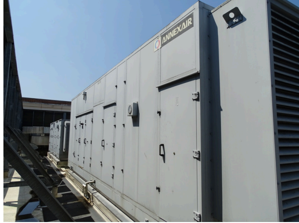
Roof top energy recovery unit
