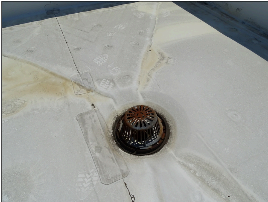
46 - Typical internal drain
