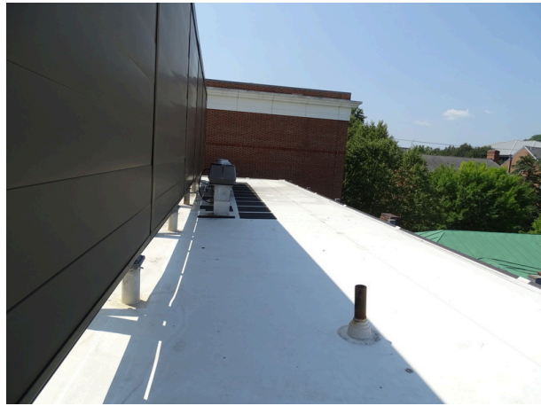
Typical plumbing vent roof penetration
