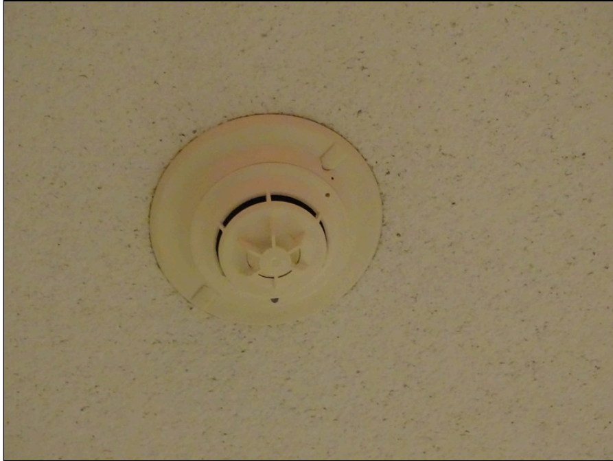
77 - Typical smoke detector
