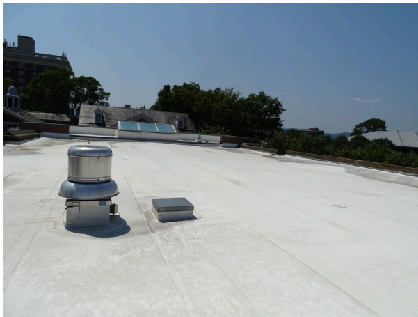
Exhaust fan located on roof top
