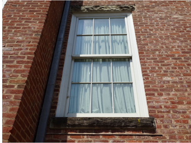
Typical window at courthouse - note efflorescence
