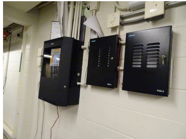
Fire sprinkler control panel
