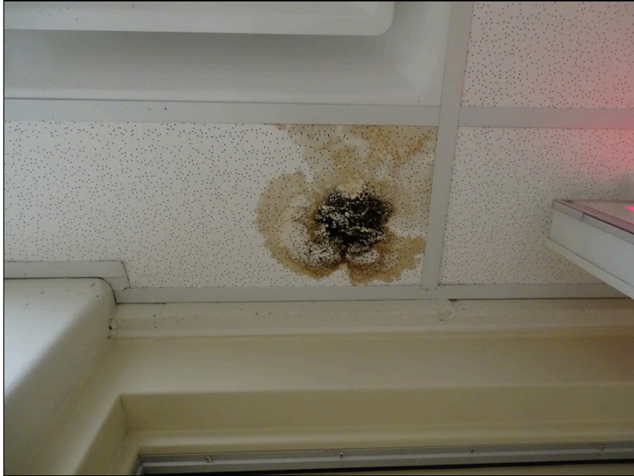
99 - Stained in the ceiling panel
