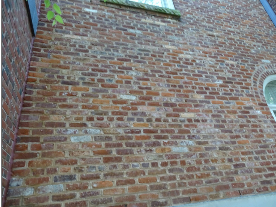
25 - Exterior wall- note efflorescence
