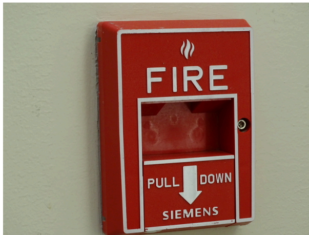
Typical fire alarm pull station
