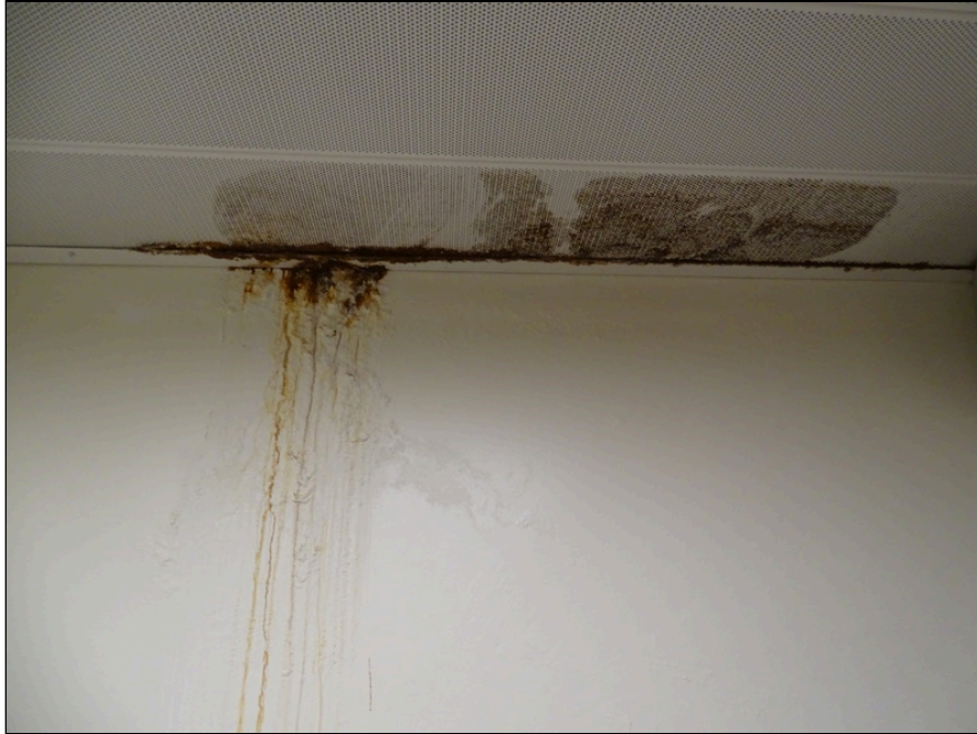
109 - Parking garage - note water leakage
