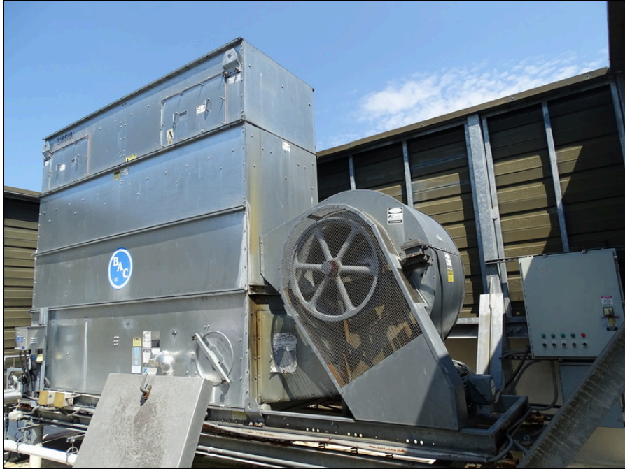
53 - Roof top cooling tower
