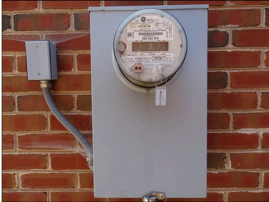
57 - Electric meter at the north side of the building
