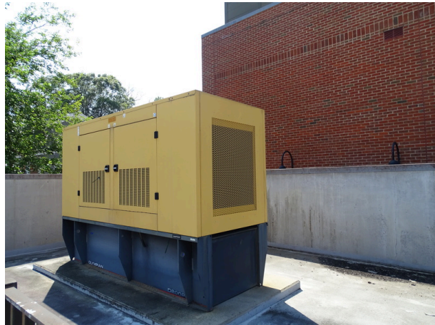
Emergency back up power generator
