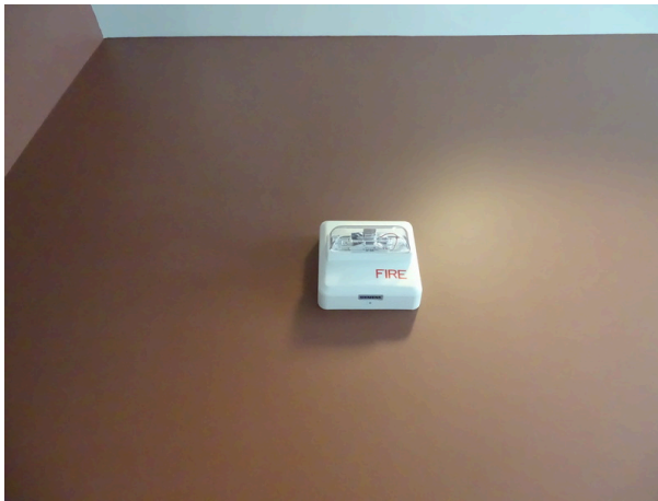
Typical fire alarm bell and strobe
