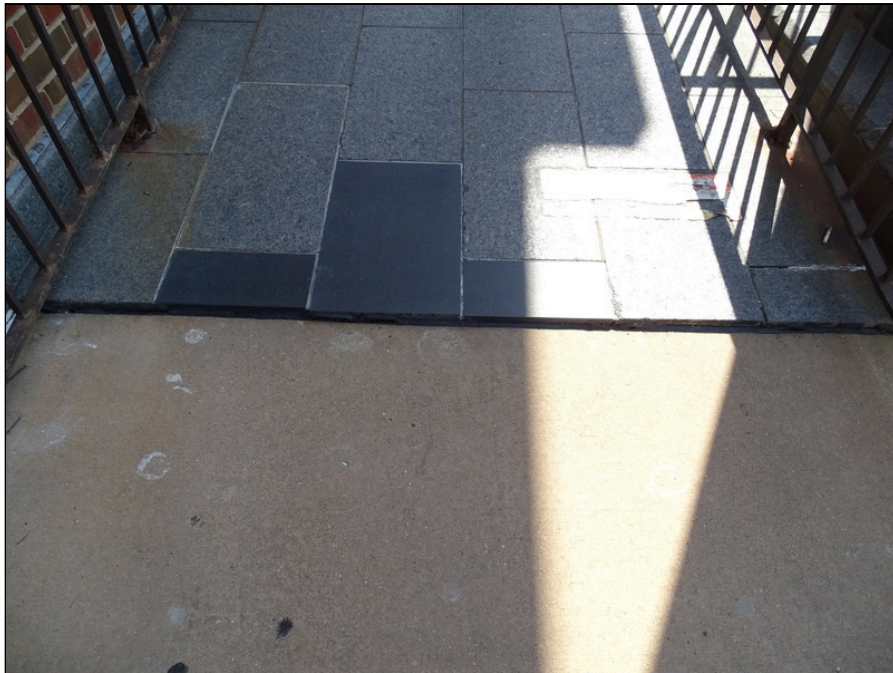
4 - Ramp at southwest side of courthouse building - note trip hazard
