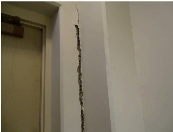
Building frame at sheriffs office north side at lower level entrance - note cracking
