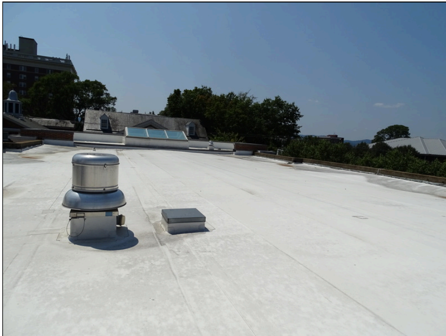
48 - Exhaust fan located on roof top
