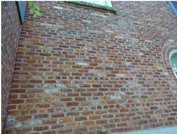
Exterior wall- note efflorescence
