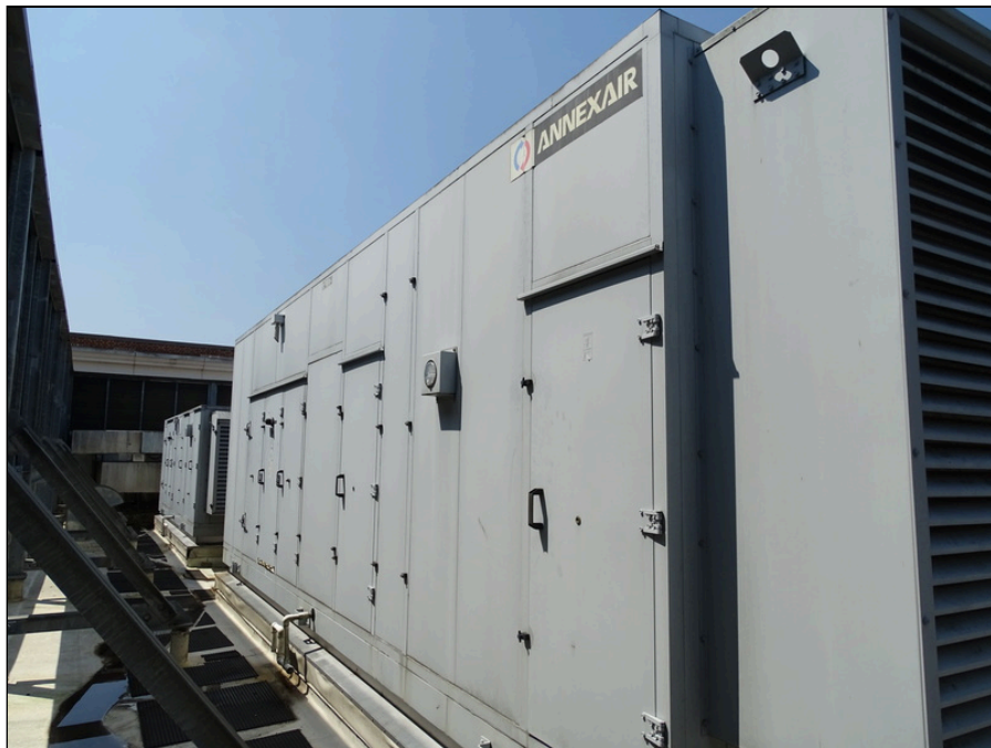
52 - Roof top energy recovery unit
