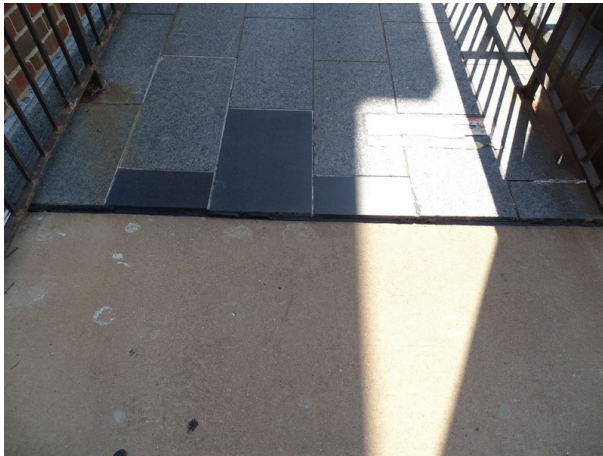
Ramp at southwest side of courthouse building - note trip hazard
