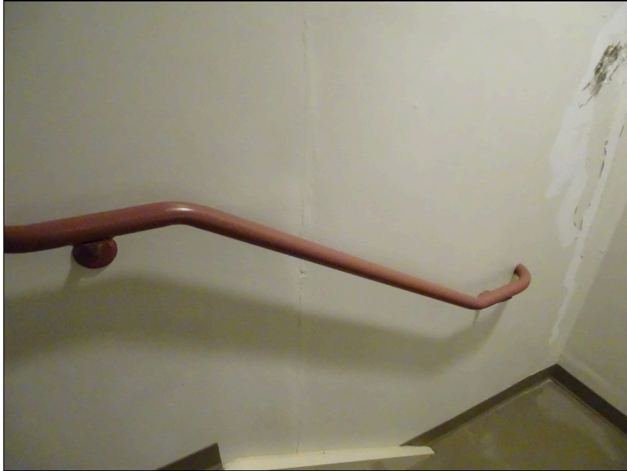
95 - Interior stair - note efflorescence
