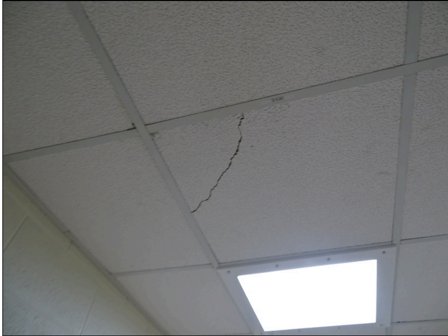
101 - Interior lobby - note ceiling panel deterioration
