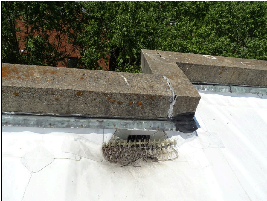
42 - Parapet wall on courts building center portion - note patching
