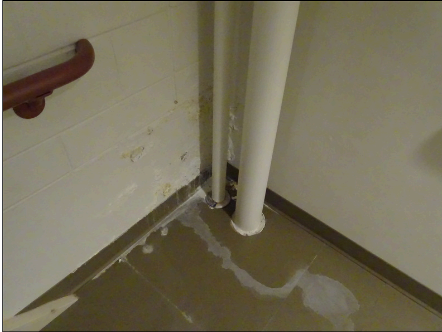
97 - Interior stair - note efflorescence
