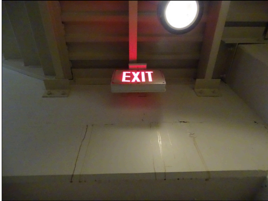
105 - Parking garage - note water leakage
