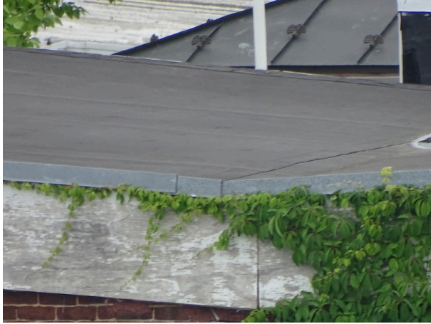
Single-ply membrane roofing system
