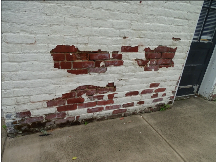
11 - Building exterior at north end of the building - note peeling paint
