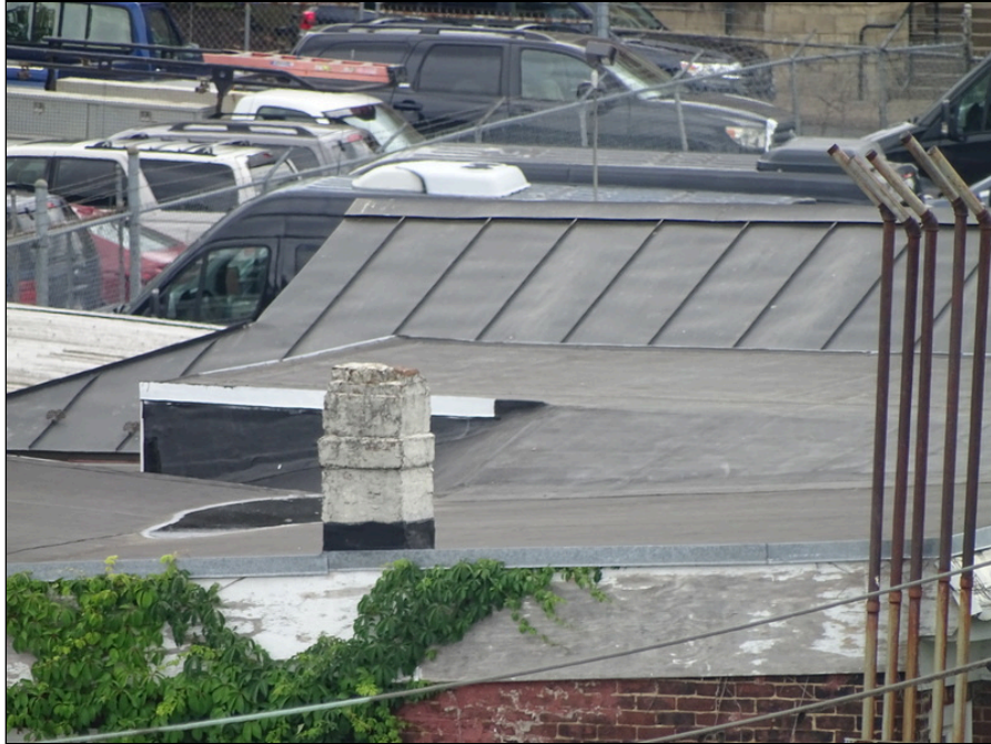
25 - Single-ply membrane roofing system
