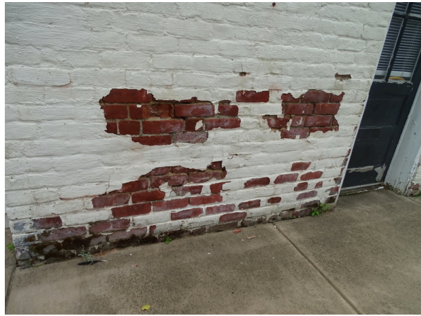
Building exterior at north end of the building - note peeling paint
