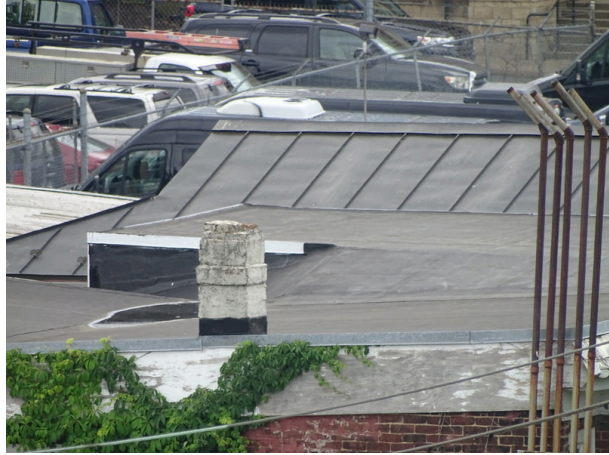
Single-ply membrane roofing system
