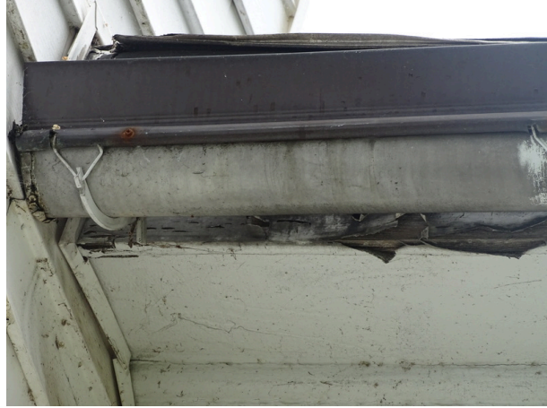
Typical gutter - note deterioration
