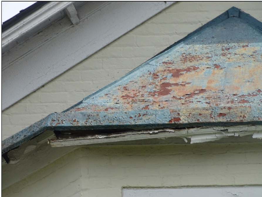
28 - Typical wood trim - note deterioration
