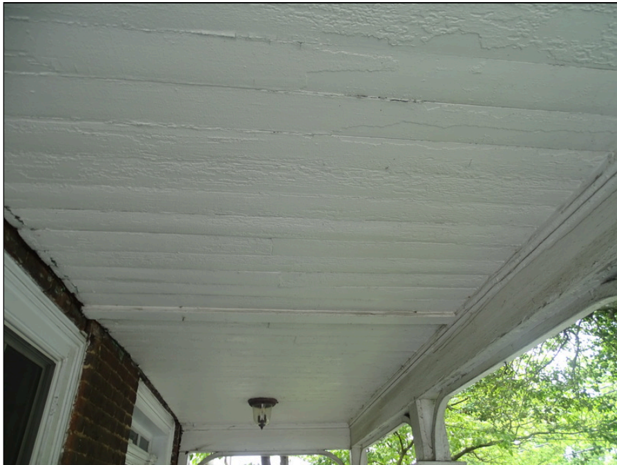
52 - Typical Patio ceiling - note deterioration
