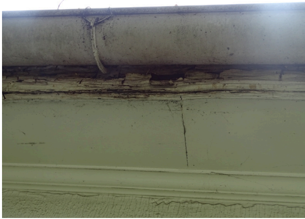
Typical gutter - note deterioration
