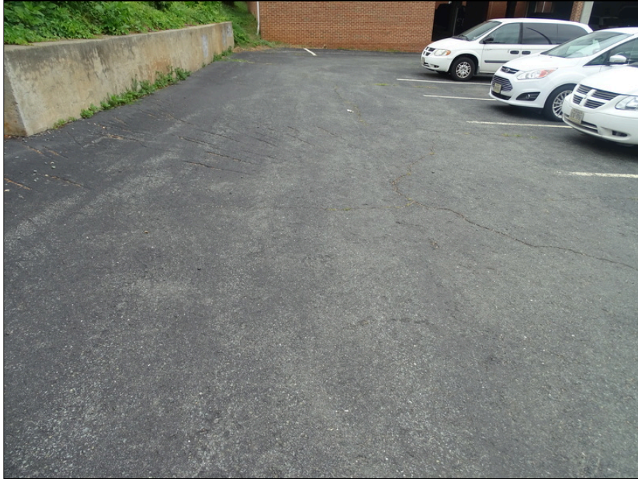
3 - Asphalt parking north side of the building - note stripping faded
