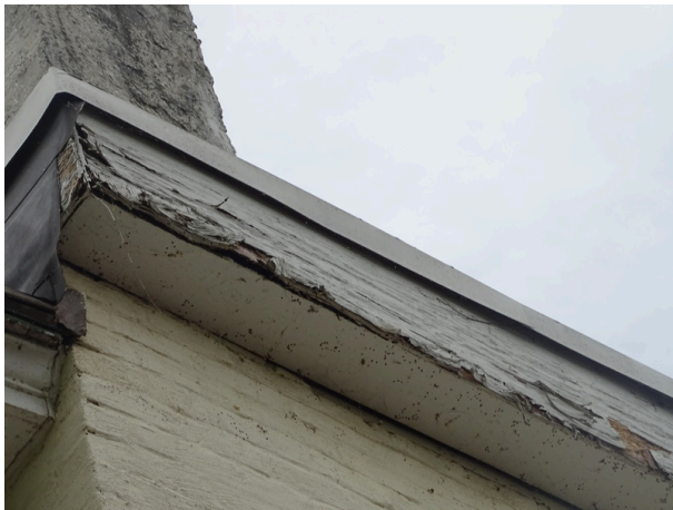
Building exterior at north end of the building - note deteriorated wood trim
