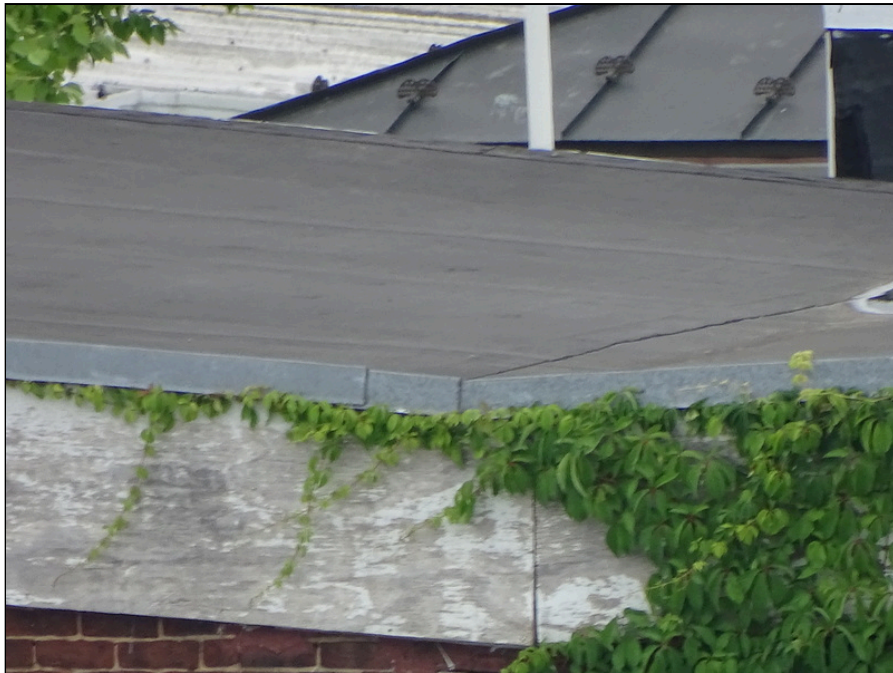
24 - Single-ply membrane roofing system
