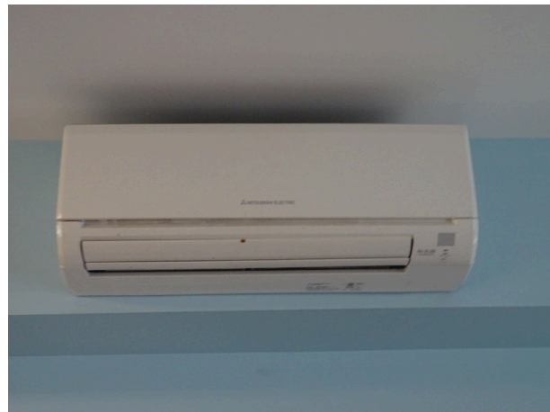
Wall mounted split system unit servicing meeting room area
