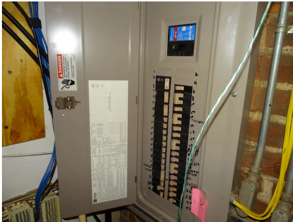
Main electrical disconnect and circuit breaker panel
