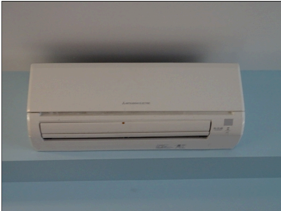
34 - Wall mounted split system unit servicing meeting room area
