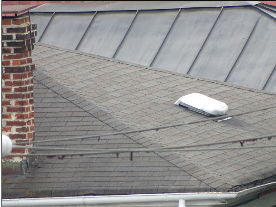
23 - Asphalt shingle roofing system
