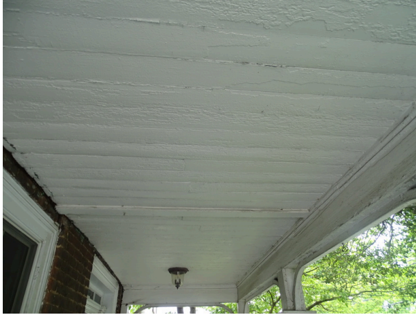
Typical Patio ceiling - note deterioration
