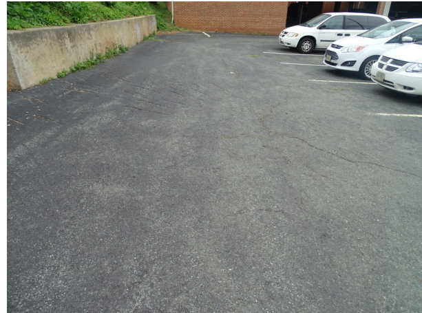
Asphalt parking north side of the building - note stripping faded
