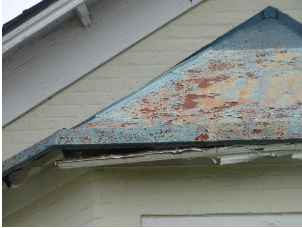
Typical wood trim - note deterioration
