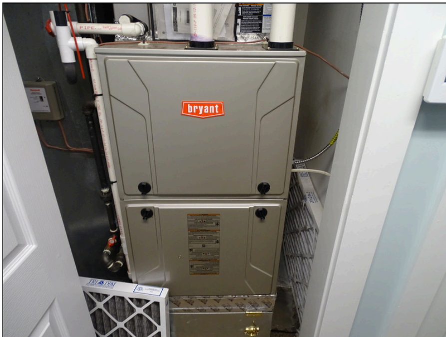
32 - Gas Furnace - Air Handler Unit located in utility closet
