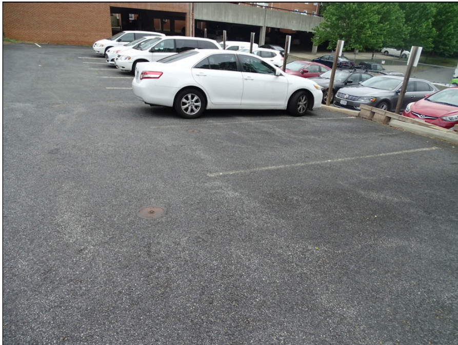
2 - Asphalt parking north side of the building - note stripping faded
