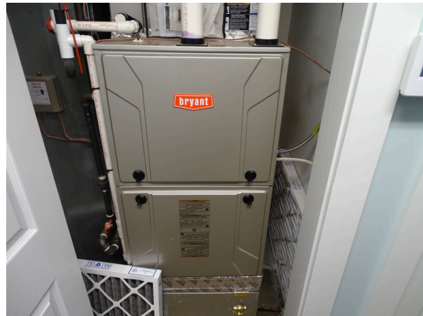
Gas Furnace - Air Handler Unit located in utility closet
