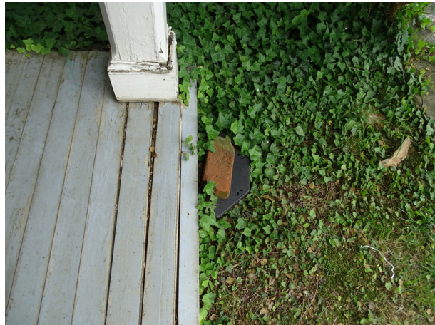
Typical column - note deterioration
