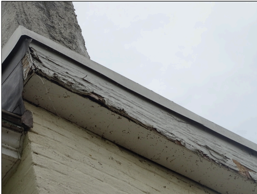
26 - Building exterior at north end of the building - note deteriorated wood trim
