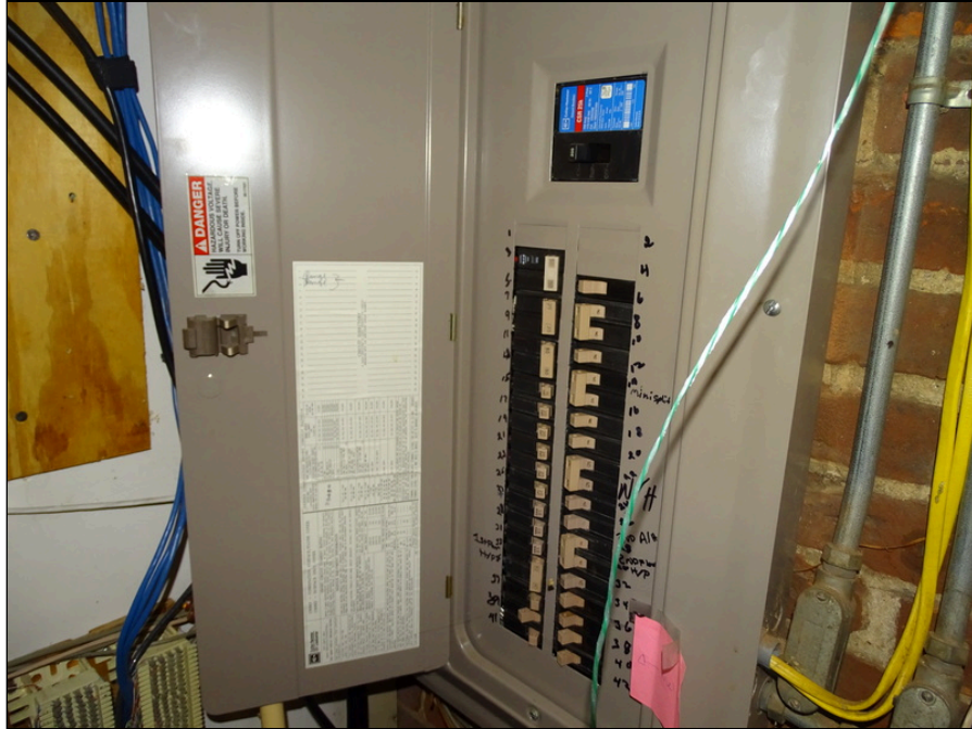
39 - Main electrical disconnect and circuit breaker panel
