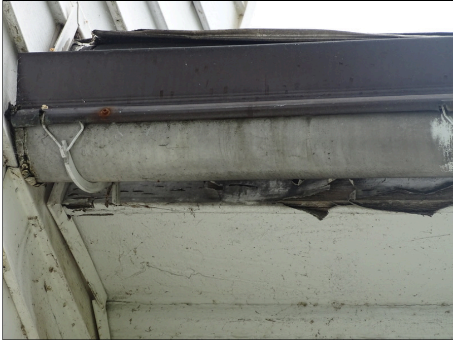
29 - Typical gutter - note deterioration
