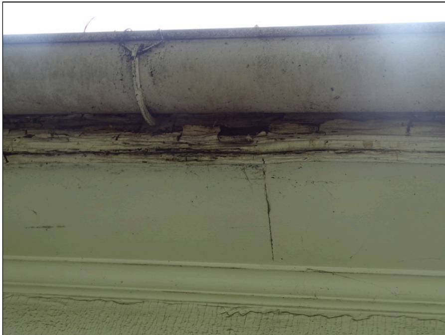
30 - Typical gutter - note deterioration
