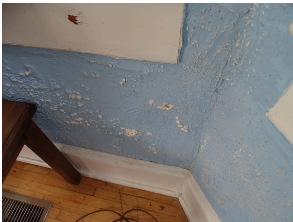
Interior finishes meeting area - note efflorescence
