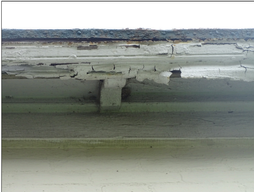
46 - Typical soffit - note peeling paint
