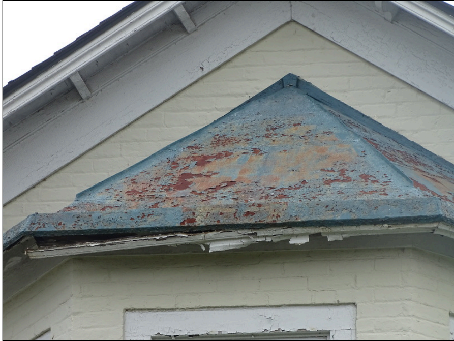
51 - Wood trim - note deterioration
