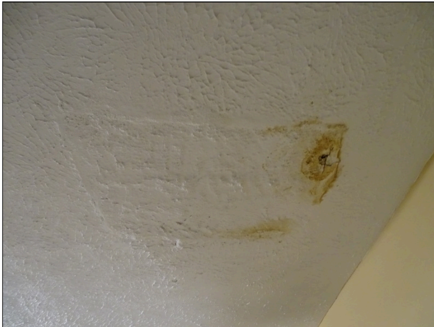
40 - Reported leakage of roofing system
