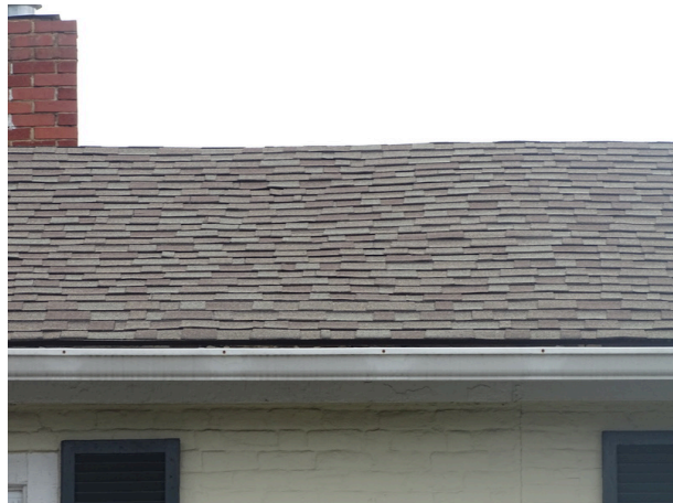
Asphalt shingle roofing system
