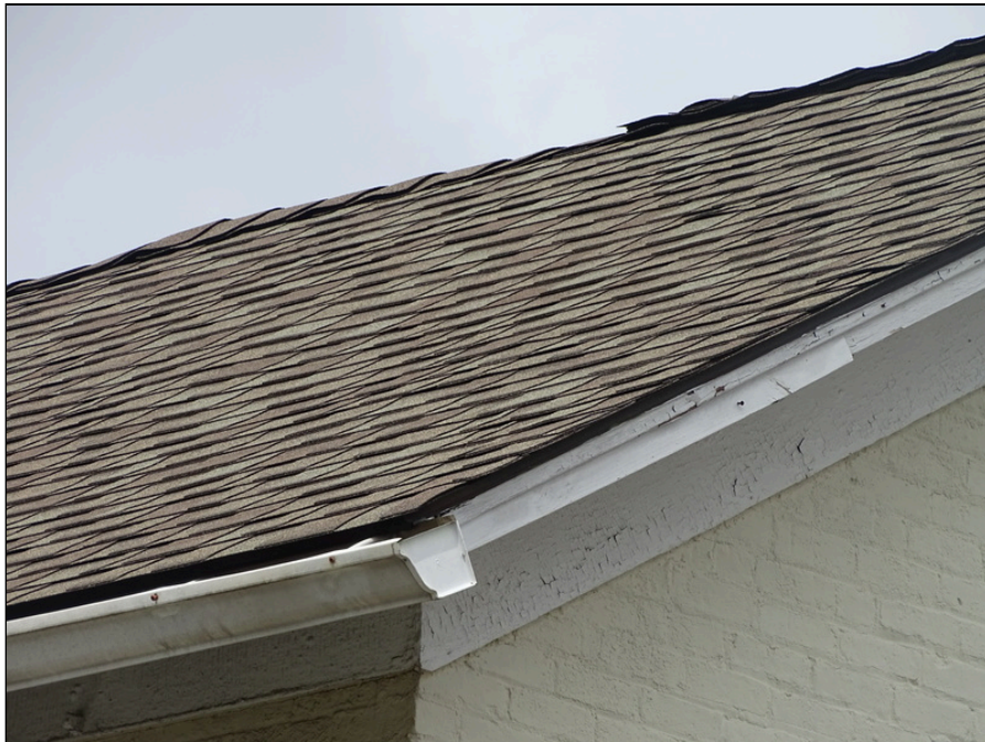
32 - Asphalt shingle roofing system
