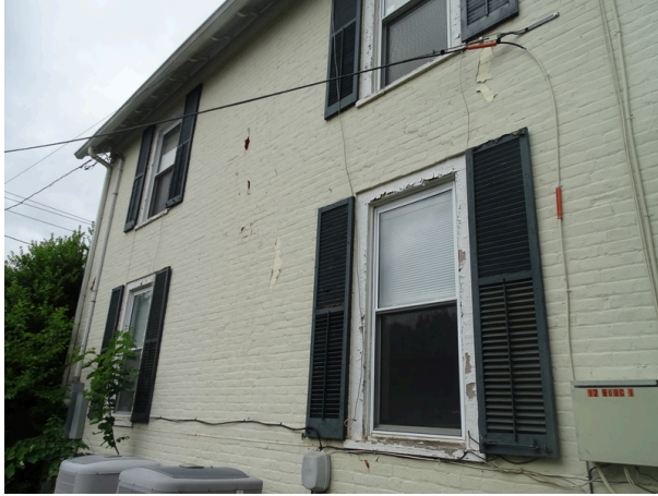
Building exterior east side of the building - note peeling paint
