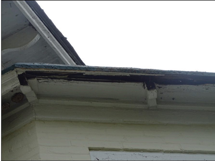
47 - Typical soffit - note peeling paint
