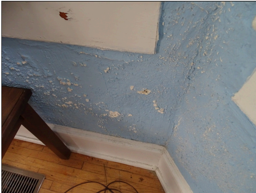
70 - Interior finishes meeting area - note efflorescence
