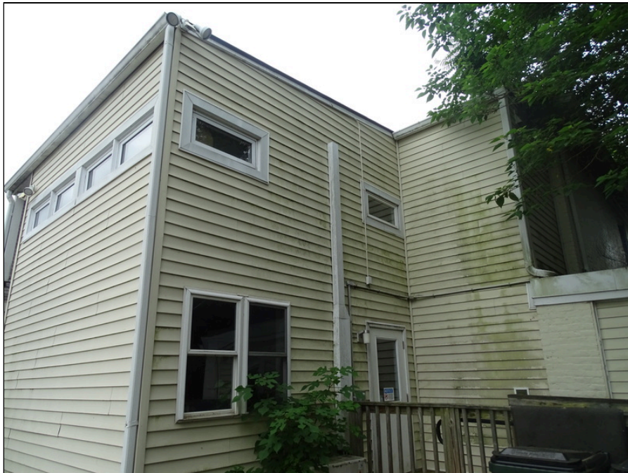
20 - Vinyl siding at north addition
