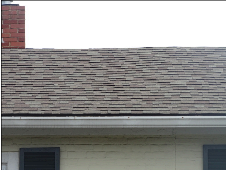
35 - Asphalt shingle roofing system
