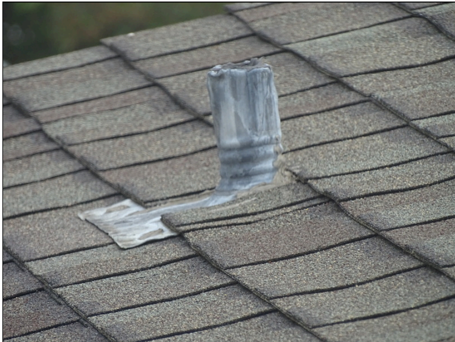
38 - Typical plumbing penetration
