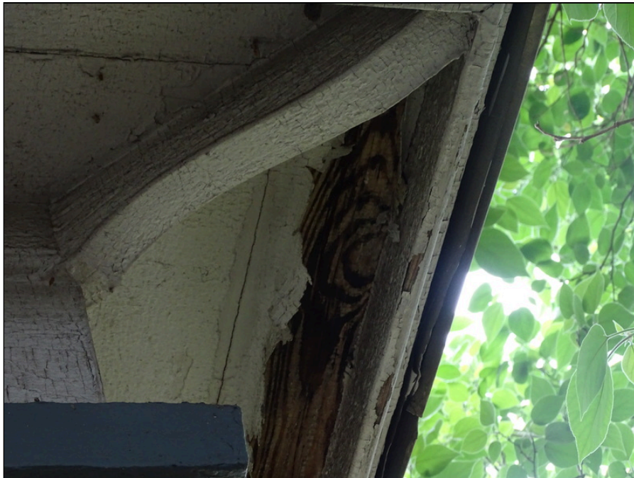
48 - Typical soffit - note peeling paint
