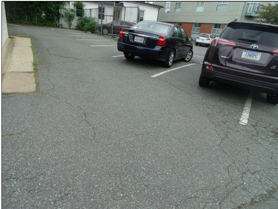
2 - Asphalt parking north side of the building - note cracking
