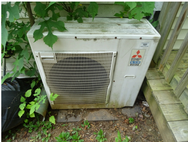
Split system exterior condenser
