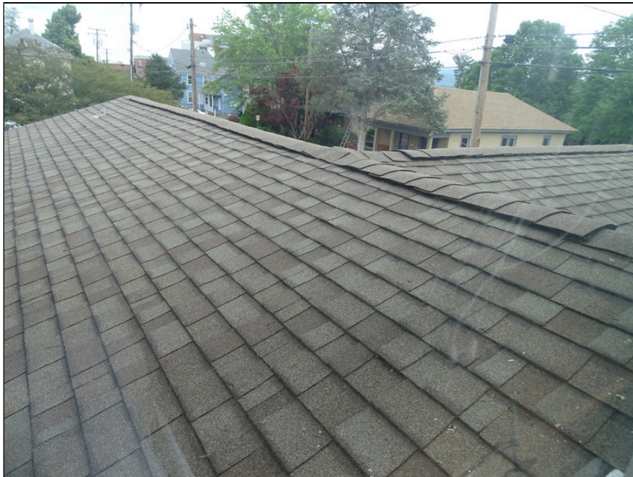
36 - Asphalt shingle roofing system
