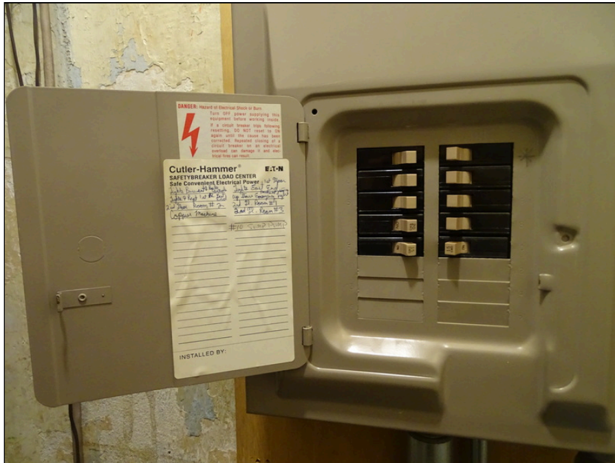
62 - Typical circuit breaker panel
