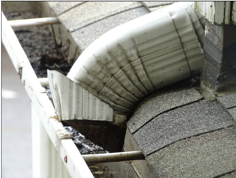
44 - Gutter and downspout - note derterioration
