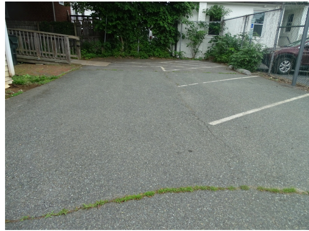
Asphalt parking north side of the building - note cracking
