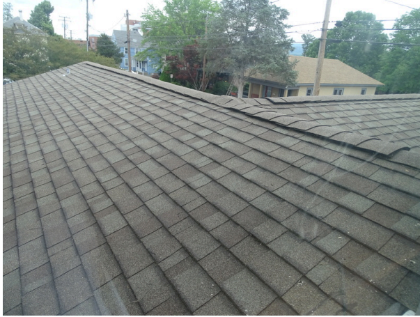
Asphalt shingle roofing system
