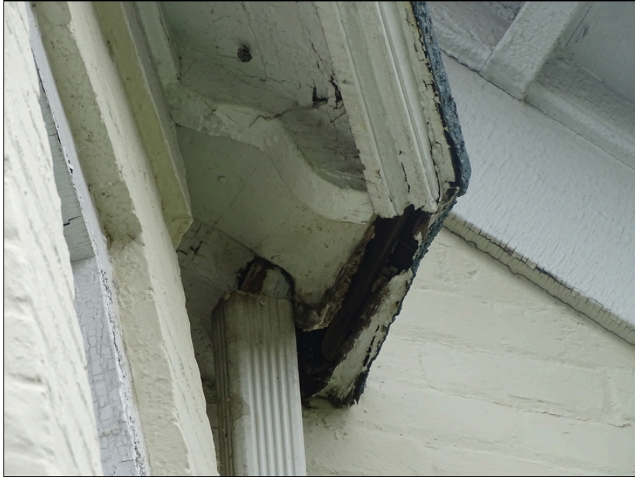
49 - Typical soffit - note deterioration
