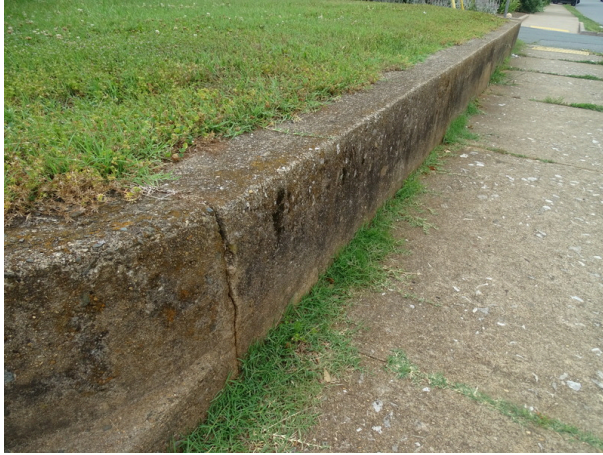
Concrete ramp at south side of the building - note cracking of concrete wall
