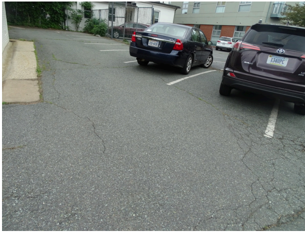
Asphalt parking north side of the building - note cracking
