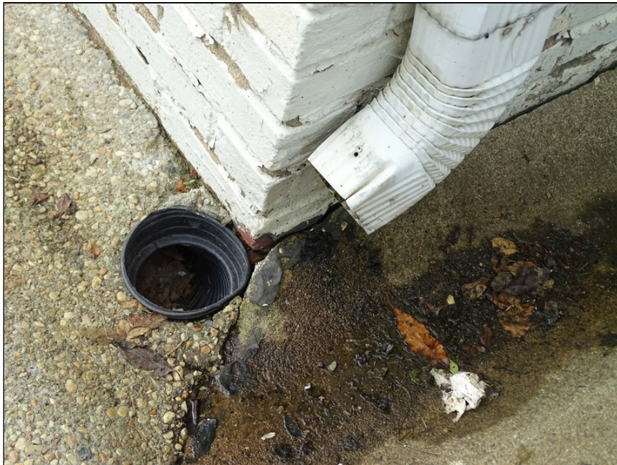
12 - Typical downspout - note deterioration
