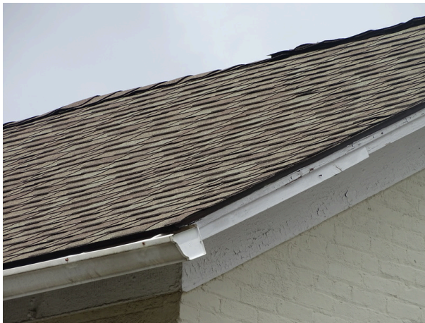
Asphalt shingle roofing system
