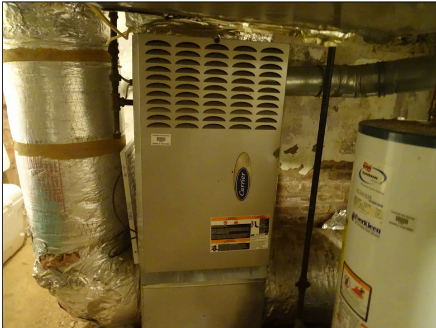
54 - Gas furnace - air handler unit
