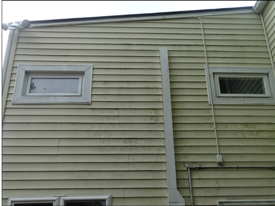
21 - Vinyl siding at north addition - note needed maintenance
