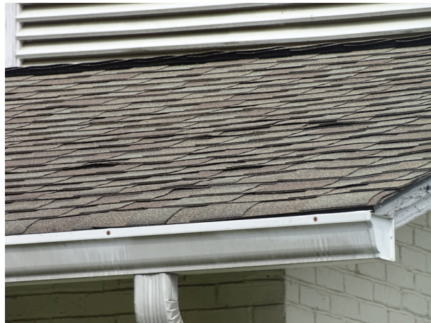
Asphalt shingle roofing system
