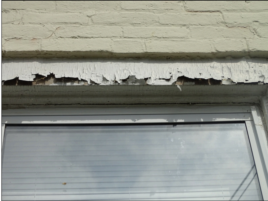
31 - Exterior window with wood framing - note peeling paint
