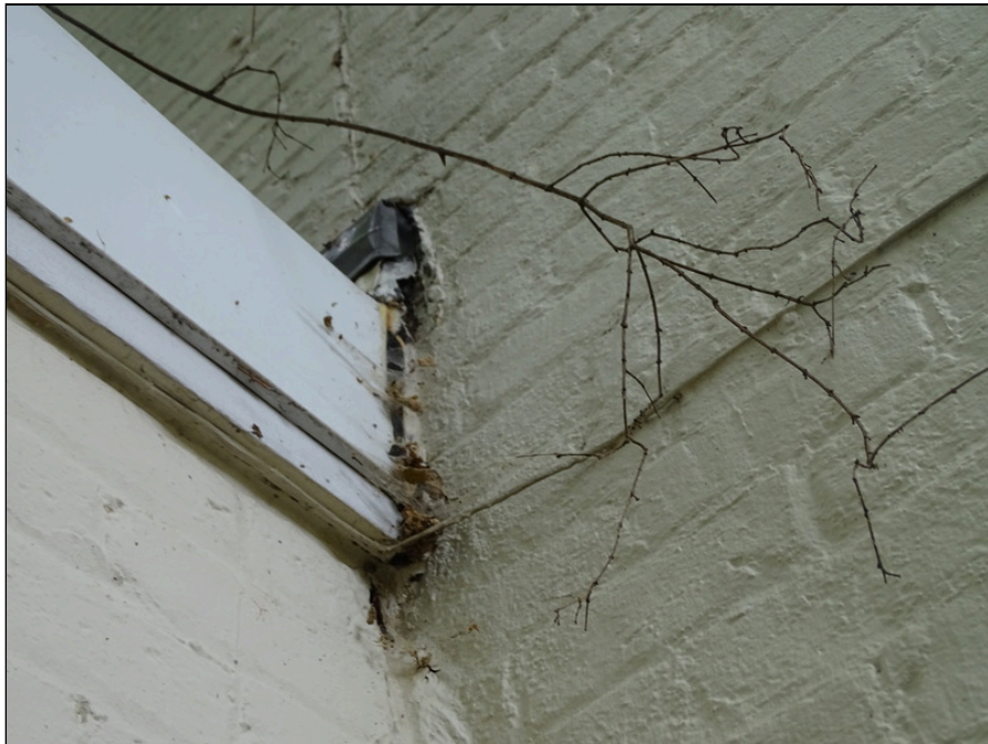
50 - Typical soffit - note deterioration
