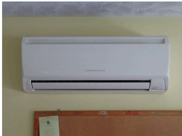
Split system wall mounted unit
