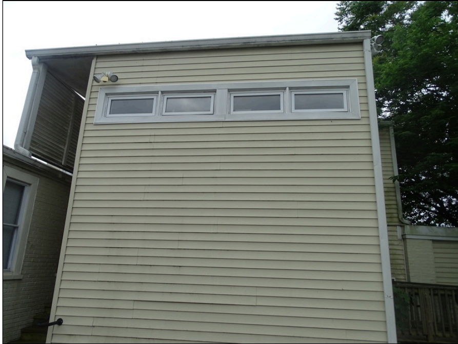
19 - Vinyl siding at north addition
