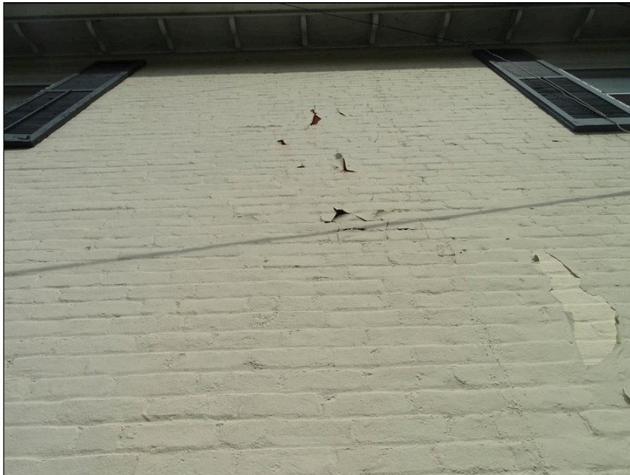
24 - Building exterior east side of the building - note peeling paint
