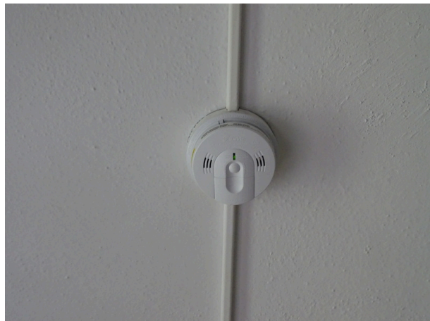
Typical smoke detector
