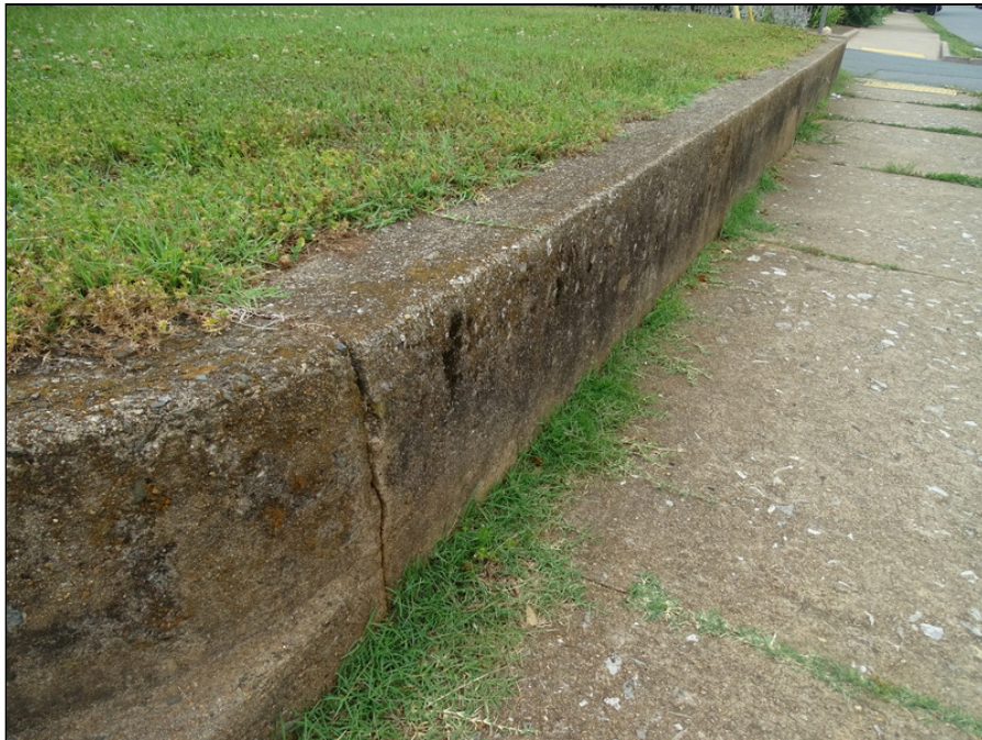
6 - Concrete ramp at south side of the building - note cracking of concrete wall
