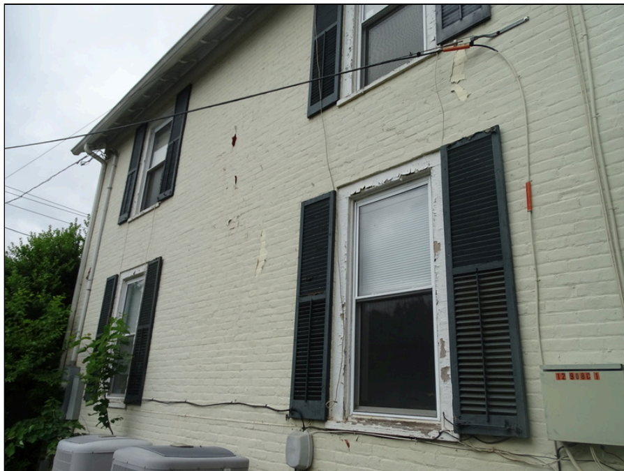
22 - Building exterior east side of the building - note peeling paint
