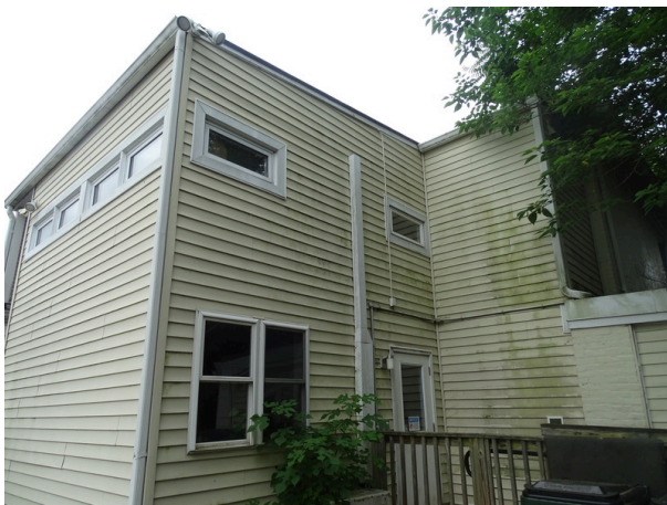
Vinyl siding at north addition
