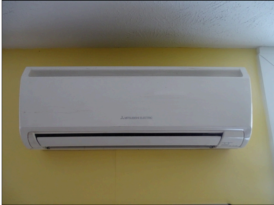
57 - Split system wall mounted unit
