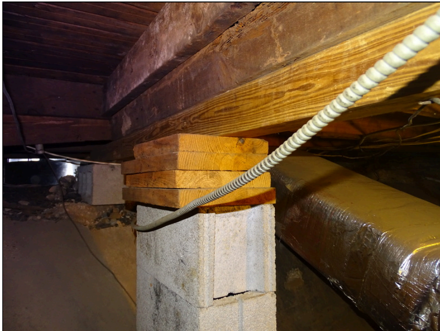
14 - Structural framing - note CMU column deterioration
