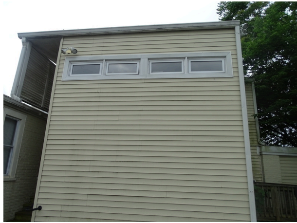
Vinyl siding at north addition
