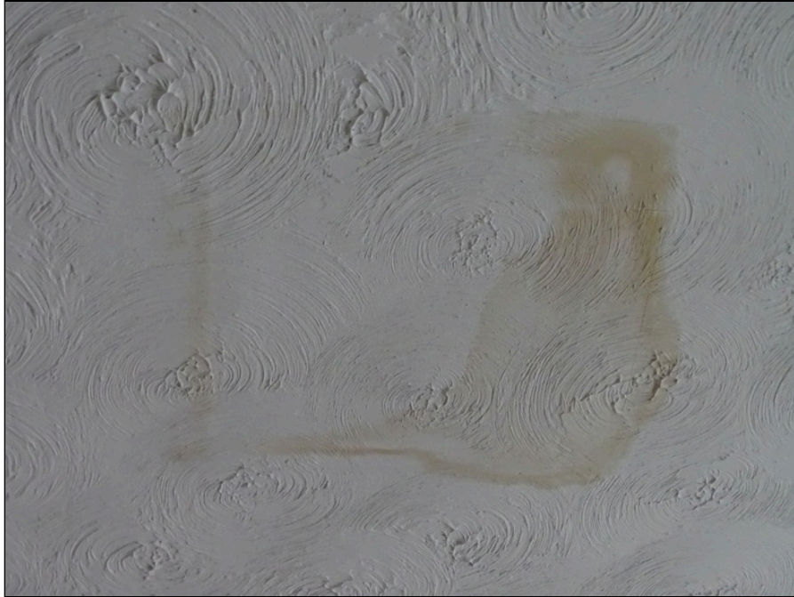
41 - Reported leakage of roofing system
