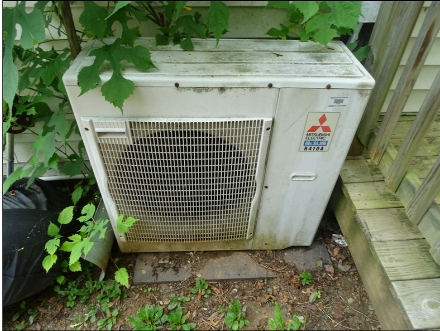
55 - Split system exterior condenser
