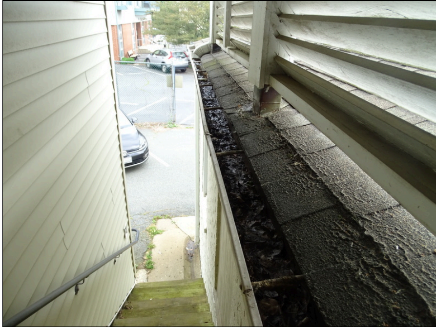
43 - Gutter - note deterioration
