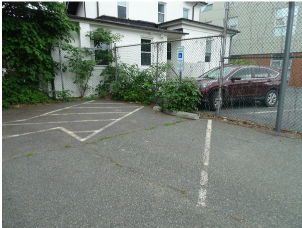
Accessible parking north side of the building - note stripping faded
