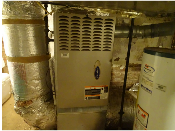
Gas furnace - air handler unit
