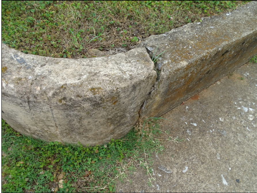
5 - Concrete curb driveway at south side - note cracking of concrete
