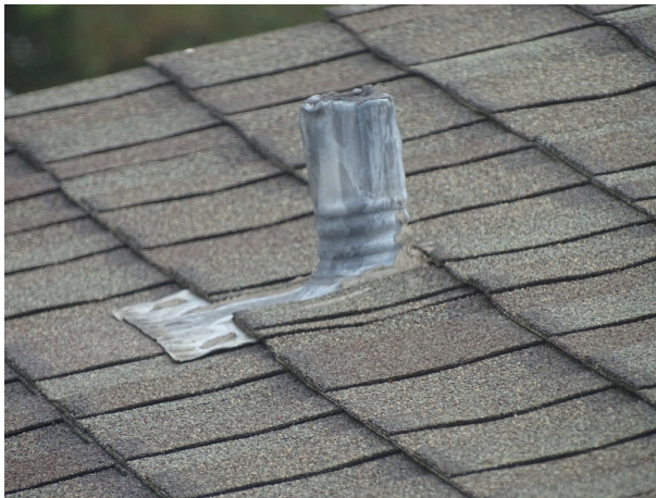
Typical plumbing penetration
