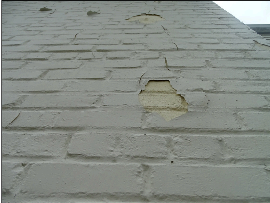
23 - Building exterior east side of the building - note peeling paint
