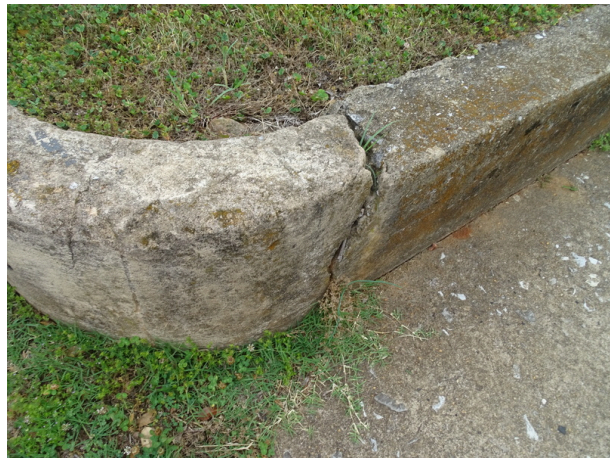
Concrete curb driveway at south side - note cracking of concrete
