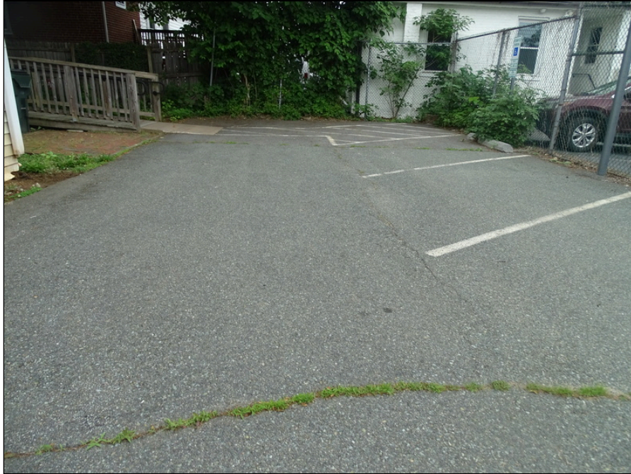
3 - Asphalt parking north side of the building - note cracking
