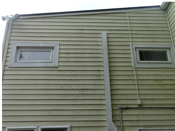
Vinyl siding at north addition - note needed maintenance
