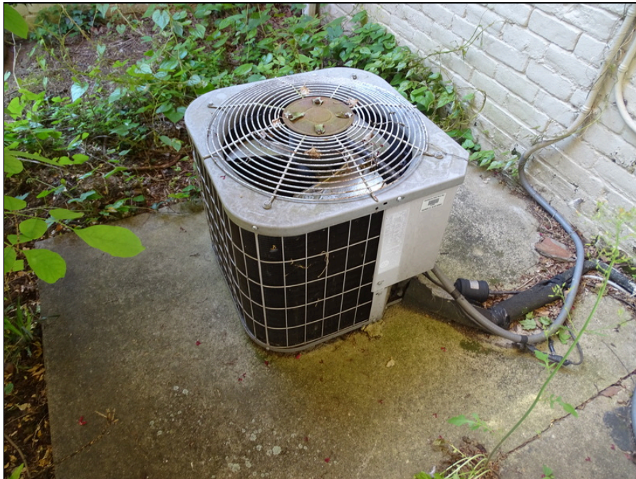
28 - Typical condenser unit
