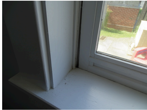
Exterior window - note operation of window difficult
