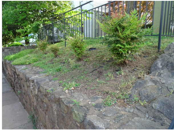
Retaining wall - note mortar deterioration
