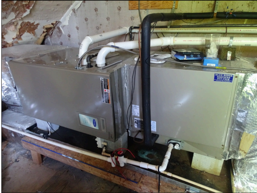
29 - Typical furnace unit and air handler
