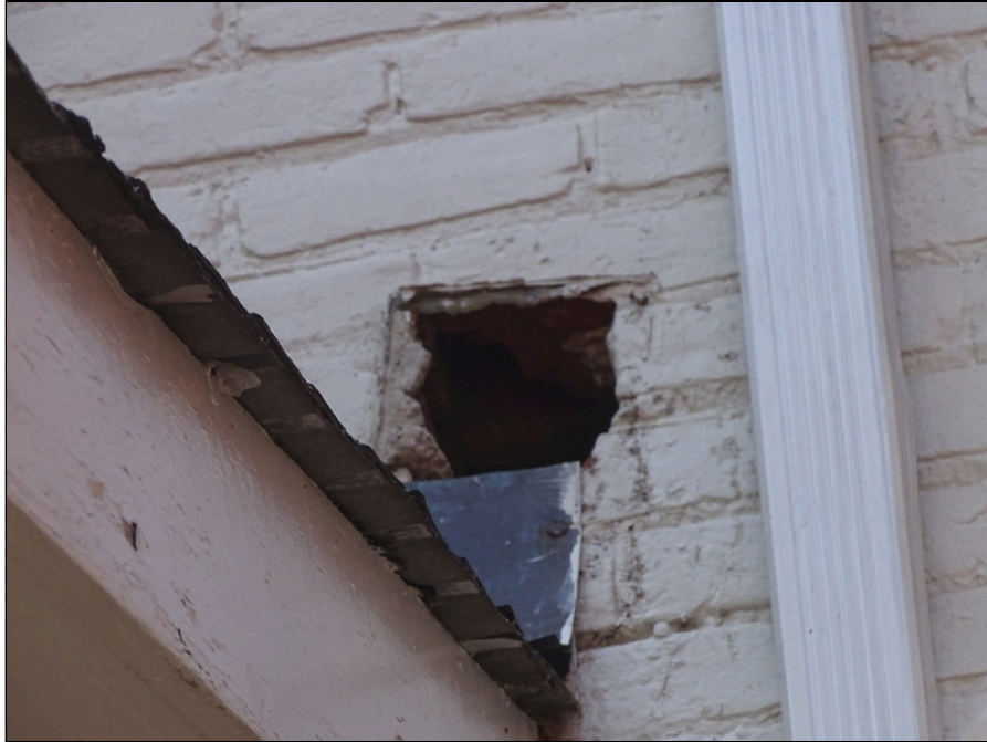
17 - Building exteriors north side of the building - note penetration in exterior needing repair
