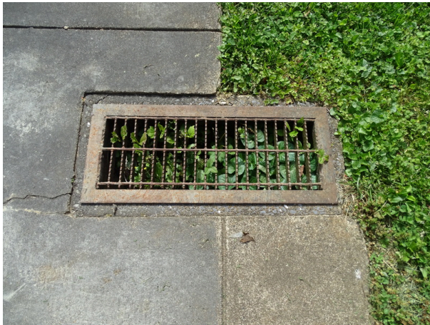
Typical yard drop inlet
