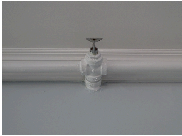
Fire sprinkler piping and head
