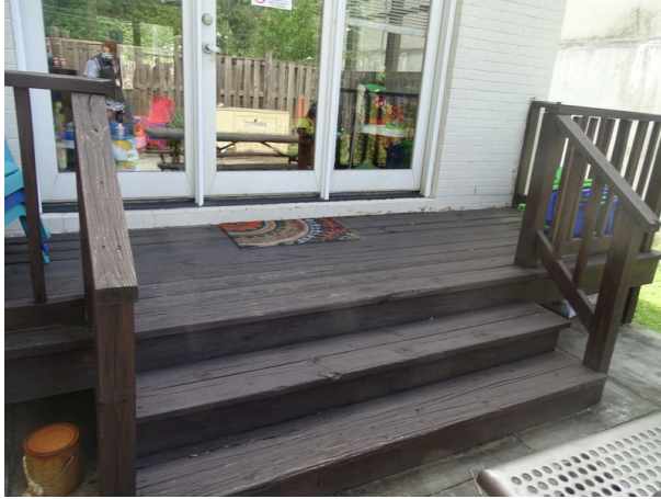
Wood deck on south side of building - note deterioration and railing loose
