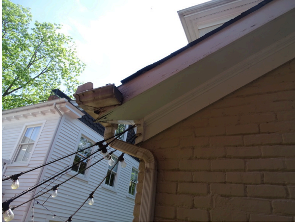
Building exteriors west side of the building - note deterioration of wood trim
