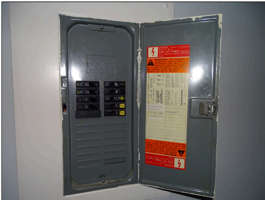
34 - Typical older circuit breaker panel
