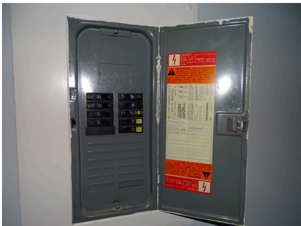
Typical older circuit breaker panel
