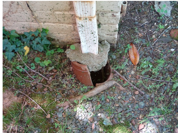
Storm drainage from gutter - note repair needed as maintenance item
