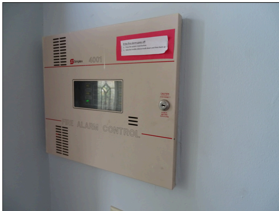
40 - Fire alarm control panel
