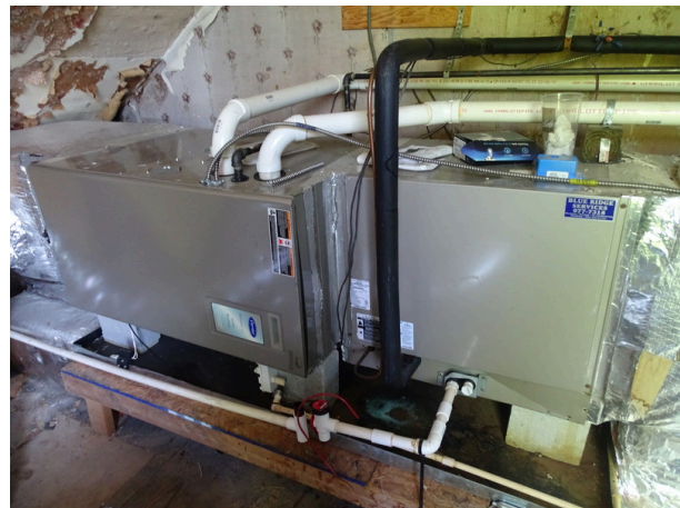
Typical furnace unit and air handler
