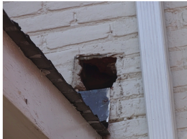
Building exteriors north side of the building - note penetration in exterior needing repair
