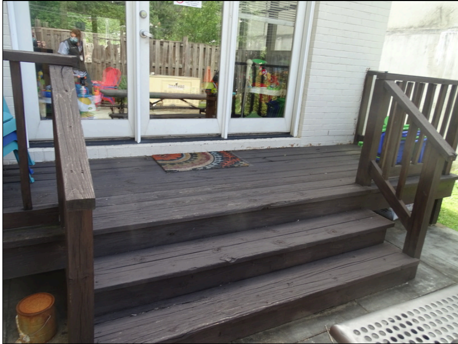
9 - Wood deck on south side of building - note deterioration and railing loose
