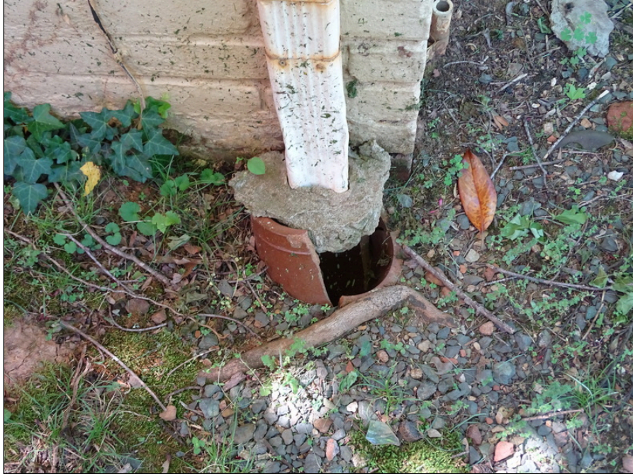
3 - Storm drainage from gutter - note repair needed as maintenance item
