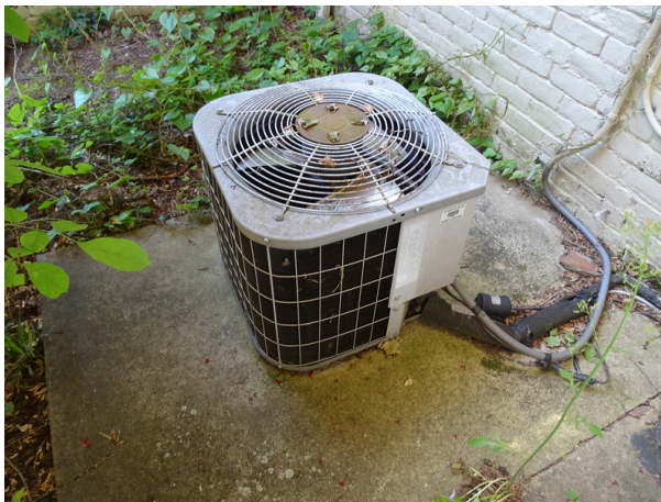
Typical condenser unit
