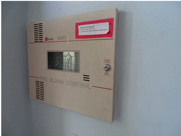
Fire alarm control panel
