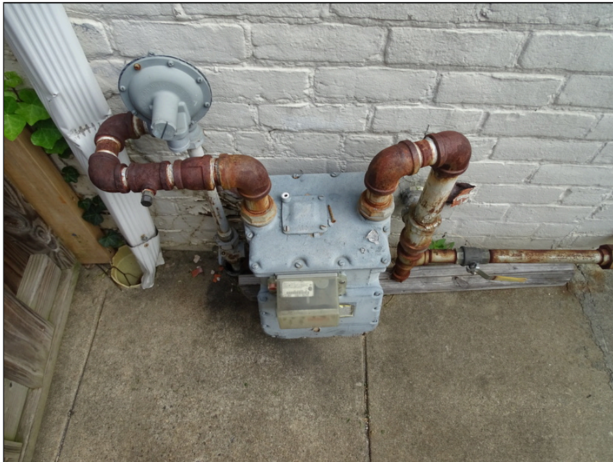
26 - Natural gas utility supply and meter
