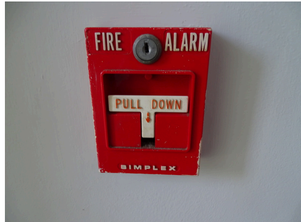
Fire alarm pull station
