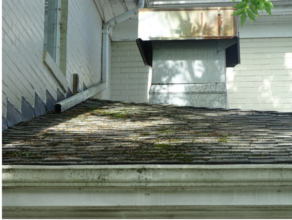
Roofing system - note deterioration
