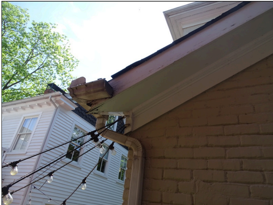
18 - Building exteriors west side of the building - note deterioration of wood trim
