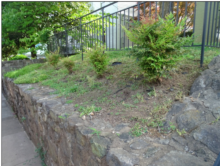
8 - Retaining wall - note mortar deterioration
