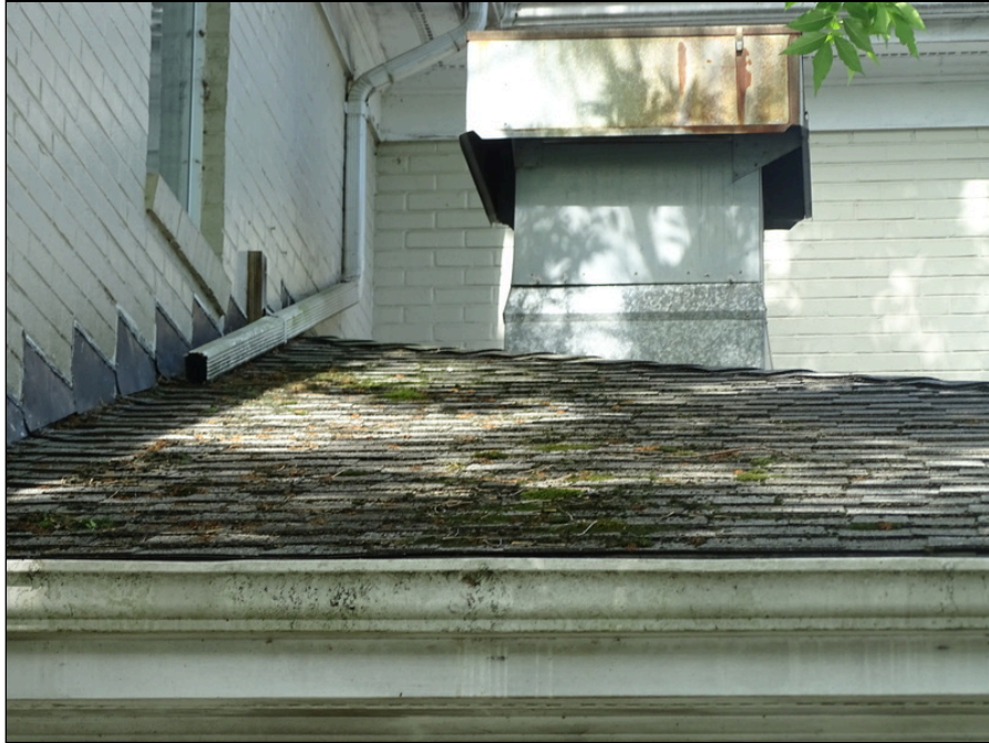
25 - Roofing system - note deterioration
