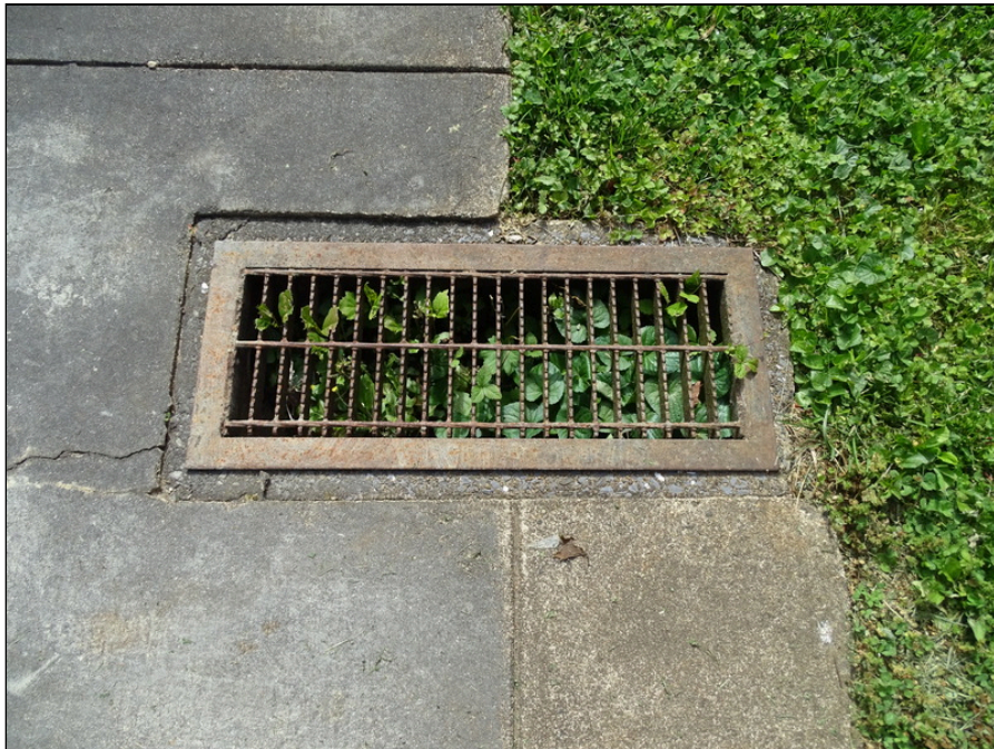
2 - Typical yard drop inlet
