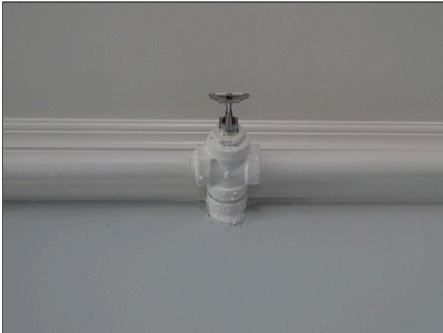
38 - Fire sprinkler piping and head
