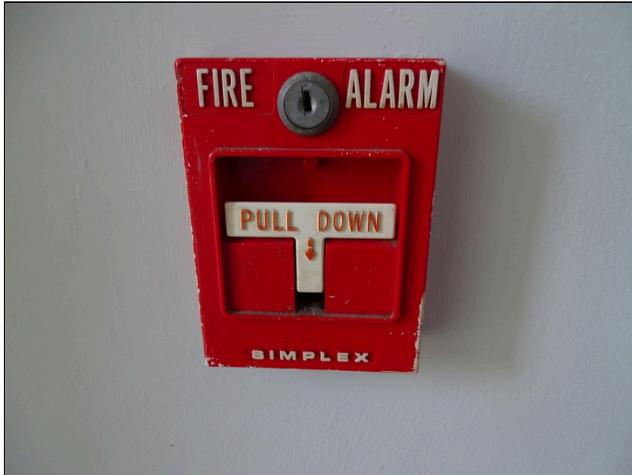
41 - Fire alarm pull station
