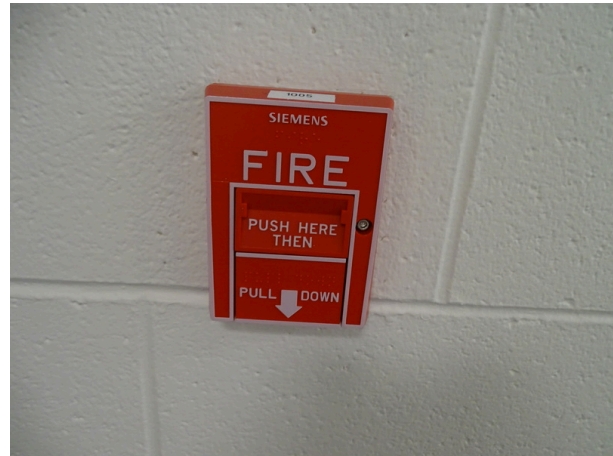
Typical Pull down station
