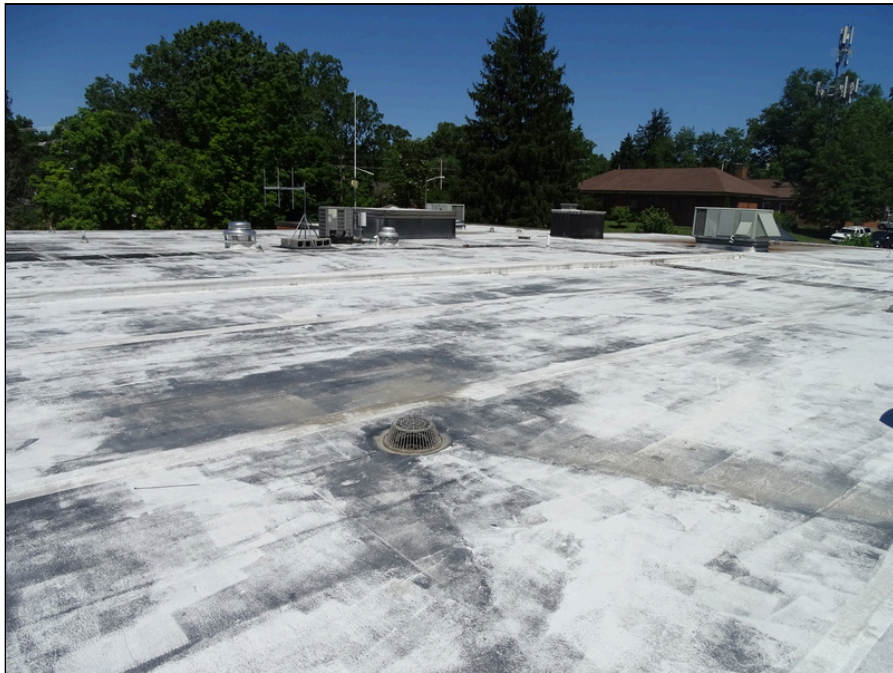
34 - Single-ply roofing system side of the building - note deterioration
