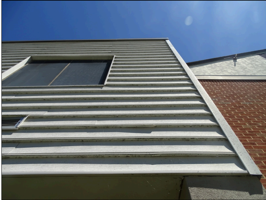
29 - Exterior wall wood siding
