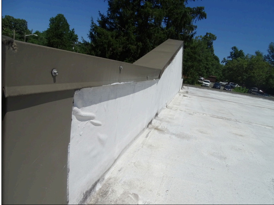
37 - Single-ply roofing system side of the building - note metal coping
