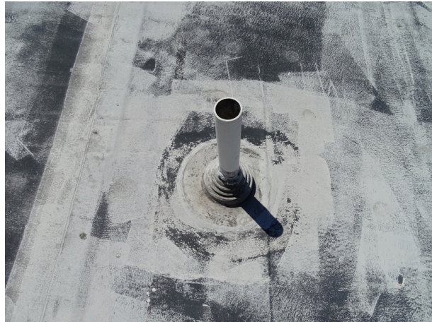
Single-ply roofing system side of the building - note plumbing penetration
