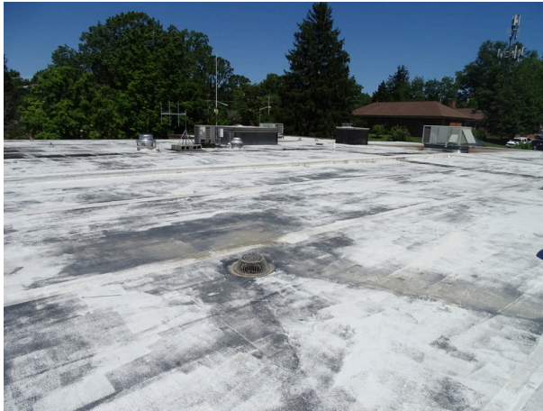
Single-ply roofing system side of the building - note deterioration
