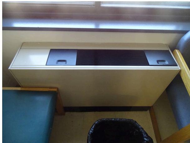
Typical Water Source Heat Pump
