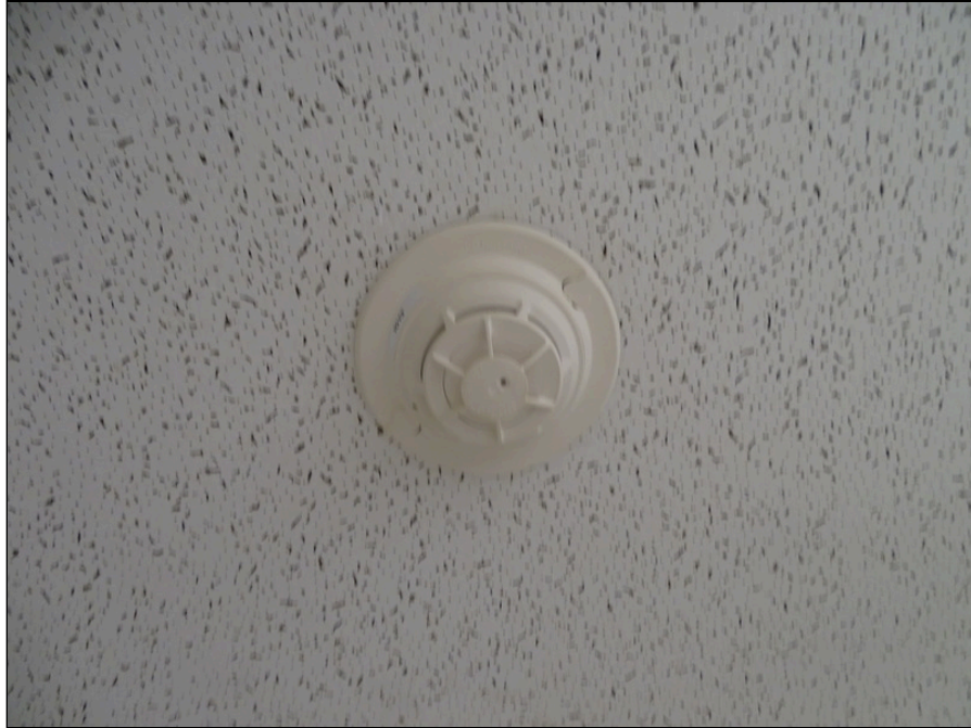
73 - Typical smoke detector
