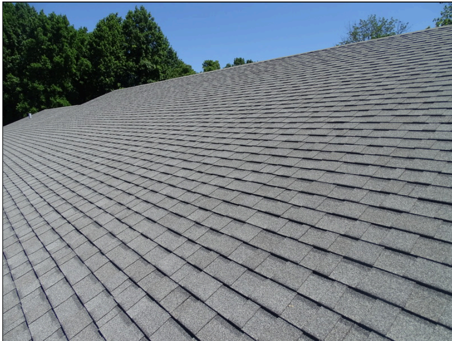
38 - Asphalt shingle roofing
