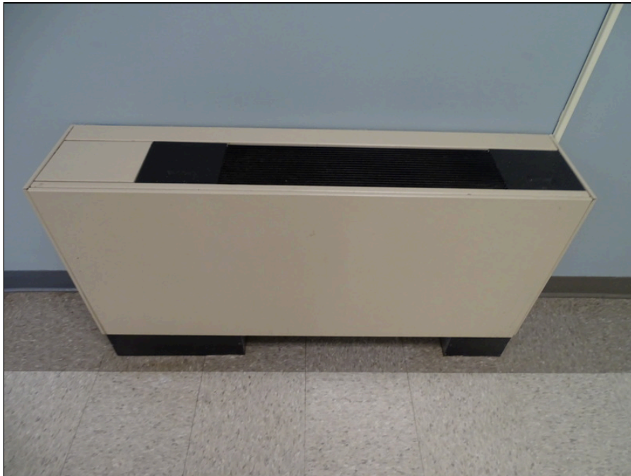
52 - Typical Water Source Heat Pump
