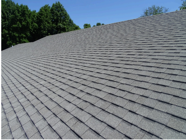
Asphalt shingle roofing
