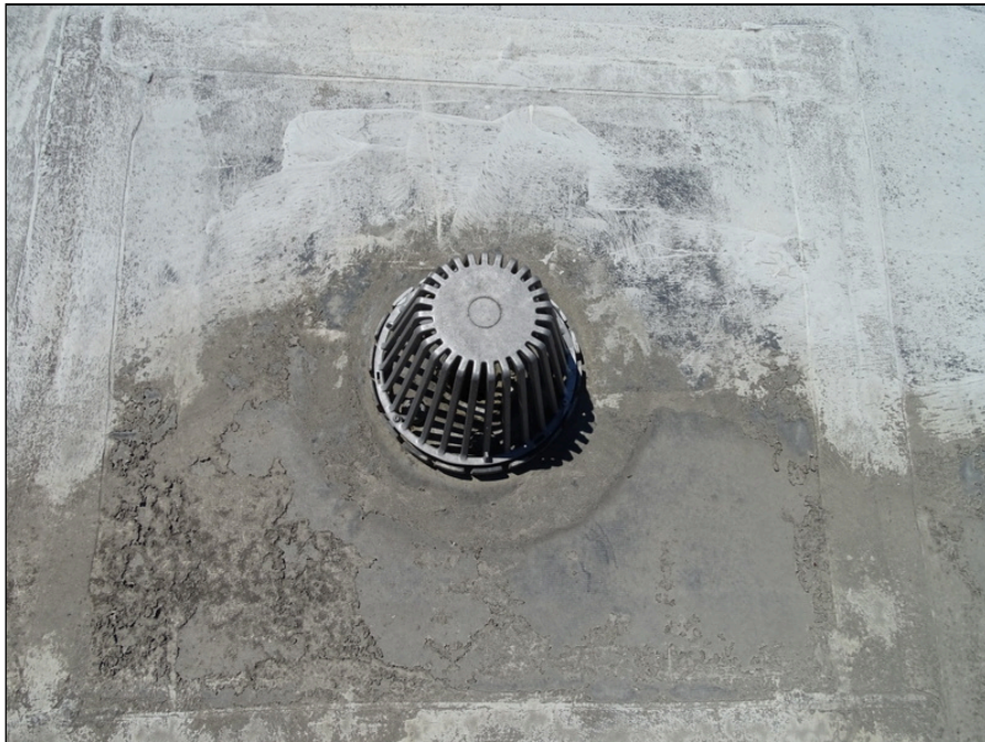
36 - Single-ply roofing system side of the building - note internal drain
