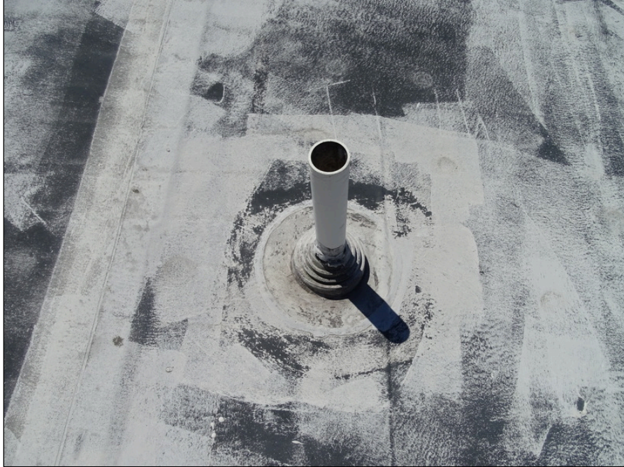
35 - Single-ply roofing system side of the building - note plumbing penetration
