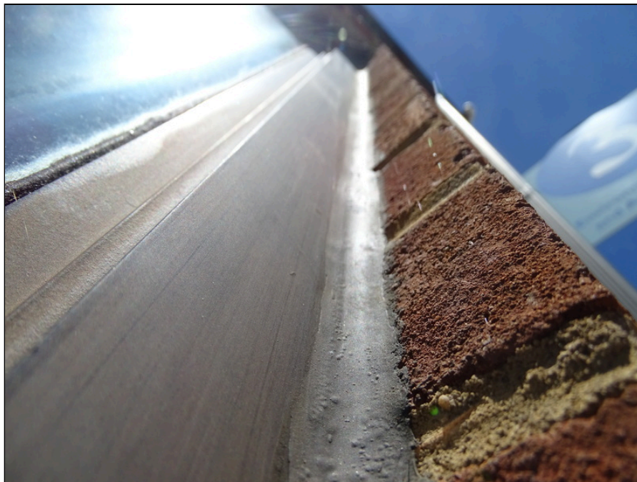
32 - Exterior window finishes - note sealant condition
