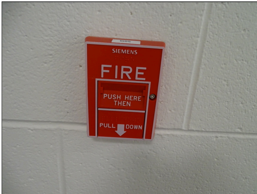
72 - Typical Pull down station
