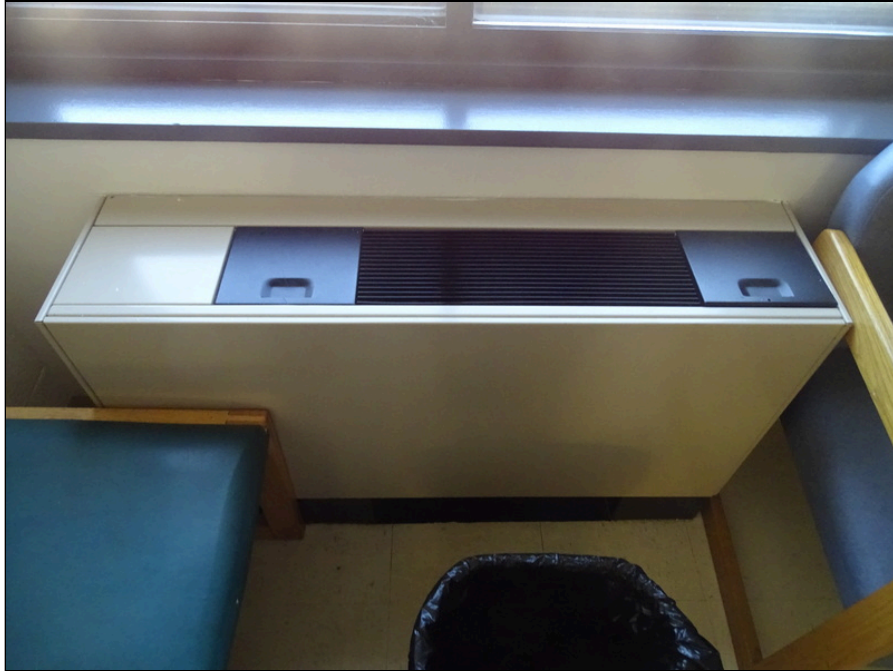
51 - Typical Water Source Heat Pump
