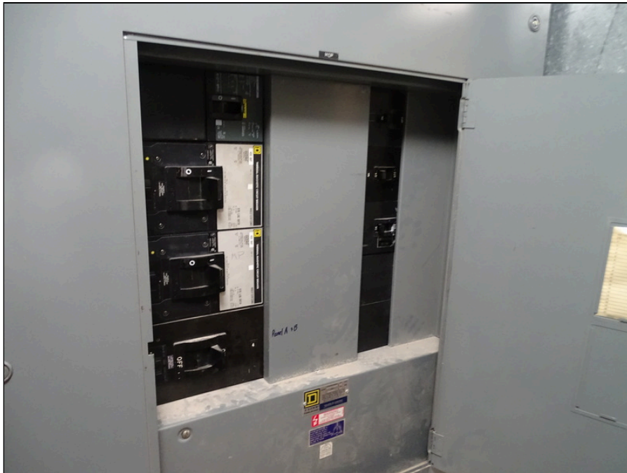
62 - Main electrical switchgear
