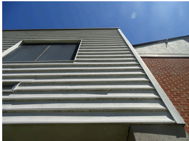
Exterior wall wood siding
