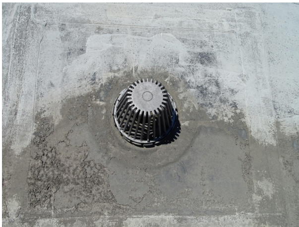
Single-ply roofing system side of the building - note internal drain
