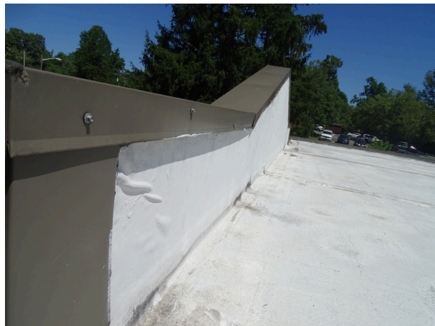
Single-ply roofing system side of the building - note metal coping
