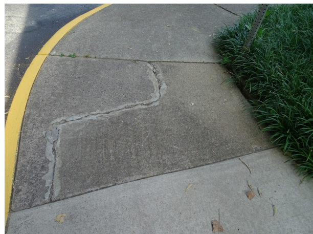
Concrete curb ramp - note cracking
