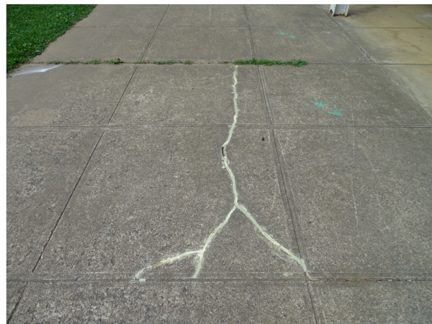
Concrete pavement - note sealant
