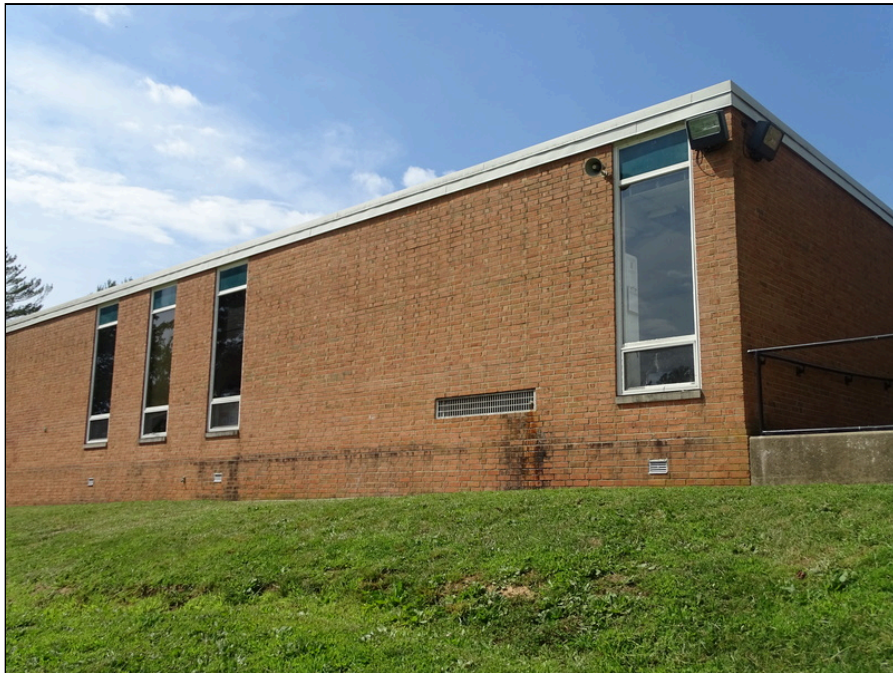
42 - Exterior overview - note efflorescence
