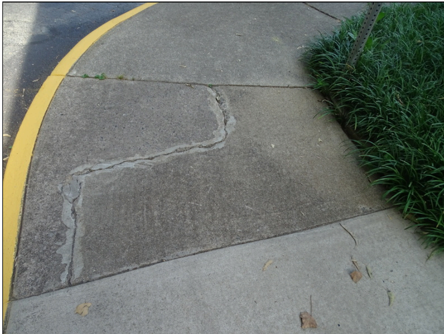
16 - Concrete curb ramp - note cracking
