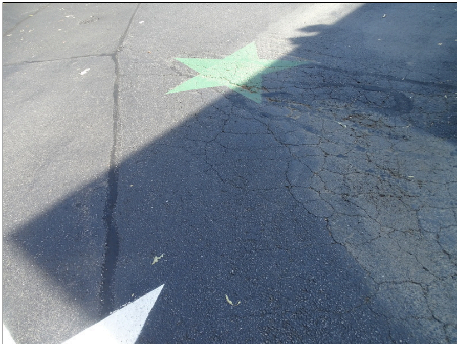
8 - Alligator cracking in asphalt pavement
