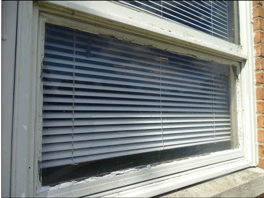
51 - Deteriorated window sealant
