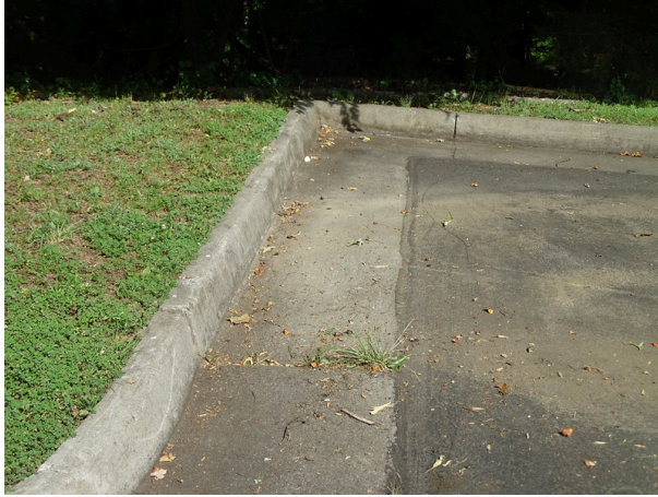
Concrete curb - note cracking
