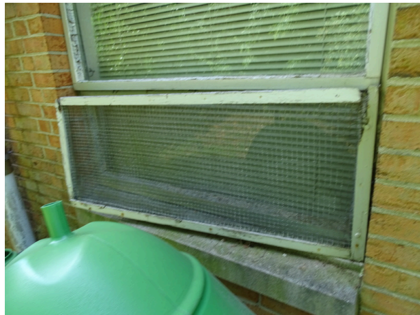
Deteriorated window sealant and glazing
