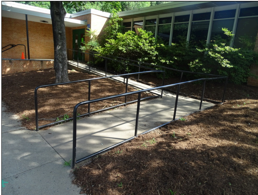
134 - Accessible concrete ramp
