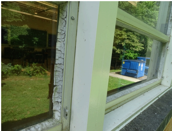
Deteriorated window sealant and glazing
