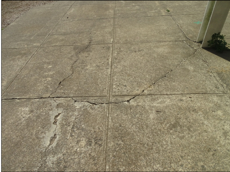
15 - Concrete sidewalk - cracking
