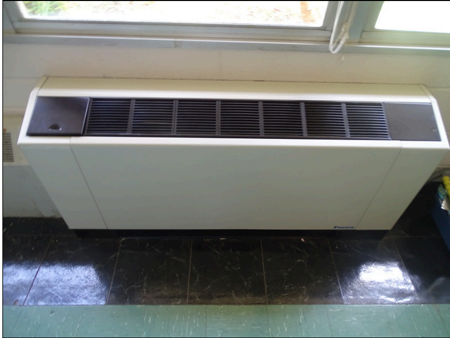
73 - Water source heat pump
