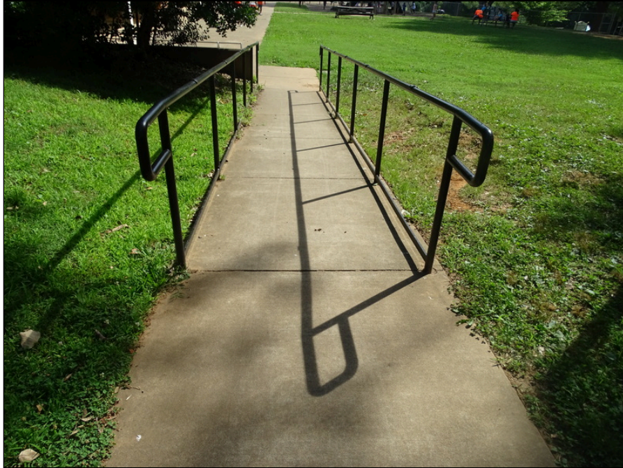
135 - Accessible concrete ramp
