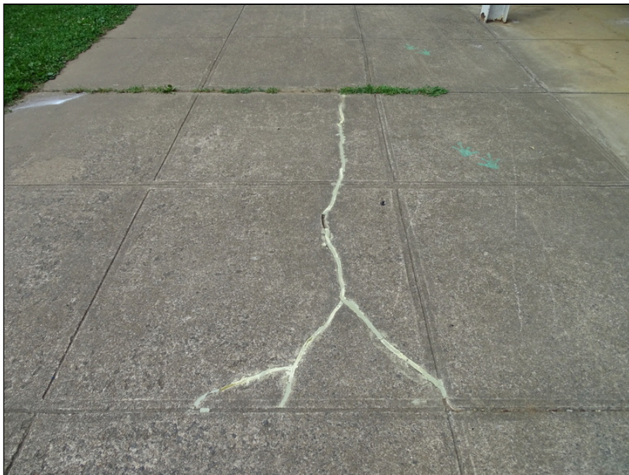
14 - Concrete pavement - note sealant
