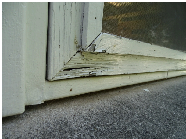
Deteriorated window sealant and glazing
