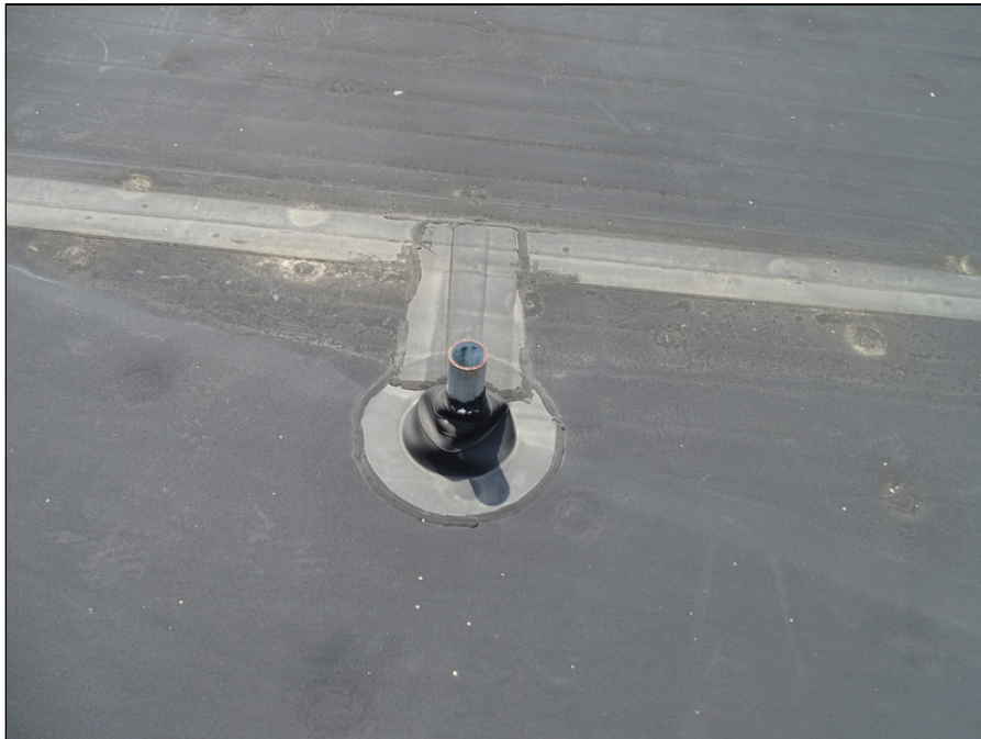
66 - Typical penetration pipe
