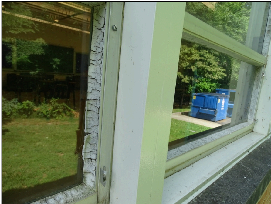
52 - Deteriorated window sealant and glazing
