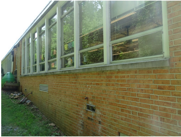
Exterior overview - note efflorescence
