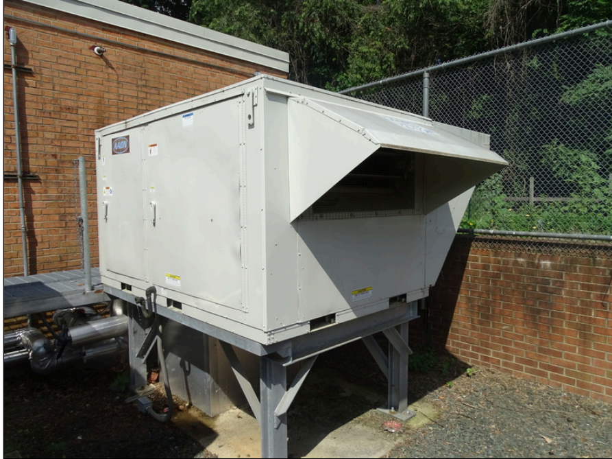
71 - Air handler at building exterior
