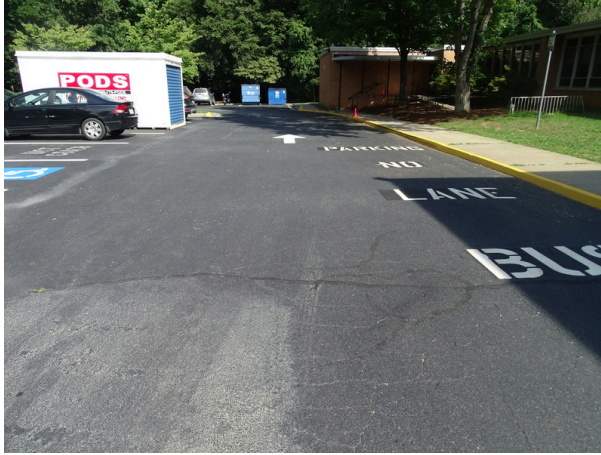
Previous repair of asphalt pavement
