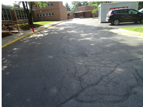
Alligator cracking in asphalt pavement
