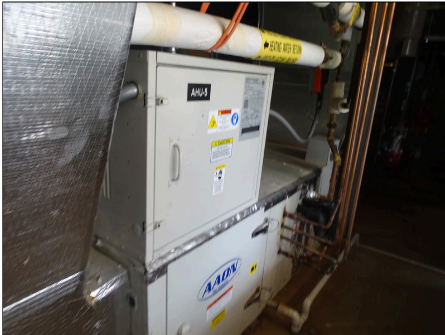
70 - Air handler in mechanical room
