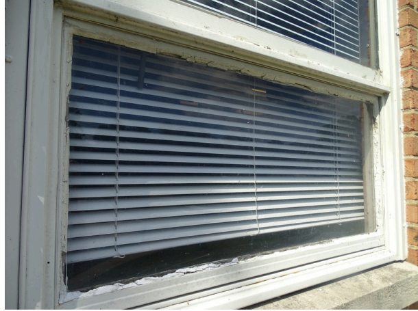
Deteriorated window sealant
