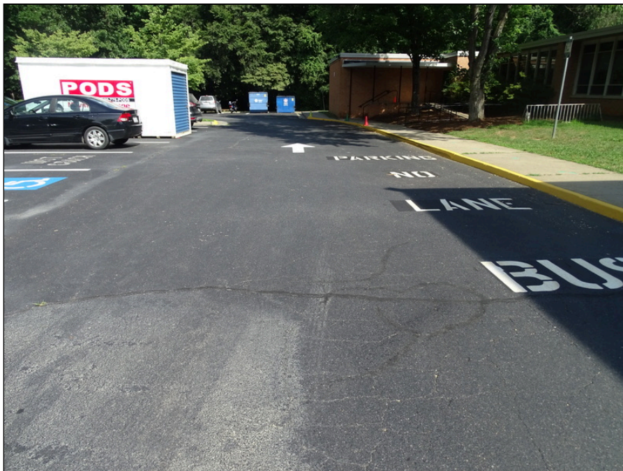
10 - Previous repair of asphalt pavement
