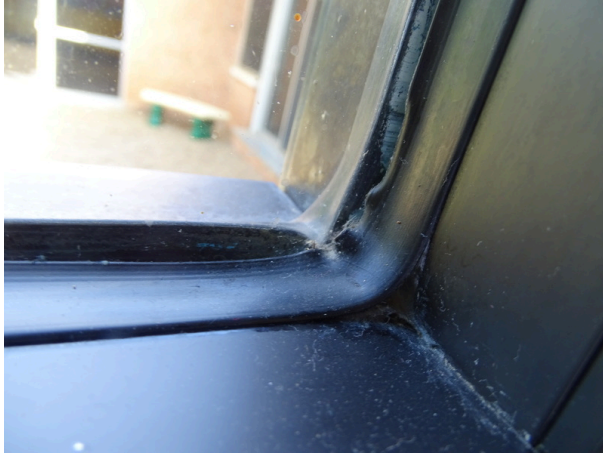
Deteriorated window glazing
