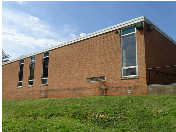
Exterior overview - note efflorescence
