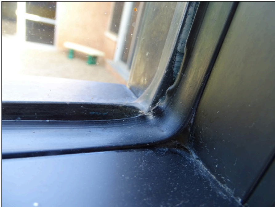
50 - Deteriorated window glazing
