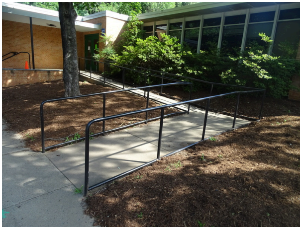
Accessible concrete ramp
