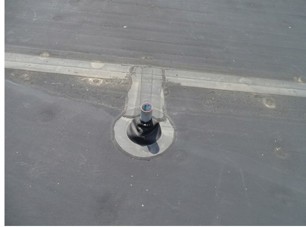
Typical penetration pipe
