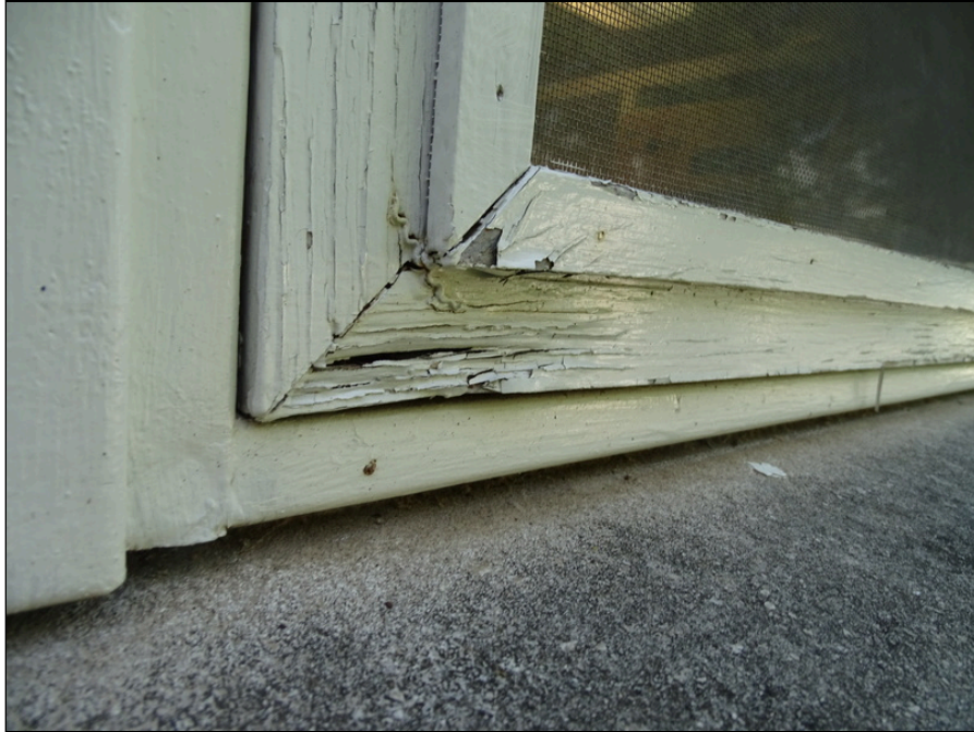
49 - Deteriorated window sealant and glazing
