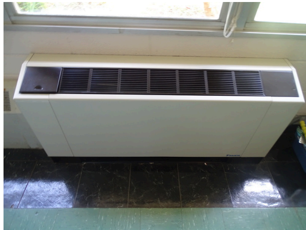
Water source heat pump
