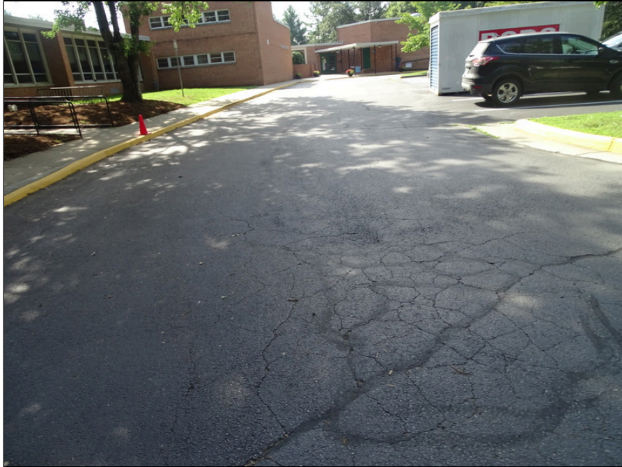
9 - Alligator cracking in asphalt pavement
