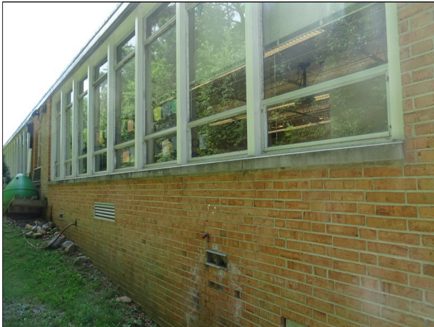
44 - Exterior overview - note efflorescence
