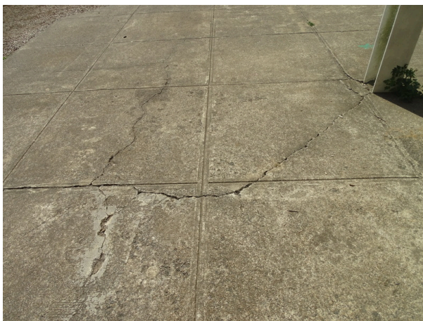
Concrete sidewalk - cracking
