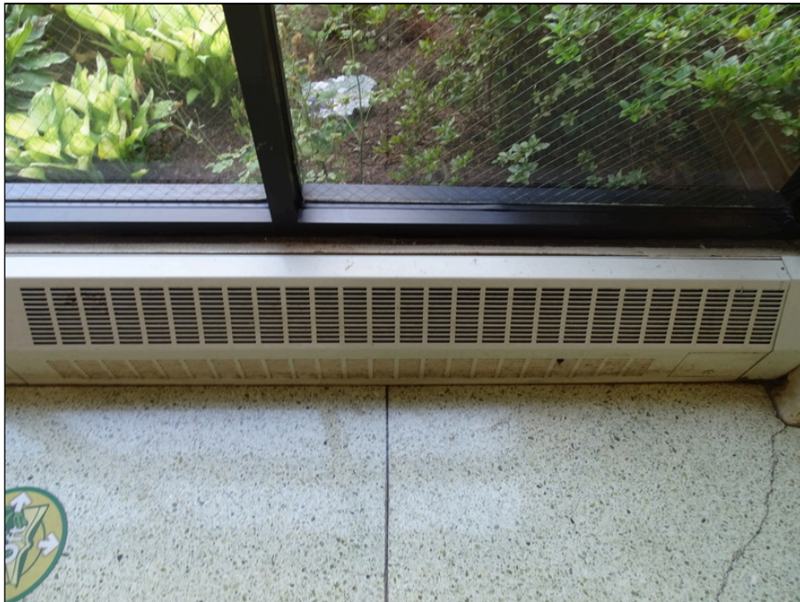
74 - Water source heat pumps
