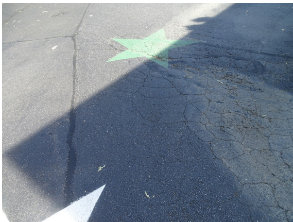
Alligator cracking in asphalt pavement
