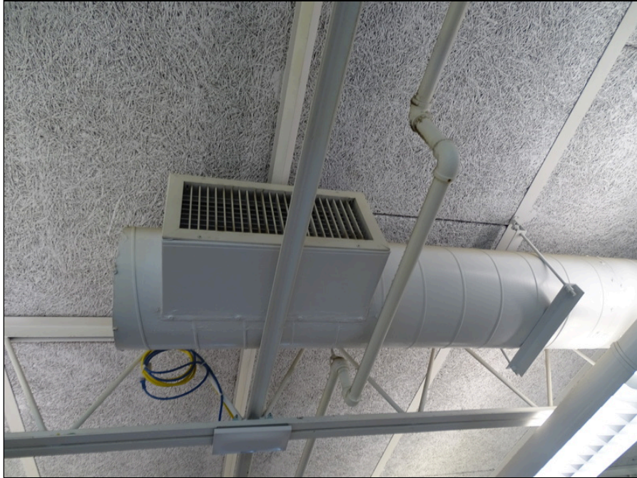
83 - Exposed ductwork
