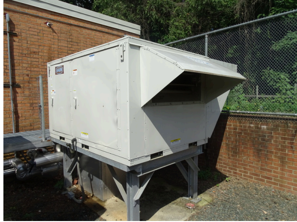
Air handler at building exterior
