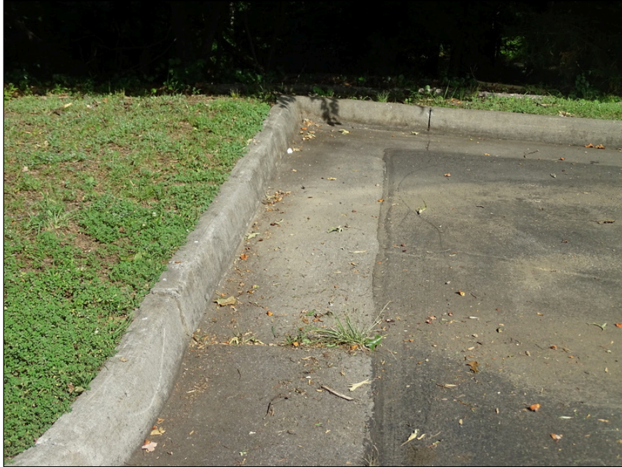
17 - Concrete curb - note cracking
