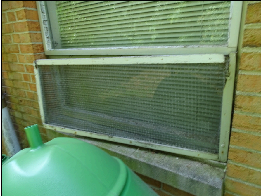
53 - Deteriorated window sealant and glazing
