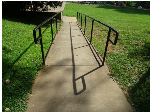
Accessible concrete ramp
