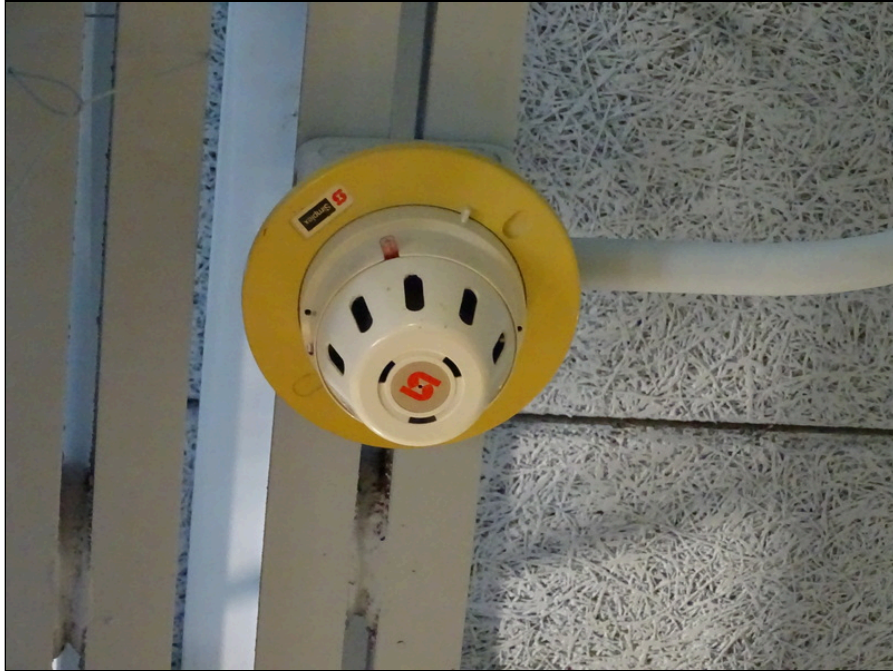
53 - Typical smoke detector
