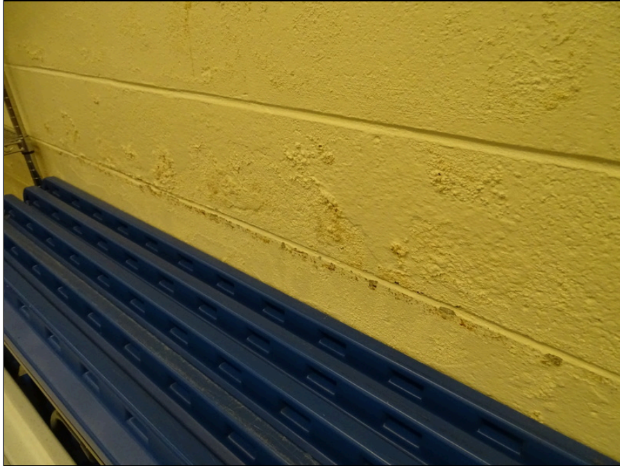
67 - Interior wall - note efflorescence
