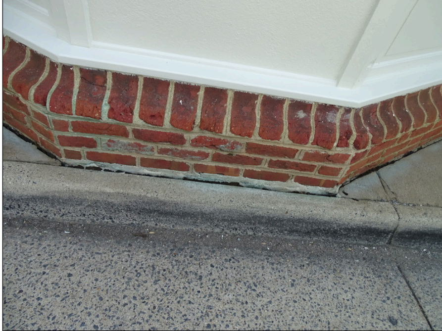
73 - Brick at bay - note deterioration
