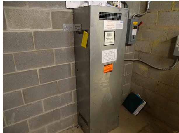
Elevator machine and controls
