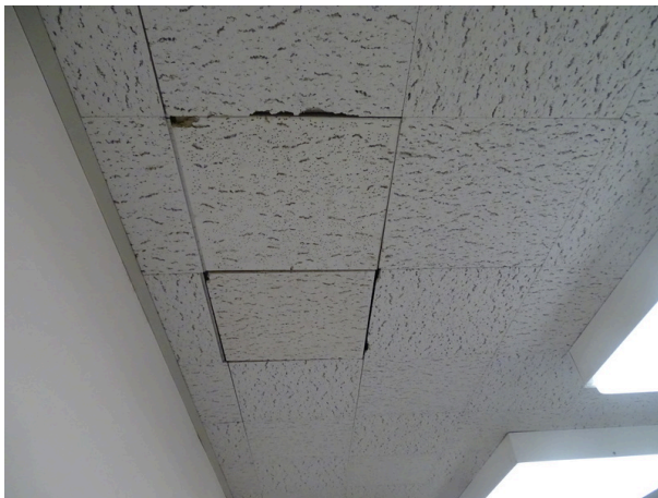
Typical acoustical tile - note deterioration
