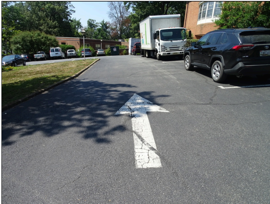
4 - Asphalt pavement north side of the site - note cracking
