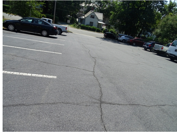
Asphalt pavement east side of the site - note cracking
