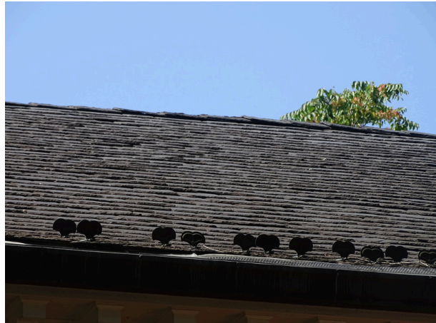
Slate shingle roofing system - note deterioration
