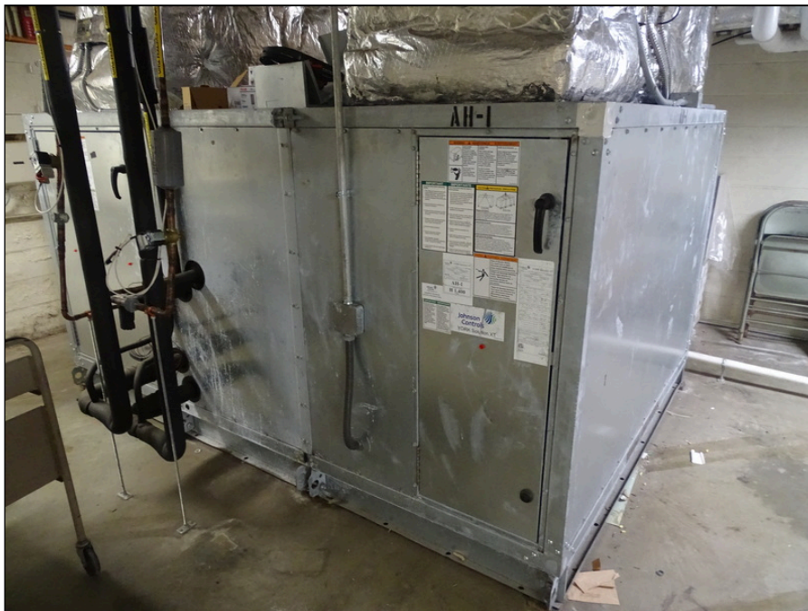
36 - Air Handler Unit located in main utility room
