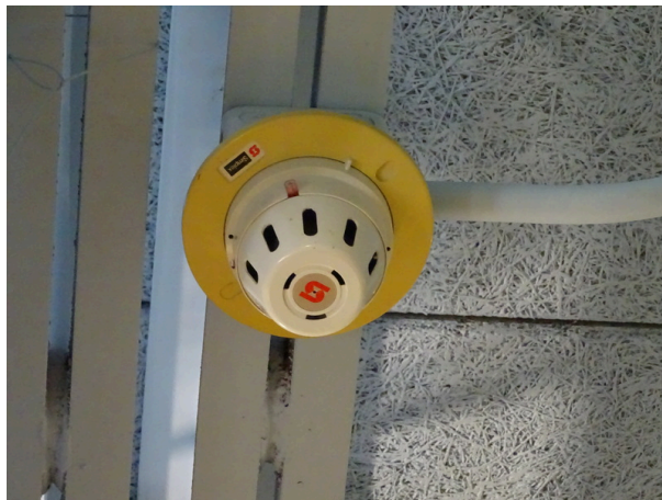
Typical smoke detector
