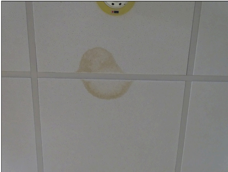
32 - Water leakage at ceiling
