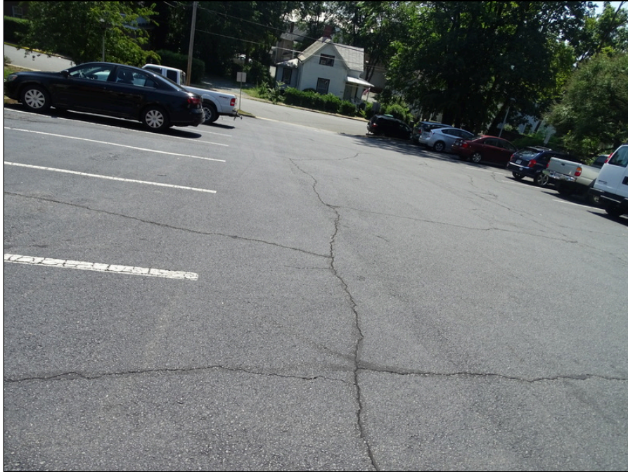
3 - Asphalt pavement east side of the site - note cracking
