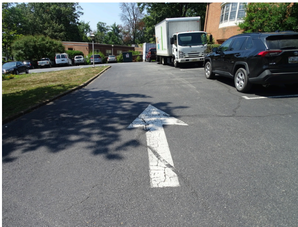
Asphalt pavement north side of the site - note cracking
