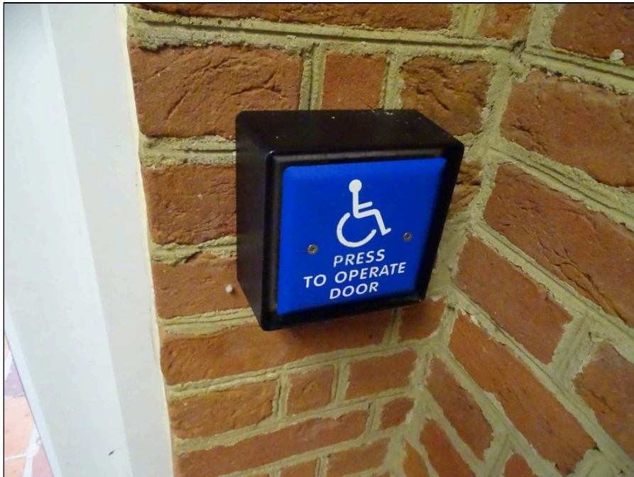
70 - Accessible door controls at main entrance
