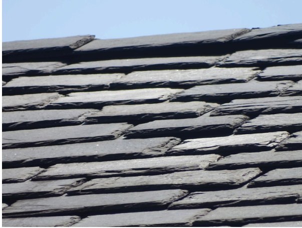
Slate shingle roofing system - note deterioration
