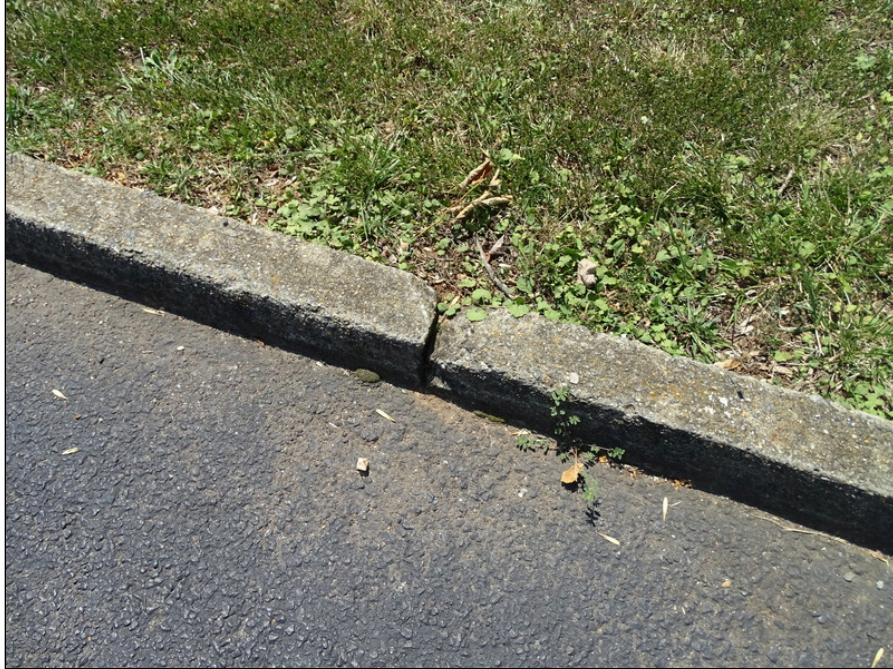
11 - Concrete curb - note deterioration
