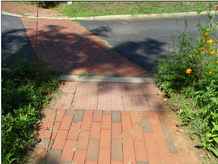
10 - Brick sidewalk with truncated domes
