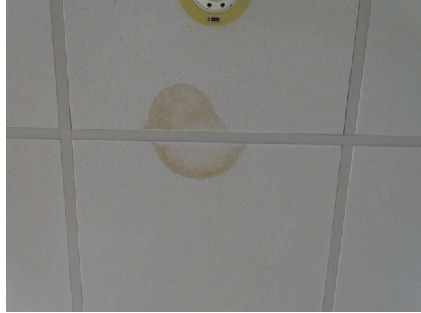
Water leakage at ceiling
