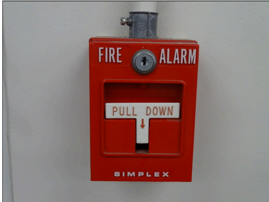
51 - Typical fire alarm pull station
