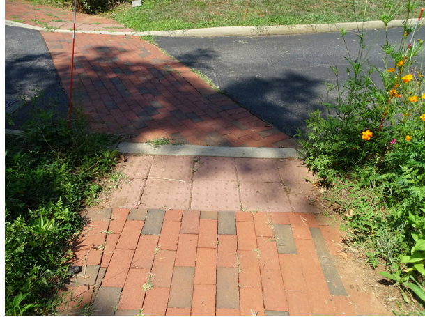
Brick sidewalk with truncated domes
