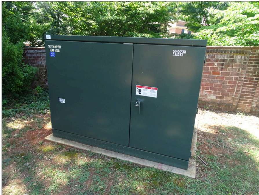
42 - Electric utility transformer
