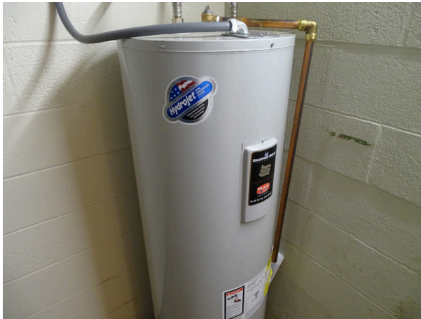
Electric domestic water heater
