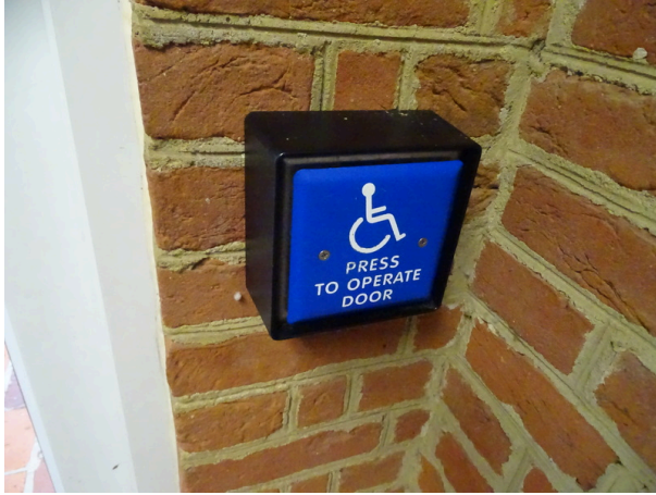
Accessible door controls at main entrance
