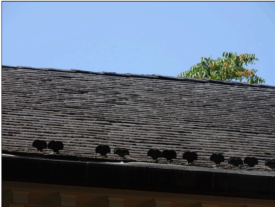
30 - Slate shingle roofing system - note deterioration
