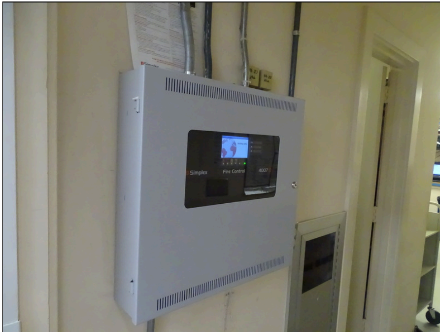
50 - Fire alarm control panel
