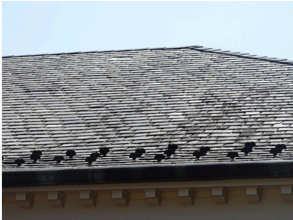
Slate shingle roofing system - note deterioration
