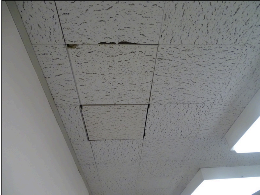
59 - Typical acoustical tile - note deterioration
