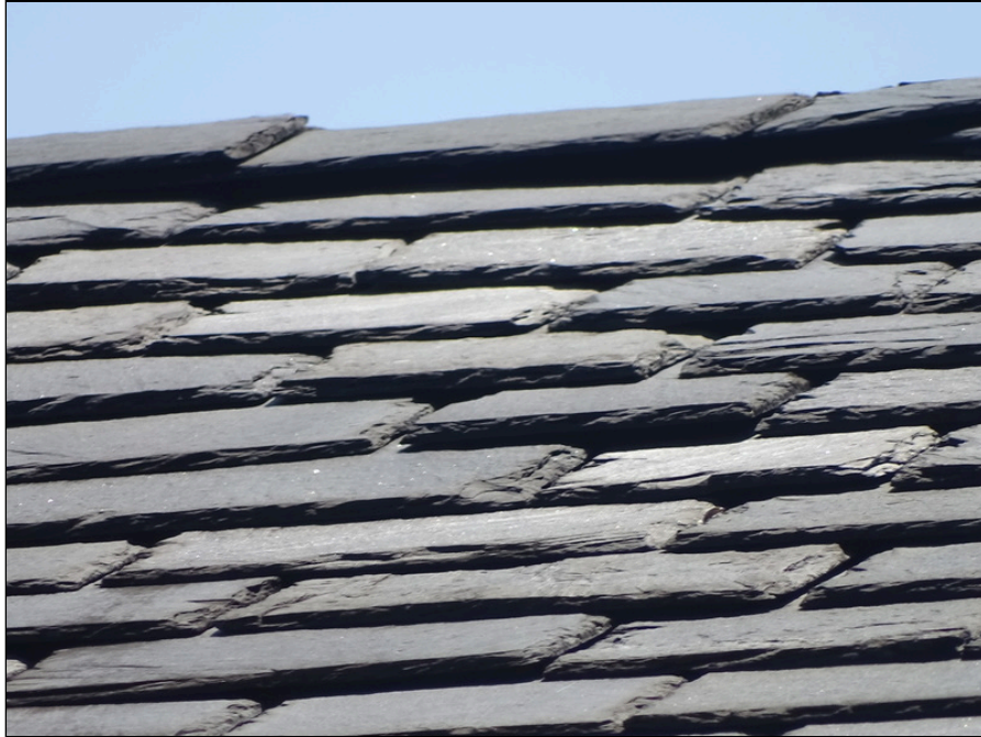
31 - Slate shingle roofing system - note deterioration
