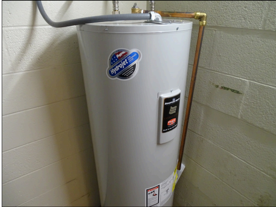
33 - Electric domestic water heater
