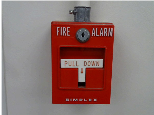
Typical fire alarm pull station
