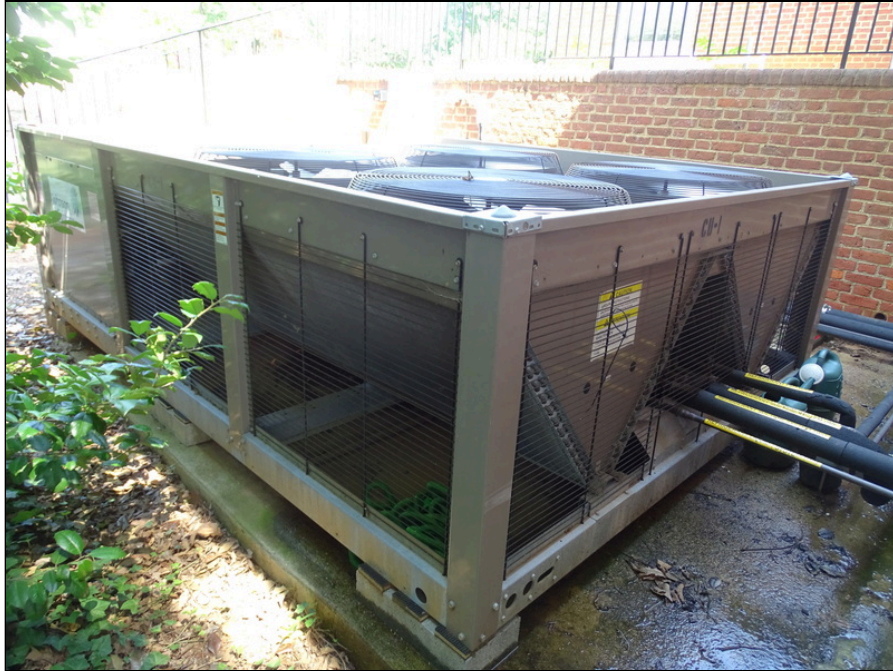
35 - Condenser Unit located at southwest side of the building
