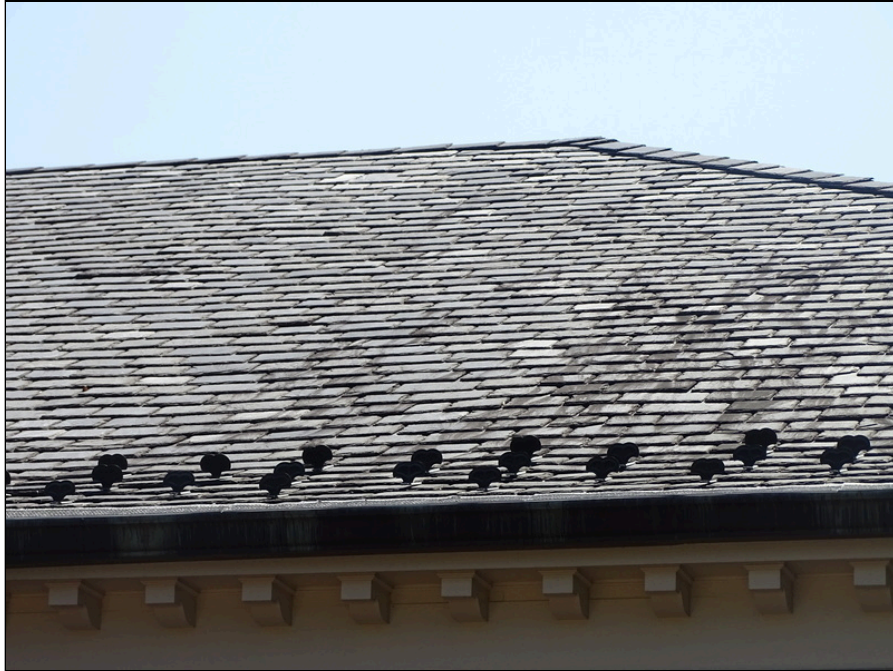
29 - Slate shingle roofing system - note deterioration
