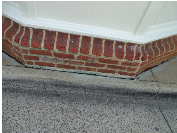
Brick at bay - note deterioration
