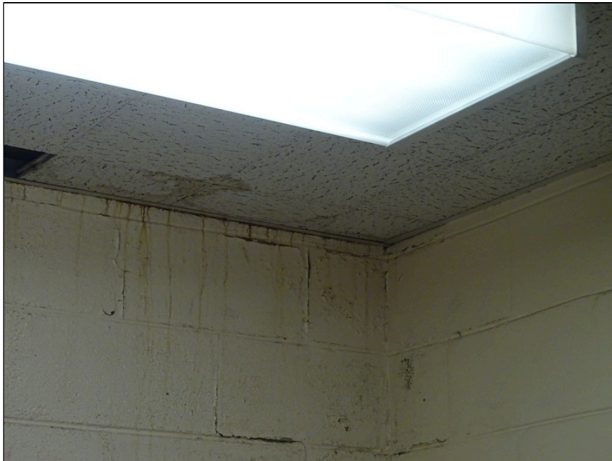
66 - Interior wall - note efflorescence
