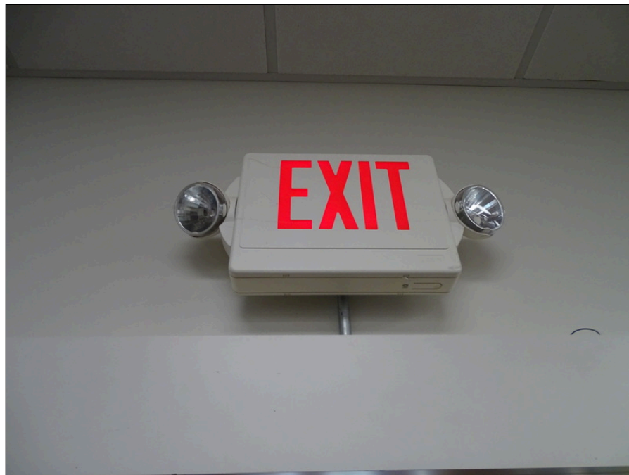
52 - Typical exit sign and emergency lighting
