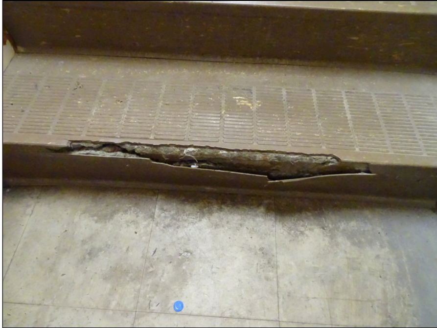
65 - Typical step - note deterioration
