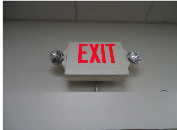
Typical exit sign and emergency lighting
