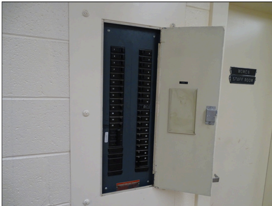
44 - Typical electrical circuit breaker panel
