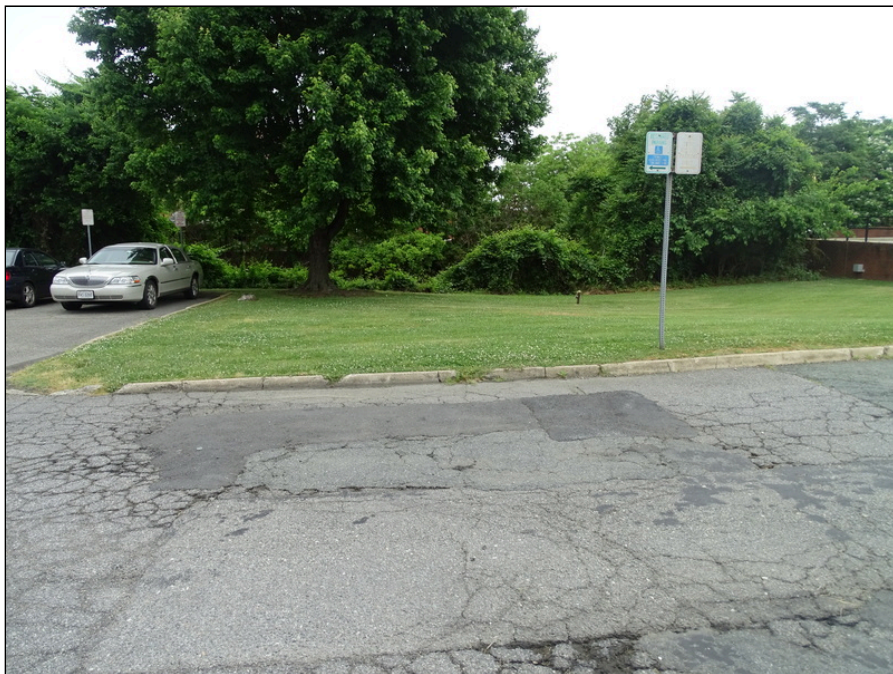
12 - Asphalt paving drive lane and parking northwest side of the building - note alligator cracking
