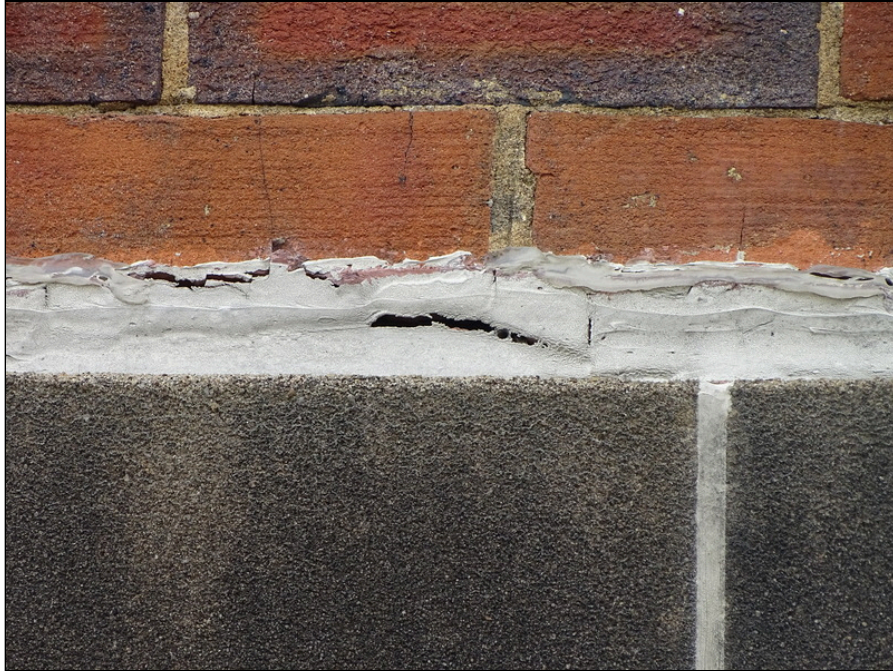
31 - Typical sealant condition
