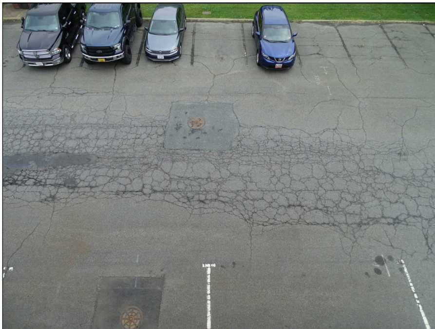
10 - Asphalt paving drive lane and parking northwest side of the building - note alligator cracking
