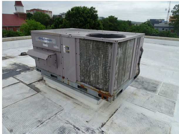
Condenser located on roof - manufactured by Carrier in 2006
