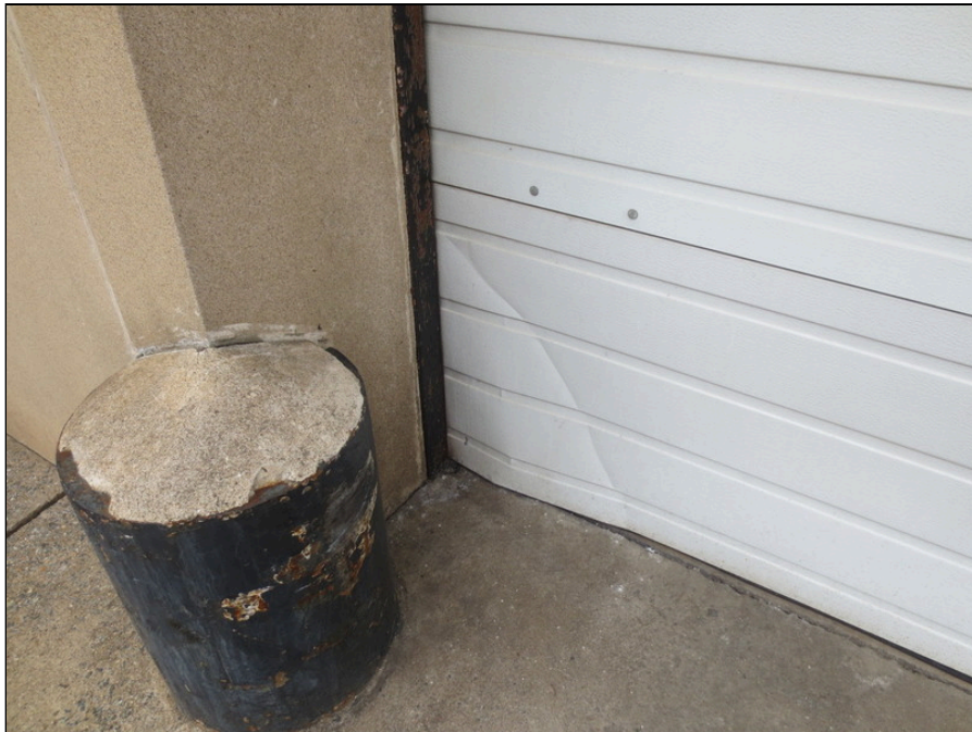
98 - Overhead door damage east
