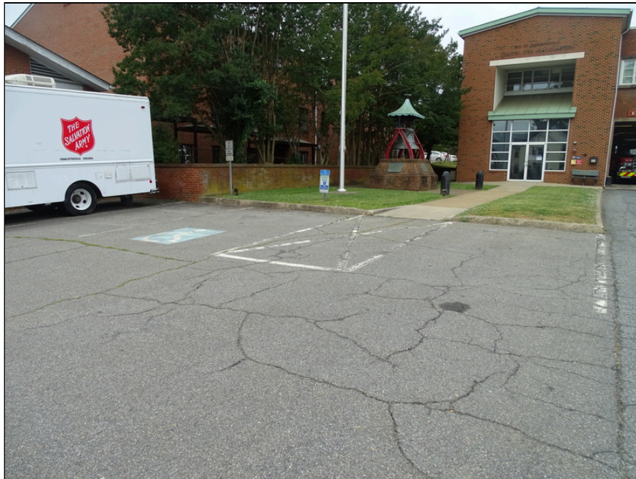
96 - Accessible parking space - note one space provided when two are required
