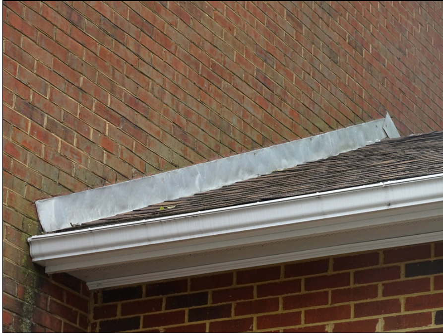
51 - Asphalt shingle roofing system over west addition - note recent replacement
