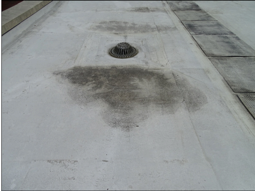
43 - Single-ply membrane roofing main building area - note areas of ponding and deterioration
