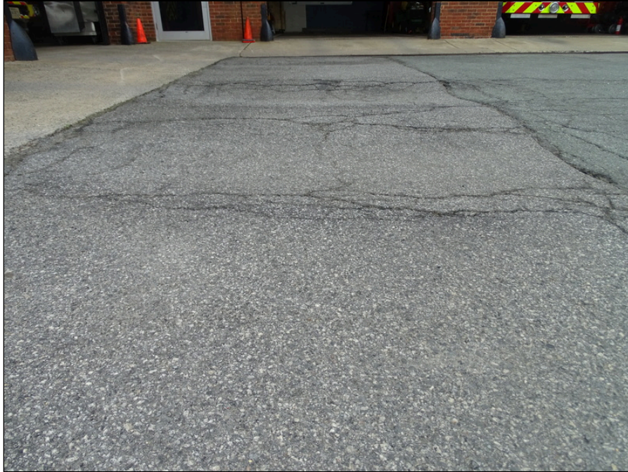
7 - Asphalt paving drive lane and parking northwest side of the building - note alligator cracking
