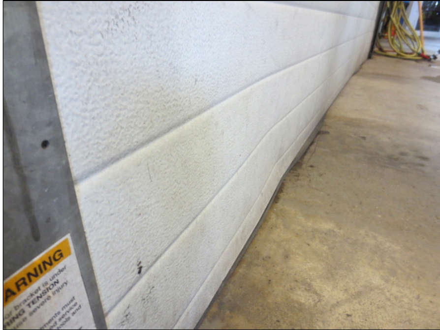
101 - Overhead door damage east
