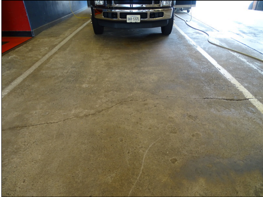
23 - Slab on grade at east bay area - note cracking and settlement
