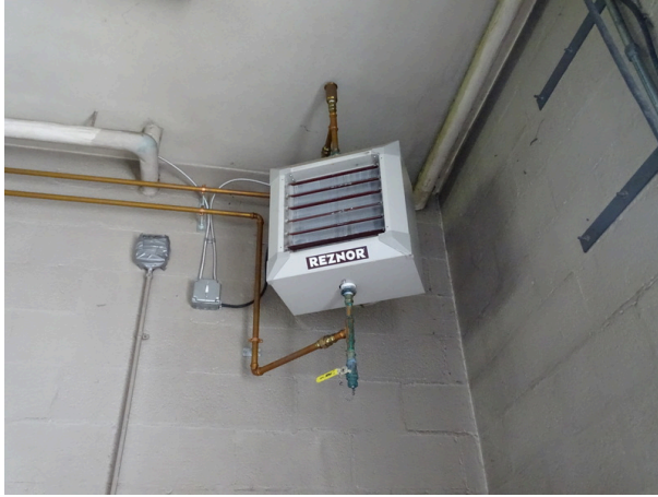
Ceiling mounted hot water heating units
