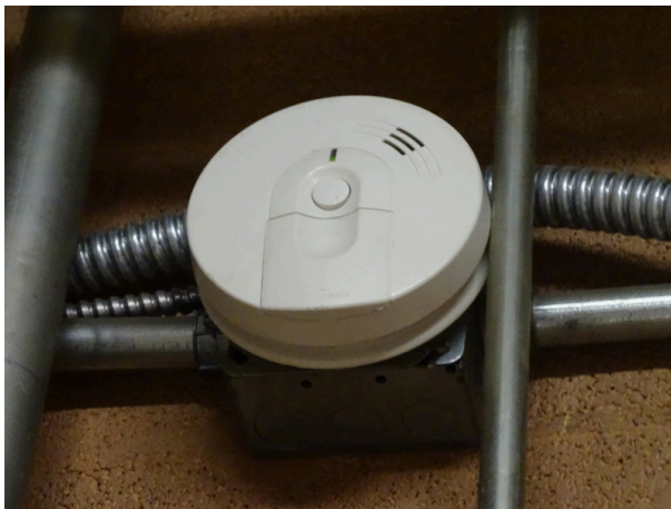
Typical smoke detector
