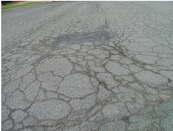
Asphalt paving drive lane and parking northwest side of the building - note alligator cracking
