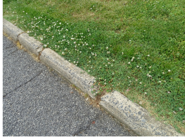
Concrete curb - note deterioration
