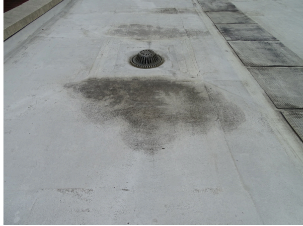
Single-ply membrane roofing main building area - note areas of ponding and deterioration
