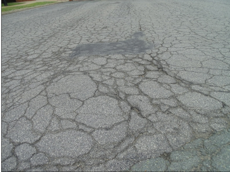
3 - Asphalt paving drive lane and parking northwest side of the building - note alligator cracking
