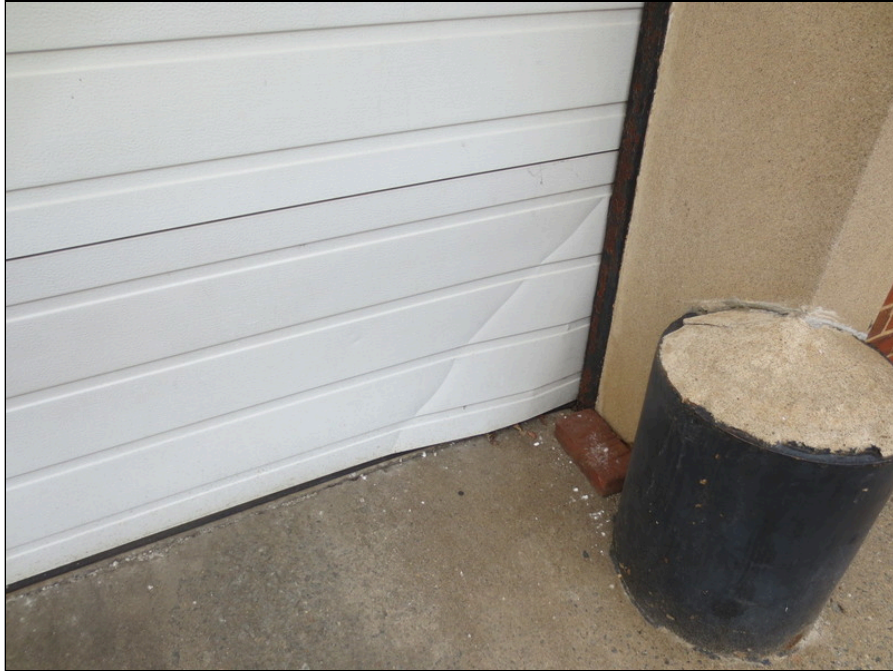
97 - Overhead door damage - east
