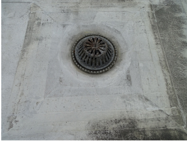
Typical internal drain for main roofing system
