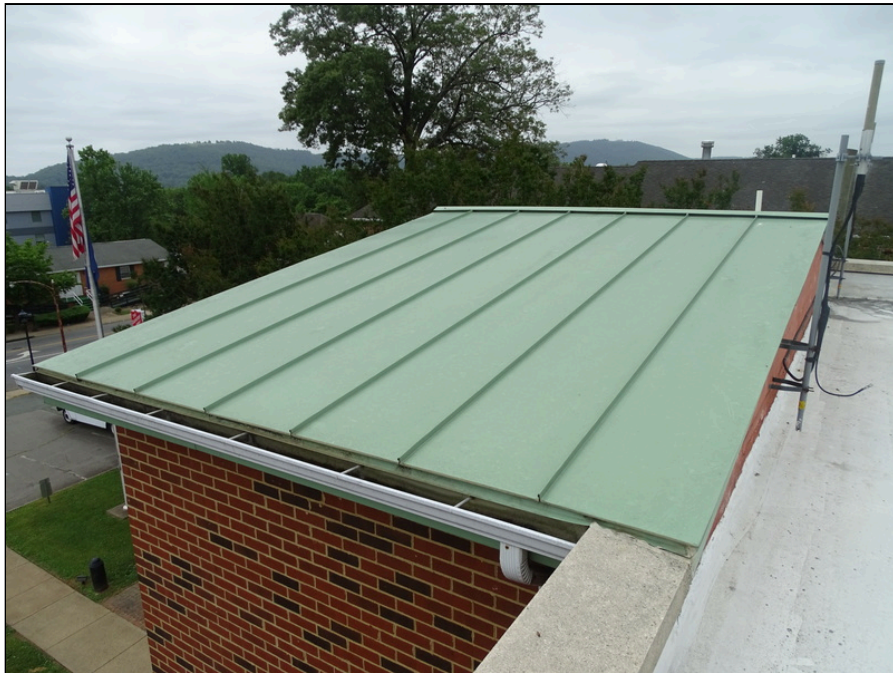
46 - Standing seam metal roofing system over east addition
