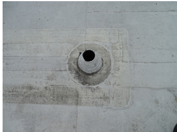
Typical plumbing penetration for main roofing system
