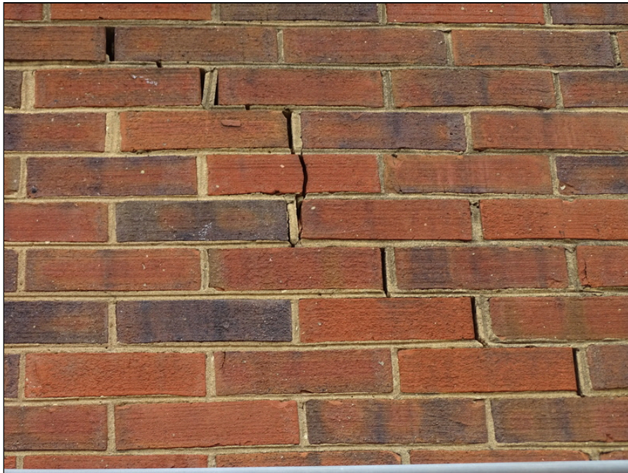
30 - Building exterior -note crack in brick work.
