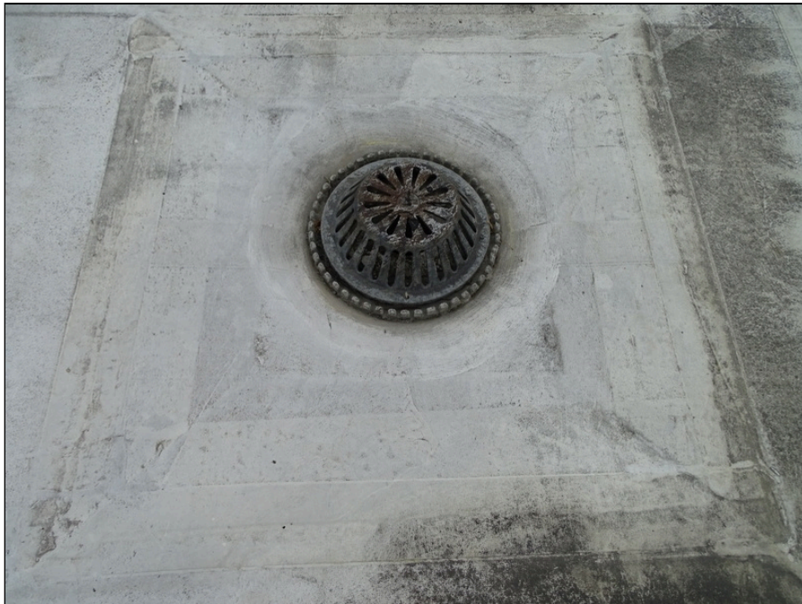
42 - Typical internal drain for main roofing system
