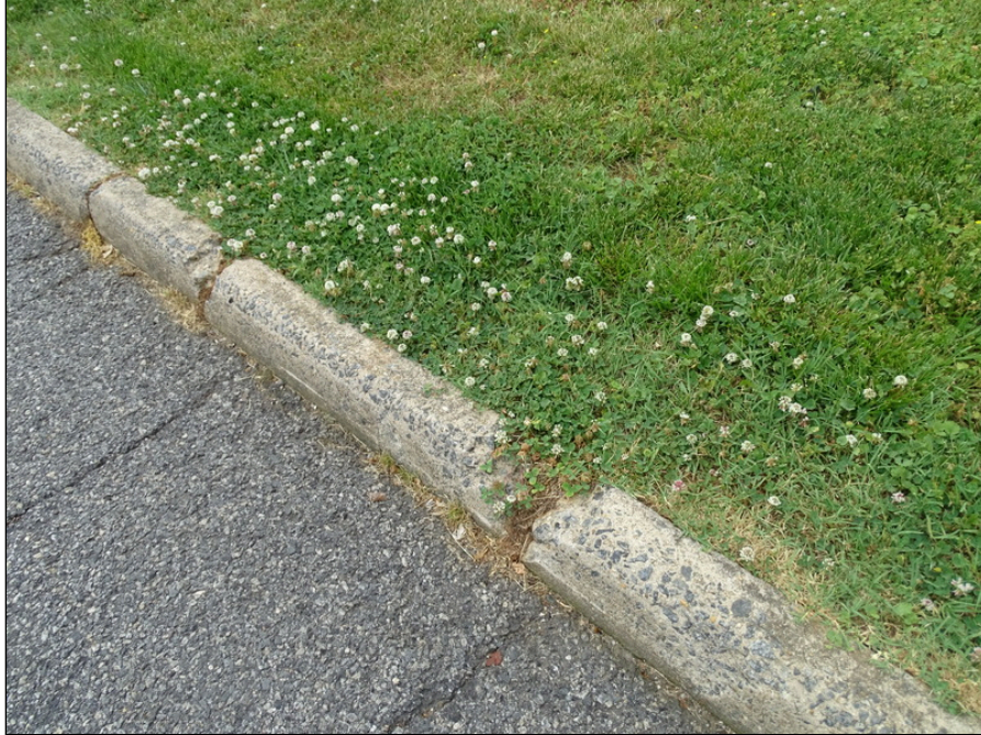
13 - Concrete curb - note deterioration
