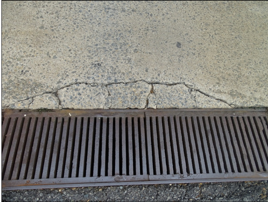
19 - Concrete crack along the drain
