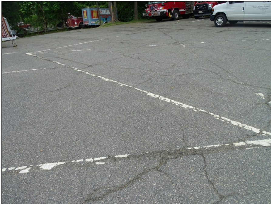
4 - Asphalt paving drive lane and parking northwest area of the site - note alligator cracking
