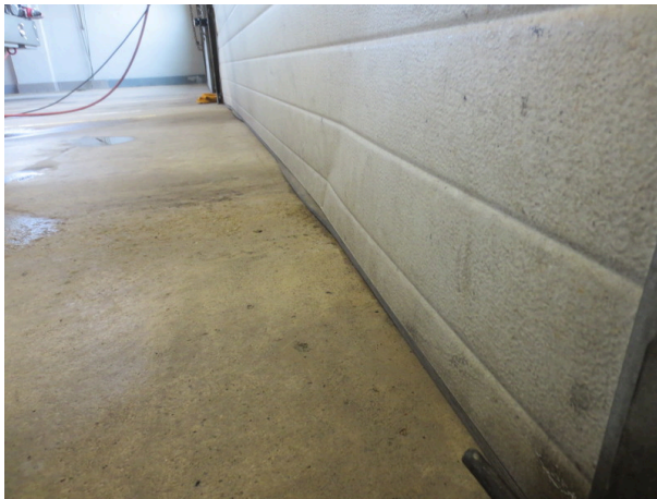
Overhead door damage east
