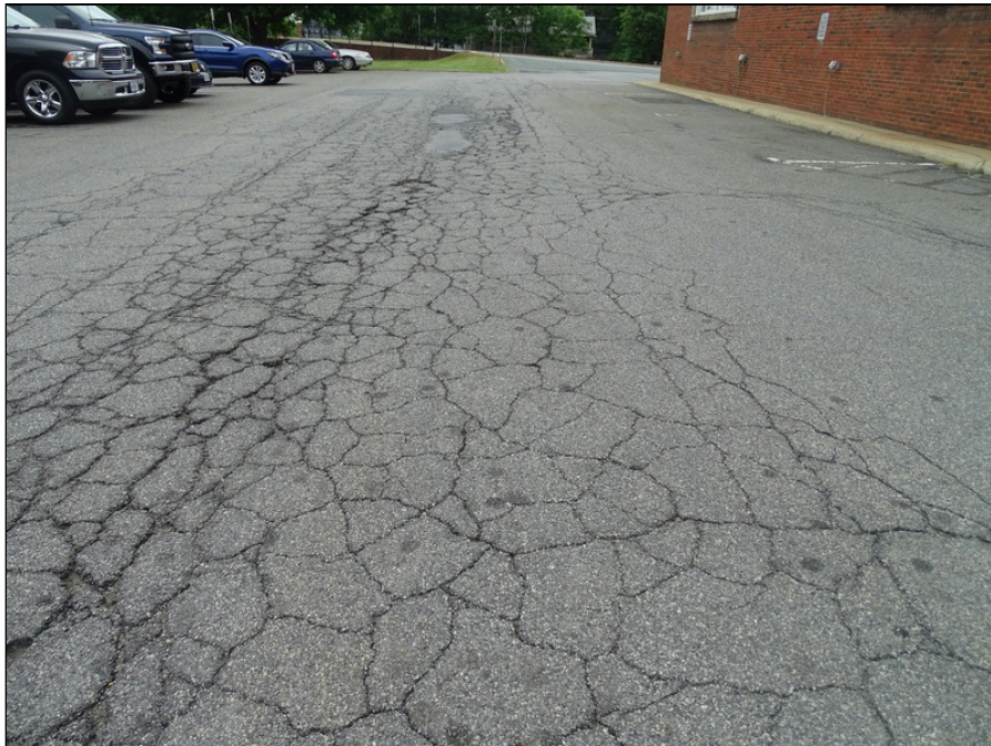
6 - Asphalt paving drive lane and parking northwest side of the building - note alligator cracking
