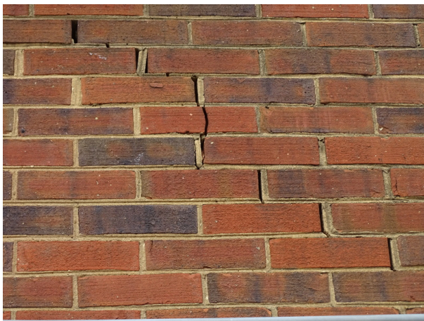
Building exterior -note crack in brick work.
