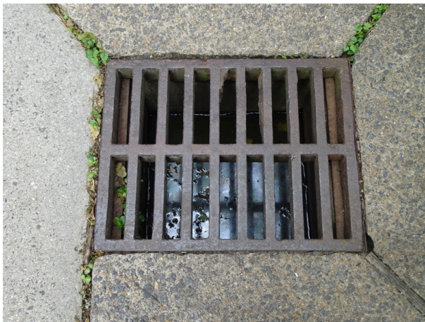
Typical yard inlet drain
