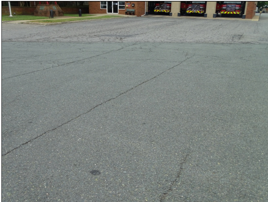
2 - Asphalt paving drive lane and parking northwest side of the building - note alligator cracking
