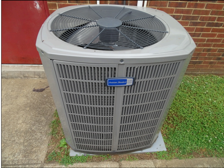
61 - Condenser located on grade - manufactured by American Standard
