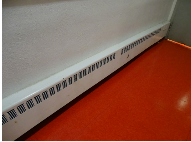
Typical hot water baseboard heater unit
