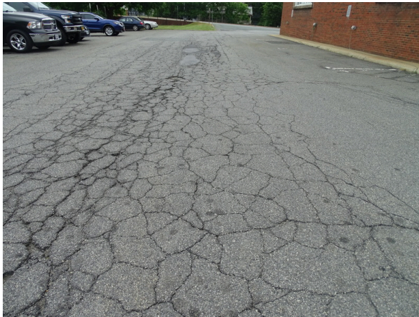
Asphalt paving drive lane and parking northwest side of the building - note alligator cracking
