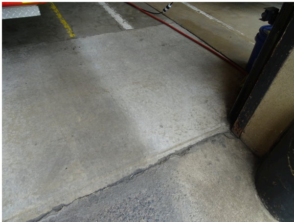
Slab on grade at east bay area - note cracking and settlement
