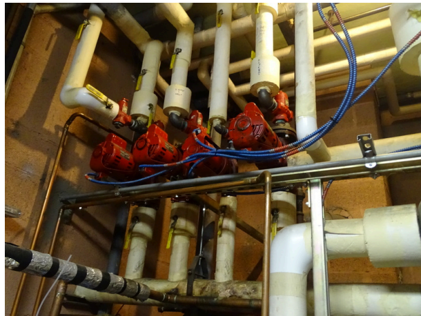
Typical hot water piping system
