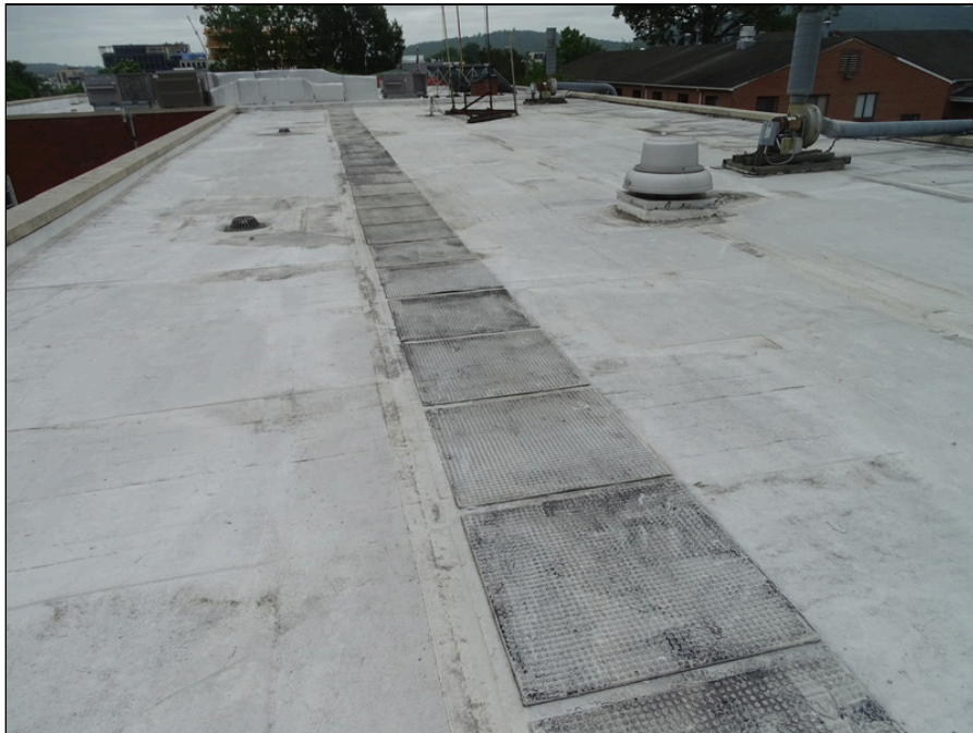
40 - Single-ply membrane roofing system over main building area
