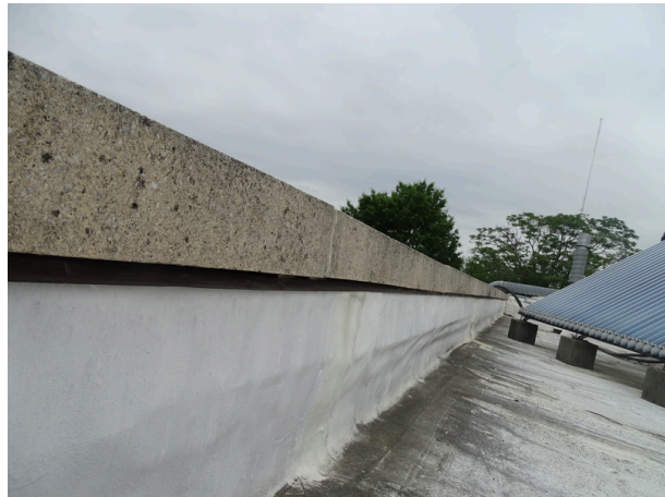
Typical parapet wall - note area of roofing system patching
