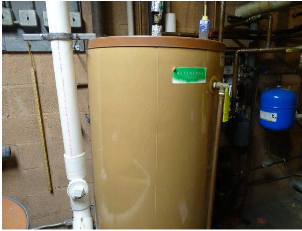
Domestic hot water storage tank
