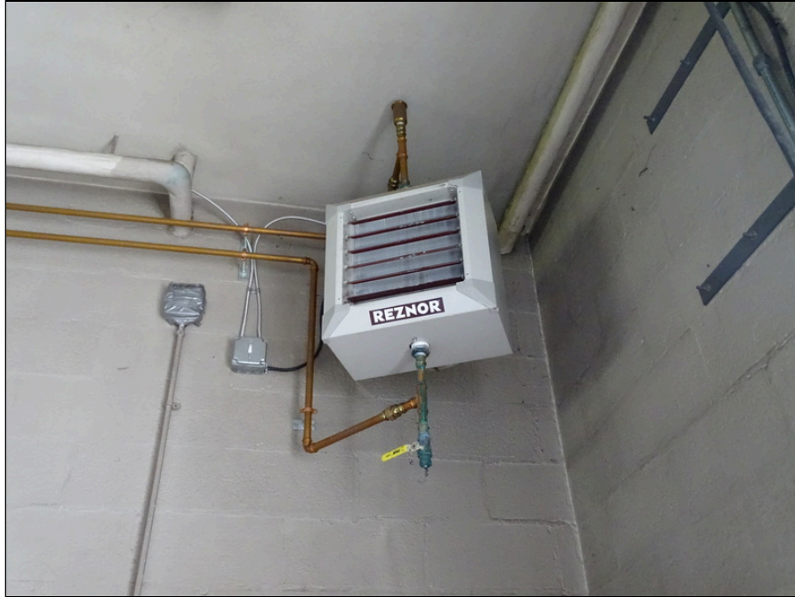
63 - Ceiling mounted hot water heating units
