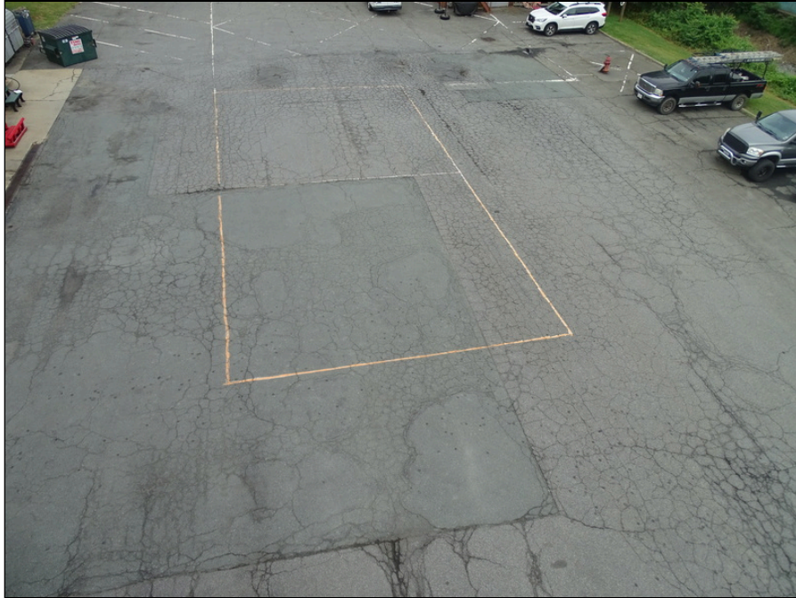
9 - Asphalt paving drive lane and parking northwest area of the site - note alligator cracking
