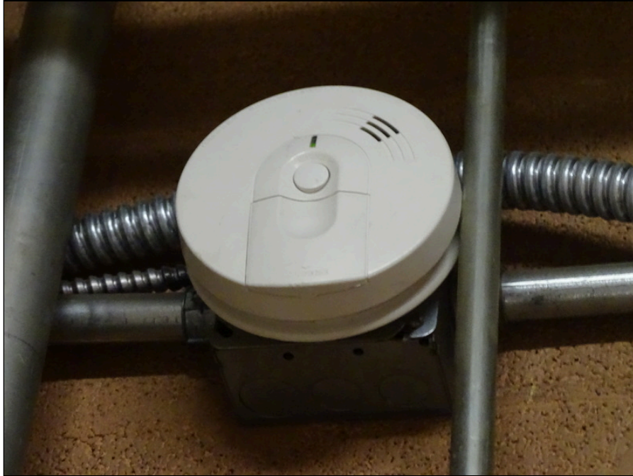
77 - Typical smoke detector
