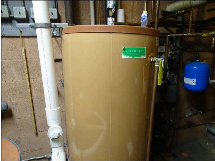
53 - Domestic hot water storage tank
