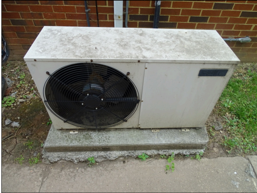
59 - Condenser located on grade - manufactured by Enviromaster International in 1996
