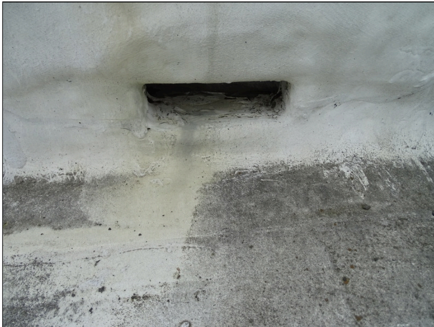
48 - Typical parapet wall and through wall scupper drain of main roofing system
