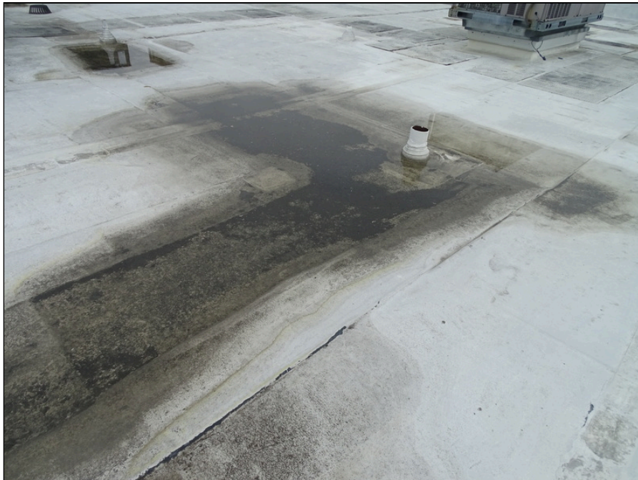
44 - Single-ply membrane roofing main building area - note areas of ponding and deterioration
