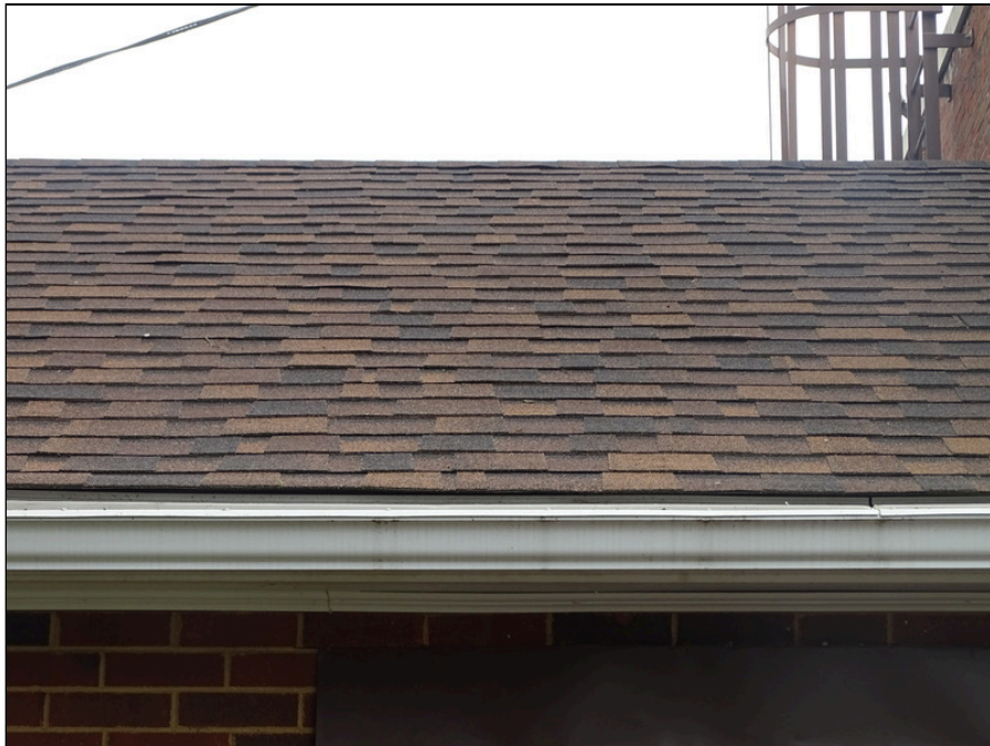
50 - Asphalt shingle roofing system over west addition - note recent replacement
