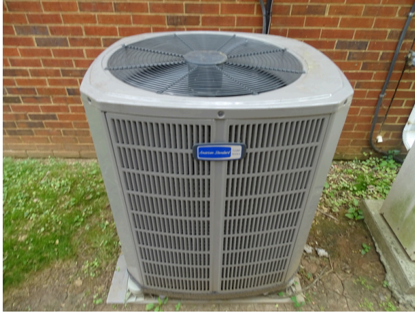
Condenser located on grade - manufactured by American Standard in 2017
