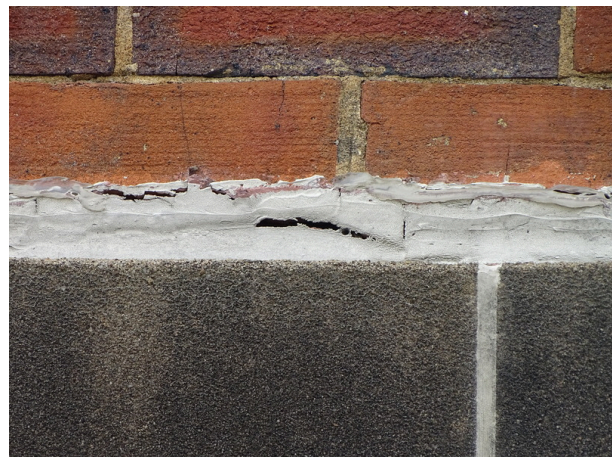
Typical sealant condition
