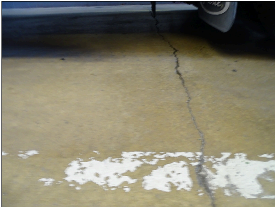
22 - Slab on grade at east bay area - note cracking and settlement
