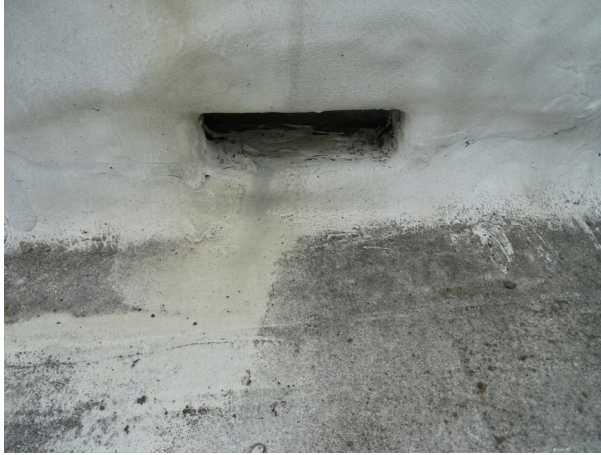
Typical parapet wall and through wall scupper drain of main roofing system
