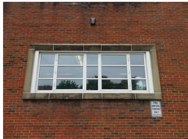
Typical window - note water staining
