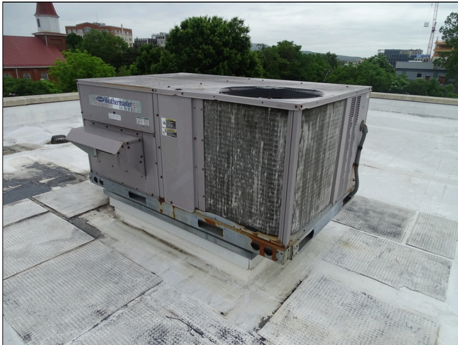
56 - Condenser located on roof - manufactured by Carrier in 2006
