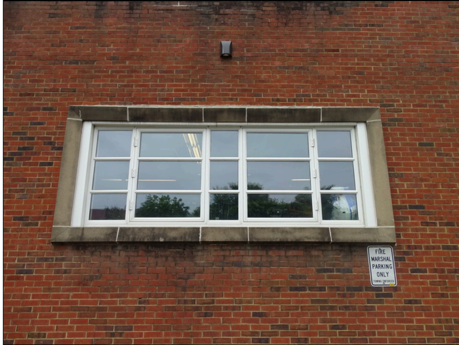
37 - Typical window - note water staining
