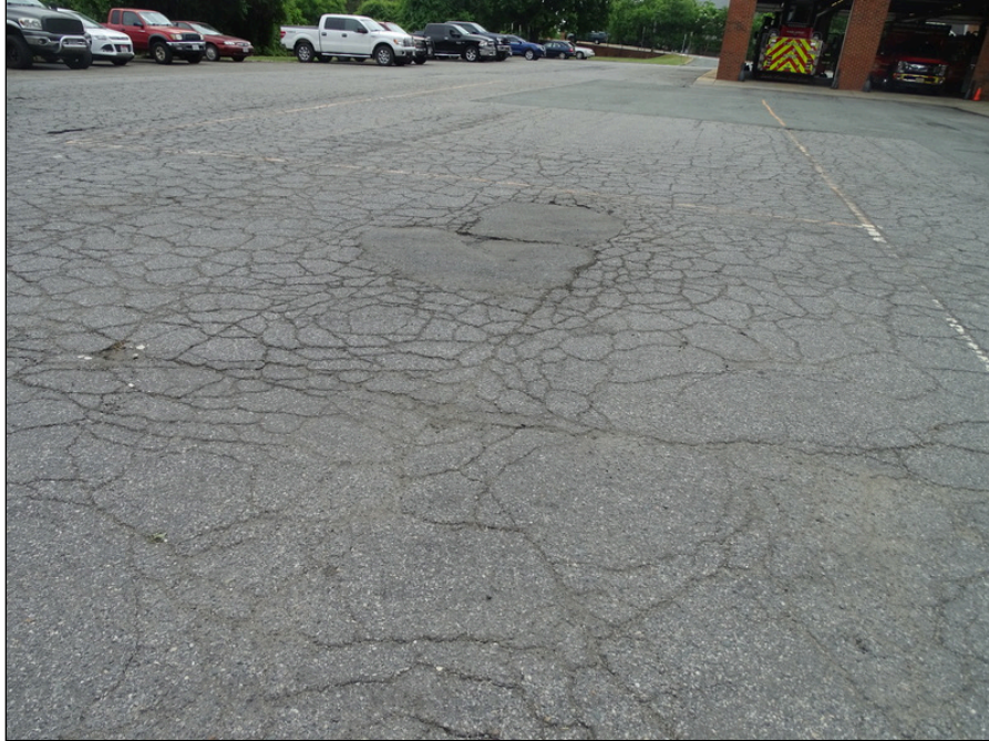
5 - Asphalt paving drive lane and parking northwest side of the building - note alligator cracking
