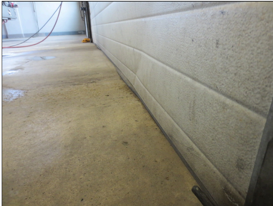
102 - Overhead door damage east
