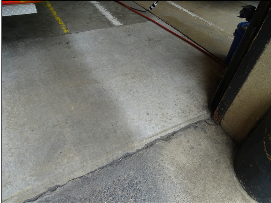
21 - Slab on grade at east bay area - note cracking and settlement
