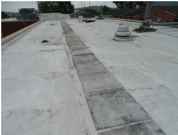
Single-ply membrane roofing system over main building area
