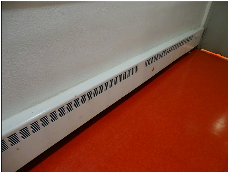
66 - Typical hot water baseboard heater unit
