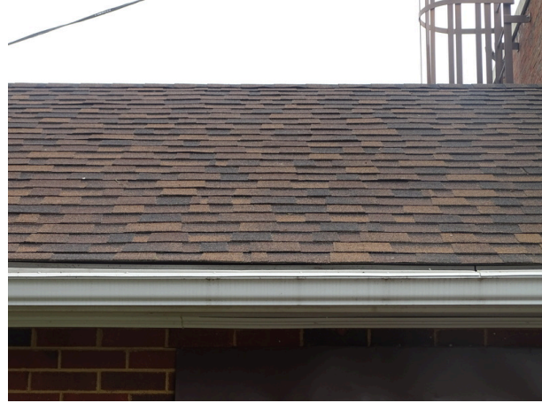
Asphalt shingle roofing system over west addition - note recent replacement
