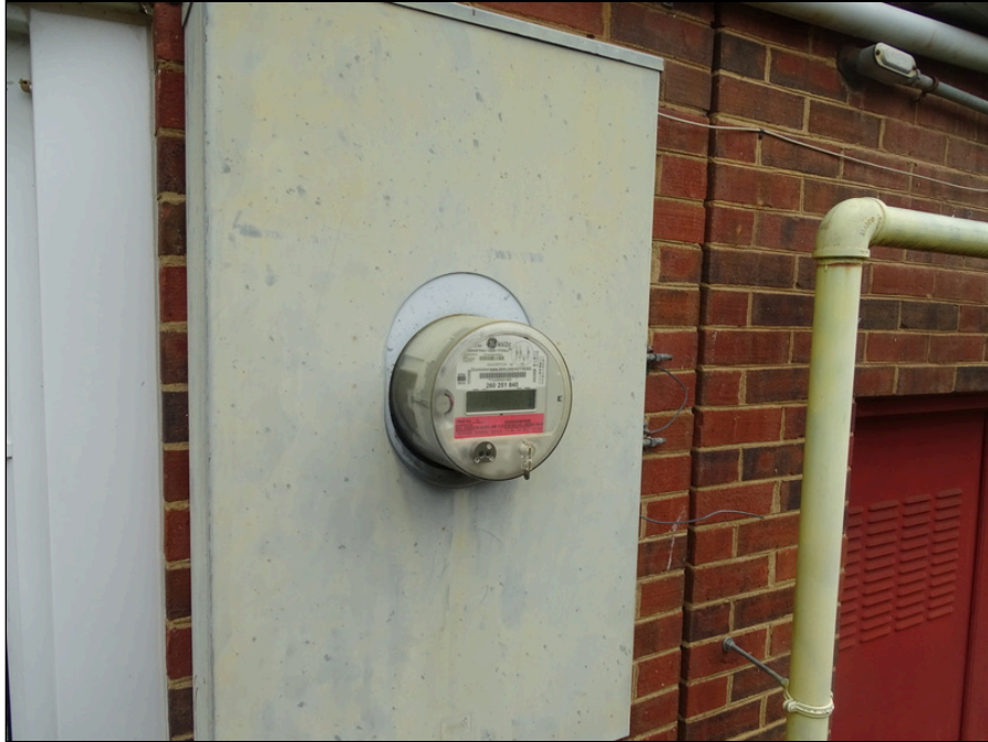
71 - Typical electric meter
