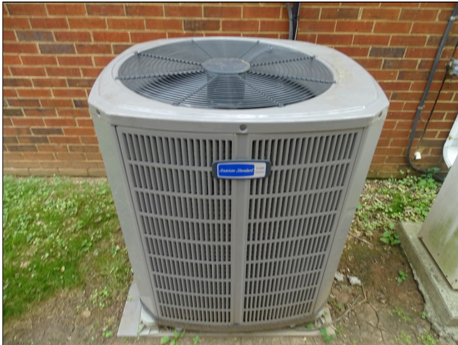
60 - Condenser located on grade - manufactured by American Standard
