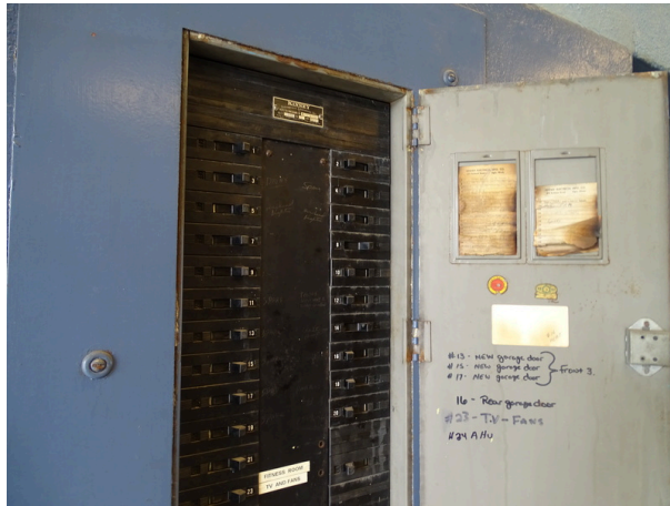
Typical electrical sub panel
