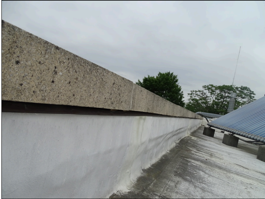
45 - Typical parapet wall - note area of roofing system patching
