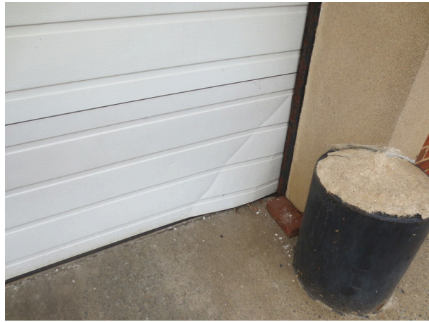
Overhead door damage - east
