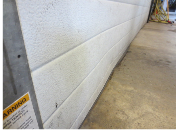
Overhead door damage east
