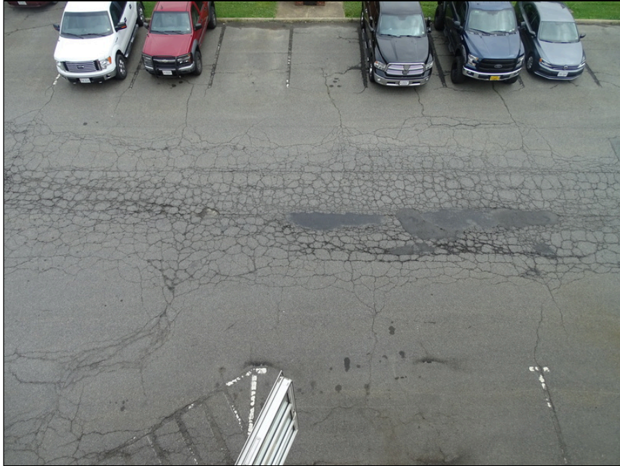
11 - Asphalt paving drive lane and parking northwest side of the building - note alligator cracking
