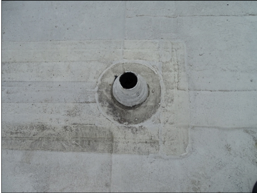
41 - Typical plumbing penetration for main roofing system
