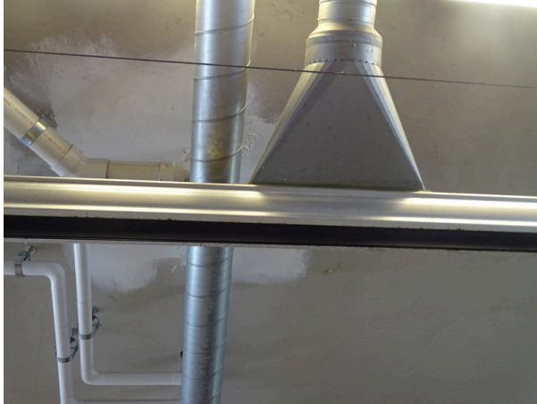
Typical interior of bay area - note peeling paint on ceiling
