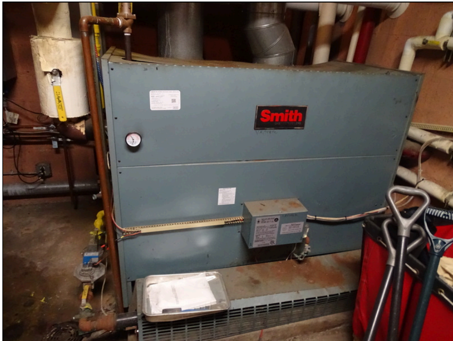
54 - Boiler located in main utility room
