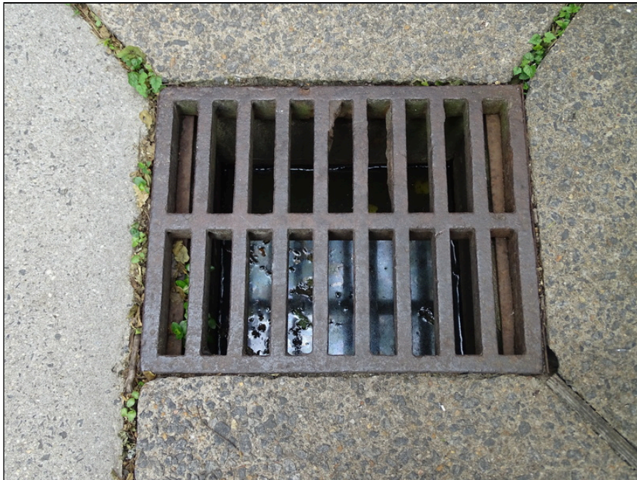
18 - Typical yard inlet drain
