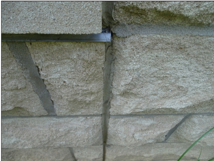
26 - Building exterior - note minor deterioration and damage to mortar
