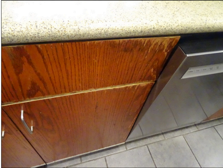
117 - Deterioration of the kitchen cabinet
