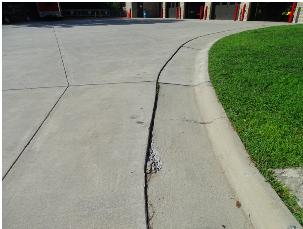
Concrete pavement - note cracked and deterioration
