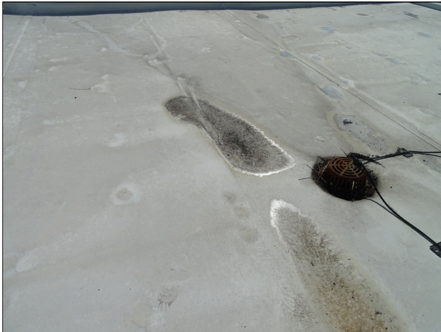
44 - Deteriorated internal drain
