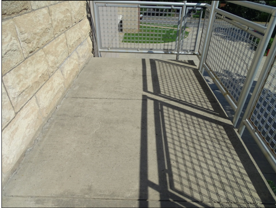
11 - Sidewalk - note concrete separated from wall
