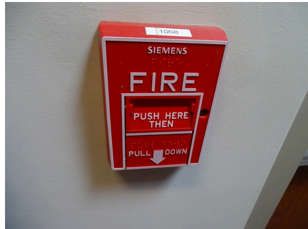
Typical pull down station
