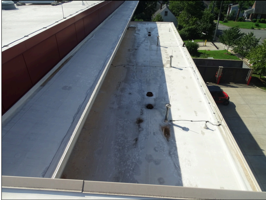
45 - Deteriorated single Ply - roof
