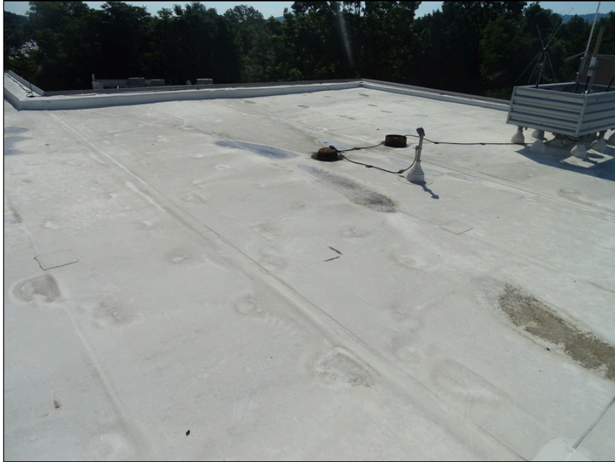
41 - Single-ply roofing system overview
