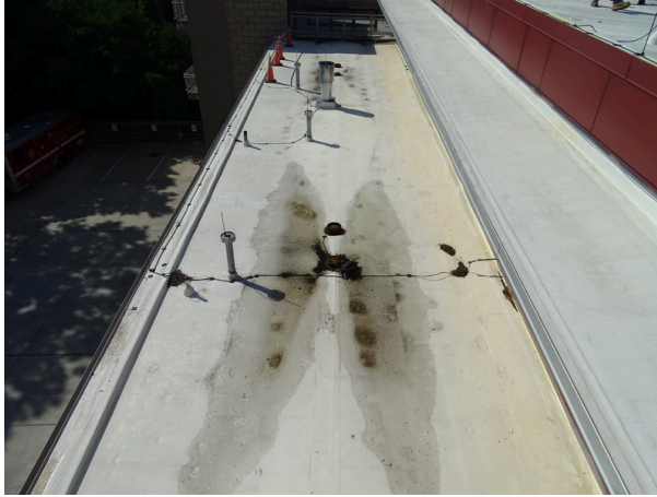
Water ponding on top of the roof
