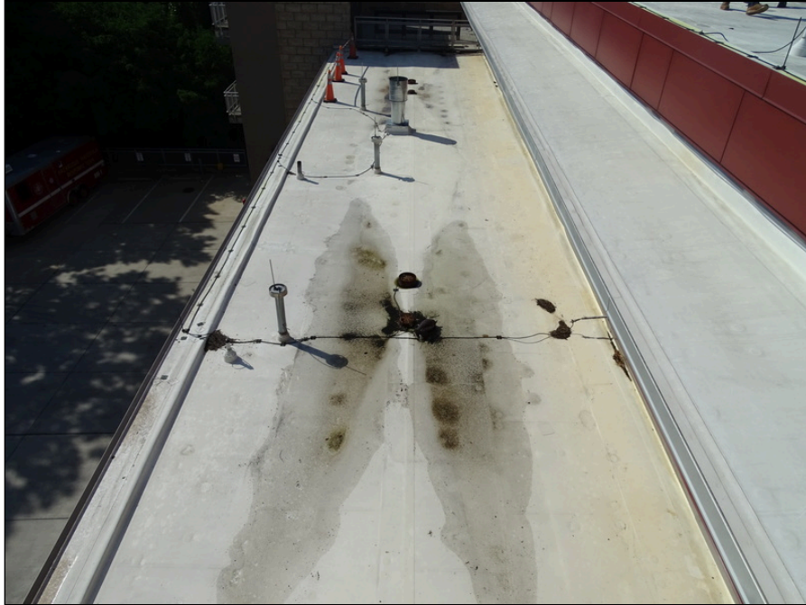
43 - Water ponding on top of the roof
