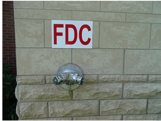
Typical Fire Department Connection
