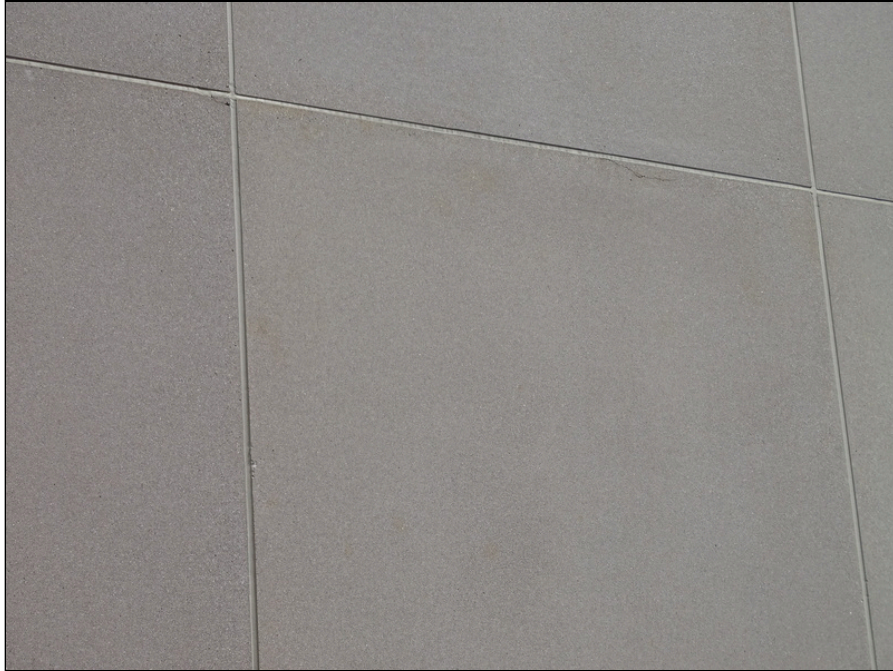
25 - Cracked in exterior wall
