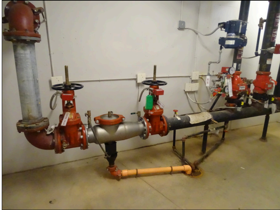
79 - wet sprinkler system piping
