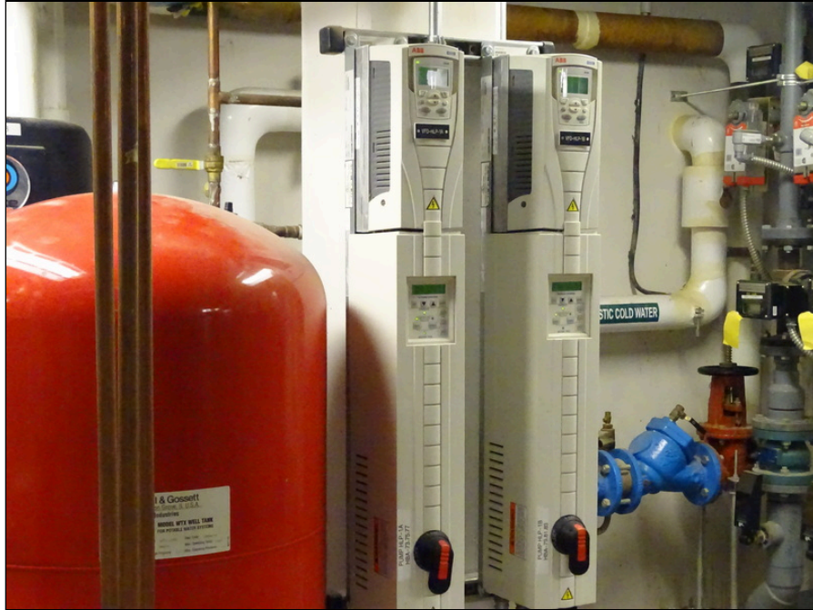
65 - Variable frequency drive mechanical controls
