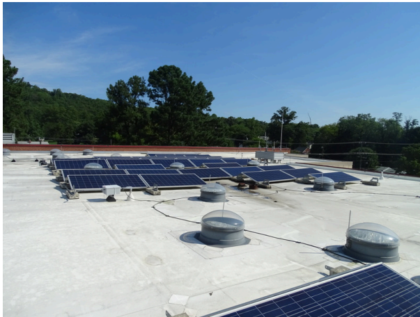
Single-ply roofing system overview
