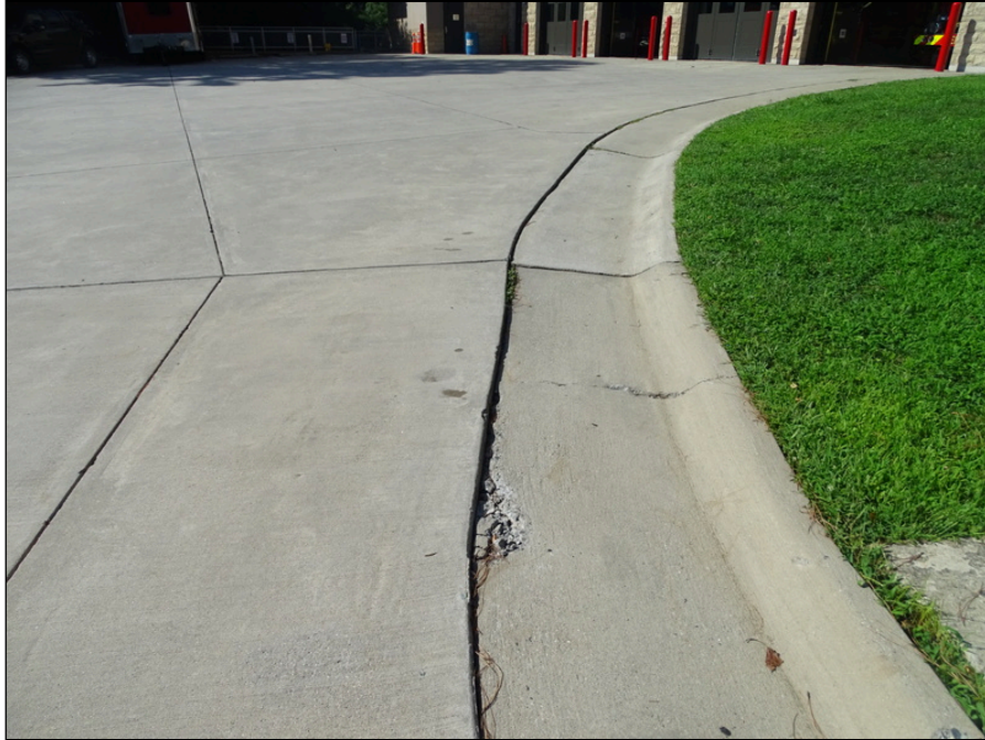
3 - Concrete pavement - note cracked and deterioration
