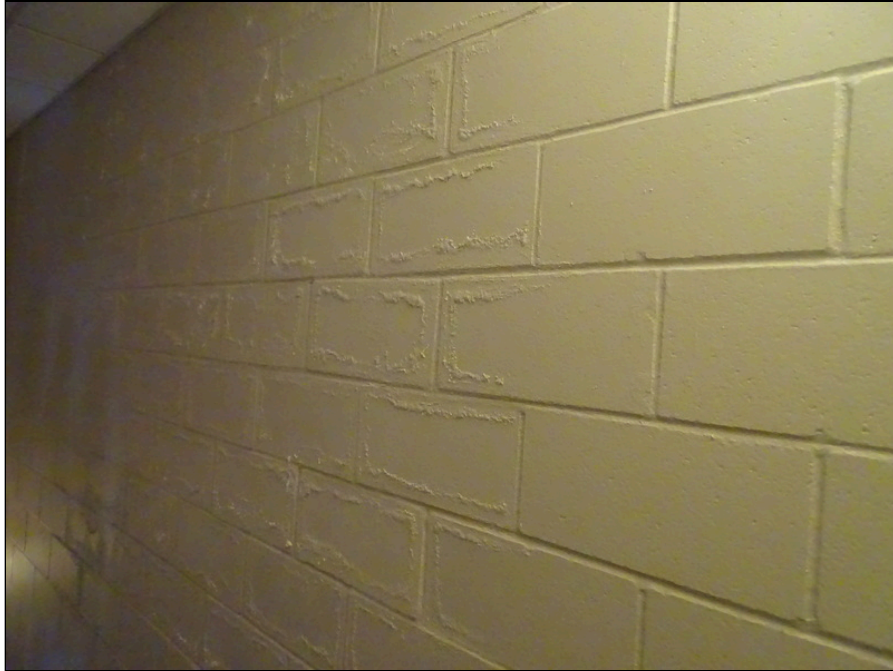
105 - Efflorescence wall interior
