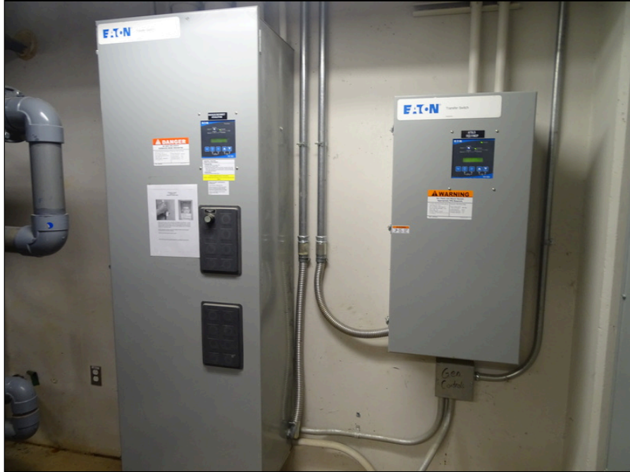
75 - Typical transfer switch
