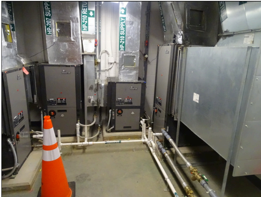
62 - Geothermal Heat Pump Vertical Package Unit
