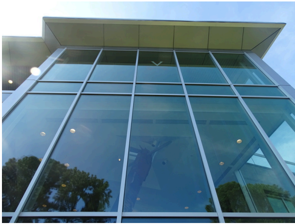
Glass curtain wall exterior window
