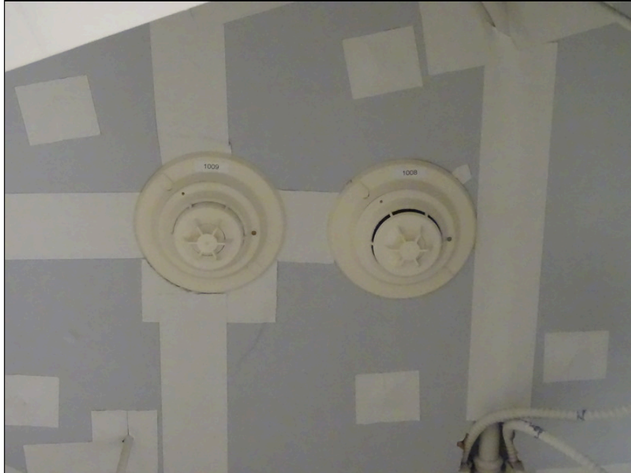
83 - Typical smoke detector
