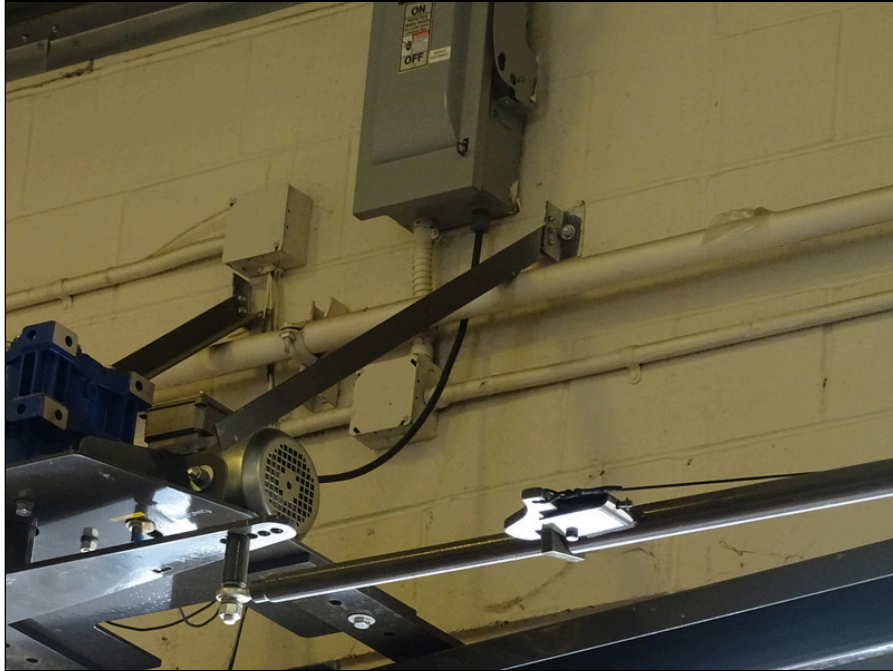
31 - Overhead doors with reported problems with bracing
