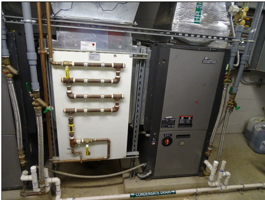
60 - Geothermal Heat Pump Vertical Package Unit
