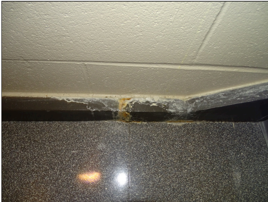
108 - Water leakage at ceiling
