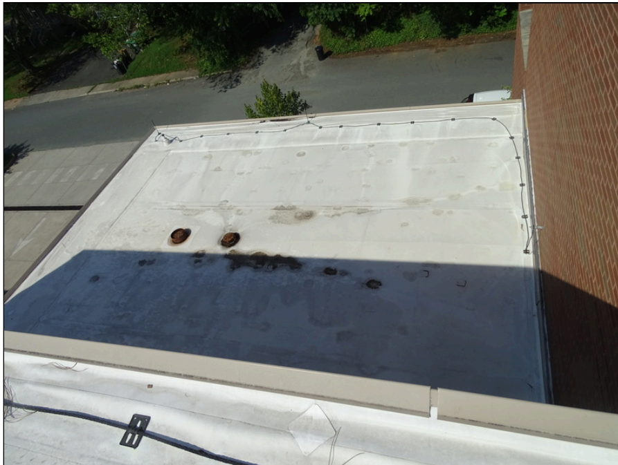
42 - Single ply roof - note deterioration
