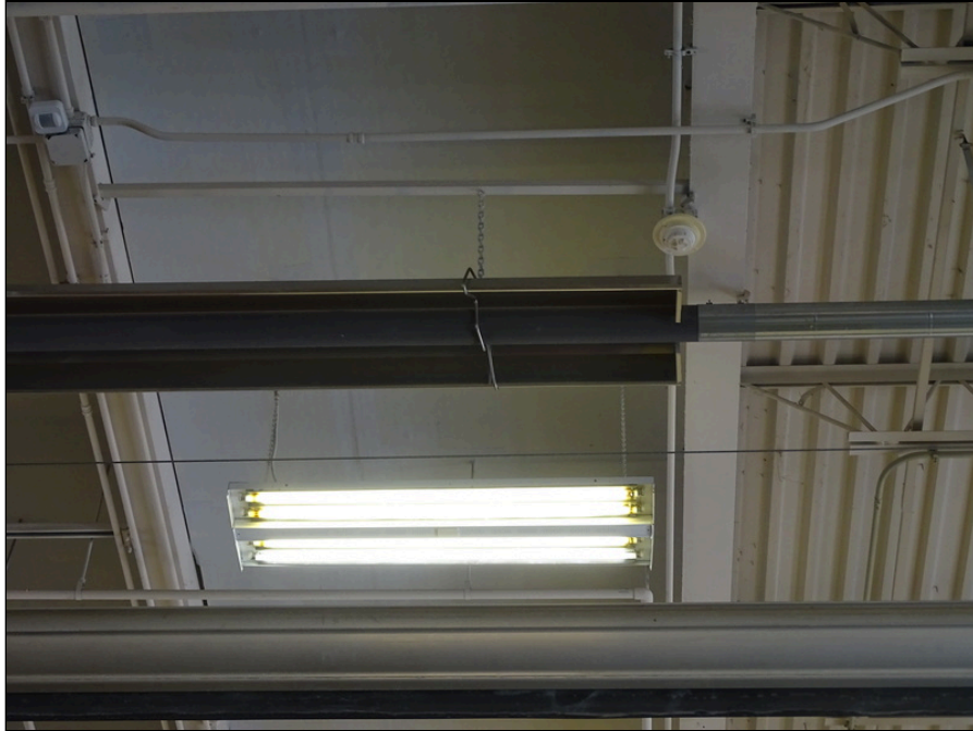
37 - Metal deck supporting an elevated level
