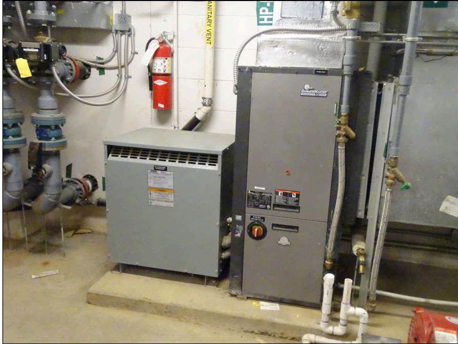
61 - Geothermal Heat Pump Vertical Package Unit
