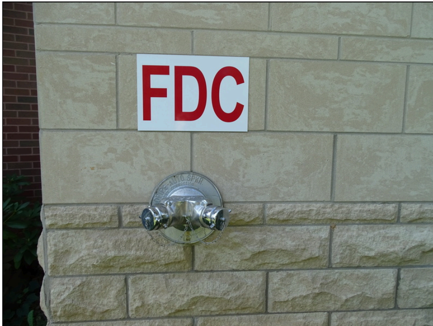
78 - Typical Fire Department Connection
