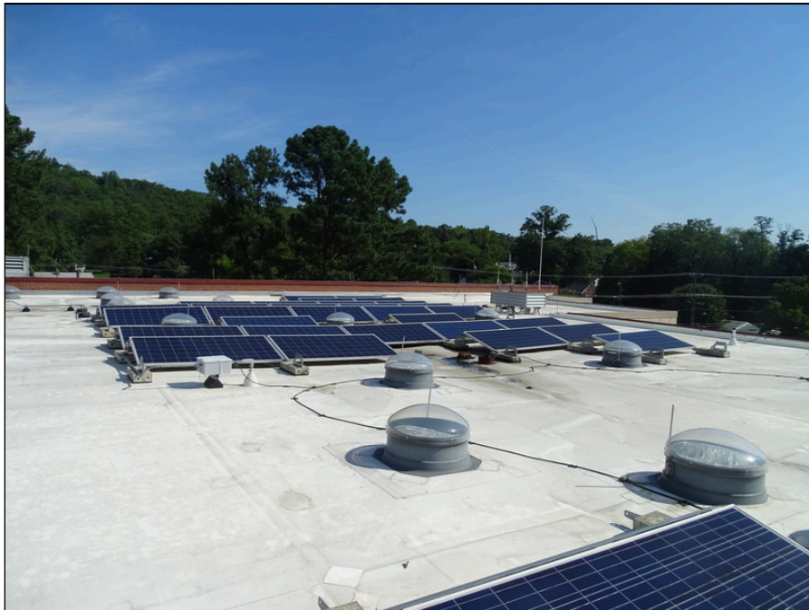
46 - Single-ply roofing system overview
