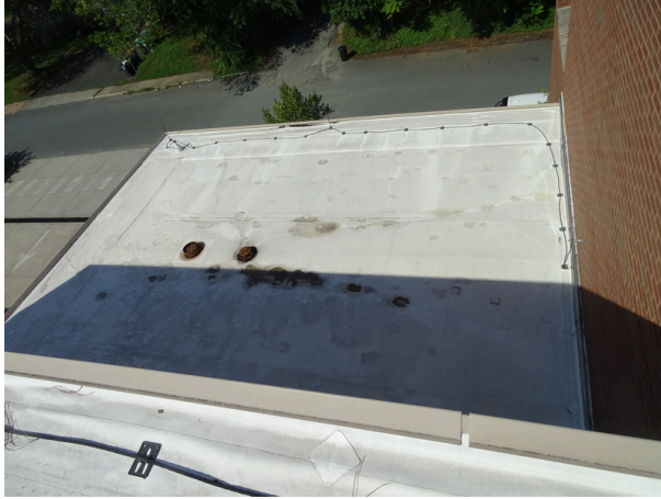
Single ply roof - note deterioration
