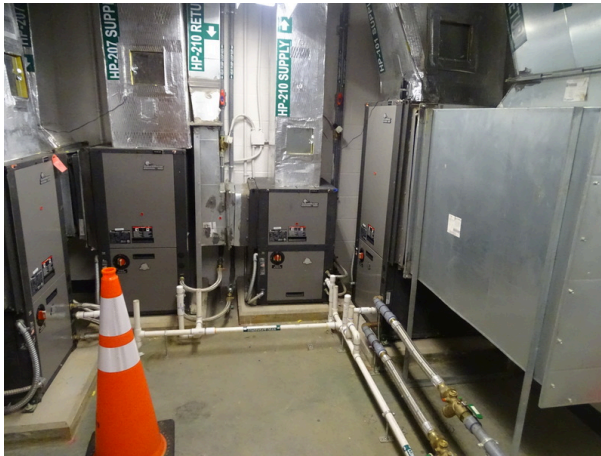
Geothermal Heat Pump Vertical Package Unit
