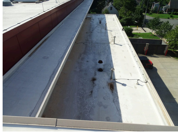
Deteriorated single Ply - roof
