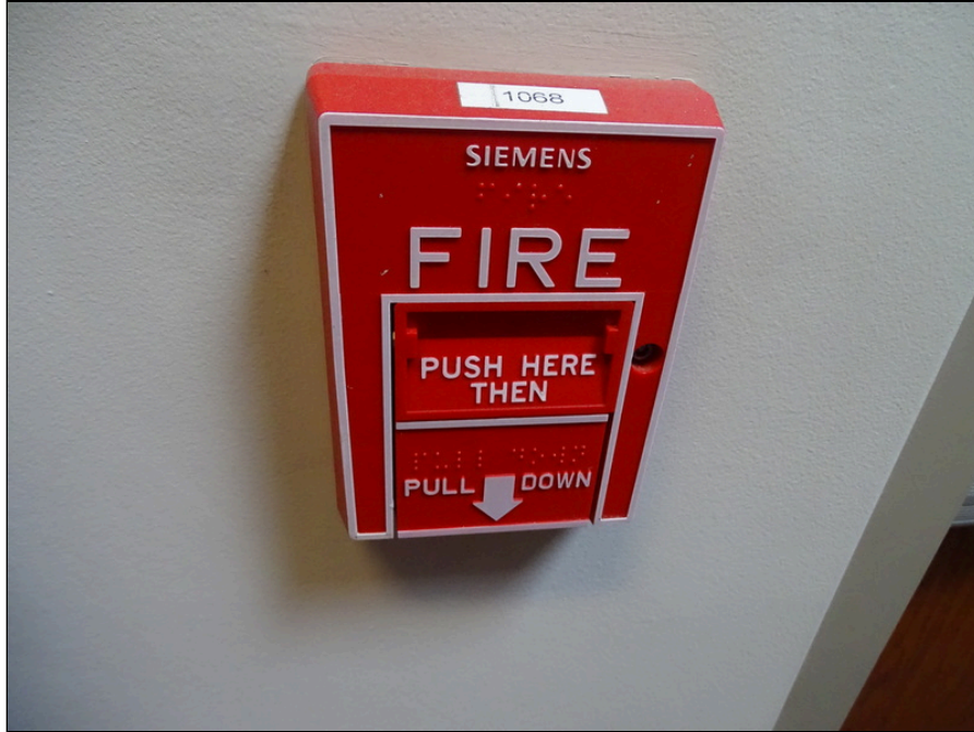
85 - Typical pull down station
