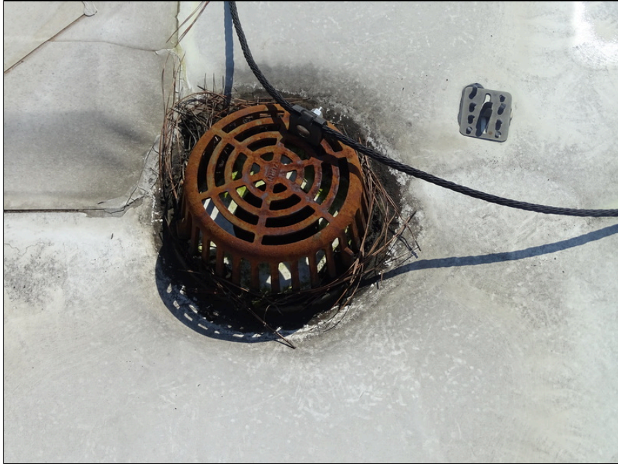
49 - Typical internal drain
