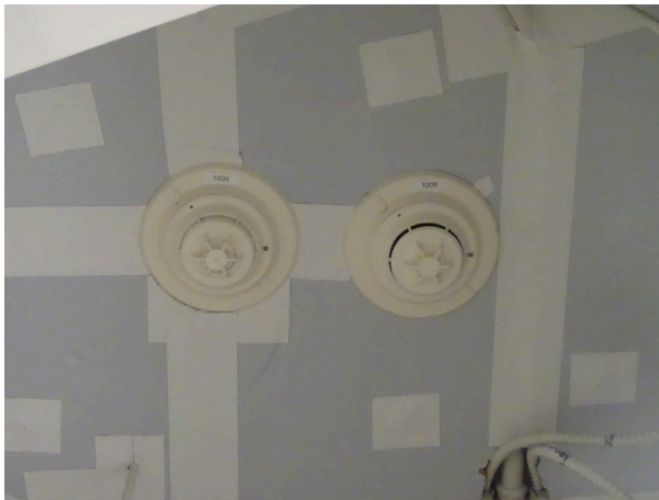
Typical smoke detector
