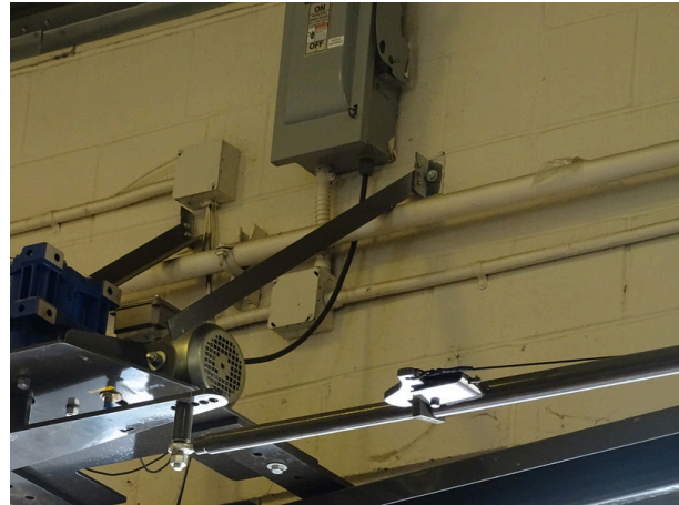
Overhead doors with reported problems with bracing
