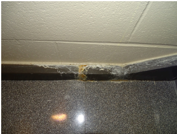
Water leakage at ceiling
