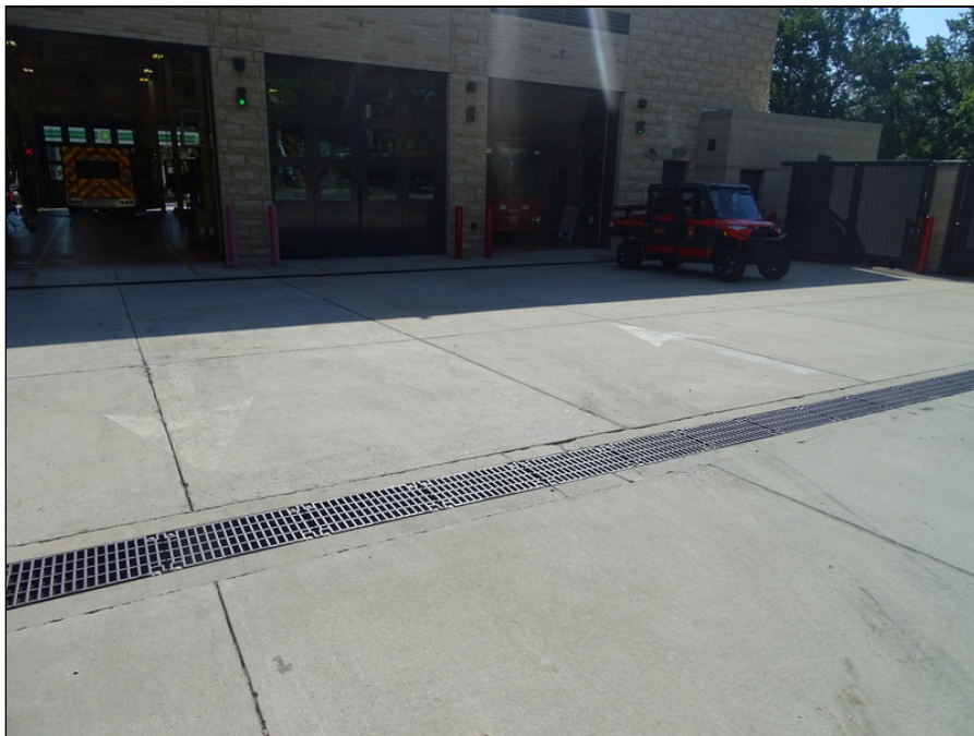
10 - Typical storm water drainage
