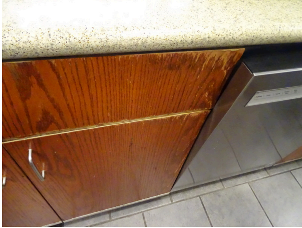
Deterioration of the kitchen cabinet
