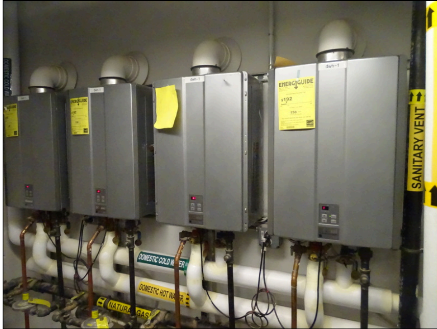
125 - Tankless domestic water heaters
