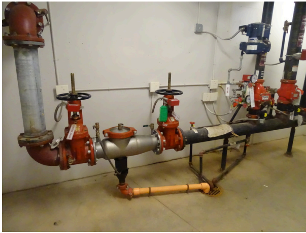
Typical sprinkler system piping
