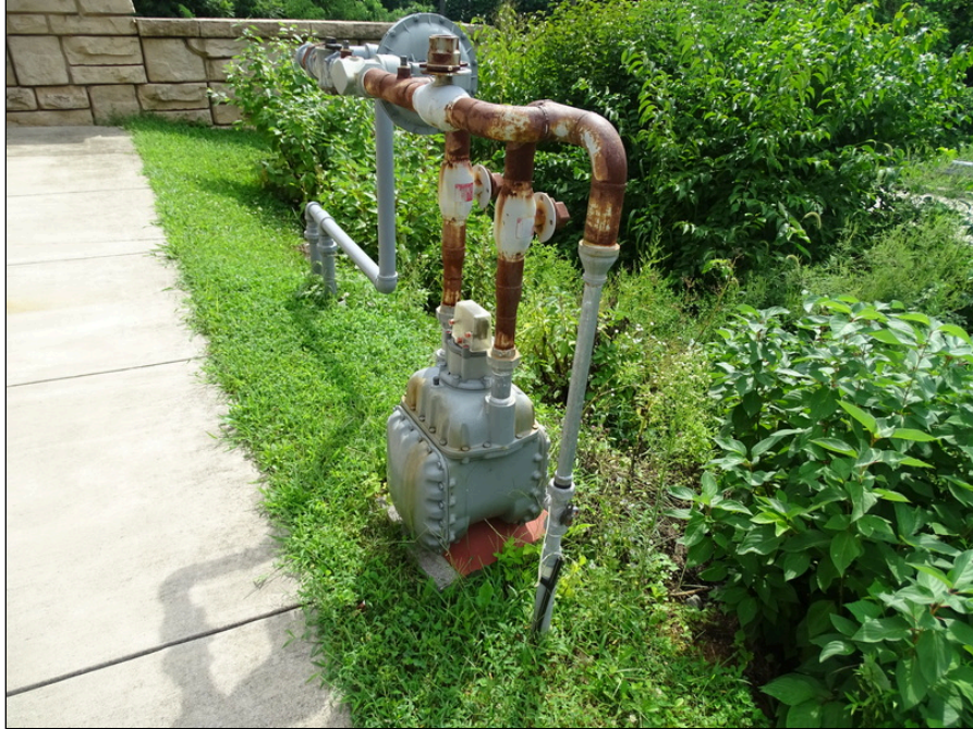
77 - Gas meter piping condition
