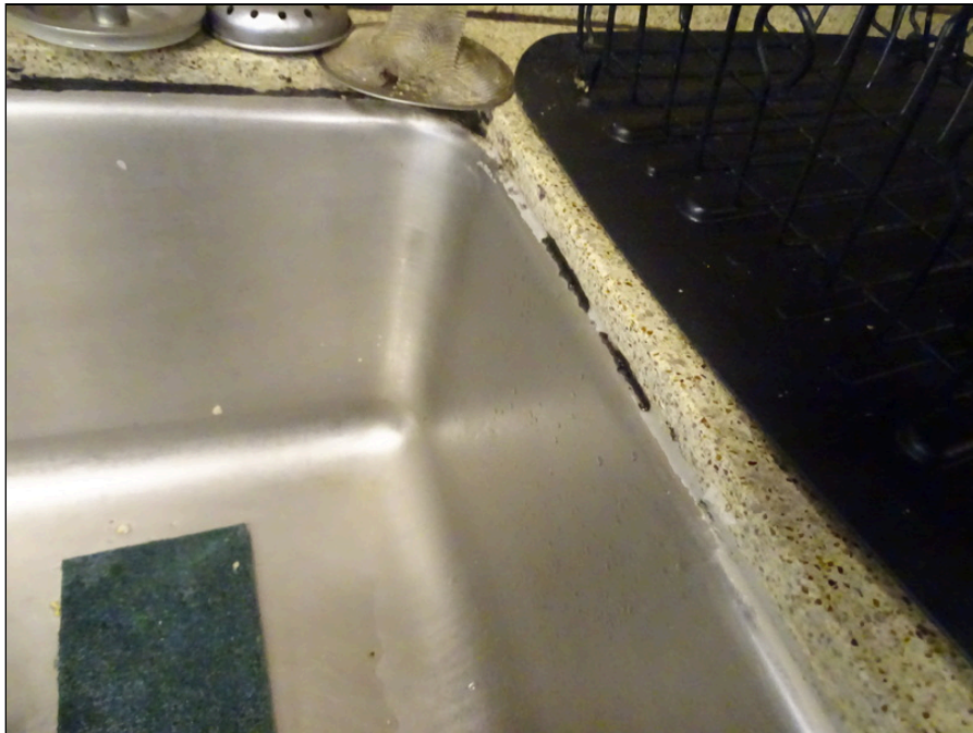
118 - Deterioration of the kitchen sink sealant
