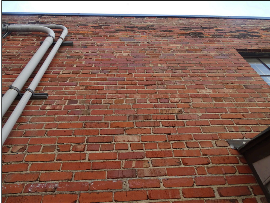
5 - Brick exterior at west side of the building - note deterioration above window
