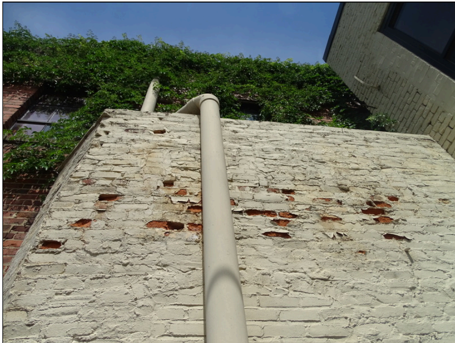
10 - Typical exterior wall - note deterioration
