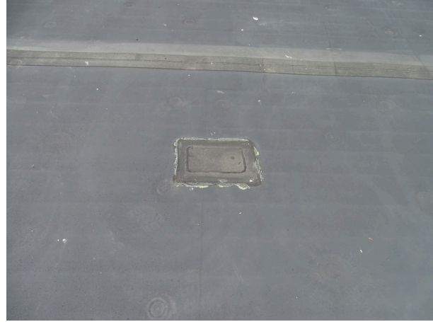
Roofing system - note patching
