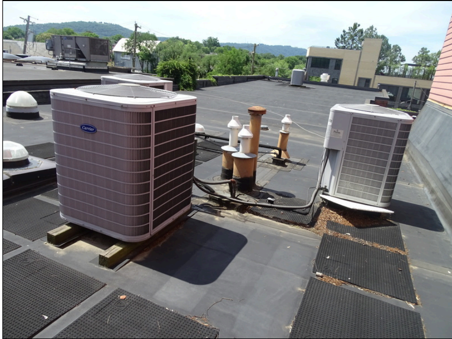
27 - Typical condenser unit
