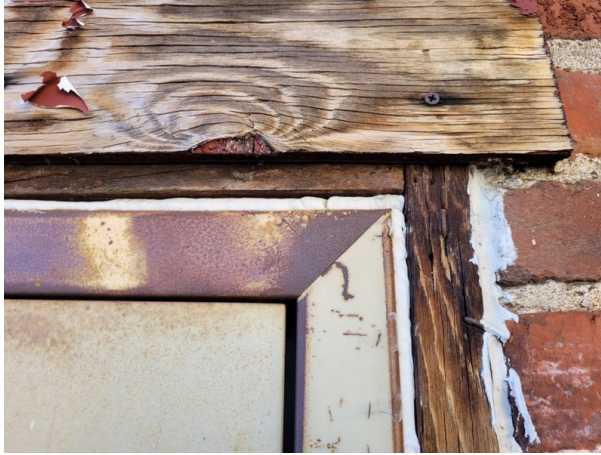
Rear door sealant condition
