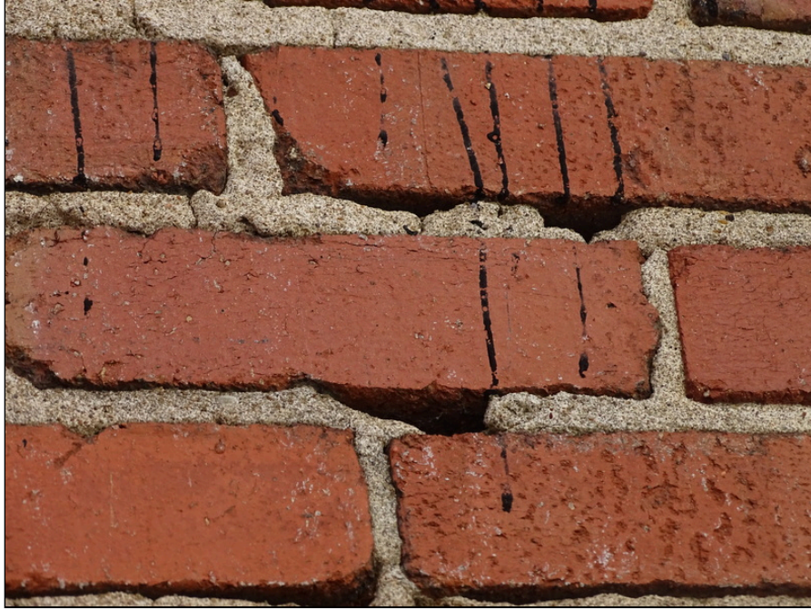
7 - Brick exterior at west side of the building - note deterioration above window
