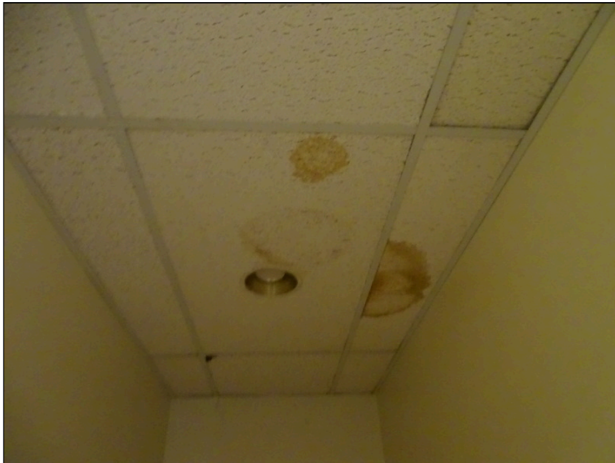
26 - Typical ceiling - note water leakage
