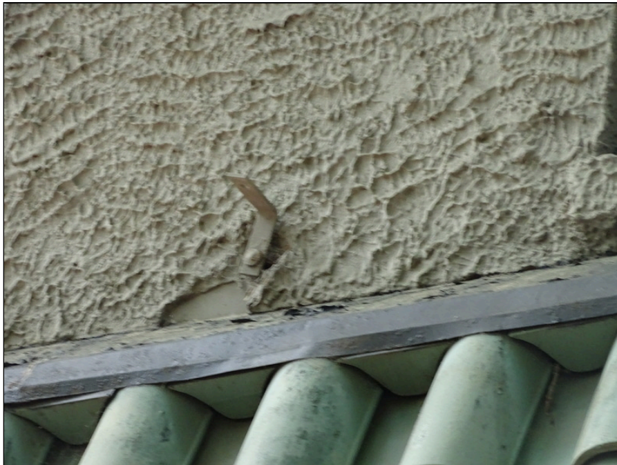
12 - Exterior stucco wall - note deterioration
