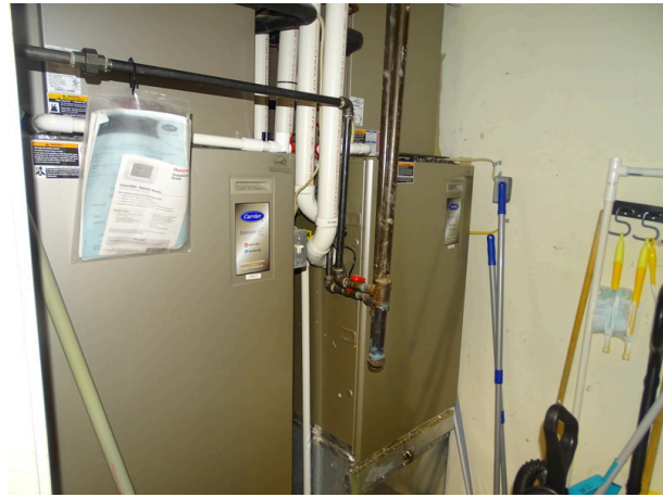
Typical gas furnace and air handler units
