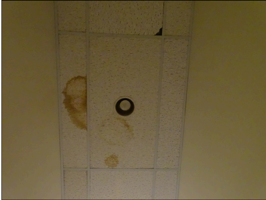
25 - Typical ceiling - note water leakage
