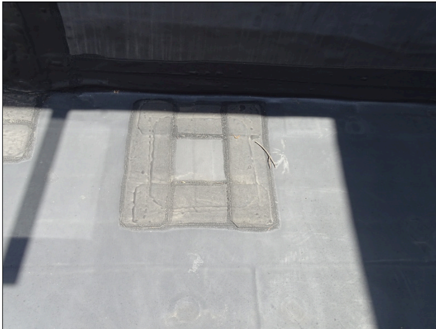
24 - Roofing system - note patching
