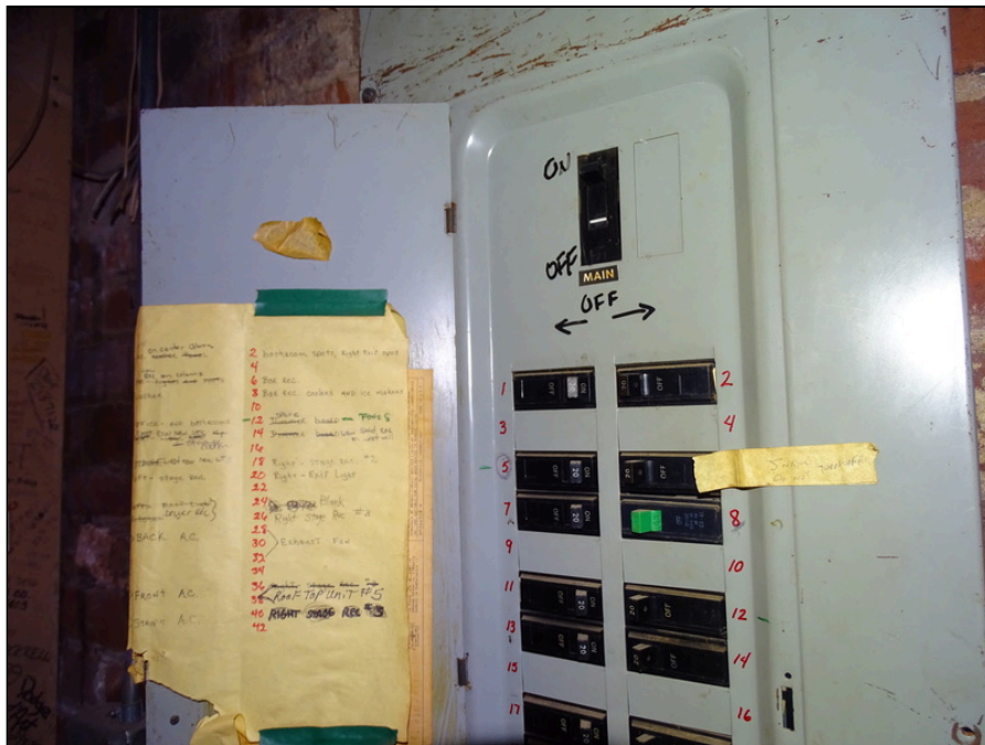
32 - Electric main disconnect panel
