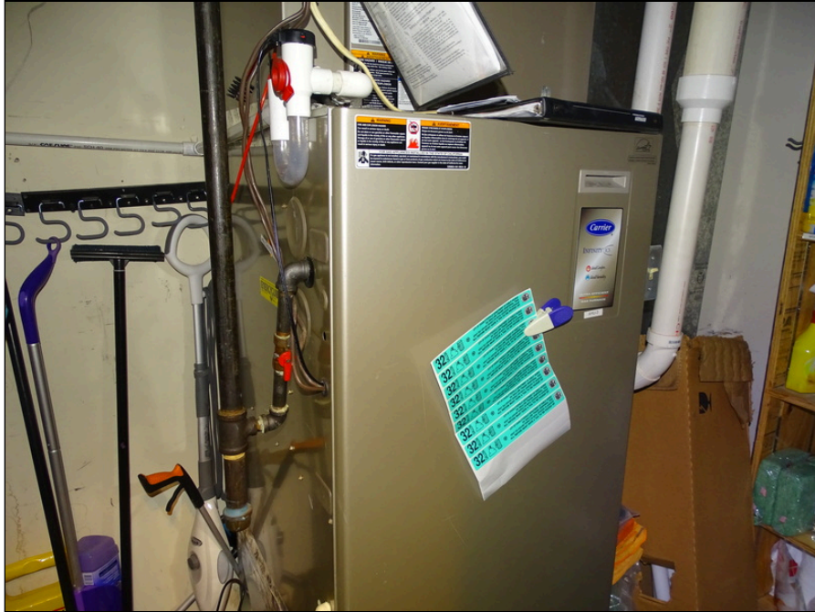
29 - Typical gas furnace and air handler units
