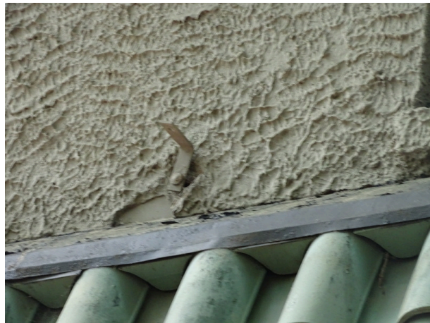
Exterior stucco wall - note deterioration
