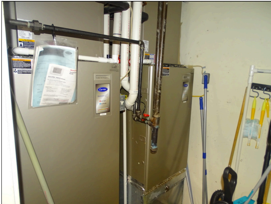
28 - Typical gas furnace and air handler units
