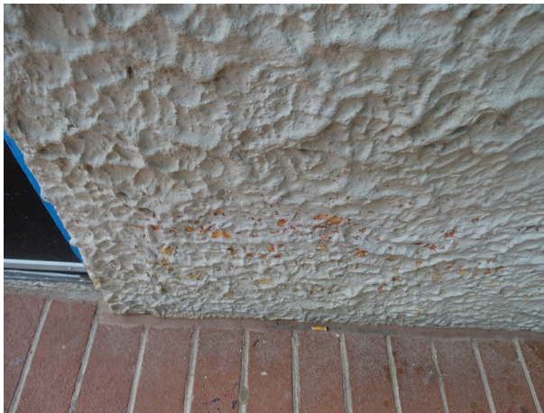
Exterior stucco wall - note deterioration
