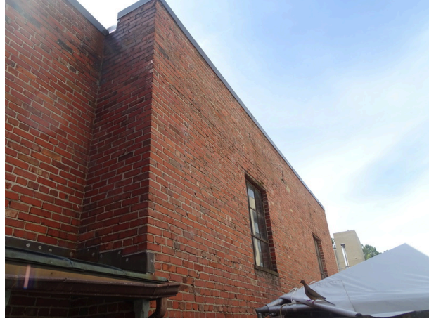
Brick exterior at west side of the building - note deterioration above window
