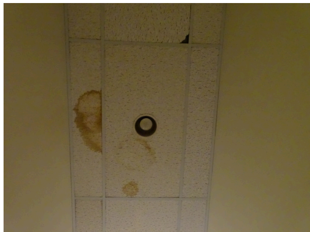
Typical ceiling - note water leakage
