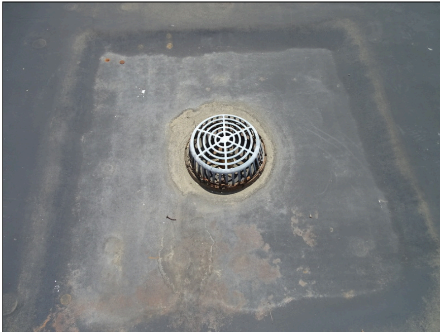
22 - Typical interior drain
