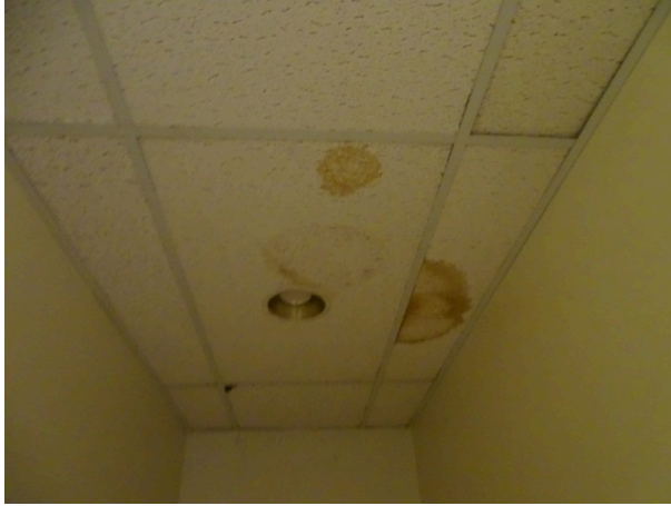
Typical ceiling - note water leakage
