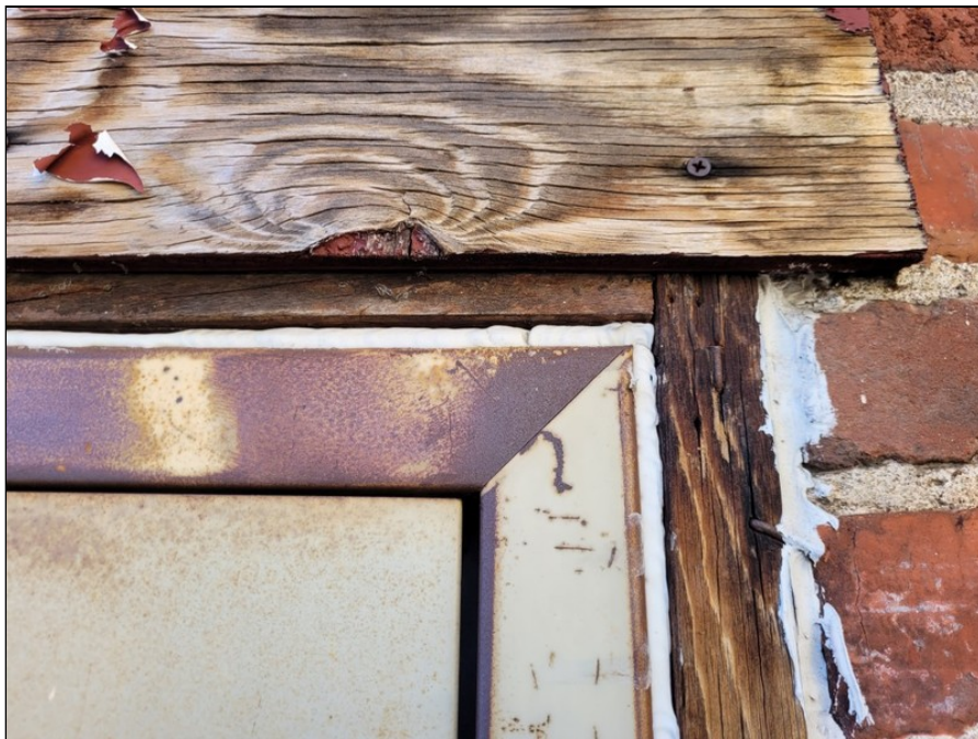
52 - Rear door sealant condition
