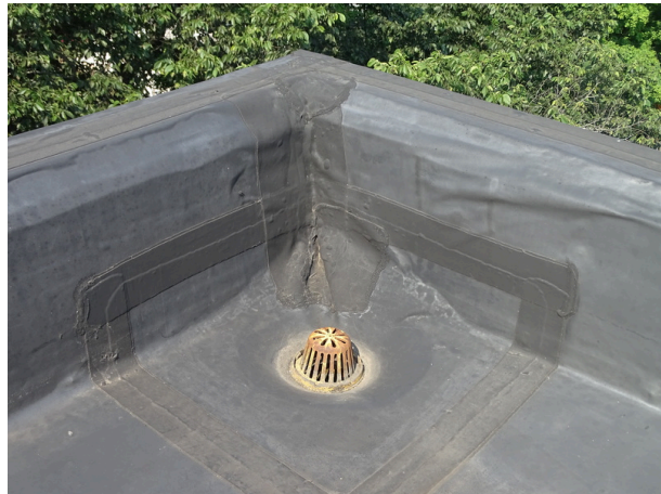
Typical internal drain
