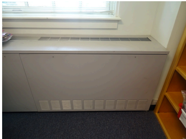
Typical water source heat pump
