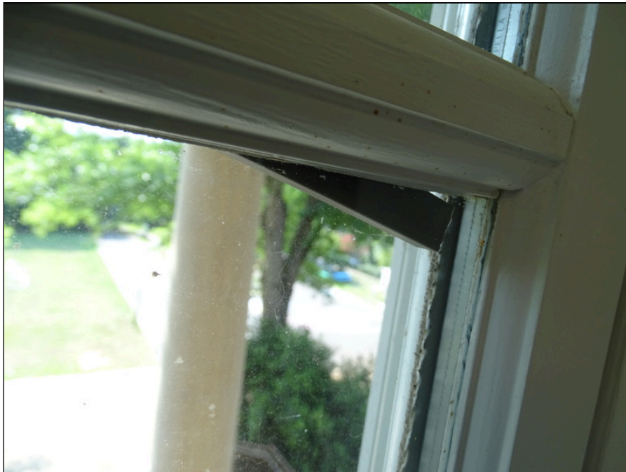
48 - Typical exterior window - note gasket damaged
