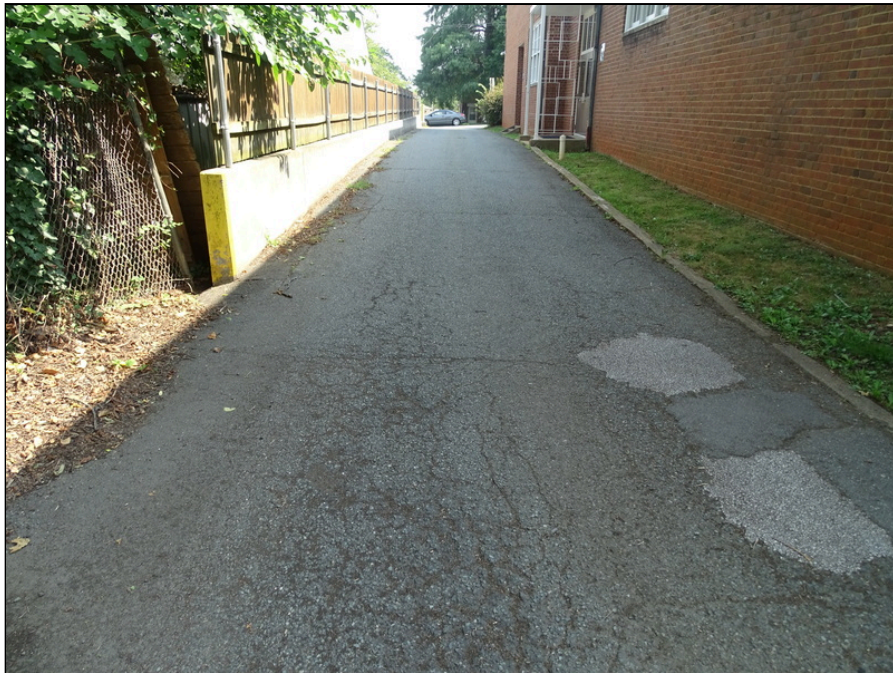
6 - Asphalt pavement - note cracking
