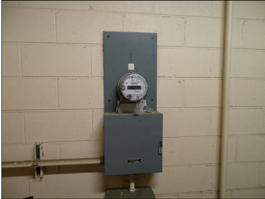
69 - Electrical meter located in main utility room
