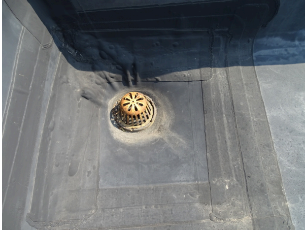
Typical internal drain
