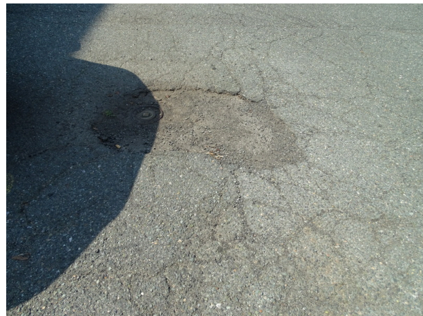
Storm water drainage on west side of building and site - note ponding reported and deterioration
