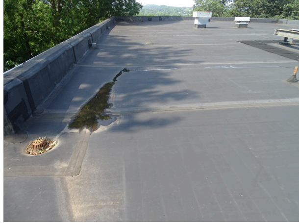
Single-ply membrane roofing system - note ponding
