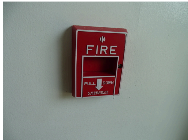
Typical fire alarm pull station
