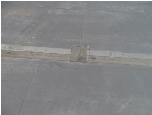
Single-ply membrane roofing system addition - note patching
