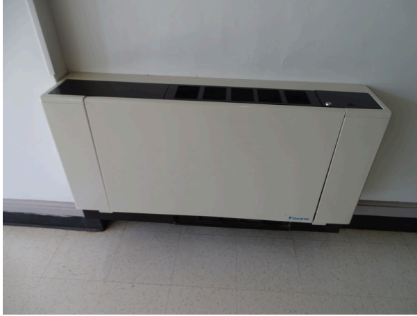
Typical water source heat pump
