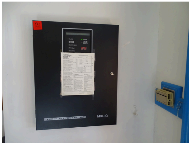
Fire alarm control panel
