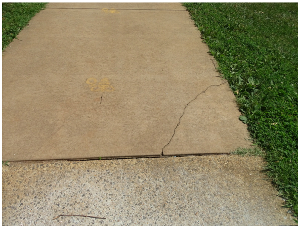
Typical concrete sidewalk - note cracking
