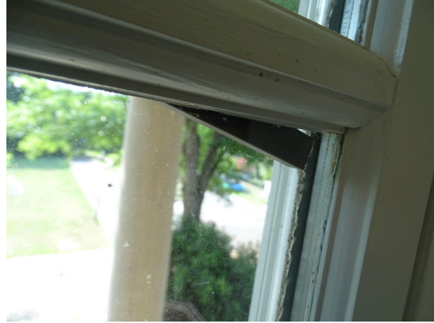
Typical exterior window - note gasket damaged
