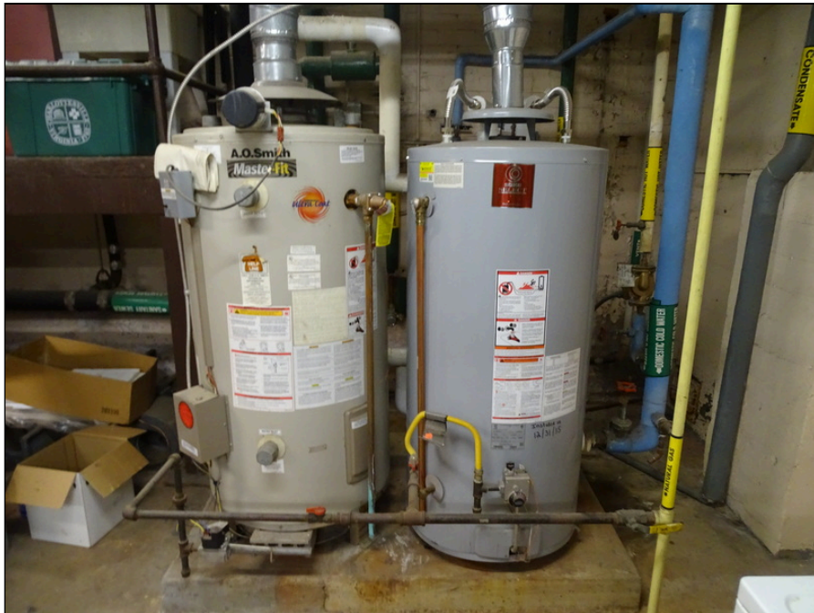
58 - Gas domestic water heaters
