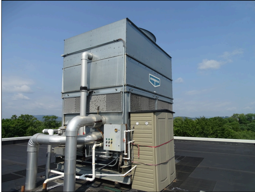
61 - Cooling tower located on roof
