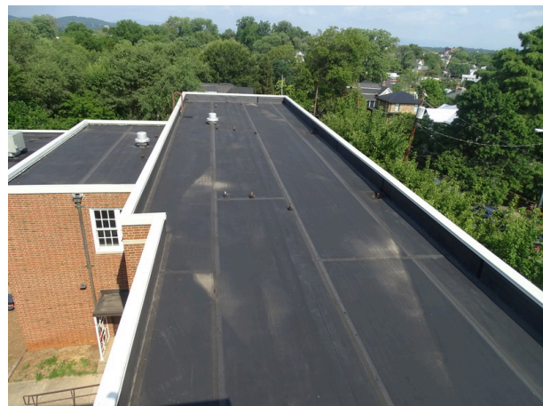
Single-ply membrane roofing system addition
