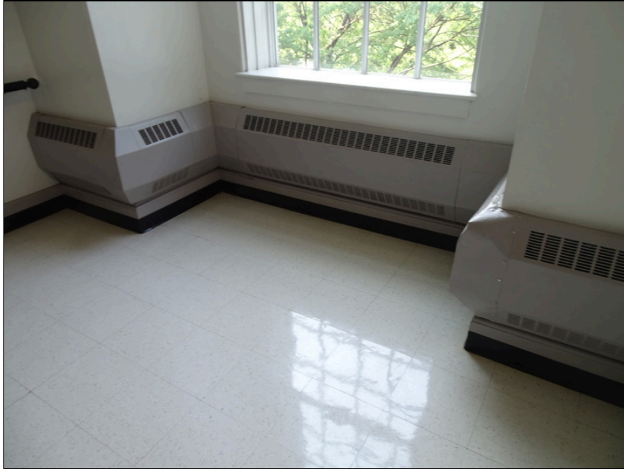
63 - Typical water source heat pump
