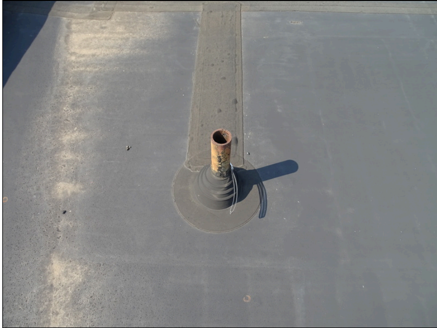
57 - Typical plumbing penetration
