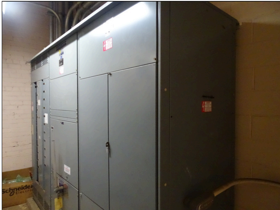
68 - Electrical main switchgear
