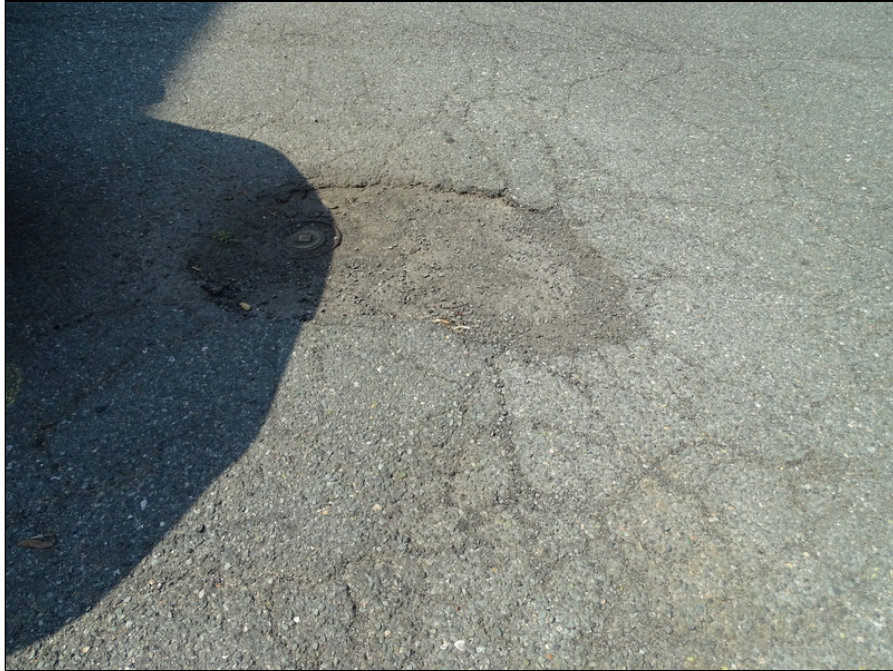
7 - Asphalt parking - note minor cracking and deterioration
