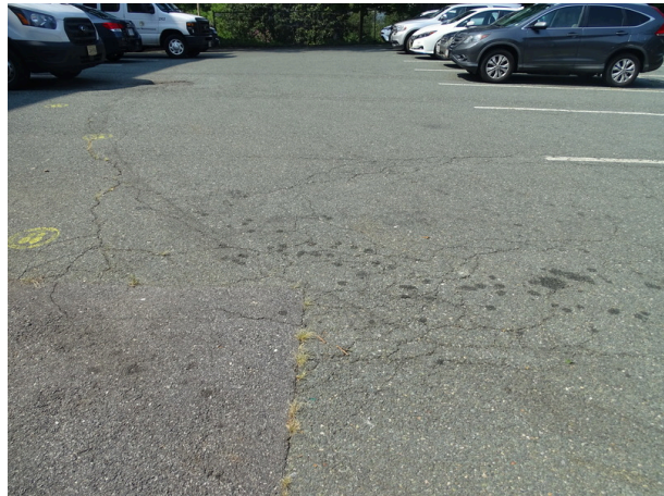
Asphalt parking - note cracking
