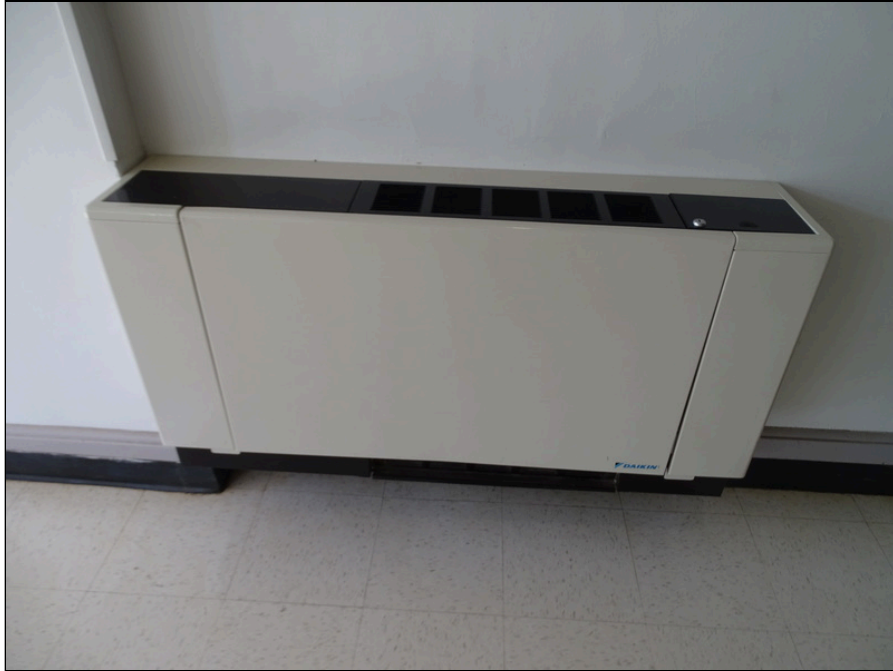
65 - Typical water source heat pump
