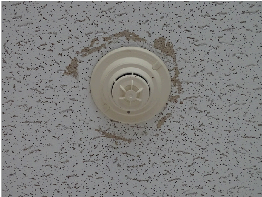
80 - Typical smoke detector
