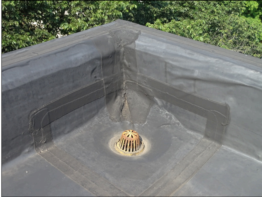
55 - Typical internal drain
