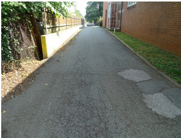
Storm water drainage on west side of building and site - note ponding reported and deterioration
