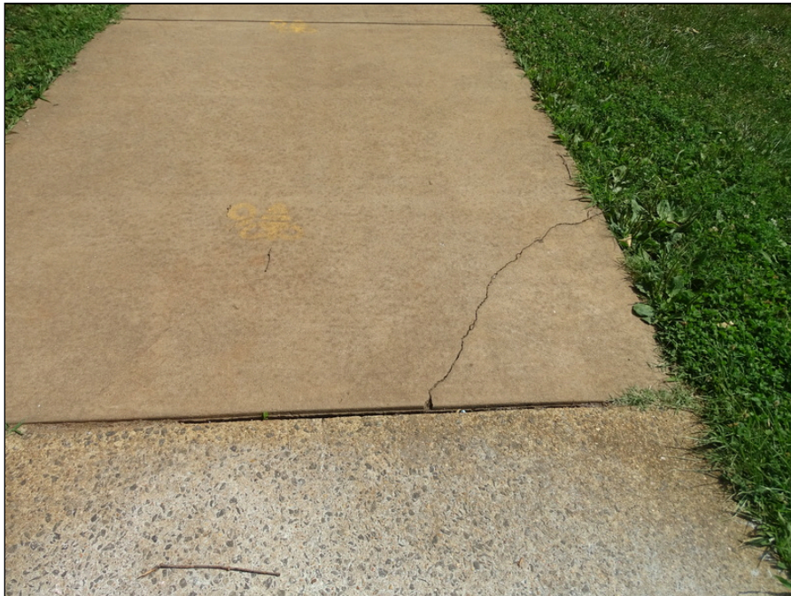
12 - Typical concrete sidewalk - note cracking
