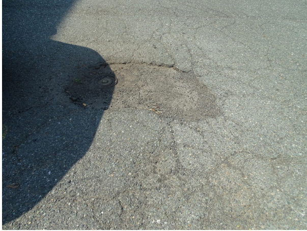
Asphalt parking - note minor cracking and deterioration
