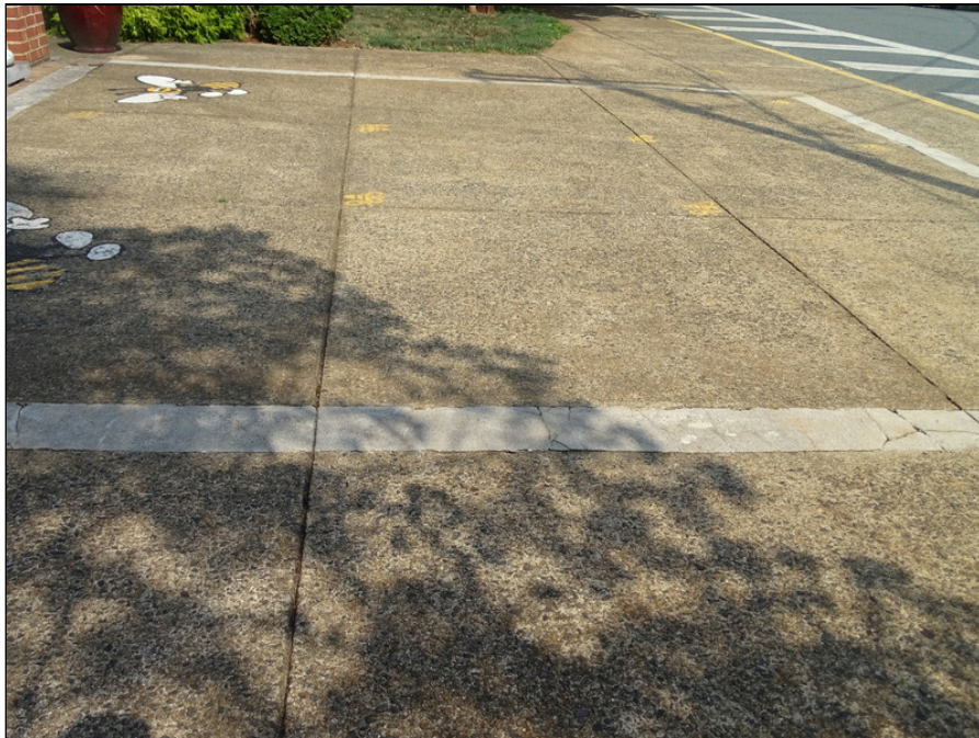
8 - Typical concrete sidewalk - note cracking
