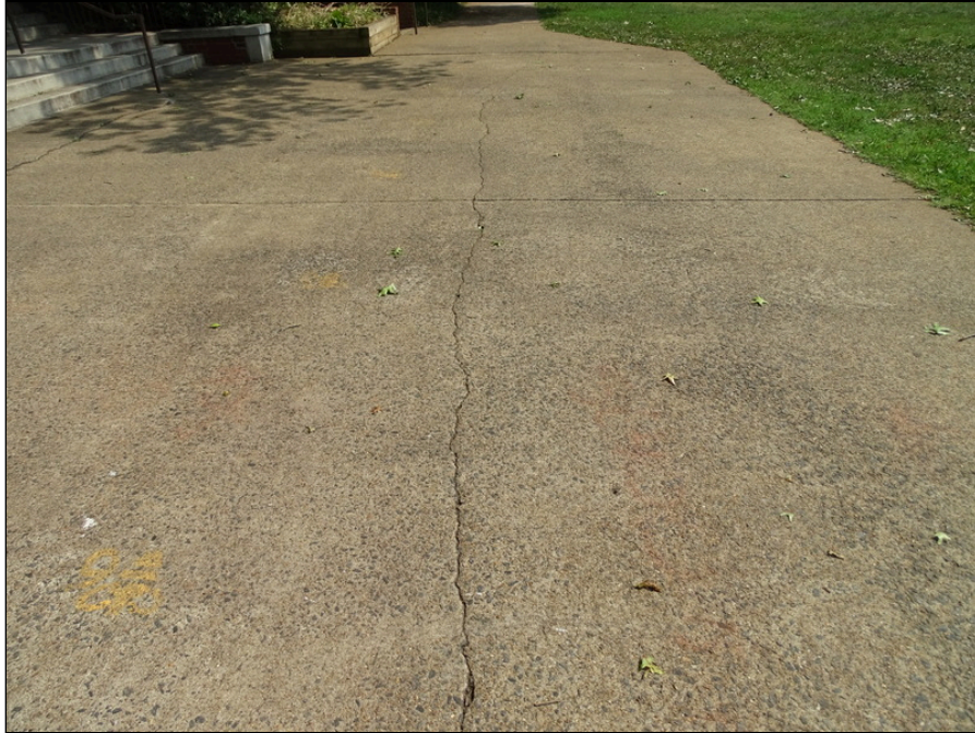
9 - Typical concrete sidewalk - note cracking
