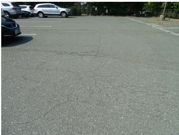
Asphalt parking - note cracking
