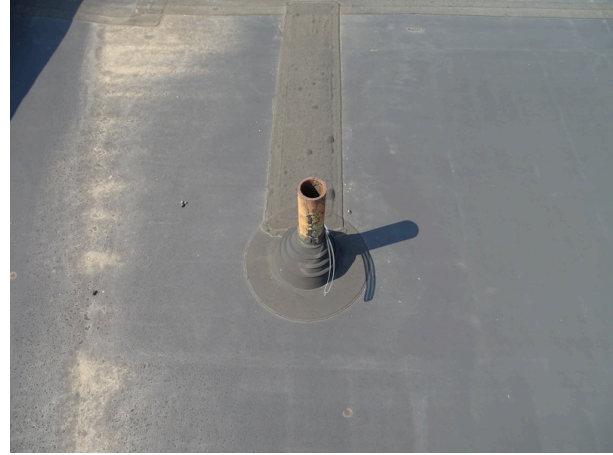
Typical plumbing penetration
