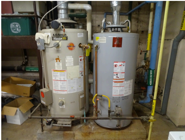
Gas domestic water heaters
