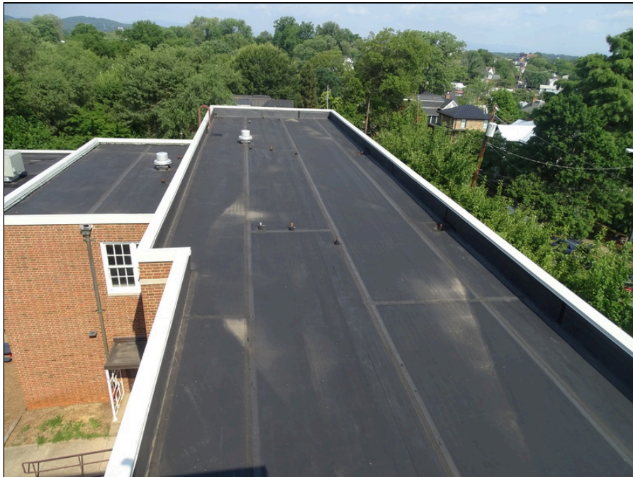
50 - Single-ply membrane roofing system addition
