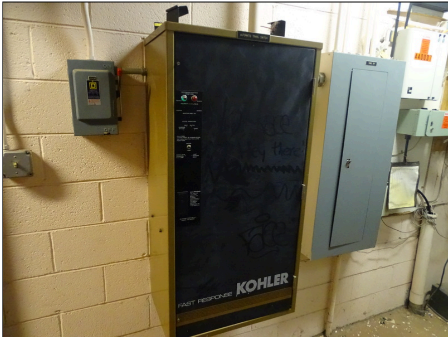
70 - Emergency power transfer switch
