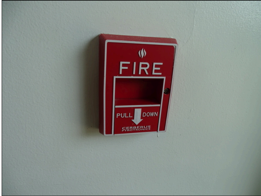
77 - Typical fire alarm pull station
