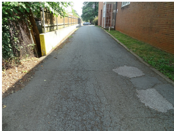
Asphalt pavement - note cracking
