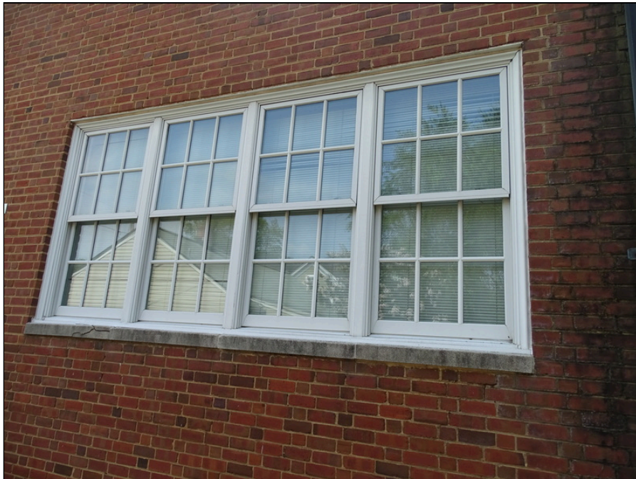
46 - Typical exterior window - note sill cracking
