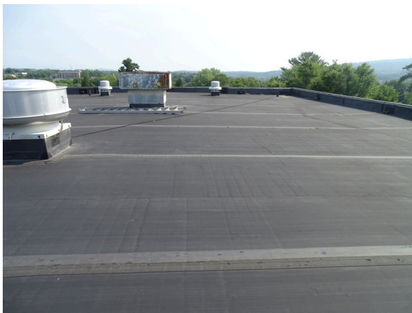
Single-ply membrane roofing system looking north
