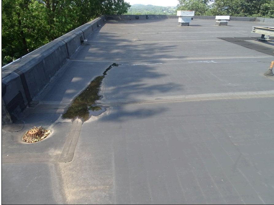
53 - Single-ply membrane roofing system - note ponding
