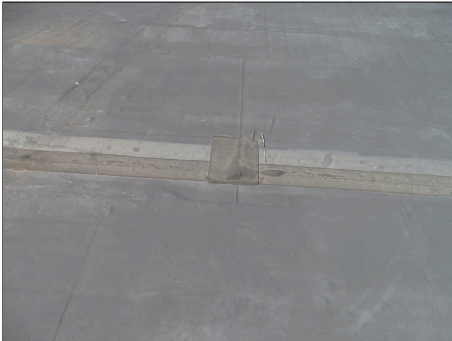
54 - Single-ply membrane roofing system addition - note patching
