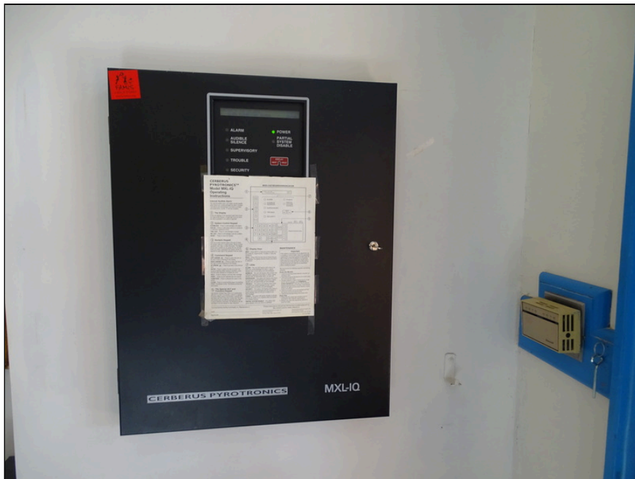
76 - Fire alarm control panel
