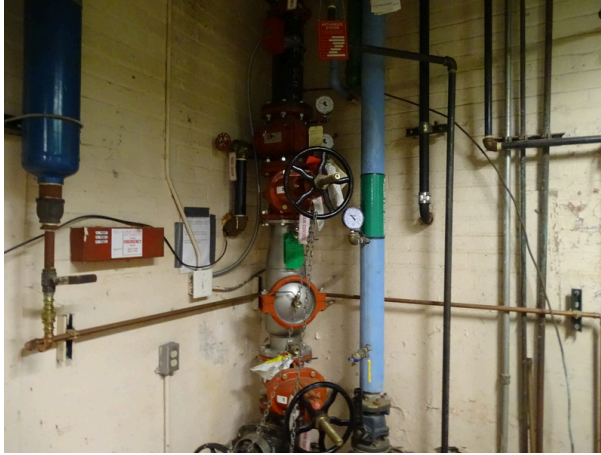
Fire sprinkler system located in main utility room
