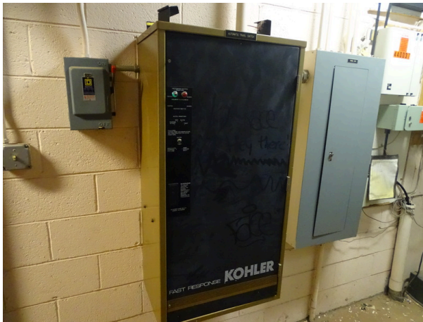
Emergency power transfer switch
