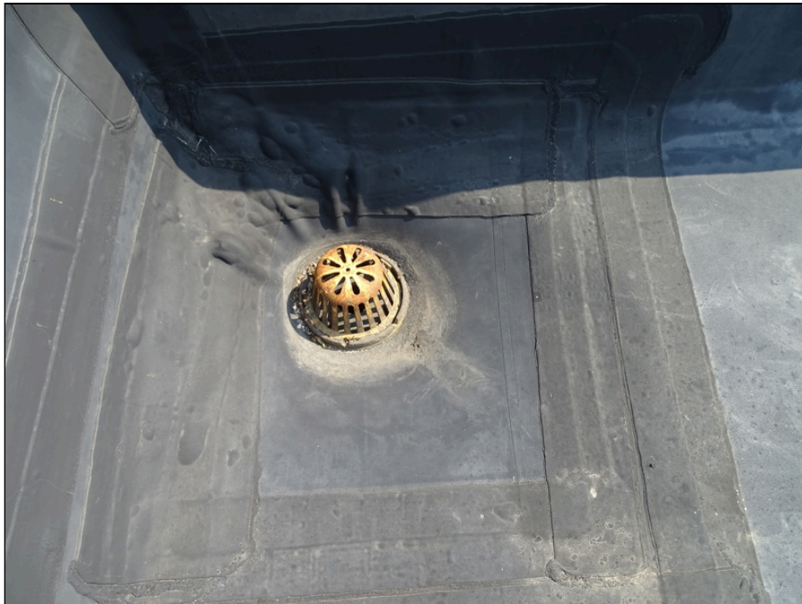
56 - Typical internal drain
