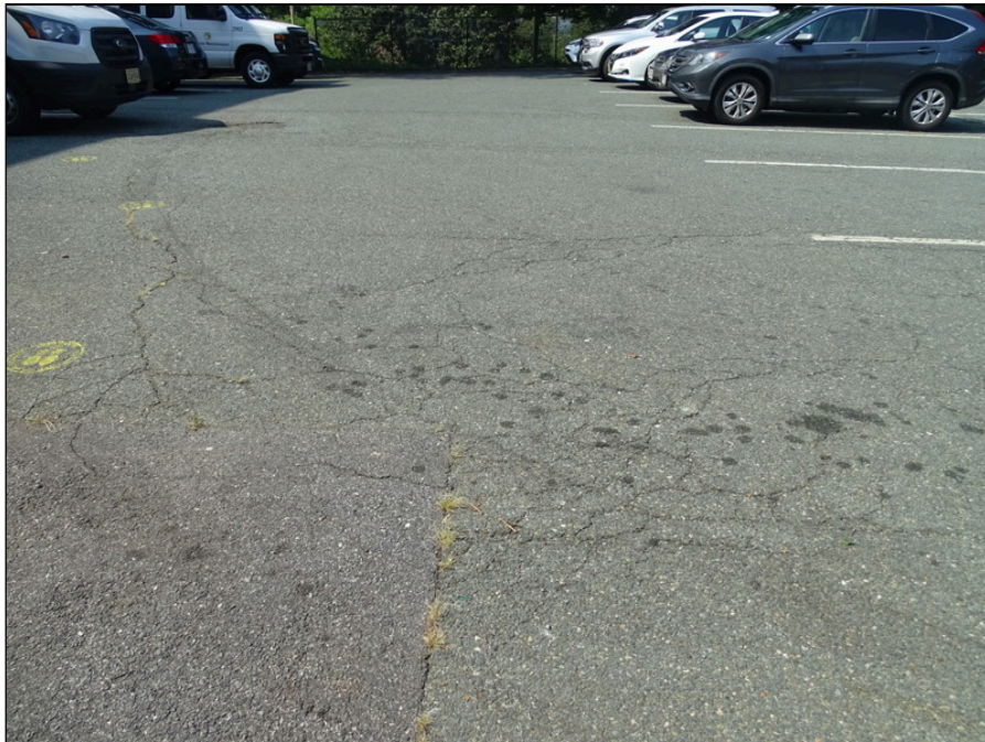
4 - Asphalt parking - note cracking
