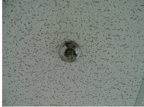
Typical fire sprinkler head
