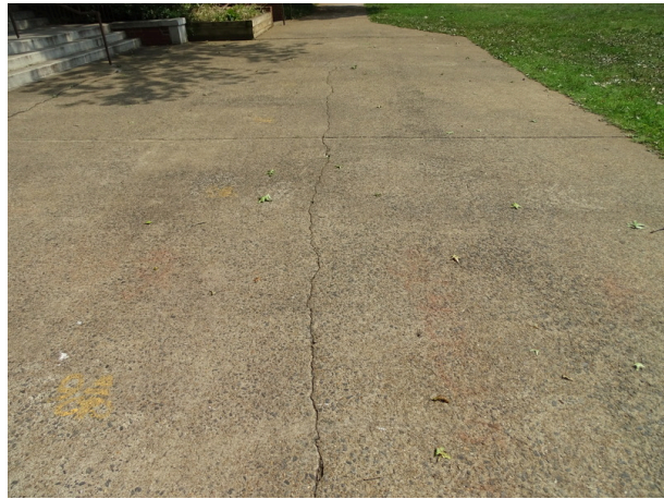
Typical concrete sidewalk - note cracking
