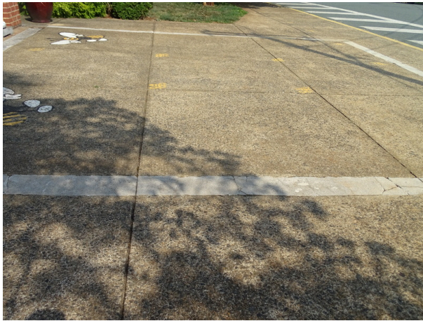
Typical concrete sidewalk - note cracking
