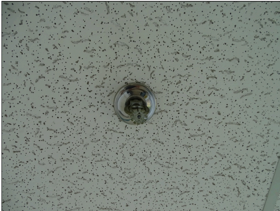
74 - Typical fire sprinkler head
