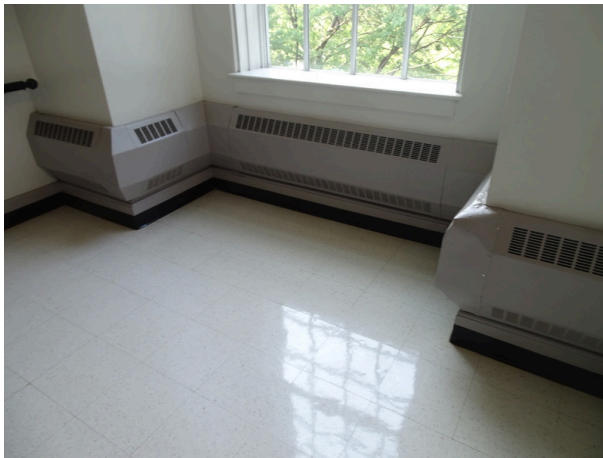
Typical water source heat pump
