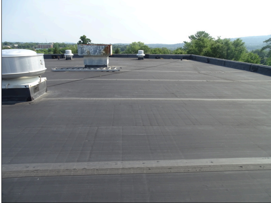
49 - Single-ply membrane roofing system looking north
