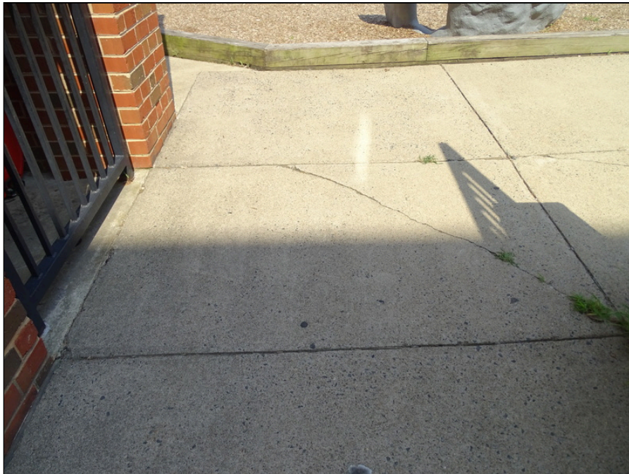
10 - Typical concrete sidewalk - note cracking
