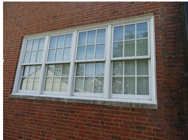
Typical exterior window - note sill cracking
