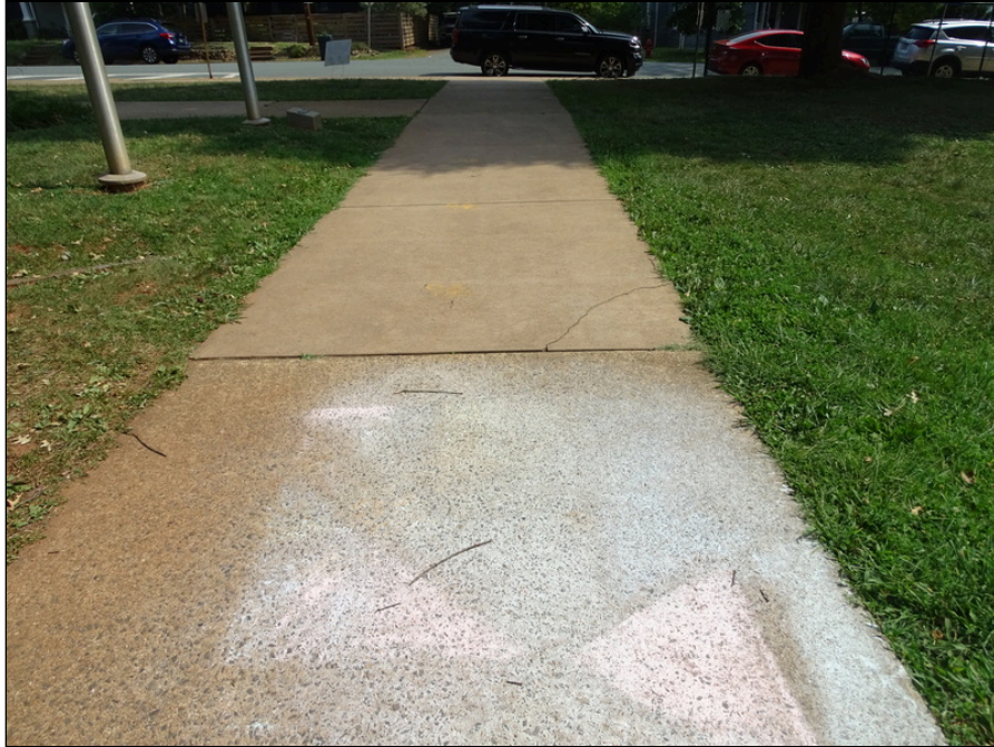
11 - Typical concrete sidewalk - note cracking
