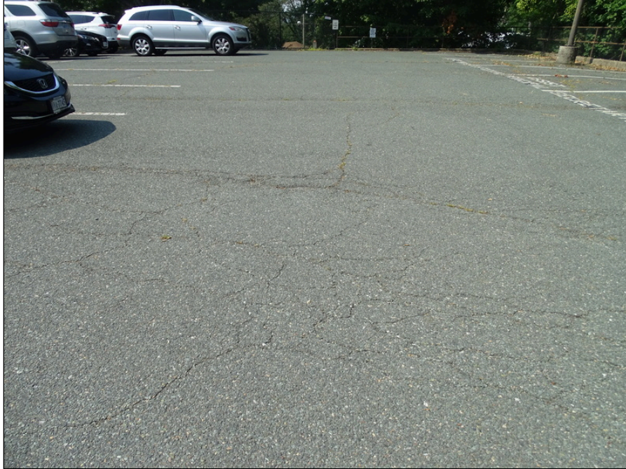
5 - Asphalt parking - note cracking
