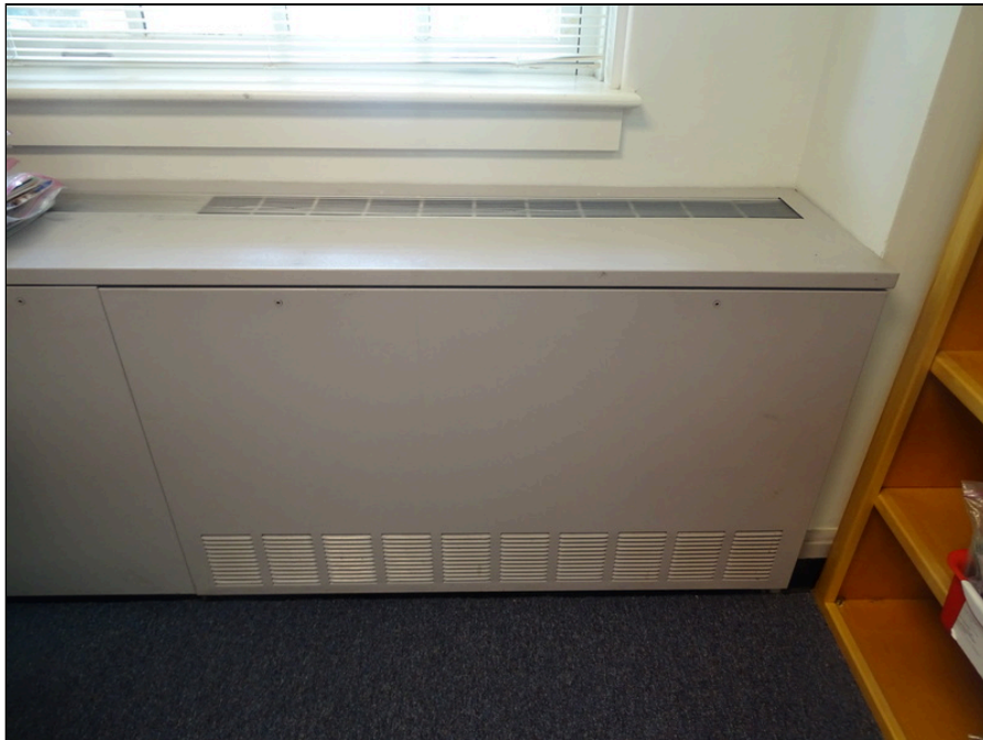
64 - Typical water source heat pump
