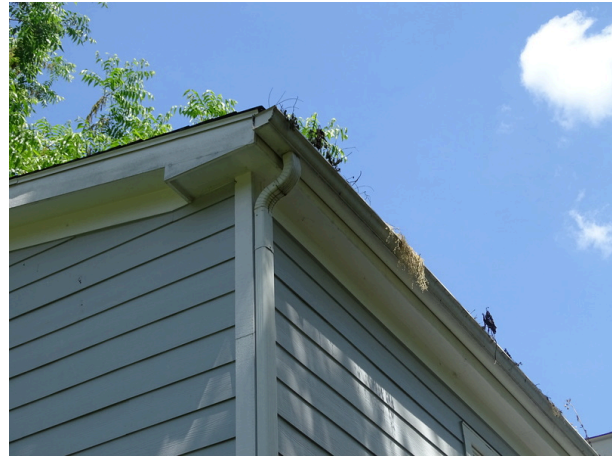
Typical gutter and downspout
