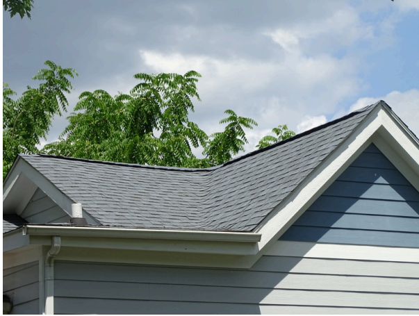
Asphalt shingle roofing system
