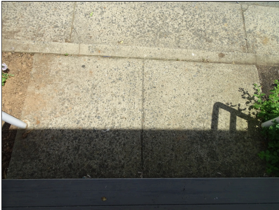
4 - Concrete sidewalk - note cracking
