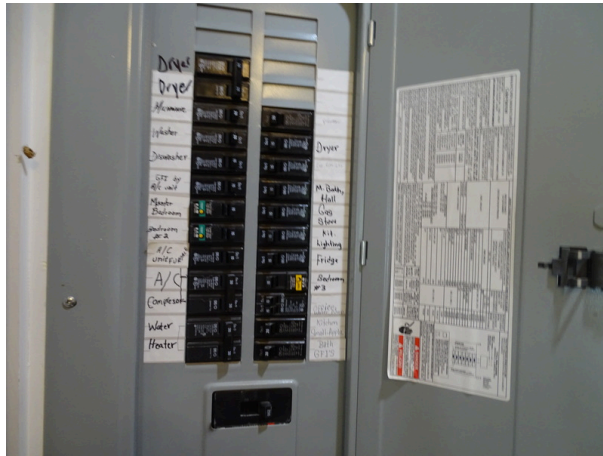
Electrical main disconnect and breaker panel
