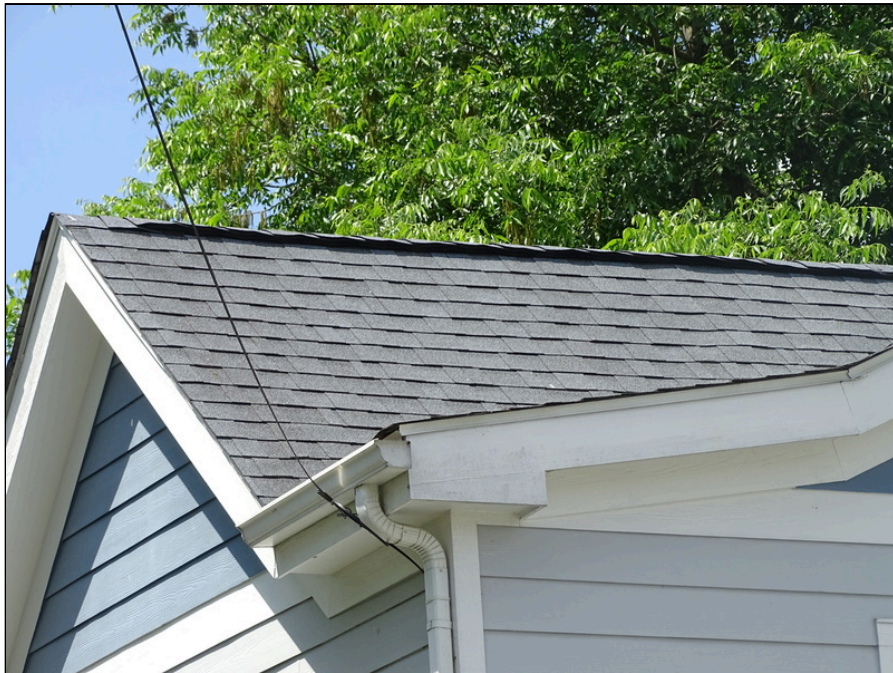
22 - Asphalt shingle roofing system
