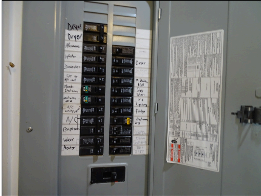
33 - Electrical main disconnect and breaker panel
