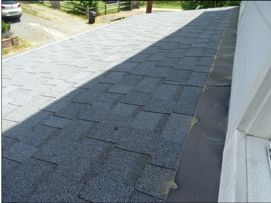
25 - Asphalt shingle roofing system
