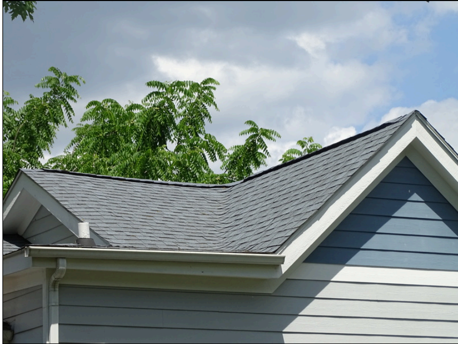
23 - Asphalt shingle roofing system
