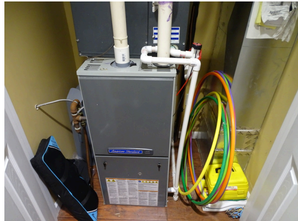
Furnace unit and Air Handler unit
