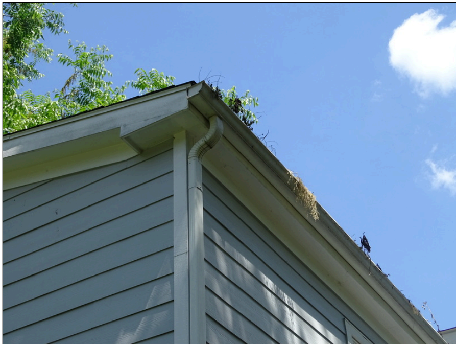
26 - Typical gutter and downspout
