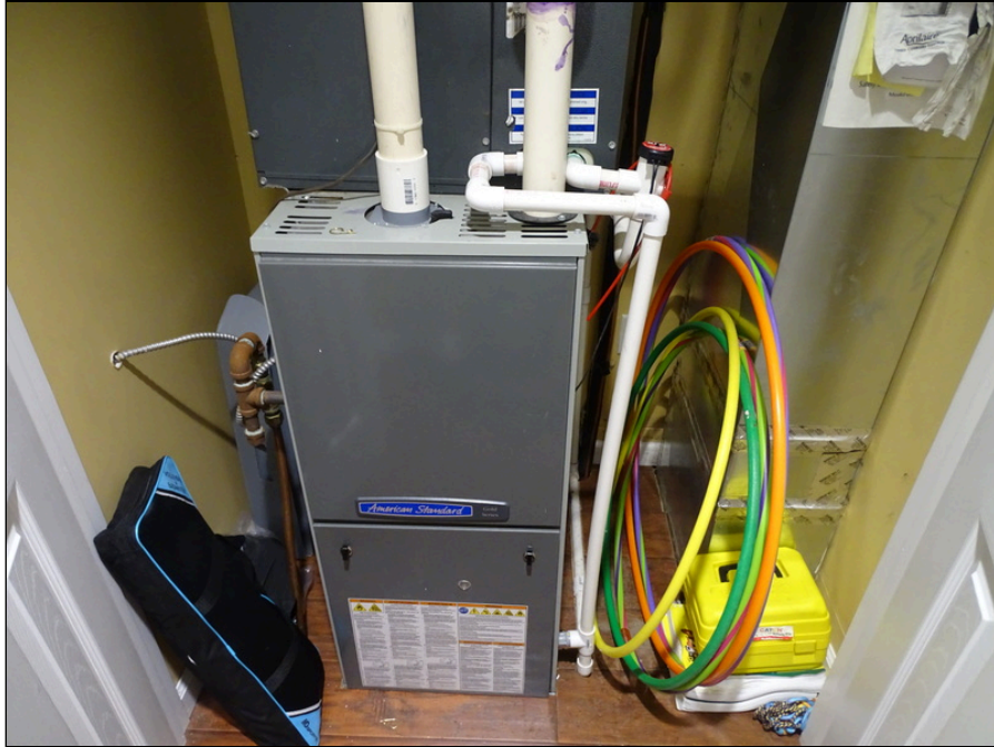
29 - Furnace unit and Air Handler unit
