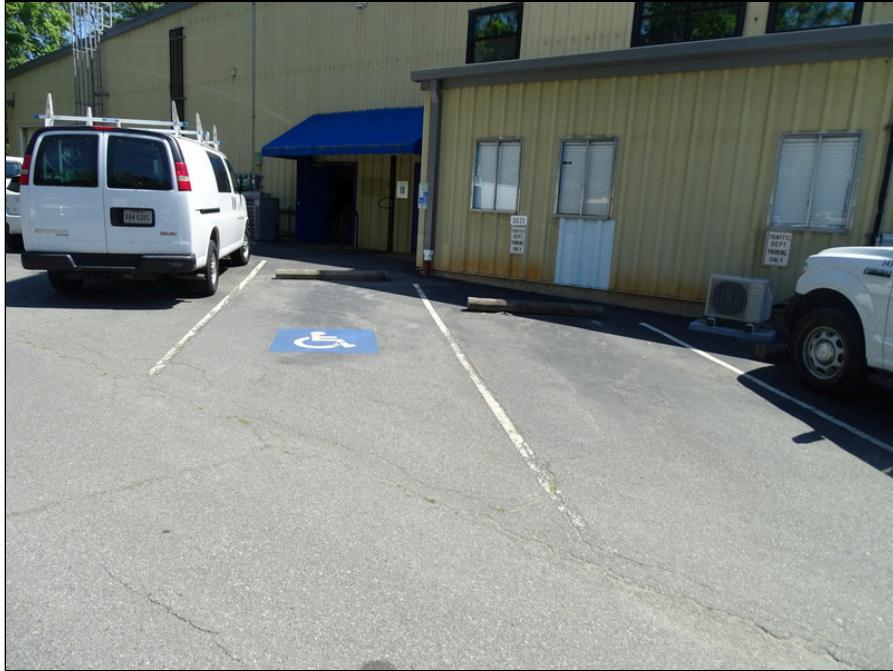
91 - Accessible parking space - note striping faded
