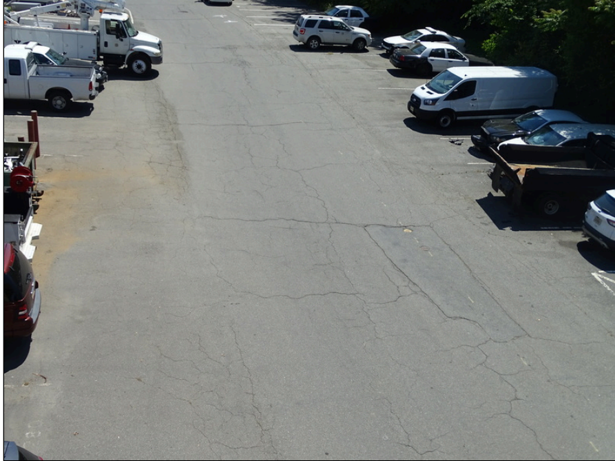
3 - Asphalt pavement west side of the site - note cracking
