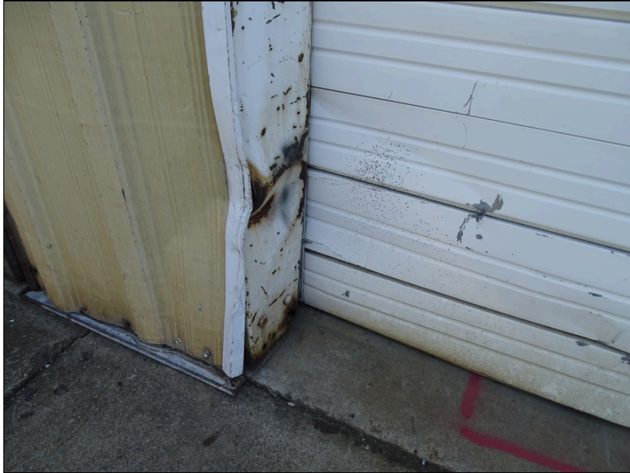
37 - Typical overhead door - note physical damaged
