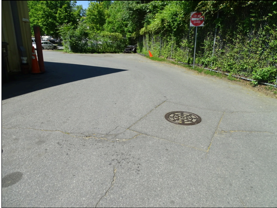
7 - Typical asphalt pavement - note cracking
