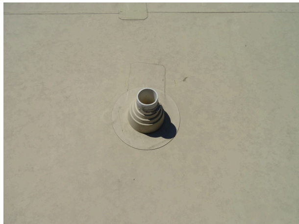
Typical plumbing penetration
