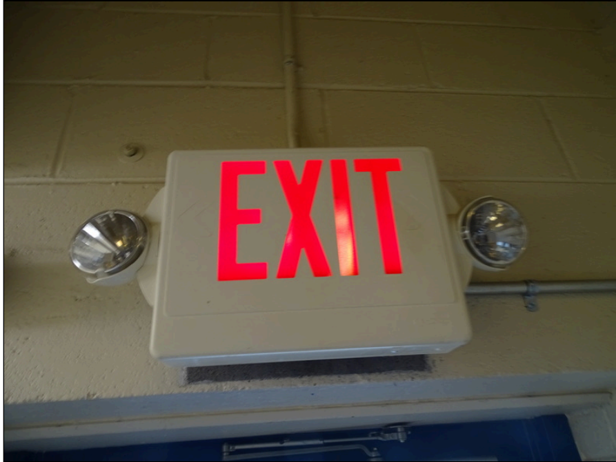
75 - Typical exit sign with emergency lighting
