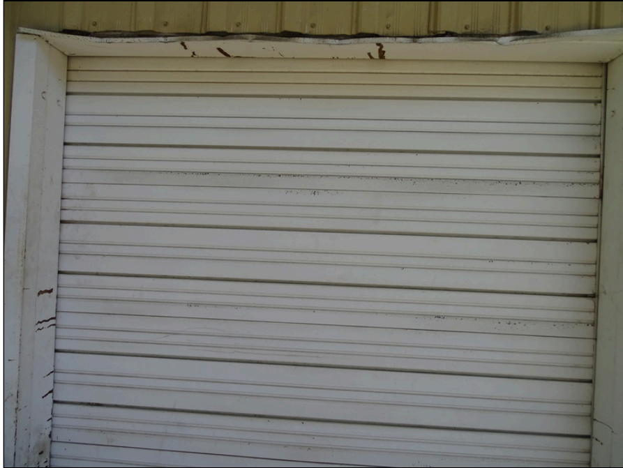
39 - Typical overhead door - note damaged
