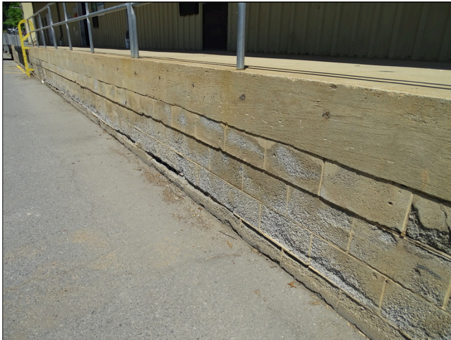
10 - Concrete sidewalk and loading area at south side of the building - note deterioration
