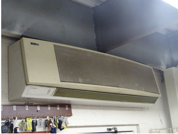
Ductless Split System Wall Mounted Unit
