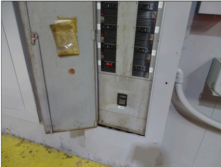
72 - Main electrical disconnect,
