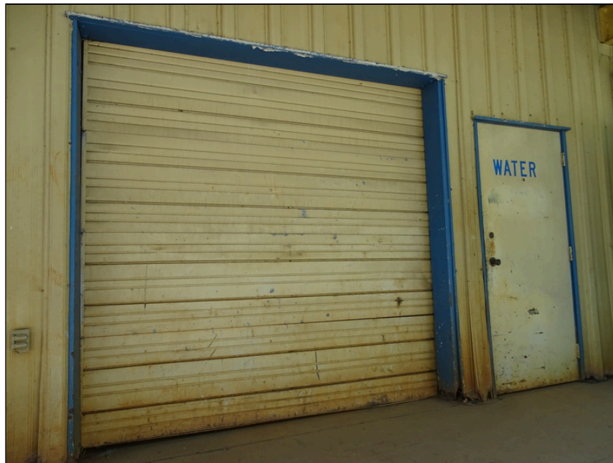
36 - Typical overhead door - note deterioration
