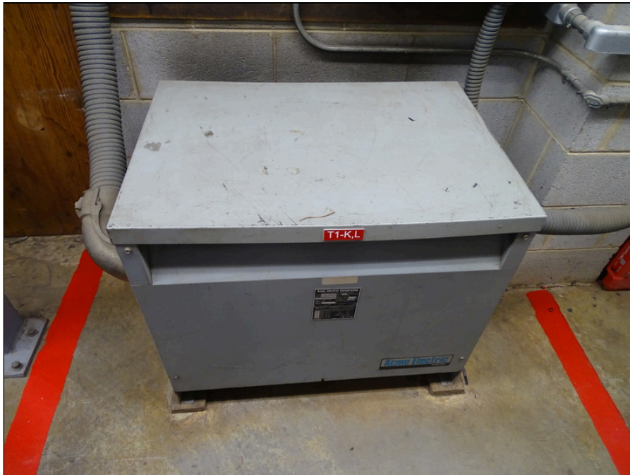
70 - Typical building transformer
