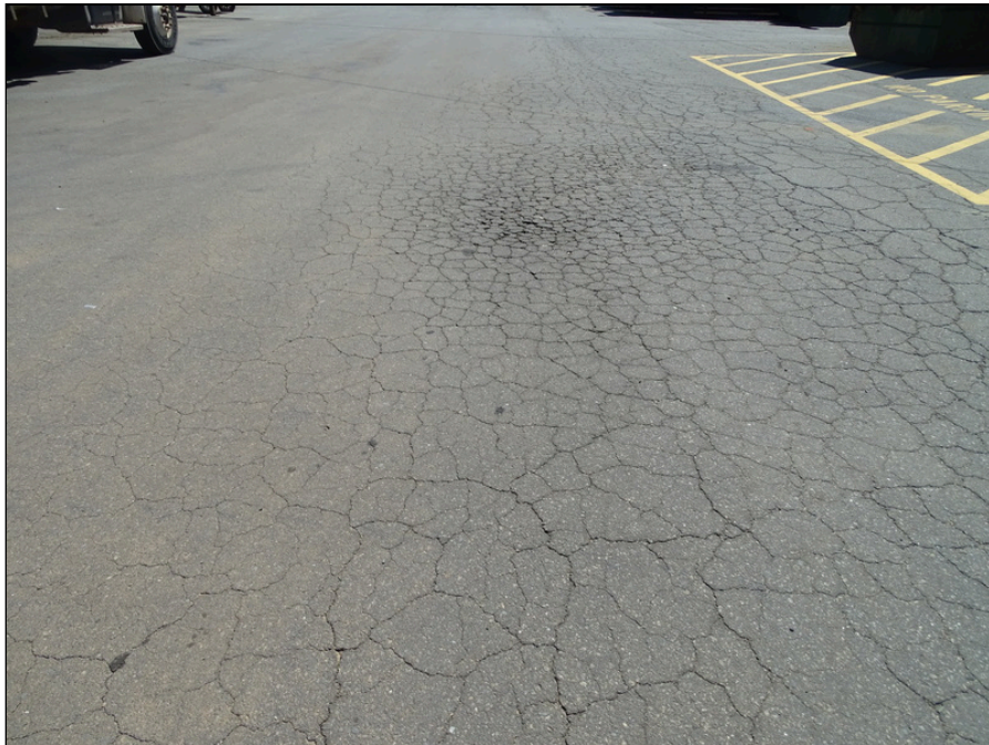
4 - Asphalt pavement west side of the site - note alligator cracks
