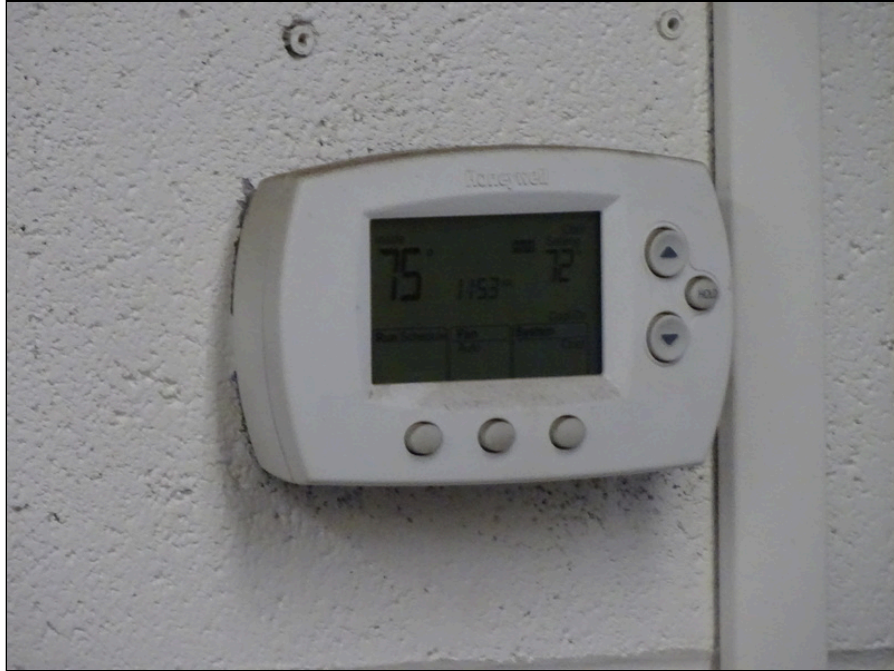
65 - Typical digital thermostat
