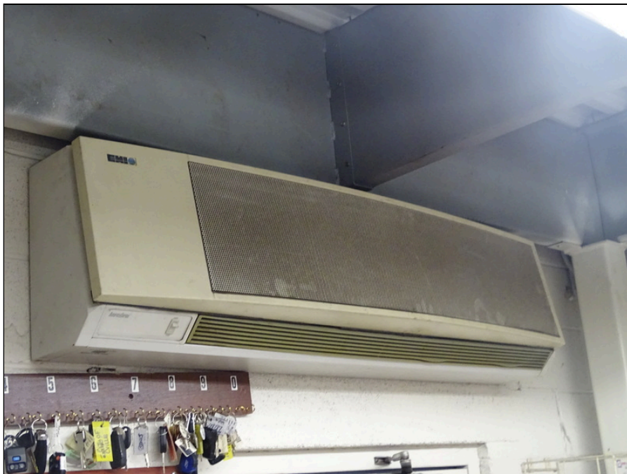
60 - Ductless Split System Wall Mounted Unit
