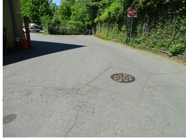
Typical asphalt pavement - note cracking
