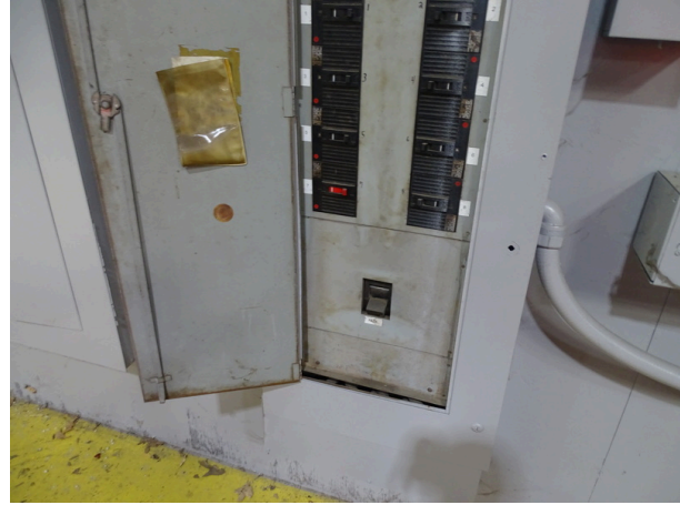
Main electrical disconnect,
