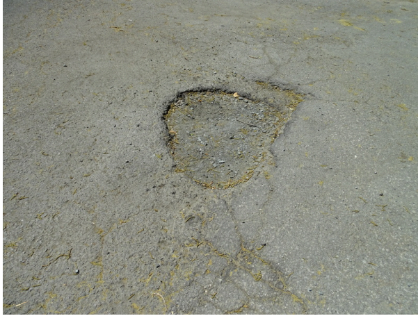
Asphalt pavement - note deterioration
