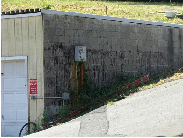
Adjacent garage wall - note efflorescence
