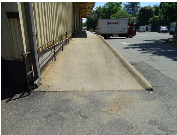
Accessible concrete ramp at southwest side of the building
