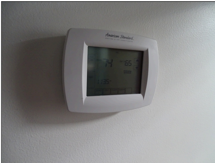
64 - Typical digital thermostat
