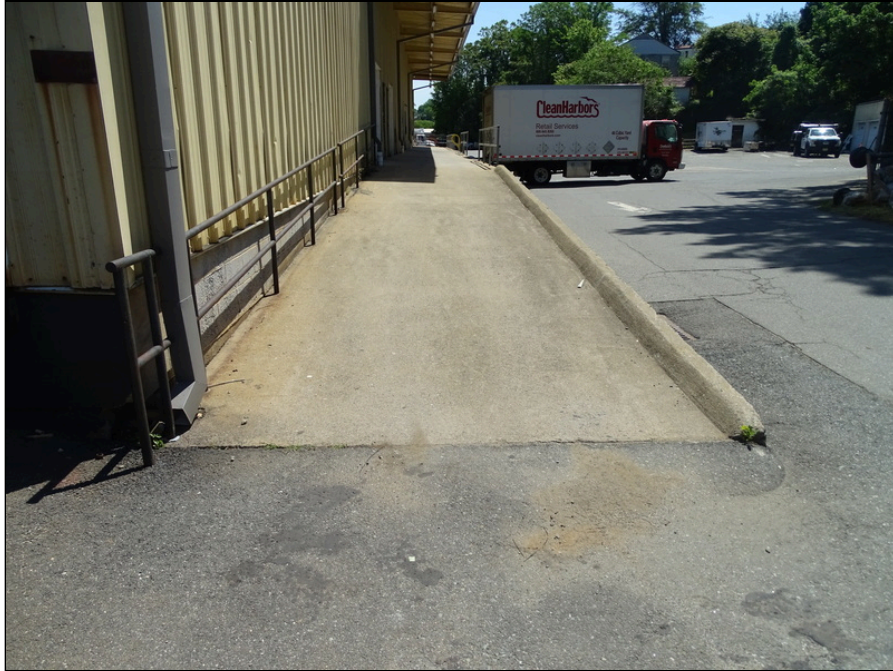
93 - Accessible concrete ramp at southwest side of the building
