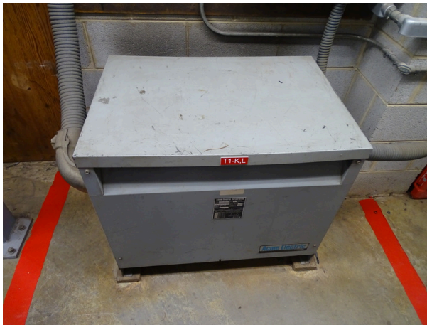
Typical building transformer
