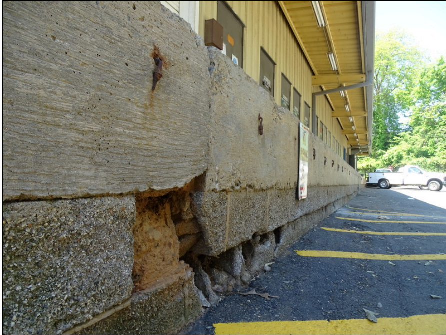
13 - Concrete loading area at north side of the building - note deterioration
