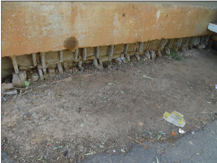
12 - Concrete loading area at north side of the building - note deterioration
