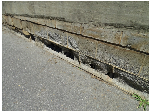
Concrete loading area at north side of the building - note deterioration
