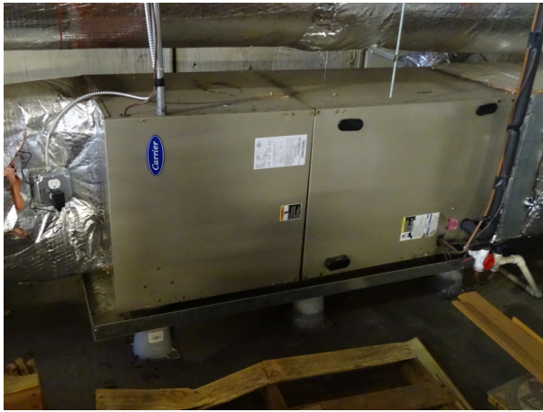
Typical air handler unit located in attic area
