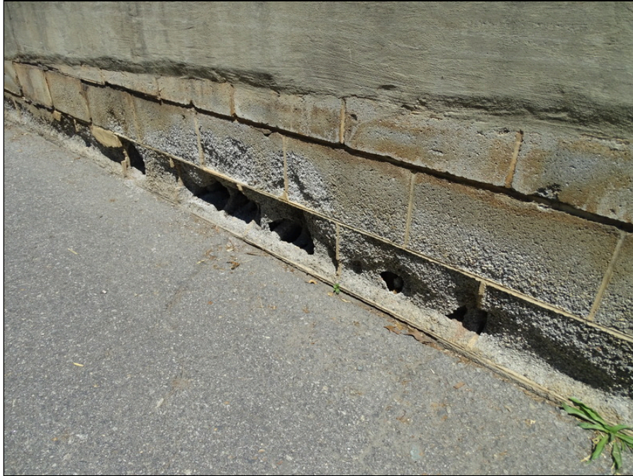
11 - Concrete loading area at north side of the building - note deterioration
