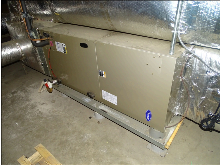
55 - Typical air handler unit located in attic area
