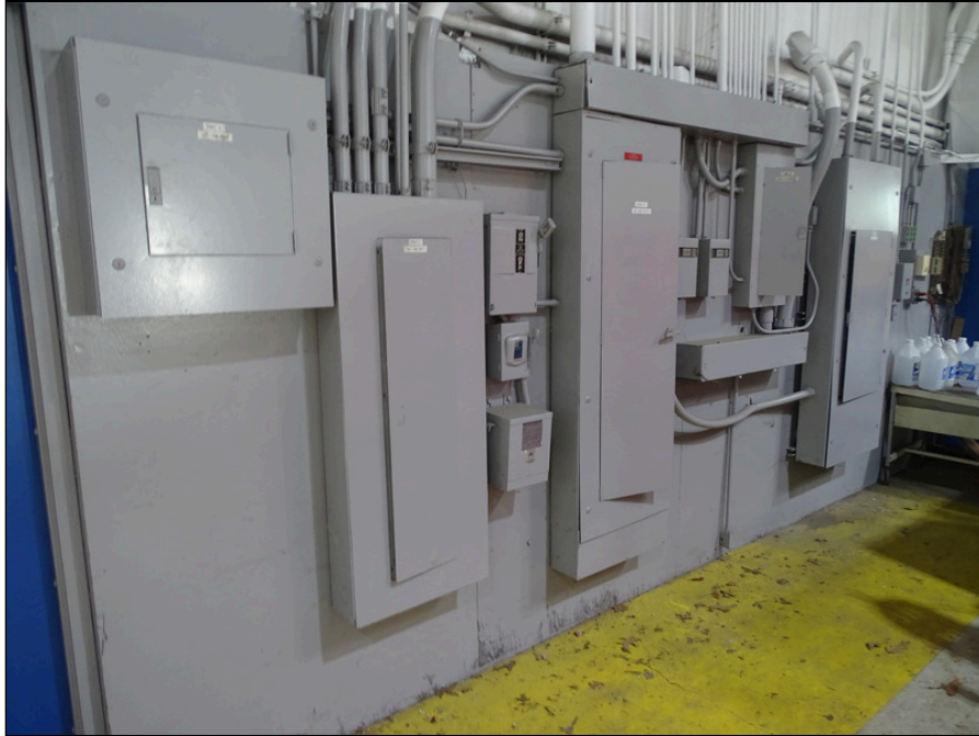
71 - Main electrical disconnect, utility meter, and emergency transfer switch
