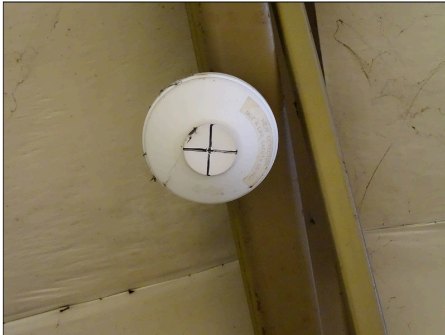
74 - Typical smoke detector
