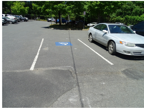
Accessible parking space - note striping faded
