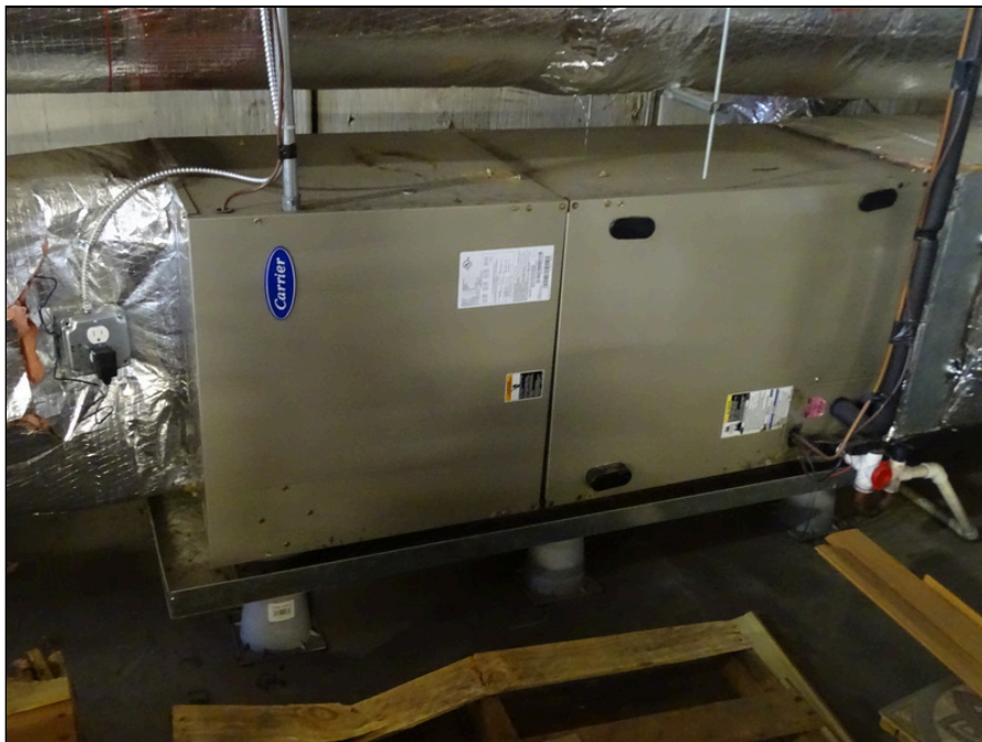
54 - Typical air handler unit located in attic area
