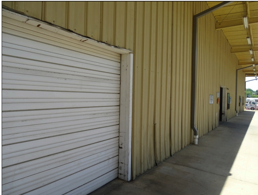
28 - Typical building exterior - note metal siding physical damage
