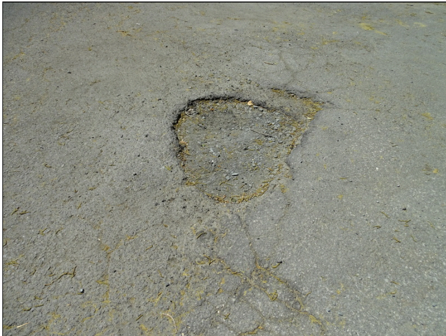
6 - Asphalt pavement - note deterioration
