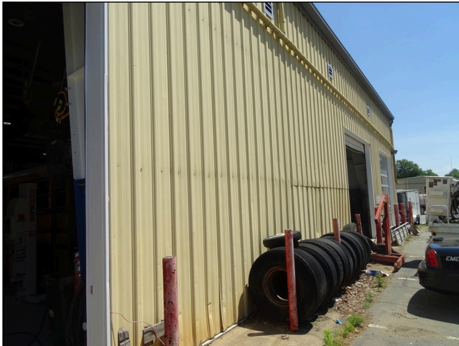
30 - Typical building exterior - note metal siding physical damage
