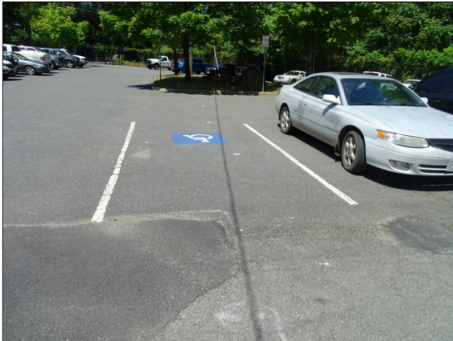
92 - Accessible parking space - note striping faded
