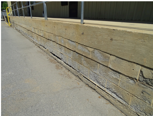
Concrete sidewalk and loading area at south side of the building - note deterioration
