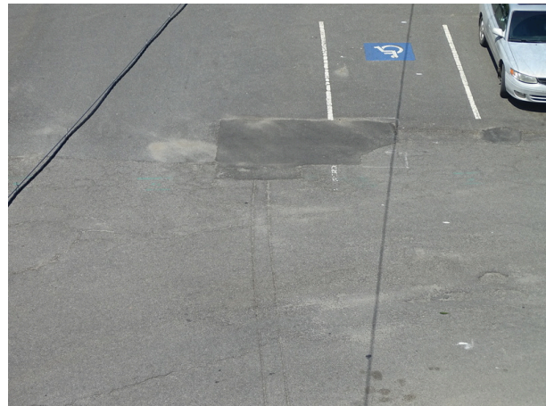
Asphalt pavement - note previous repair
