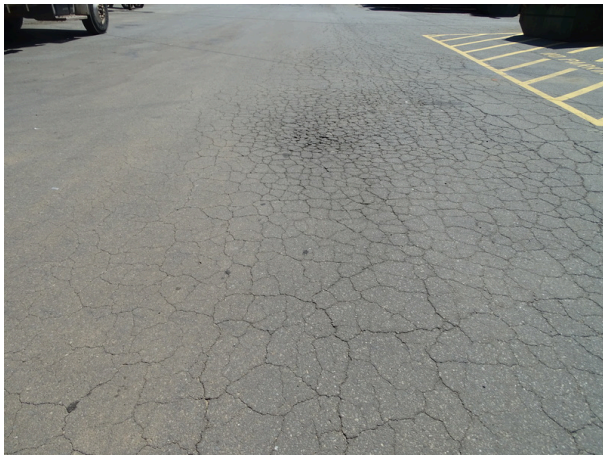
Asphalt pavement west side of the site - note alligator cracks
