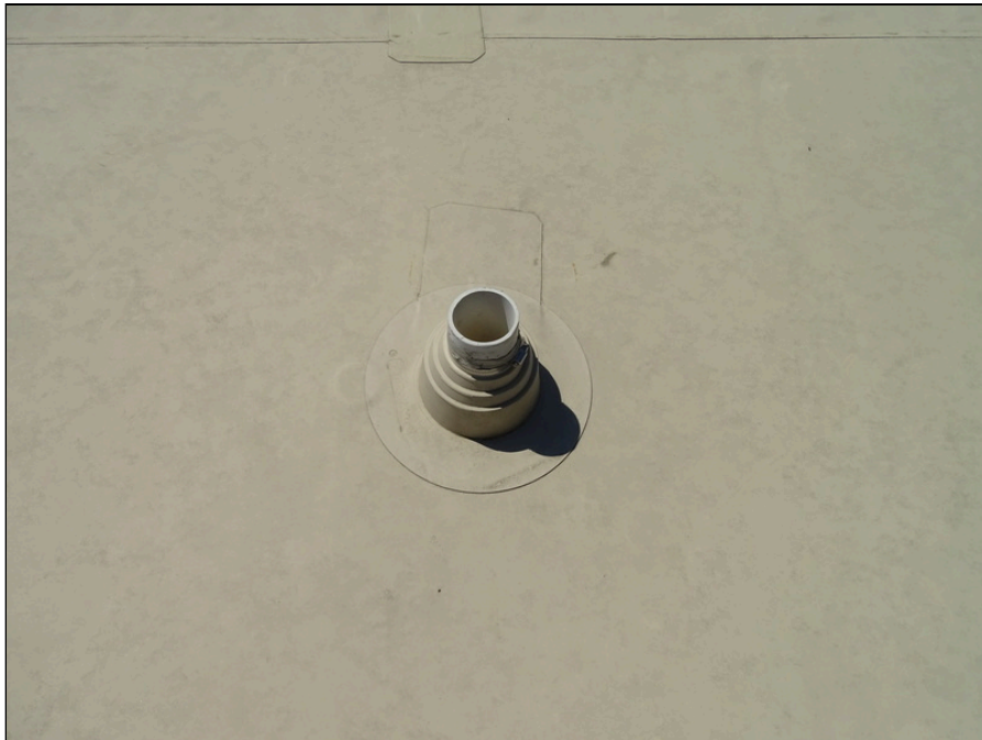
46 - Typical plumbing penetration
