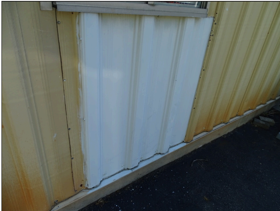
38 - Building exterior - note patching
