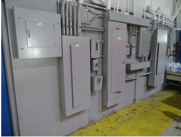
Main electrical disconnect, utility meter, and emergency transfer switch
