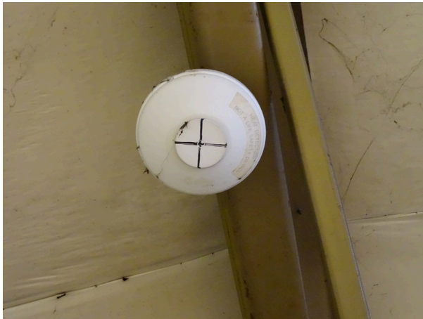
Typical smoke detector
