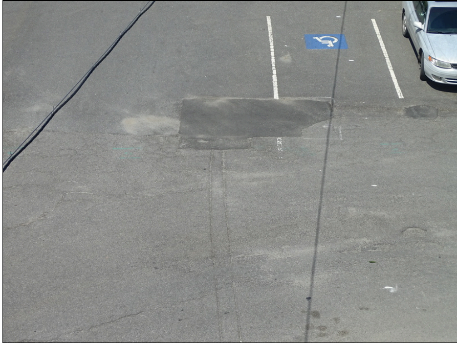
5 - Asphalt pavement - note previous repair
