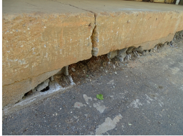
Typical concrete sidewalk - note deterioration
