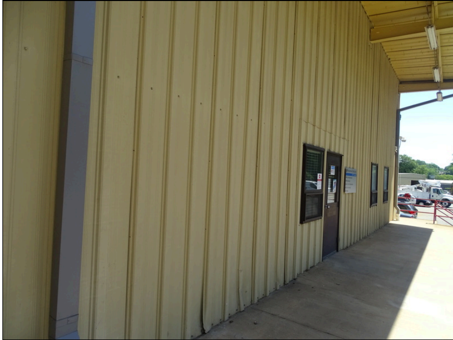
29 - Typical building exterior - note metal siding physical damage
