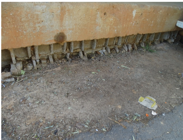
Concrete loading area at north side of the building - note deterioration
