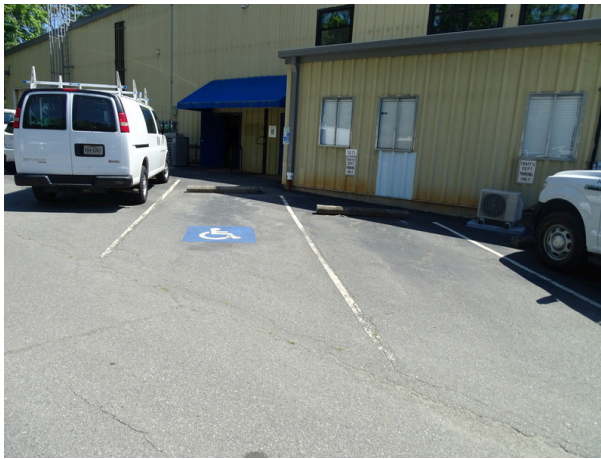
Accessible parking space - note striping faded
