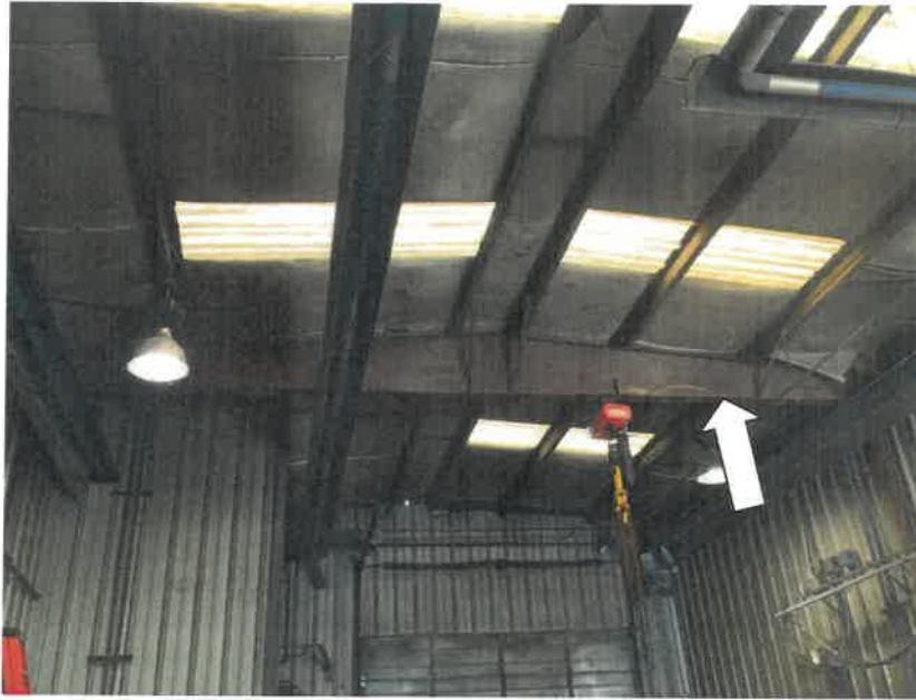
Elevated structural steel with little corrosion.
