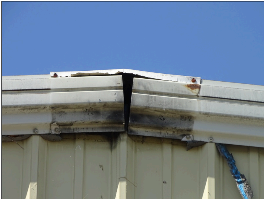
18 - Roofing system of bus wash building - note deterioration
