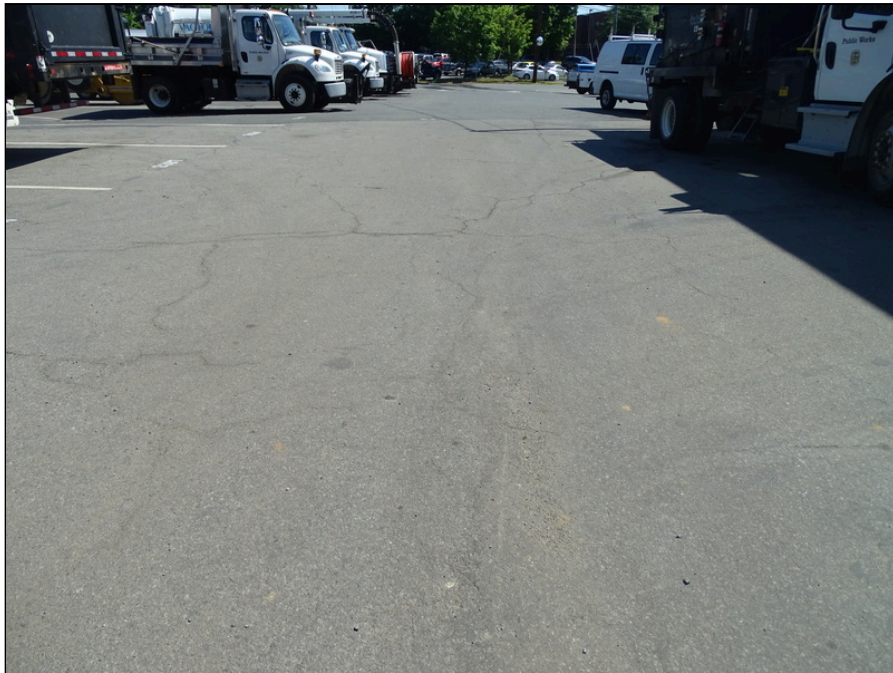
2 - Asphalt pavement and parking - note cracking
