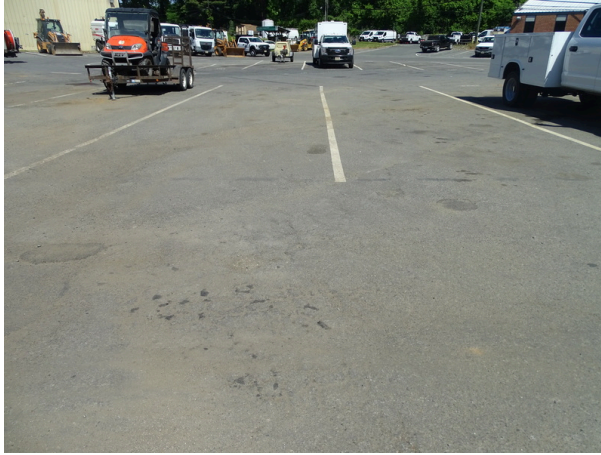
Asphalt pavement - note cracking
