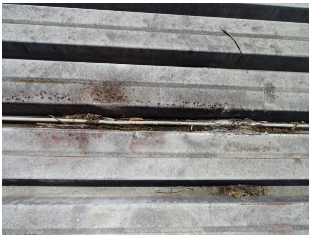
Roofing system of storage building - note deterioration
