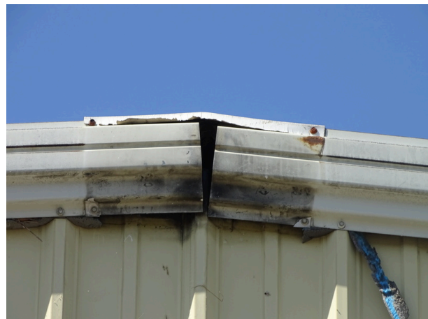
Roofing system of bus wash building - note deterioration
