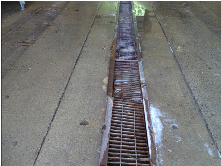
6 - Typical drainage in bus wash building
