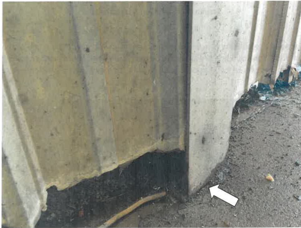
Minor surface rust on steel column and base plate
