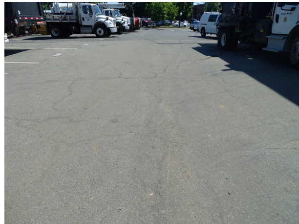
Asphalt pavement and parking - note cracking
