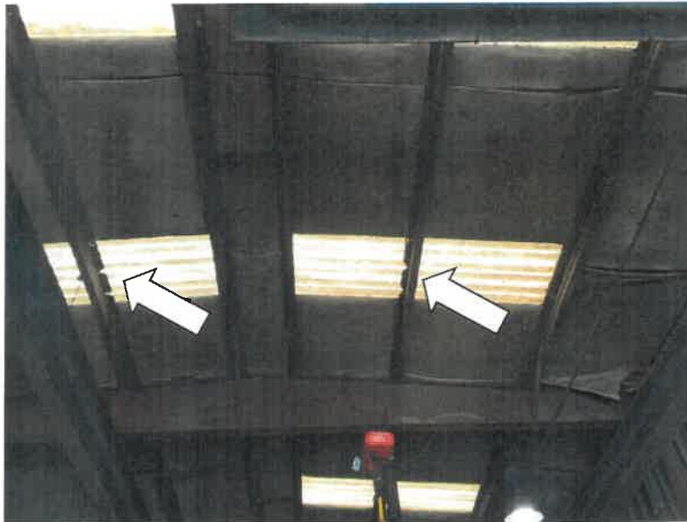
Severely corroded cold-formed z-purlin at skylight
