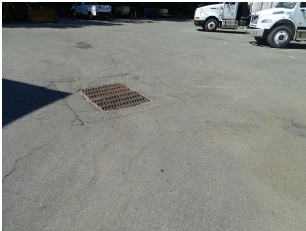
Asphalt pavement - note cracking
