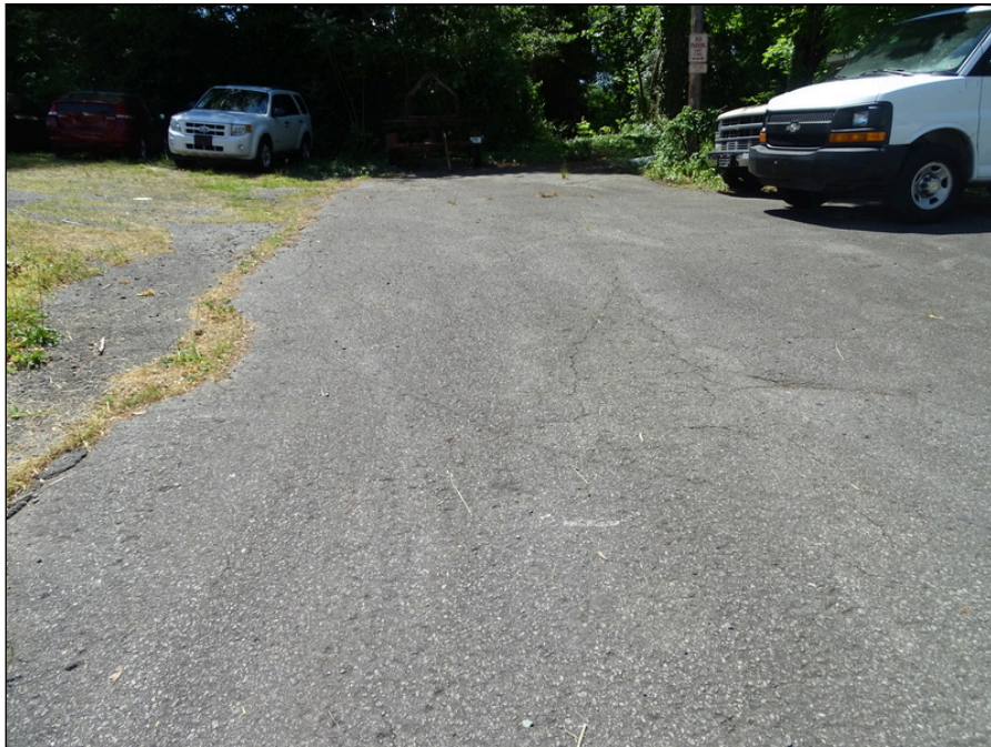
4 - Asphalt pavement - note cracking
