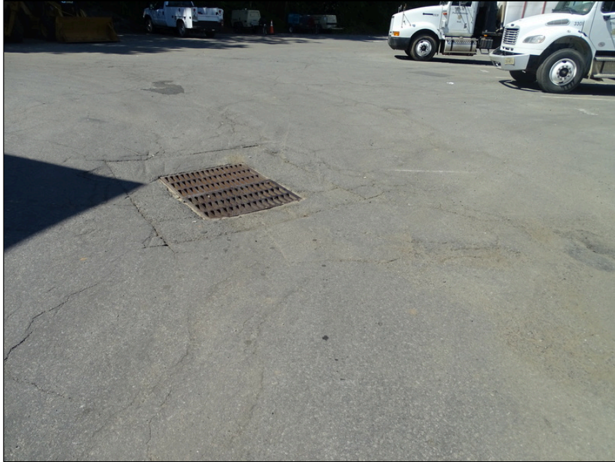
5 - Asphalt pavement - note cracking
