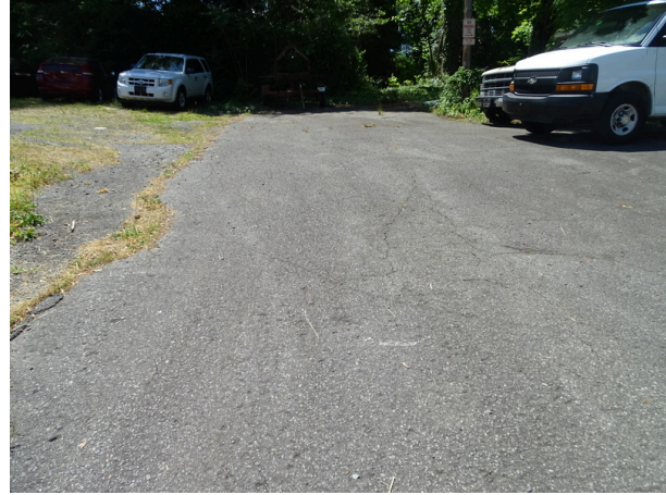
Asphalt pavement - note cracking
