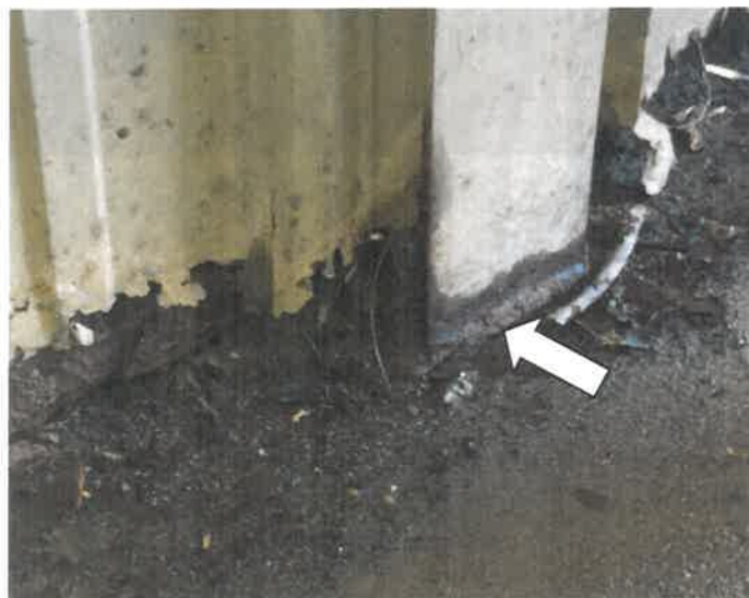
More advanced corrosion of structural steel, but little section loss.
