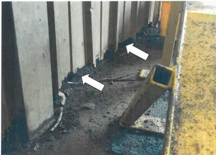
Severe corrosion and damage to bottom of interior wall panels and supporting clip angles.
