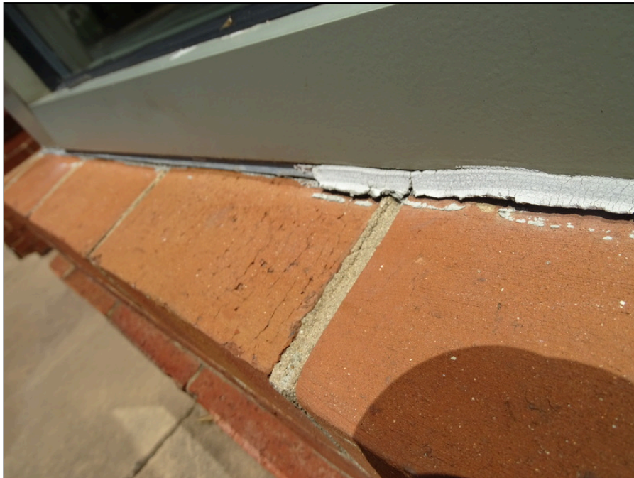
24 - Typical window - note window perimeter sealant
