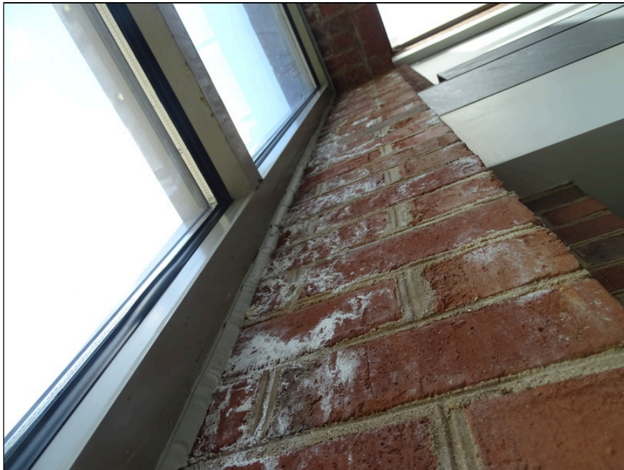
26 - Efflorescence and soiled interior
