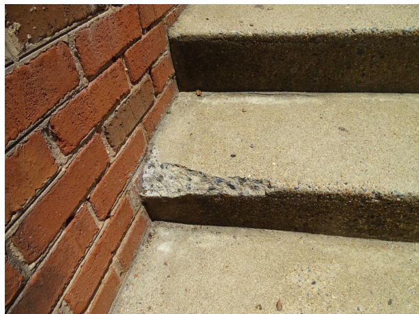
Exterior concrete stair deteriorated
