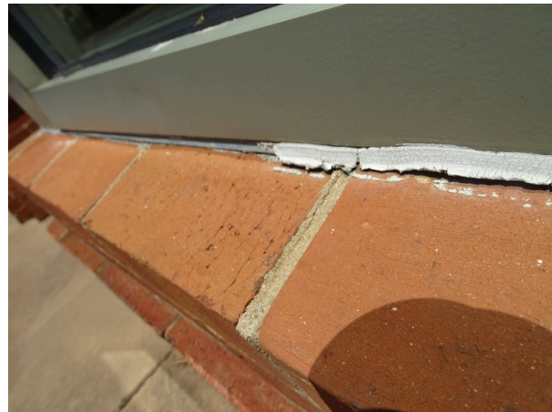
Typical window - note window perimeter sealant
