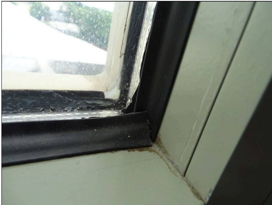
30 - Typical window - note gasket deterioration
