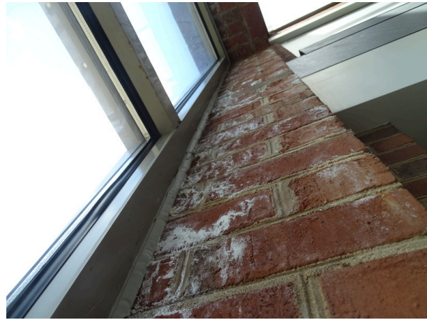
Efflorescence and soiled interior
