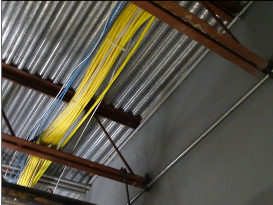
11 - Metal deck supporting an elevated level
