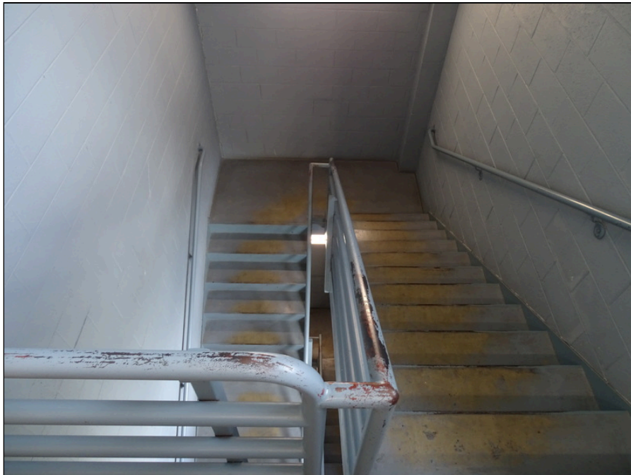
68 - Peeled stair handrail
