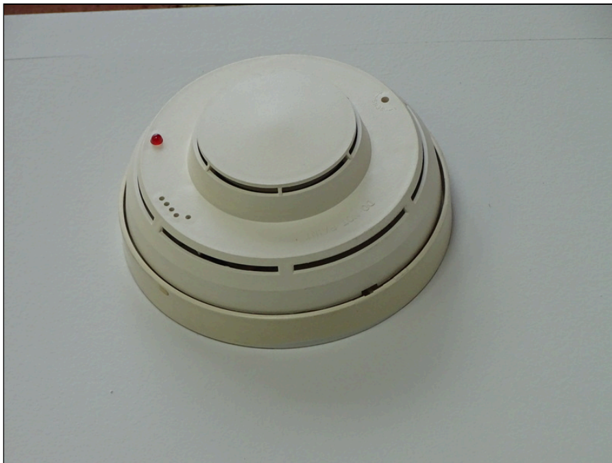
60 - Typical smoke detector
