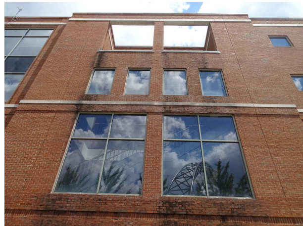
Typical exterior - note efflorescence
