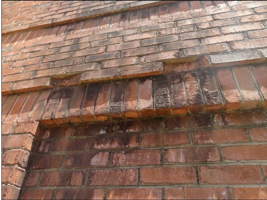
19 - Typical exterior - note spalled bricks
