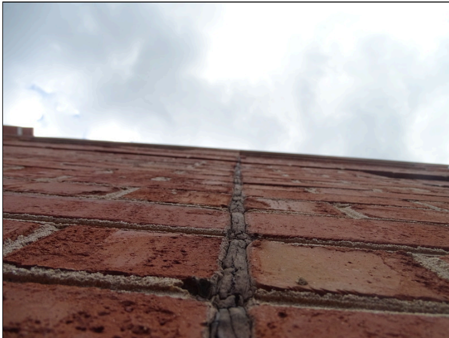
20 - Typical exterior - note vertical joint sealant
