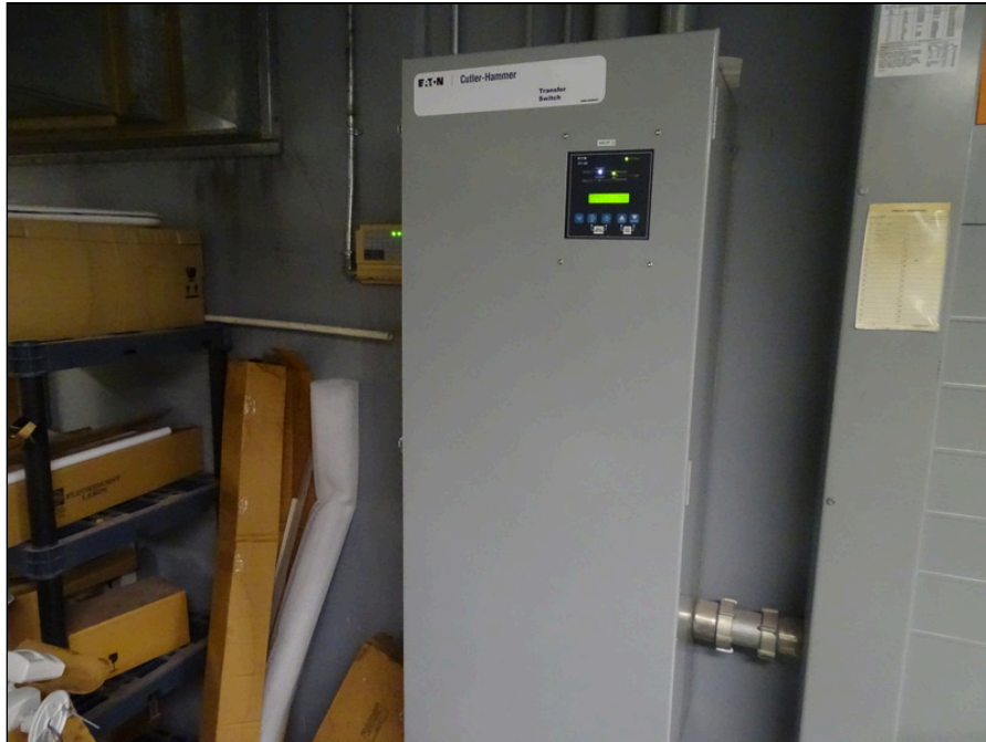
45 - Typical transfer switch
