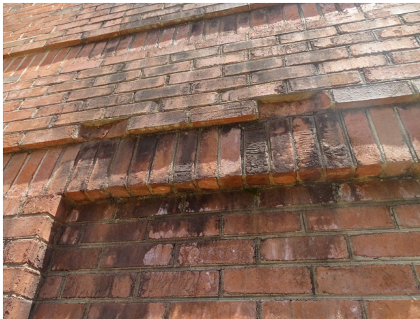
Typical exterior - note spalled bricks
