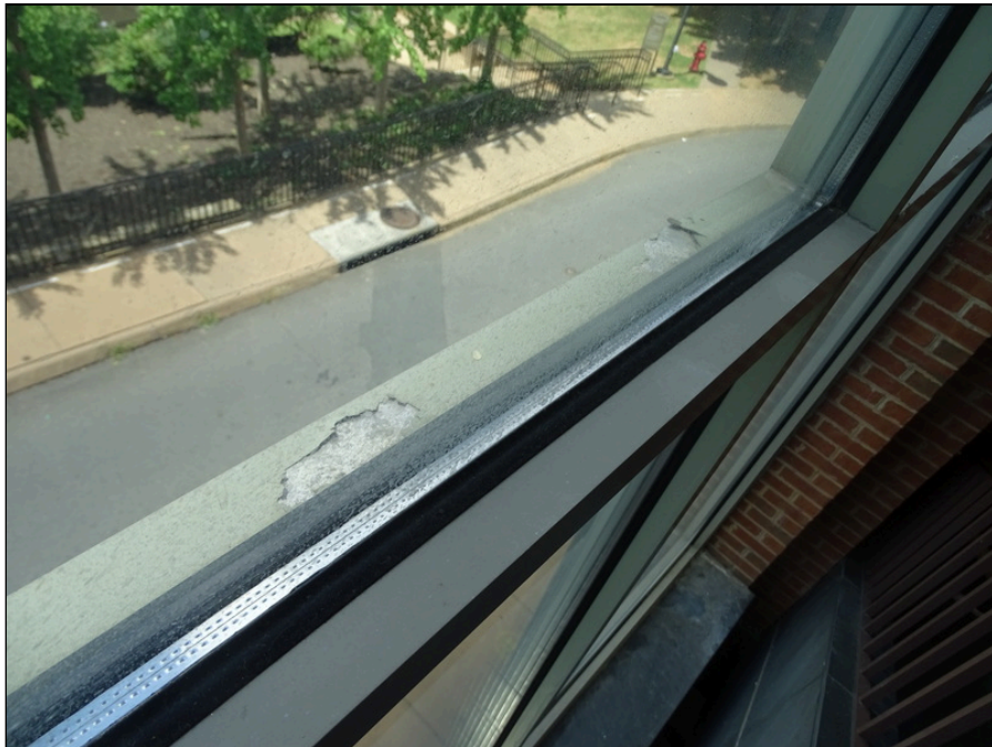
28 - Typical window - note peeling paint
