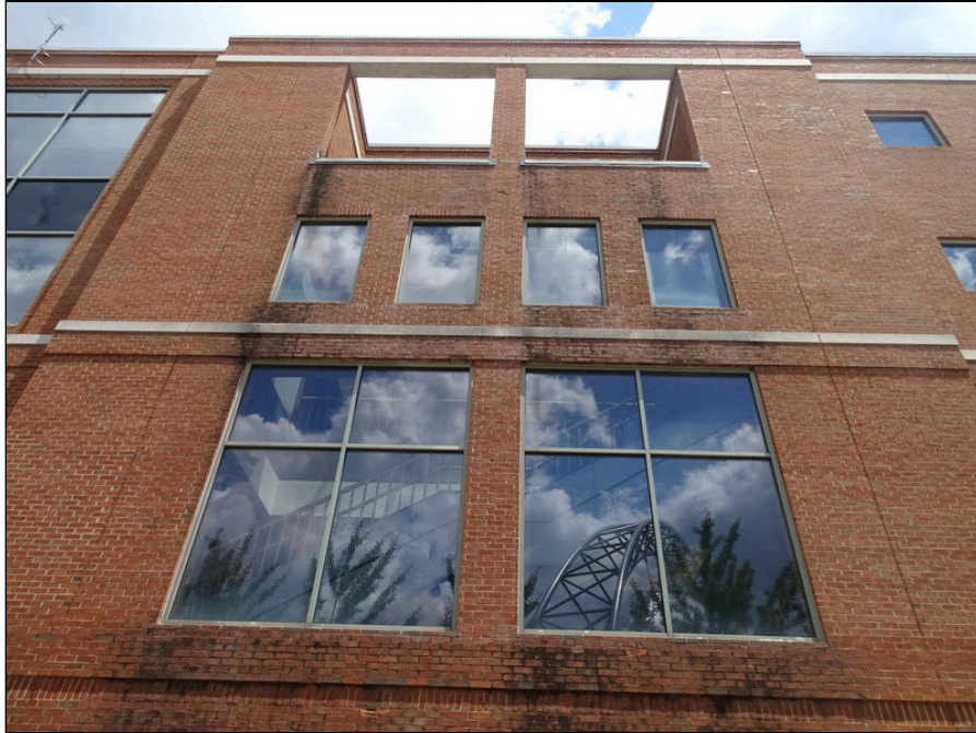
17 - Typical exterior - note efflorescence
