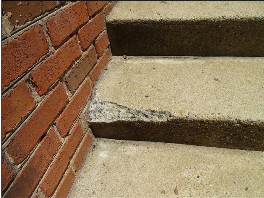
7 - Exterior concrete stair deteriorated
