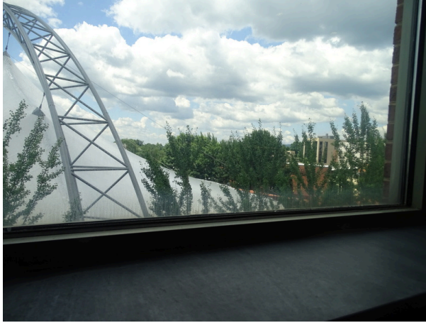
Typical window - note fogged glass
