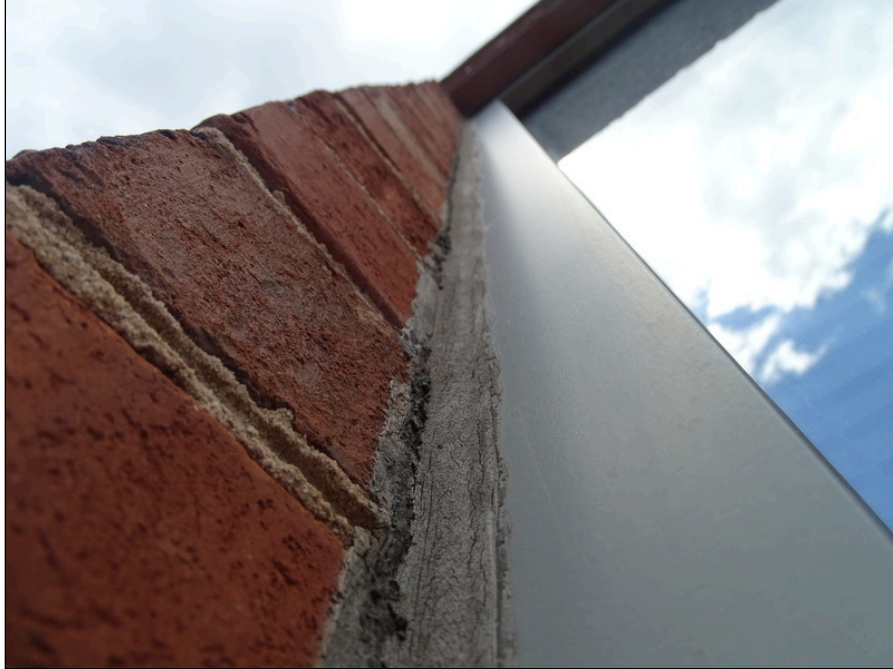
31 - Window perimeter sealant
