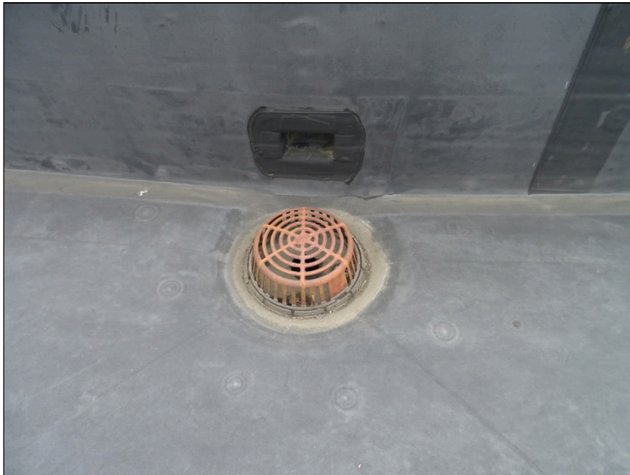
36 - Roof drain and overflow scupper
