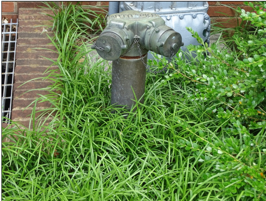
54 - Typical fire department connections
