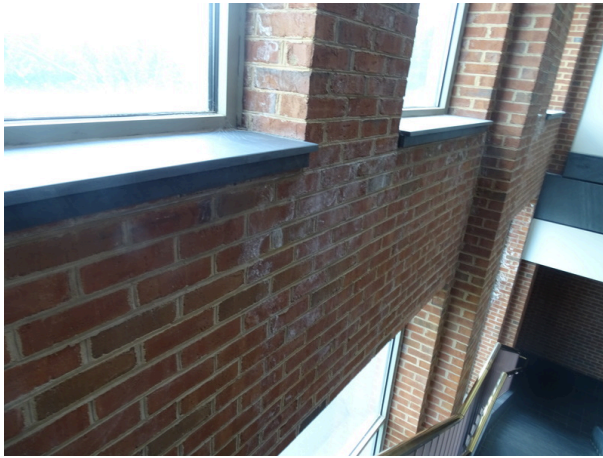
Efflorescence and soiled interior
