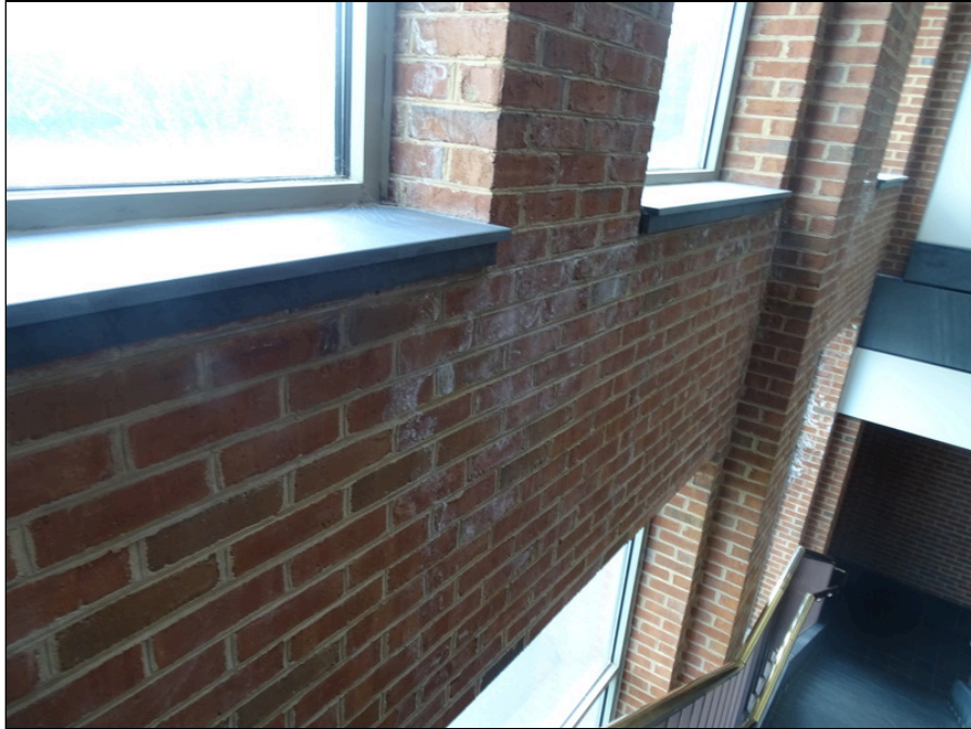
25 - Efflorescence and soiled interior
