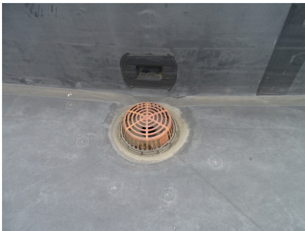
Roof drain and overflow scupper
