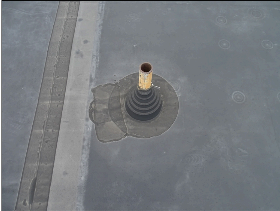
37 - Typical pipe flashing
