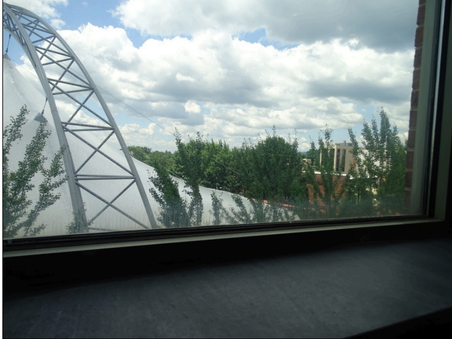
29 - Typical window - note fogged glass
