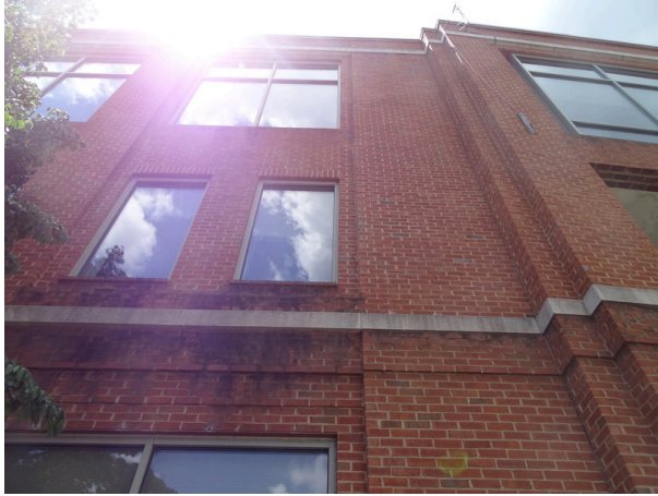
Efflorescence and soiled exterior
