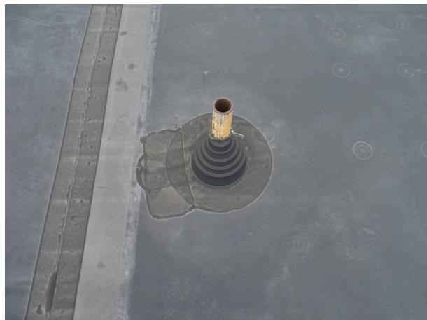
Typical pipe flashing
