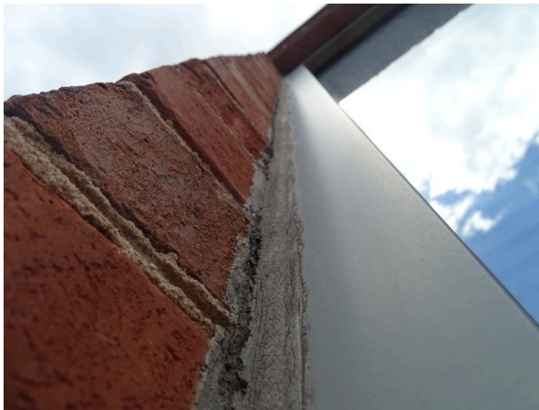
Window perimeter sealant
