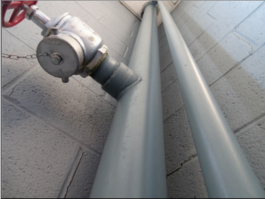
57 - Sprinkler standpipe
