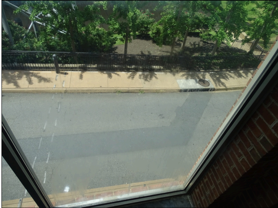
27 - Typical window - note fogged glass
