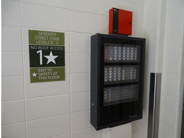
Fire alarm annunciator and control panel
