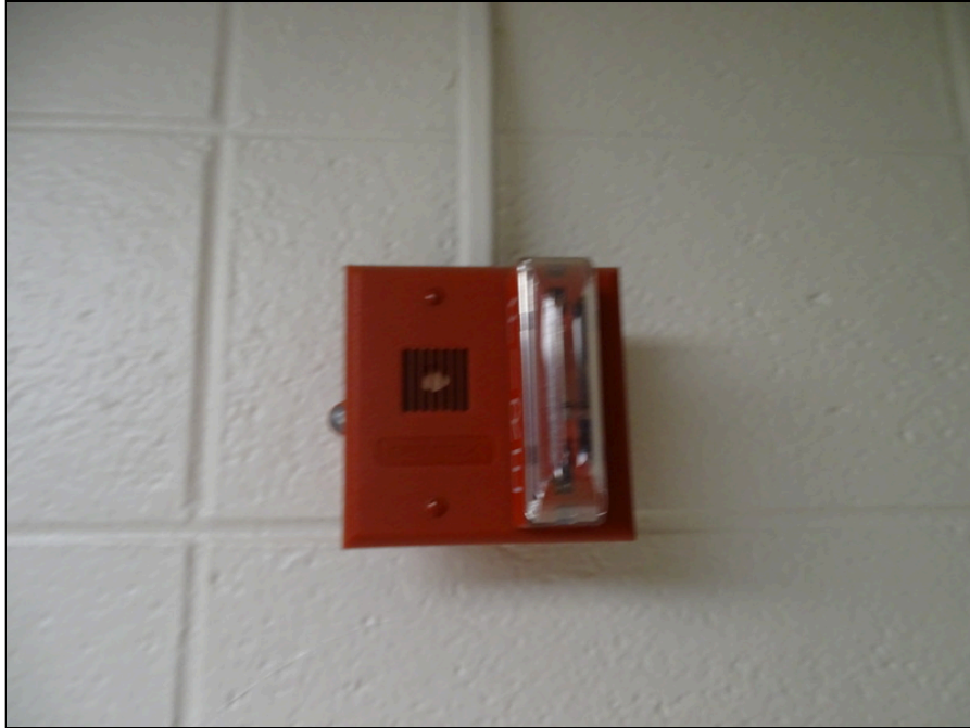
49 - Typical fire alarm bell and strobe
