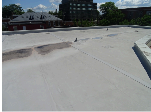
Single-ply roofing system east side of the building - note ponding
