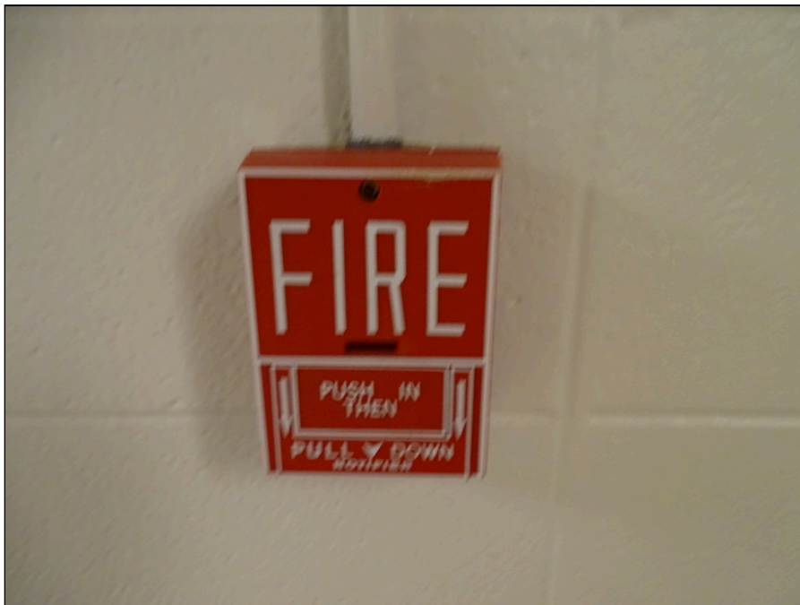
50 - Typical fire alarm pull station
