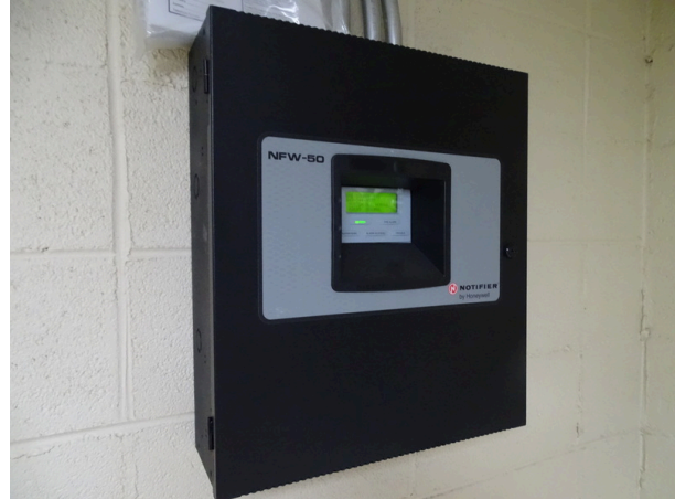
Fire alarm notifier electronics
