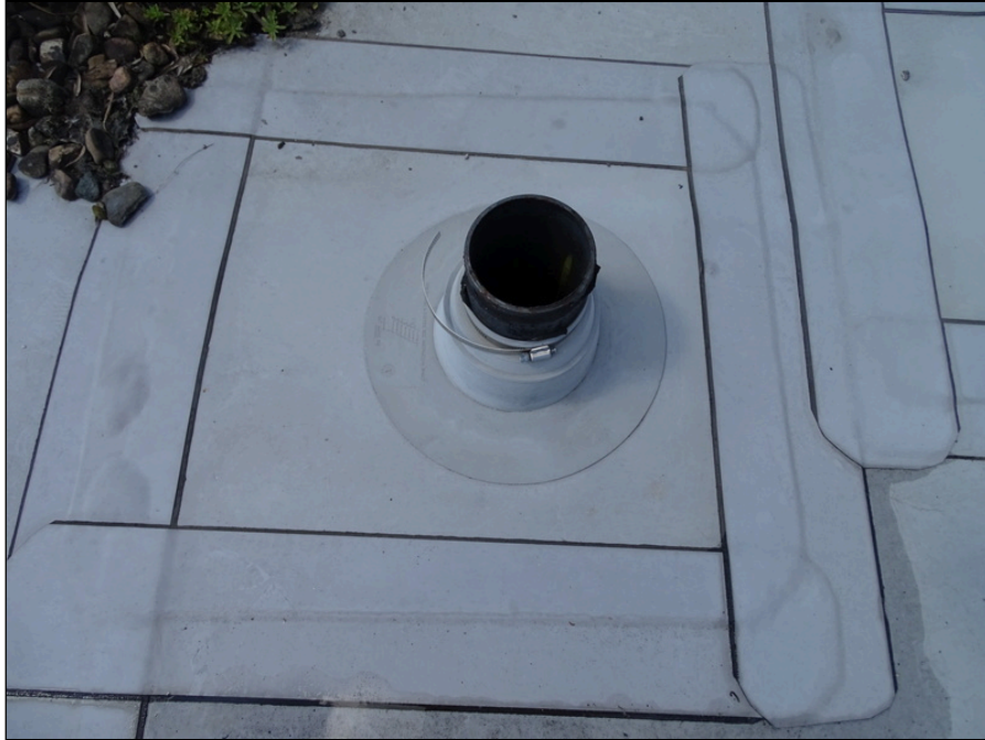
23 - Typical plumbing penetration
