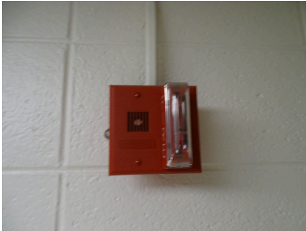
Typical fire alarm bell and strobe
