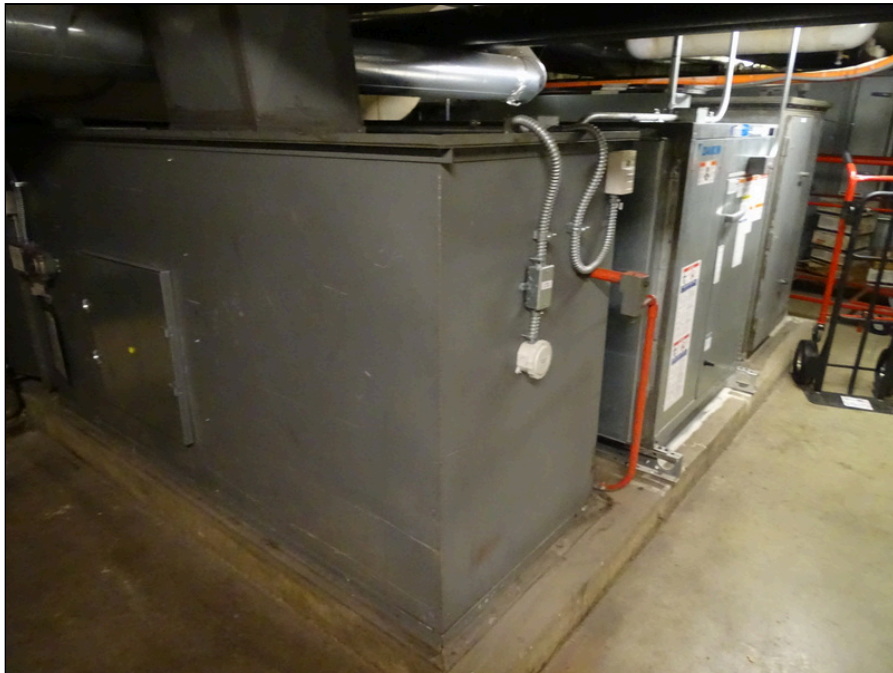
32 - Typical older Air Handler Unit located in the City Hall Building
