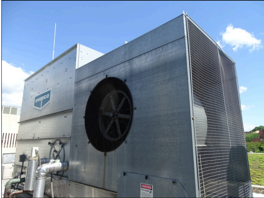
29 - Cooling Towers located on the roof of City Hall Building
