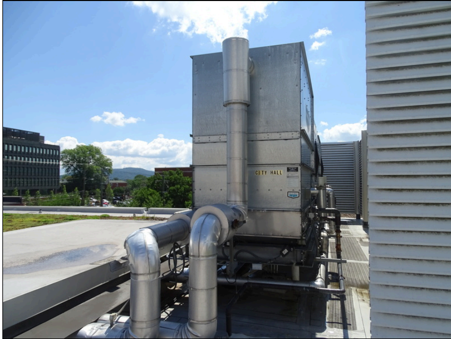
31 - Cooling Towers located on the roof of City Hall Building
