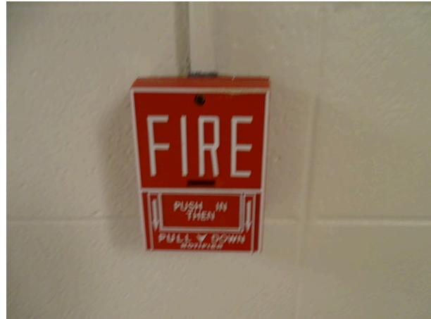
Typical fire alarm pull station
