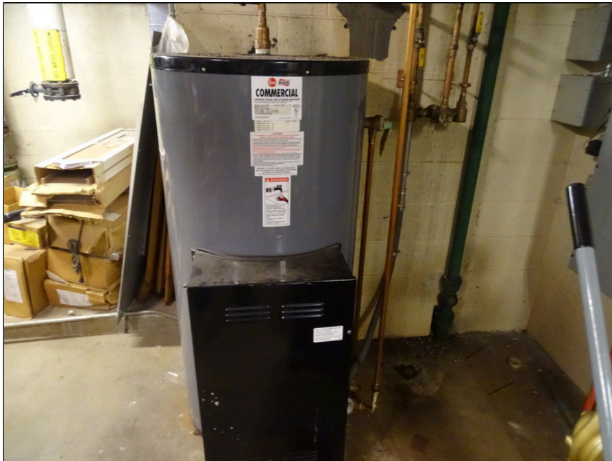
26 - Electric water heater located in main utility room
