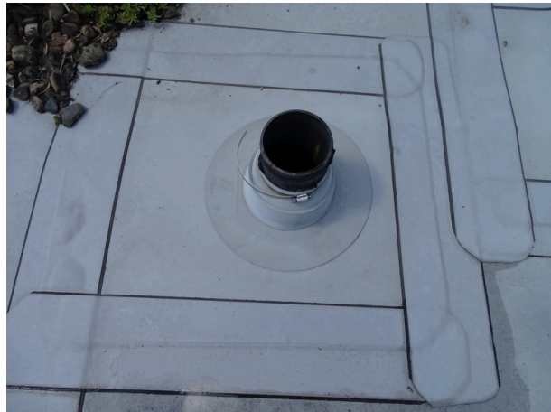
Typical plumbing penetration
