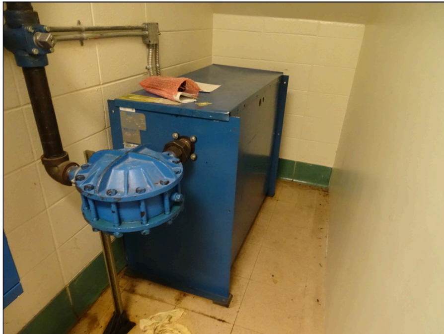
44 - Passenger elevator machine
