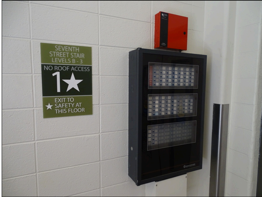
47 - Fire alarm annunciator and control panel
