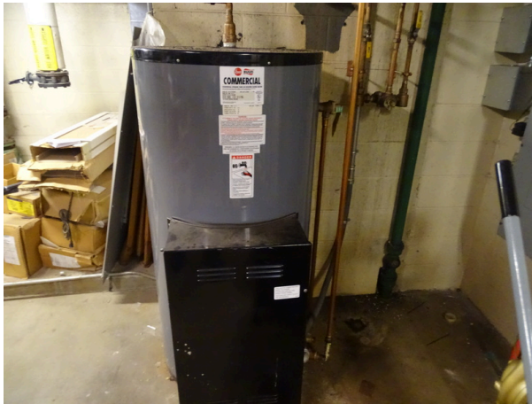
Electric water heater located in main utility room
