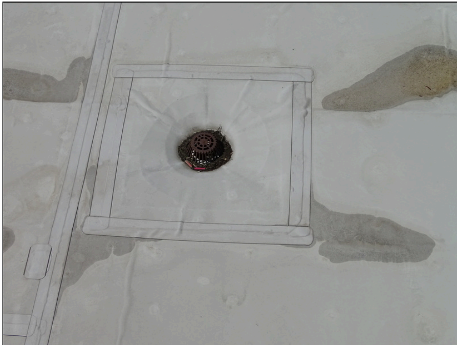
22 - Typical internal drain
