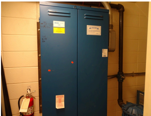
Passenger elevator controls
