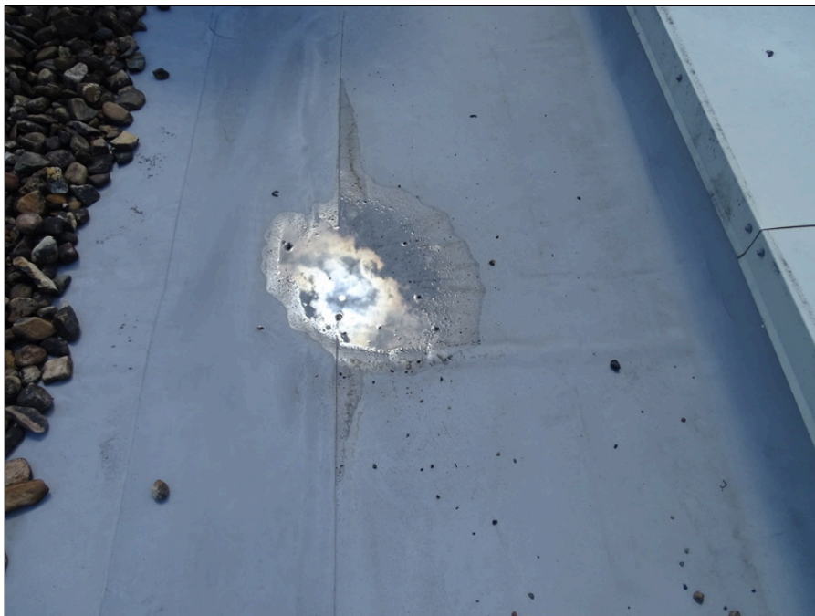
20 - single-ply roofing system west side of the building - note ponding
