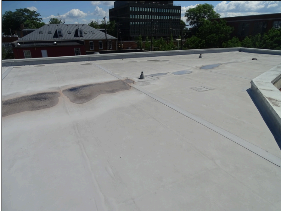
21 - Single-ply roofing system east side of the building - note ponding
