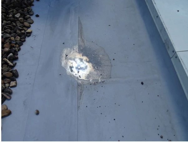
single-ply roofing system west side of the building - note ponding
