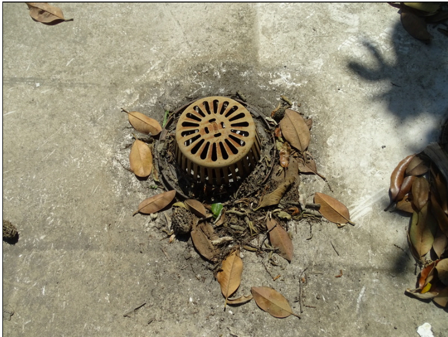
38 - Typical internal drain
