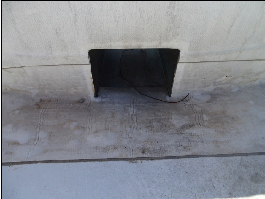
33 - Typical parapet wall and through-wall scupper drain
