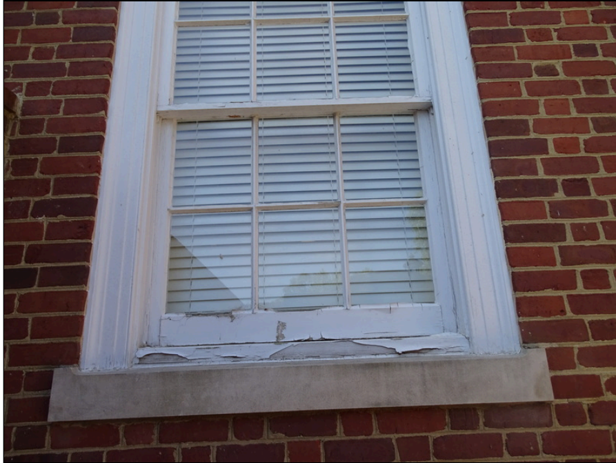
29 - Typical exterior window - note deterioration
