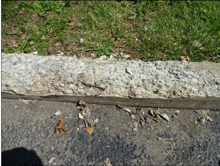
9 - Concrete curb - note deterioration
