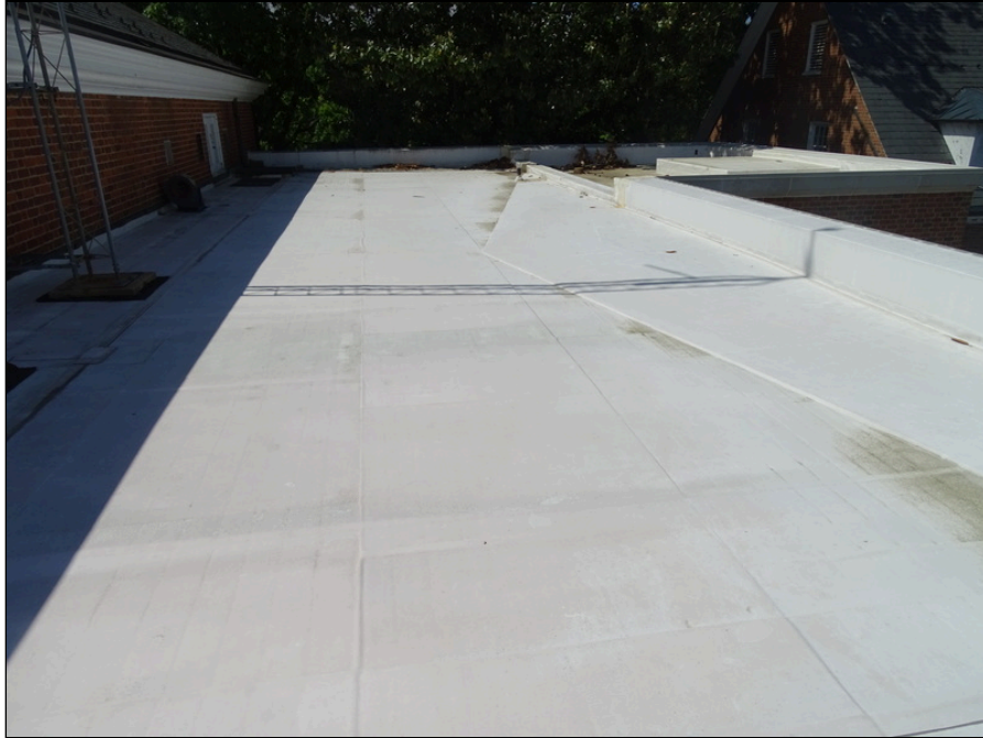
31 - Single-ply membrane roofing system
