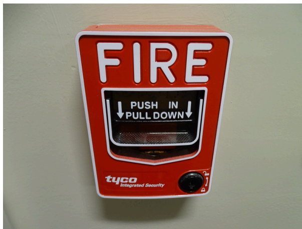
Typical pull down station
