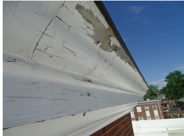
Exterior cornice - note deterioration
