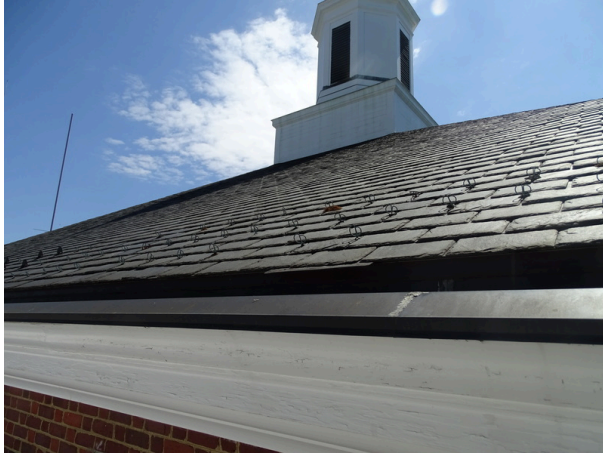
Slate roofing system
