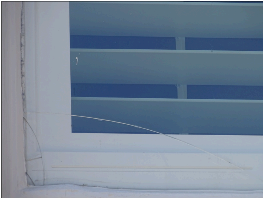
30 - Typical window exterior - note cracks in glass
