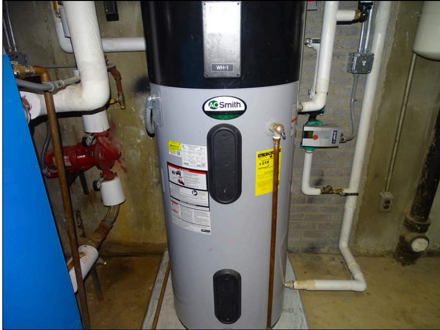
43 - Electric water heater
