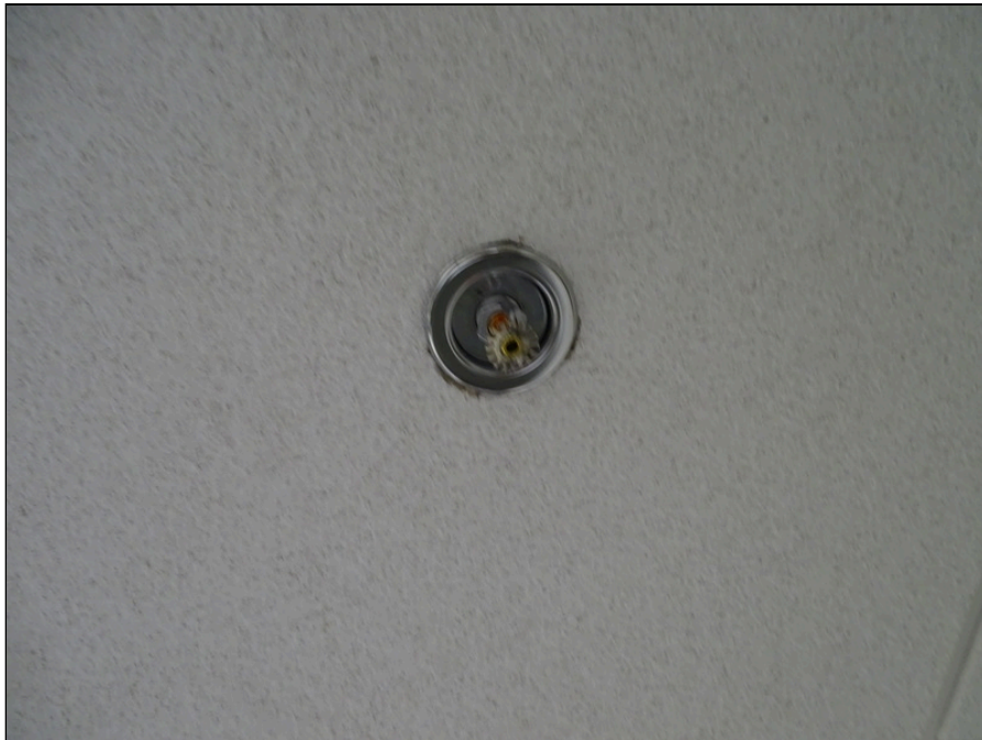
66 - Typical fire sprinkler head
