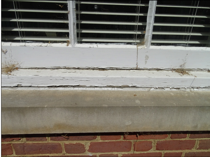
23 - Typical exterior window - note deterioration
