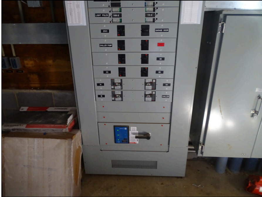
59 - Main electrical switchgear
