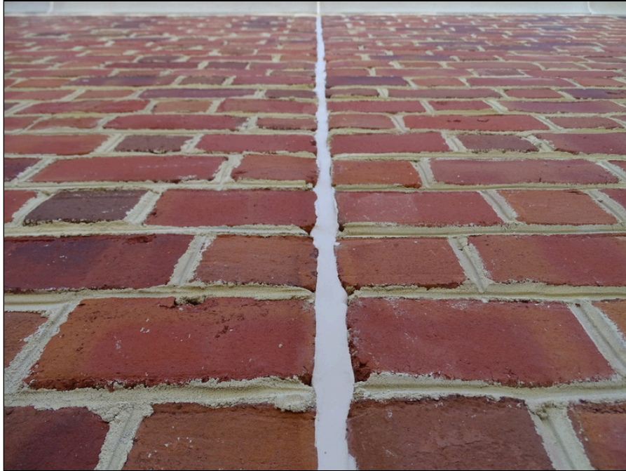
19 - Building exterior vertical joint
