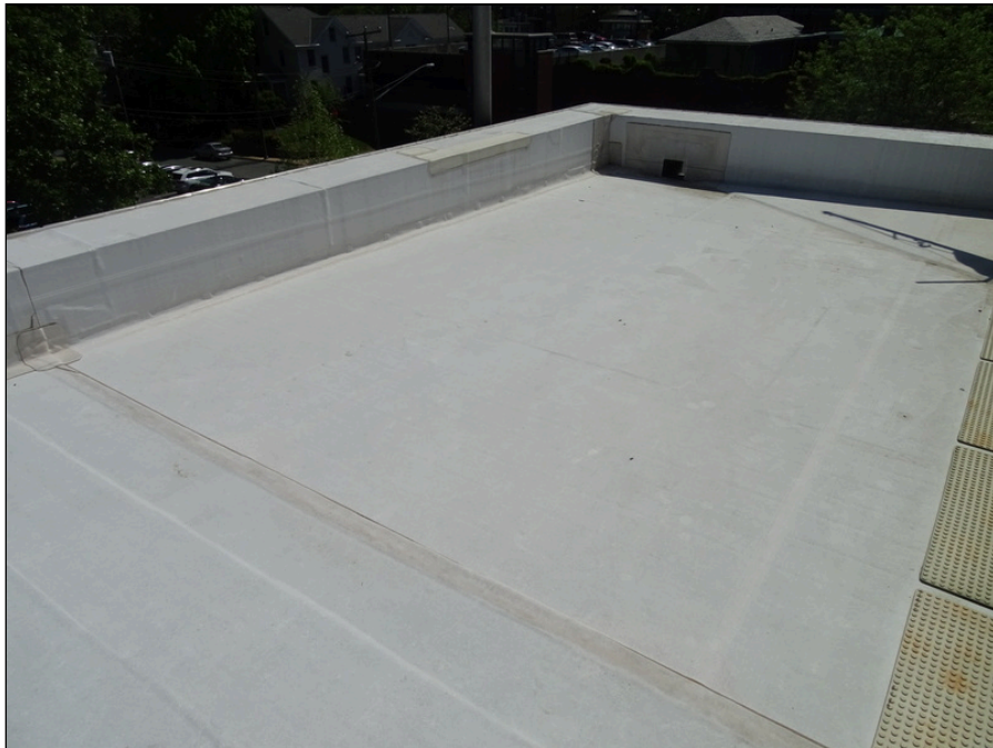
32 - Typical parapet wall and through-wall scupper drain
