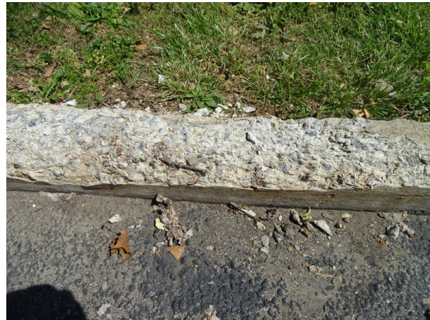
Concrete curb - note deterioration
