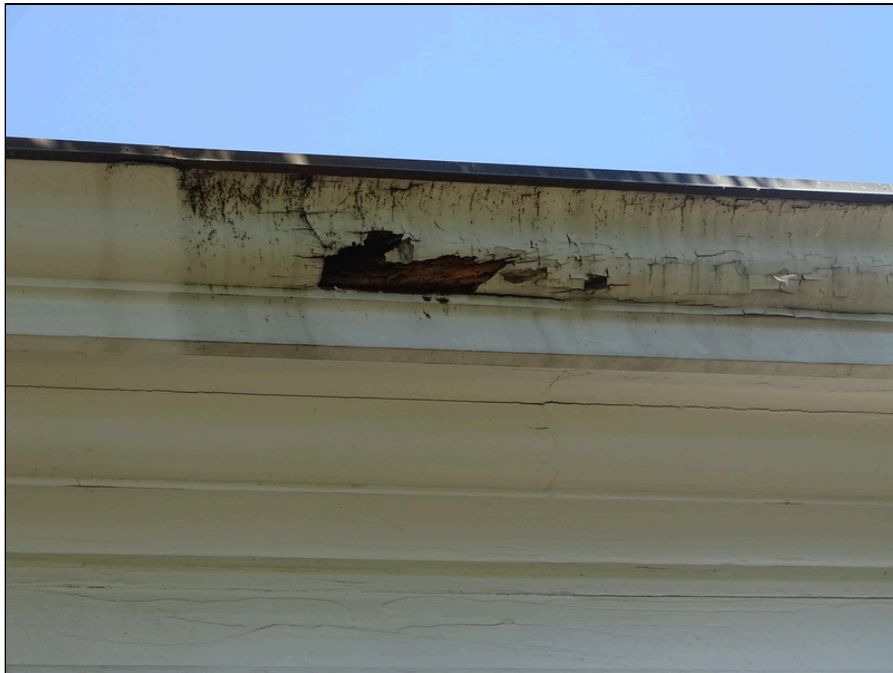
22 - Exterior cornice - note deterioration
