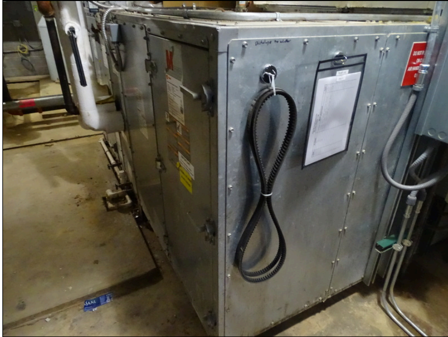
49 - Air Handler Unit located in attic space
