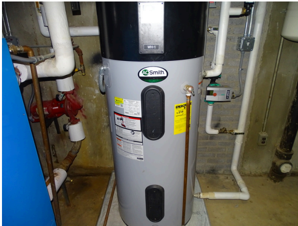
Electric water heater
