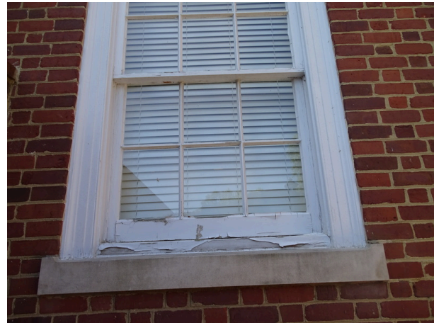
Typical exterior window - note deterioration
