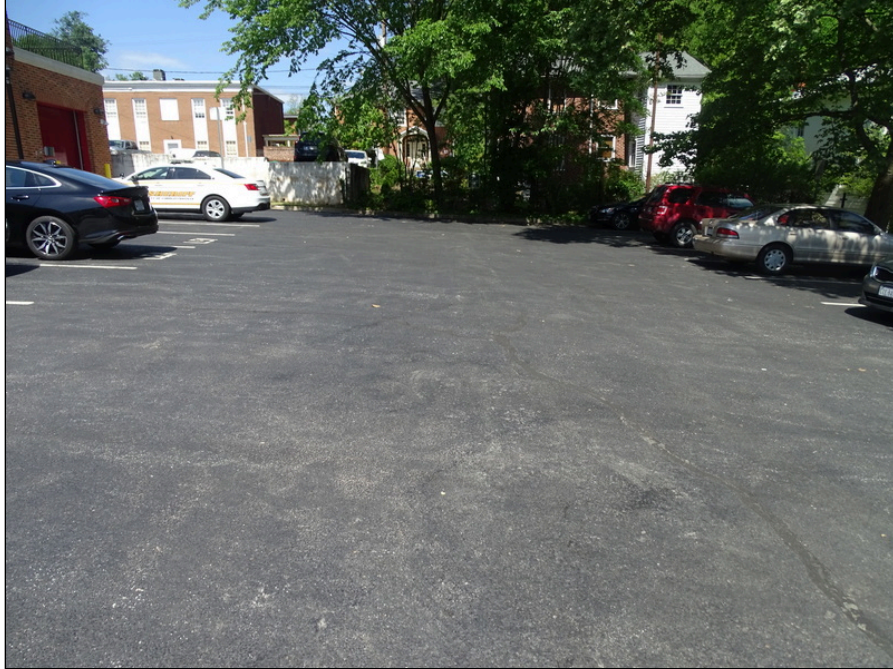
3 - Asphalt pavement on north side of site - note cracking
