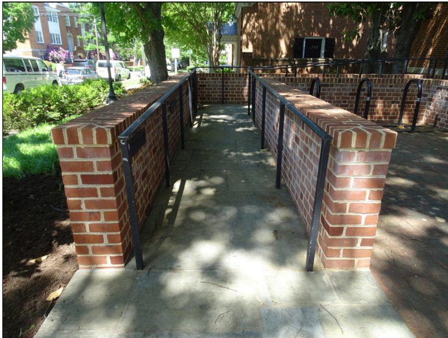
106 - Typical accessible ramp
