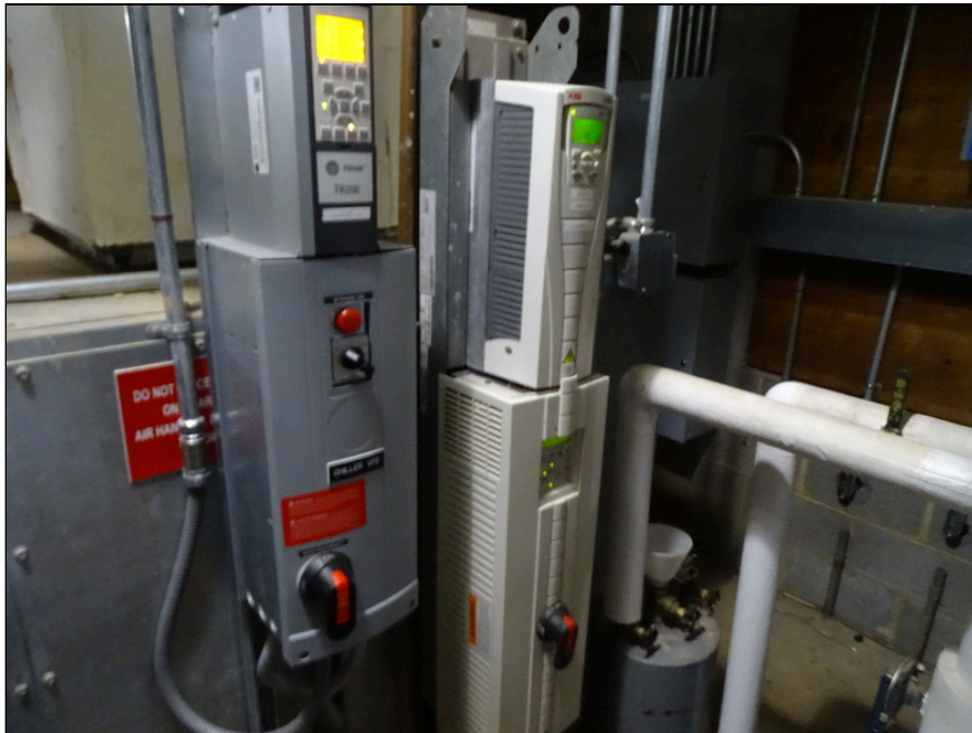
50 - Variable frequency drive system
