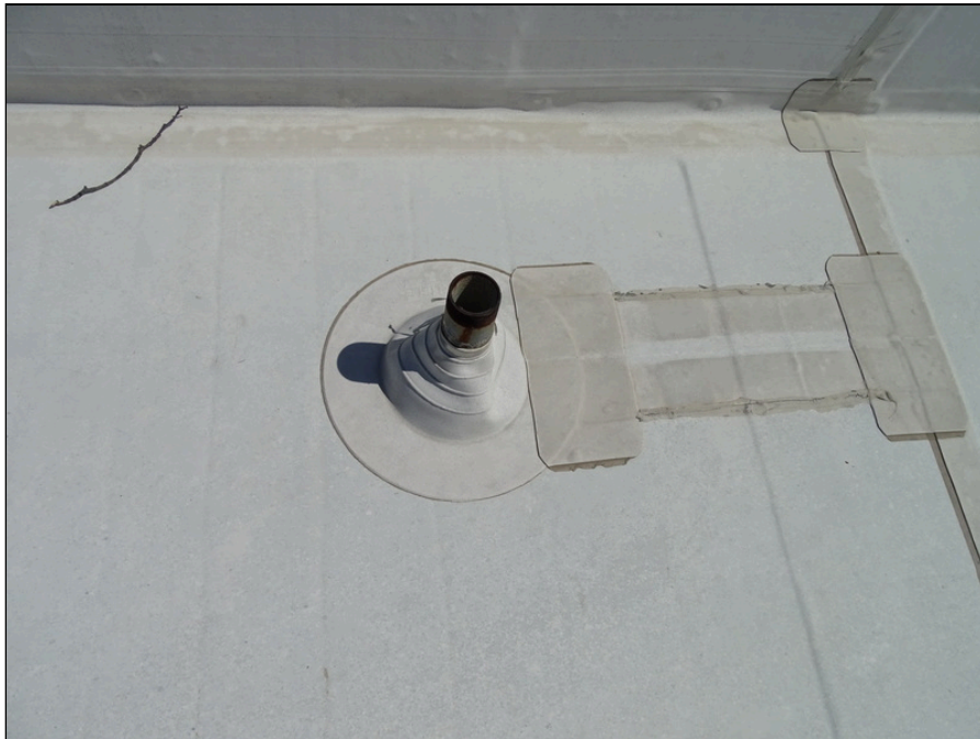
34 - Typical plumbing penetration
