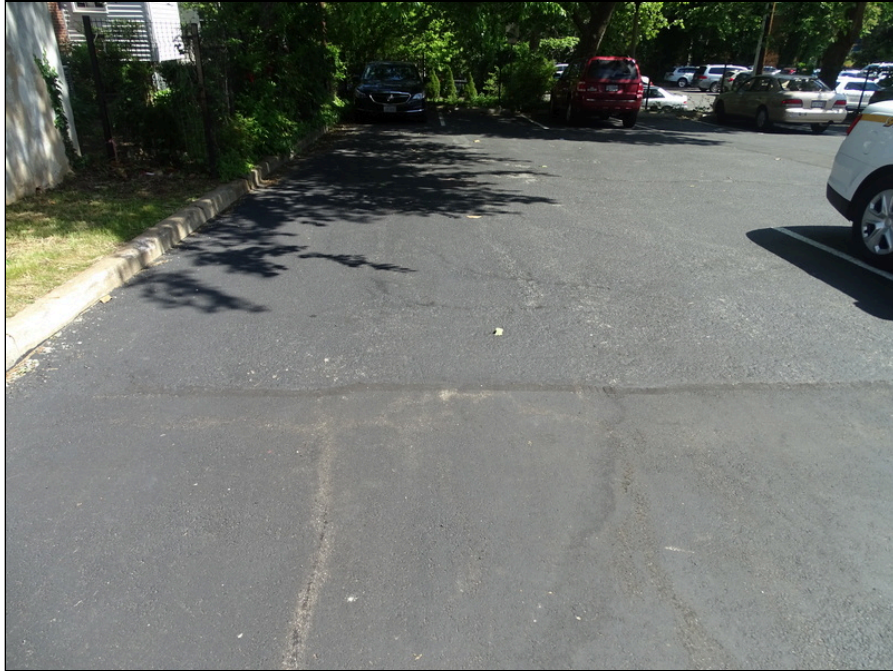
5 - Asphalt pavement on north side of site - note cracking
