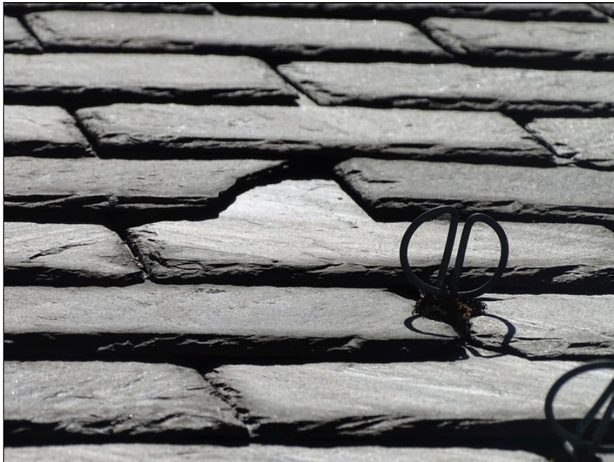
40 - Slate roofing system - note deterioration
