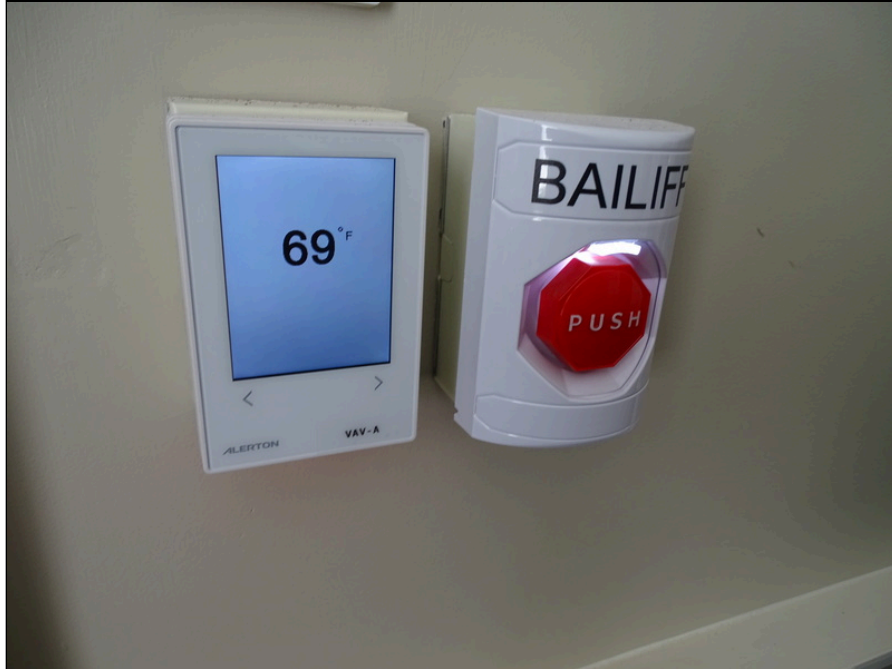
57 - Mechanical system thermostat controls
