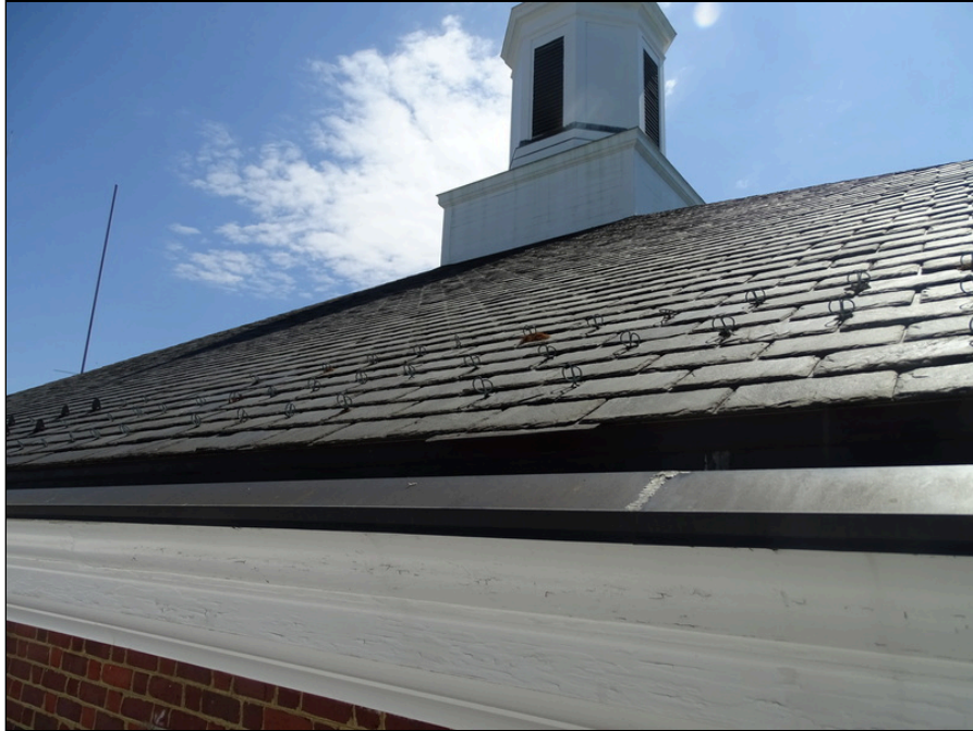
39 - Slate roofing system
