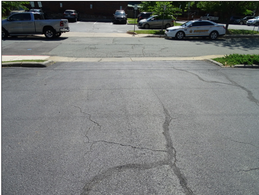
4 - Asphalt pavement on north side of site - note cracking
