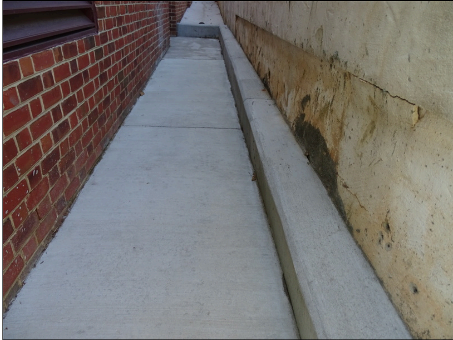
7 - Concrete side walk - note wall deterioration
