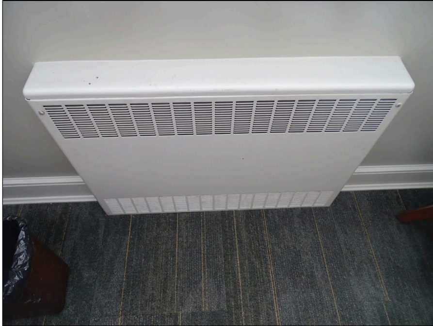
55 - Typical water source heat pump
