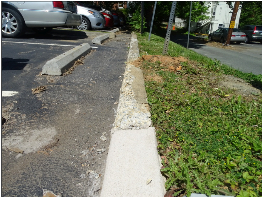
8 - Concrete curb - note deterioration
