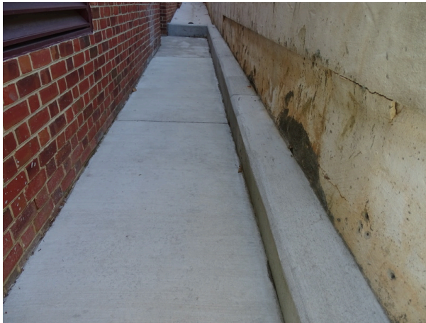
Concrete side walk - note wall deterioration
