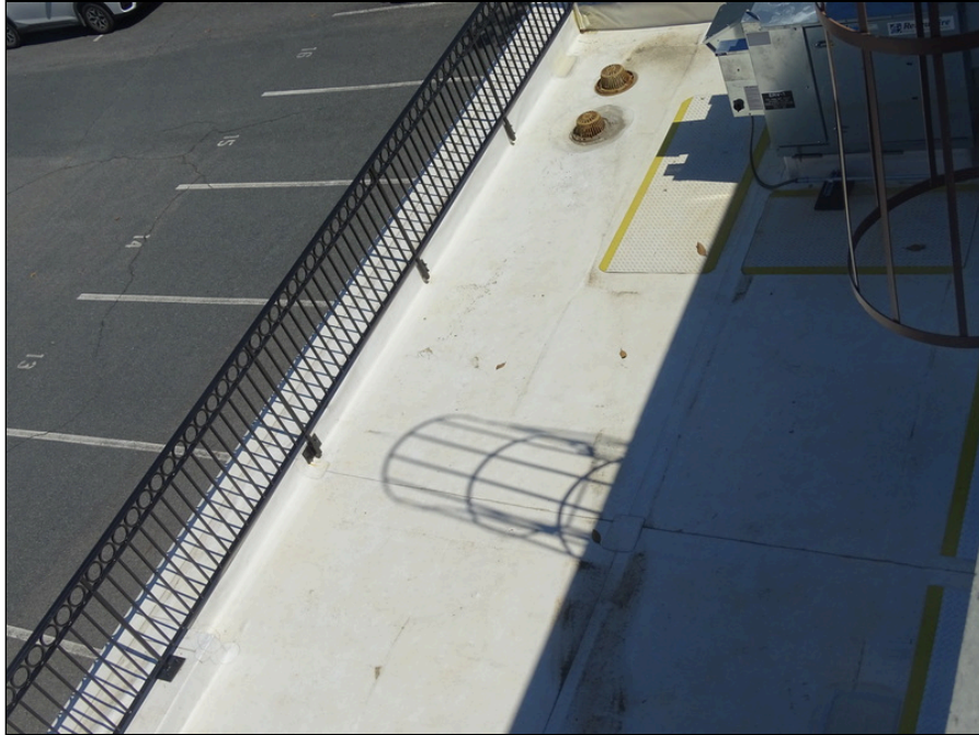
37 - Single-ply membrane roofing system
