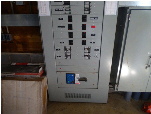
Main electrical switchgear
