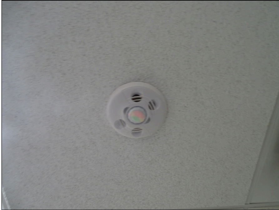
67 - Typical smoke detector
