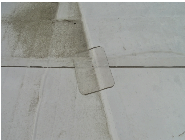
Single-ply membrane roofing system at parapet wall - note patching
