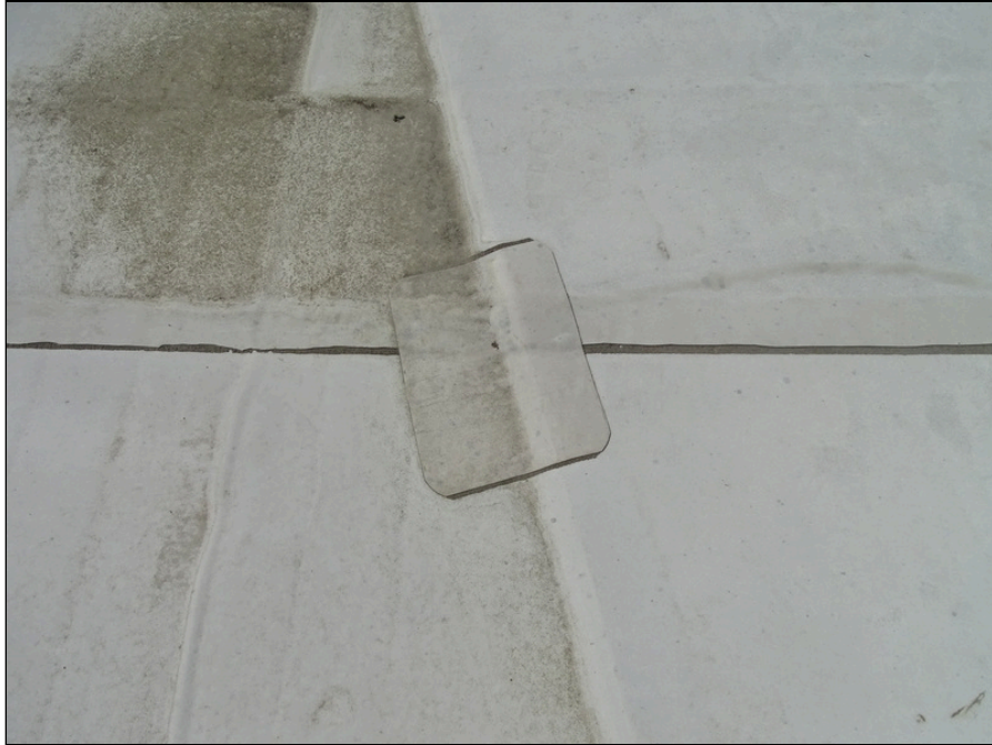
35 - Single-ply membrane roofing system at parapet wall - note patching
