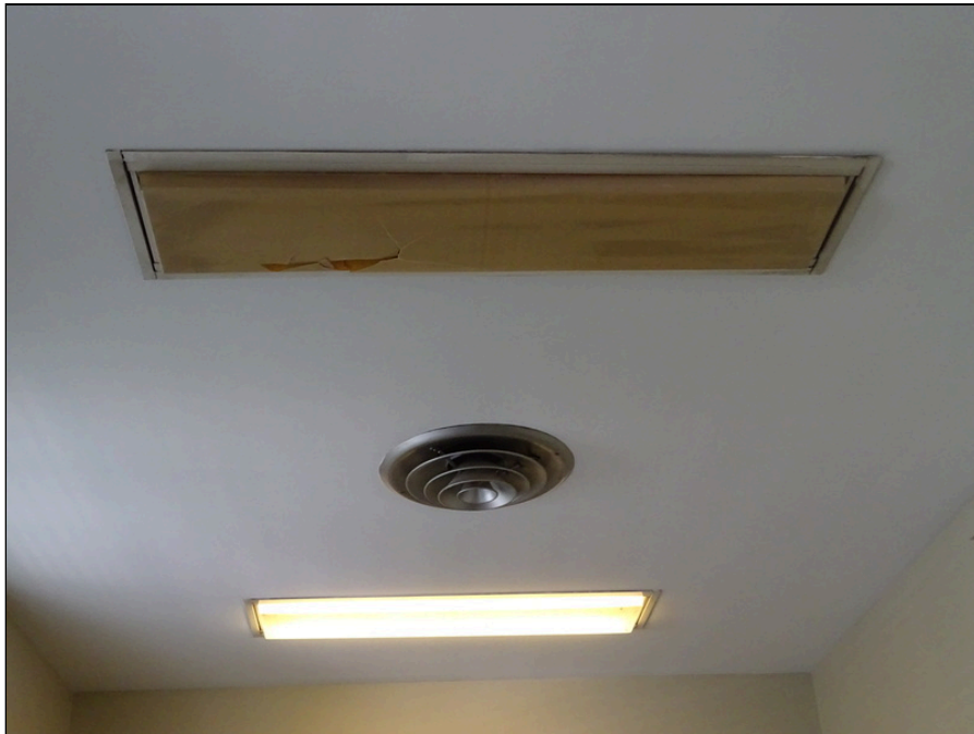
54 - Typical ducted supply
