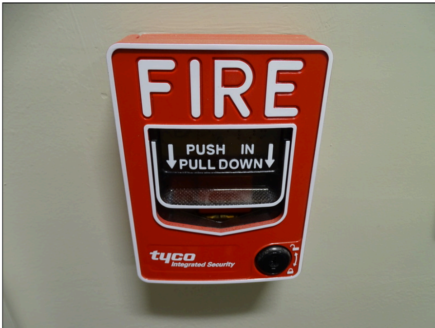
68 - Typical pull down station
