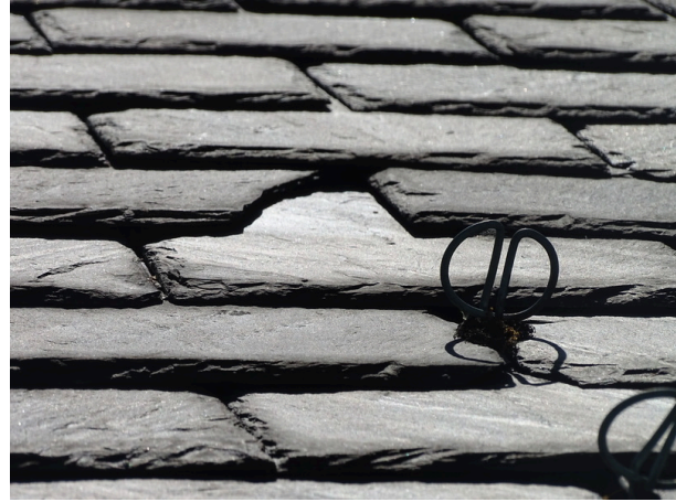
Slate roofing system - note deterioration
