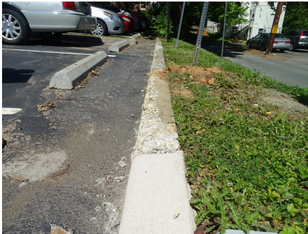
Concrete curb - note deterioration
