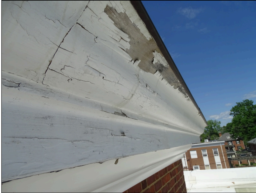
41 - Exterior cornice - note deterioration
