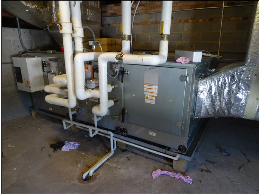
47 - Air Handler Unit located in attic space
