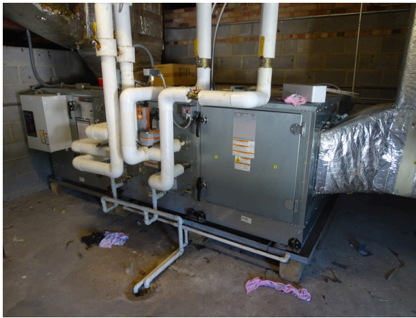
Air Handler Unit located in attic space
