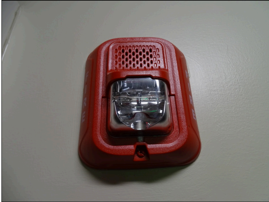
69 - Typical fire alarm, bell, and strobe
