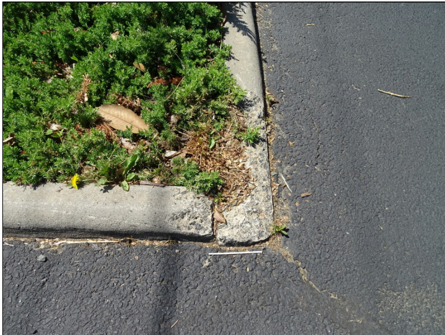
10 - Concrete curb - note deterioration
