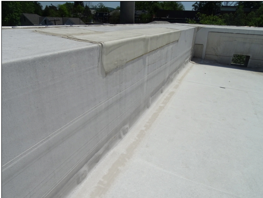
36 - Single-ply membrane roofing system at parapet wall - note patching
