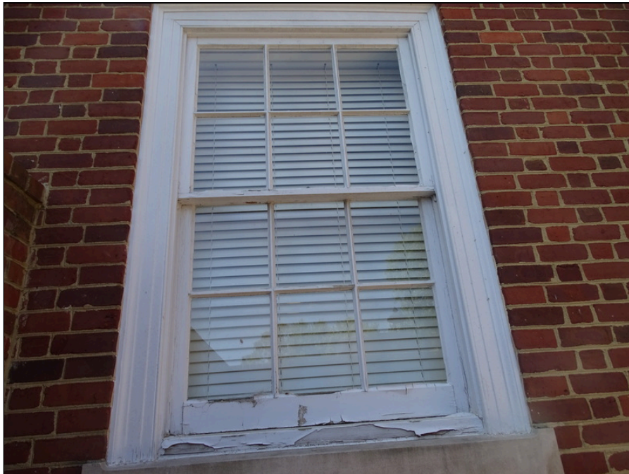
28 - Typical exterior window - note deterioration
