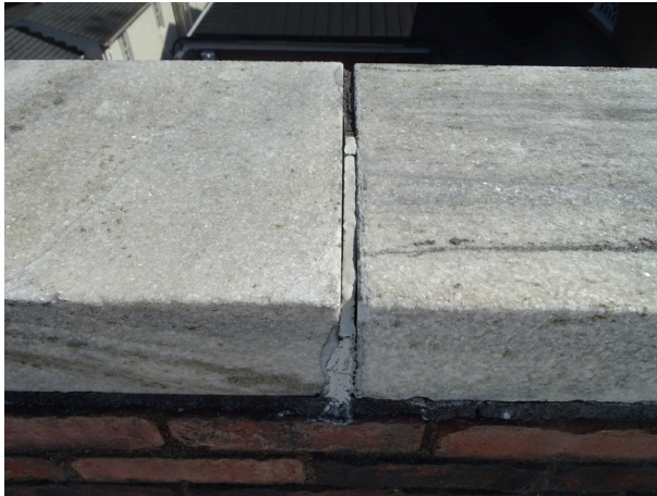
Typical parapet wall - note mortar joint deterioration
