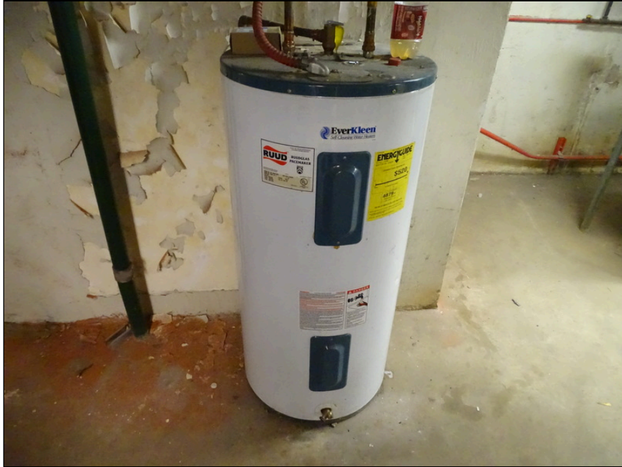
29 - Electric domestic water heater
