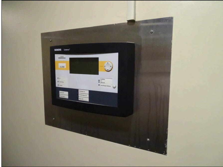
49 - Fire alarm control panel
