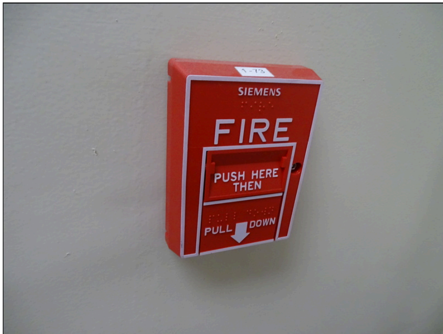
50 - Typical fire alarm pull station
