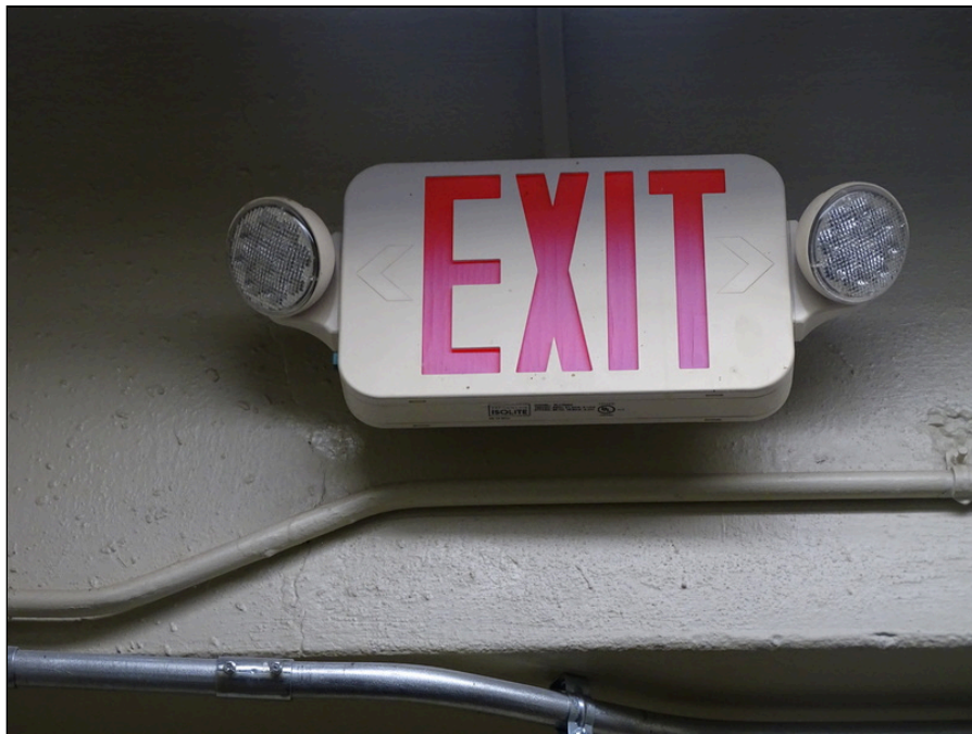
52 - Typical exit sign and emergency light
