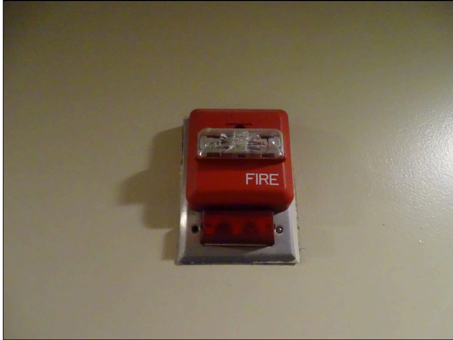
51 - Typical fire alarm bell and strobe
