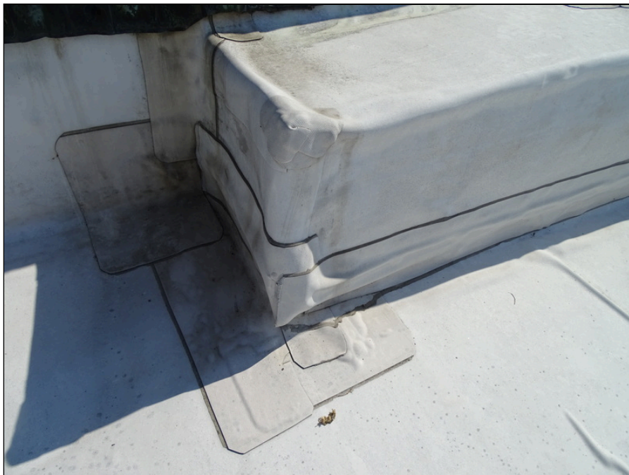
22 - Typical parapet wall - note patching
