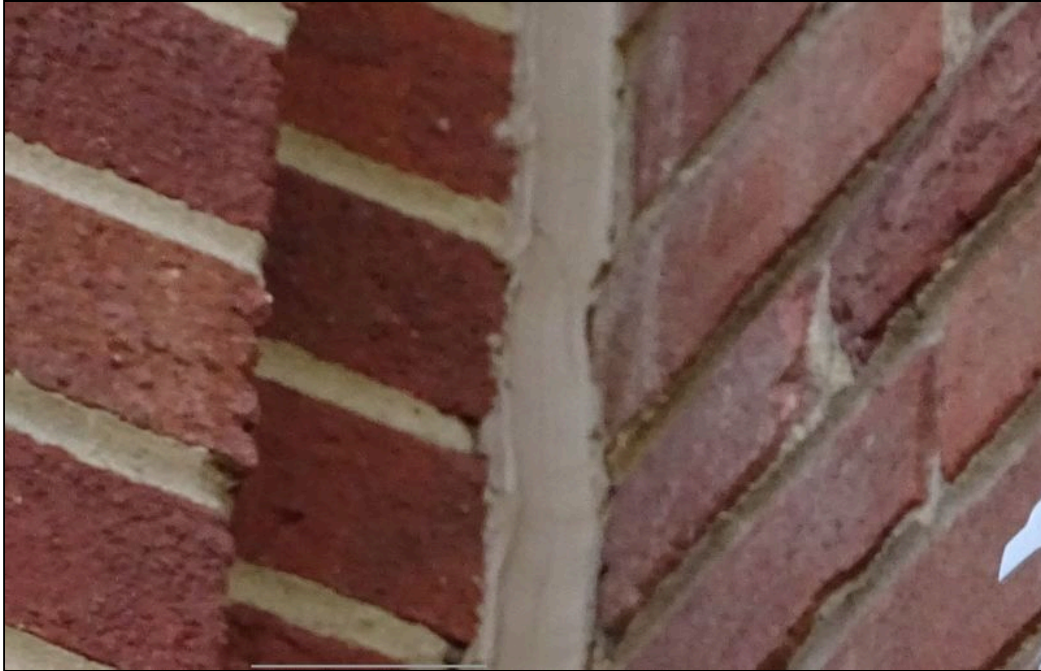
15 - Exterior sealants - note deterioration
