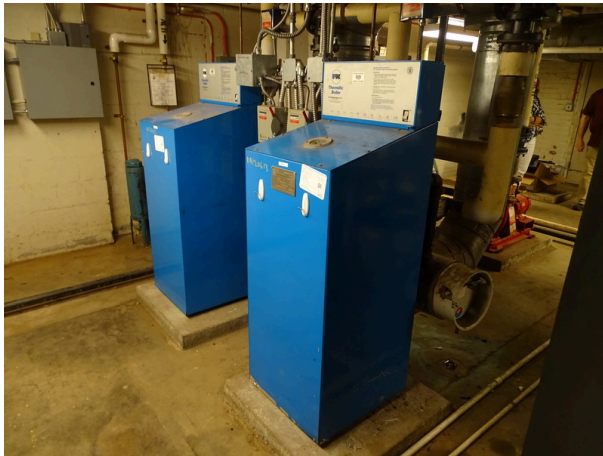
Boilers located in main utility room
