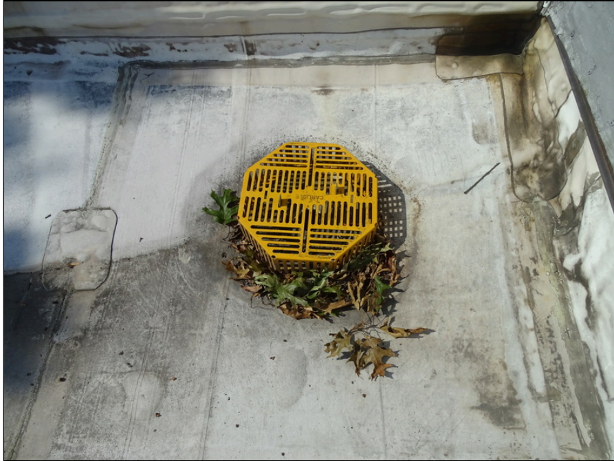
25 - Typical internal drain
