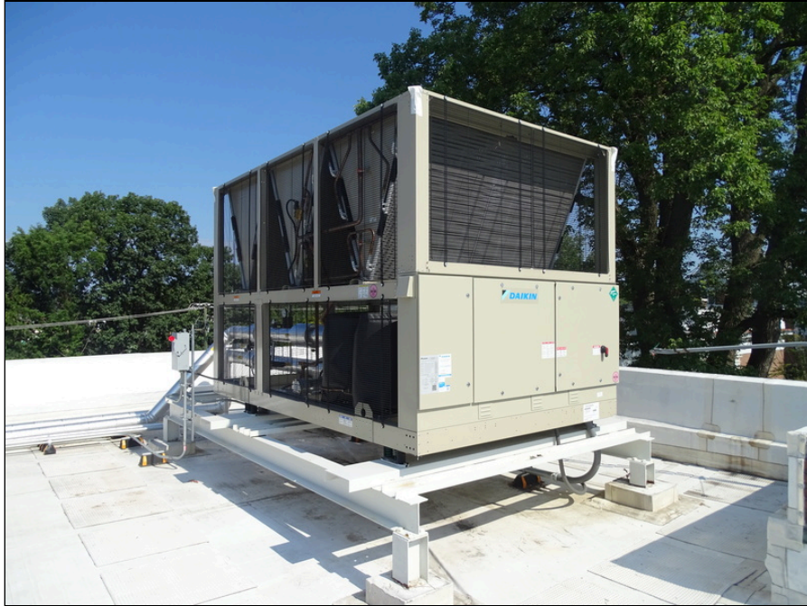
31 - Condenser Unit located on roof
