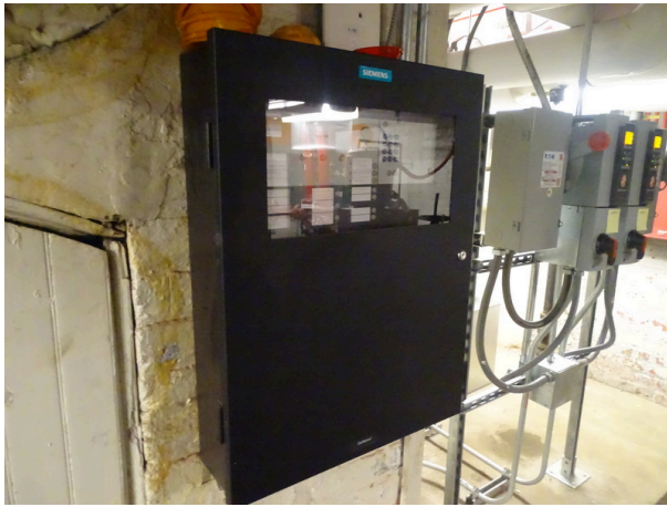
Fire sprinkler electronic controls
