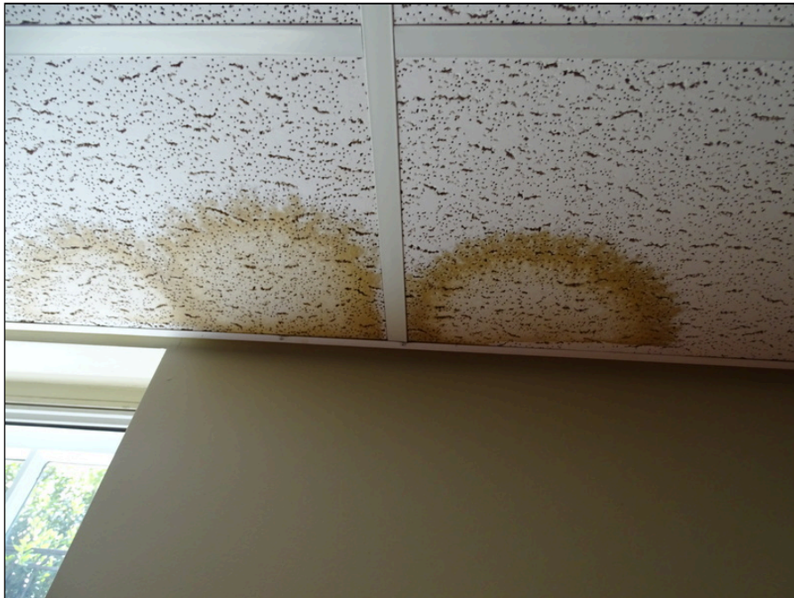
28 - Water leakage at ceiling
