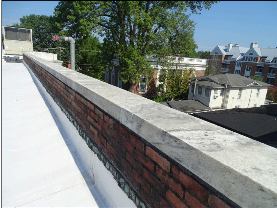
23 - Typical parapet wall - note patching
