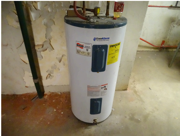
Electric domestic water heater
