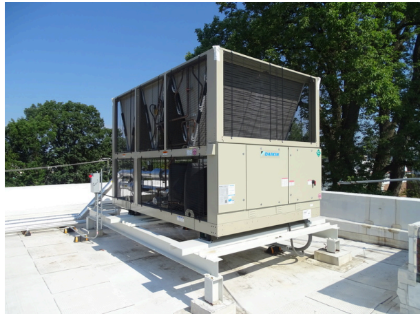
Condenser Unit located on roof
