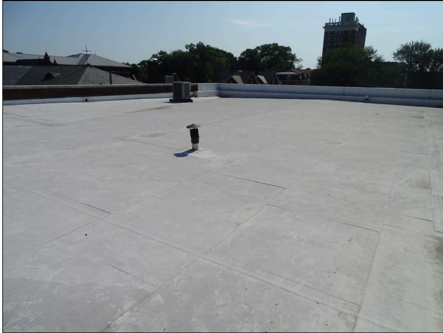
19 - Single-ply sheet membrane roofing system located at the northeast side of the building
