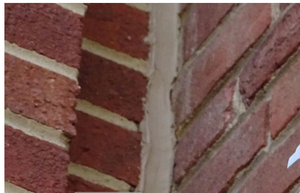
Exterior sealants - note deterioration
