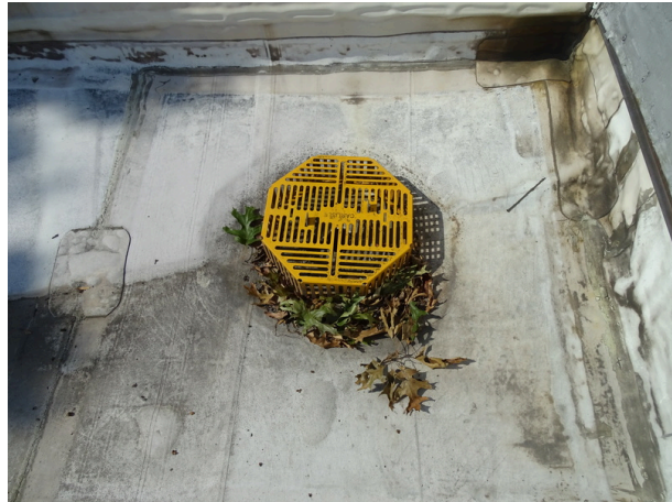
Typical internal drain
