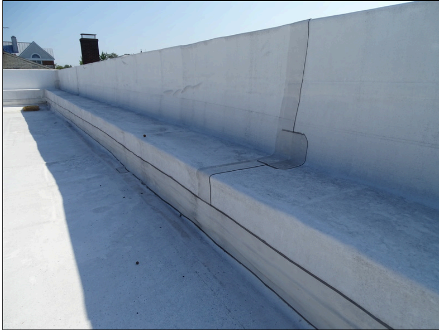
21 - Typical parapet wall - note patching
