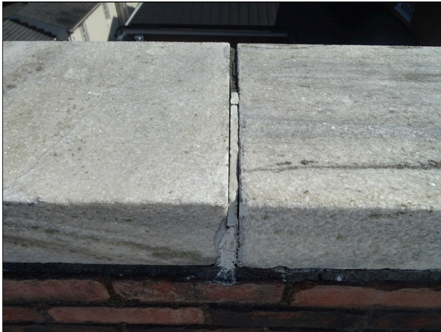
24 - Typical parapet wall - note mortar joint deterioration
