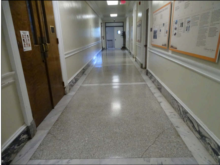
63 - Interior finishes corridor area - note cracking
