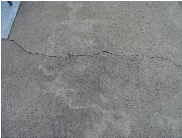
Concrete sidewalk - note cracking
