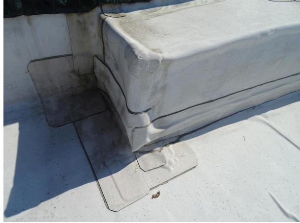
Typical parapet wall - note patching
