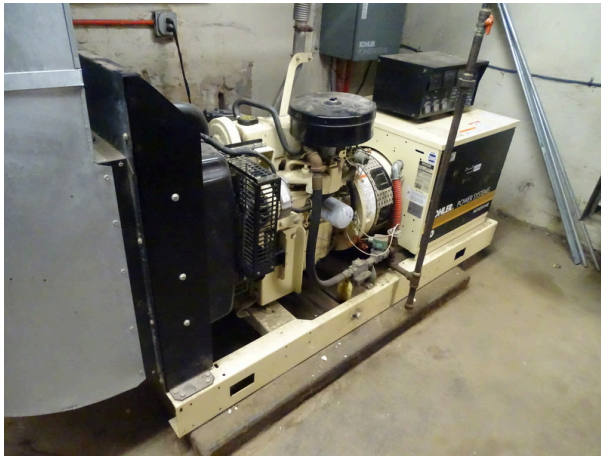
Emergency Power generator and transfer switch
