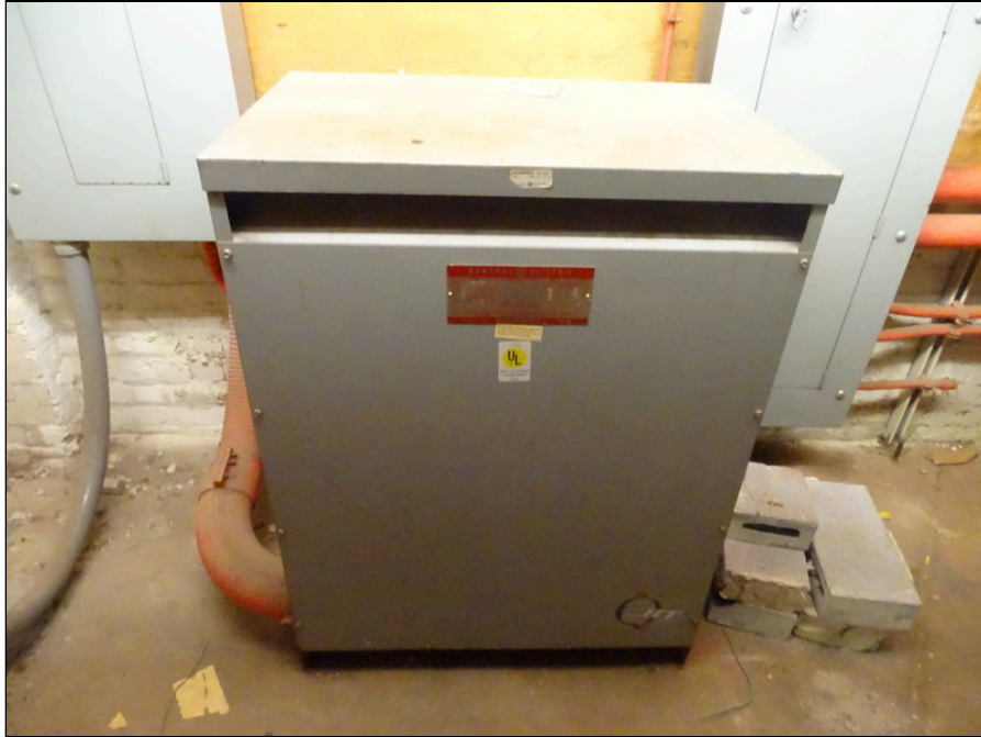
41 - Typical building transformer
