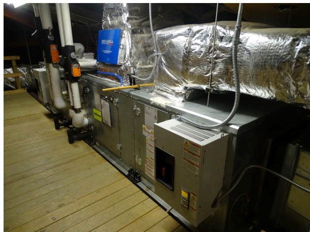
Air Handler Unit located in attic
