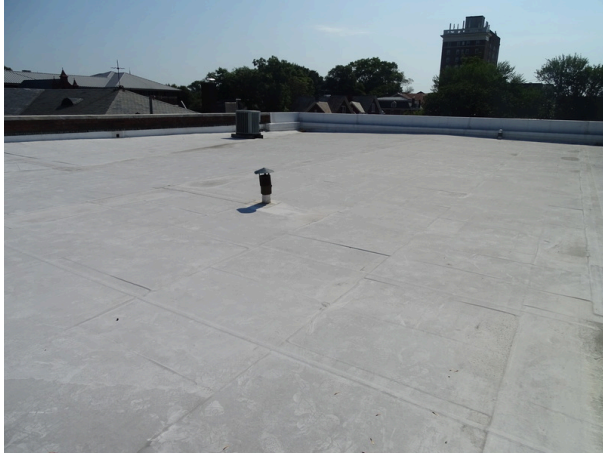
Single-ply sheet membrane roofing system located at the northeast side of the building
