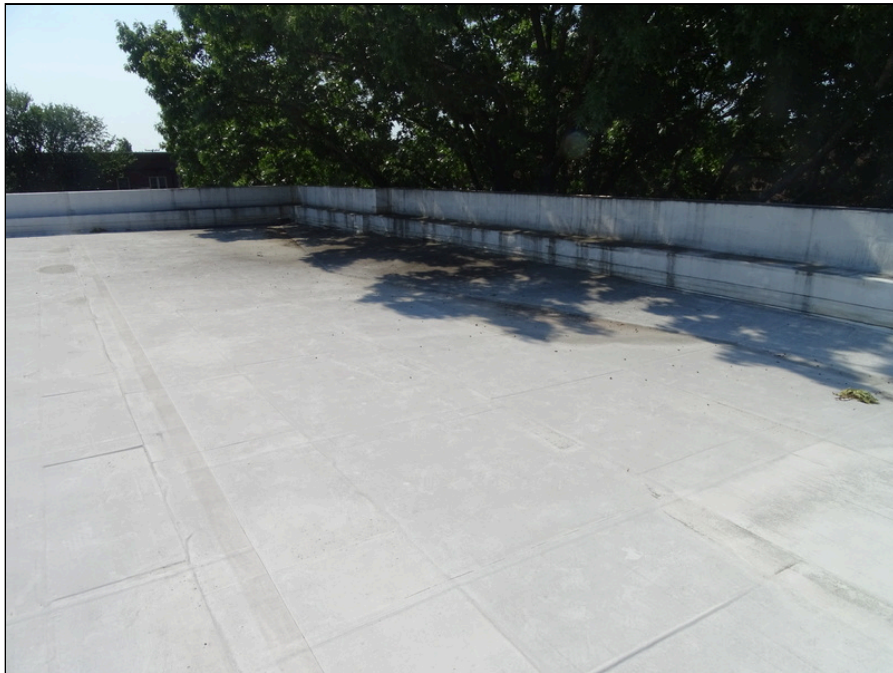
20 - Single-ply sheet membrane roofing system
