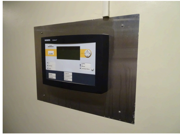
Fire alarm control panel
