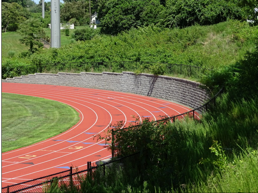
27 - Segmented block retaining wall at north side of track
