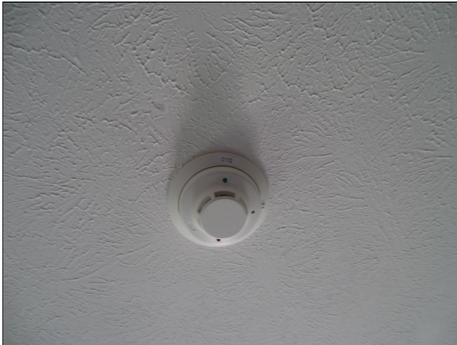
8 - PG Building smoke detector
