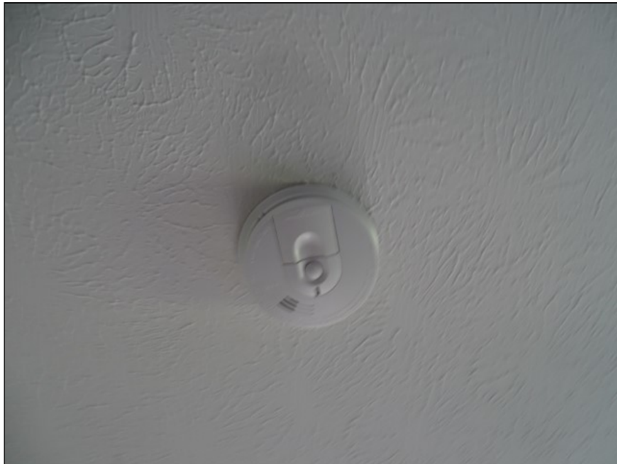
6 - PG Building smoke detector
