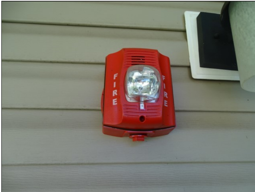
4 - PG Building typical horn/strobe
