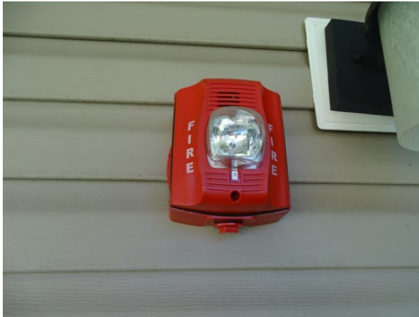
PG Building typical horn/strobe
