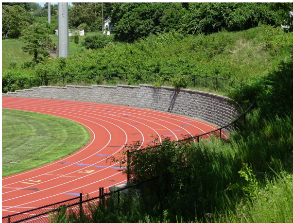
Segmented block retaining wall at north side of track
