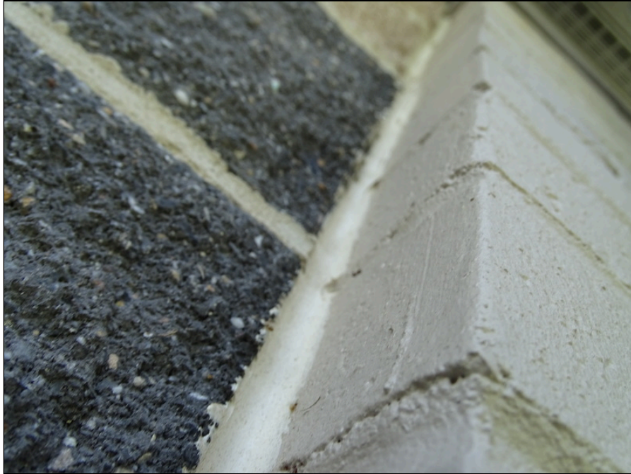
27 - Exterior sealant - note deterioration
