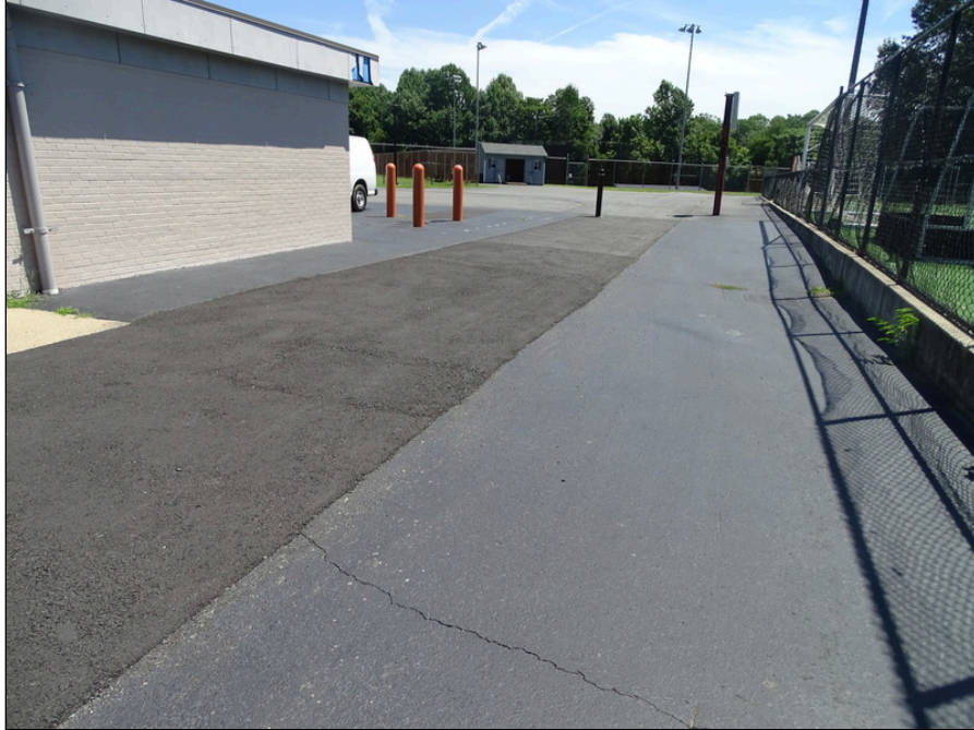
7 - Asphalt walkways - note cracking and previous repair
