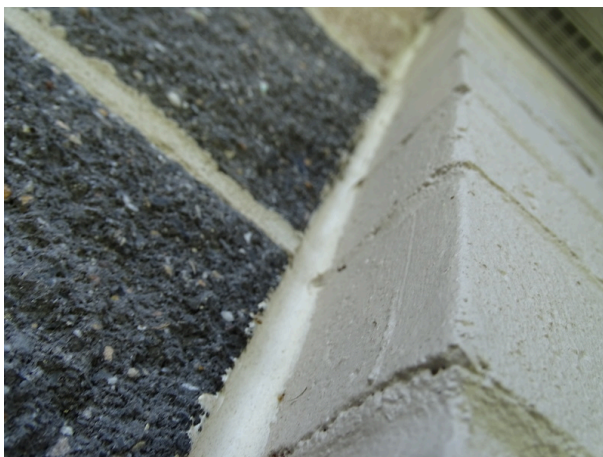
Exterior sealant - note deterioration
