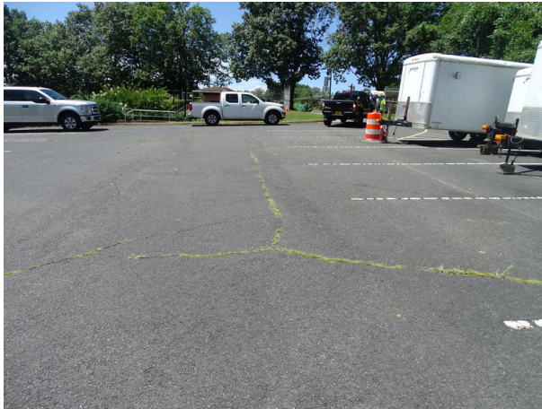
Asphalt pavement - note cracking
