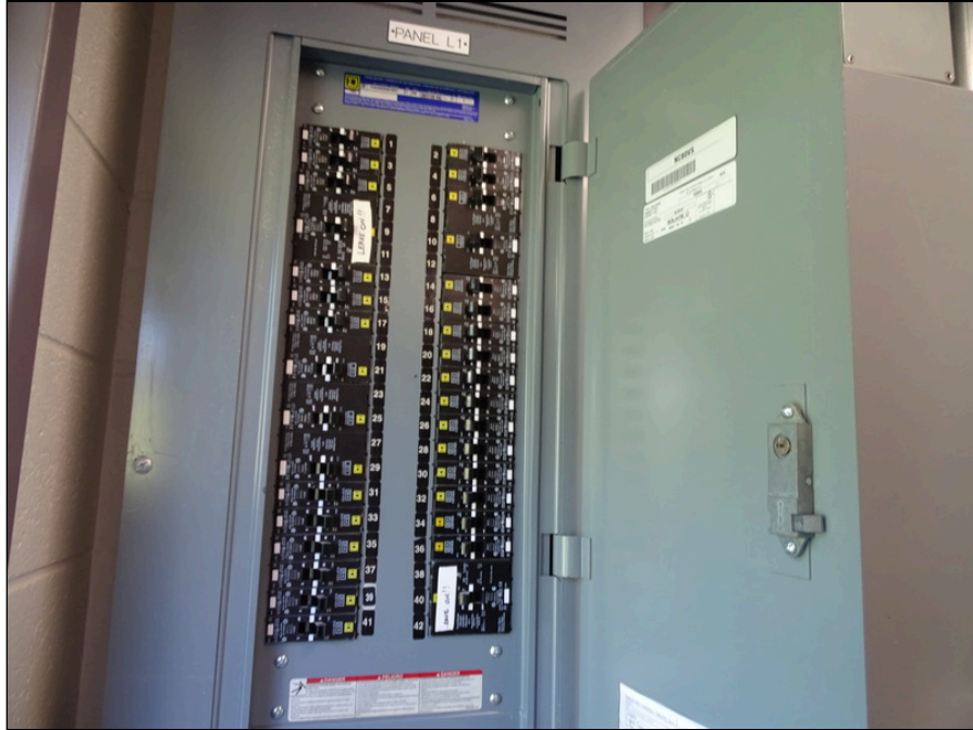
39 - Main electrical disconnect and circuit breaker panel at Maintenance Building
