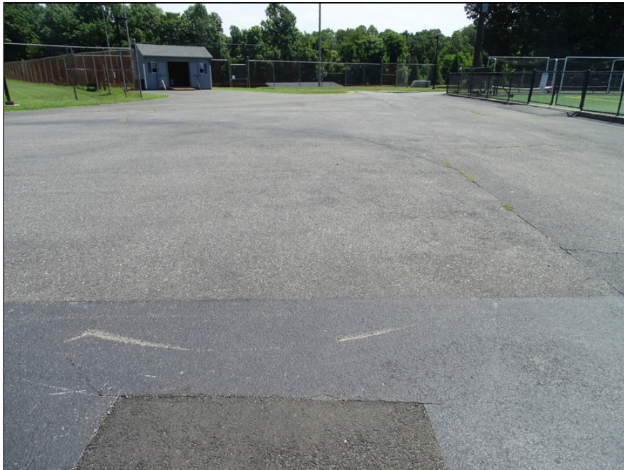
6 - Asphalt pavement - note cracking
