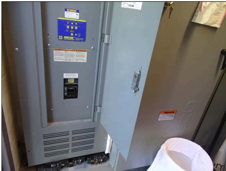
40 - Main switch disconnect
