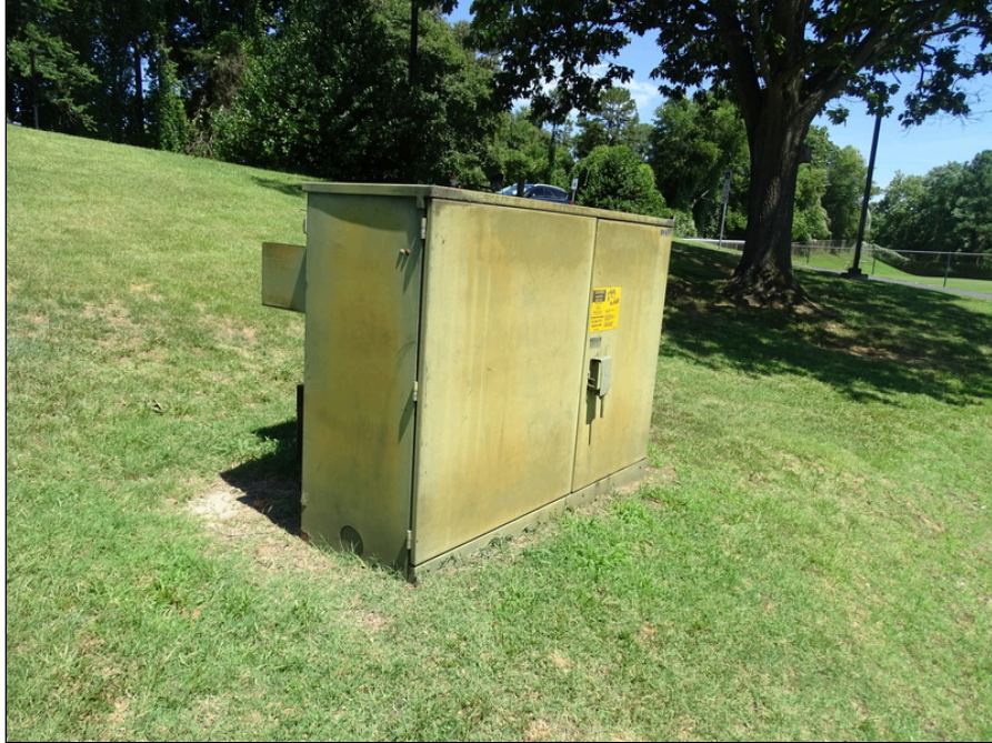
37 - Pad mounted electrical utility transformer servicing Field House Building
