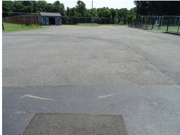
Asphalt pavement - note cracking
