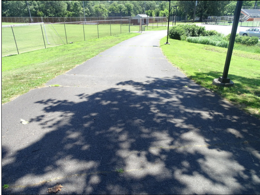
9 - Asphalt drive lane at northeast end of the site - note limited cracking
