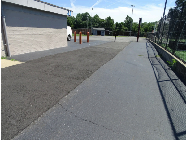
Asphalt walkways - note cracking and previous repair
