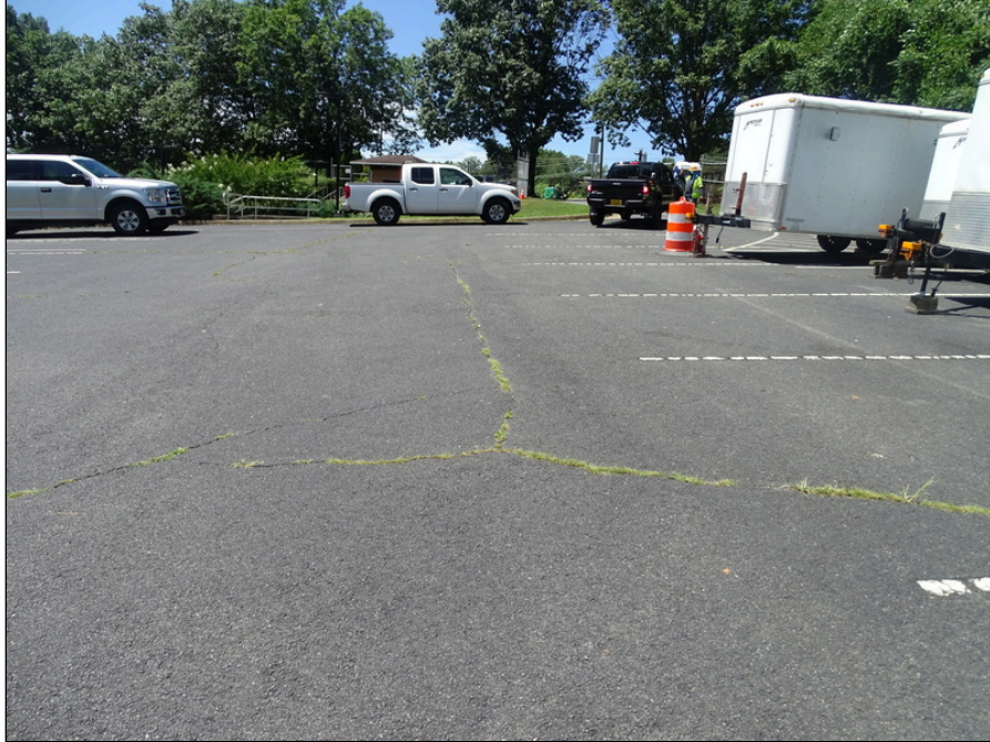
5 - Asphalt pavement - note cracking
