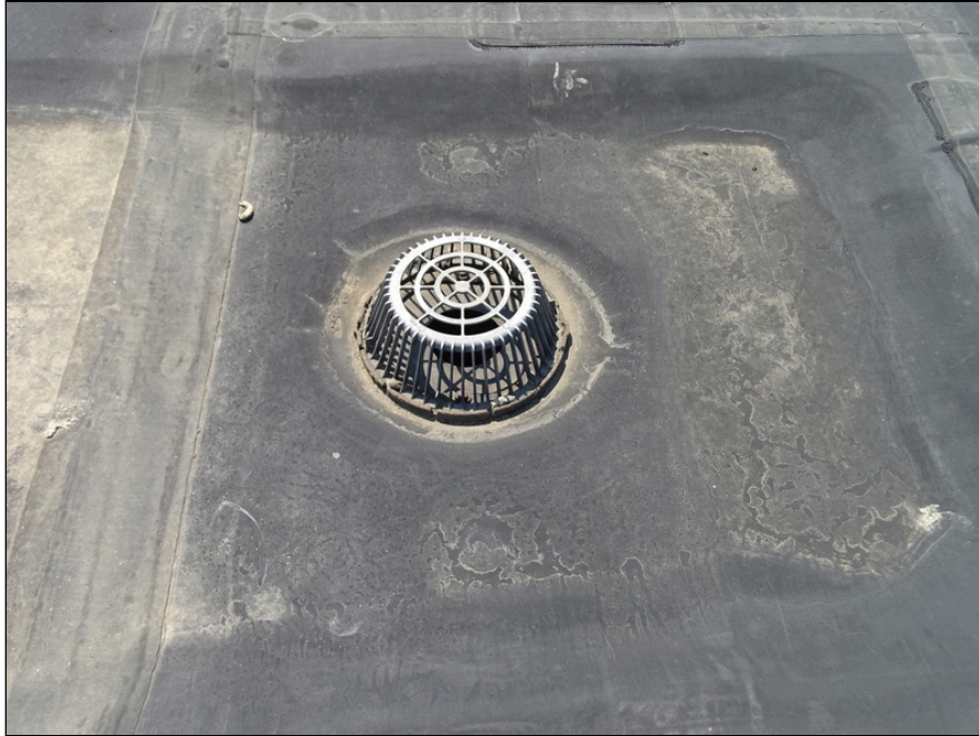
43 - Typical internal drain
