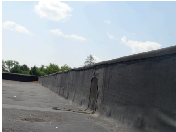
Single-ply membrane roofing system - note patching
