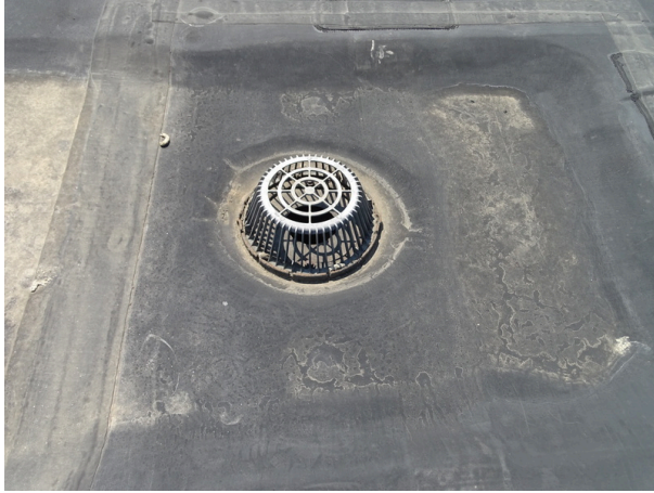
Typical internal drain
