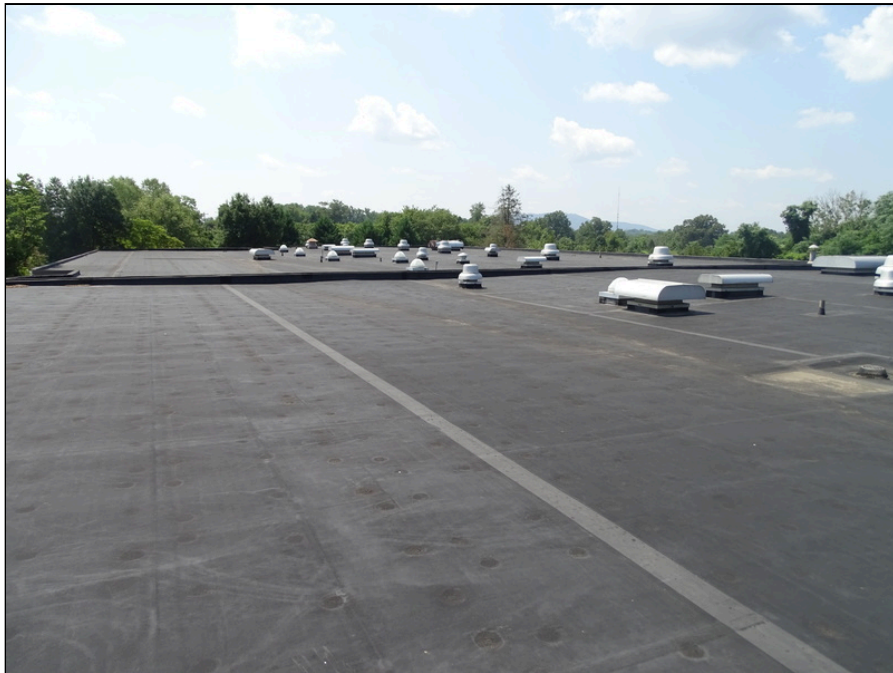
38 - Single-ply membrane roofing system looking south
