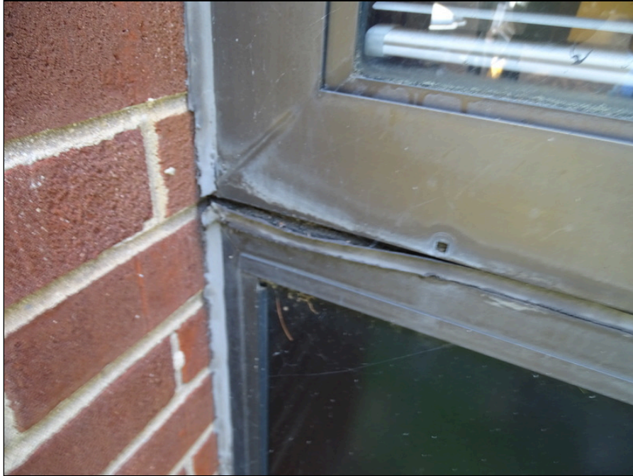
37 - Typical exterior windows - note gasket deterioration
