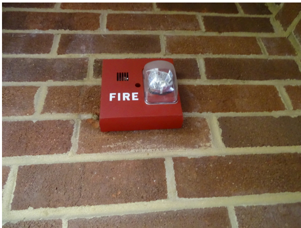
Typical fire alarm bell and strobe
