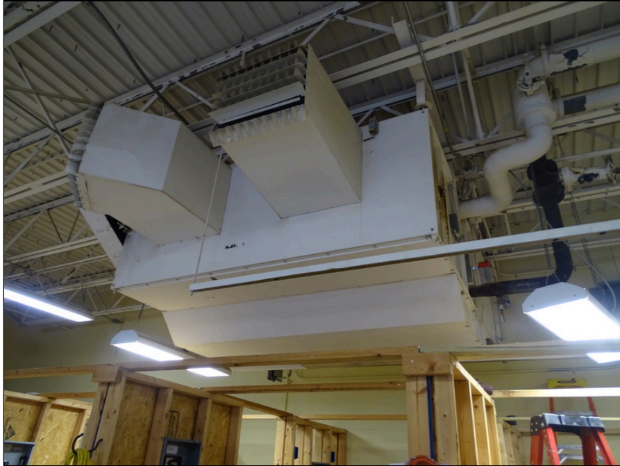
53 - Typical Unit Ventilator
