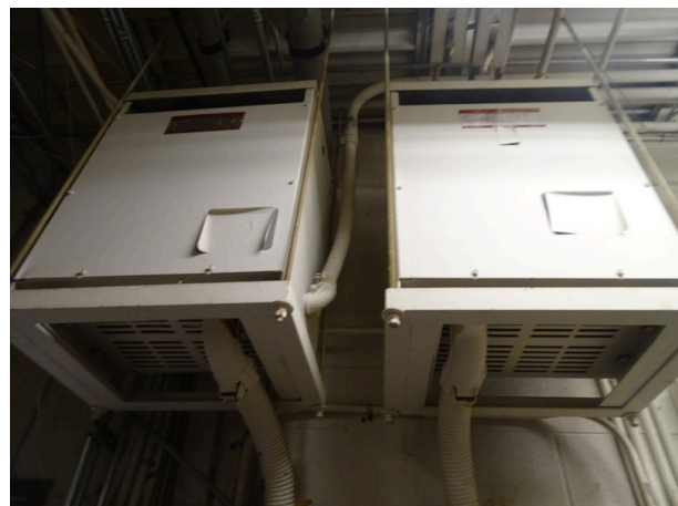
Typical building transformer
