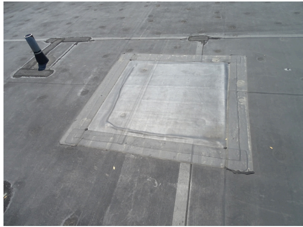
Single-ply membrane roofing system - note patching
