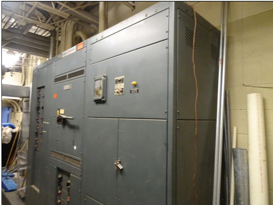
62 - Main electrical switchgear
