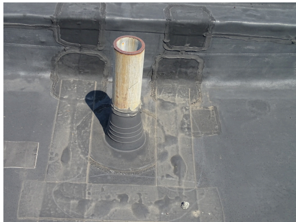
Typical plumbing penetration
