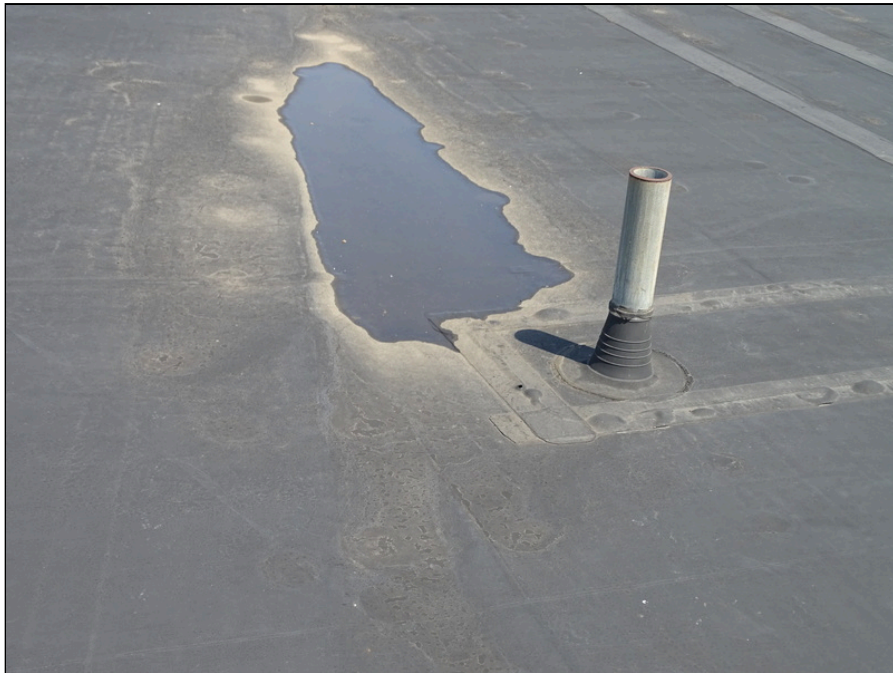
44 - Typical area of ponding
