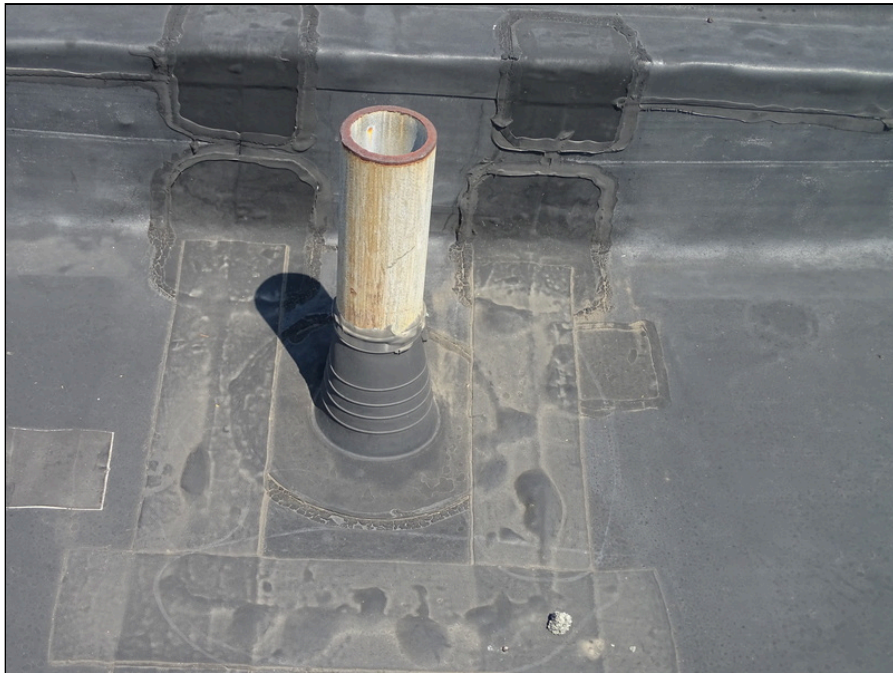
42 - Typical plumbing penetration
