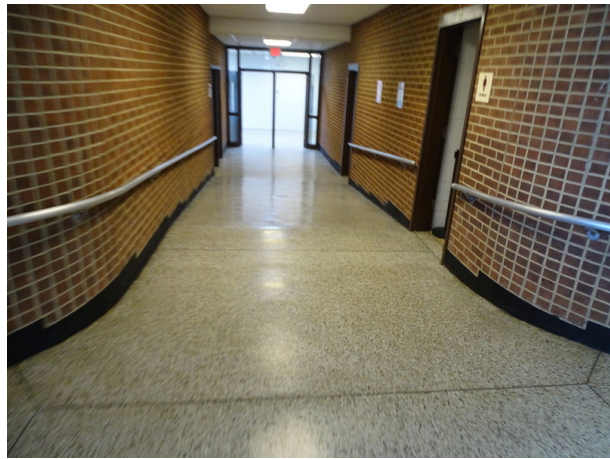
Accessible interior ramp
