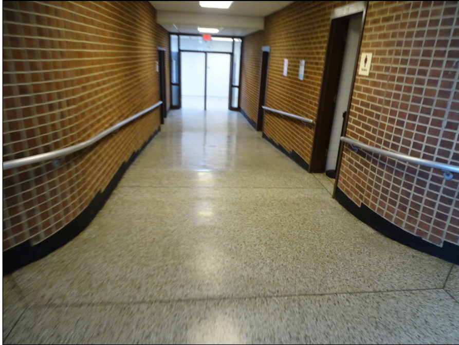
89 - Accessible interior ramp
