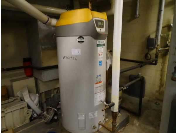
Gas water heater located in main utility room
