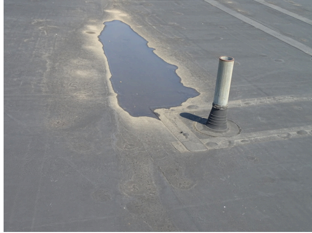
Typical area of ponding
