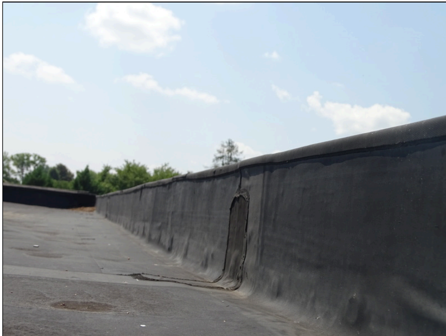
46 - Single-ply membrane roofing system - note patching
