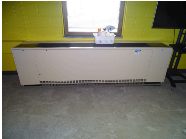
Typical larger Fan Coil Unit
