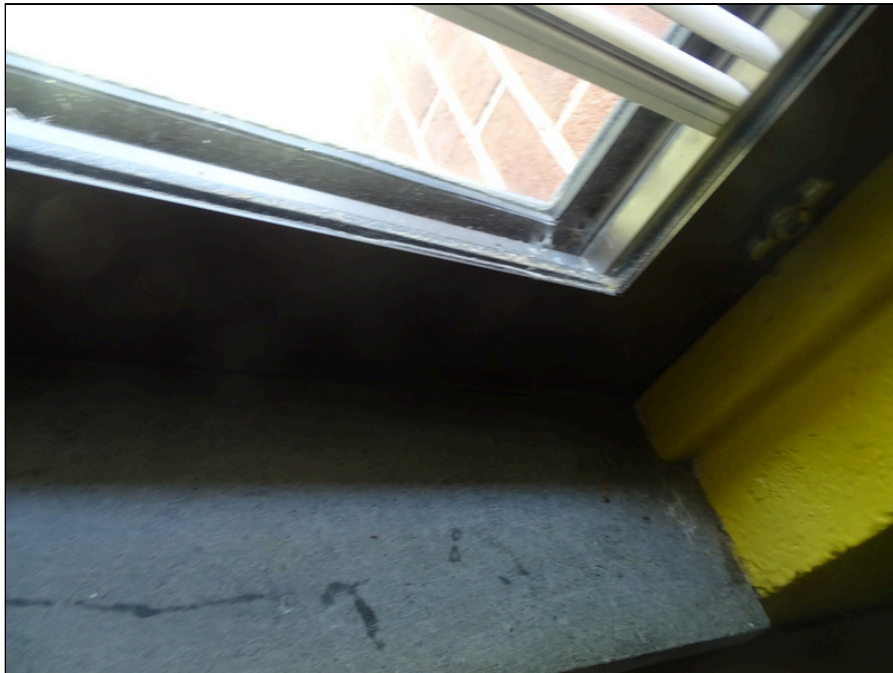
34 - Typical exterior windows - note fog inside the glass
