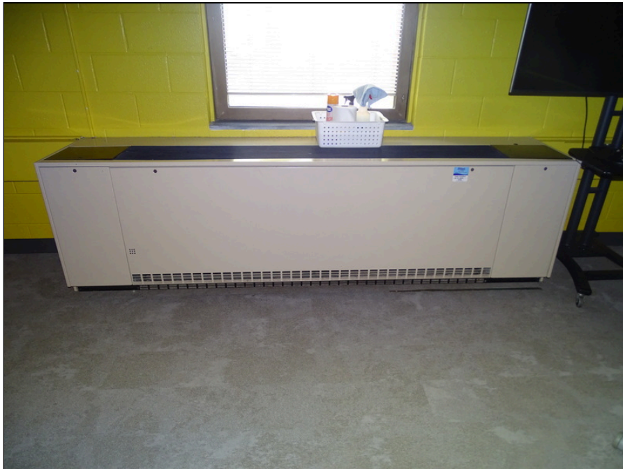
56 - Typical larger Fan Coil Unit
