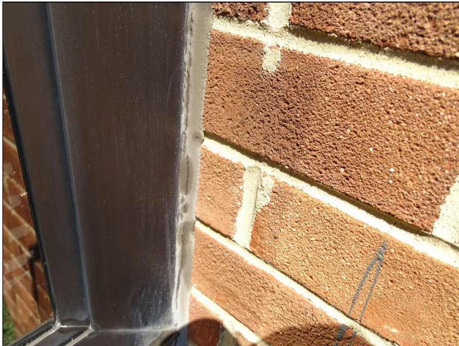
36 - Typical exterior windows - note sealant deterioration
