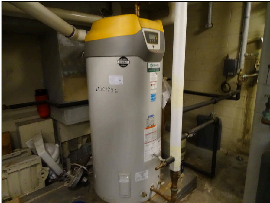
48 - Gas water heater located in main utility room
