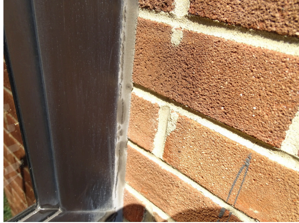
Typical exterior windows - note sealant deterioration
