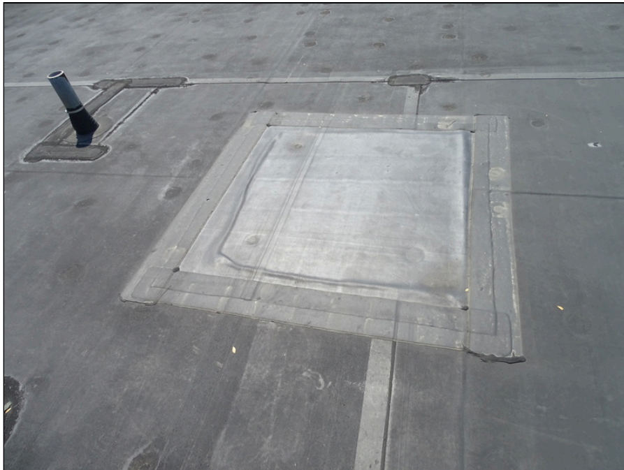
40 - Single-ply membrane roofing system - note patching
