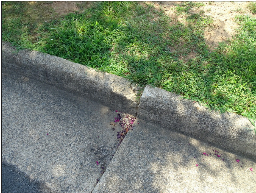
8 - Typical concrete curb - note deterioration
