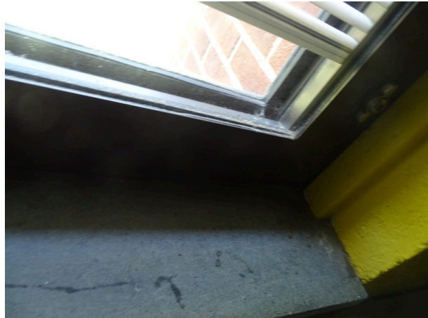
Typical exterior windows - note fog inside the glass
