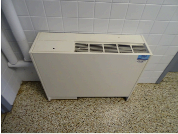
Typical Fan Coil Unit
