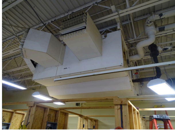
Typical Unit Ventilator
