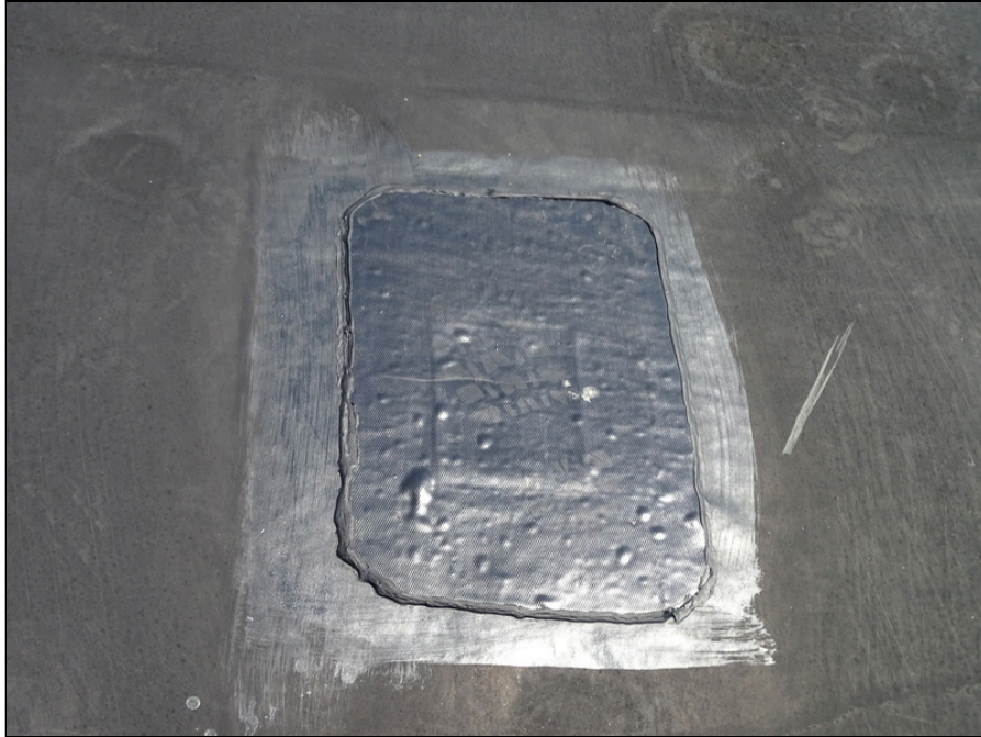
41 - Single-ply membrane roofing system - note patching
