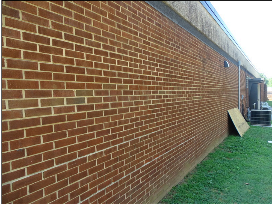
27 - Building exterior east side of the building - note efflorescence
