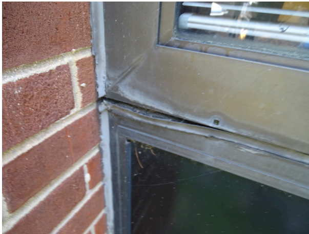
Typical exterior windows - note gasket deterioration
