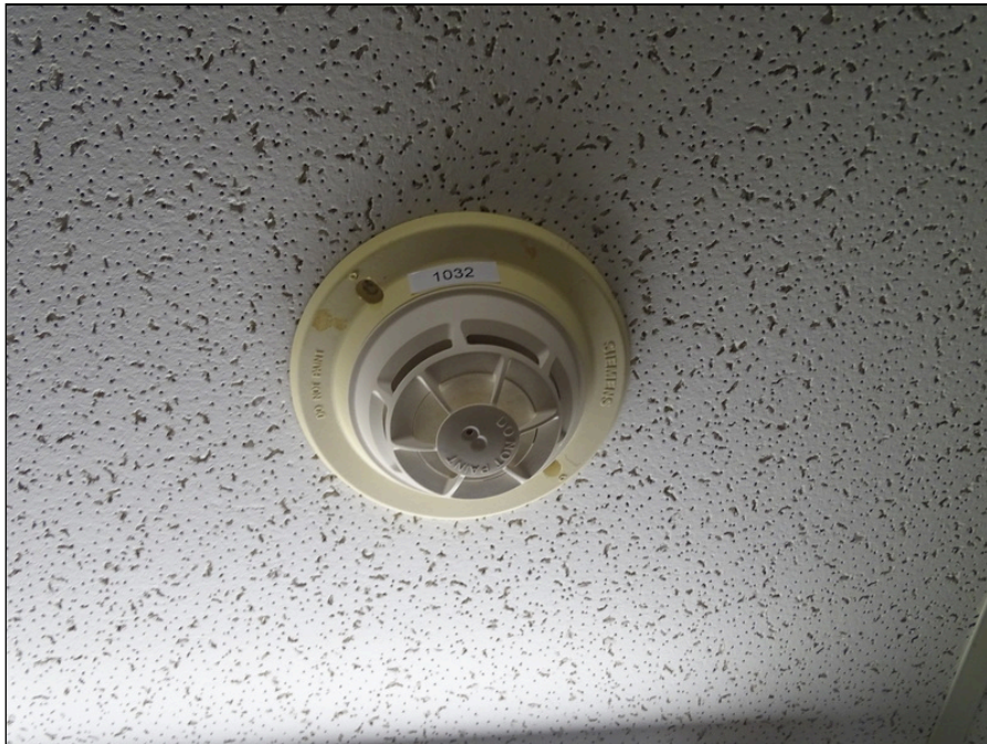
72 - Typical smoke detector
