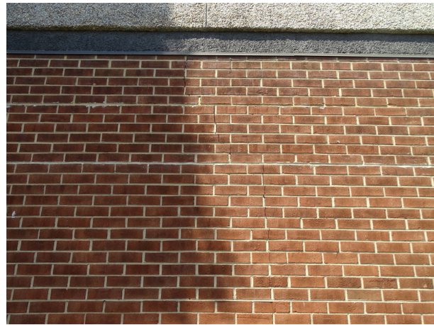
Building exterior southeast side of the building - note cracking
