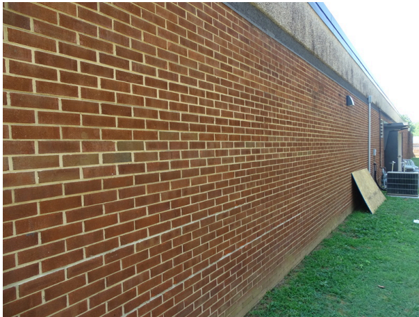
Building exterior east side of the building - note efflorescence
