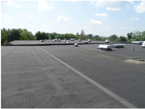
Single-ply membrane roofing system looking south
