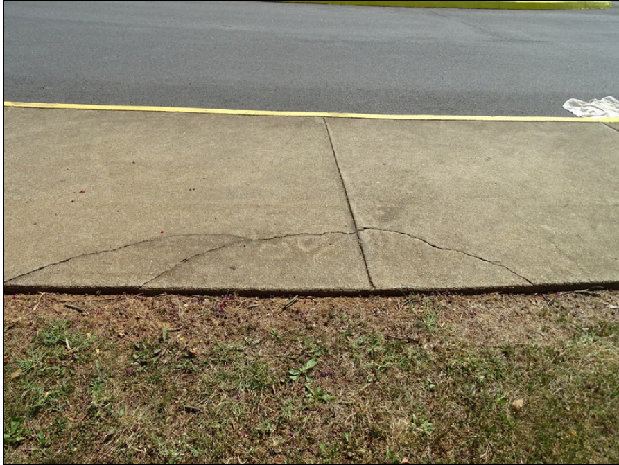
5 - Typical concrete sidewalk - note cracking
