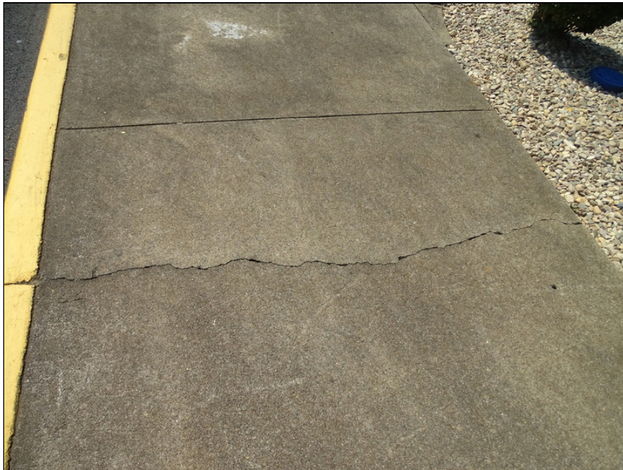
6 - Typical concrete sidewalk - note cracking
