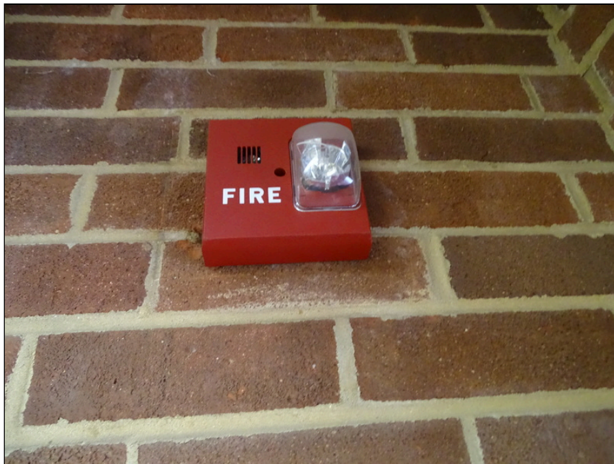
70 - Typical fire alarm bell and strobe
