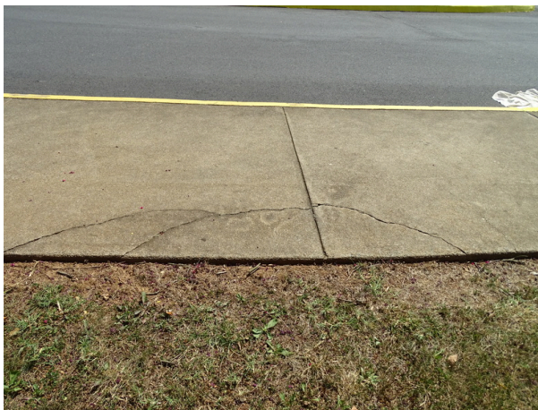
Typical concrete sidewalk - note cracking
