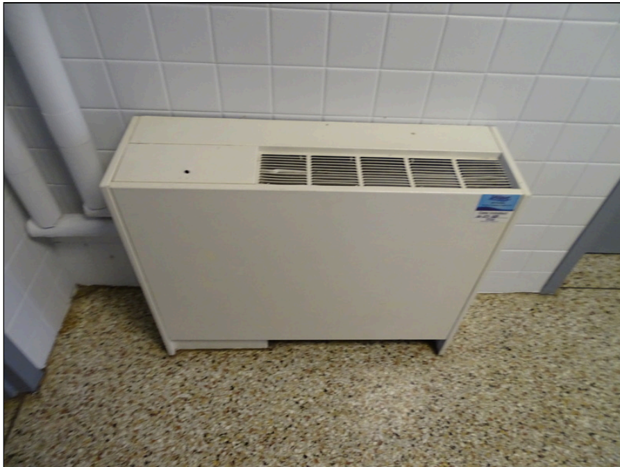
52 - Typical Fan Coil Unit
