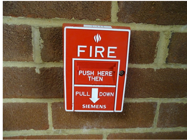
Typical fire alarm pull station
