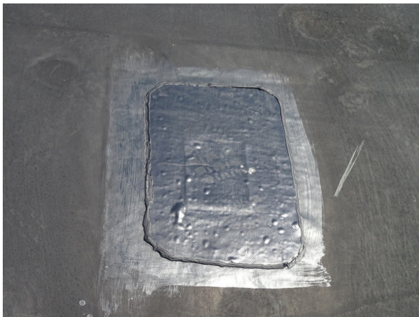
Single-ply membrane roofing system - note patching
