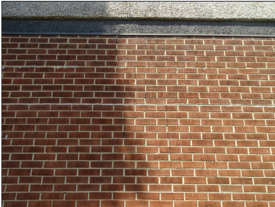
24 - Building exterior southeast side of the building - note cracking
