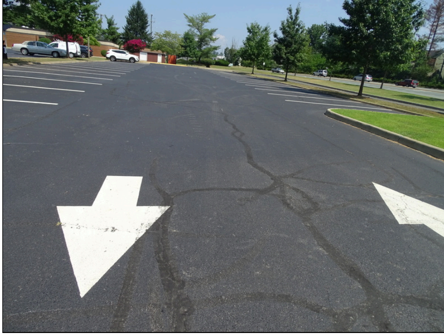
3 - Asphalt pavement center drive lane looking north - note previous repair
