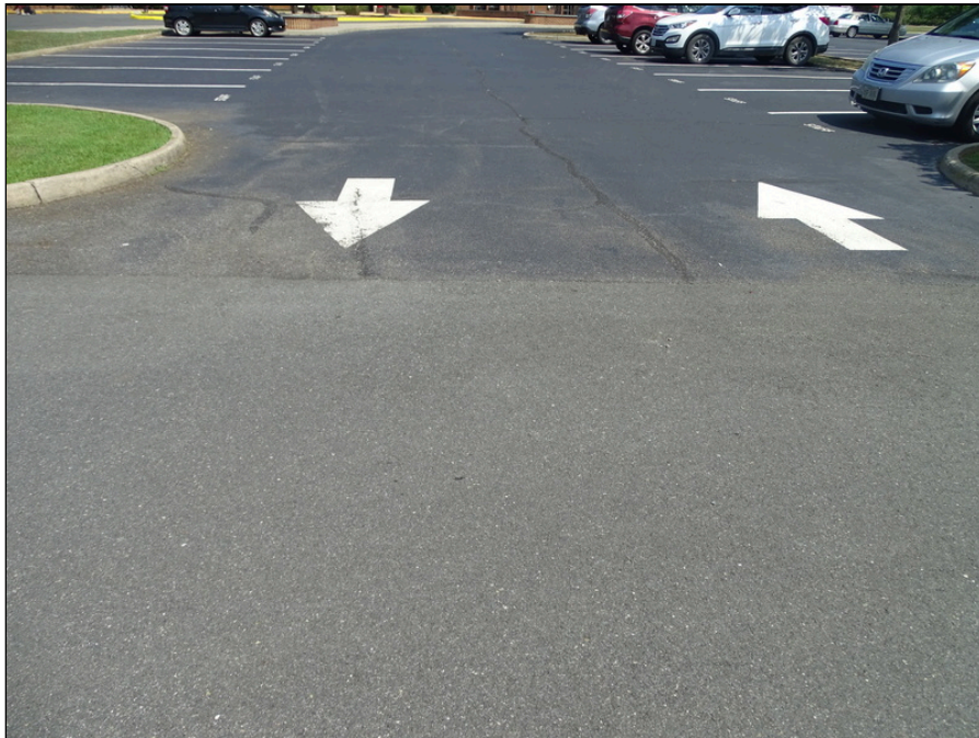
2 - Asphalt pavement center drive lane looking north - note previous repair
