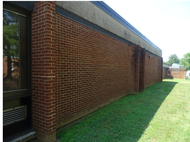
Building exterior northwest side of the building - note efflorescence
