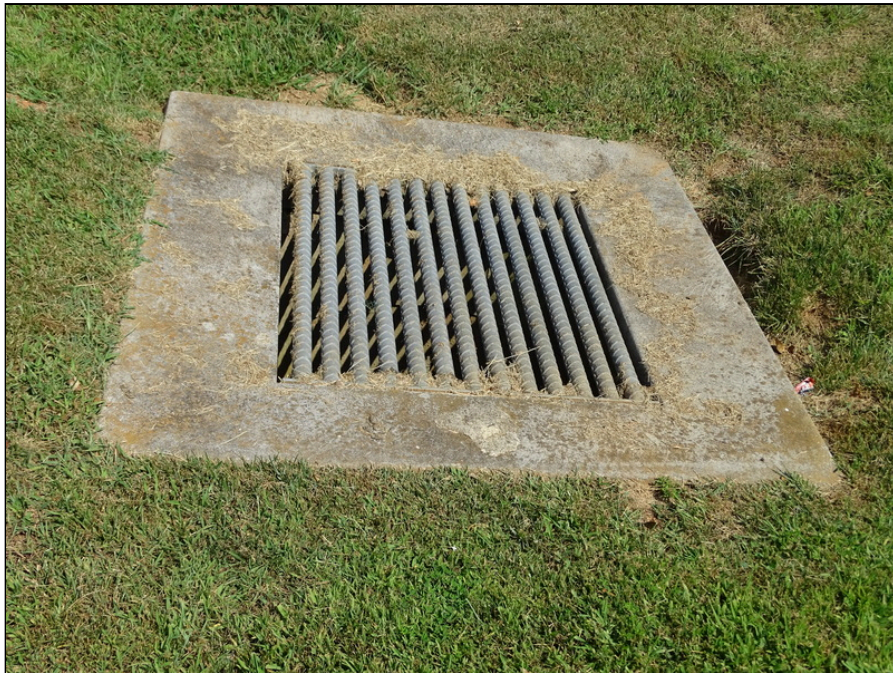
10 - Typical storm water drainage
