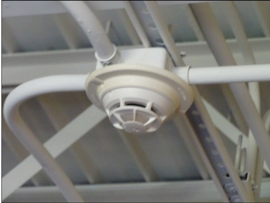
71 - Typical smoke detector
