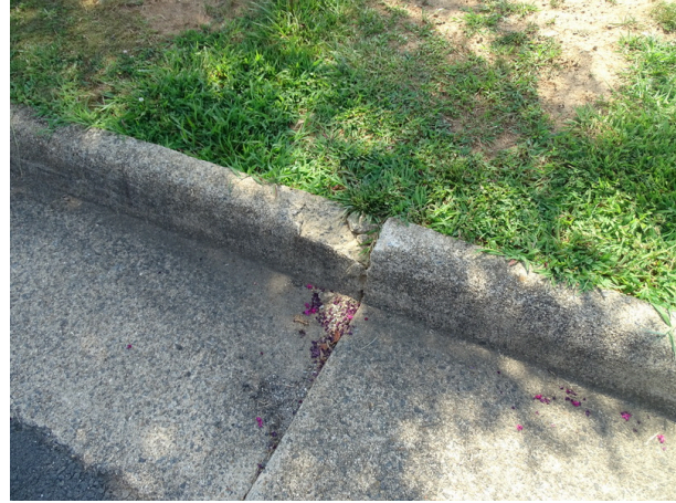
Typical concrete curb - note deterioration
