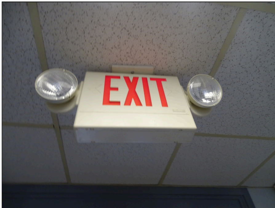
68 - Typical exit sign and emergency light
