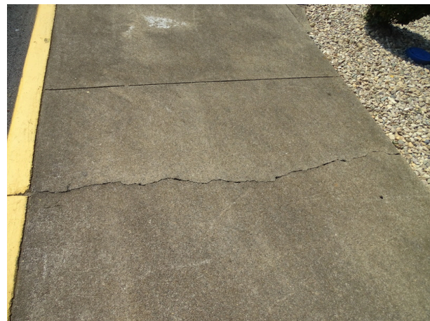
Typical concrete sidewalk - note cracking
