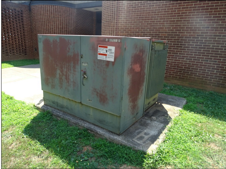
61 - Utility electrical transformer
