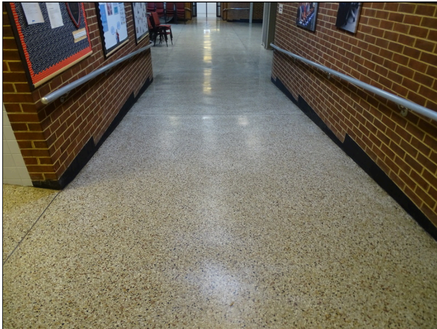
90 - Accessible interior ramp
