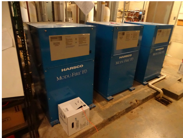
Boilers located in main utility room
