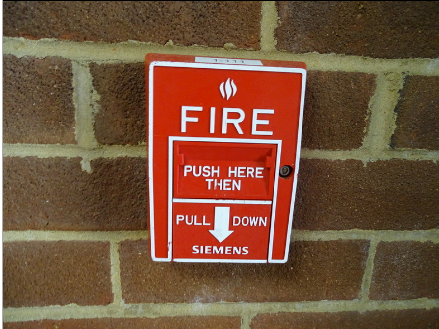
69 - Typical fire alarm pull station
