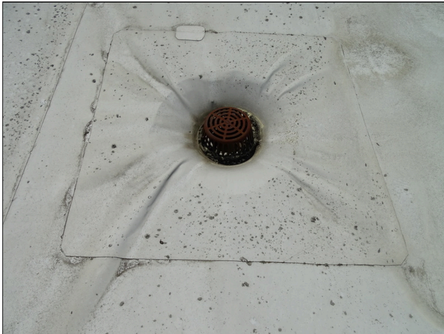
56 - Building C roof - internal drainage
