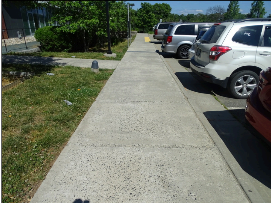
15 - Concrete sidewalk - note spalling
