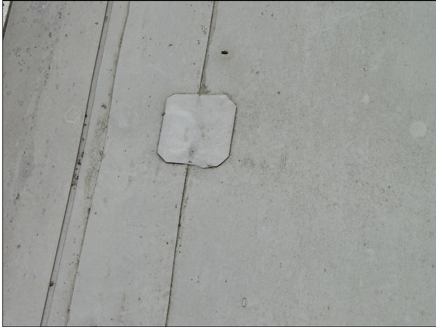
57 - Building C roof - patching
