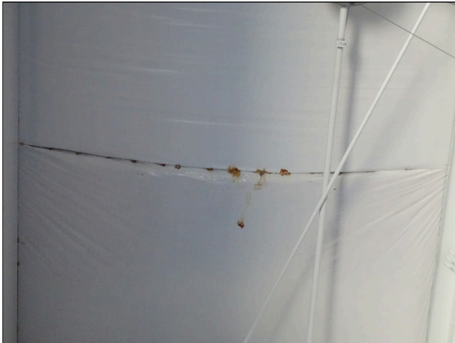
120 - Water leakage
