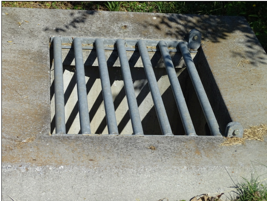
18 - Typical storm sewer drop inlet
