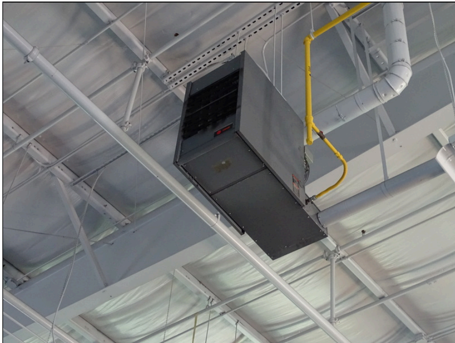
70 - Building B unit heater
