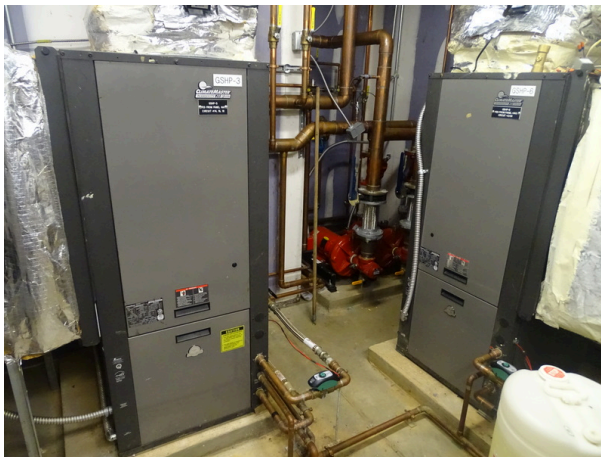
Building A geothermal heat pump
