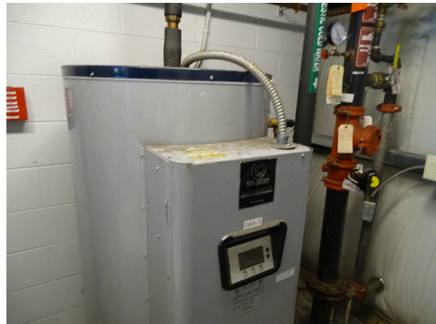
Building B water heater
