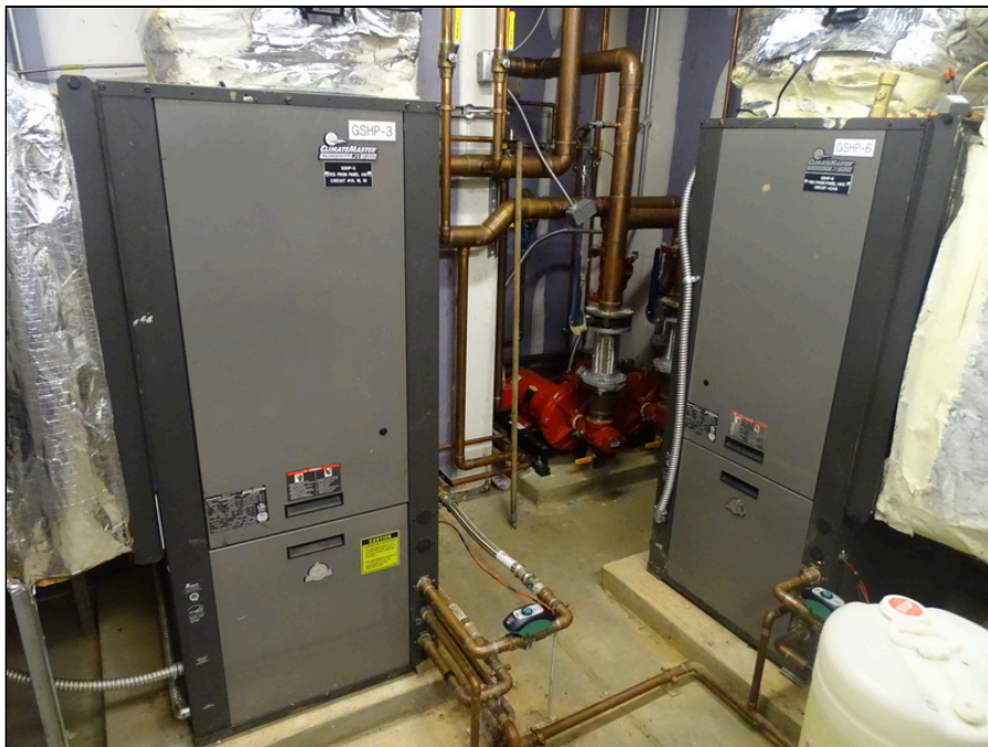
66 - Building A geothermal heat pump
