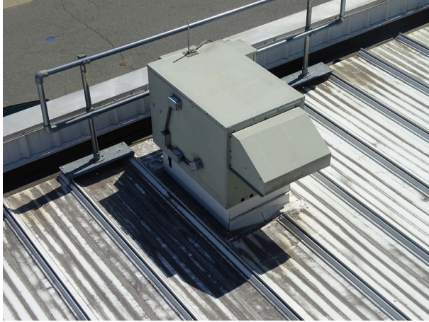
Building B energy recovery system
