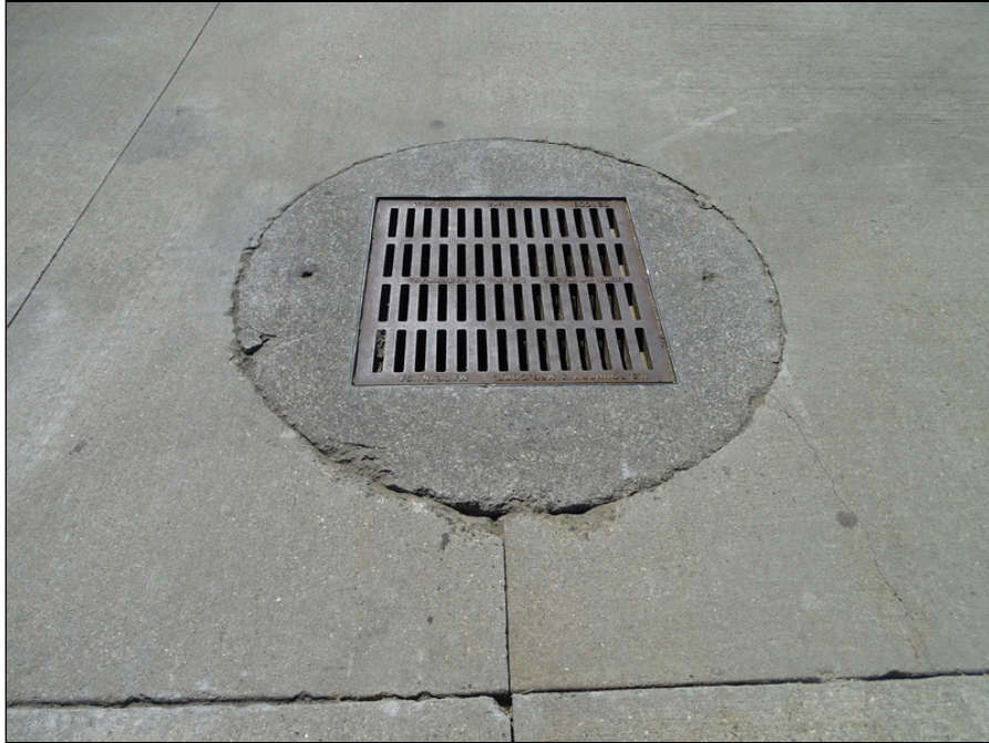
17 - Typical storm sewer drop inlet
