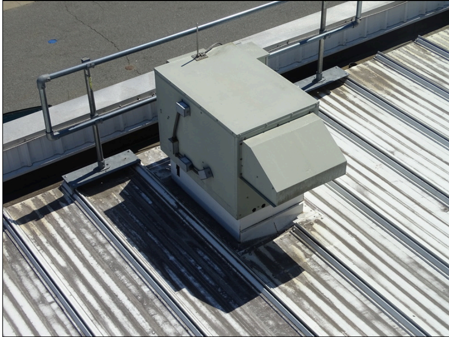
69 - Building B energy recovery system
