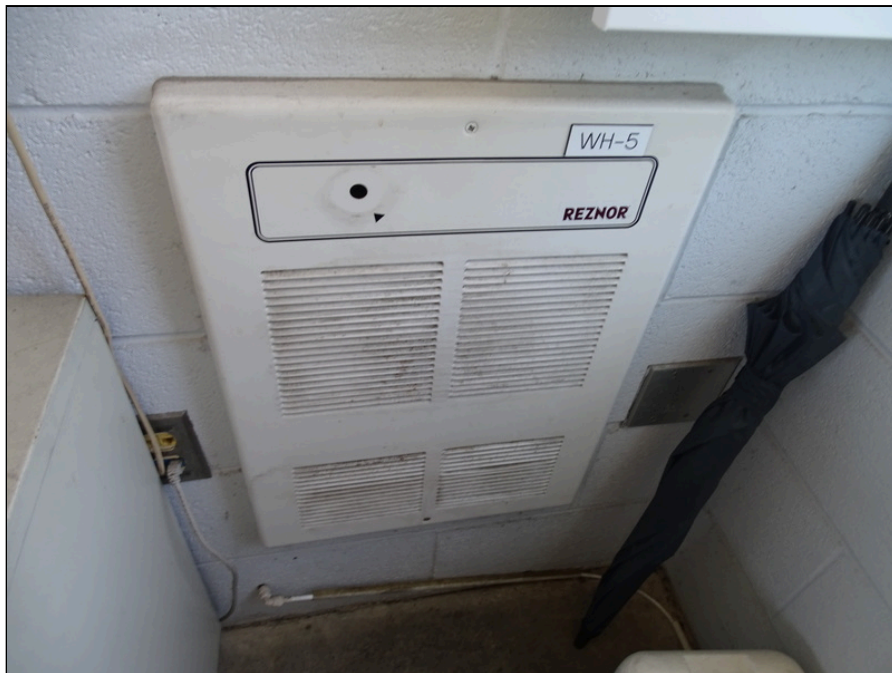
74 - Building C unit heater
