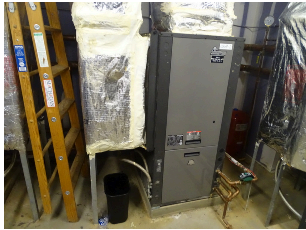
Building A geothermal heat pump
