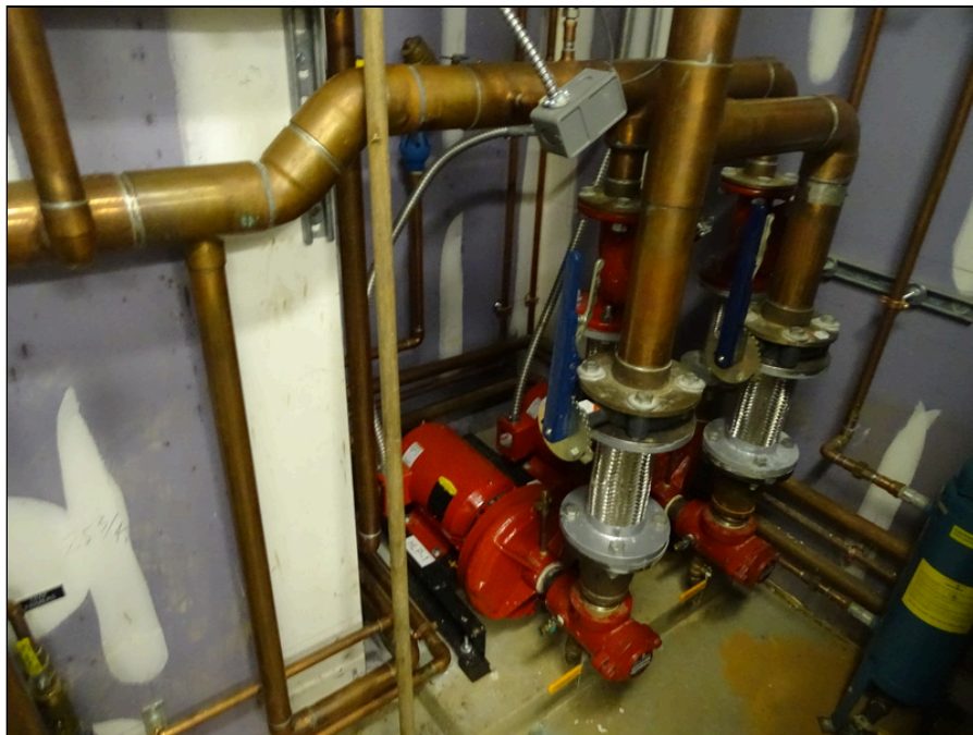
64 - Building A geothermal heat pump
