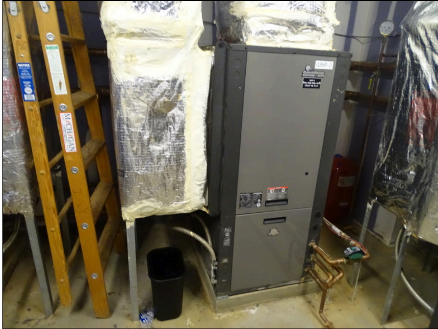
65 - Building A geothermal heat pump
