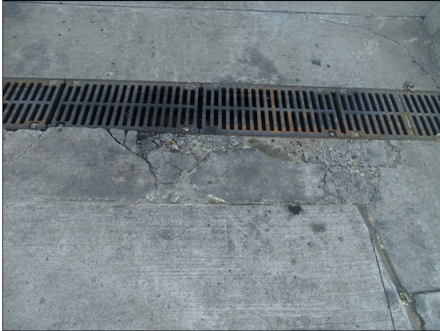
19 - Typical storm sewer drop inlet
