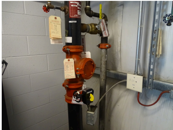
Building B sprinkler riser
