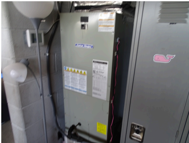
Building C electric heater and thermostat
