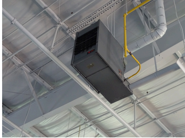
Building B unit heater
