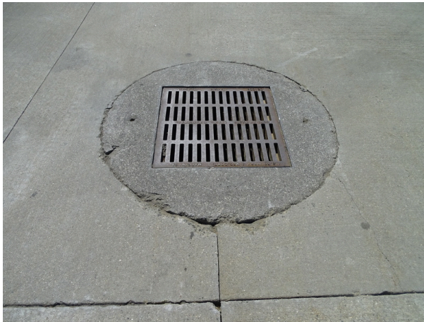
Typical storm sewer drop inlet
