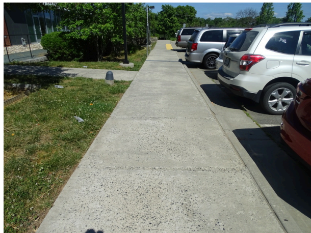
Concrete sidewalk - note spalling
