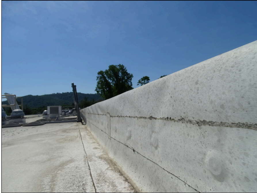
55 - Building C roof - parapet wall deterioration
