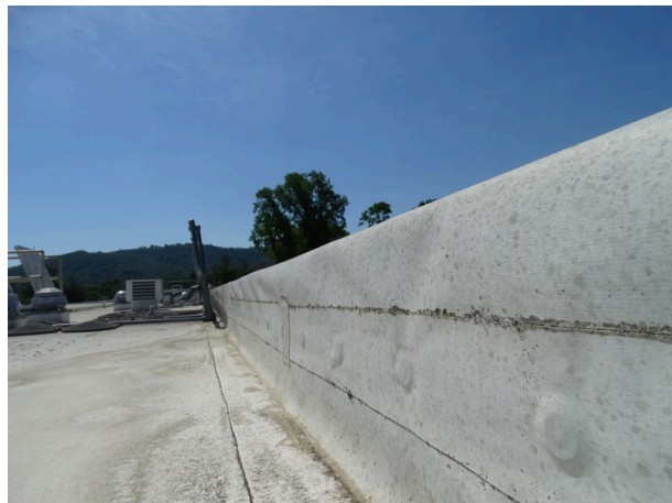
Building C roof - parapet wall deterioration
