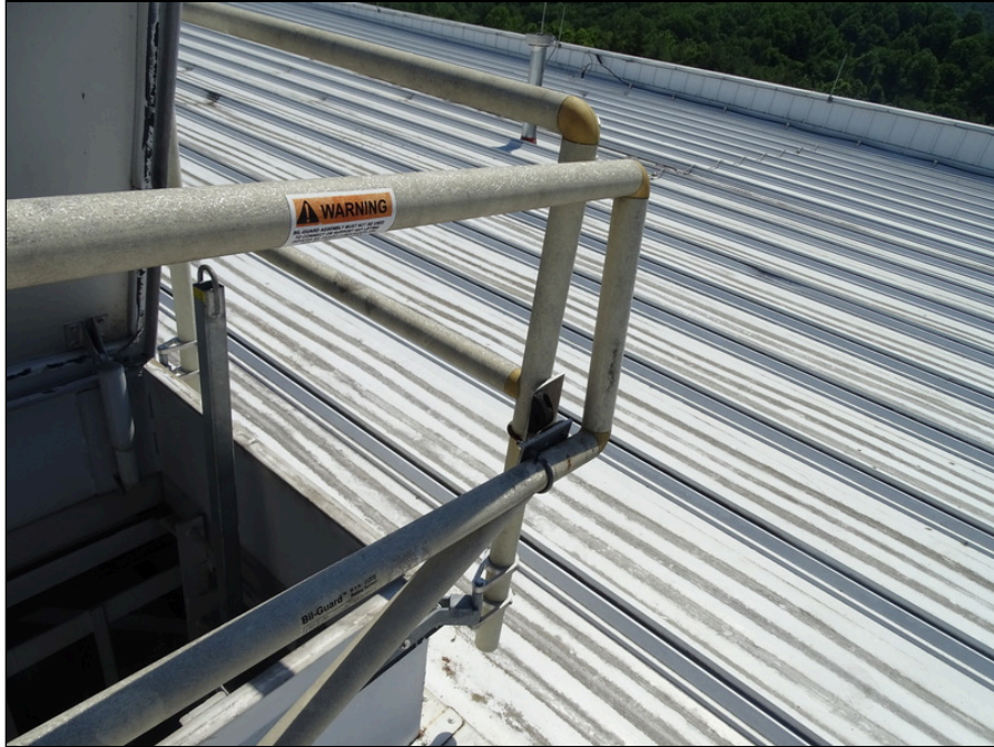
45 - Roof safety railing
