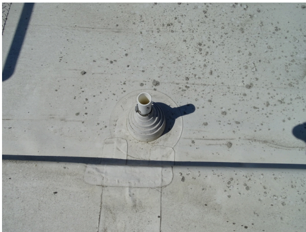
Building C roof - plumbing penetration
