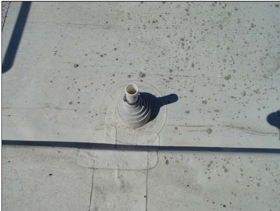
54 - Building C roof - plumbing penetration
