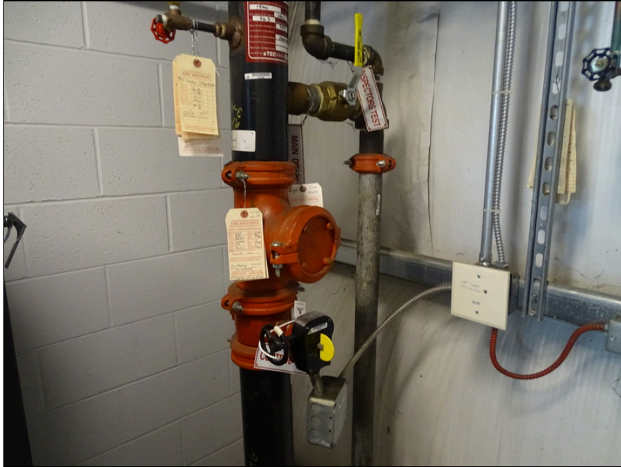
87 - Building B sprinkler riser
