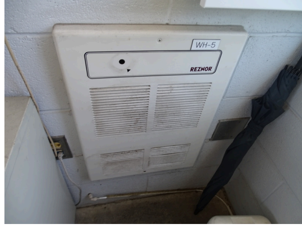
Building C unit heater
