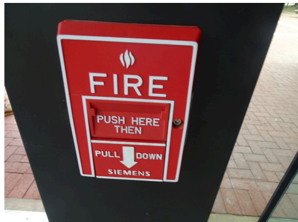
Typical fire alarm pull station
