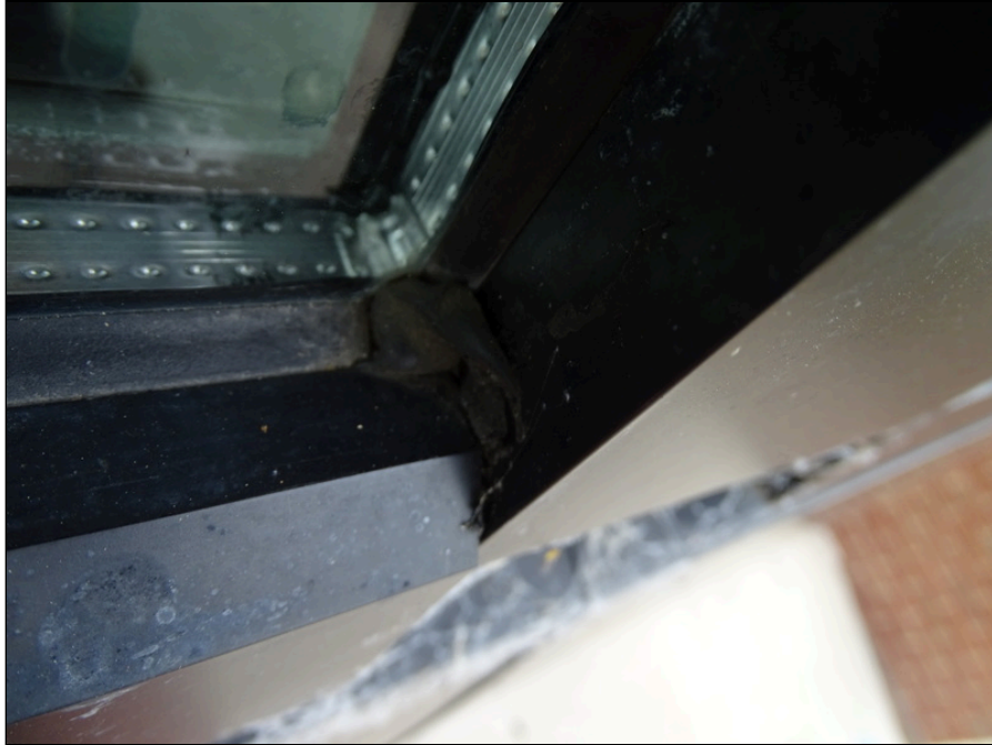
25 - Typical exterior window - note gasket deterioration
