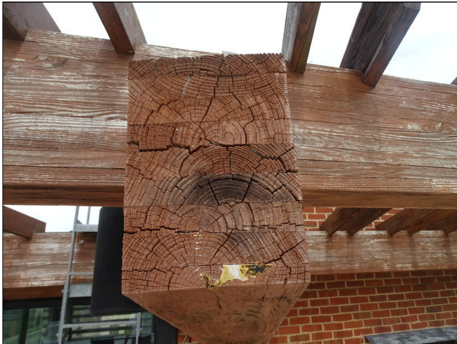
14 - Wood accent on the east side of the building - note cracking
