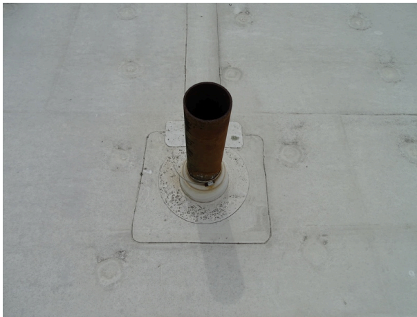
Typical plumbing penetration
