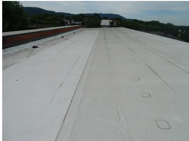
Single-ply membrane roofing system looking south
