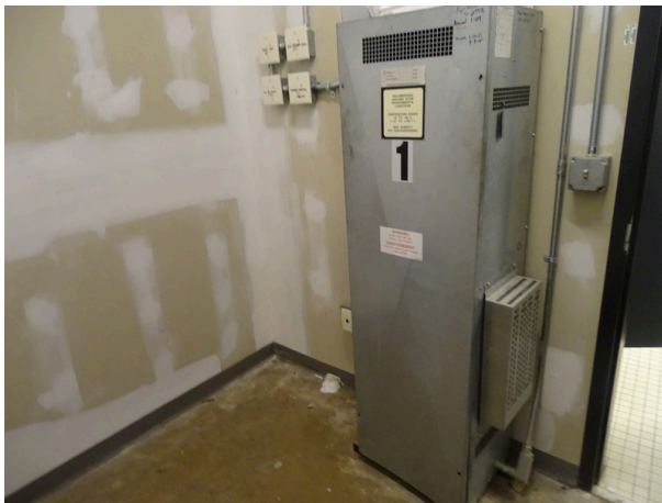
Elevator machine and controls
