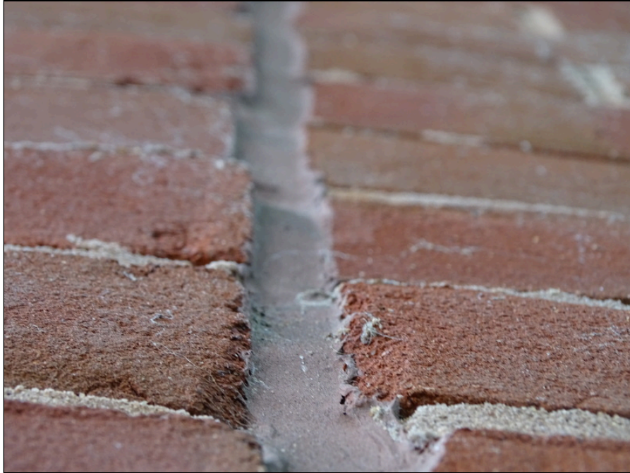
17 - Exterior wall - note sealant deterioration
