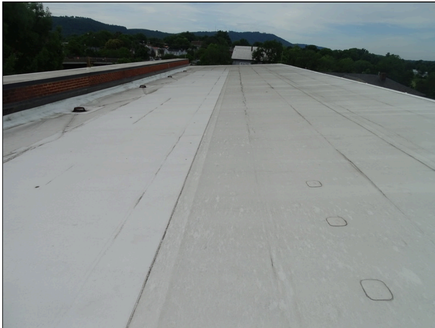
28 - Single-ply membrane roofing system looking south
