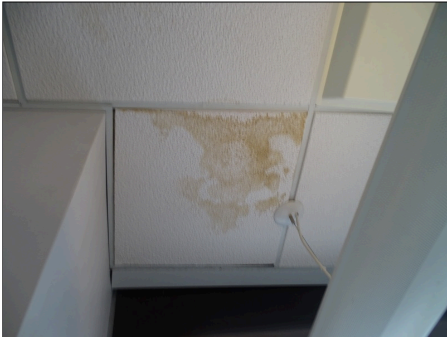
30 - Area of reported leakage of roofing system
