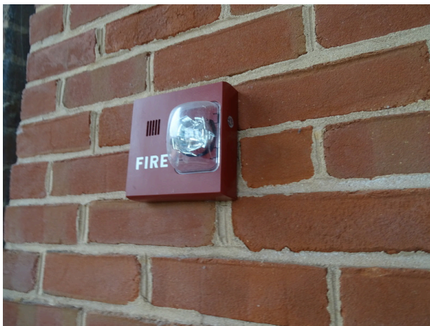
Typical fire alarm bell and strobe
