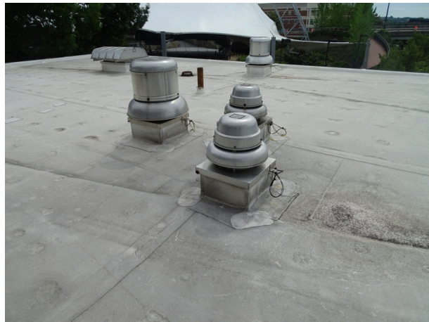
Typical exhaust fan
