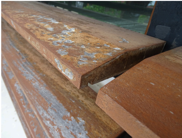
Wood shade screen on west side of the building - note deterioration
