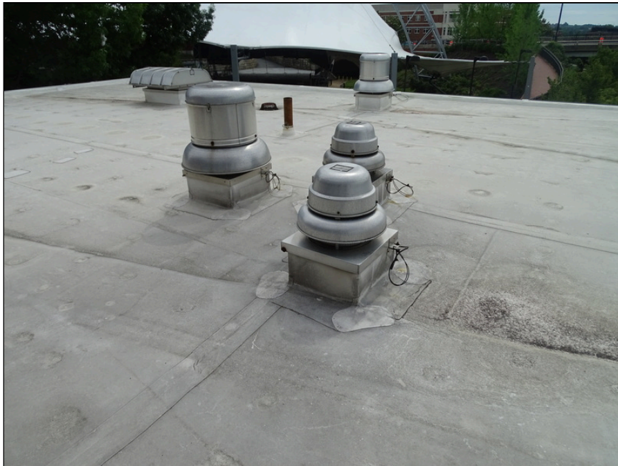
34 - Typical exhaust fan
