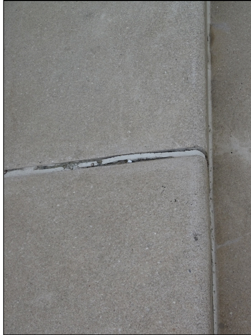
5 - Concrete steps at the west side of the building - note sealant deterioration
