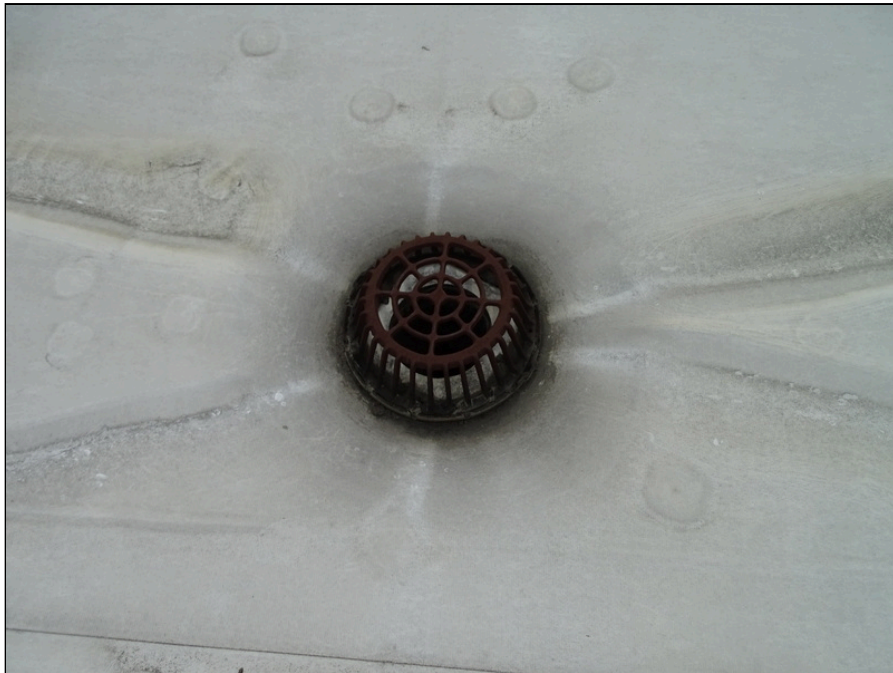
32 - Typical internal drain
