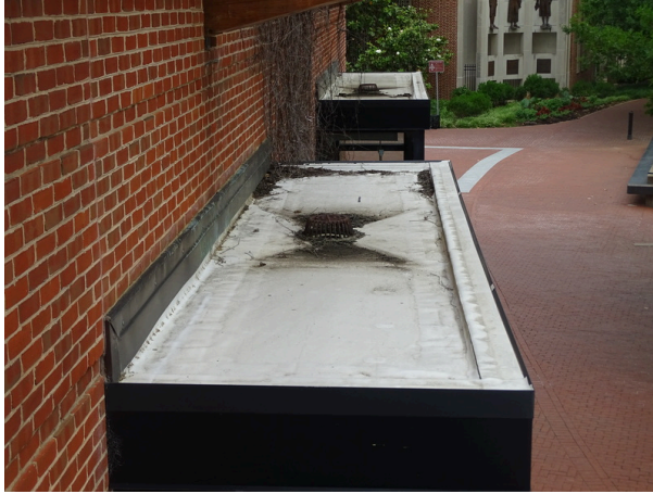
Single-ply membrane roofing system
