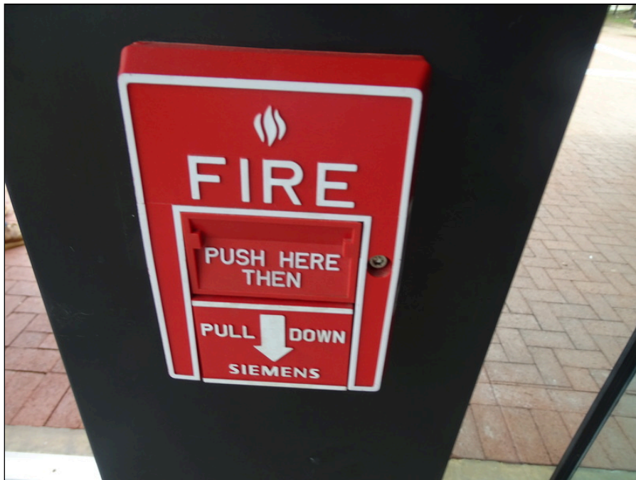
58 - Typical fire alarm pull station
