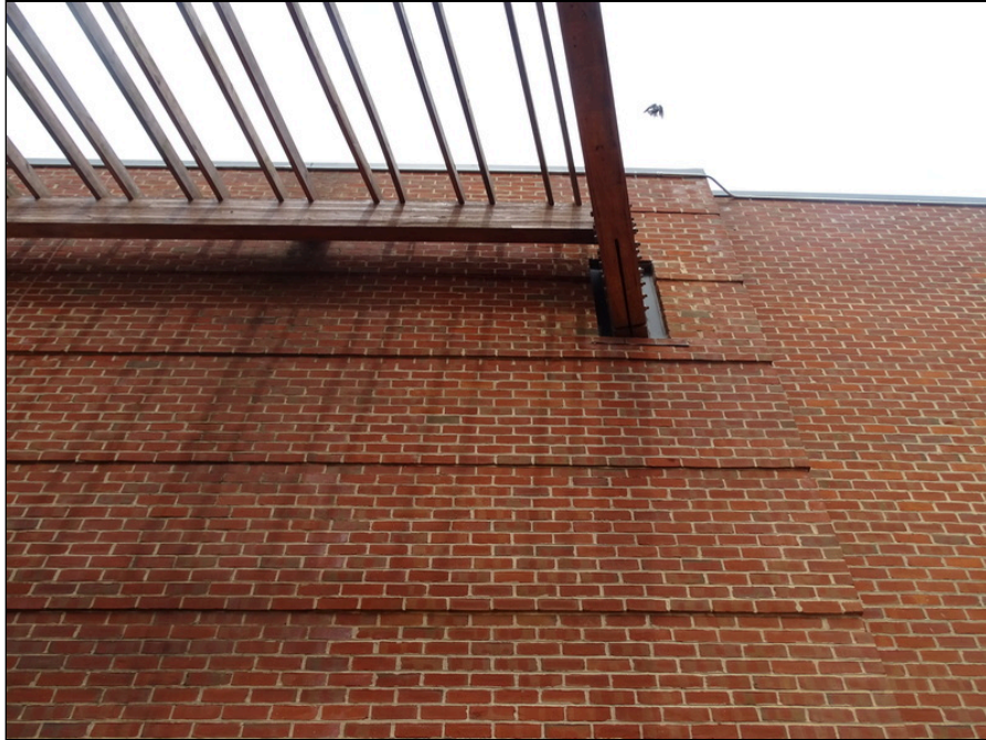
13 - Wood accent on the east side of the building - note cracking
