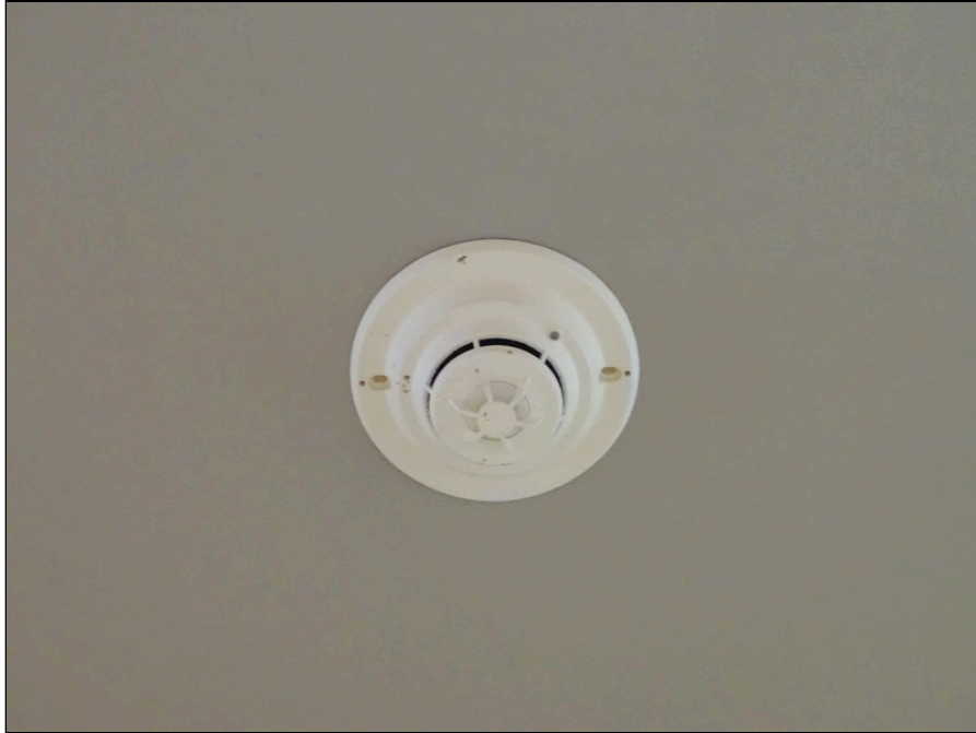
59 - Typical smoke detector
