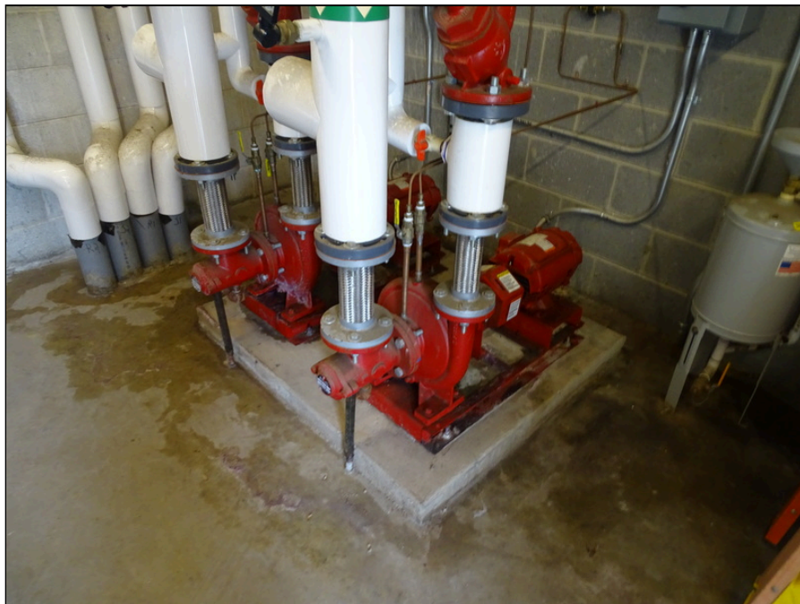
40 - Typical central plant pumps
