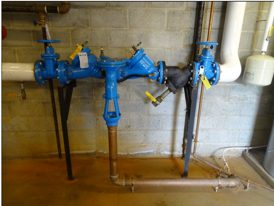
52 - Reduced Pressure Backflow Preventer
