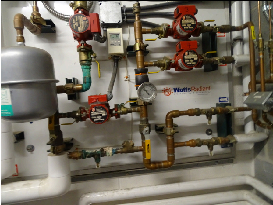
41 - Radiant floor heating system
