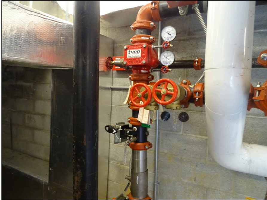
51 - Fire sprinkler system
