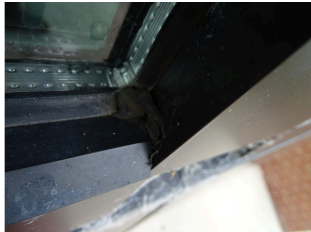
Typical exterior window - note gasket deterioration
