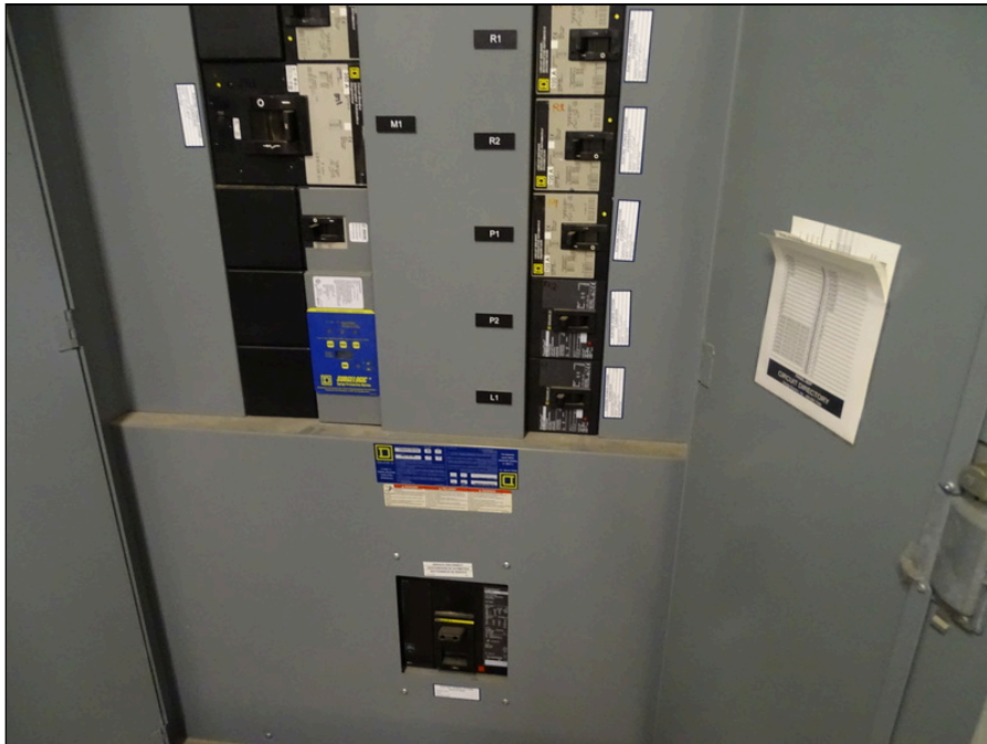
46 - Main electrical switchgear
