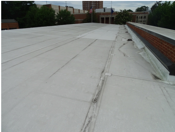
Single-ply membrane roofing system looking north
