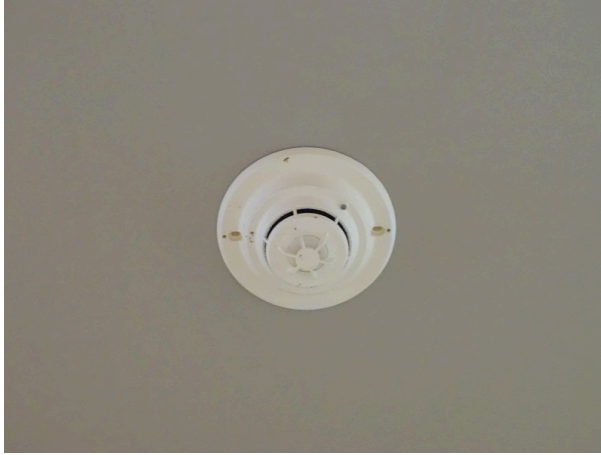
Typical smoke detector
