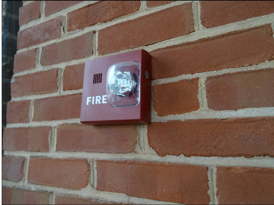
57 - Typical fire alarm bell and strobe
