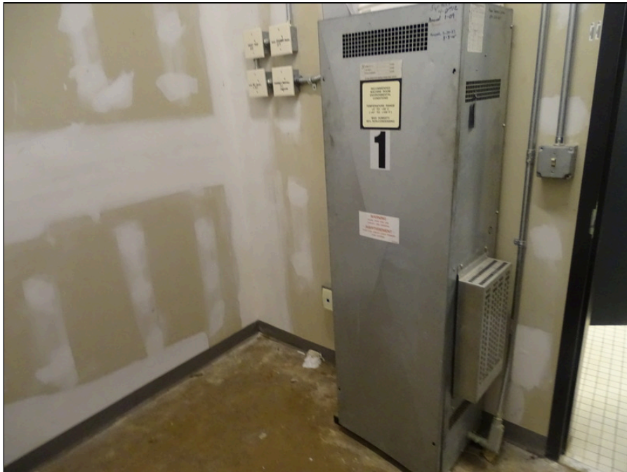
50 - Elevator machine and controls
