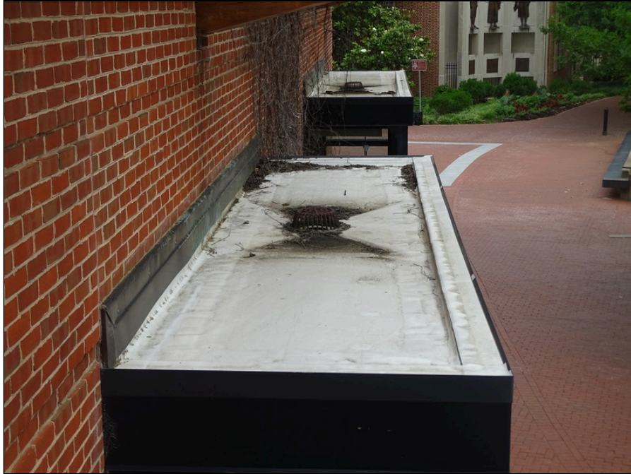
35 - Single-ply membrane roofing system
