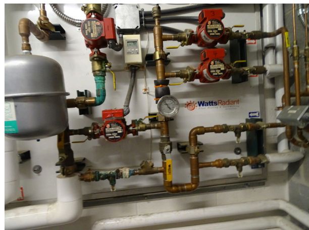
Radiant floor heating system
