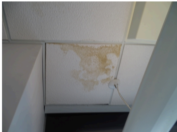
Area of reported leakage of roofing system
