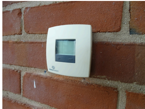
Typical thermostat control
