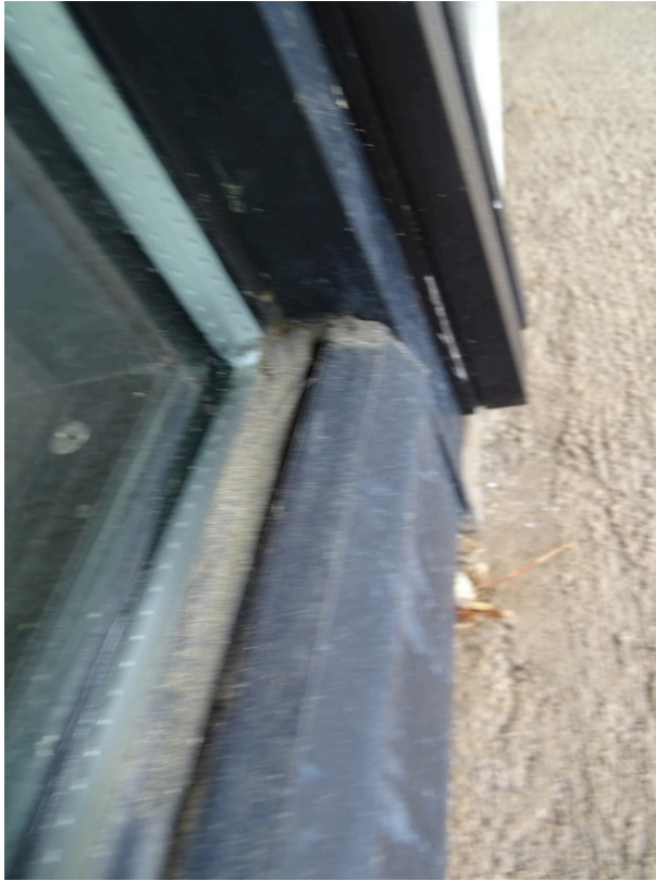
Typical exterior window - note gasket deterioration
