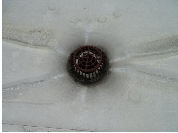
Typical internal drain
