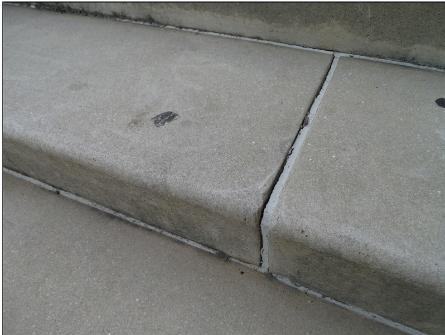
4 - Concrete steps at the west side of the building - note sealant deterioration
