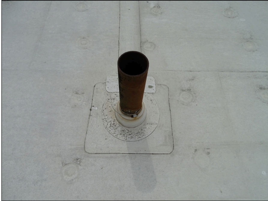
33 - Typical plumbing penetration
