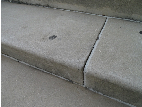
Concrete steps at the west side of the building - note sealant deterioration
