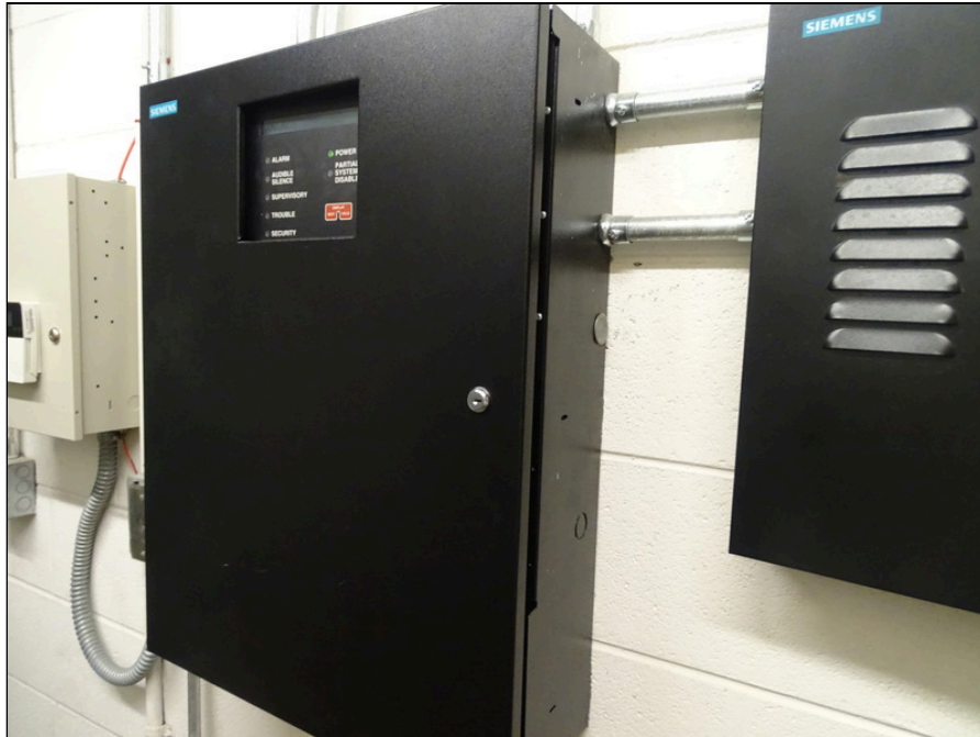
55 - Fire Alarm control panel
