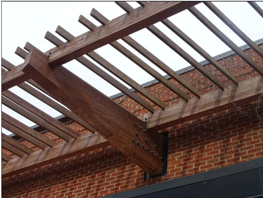
12 - Wood accent on the east side of the building - note cracking
