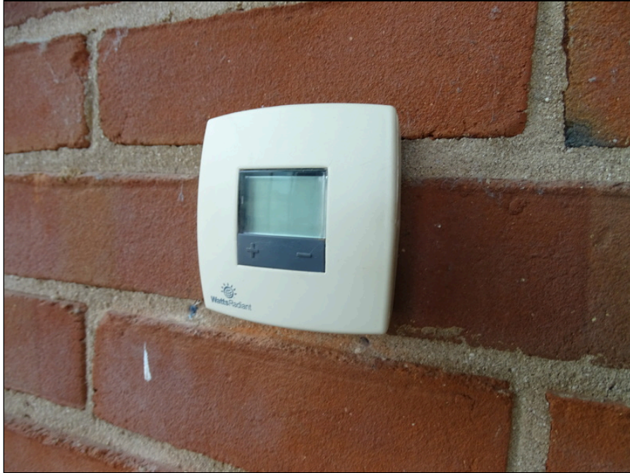
45 - Typical thermostat control
