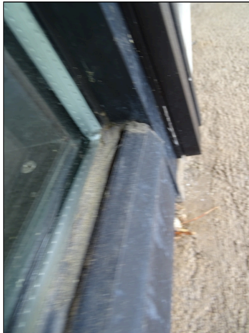
26 - Typical exterior window - note gasket deterioration
