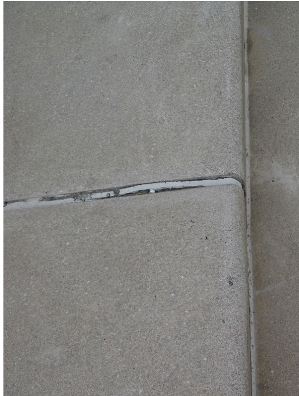
Concrete steps at the west side of the building - note sealant deterioration
