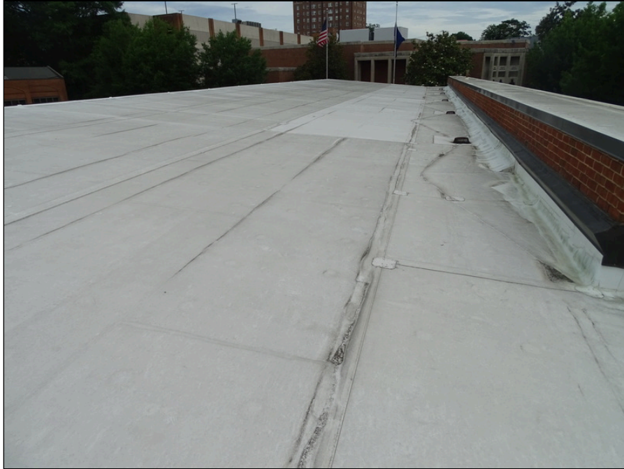
27 - Single-ply membrane roofing system looking north
