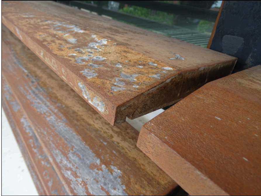
15 - Wood shade screen on west side of the building - note deterioration
