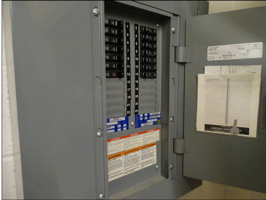
47 - Typical electrical circuit breaker panel
