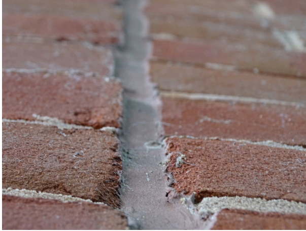
Exterior wall - note sealant deterioration
