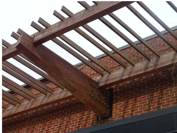
Wood accent on the east side of the building - note cracking
