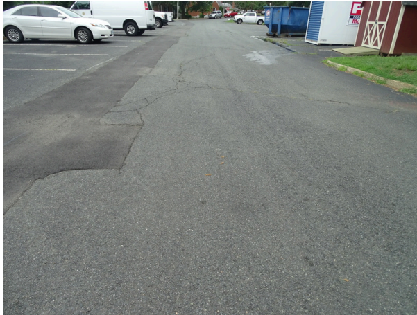
Asphalt parking area at the center of the site - note cracking and previous repair
