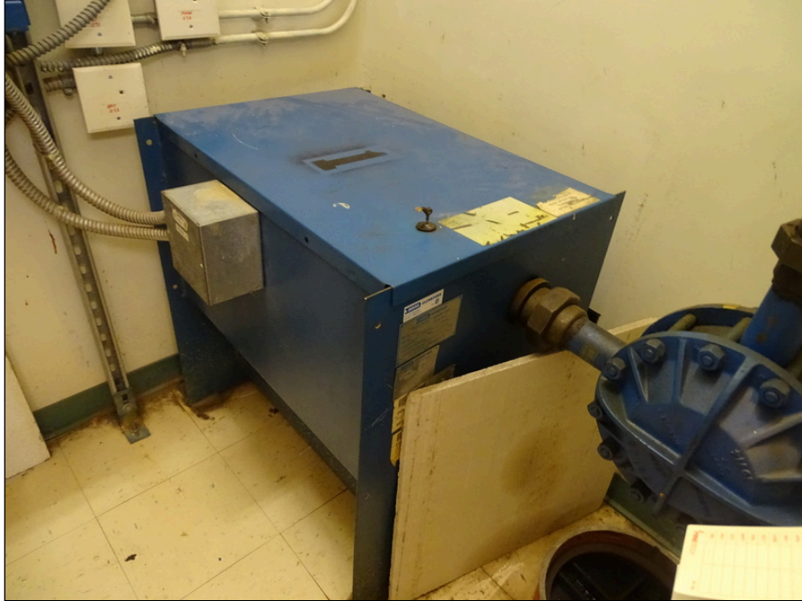
73 - Typical elevator machine and controls
