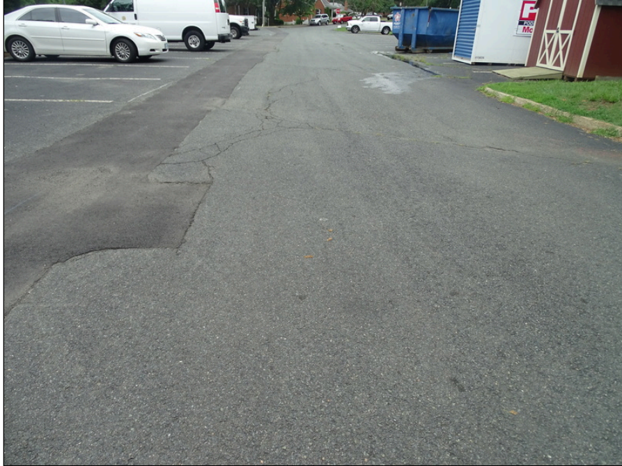
3 - Asphalt parking area at the center of the site - note cracking and previous repair
