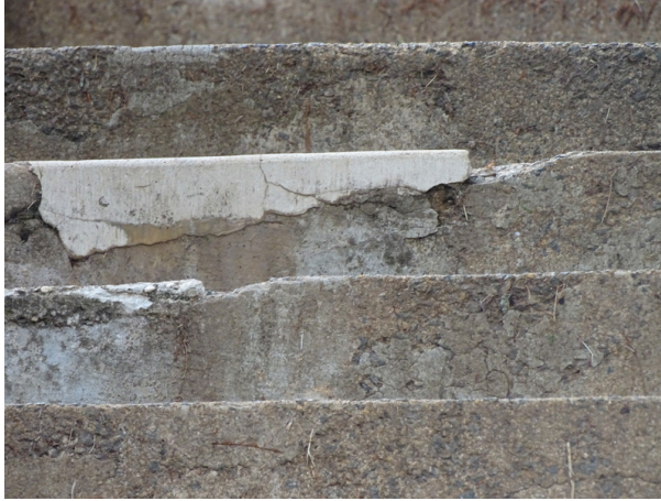
Typical exterior concrete steps - note deterioration
