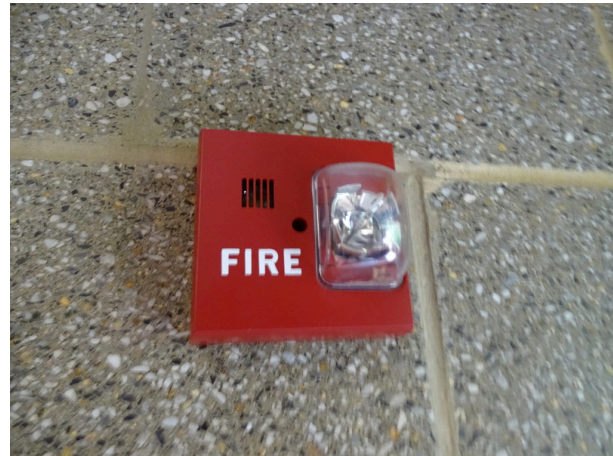
Fire alarm strobe and bell
