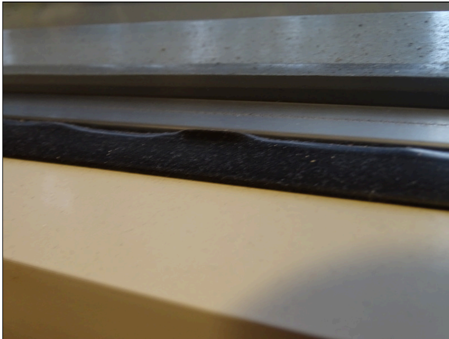
40 - Exterior window - note gasket needing replacement
