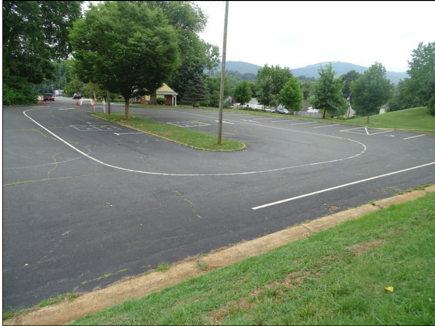
5 - Asphalt parking and drive lanes lower level north end of the site - note cracking
