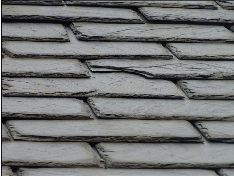
51 - Slate shingle roofing system - note repair needed
