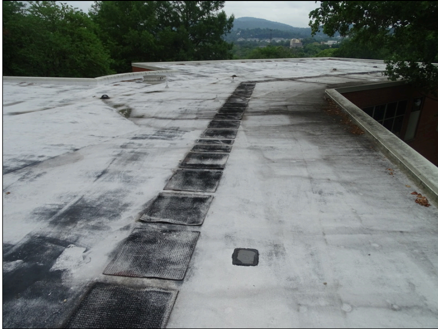
41 - Single-ply membrane roofing system east side of the building
