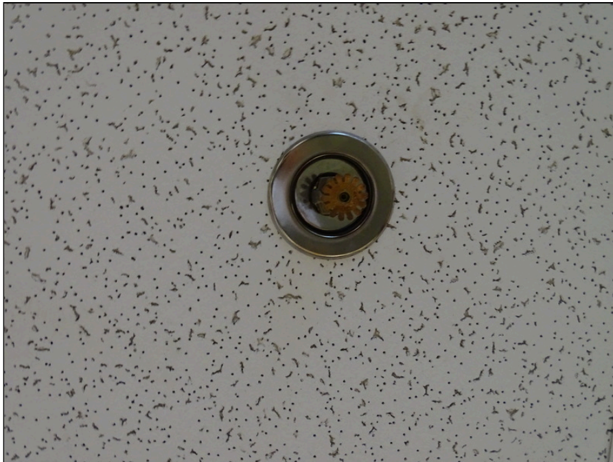
76 - Typical fire sprinkler head
