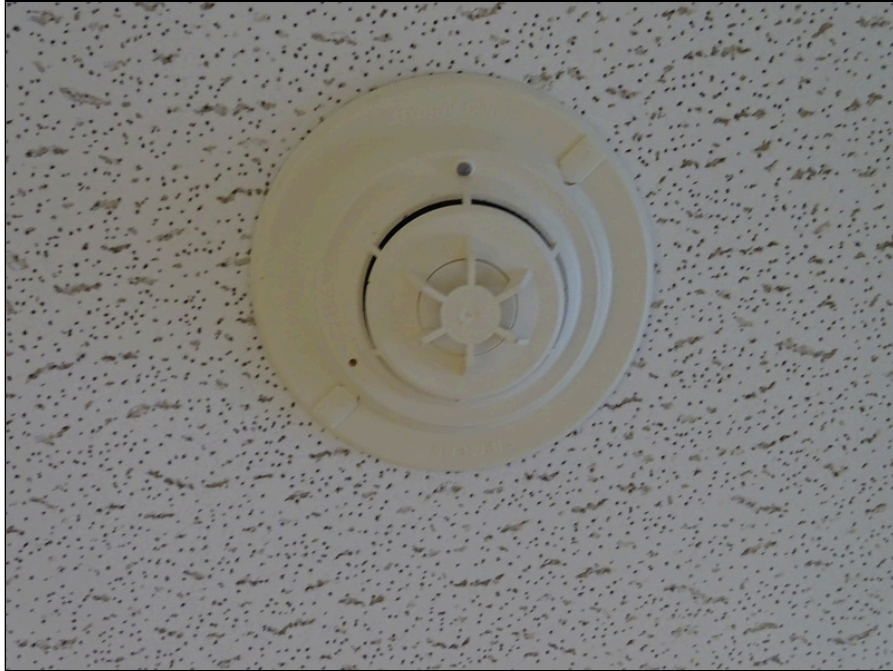
77 - Typical smoke detector
