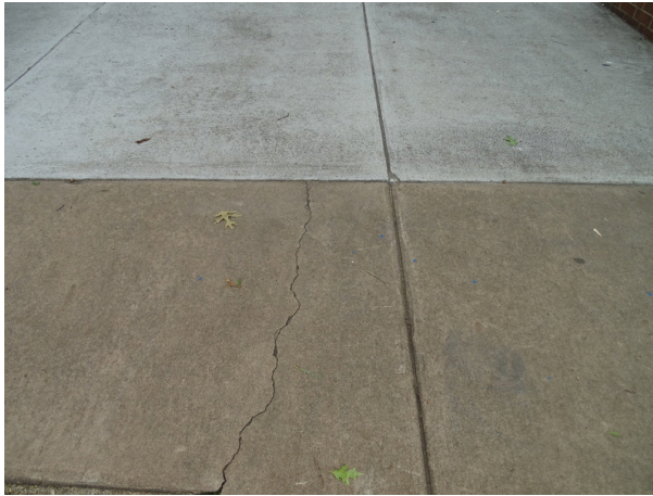
Concrete sidewalk - note cracking
