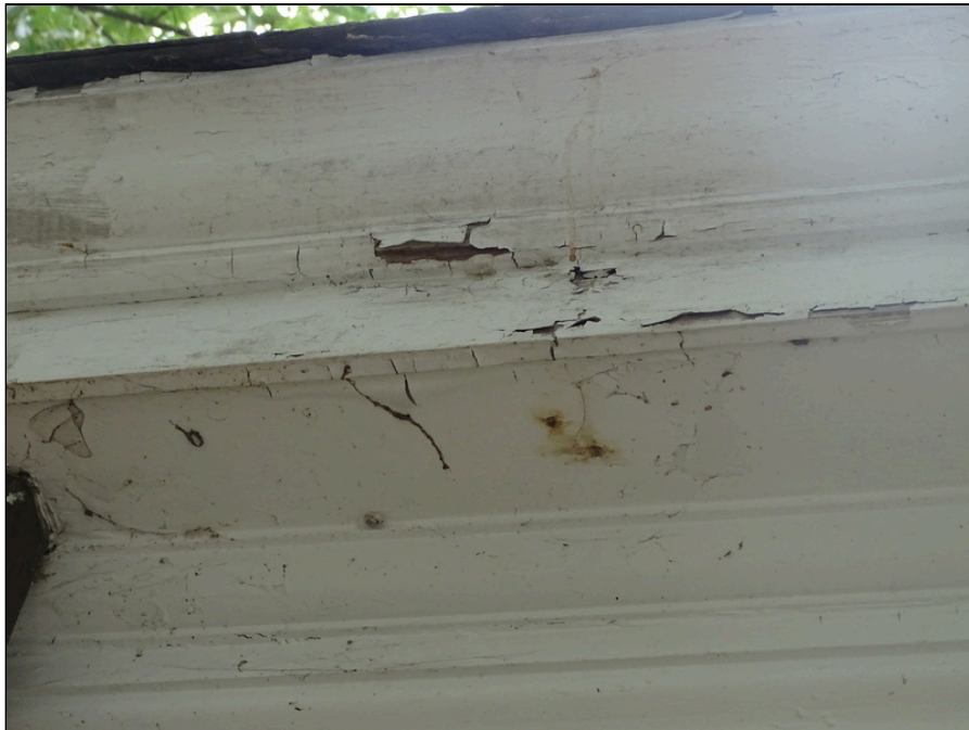
52 - Building exteriors - note deterioration of wood cornice
