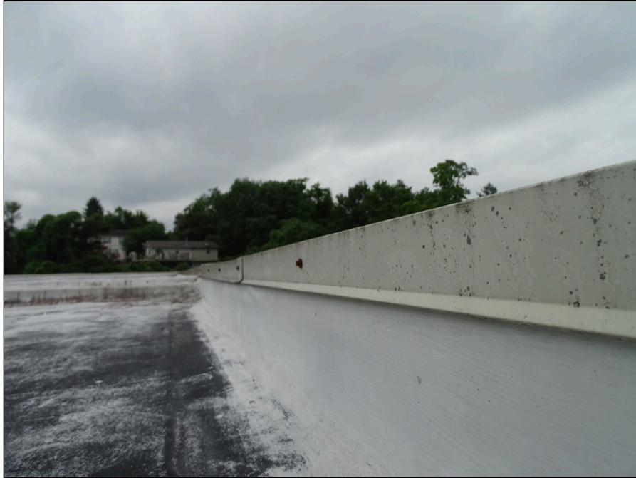
49 - Typical metal coping and parapet wall - note deterioration
