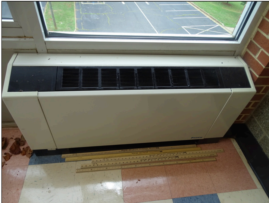
62 - Typical Water Source Heat Pump
