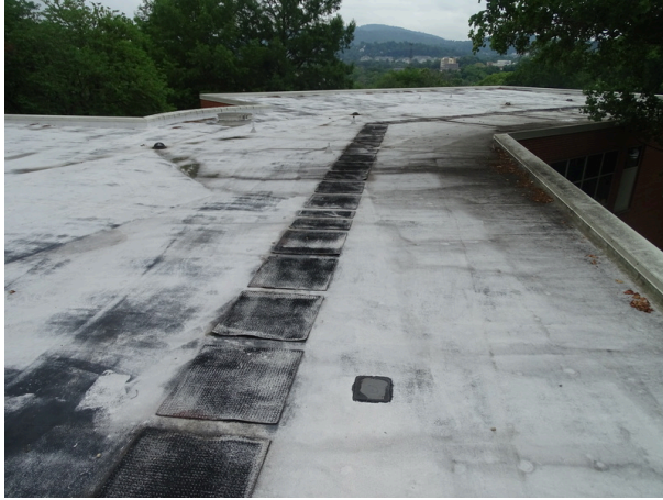
Single-ply membrane roofing system east side of the building
