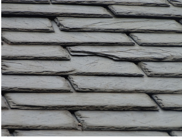
Slate shingle roofing system - note repair needed
