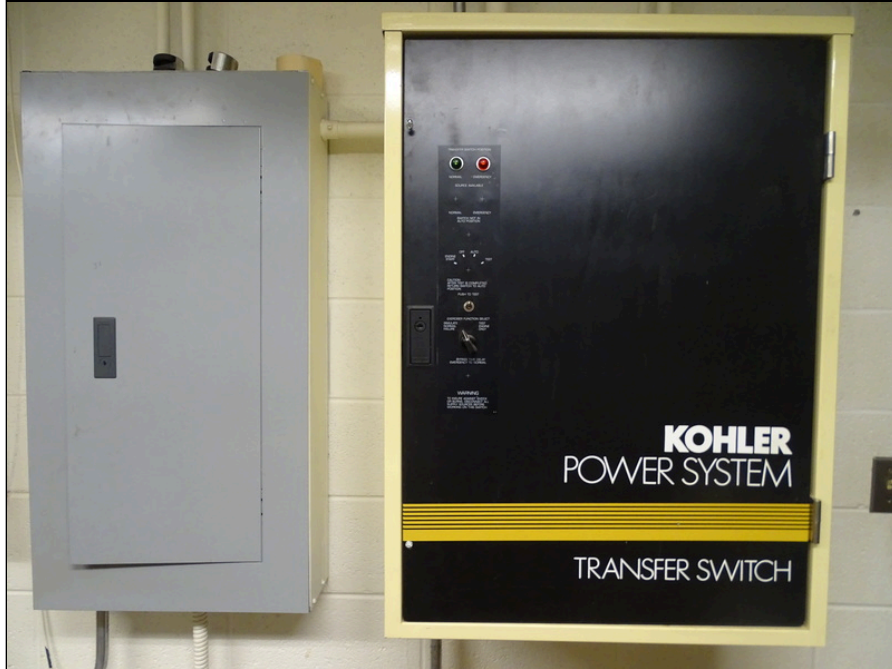
71 - Emergency power transfer switch
