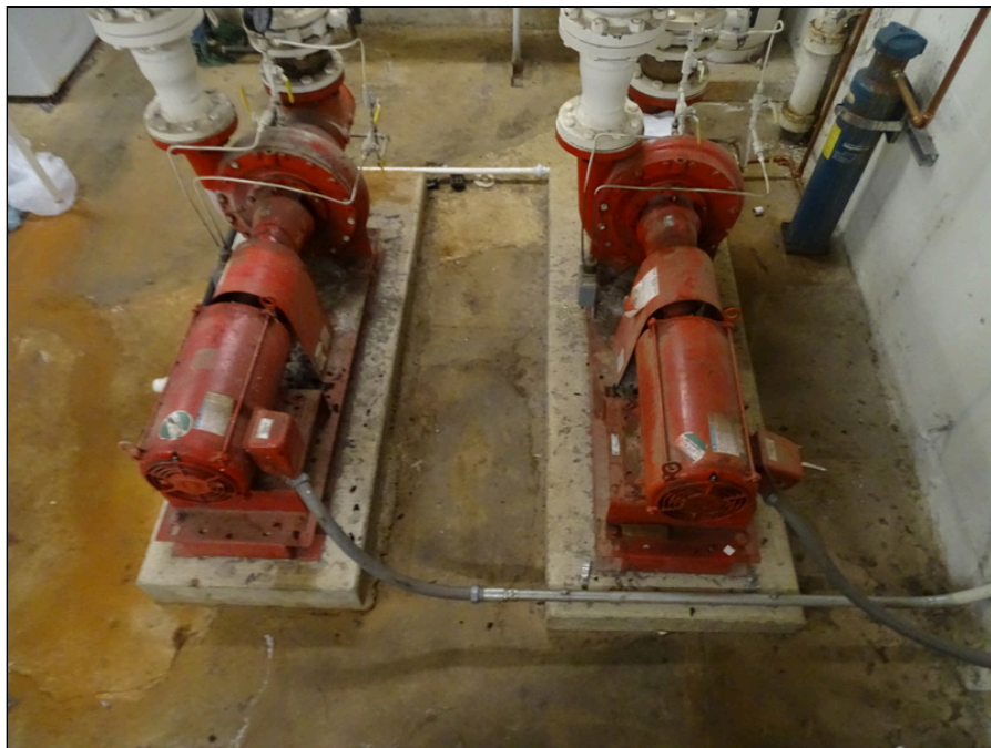
58 - Central plant pumps located in mechanical room
