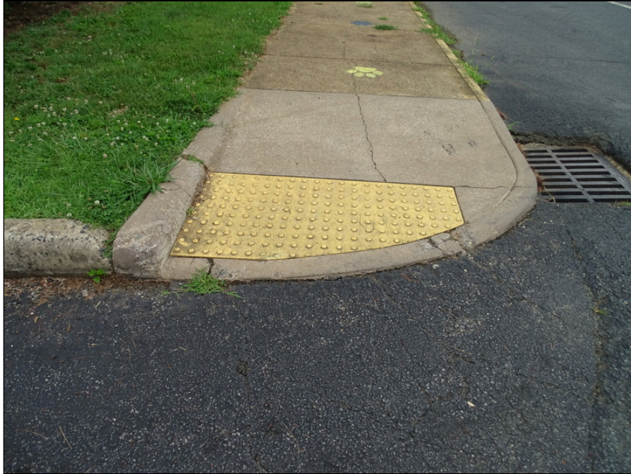
103 - Concrete curb cut ramp with truncated domes
