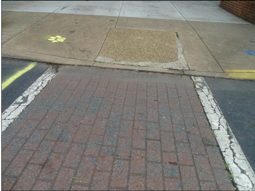
13 - Concrete ramp- note need to install truncated domes
