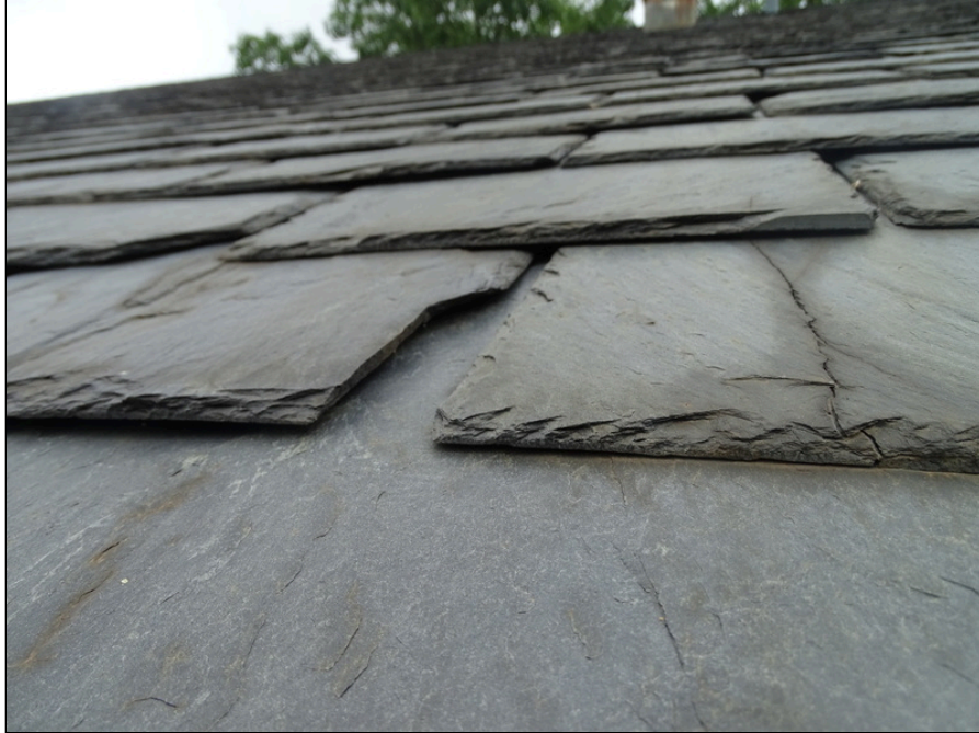
45 - Slate shingle roofing system
