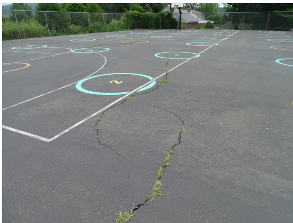
Basketball court surface - note cracking and deterioration
