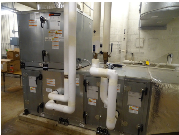
Air Handler Unit in mechanical room
