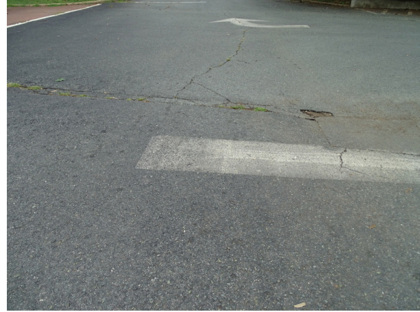
Asphalt parking area at the center of the site - note cracking
