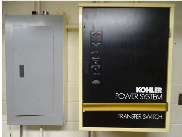
Emergency power transfer switch
