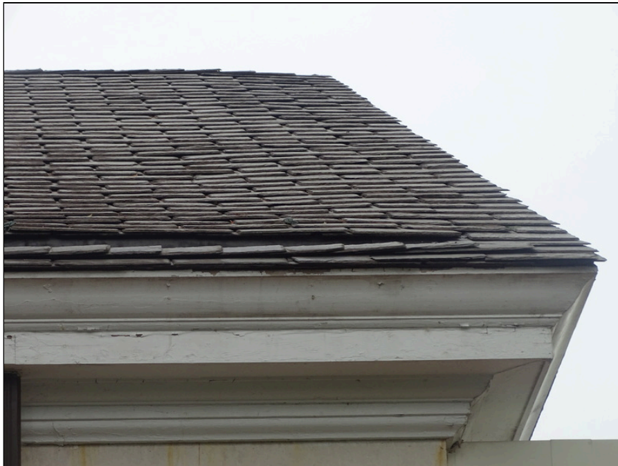
50 - Slate shingle roofing system
