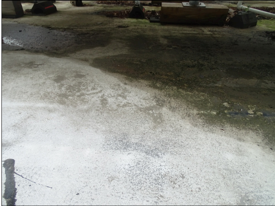
43 - Single-ply membrane roofing system - note ponding
