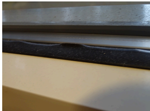
Exterior window - note gasket needing replacement
