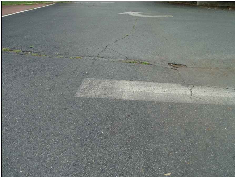
8 - Asphalt parking area at the center of the site - note cracking
