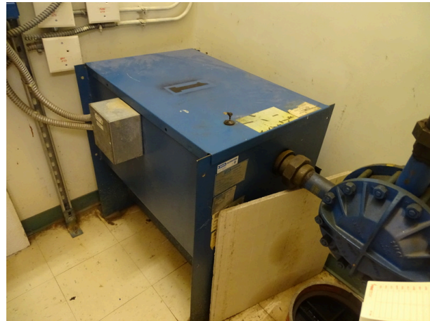
Typical elevator machine and controls
