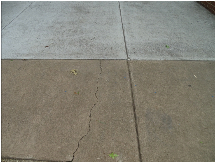
12 - Concrete sidewalk - note cracking
