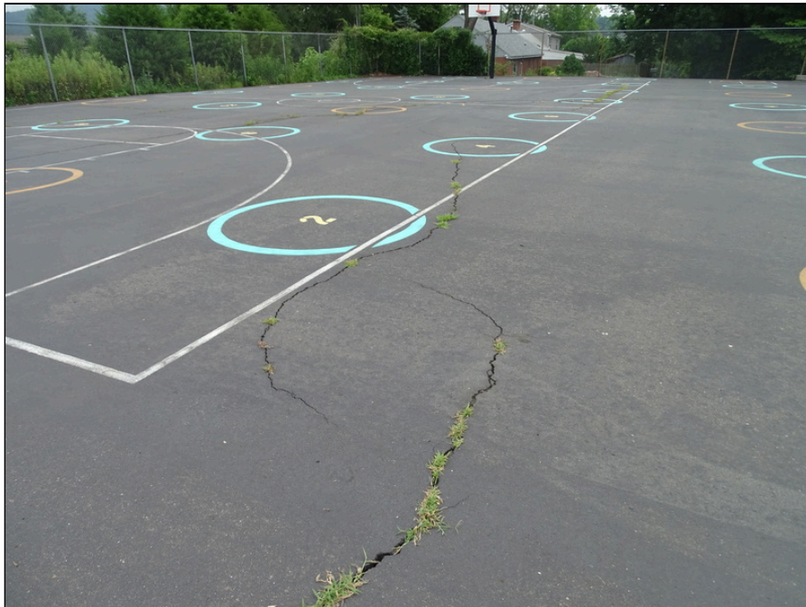
26 - Basketball court surface - note cracking and deterioration
