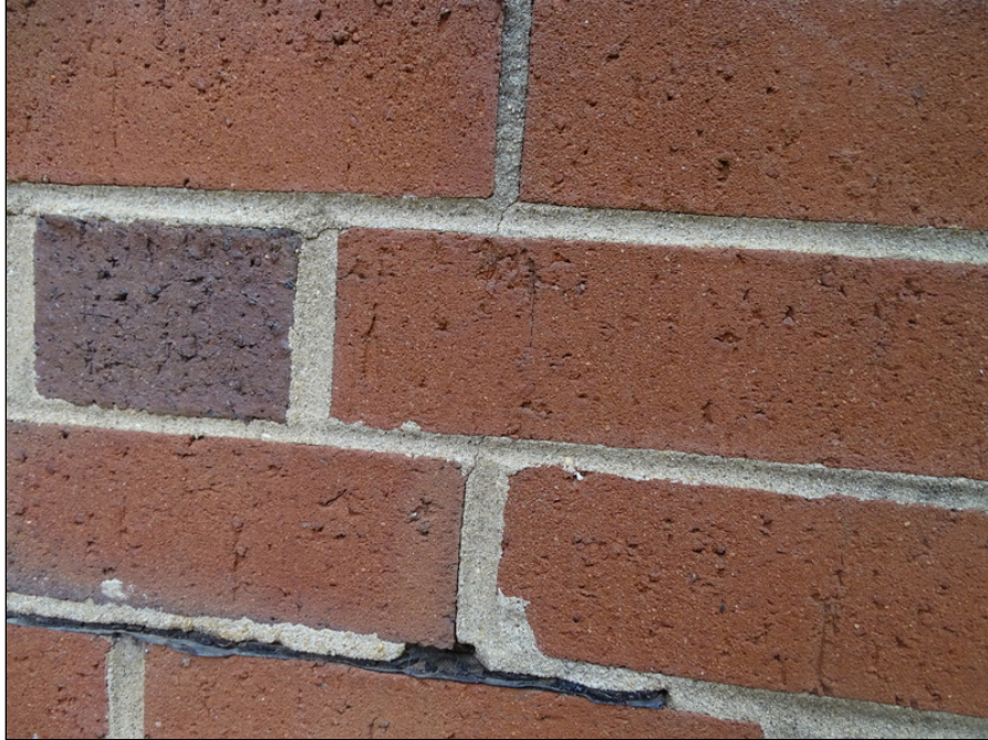
33 - Building exterior finishes - note mortar joint deterioration
