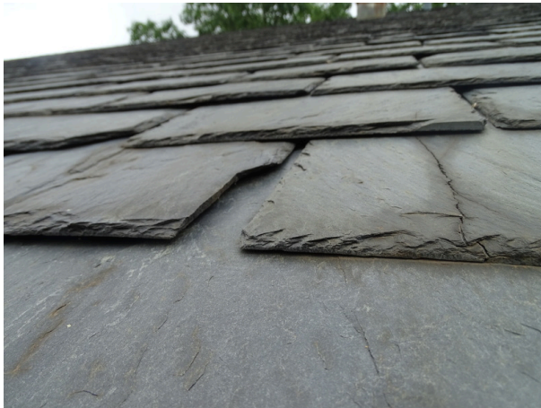
Slate shingle roofing system
