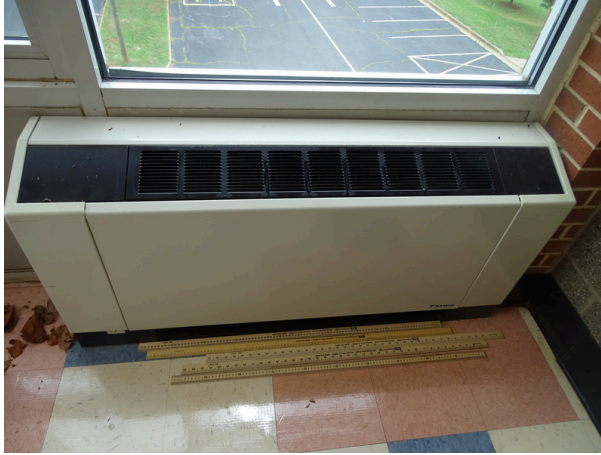
Typical Water Source Heat Pump
