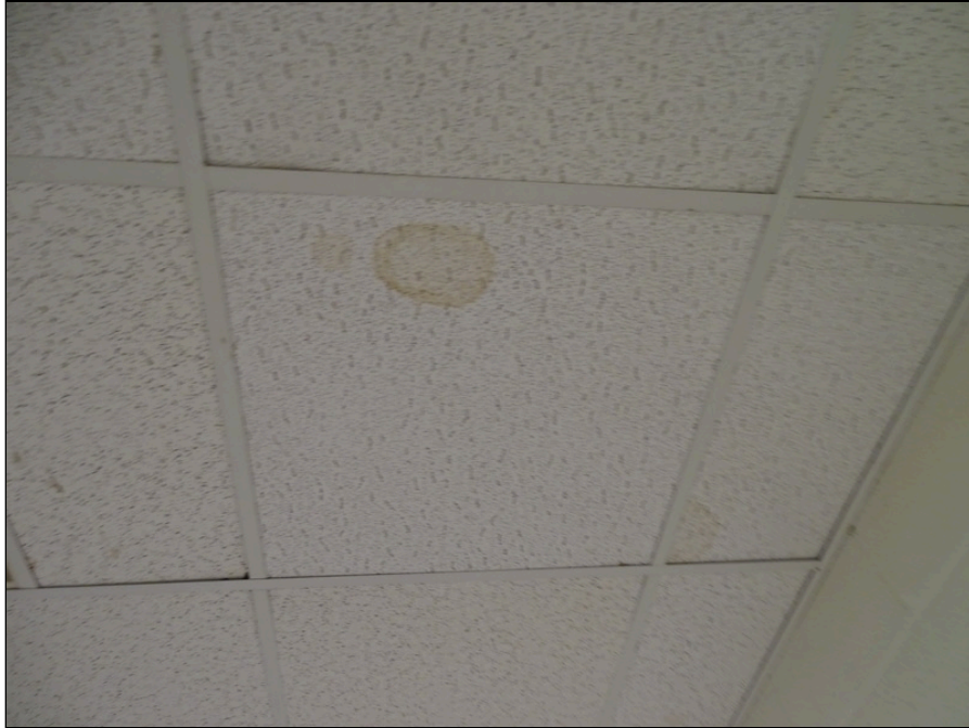
97 - Interior ceiling - note water leakage
