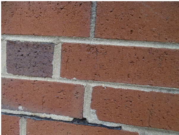
Building exterior finishes - note mortar joint deterioration
