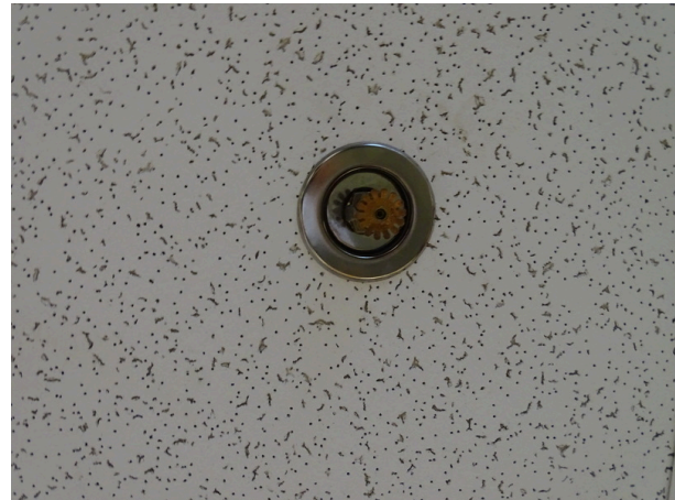
Typical fire sprinkler head
