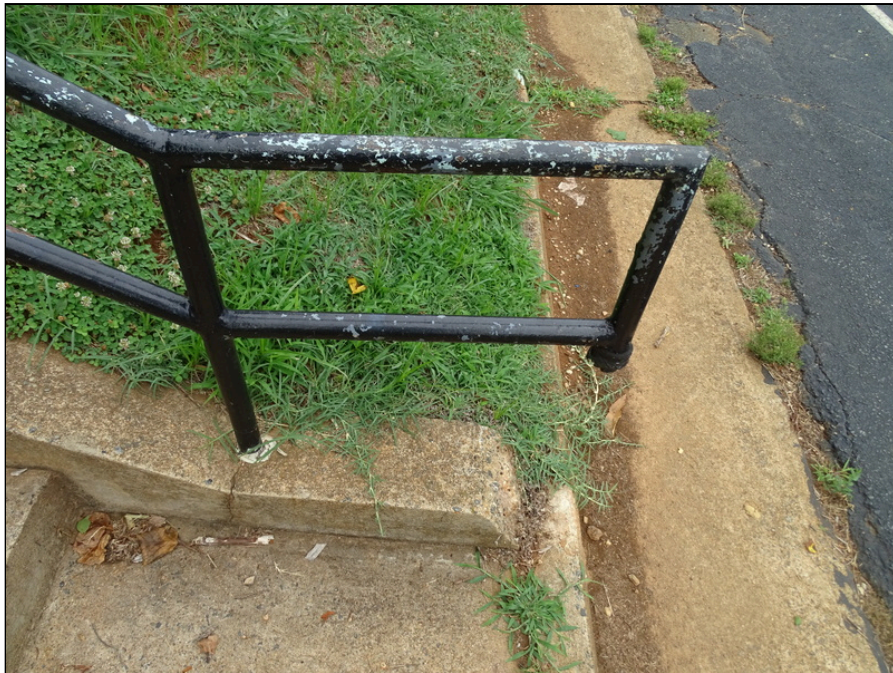
16 - Typical exterior concrete steps - note handrail peeled
