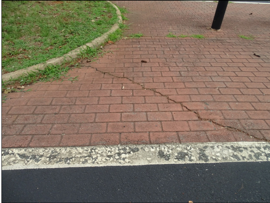
9 - Brick sidewalk - note cracking
