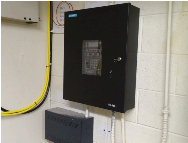
Fire alarm controls
