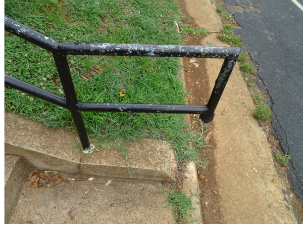
Typical exterior concrete steps - note handrail peeled
