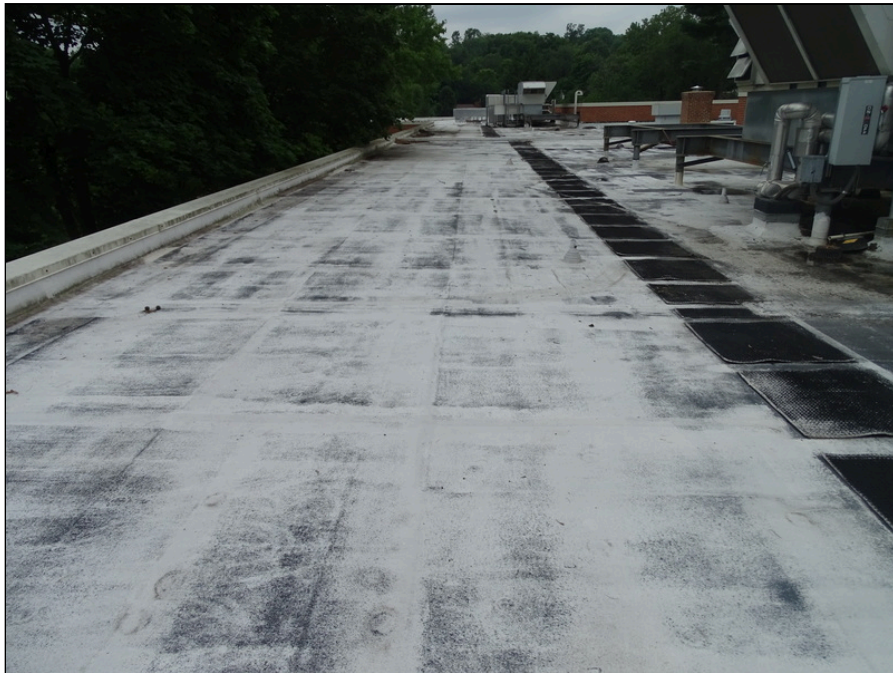
42 - Single-ply membrane roofing system
