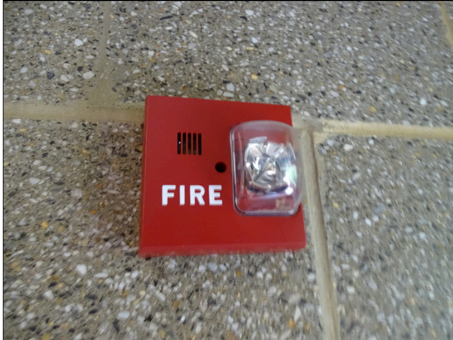
79 - Fire alarm strobe and bell
