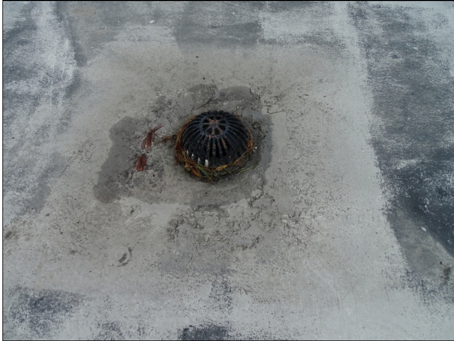
47 - Internal roof drain - note debris needing routine maintenance
