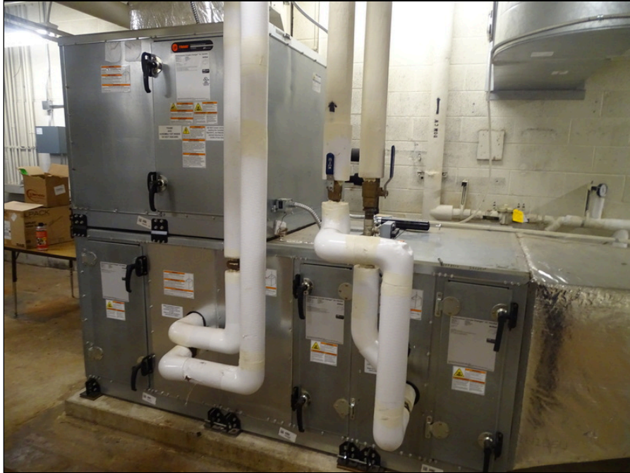
59 - Air Handler Unit in mechanical room
