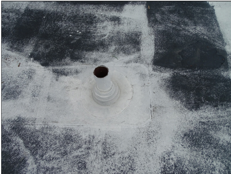
48 - Typical plumbing penetration
