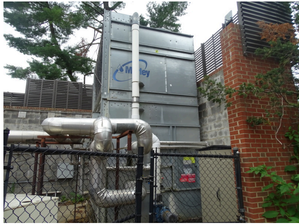
Cooling Tower at north side of the building
