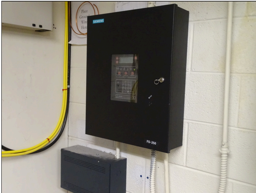
78 - Fire alarm controls
