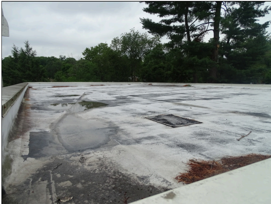
44 - Single-ply membrane roofing system - note ponding
