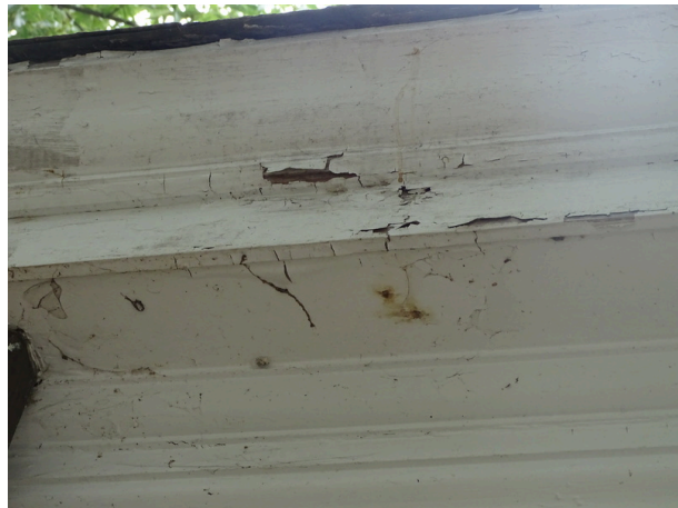
Building exteriors - note deterioration of wood cornice
