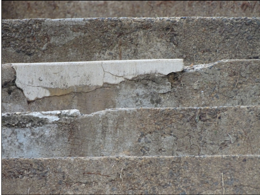
15 - Typical exterior concrete steps - note deterioration
