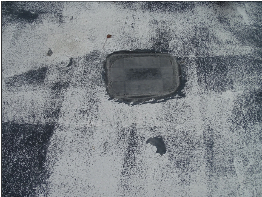
46 - Typical roof patch
