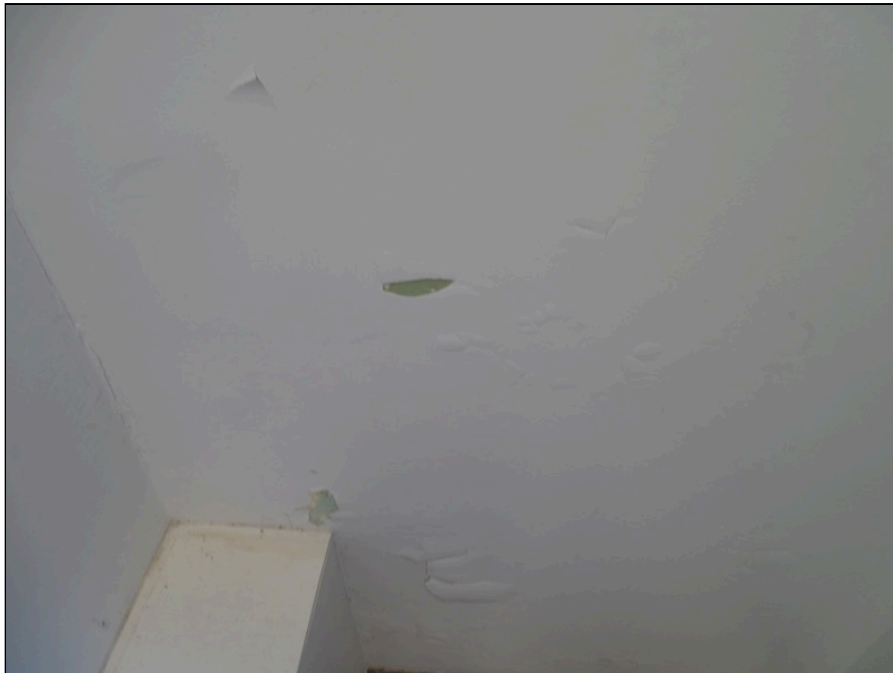
92 - Interior ceiling - note peeled paint
