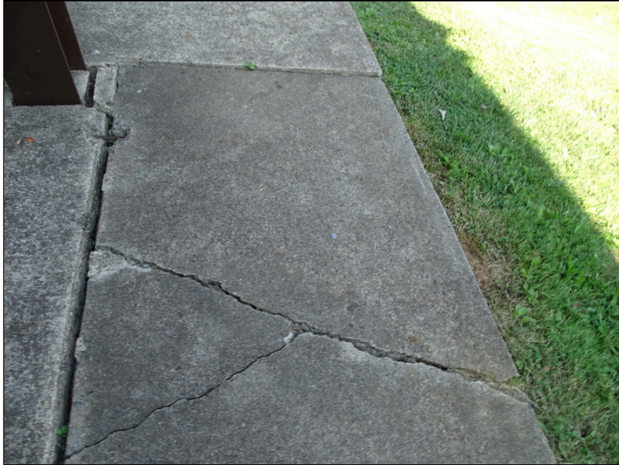
11 - Typical concrete sidewalk - note cracking
