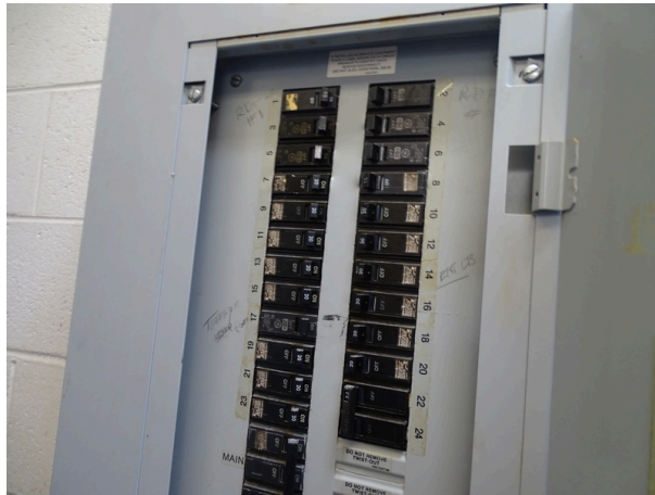
Typical newer electrical circuit breaker panel
