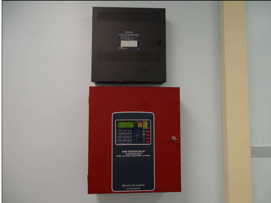
65 - Fire alarm control panel
