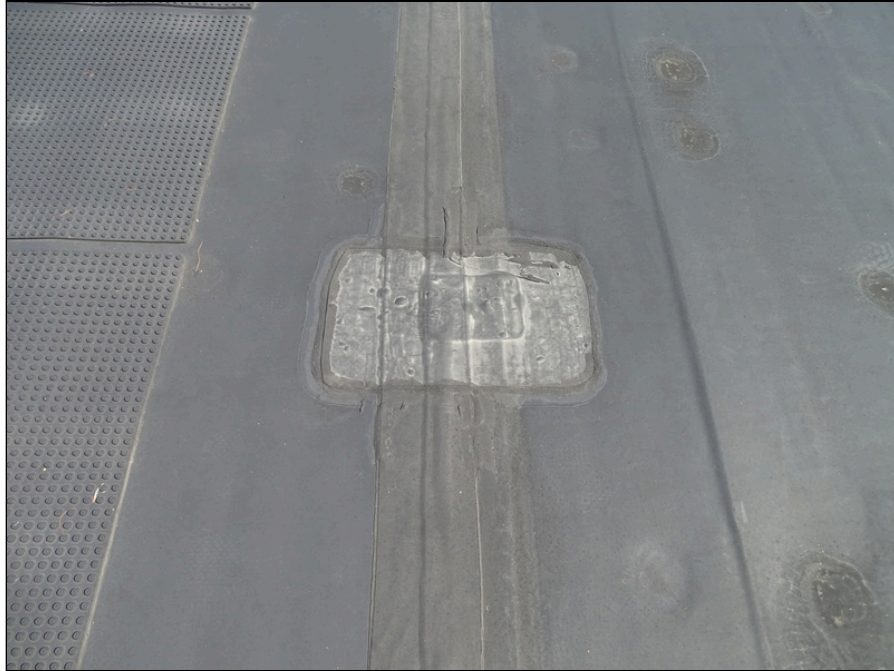
31 - Single-ply roofing system - note patching
