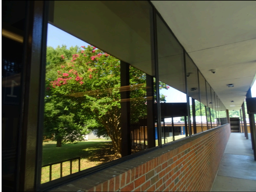
25 - Older exterior windows - note reportedly wide temperature fluctuation in offices
