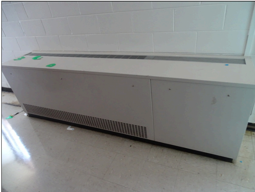
46 - Typical Water Source Heat Pump
