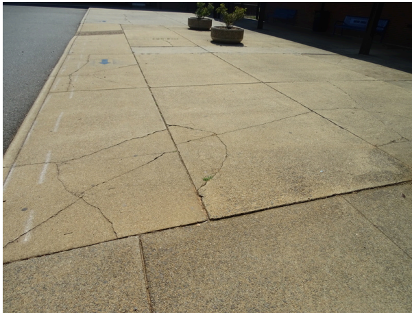
Concrete sidewalk west side of Building B - note cracking
