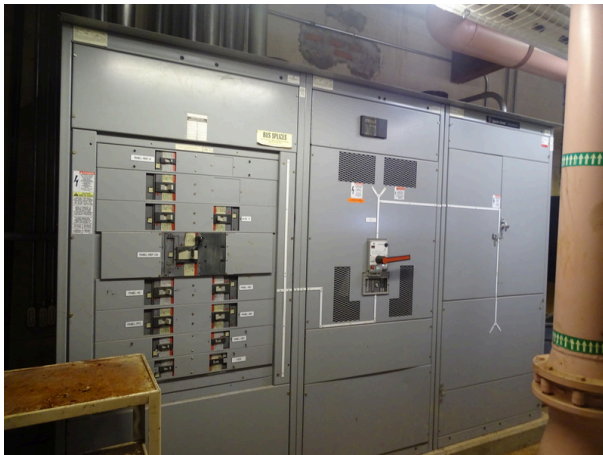
Main electrical switchgear
