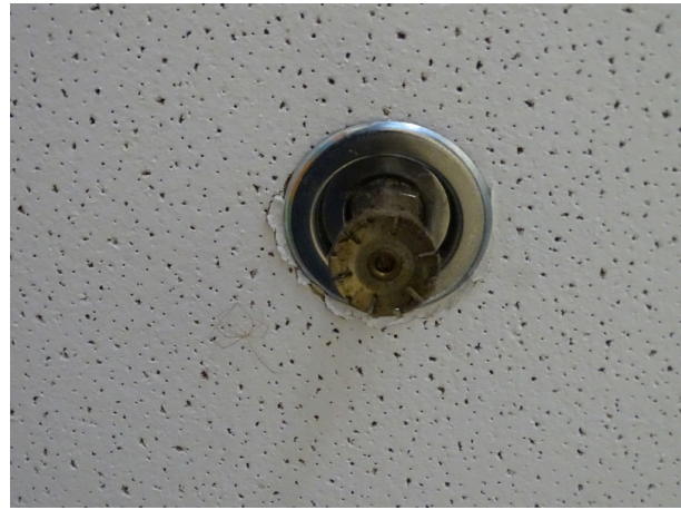
Typical fire sprinkler head
