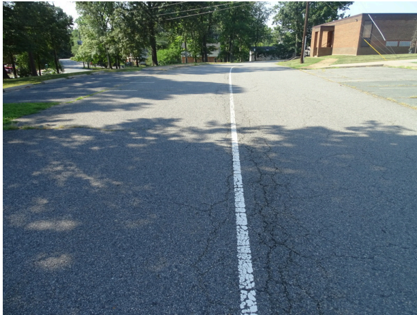
Asphalt pavements east side of the site drive lane - note cracking
