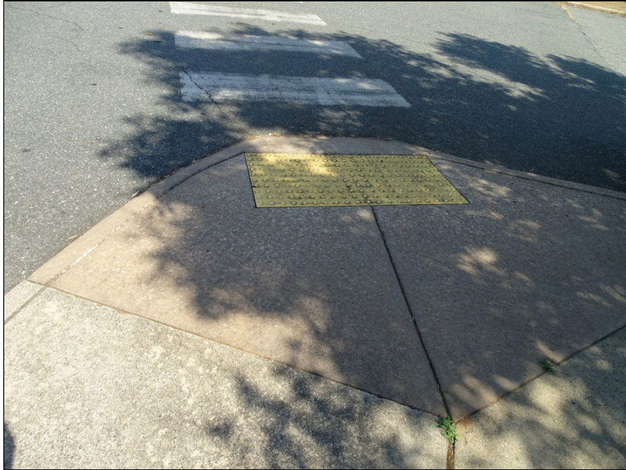
87 - Accessible curb cut ramp with truncated domes
