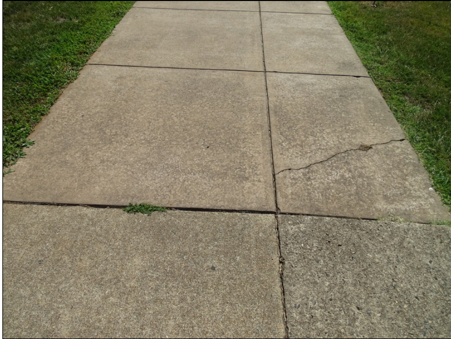
9 - Typical concrete sidewalk - note cracking
