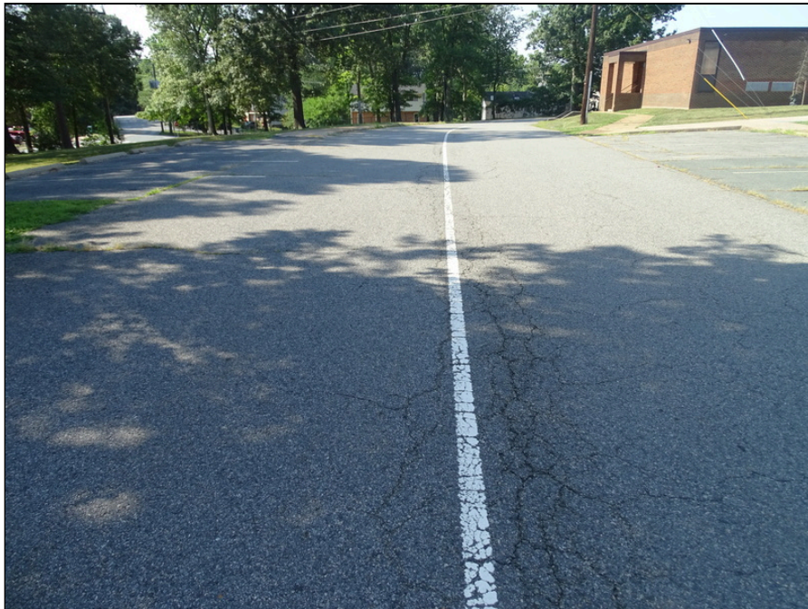
4 - Asphalt pavements east side of the site drive lane - note cracking
