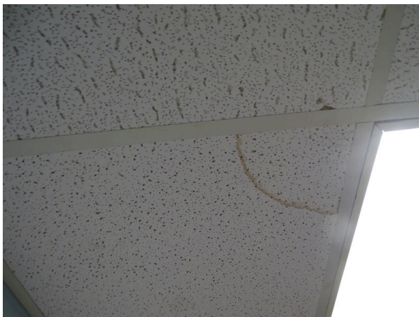
Typical interior ceiling - note water leakage
