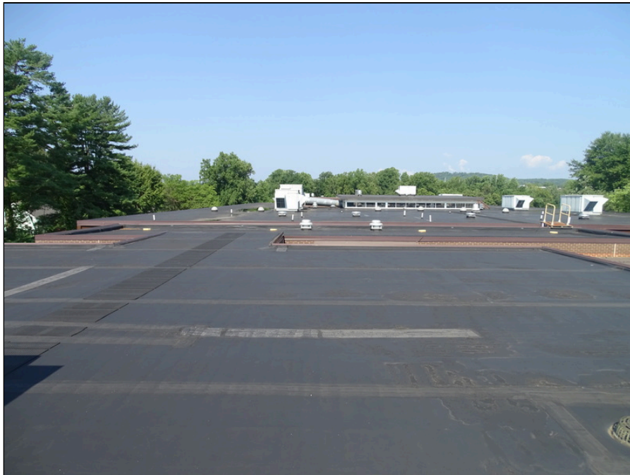
30 - Single-ply roofing system looking west
