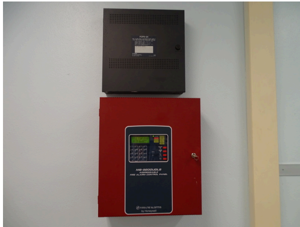
Fire alarm control panel
