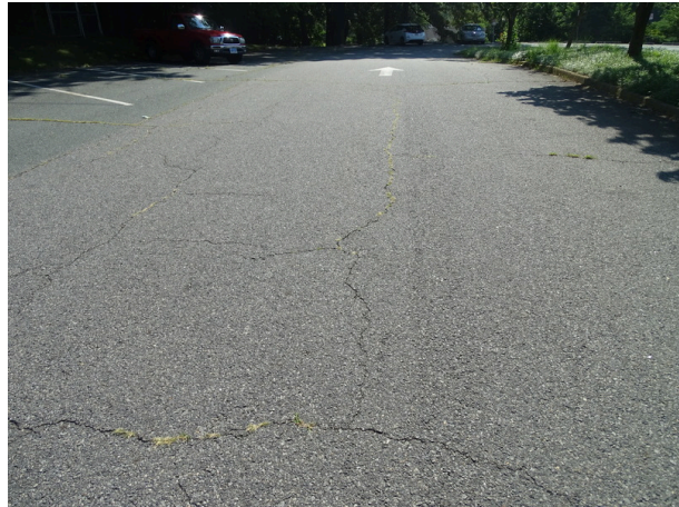
Asphalt pavements - note alligator cracks
