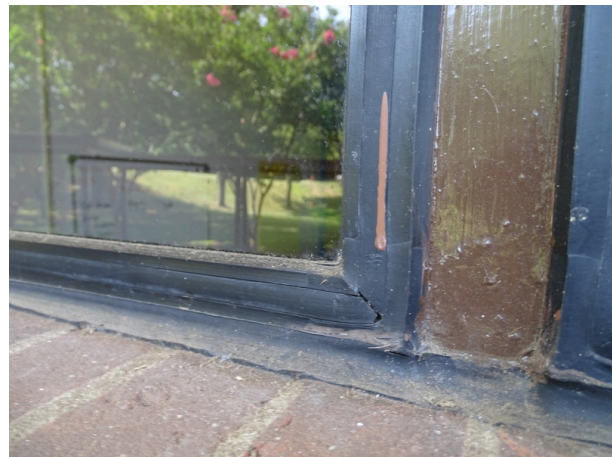
Typical exterior window - note gasket deterioration
