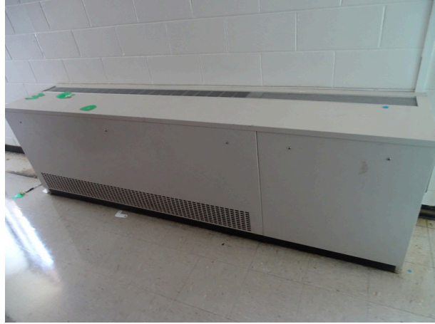
Typical Water Source Heat Pump
