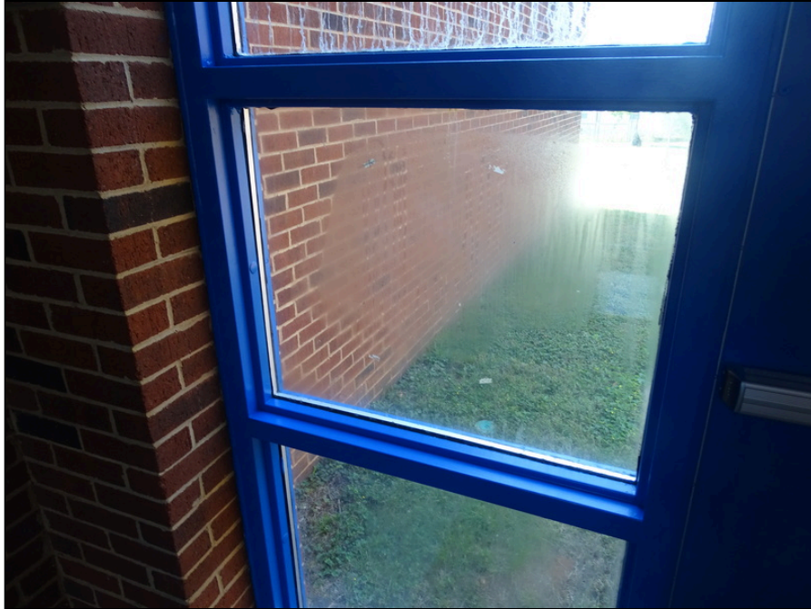
27 - Typical exterior window - note fog inside the glass
