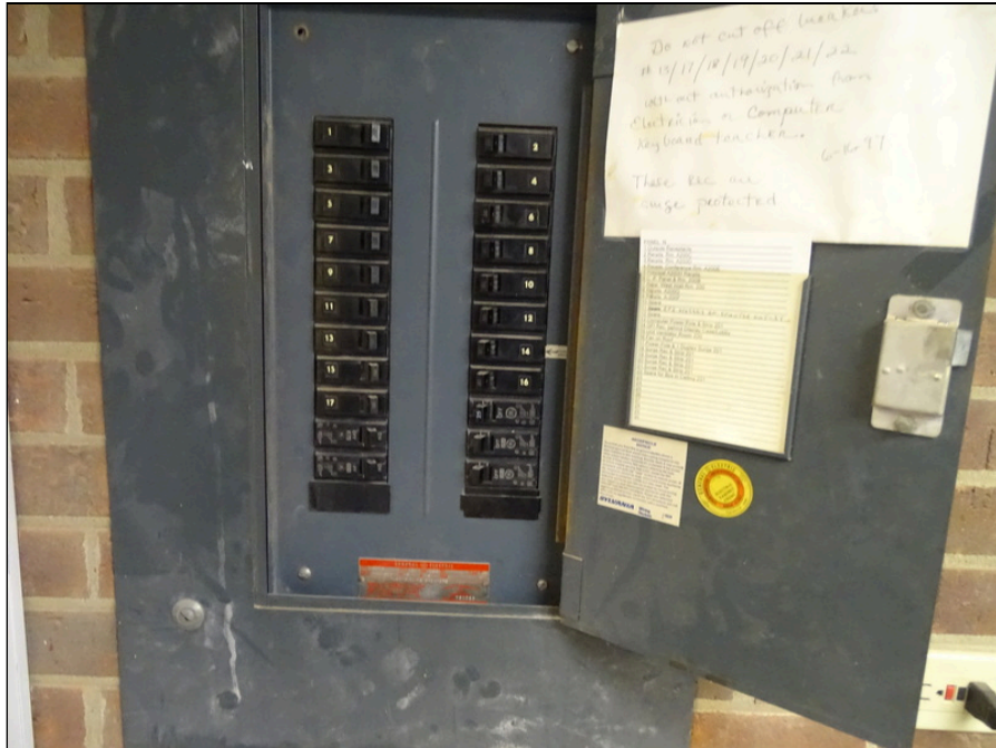
57 - Typical older electrical circuit breaker panel
