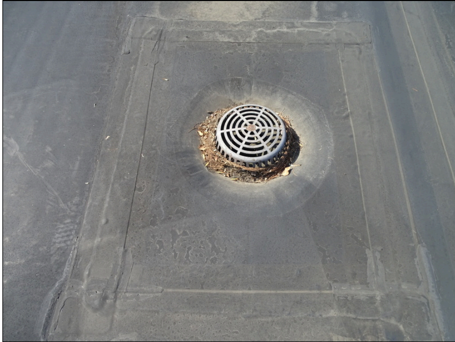
35 - Typical internal drain
