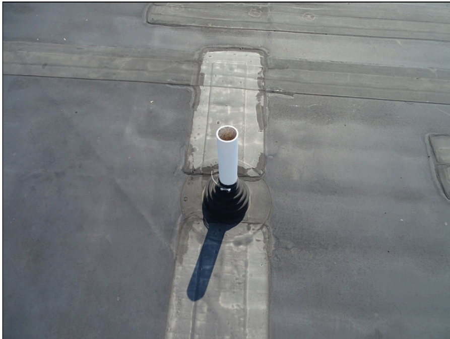
36 - Typical plumbing penetration
