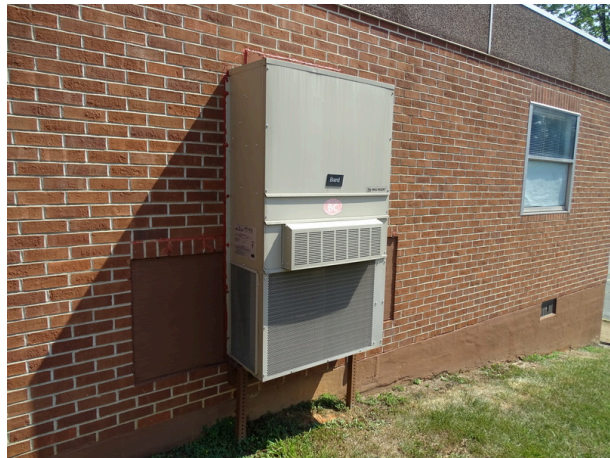
Wall mounted air conditioner unit
