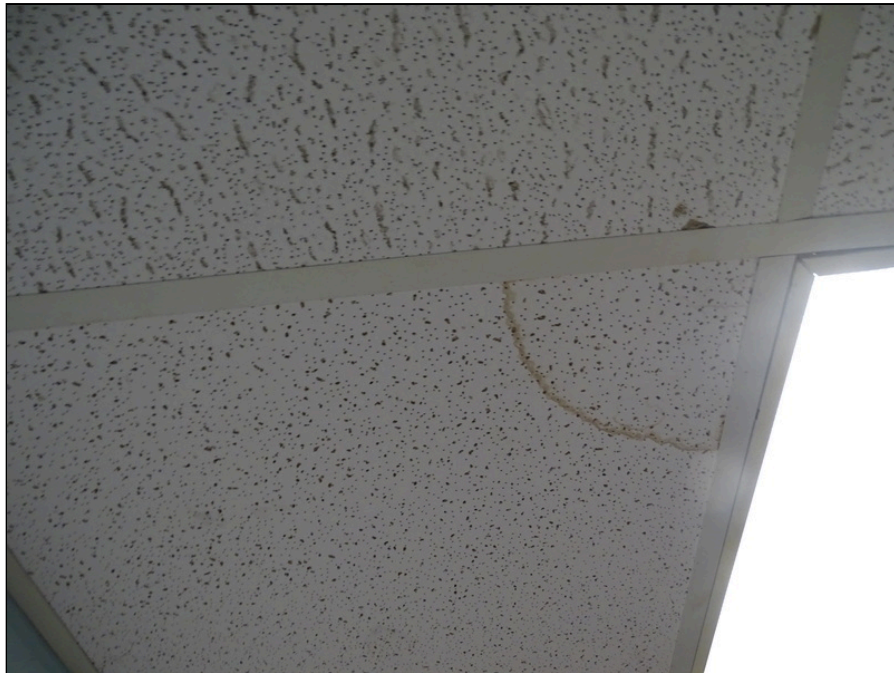
32 - Typical interior ceiling - note water leakage
