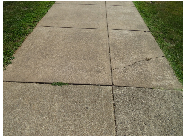
Typical concrete sidewalk - note cracking
