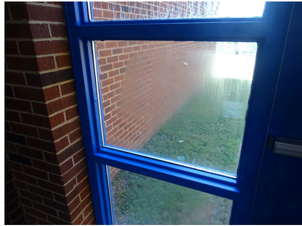
Typical exterior window - note fog inside the glass
