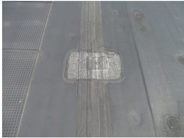
Single-ply roofing system - note patching
