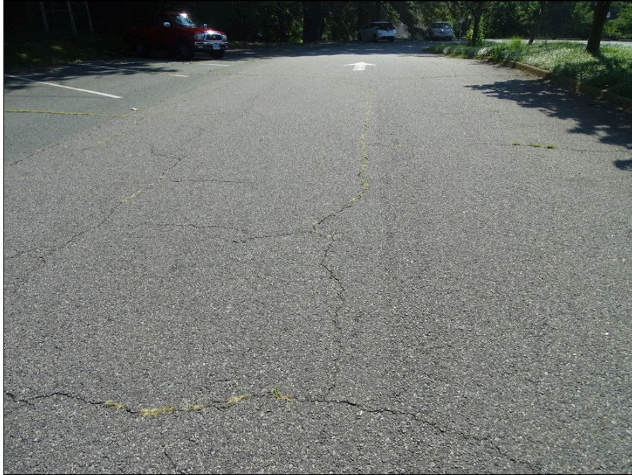
5 - Asphalt pavements - note alligator cracks
