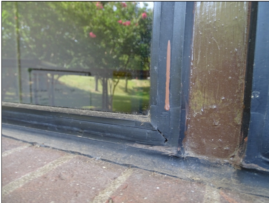
28 - Typical exterior window - note gasket deterioration
