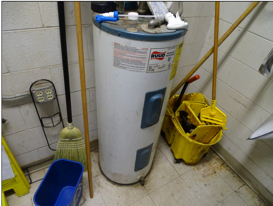
40 - Electric water heater located in janitor's closet
