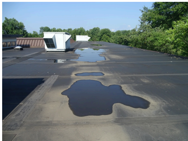
Single-ply roofing system - note ponding
