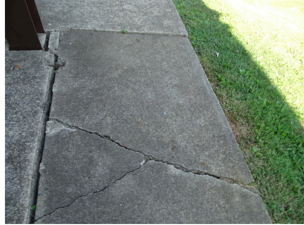
Typical concrete sidewalk - note cracking
