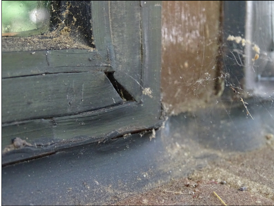
29 - Typical exterior window - note gasket deterioration
