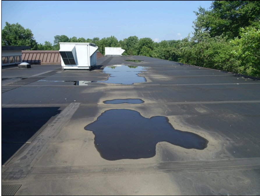
33 - Single-ply roofing system - note ponding
