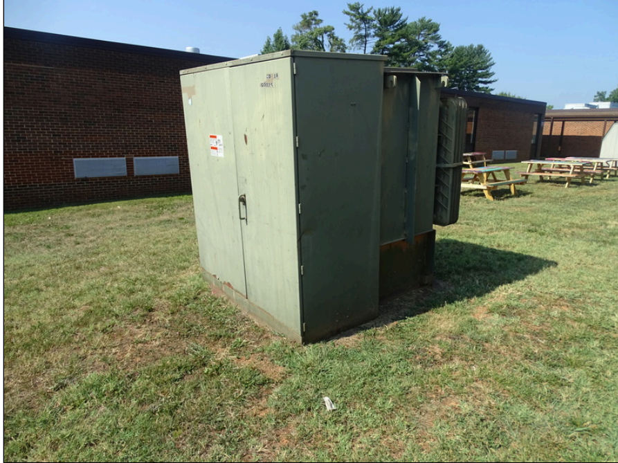
53 - Electric utility transformer
