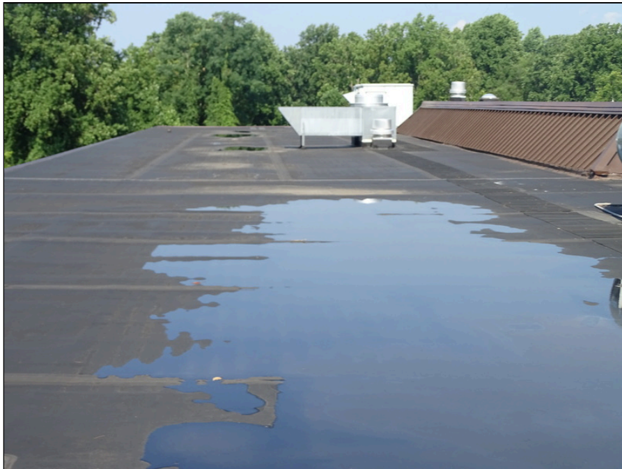
34 - Single-ply roofing system - note ponding
