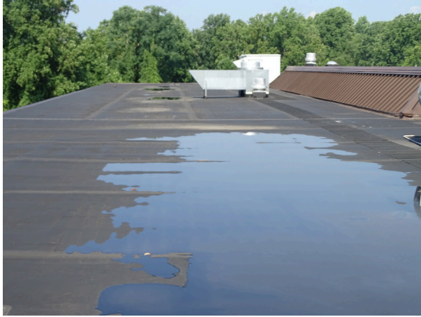
Single-ply roofing system - note ponding
