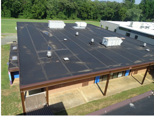
Typical Make Up Air Unit located on roof
