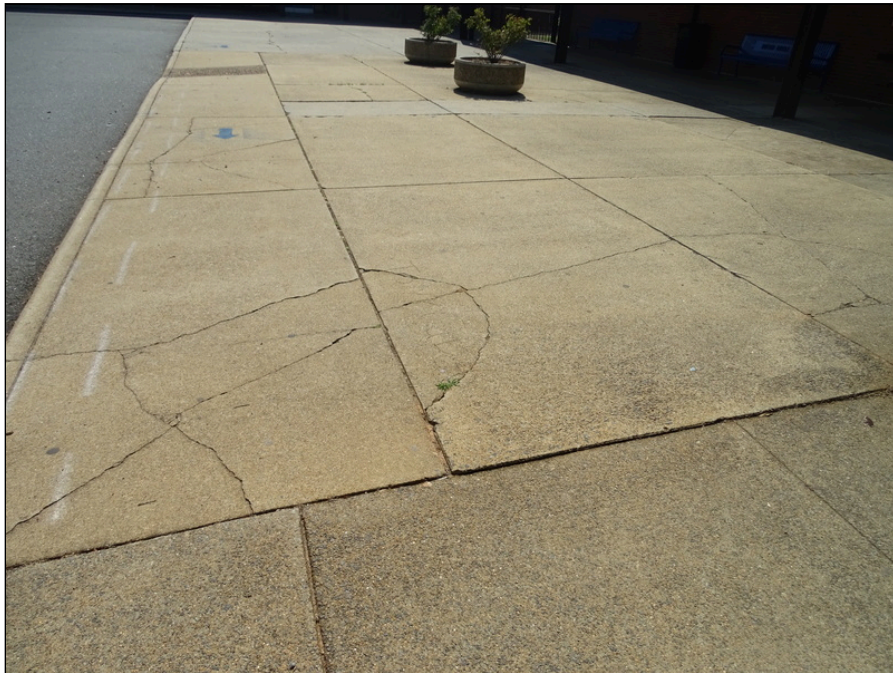
8 - Concrete sidewalk west side of Building B - note cracking
