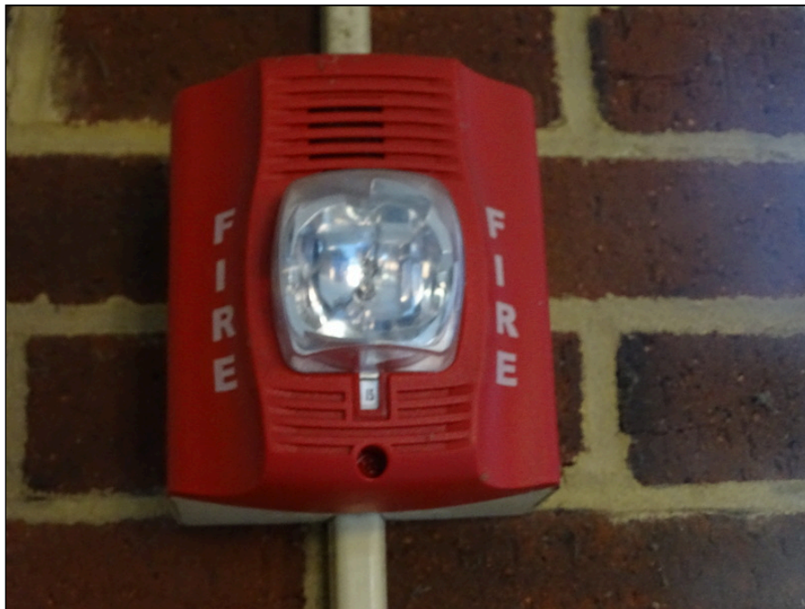
66 - Typical fire alarm bell, strobe
