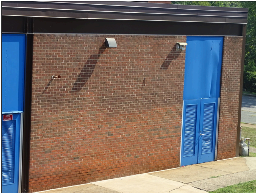
18 - Building exterior - note efflorescence
