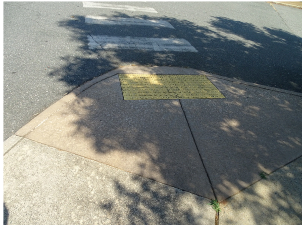
Accessible curb cut ramp with truncated domes
