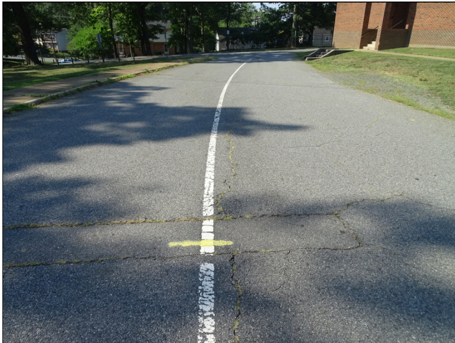
6 - Asphalt pavements east side of the site drive lane - note cracking and previous repair
