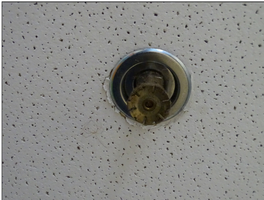
62 - Typical fire sprinkler head
